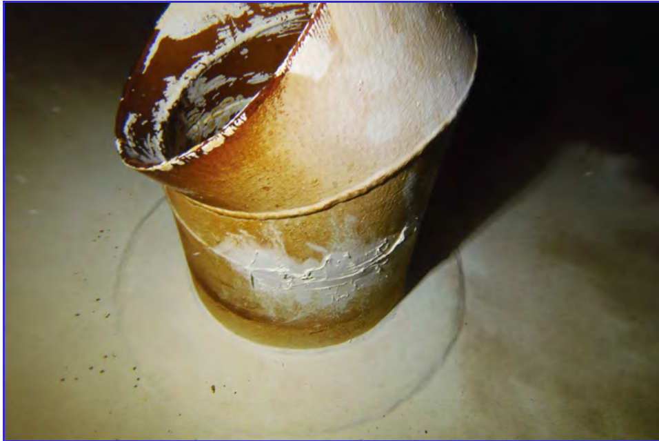
INTERIOR - CPUD - Railroad Flat Reservoir - Maintenance Inspection -104
