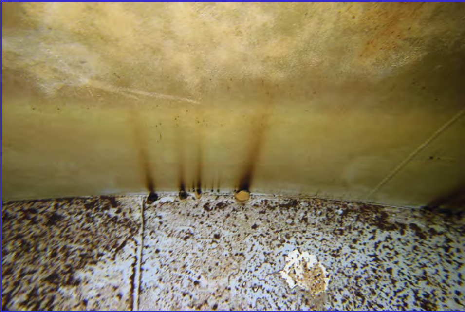
INTERIOR - CPUD - Mokelumne Hill Reservoir - Maintenance Inspection -100
