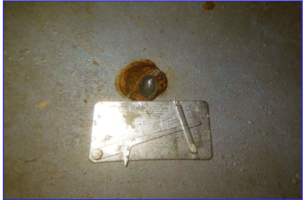
INTERIOR - CPUD - San Andaras Reservoir - Maintenance Inspection -241
