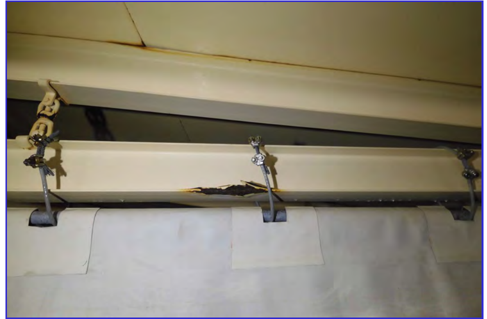
INTERIOR - CPUD - Railroad Flat Reservoir - Maintenance Inspection -029
