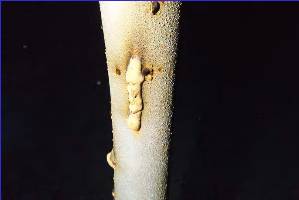
INTERIOR - CPUD - San Andaras Reservoir - Maintenance Inspection -156
