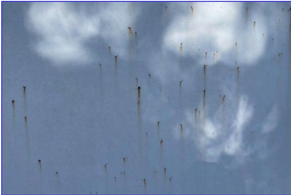
EXTERIOR - CPUD - Mokelumne Reservoir - Maintenance Inspection -098
