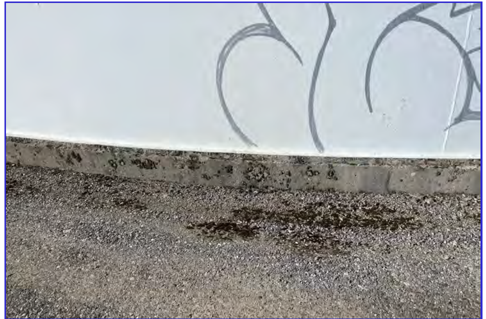
EXTERIOR - CPUD - San Andreas Reservoir - Maintenance Inspection -123
