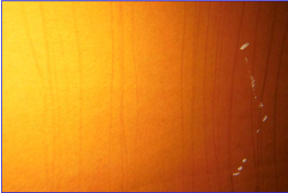
INTERIOR - CPUD - Railroad Flat Reservoir - Maintenance Inspection -092
