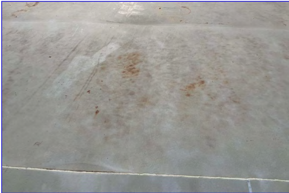
EXTERIOR - CPUD - San Andreas Reservoir - Maintenance Inspection -074
