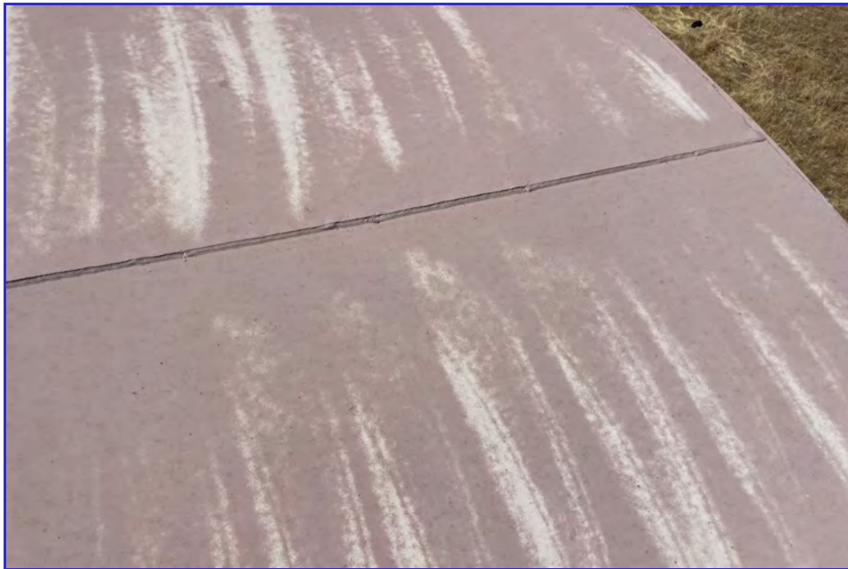
EXTERIOR - CPUD - Paloma Reservoir - Maintenance Inspection -014
