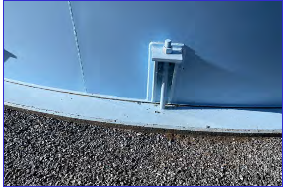
EXTERIOR - CPUD - Railroad Flat Reservoir - Maintenance Inspection -093
