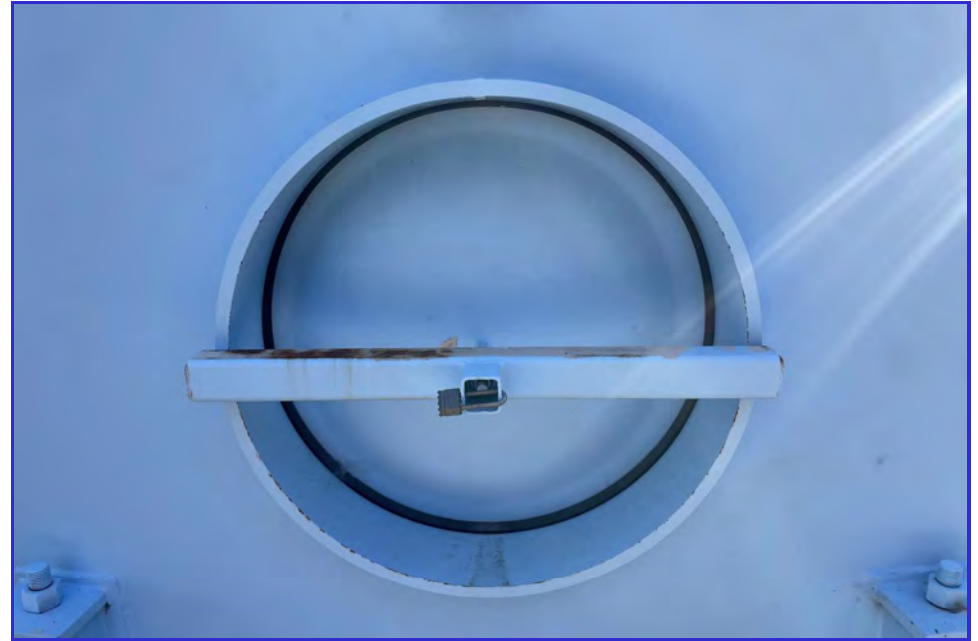
EXTERIOR - CPUD - Railroad Flat Reservoir - Maintenance Inspection -077
