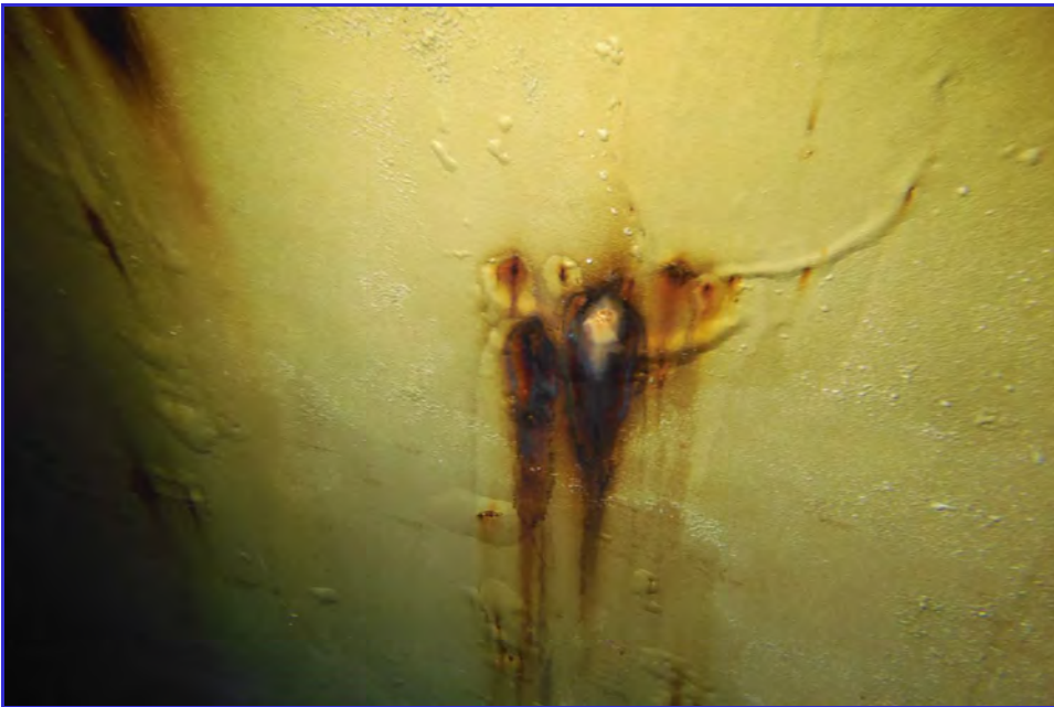
INTERIOR - CPUD - San Andaras Reservoir - Maintenance Inspection -106
