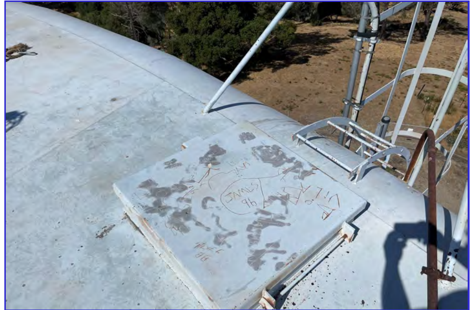
EXTERIOR - CPUD - San Andreas Reservoir - Maintenance Inspection -001
