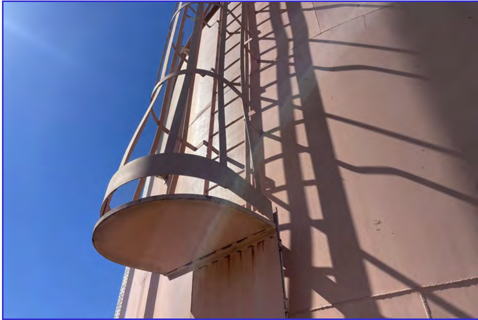
EXTERIOR - CPUD - Paloma Reservoir - Maintenance Inspection -060
