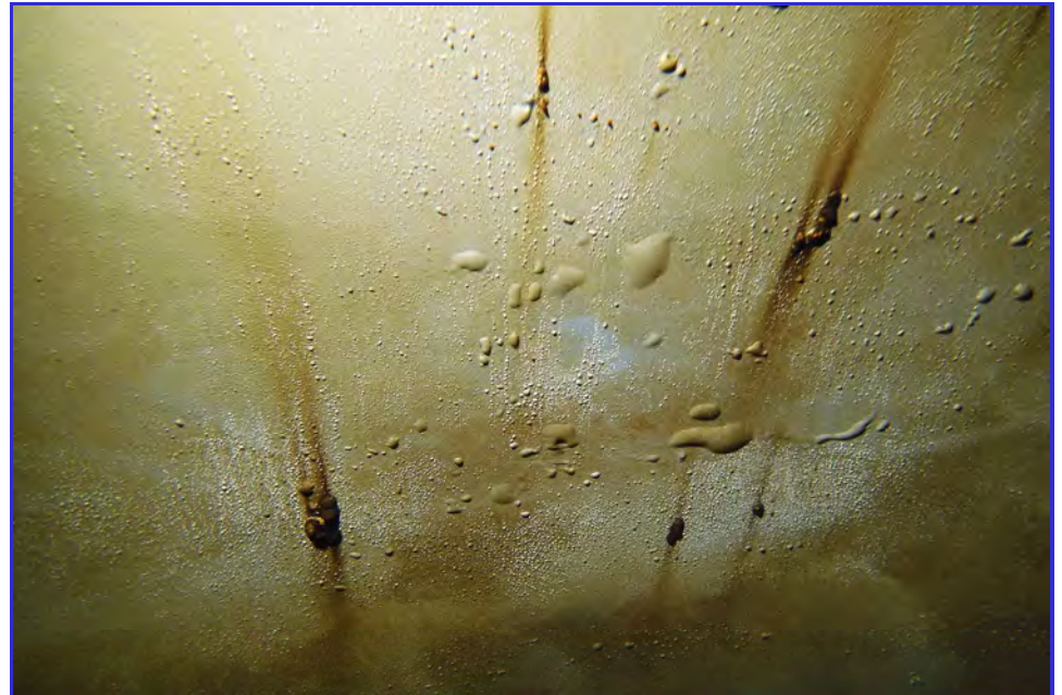
INTERIOR - CPUD - San Andaras Reservoir - Maintenance Inspection -169
