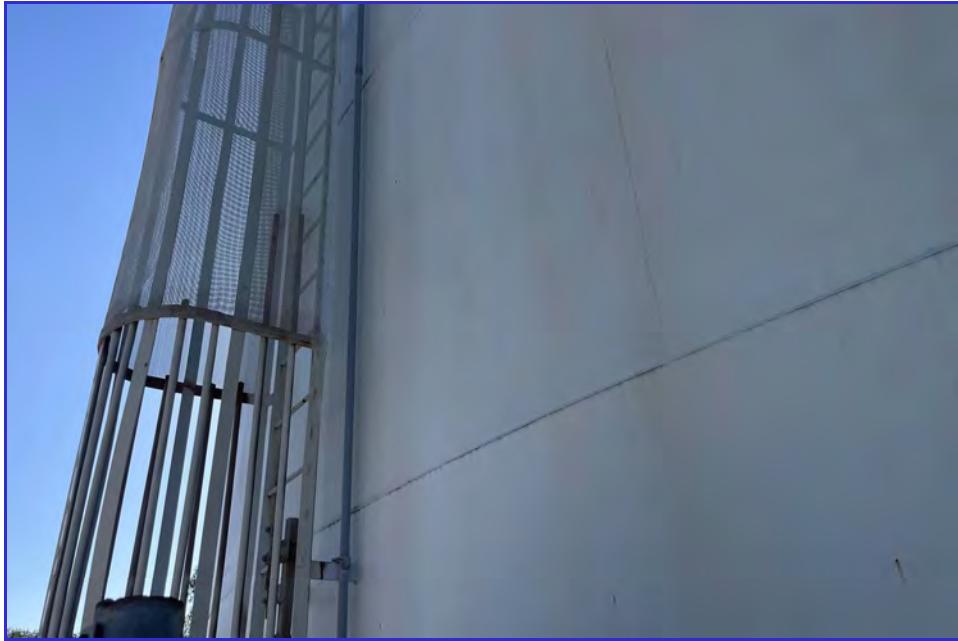
EXTERIOR - CPUD - Mokelumne Reservoir - Maintenance Inspection -136
