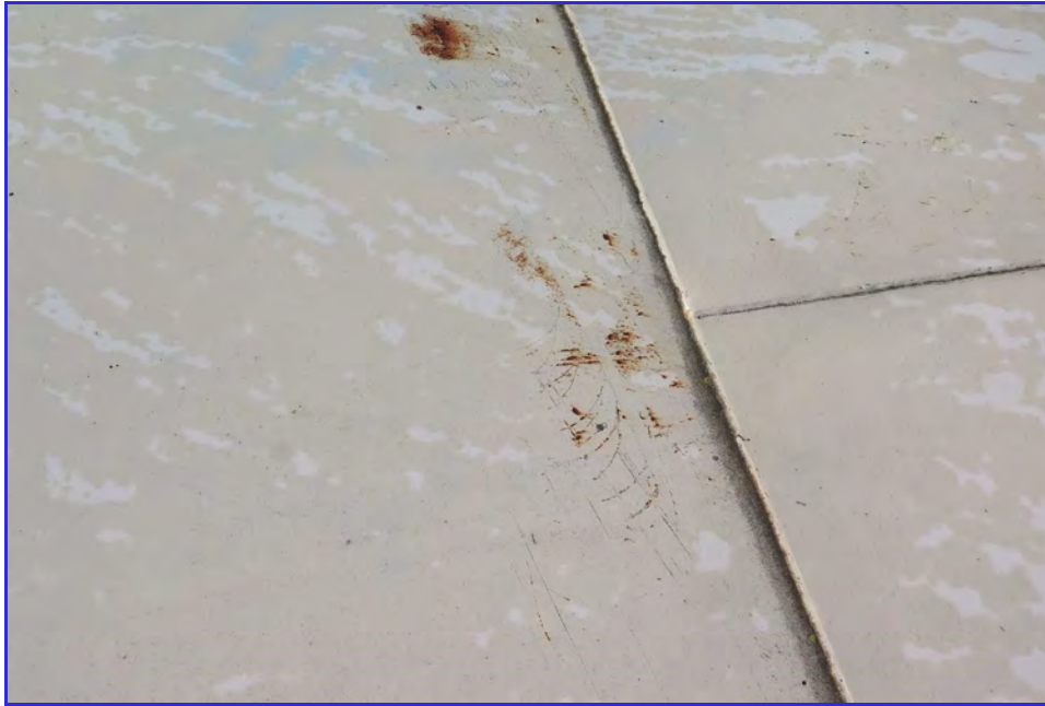
EXTERIOR - Calaveras Public Utility District - Clear Well Tank - Maintenance Inspection -016
