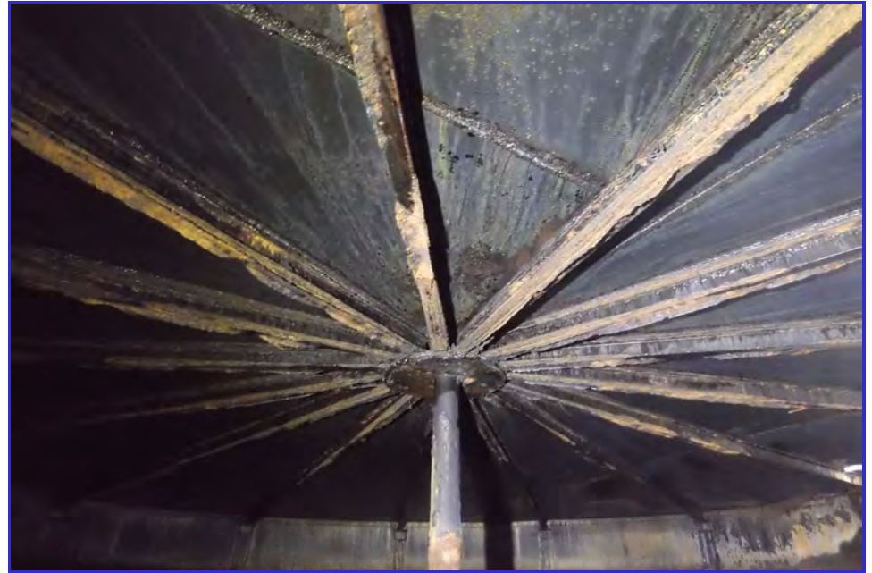
INTERIOR - CPUD - Paloma Reservoir - Maintenance Inspection -013
