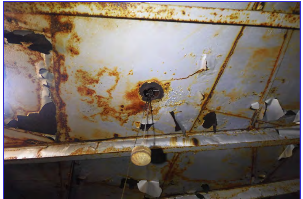
INTERIOR - CPUD - San Andaras Reservoir - Maintenance Inspection -007
