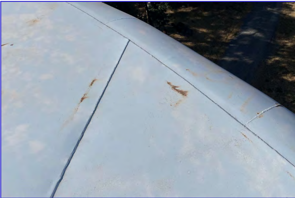
EXTERIOR - CPUD - Mokelumne Reservoir - Maintenance Inspection -070
