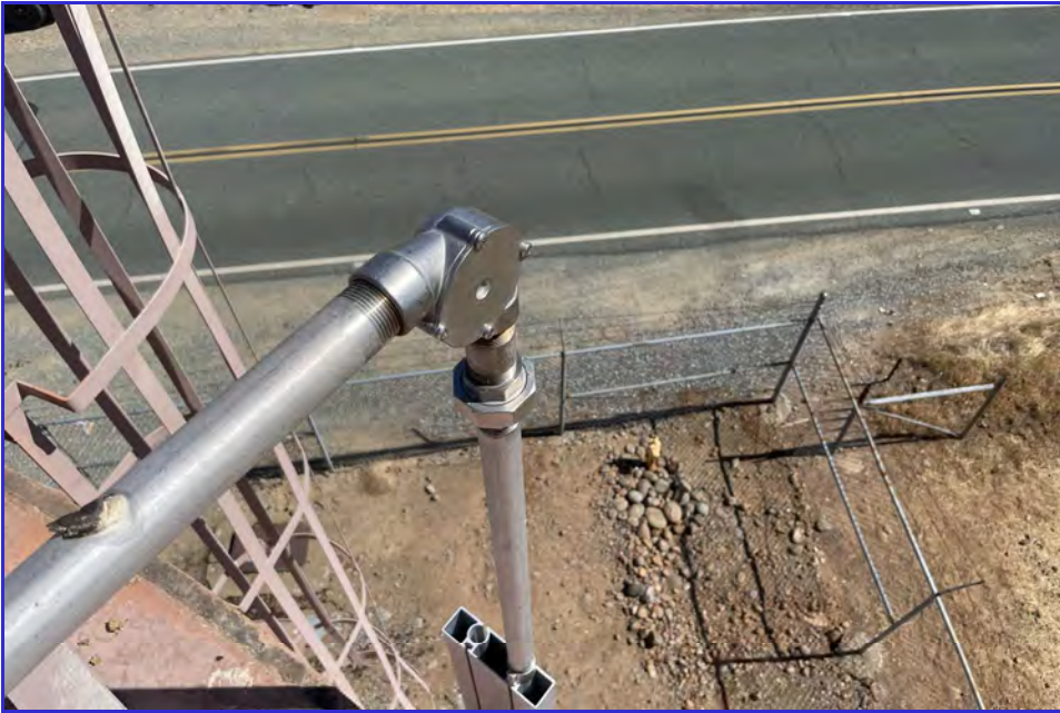
EXTERIOR - CPUD - Paloma Reservoir - Maintenance Inspection -004
