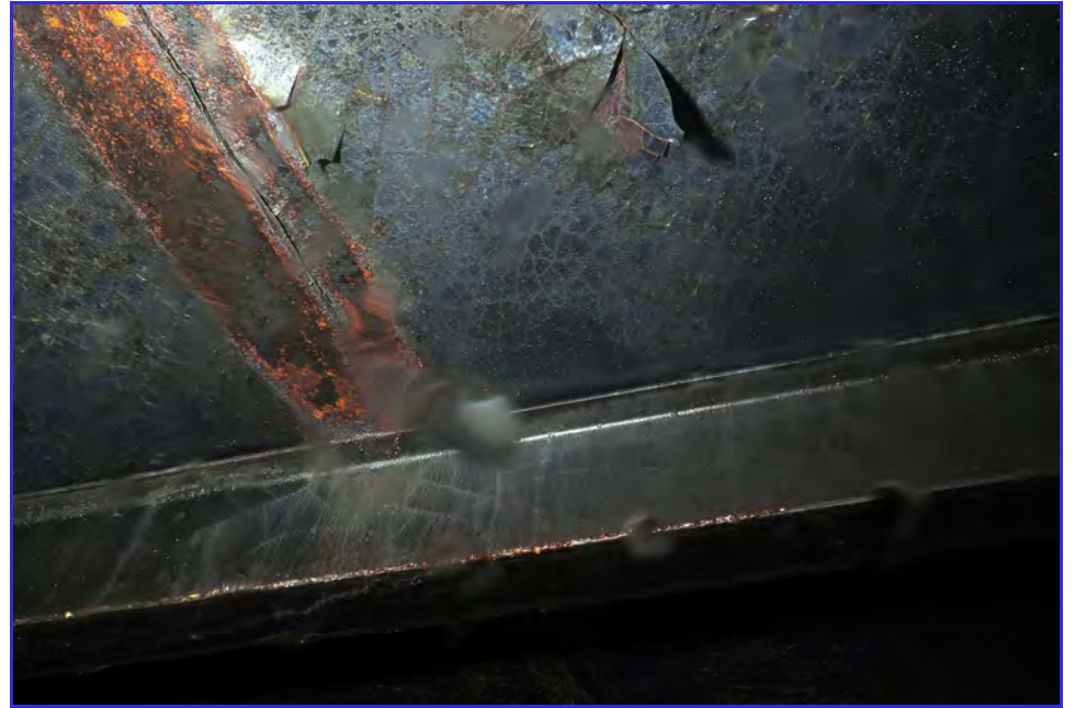
INTERIOR - Calaveras Public Utility District - Clear Well Tank - Maintenance Inspection -005
