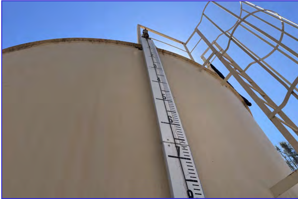
EXTERIOR - CPUD - Golden Hills - Maintenance Inspection -060
