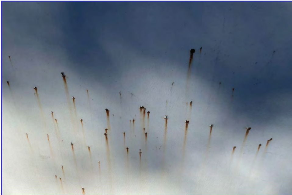
EXTERIOR - CPUD - Mokelumne Reservoir - Maintenance Inspection -092
