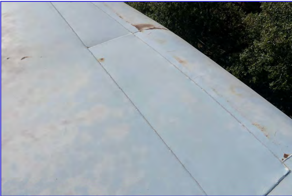
EXTERIOR - CPUD - Mokelumne Reservoir - Maintenance Inspection -066
