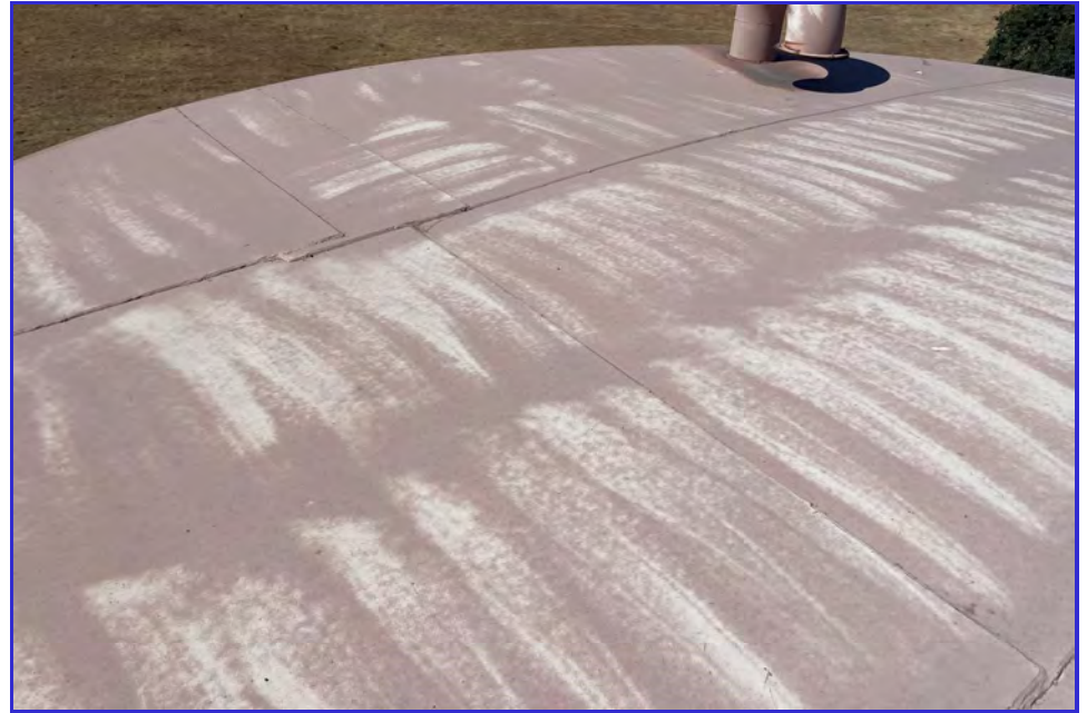
EXTERIOR - CPUD - Paloma Reservoir - Maintenance Inspection -009
