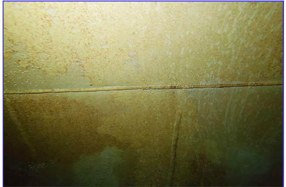
INTERIOR - CPUD - San Anderas Reservoir - Maintenance Inspection -125
