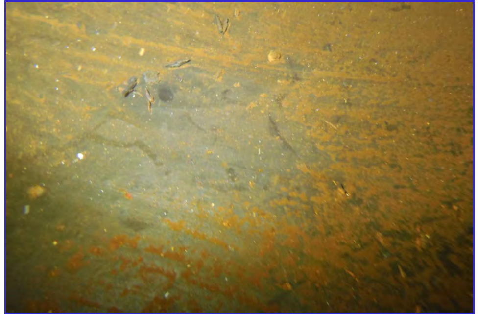
INTERIOR - CPUD - Paloma Reservoir - Maintenance Inspection -129
