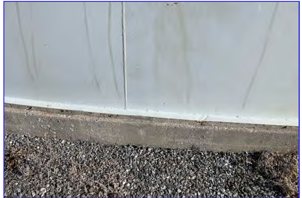
EXTERIOR - CPUD - San Andreas Reservoir - Maintenance Inspection -183
