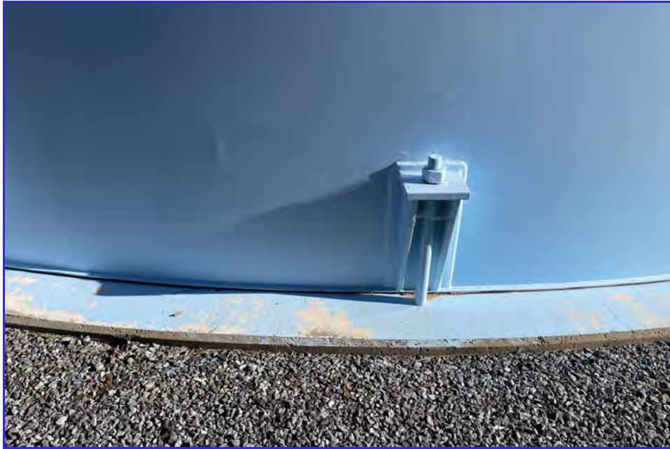
EXTERIOR - CPUD - Railroad Flat Reservoir - Maintenance Inspection -084
