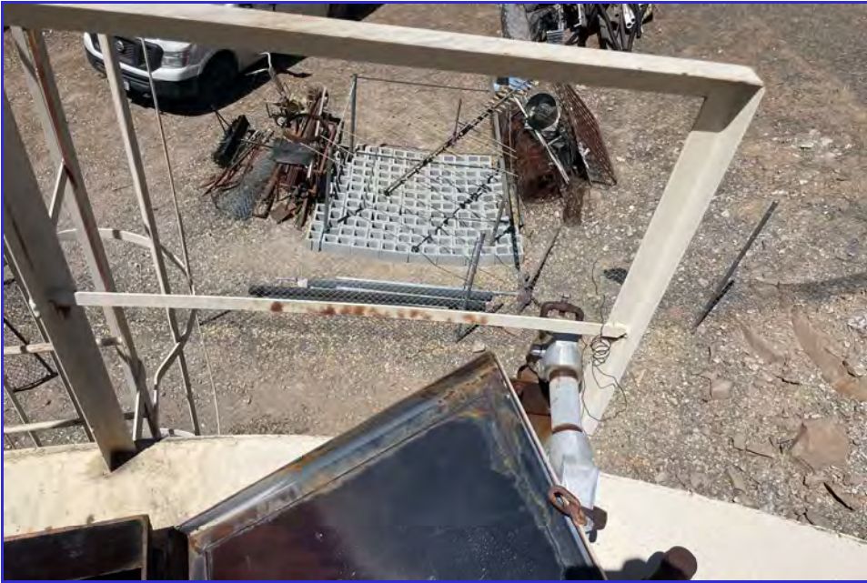
EXTERIOR - CPUD - Golden Hills - Maintenance Inspection -020
