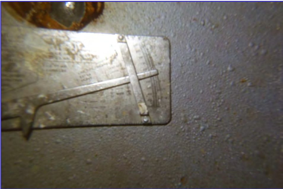
INTERIOR - CPUD - San Andaras Reservoir - Maintenance Inspection -242
