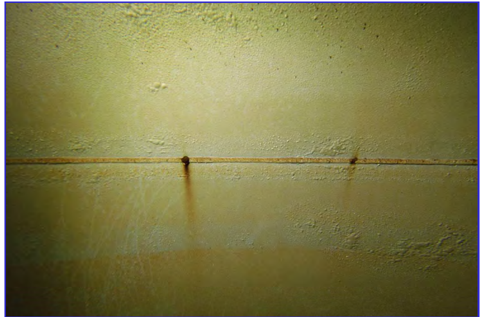
INTERIOR - CPUD - San Andaras Reservoir - Maintenance Inspection -115
