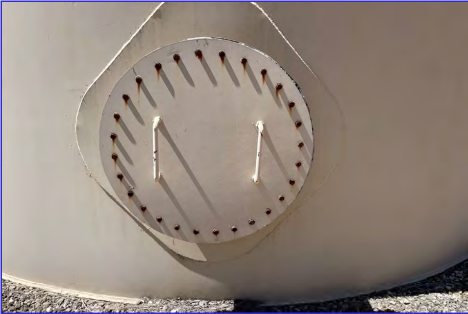
EXTERIOR - CPUD - Golden Hills - Maintenance Inspection -048
