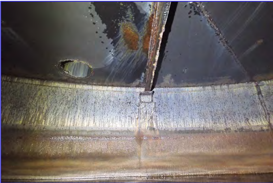
INTERIOR - CPUD - Paloma Reservoir - Maintenance Inspection -022
