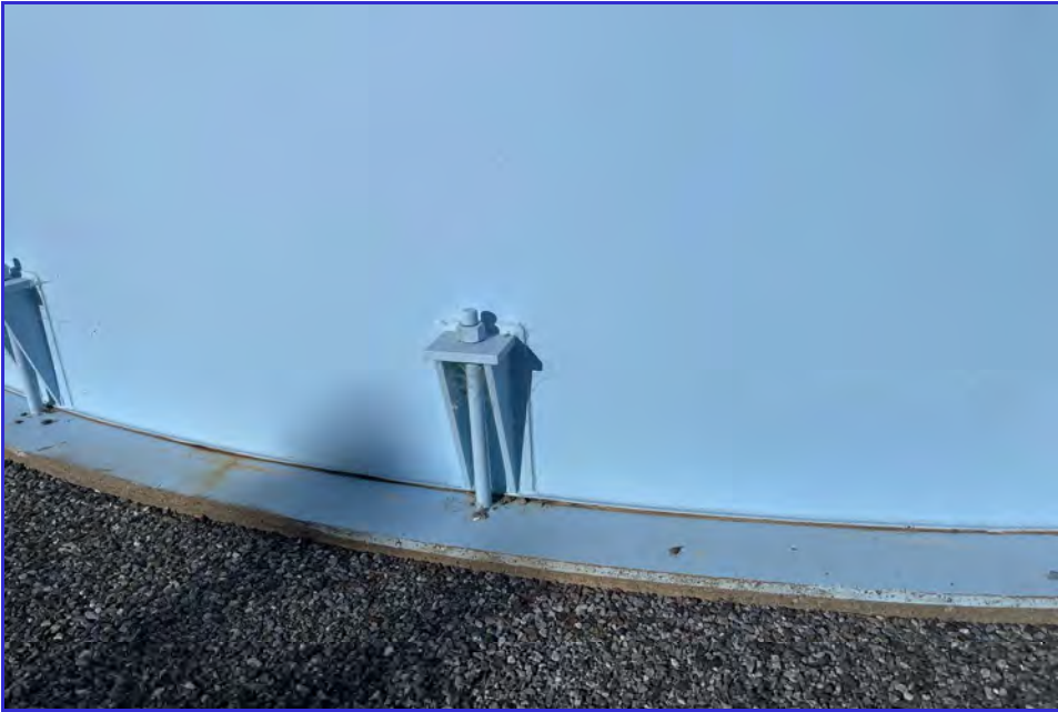
EXTERIOR - CPUD - Railroad Flat Reservoir - Maintenance Inspection -088
