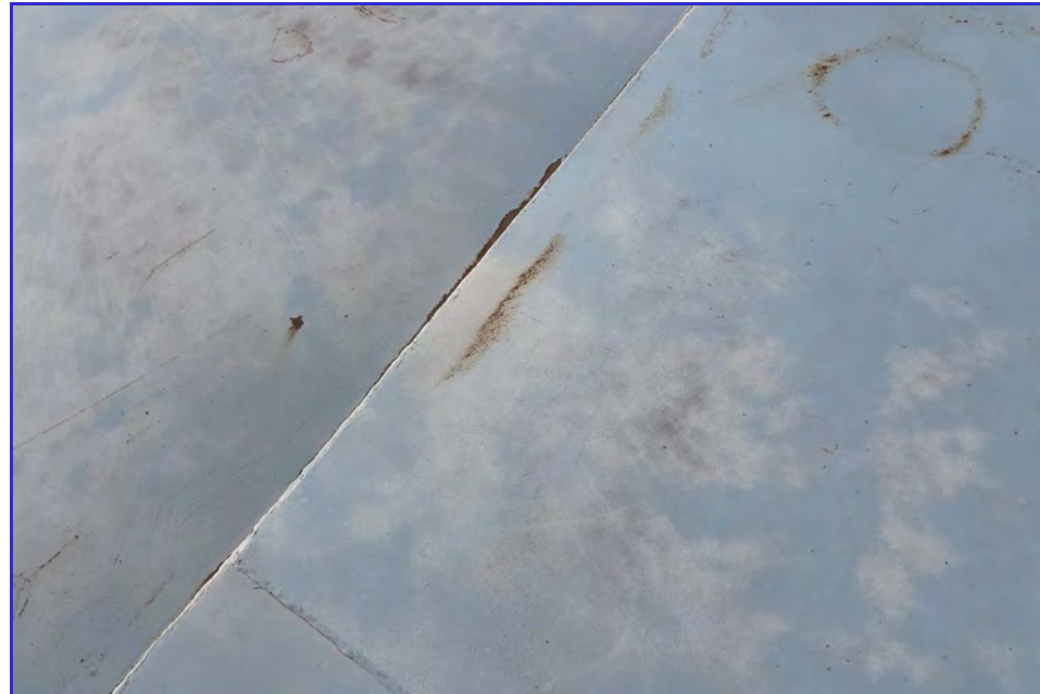
EXTERIOR - CPUD - Mokelumne Reservoir - Maintenance Inspection -009
