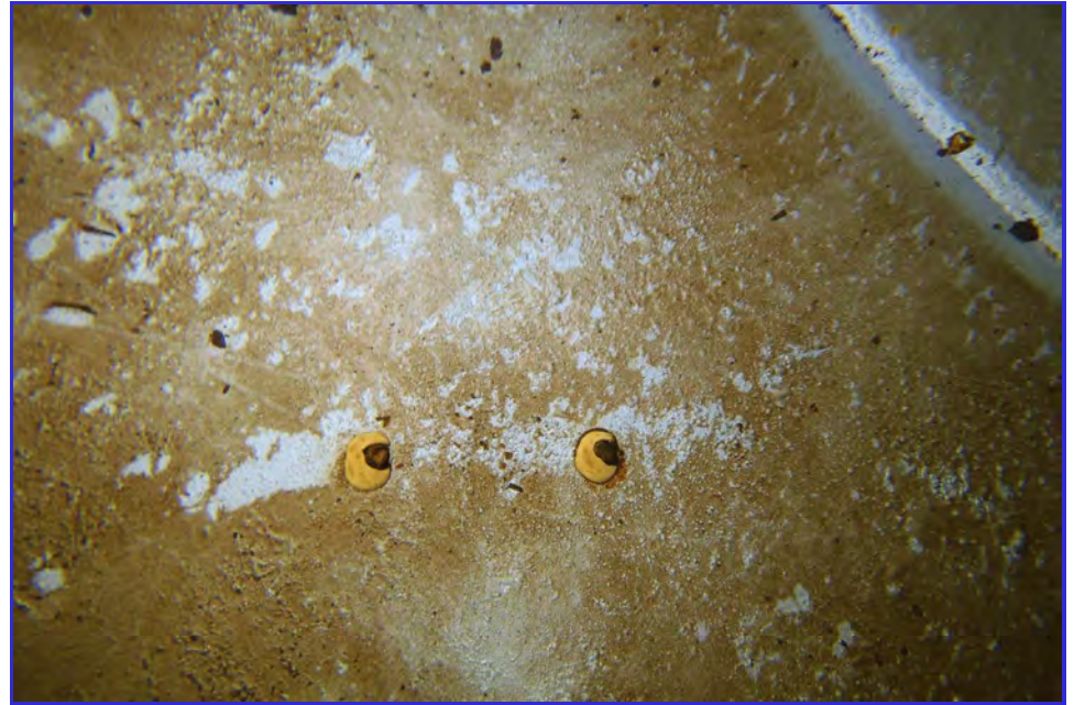
INTERIOR - CPUD - San Andaras Reservoir - Maintenance Inspection -189
