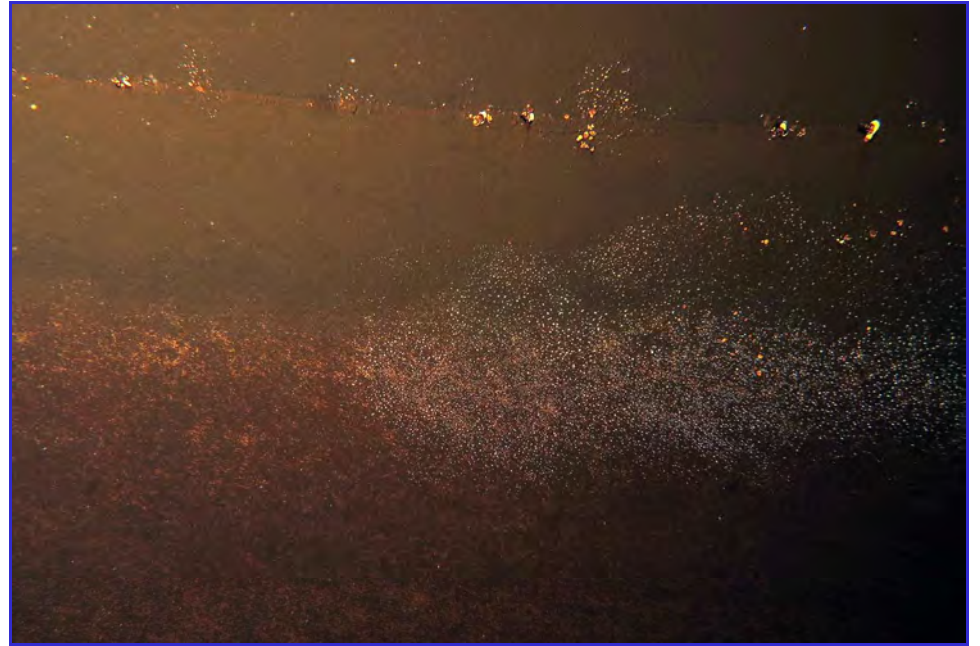
INTERIOR - Calaveras Public Utility District - Clear Well Tank - Maintenance Inspection -089
