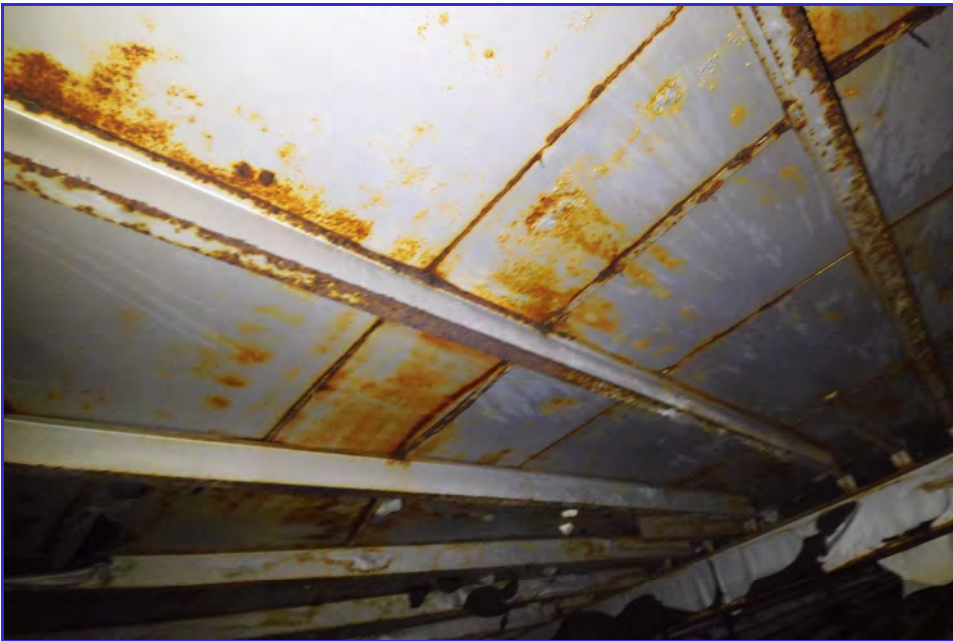
INTERIOR - CPUD - San Andreas Reservoir - Maintenance Inspection -046
