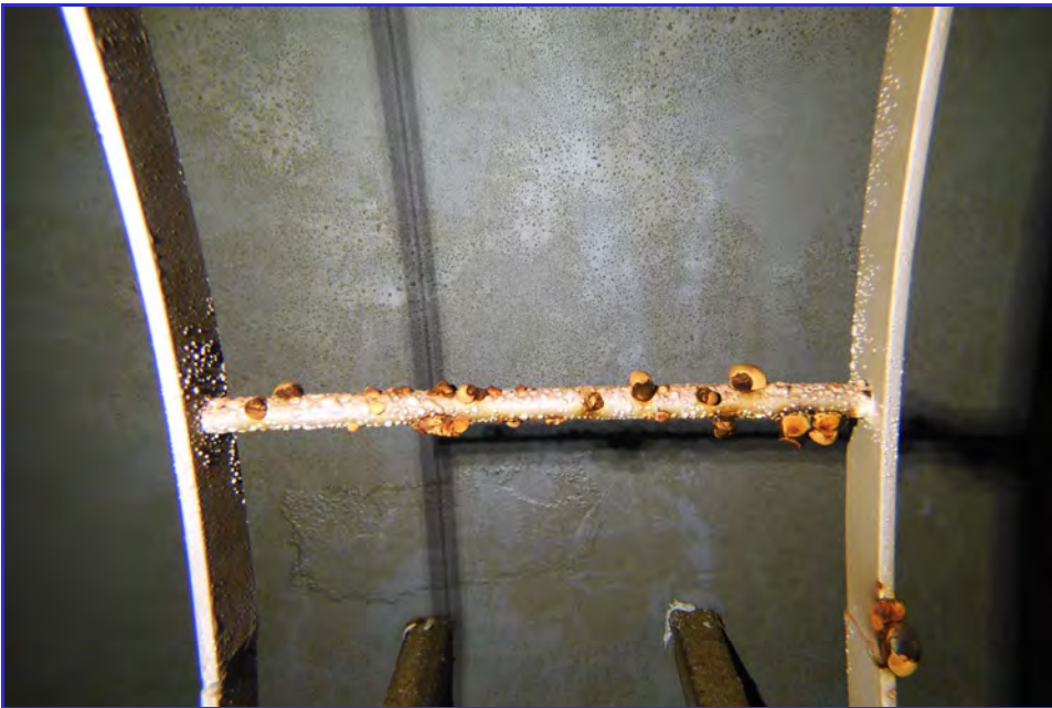
INTERIOR - CPUD - San Anderas Reservoir - Maintenance Inspection -166
