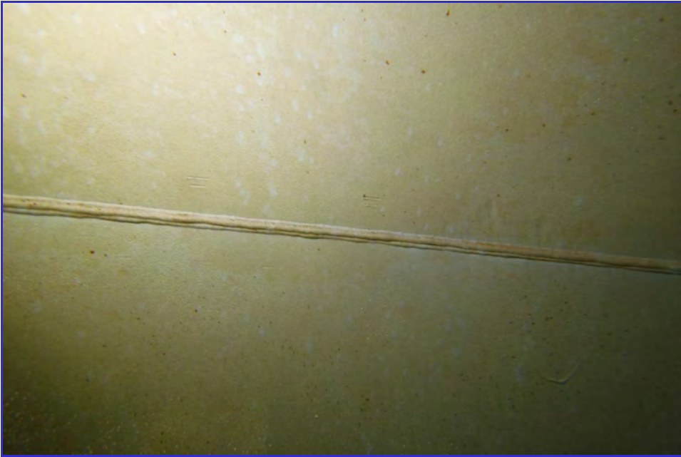
INTERIOR - CPUD - Mokelumne Hill Reservoir - Maintenance Inspection -104
