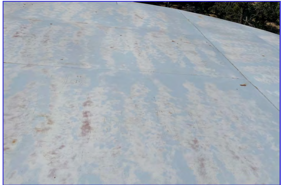
EXTERIOR - CPUD - Mokelumne Reservoir - Maintenance Inspection -031
