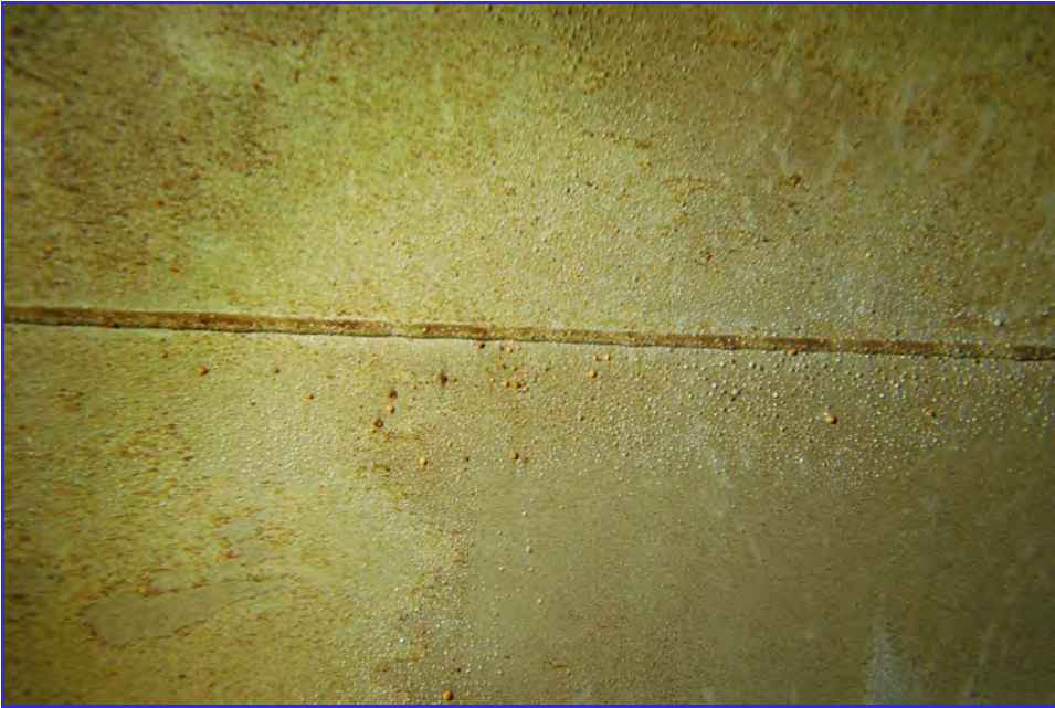
INTERIOR - CPUD - San Andaras Reservoir - Maintenance Inspection -128
