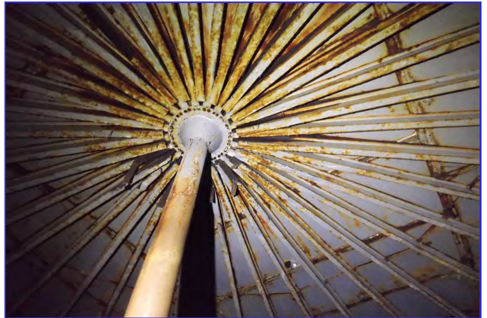
INTERIOR - CPUD - Mokelumne Hill Reservoir - Maintenance Inspection -051
