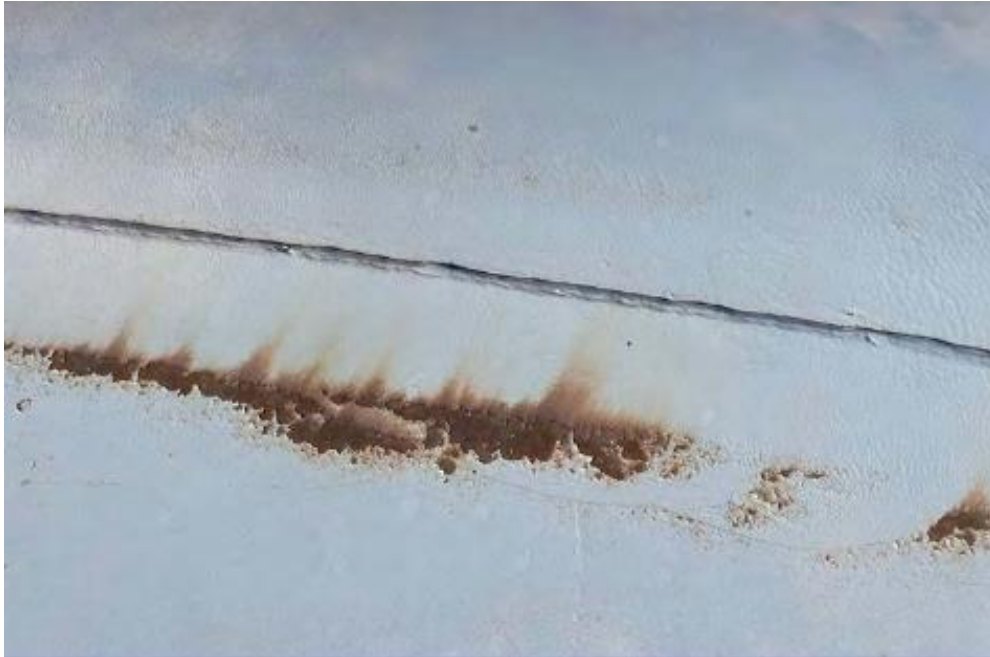
Figure 9-5. Example of Mokelumne Hill Tank Roof
