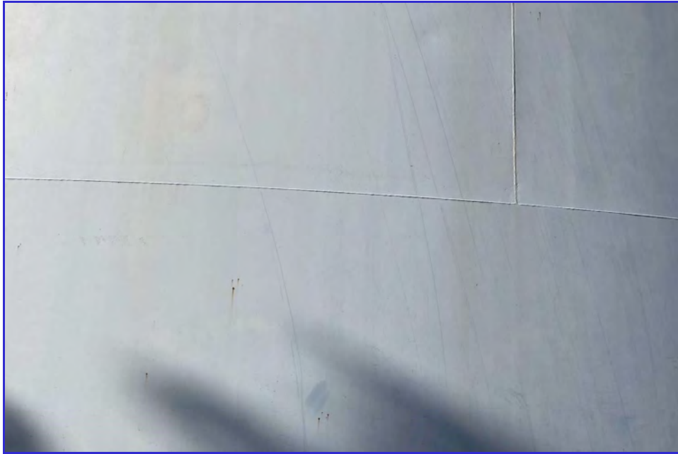
EXTERIOR - CPUD - Mokelumne Reservoir - Maintenance Inspection -084
