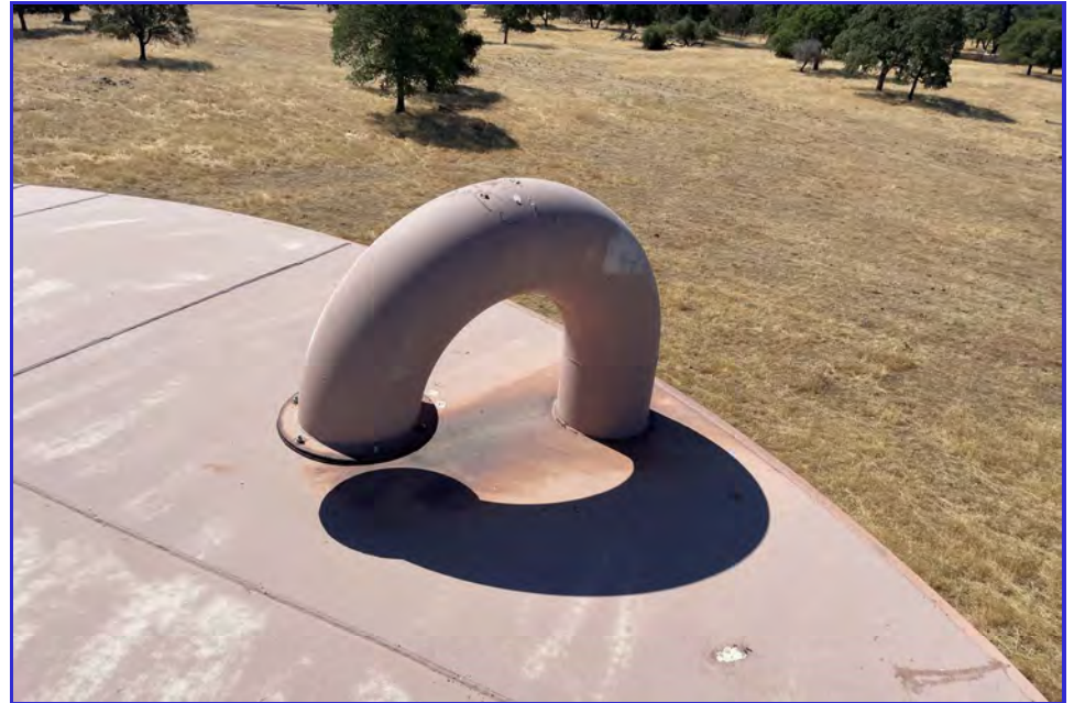
EXTERIOR - CPUD - Paloma Reservoir - Maintenance Inspection -029
