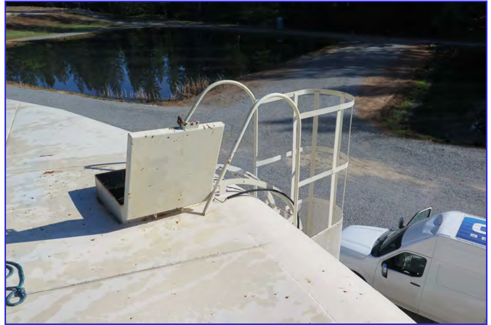
EXTERIOR - Calaveras Public Utility District - Clear Well Tank - Maintenance Inspection -041
