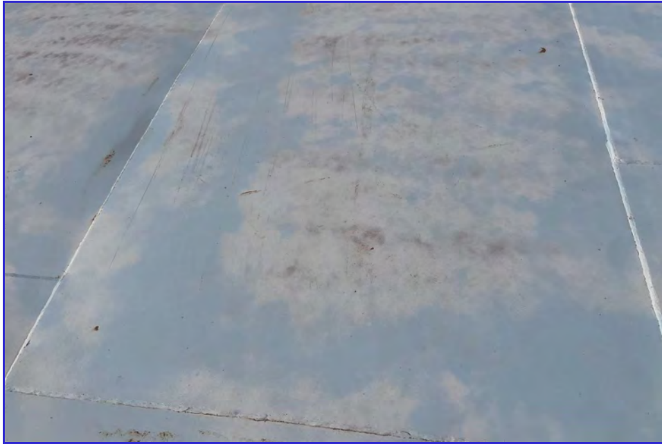
EXTERIOR - CPUD - Mokelumne Reservoir - Maintenance Inspection -012
