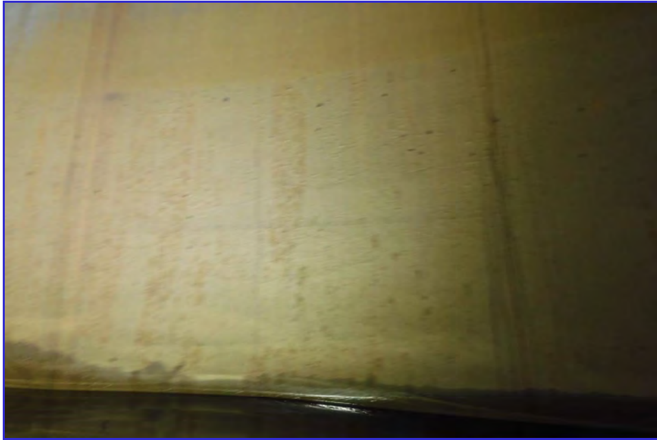
INTERIOR - CPUD - Golden Hills - Maintenance Inspection -032
