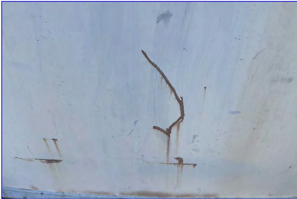
EXTERIOR - CPUD - Mokelumne Reservoir - Maintenance Inspection -130
