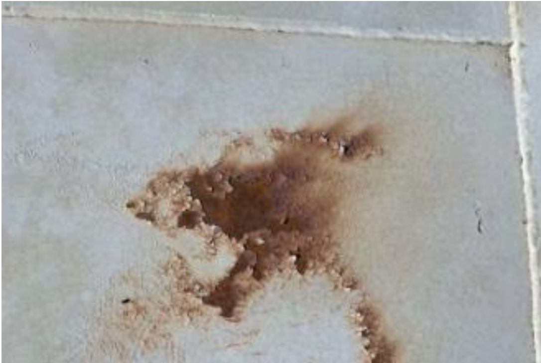
Figure 9-15. Example of San Andreas Tank Exterior Roof
