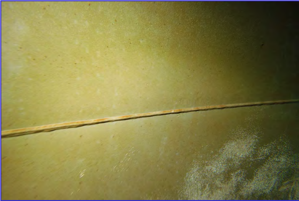
INTERIOR - CPUD - Mokelumne Hill Reservoir - Maintenance Inspection -092
