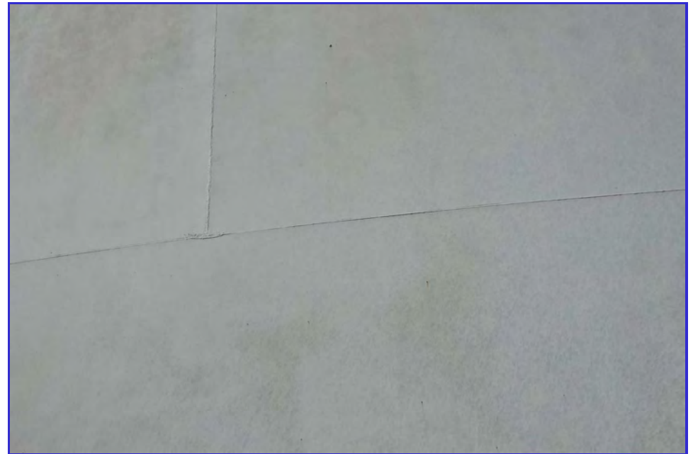
EXTERIOR - CPUD - San Andreas Reservoir - Maintenance Inspection -127
