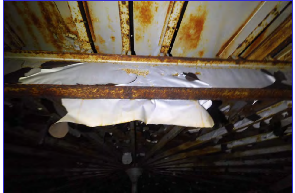
INTERIOR - CPUD - San Andaras Reservoir - Maintenance Inspection -053
