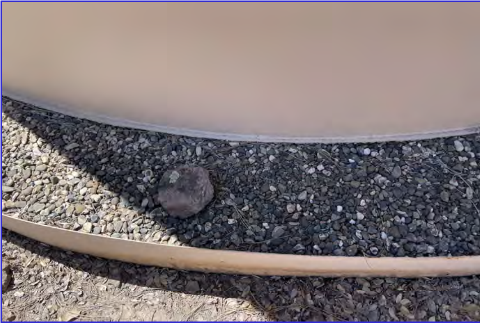
EXTERIOR - CPUD - Golden Hills - Maintenance Inspection -052
