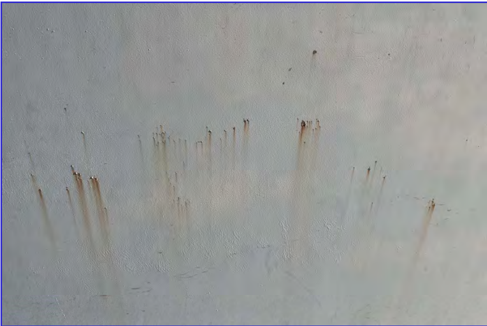
EXTERIOR - CPUD - Mokelumne Reservoir - Maintenance Inspection -106
