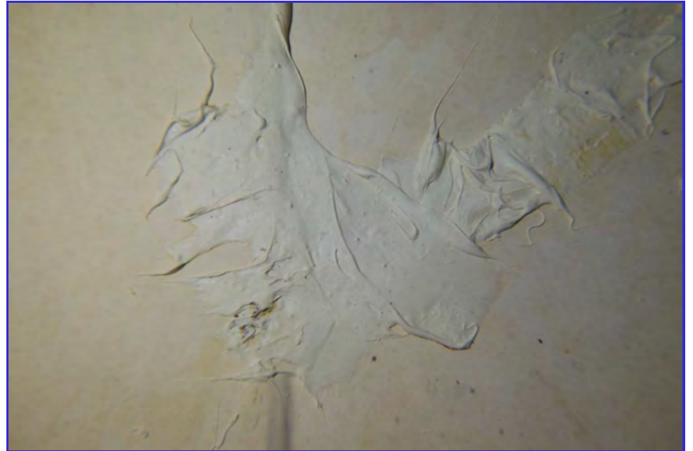
INTERIOR - CPUD - Railroad Flat Reservoir - Maintenance Inspection -157
