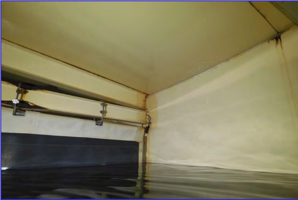
INTERIOR - CPUD - Railroad Flat Reservoir - Maintenance Inspection -052
