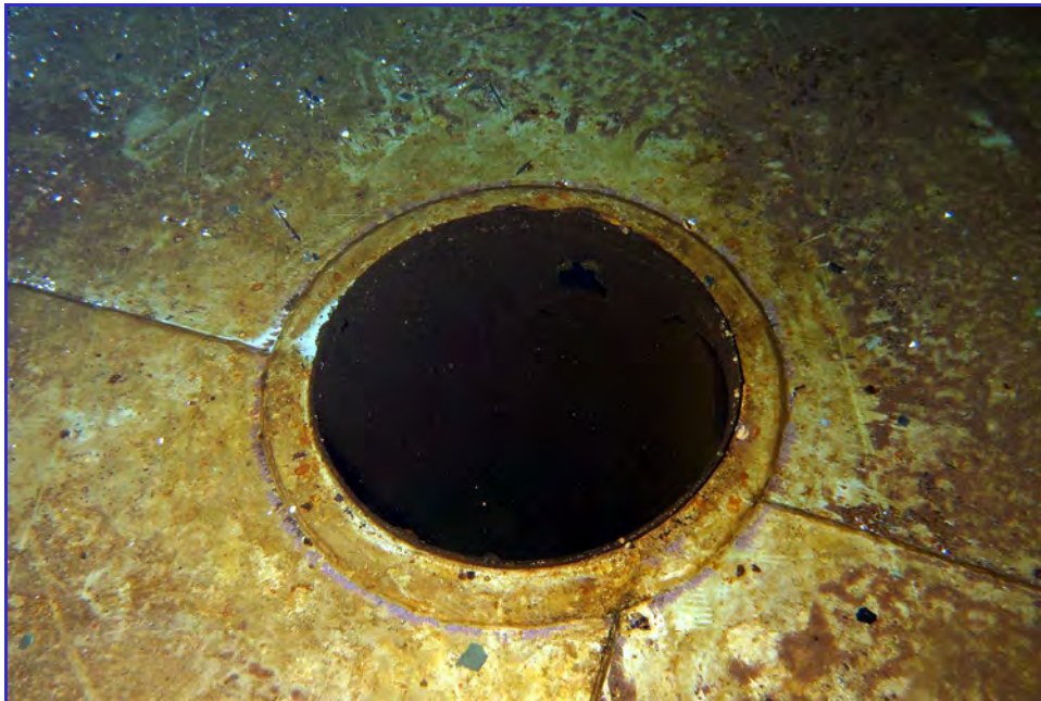
INTERIOR - Calaveras Public Utility District - Clear Well Tank - Maintenance Inspection -098
