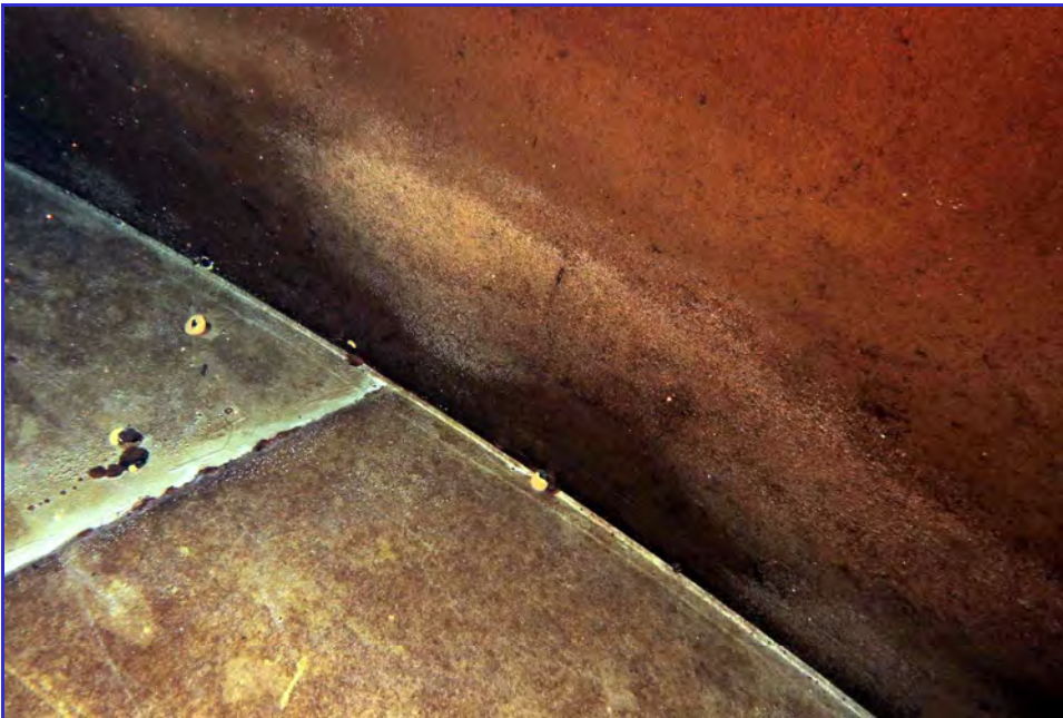
INTERIOR - Calaveras Public Utility District - Clear Well Tank - Maintenance Inspection -066
