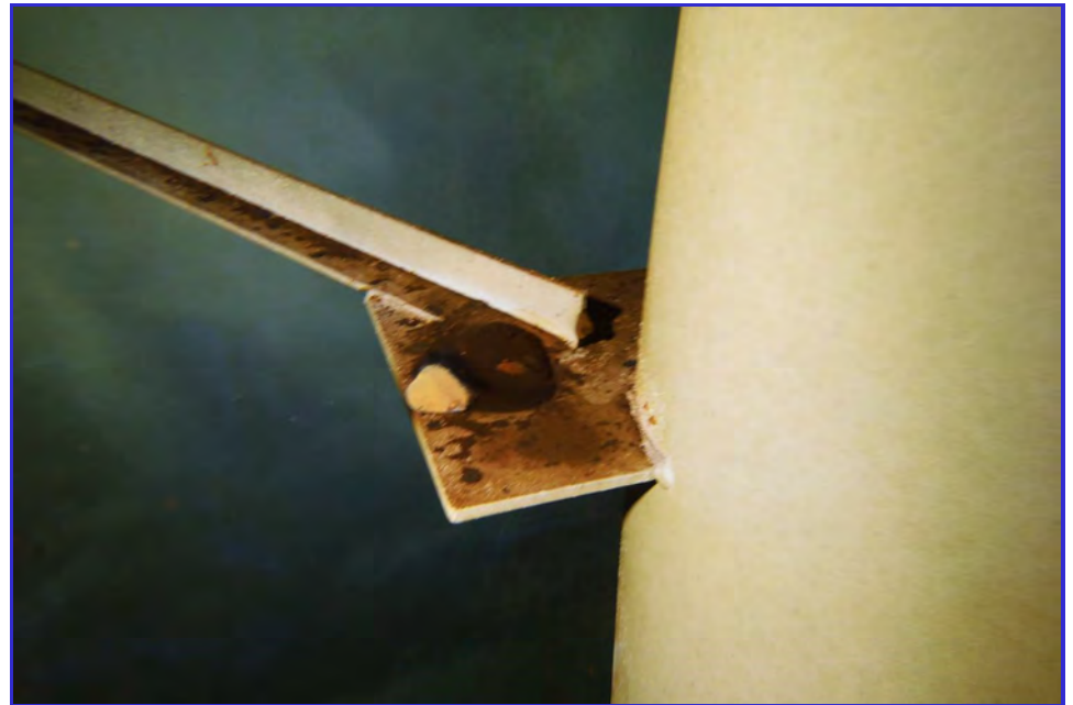
INTERIOR - CPUD - Mokelumne Hill Reservoir - Maintenance Inspection -111
