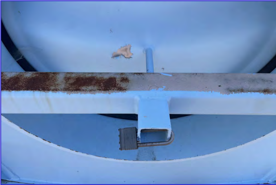
EXTERIOR - CPUD - Railroad Flat Reservoir - Maintenance Inspection -076
