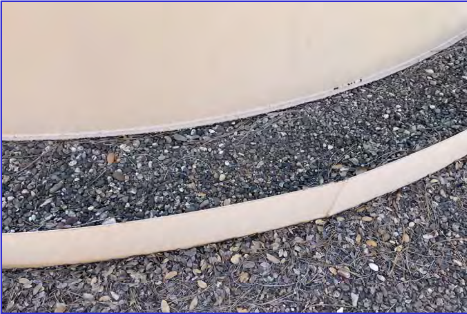
EXTERIOR - CPUD - Golden Hills - Maintenance Inspection -040
