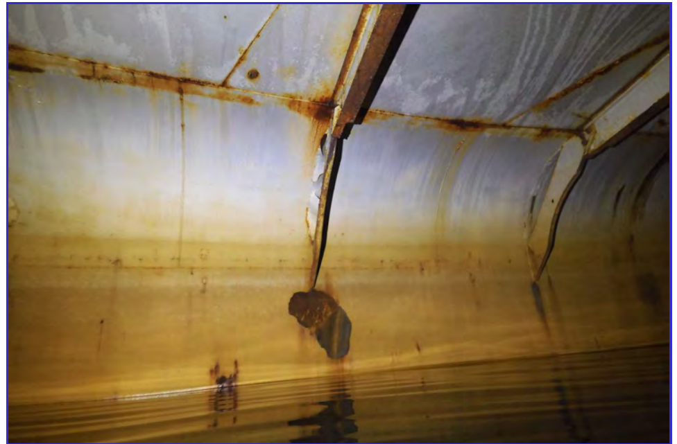
INTERIOR - CPUD - San Andaras Reservoir - Maintenance Inspection -095
