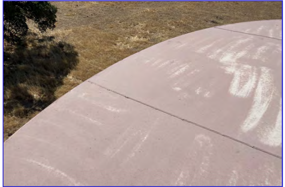
EXTERIOR - CPUD - Paloma Reservoir - Maintenance Inspection -033
