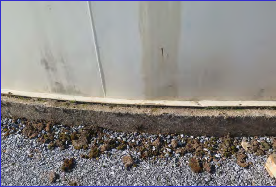
EXTERIOR - Calaveras Public Utility District - Clear Well Tank - Maintenance Inspection -116
