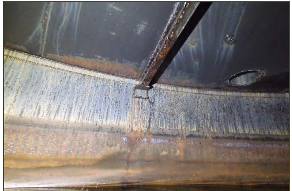
INTERIOR - CPUD - Paloma Reservoir - Maintenance Inspection -019
