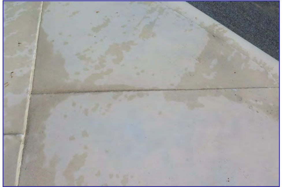
EXTERIOR - Calaveras Public Utility District - Clear Well Tank - Maintenance Inspection -005
