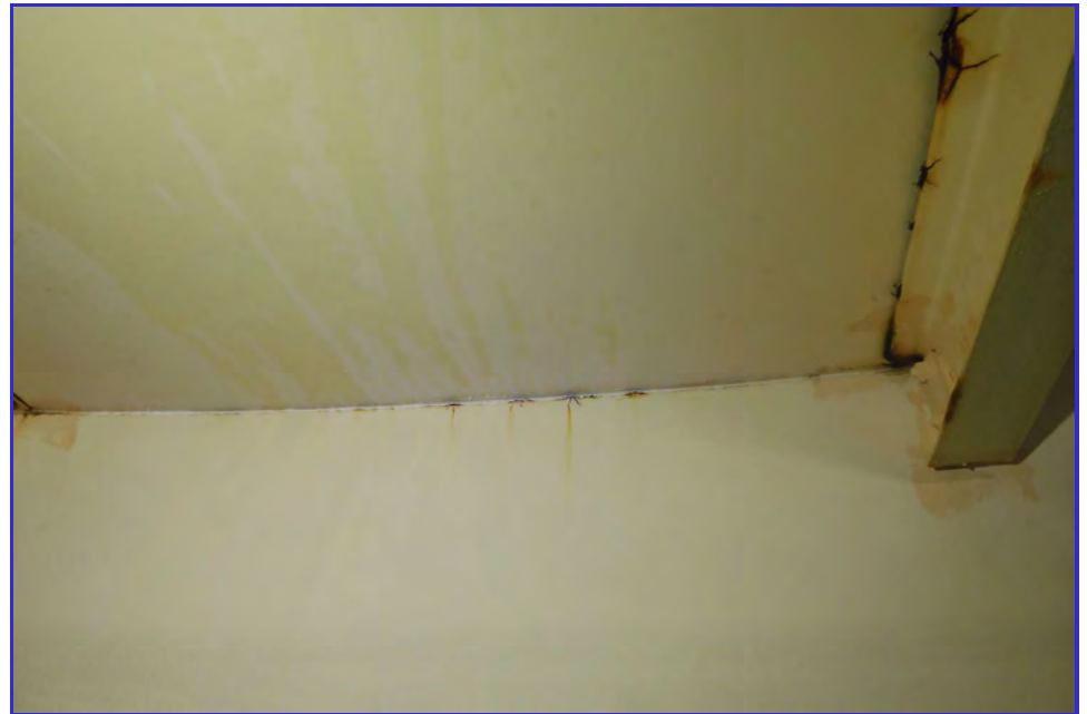
INTERIOR - CPUD - Railroad Flat Reservoir - Maintenance Inspection -063
