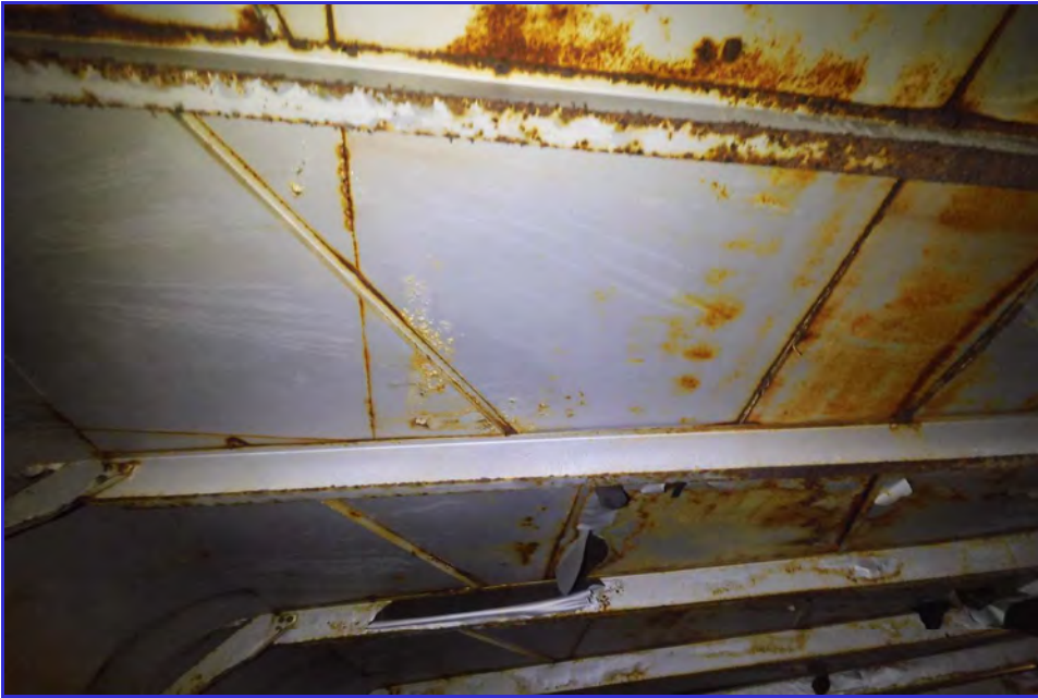
INTERIOR - CPUD - San Andreas Reservoir - Maintenance Inspection -044
