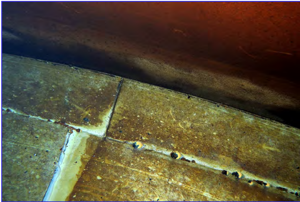
INTERIOR - Calaveras Public Utility District - Clear Well Tank - Maintenance Inspection -078
