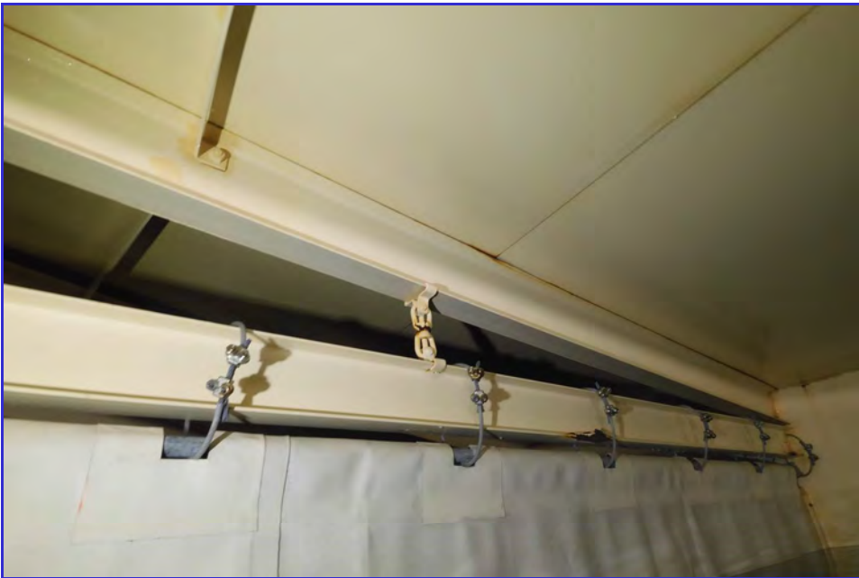
INTERIOR - CPUD - Railroad Flat Reservoir - Maintenance Inspection -030
