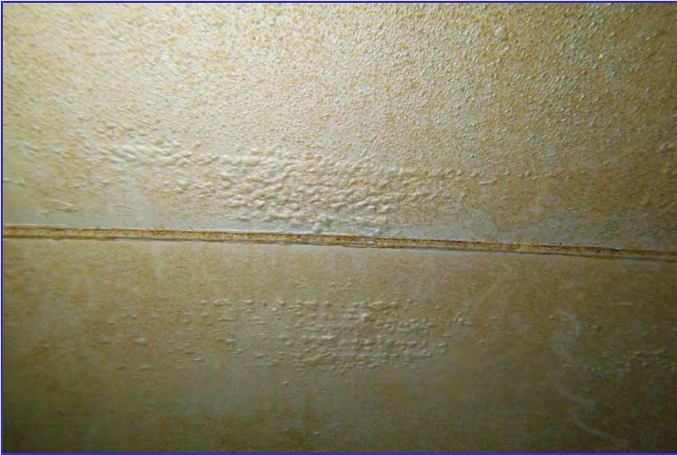
INTERIOR - CPUD - San Andaras Reservoir - Maintenance Inspection -144
