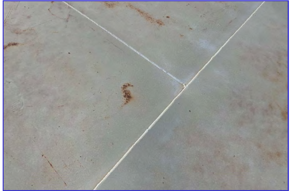
EXTERIOR - CPUD - San Andreas Reservoir - Maintenance Inspection -077
