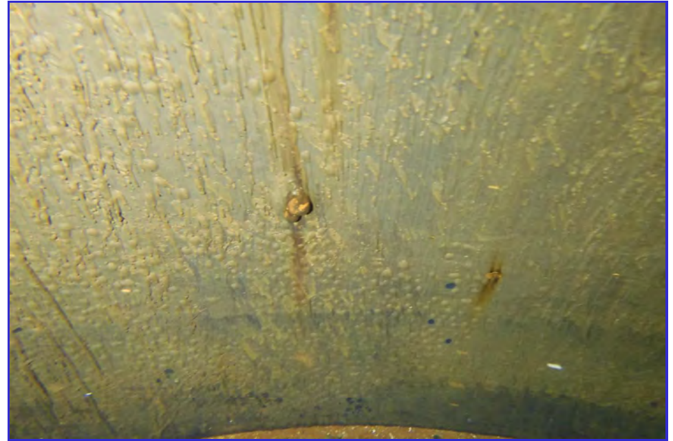
INTERIOR - CPUD - Paloma Reservoir - Maintenance Inspection -105
