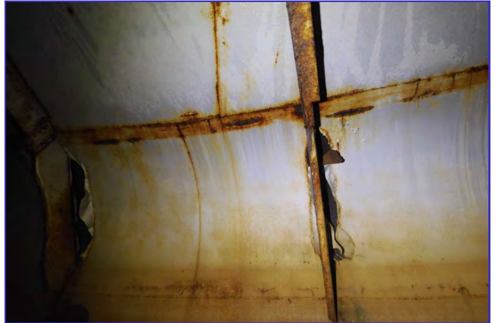
INTERIOR - CPUD - San Andaras Reservoir - Maintenance Inspection -097
