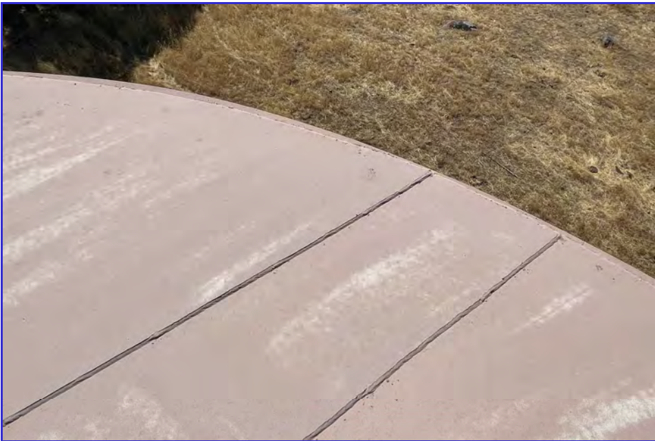
EXTERIOR - CPUD - Paloma Reservoir - Maintenance Inspection -026
