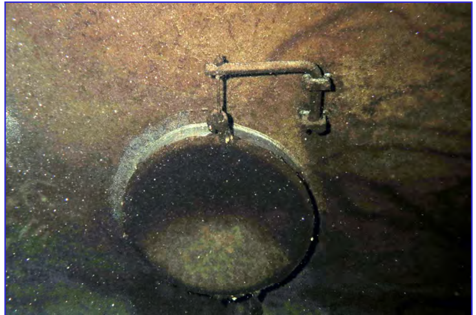
INTERIOR - Calaveras Public Utility District - Clear Well Tank - Maintenance Inspection -063
