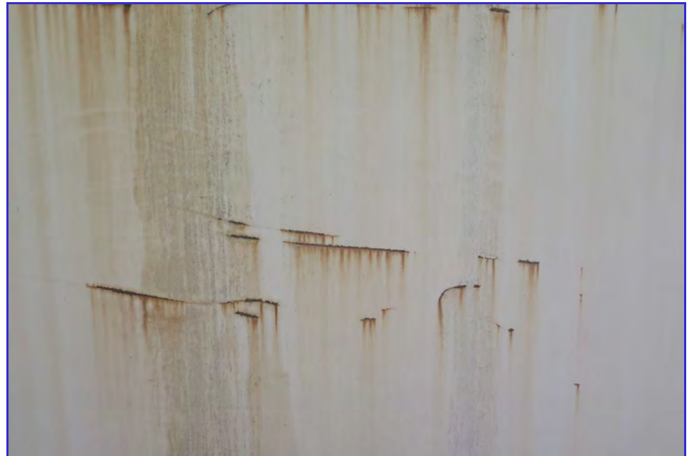
EXTERIOR - Calaveras Public Utility District - Clear Well Tank - Maintenance Inspection -091
