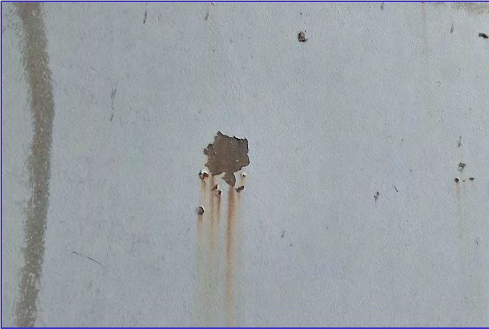
EXTERIOR - CPUD - San Andreas Reservoir - Maintenance Inspection -152
