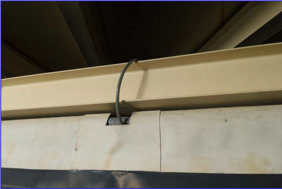
INTERIOR - CPUD - Railroad Flat Reservoir - Maintenance Inspection -020
