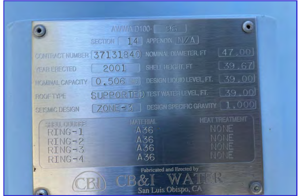
EXTERIOR - CPUD - Railroad Flat Reservoir - Maintenance Inspection -073
