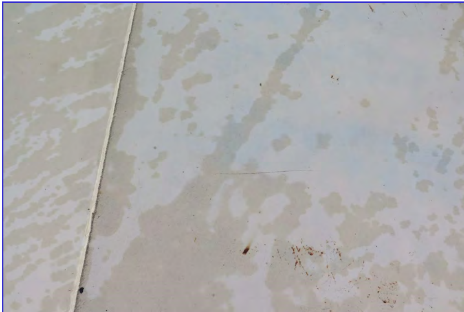
EXTERIOR - Calaveras Public Utility District - Clear Well Tank - Maintenance Inspection -006
