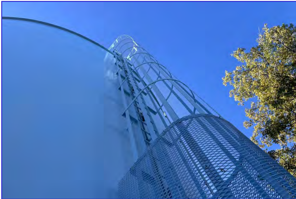
EXTERIOR - CPUD - Railroad Flat Reservoir - Maintenance Inspection -062
