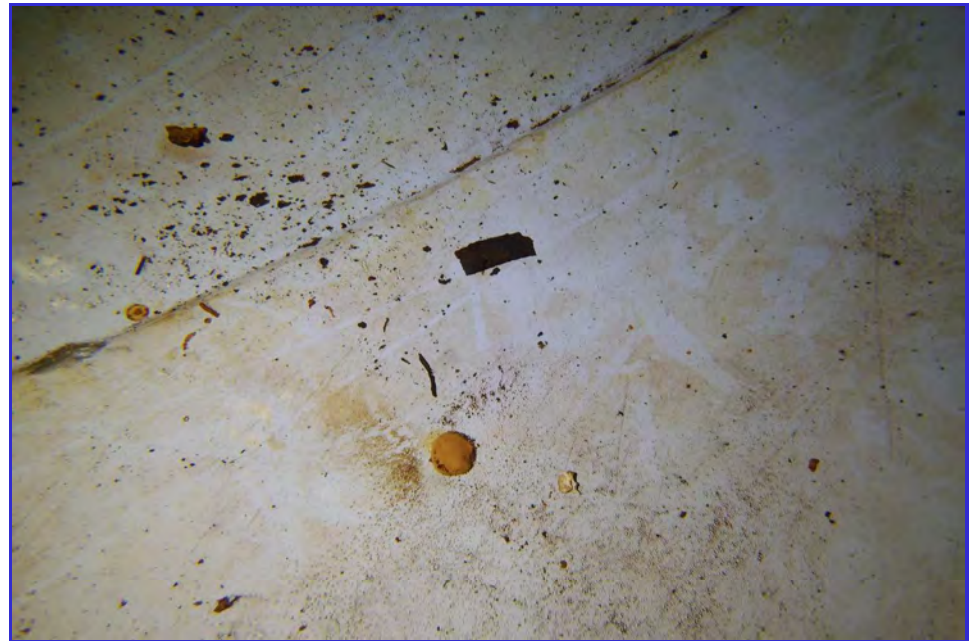
INTERIOR - CPUD - Mokelumne Hill Reservoir - Maintenance Inspection -163
