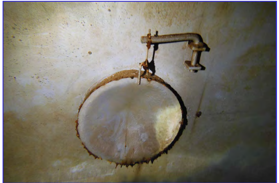
INTERIOR - CPUD - San Anderas Reservoir - Maintenance Inspection -167
