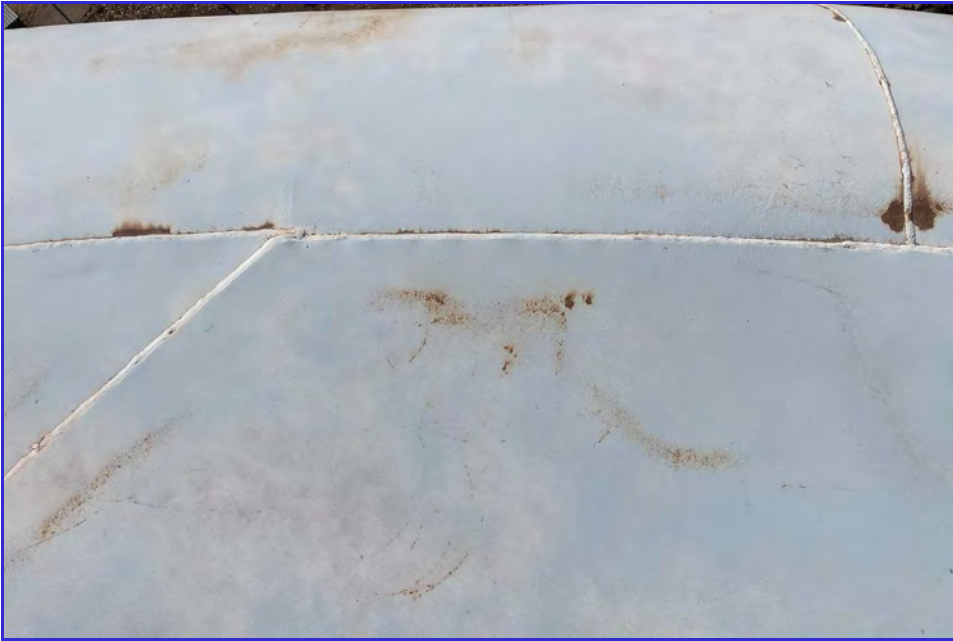
EXTERIOR - CPUD - Mokelumne Reservoir - Maintenance Inspection -044
