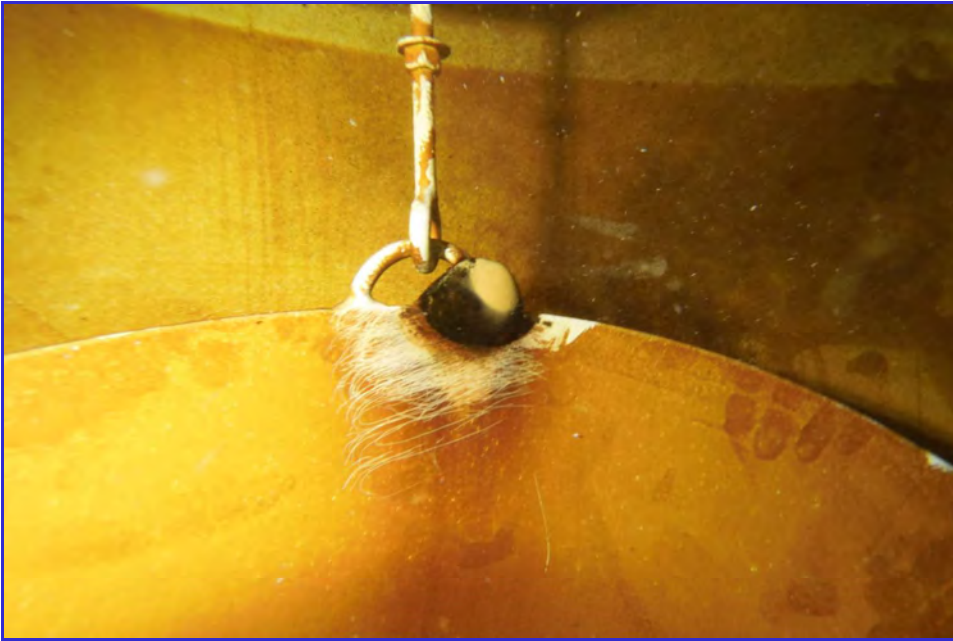
INTERIOR - CPUD - Railroad Flat Reservoir - Maintenance Inspection -124
