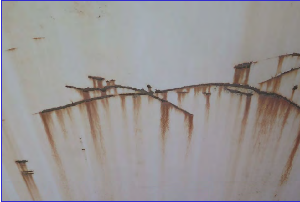
EXTERIOR - Calaveras Public Utility District - Clear Well Tank - Maintenance Inspection -108
