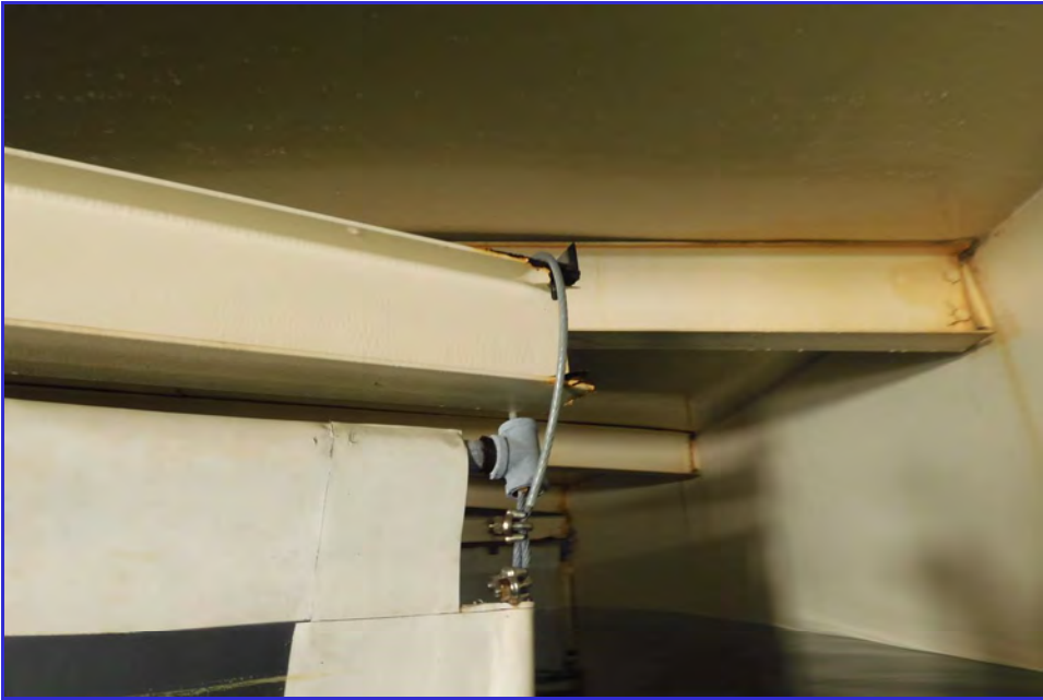
INTERIOR - CPUD - Railroad Flat Reservoir - Maintenance Inspection -024
