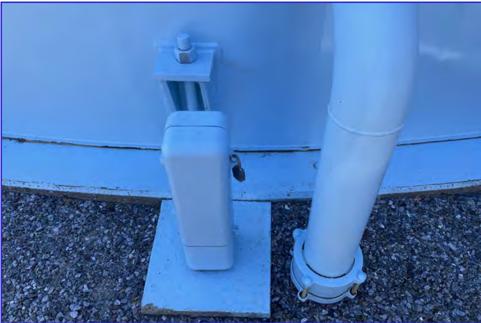
EXTERIOR - CPUD - Railroad Flat Reservoir - Maintenance Inspection -098
