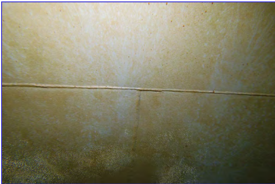
INTERIOR - CPUD - Mokelumne Hill Reservoir - Maintenance Inspection -082
