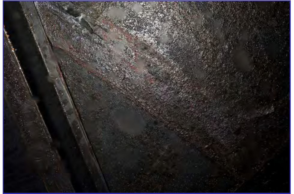
INTERIOR - Calaveras Public Utility District - Clear Well Tank - Maintenance Inspection -025
