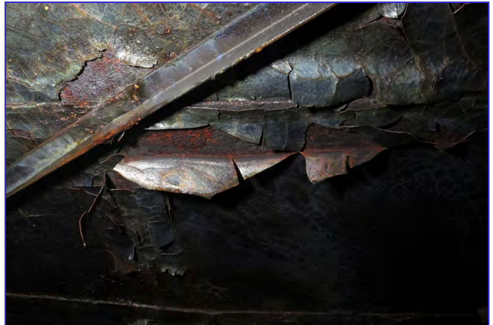
INTERIOR - Calaveras Public Utility District - Clear Well Tank - Maintenance Inspection -055
