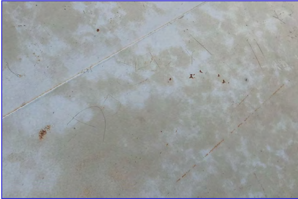
EXTERIOR - CPUD - San Andreas Reservoir - Maintenance Inspection -084
