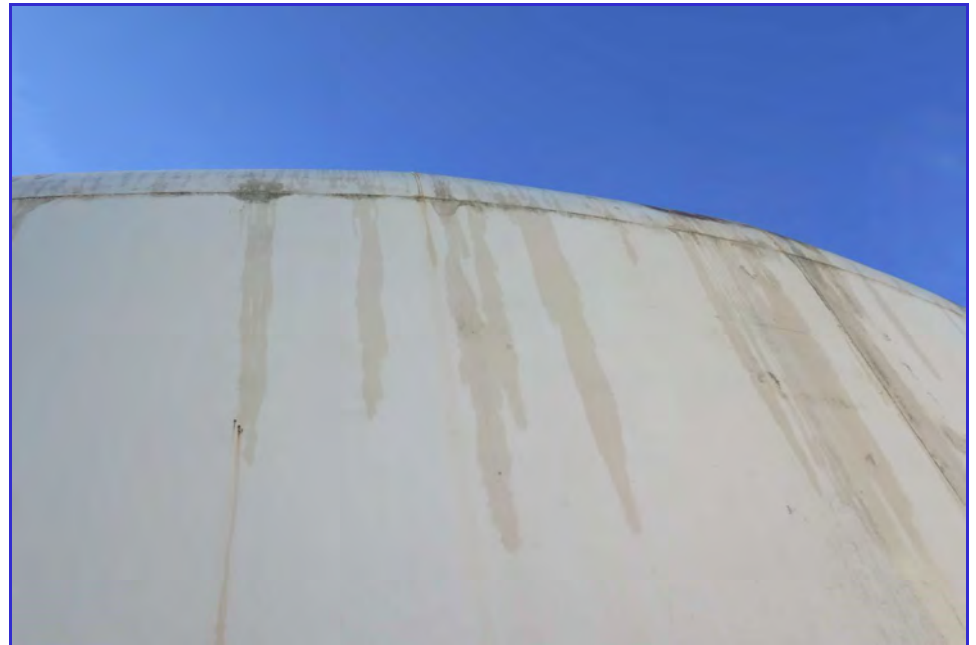
EXTERIOR - Calaveras Public Utility District - Clear Well Tank - Maintenance Inspection -115
