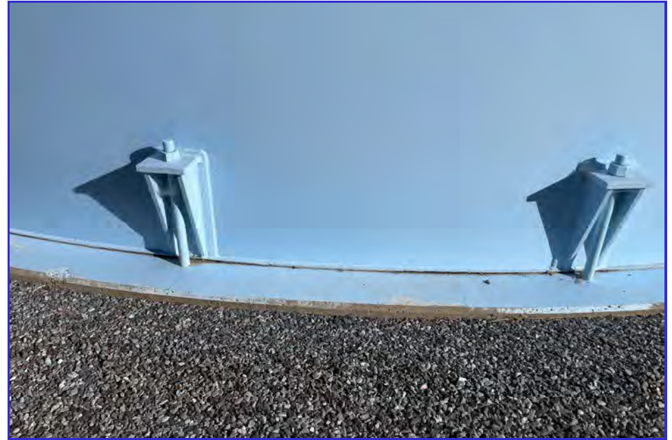
EXTERIOR - CPUD - Railroad Flat Reservoir - Maintenance Inspection -085
