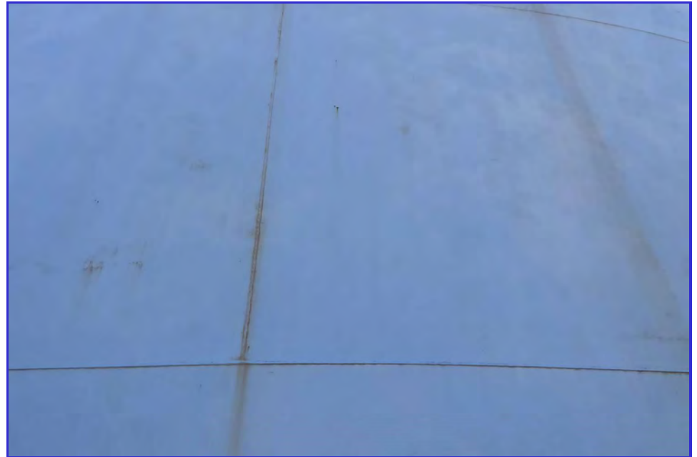
EXTERIOR - CPUD - Mokelumne Reservoir - Maintenance Inspection -117
