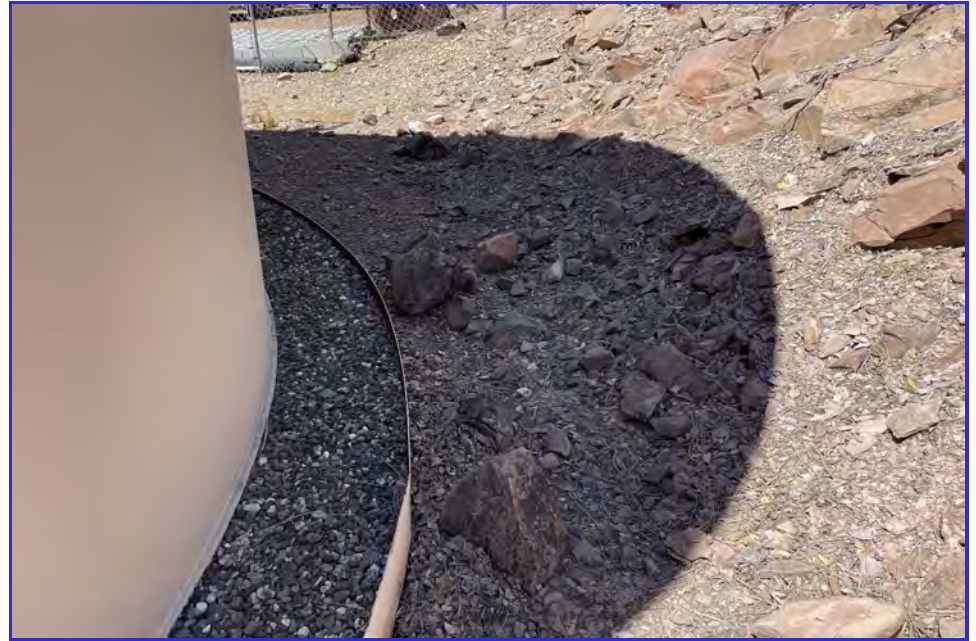
EXTERIOR - CPUD - Golden Hills - Maintenance Inspection -049
