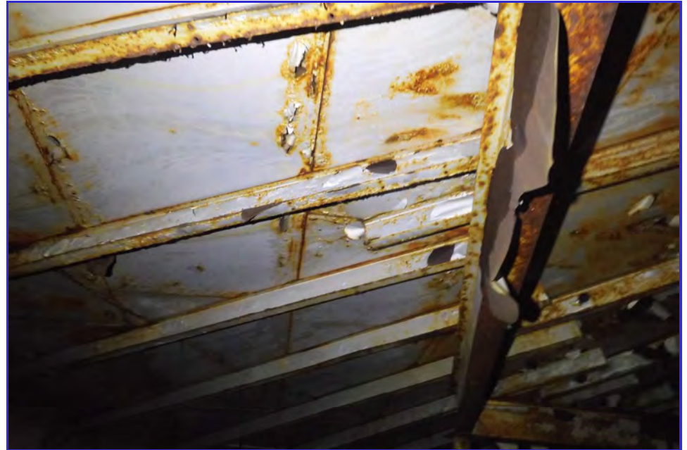
INTERIOR - CPUD - San Andaras Reservoir - Maintenance Inspection -069
