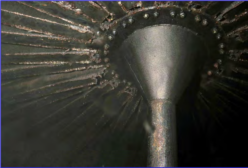
INTERIOR - Calaveras Public Utility District - Clear Well Tank - Maintenance Inspection -016
