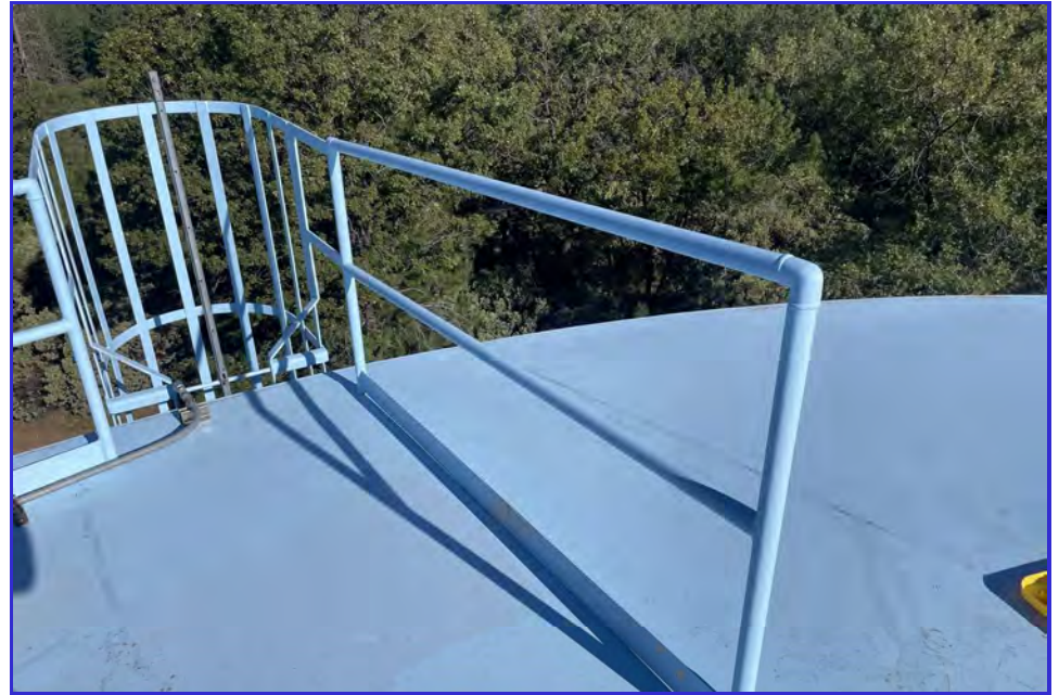
EXTERIOR - CPUD - Railroad Flat Reservoir - Maintenance Inspection -001
