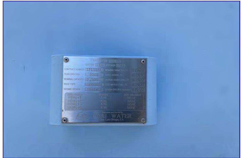
EXTERIOR - CPUD - Railroad Flat Reservoir - Maintenance Inspection -059
