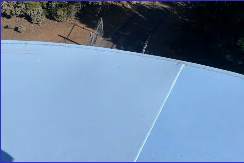
EXTERIOR - CPUD - Railroad Flat Reservoir - Maintenance Inspection -008
