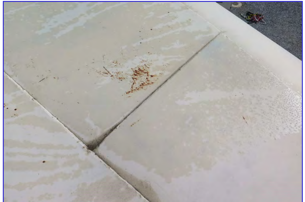
EXTERIOR - Calaveras Public Utility District - Clear Well Tank - Maintenance Inspection -039
