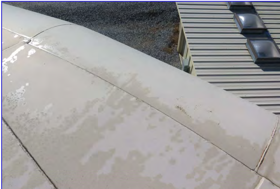
EXTERIOR - Calaveras Public Utility District - Clear Well Tank - Maintenance Inspection -030
