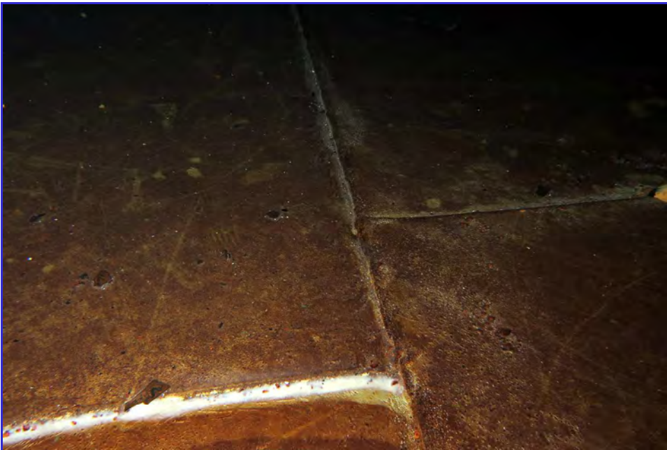
INTERIOR - Calaveras Public Utility District - Clear Well Tank - Maintenance Inspection -134
