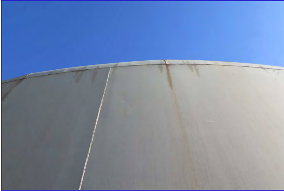
EXTERIOR - Calaveras Public Utility District - Clear Well Tank - Maintenance Inspection -080
