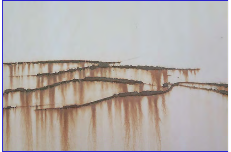
EXTERIOR - Calaveras Public Utility District - Clear Well Tank - Maintenance Inspection -109
