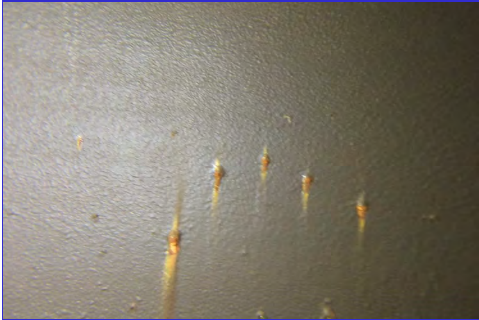
INTERIOR - CPUD - Paloma Reservoir - Maintenance Inspection -060
