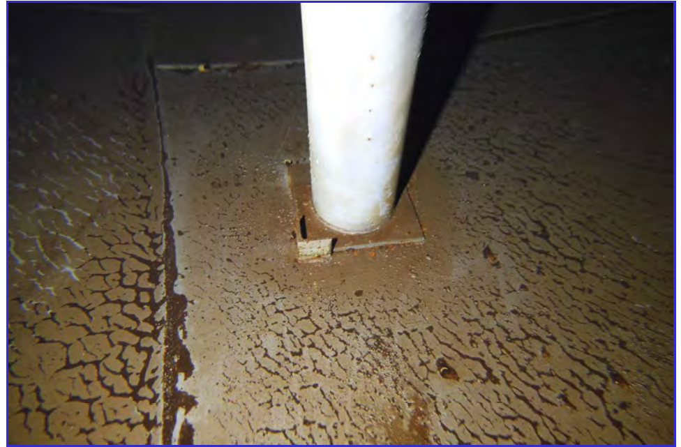
INTERIOR - CPUD - San Andaras Reservoir - Maintenance Inspection -229
