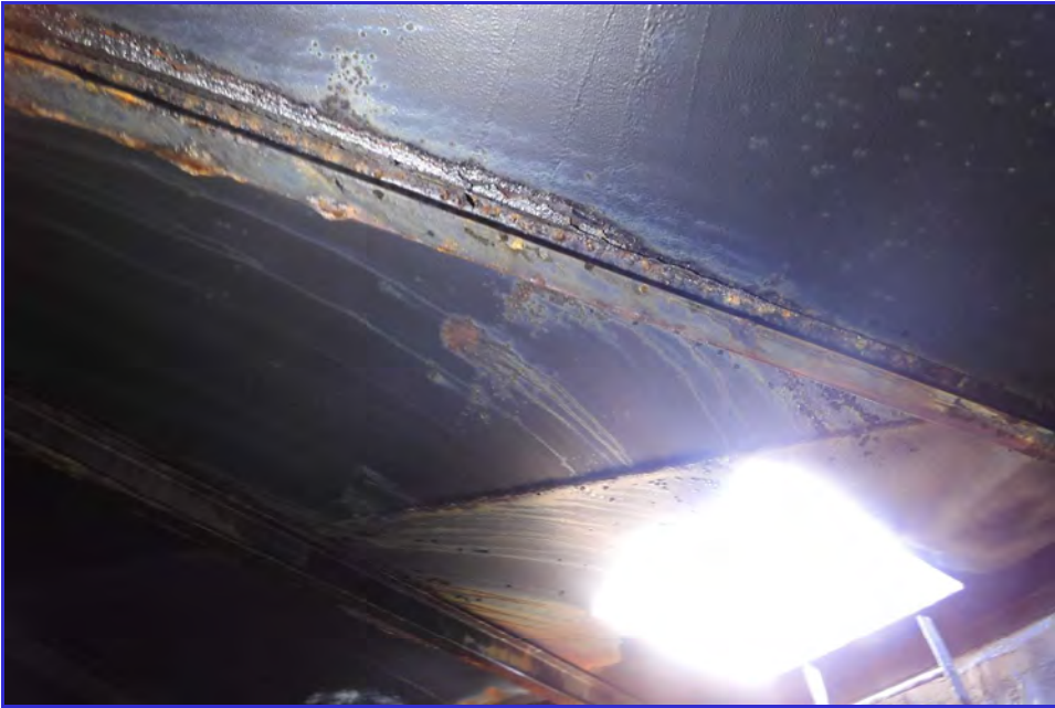
INTERIOR - CPUD - Paloma Reservoir - Maintenance Inspection -004
