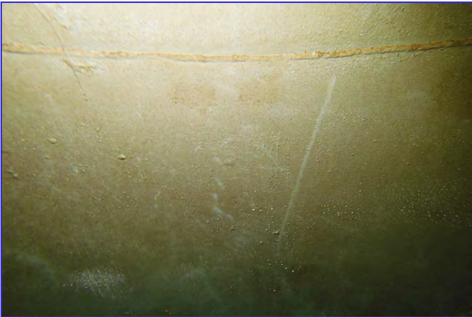
INTERIOR - CPUD - San Andaras Reservoir - Maintenance Inspection -134
