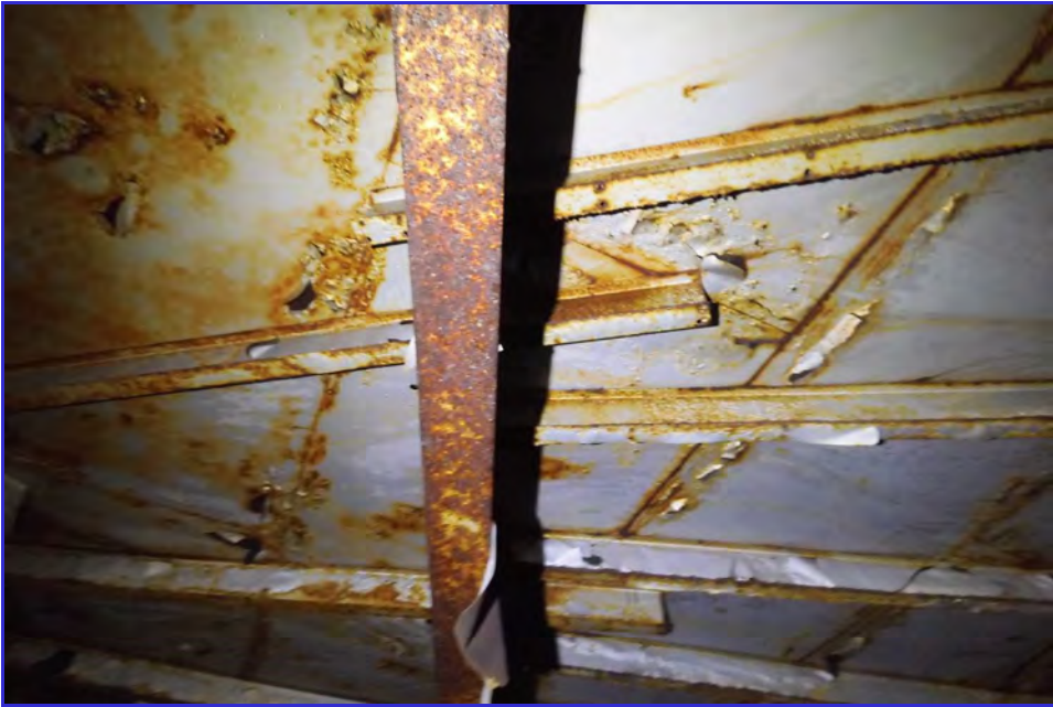
INTERIOR - CPUD - San Andaras Reservoir - Maintenance Inspection -064
