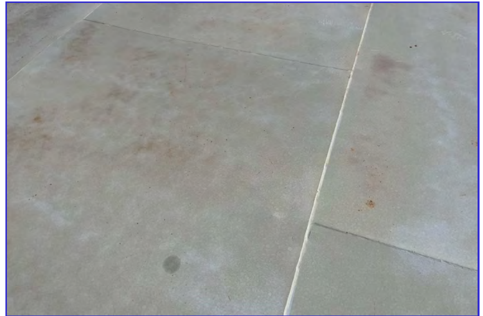
EXTERIOR - CPUD - San Andreas Reservoir - Maintenance Inspection -015
