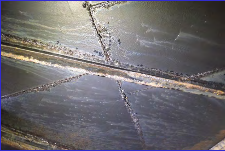
INTERIOR - CPUD - Paloma Reservoir - Maintenance Inspection -016
