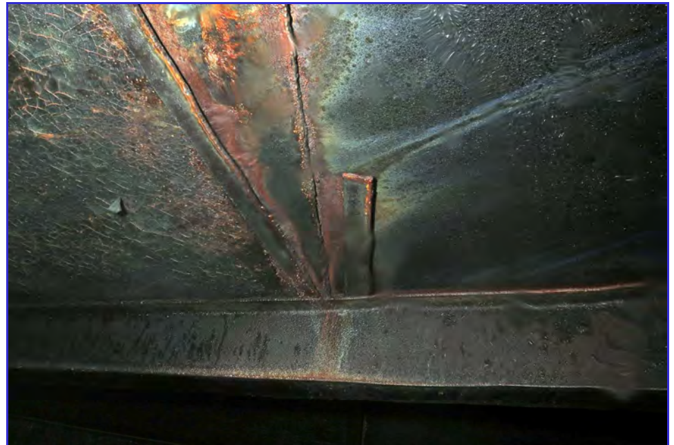
INTERIOR - Calaveras Public Utility District - Clear Well Tank - Maintenance Inspection -047
