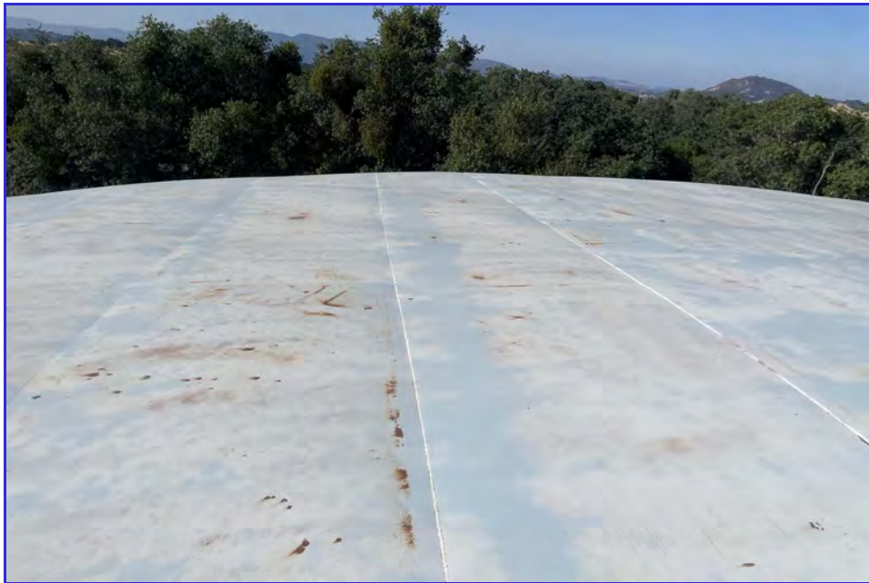
EXTERIOR - CPUD - Mokelumne Reservoir - Maintenance Inspection -014
