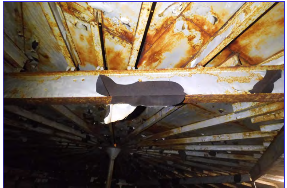
INTERIOR - CPUD - San Andaras Reservoir - Maintenance Inspection -091
