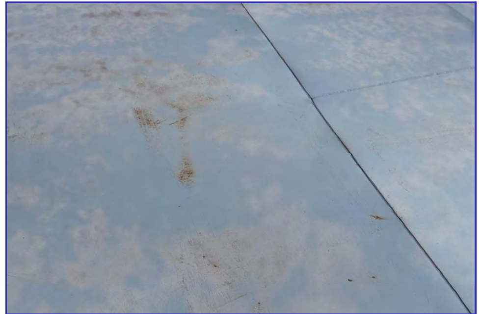
EXTERIOR - CPUD - Mokelumne Reservoir - Maintenance Inspection -035
