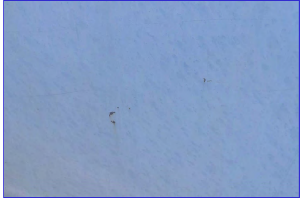
EXTERIOR - CPUD - San Andreas Reservoir - Maintenance Inspection -109
