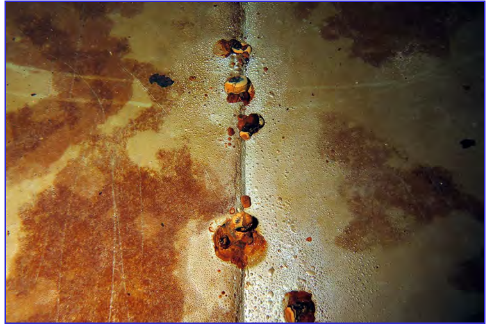
INTERIOR - Calaveras Public Utility District - Clear Well Tank - Maintenance Inspection -117
