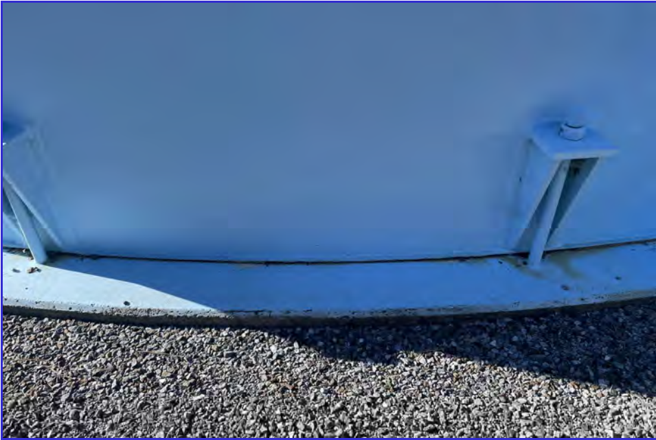
EXTERIOR - CPUD - Railroad Flat Reservoir - Maintenance Inspection -096
