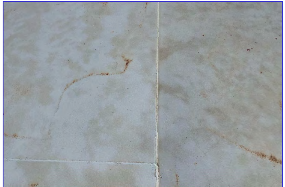
EXTERIOR - CPUD - San Andreas Reservoir - Maintenance Inspection -063
