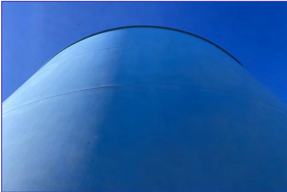
EXTERIOR - CPUD - Railroad Flat Reservoir - Maintenance Inspection -094
