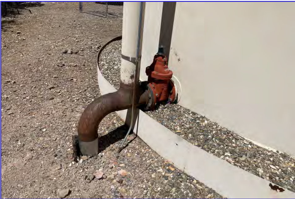
EXTERIOR - CPUD - Golden Hills - Maintenance Inspection -042
