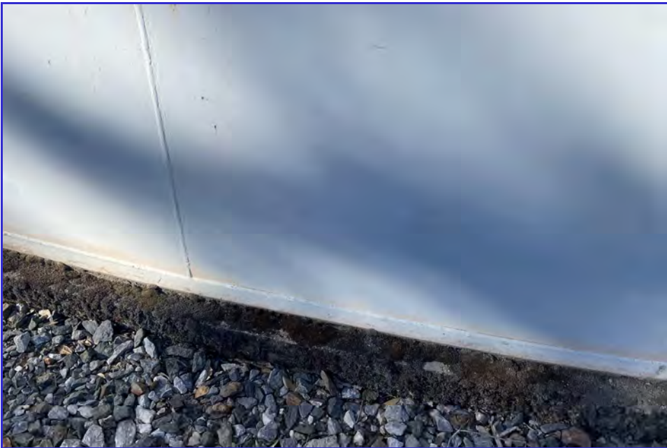
EXTERIOR - CPUD - Mokelumne Reservoir - Maintenance Inspection -174
