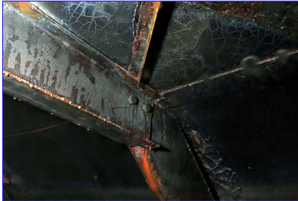
INTERIOR - Calaveras Public Utility District - Clear Well Tank - Maintenance Inspection -037
