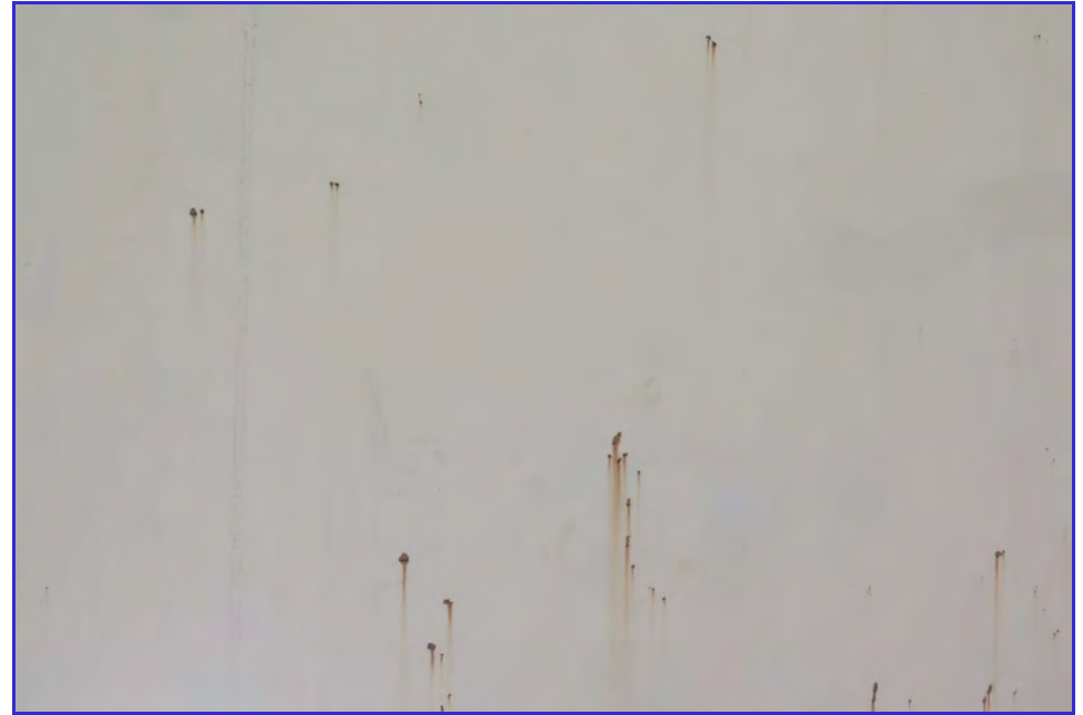
EXTERIOR - Calaveras Public Utility District - Clear Well Tank - Maintenance Inspection -061
