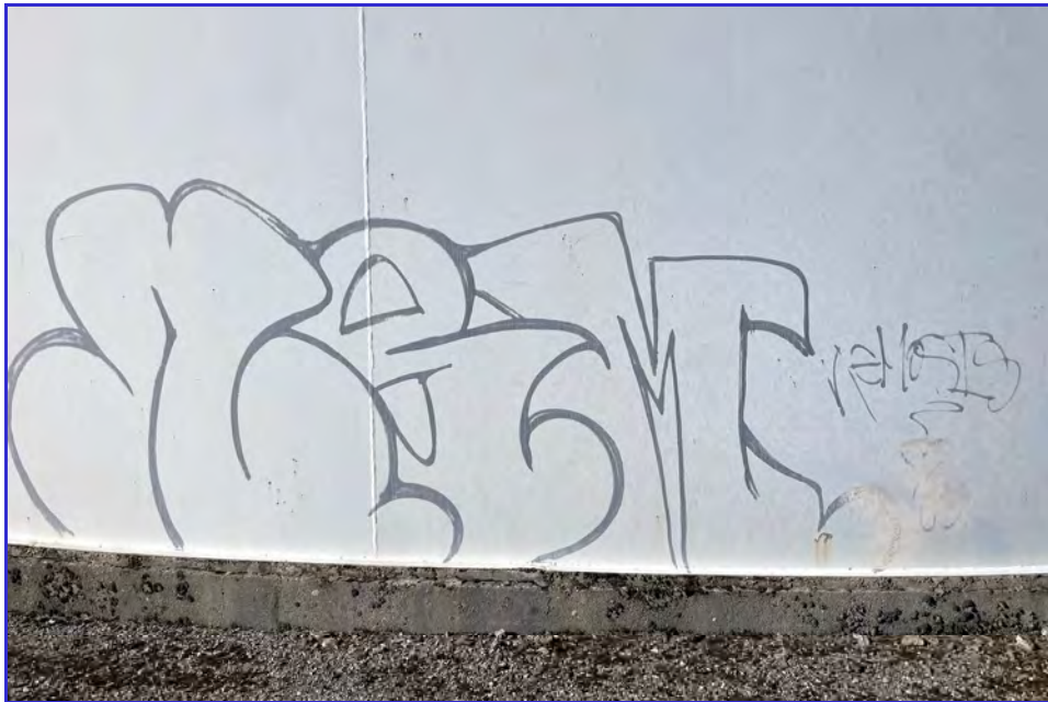
EXTERIOR - CPUD - San Andreas Reservoir - Maintenance Inspection -122
