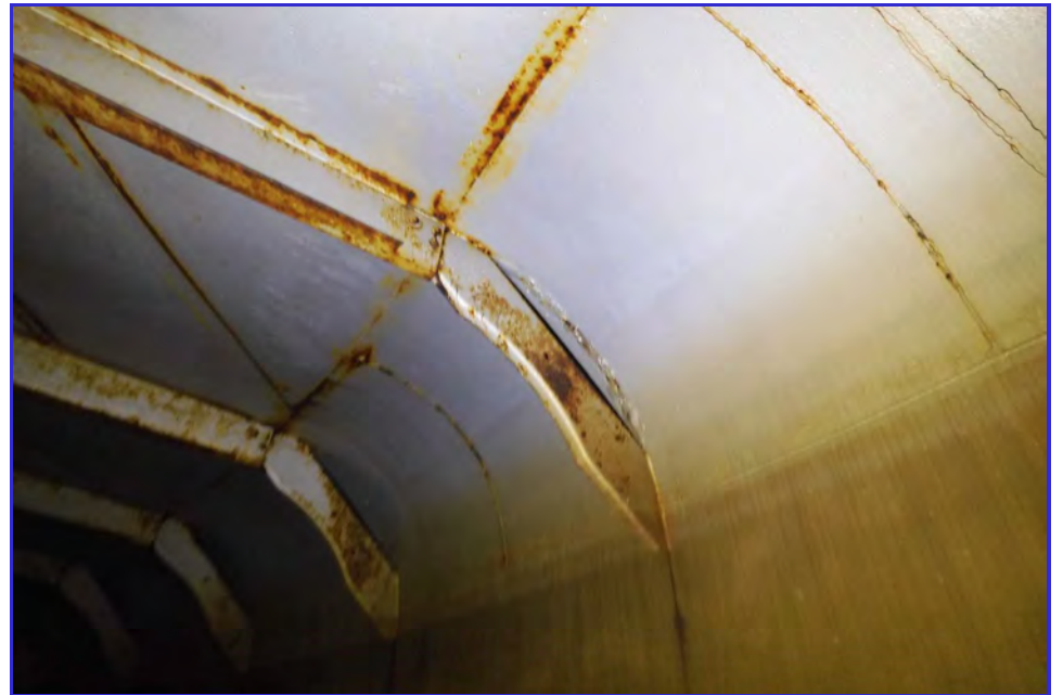
INTERIOR - CPUD - San Andaras Reservoir - Maintenance Inspection -023
