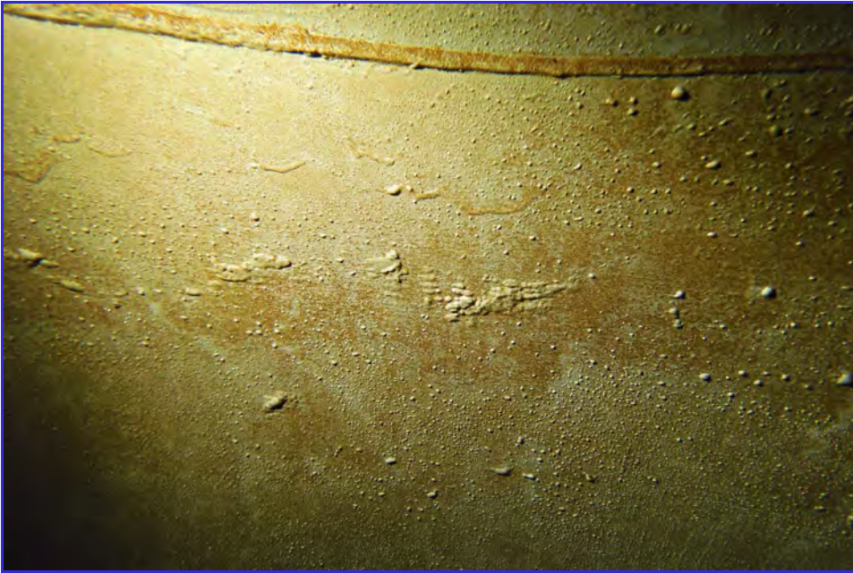
INTERIOR - CPUD - San Andaras Reservoir - Maintenance Inspection -140
