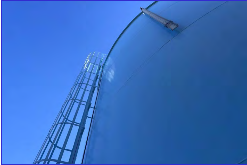
EXTERIOR - CPUD - Railroad Flat Reservoir - Maintenance Inspection -068
