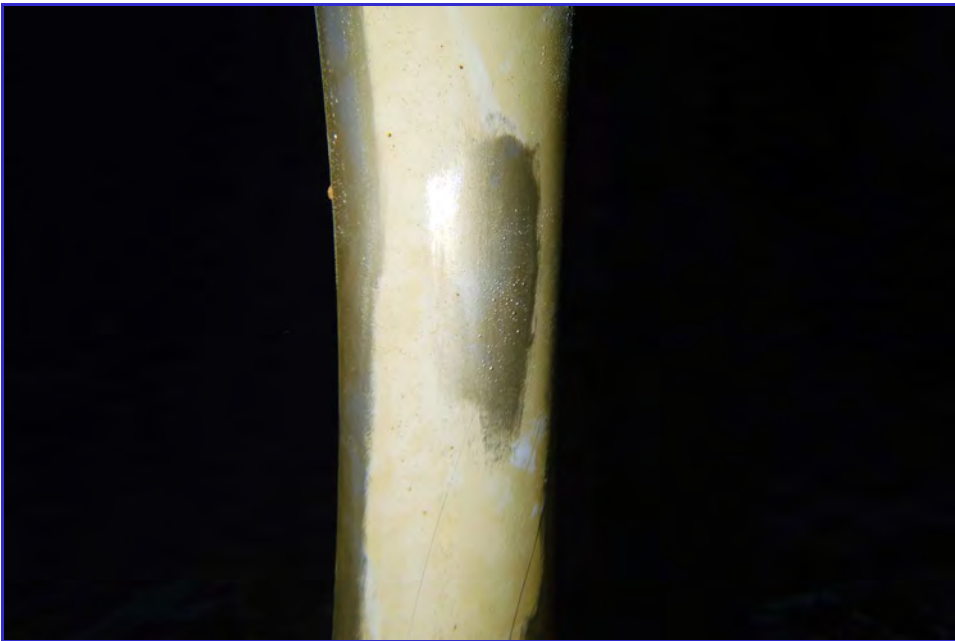
INTERIOR - CPUD - Mokelumne Hill Reservoir - Maintenance Inspection -114
