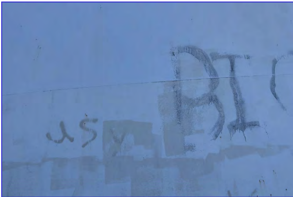
EXTERIOR - CPUD - San Andreas Reservoir - Maintenance Inspection -170
