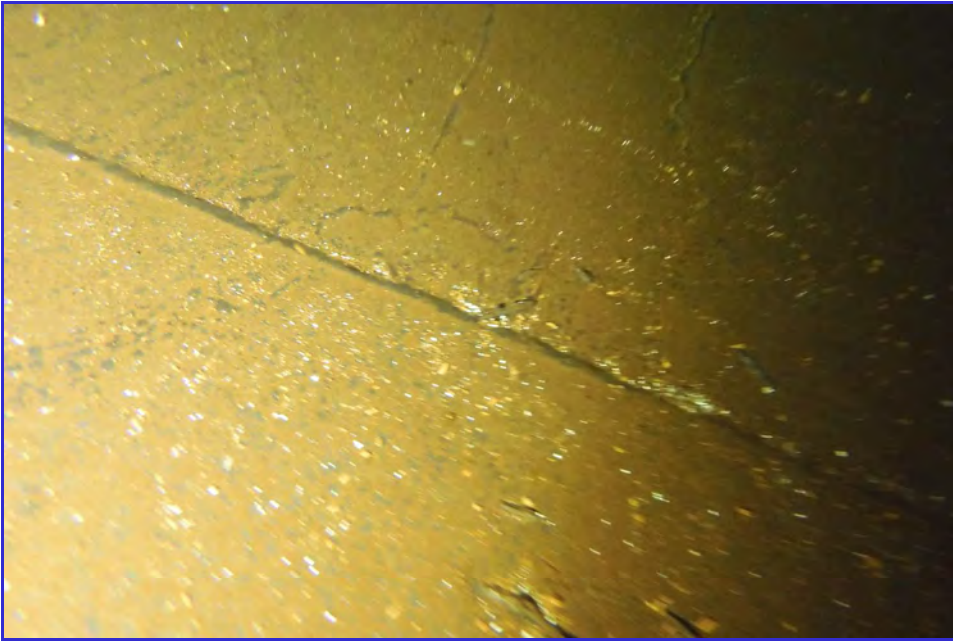
INTERIOR - CPUD - Paloma Reservoir - Maintenance Inspection -132
