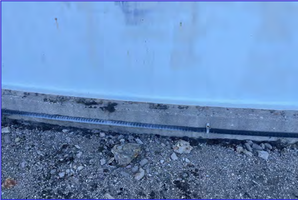
EXTERIOR - CPUD - San Andreas Reservoir - Maintenance Inspection -176
