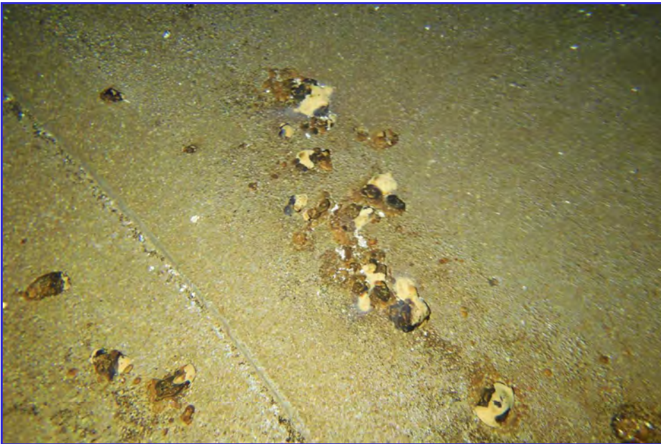
INTERIOR - CPUD - San Andaras Reservoir - Maintenance Inspection -174
