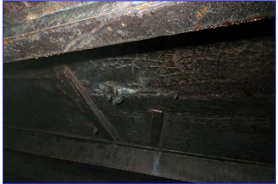
INTERIOR - Calaveras Public Utility District - Clear Well Tank - Maintenance Inspection -045
