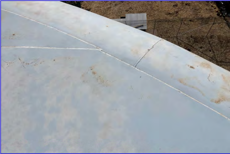
EXTERIOR - CPUD - Mokelumne Reservoir - Maintenance Inspection -060
