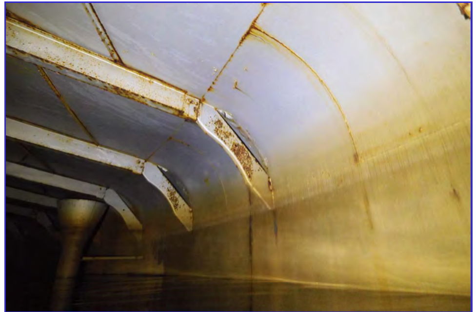
INTERIOR - CPUD - San Andaras Reservoir - Maintenance Inspection -035
