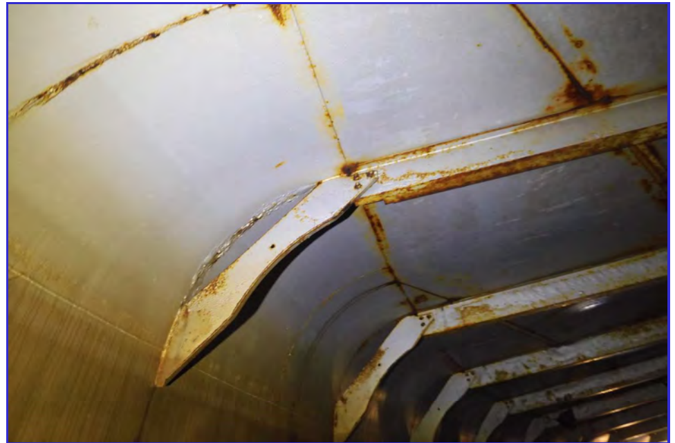
INTERIOR - CPUD - San Andaras Reservoir - Maintenance Inspection -027
