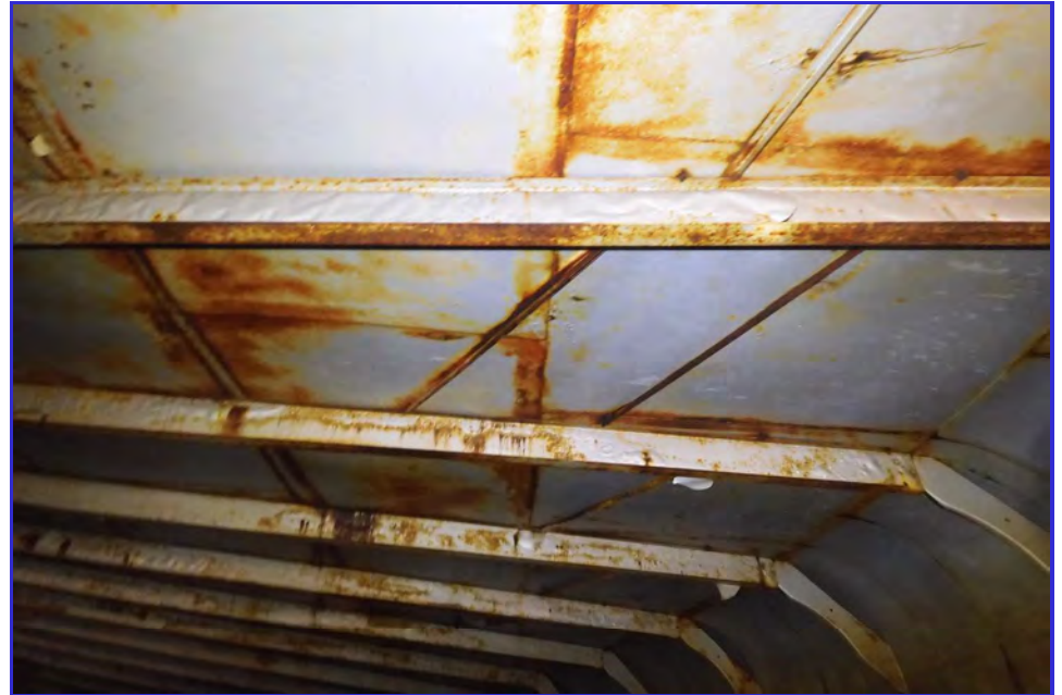
INTERIOR - CPUD - San Andaras Reservoir - Maintenance Inspection -005
