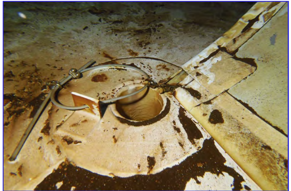
INTERIOR - CPUD - Railroad Flat Reservoir - Maintenance Inspection -167
