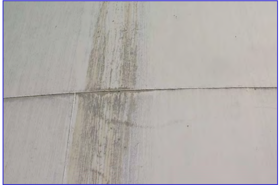
EXTERIOR - Calaveras Public Utility District - Clear Well Tank - Maintenance Inspection -073
