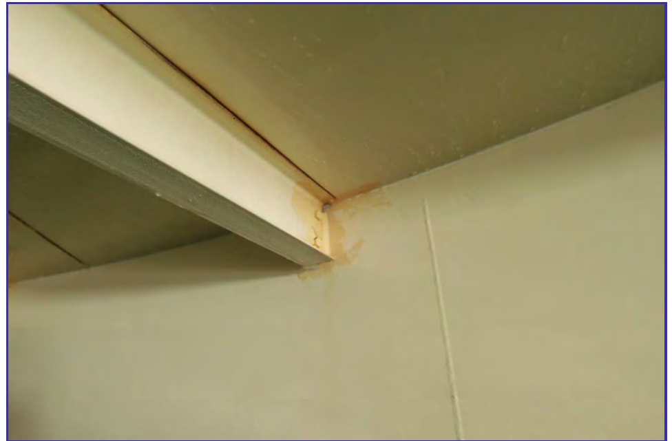
INTERIOR - CPUD - Railroad Flat Reservoir - Maintenance Inspection -023
