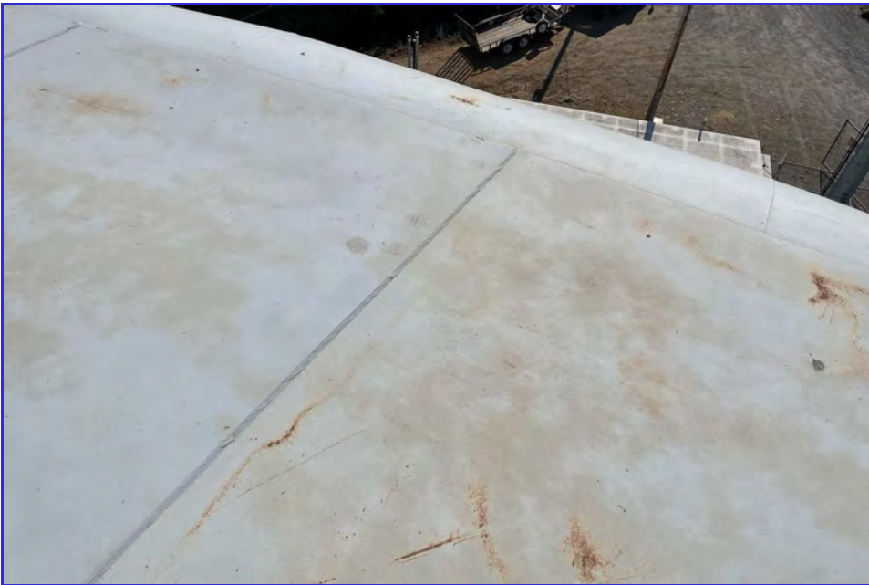
EXTERIOR - CPUD - San Andreas Reservoir - Maintenance Inspection -094
