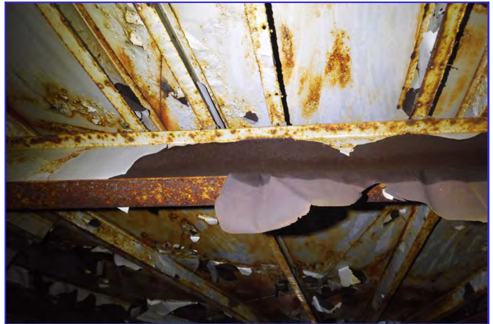
INTERIOR - CPUD - San Andaras Reservoir - Maintenance Inspection -067
