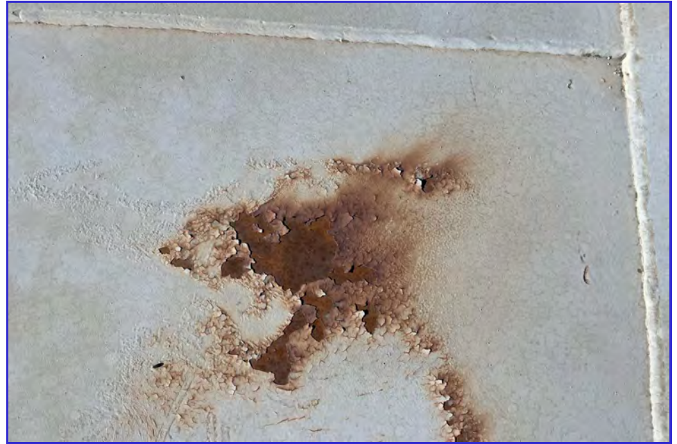
EXTERIOR - CPUD - San Andreas Reservoir - Maintenance Inspection -081
