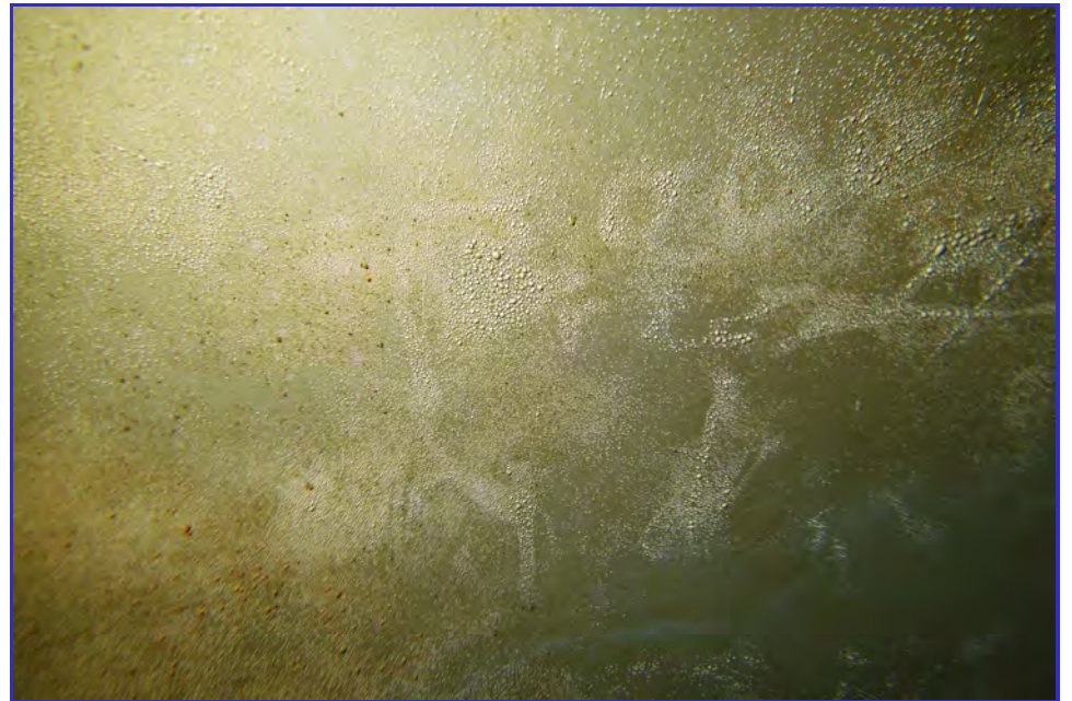
INTERIOR - CPUD - Mokelumne Hill Reservoir - Maintenance Inspection -095
