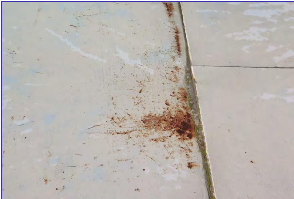
EXTERIOR - Calaveras Public Utility District - Clear Well Tank - Maintenance Inspection -018
