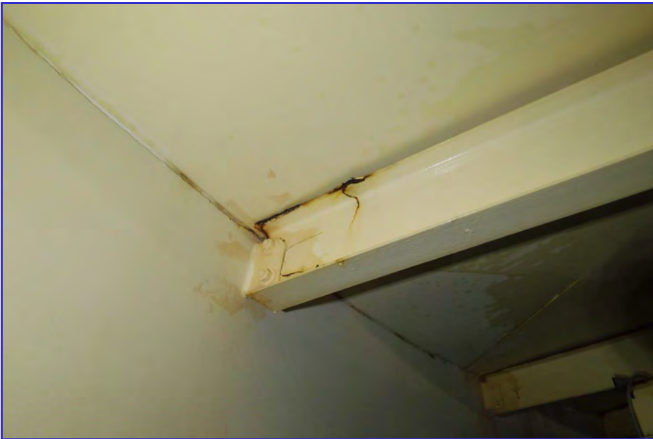
INTERIOR - CPUD - Railroad Flat Reservoir - Maintenance Inspection -066
