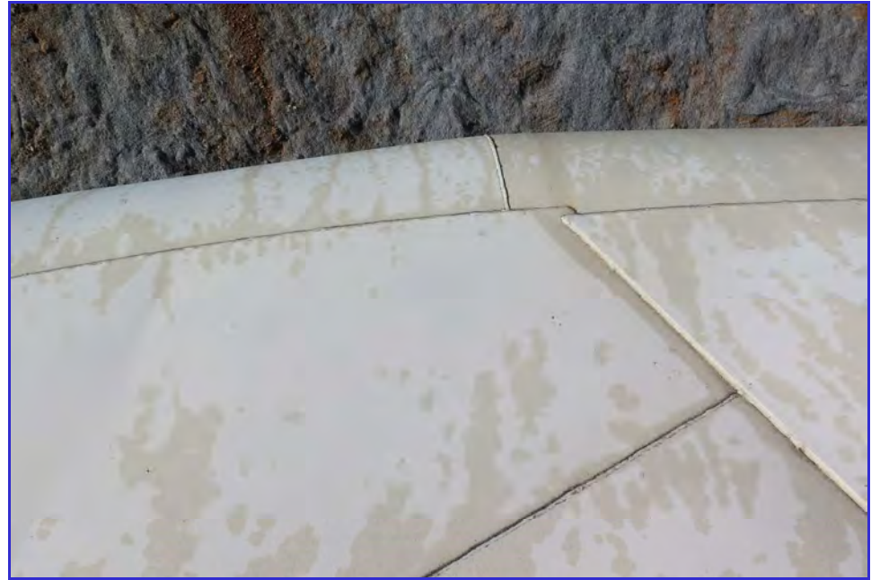
EXTERIOR - Calaveras Public Utility District - Clear Well Tank - Maintenance Inspection -025
