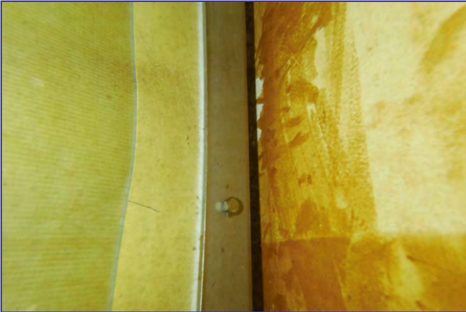
INTERIOR - CPUD - Railroad Flat Reservoir - Maintenance Inspection -144
