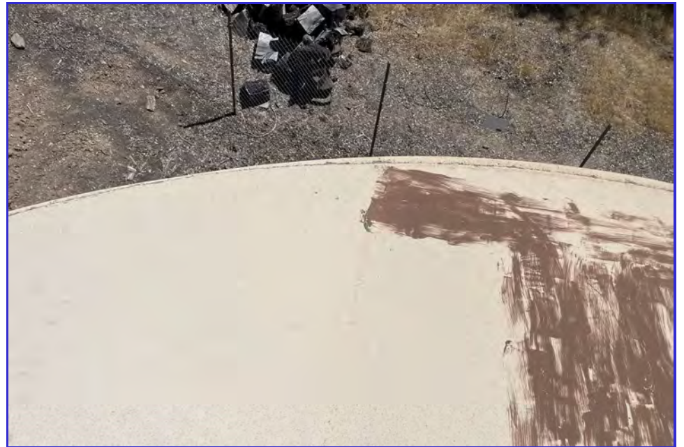
EXTERIOR - CPUD - Golden Hills - Maintenance Inspection -007
