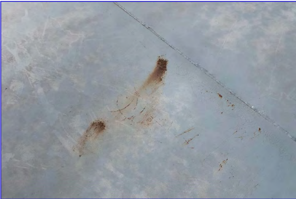
EXTERIOR - CPUD - Mokelumne Reservoir - Maintenance Inspection -006
