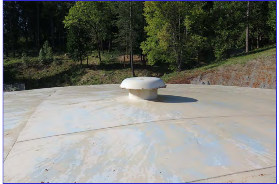
EXTERIOR - Calaveras Public Utility District - Clear Well Tank - Maintenance Inspection -009
