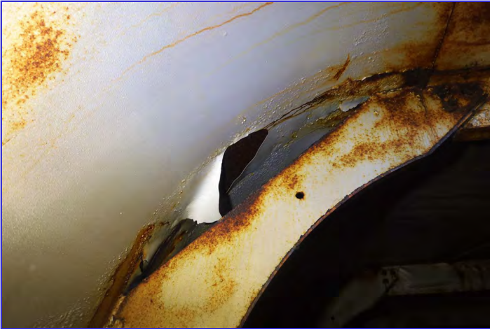
INTERIOR - CPUD - San Andreas Reservoir - Maintenance Inspection -002
