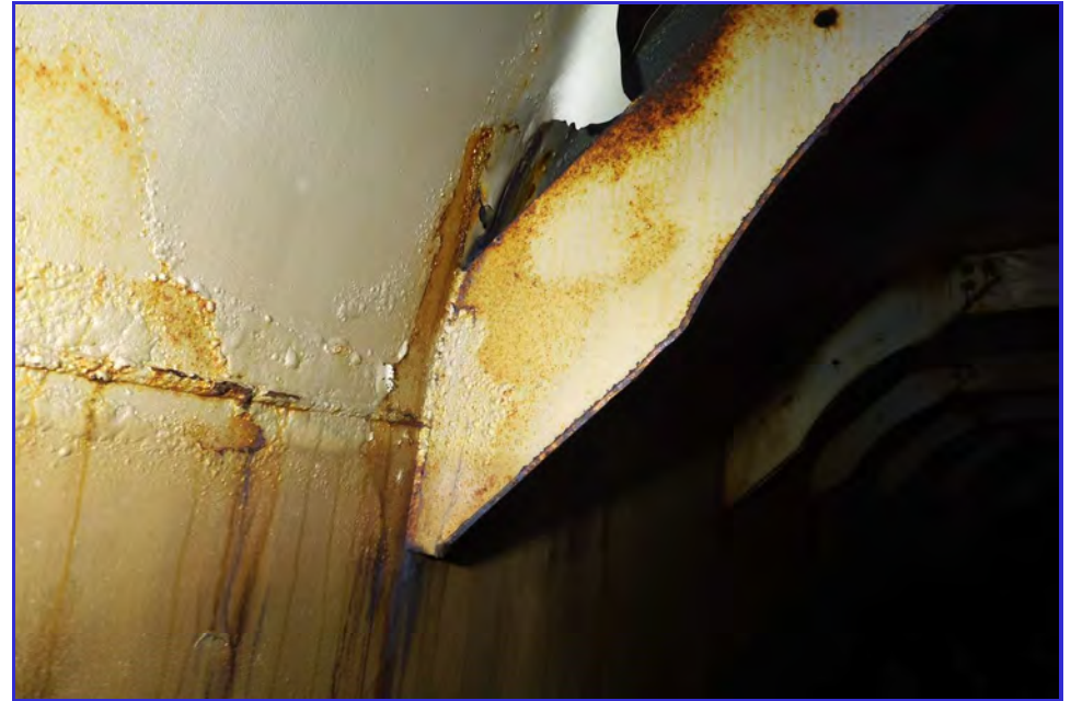
INTERIOR - CPUD - San Andreas Reservoir - Maintenance Inspection -003
