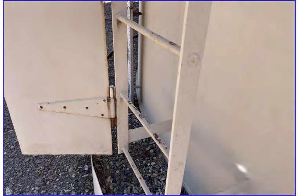
EXTERIOR - CPUD - Golden Hills - Maintenance Inspection -037
