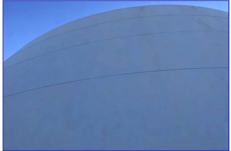
EXTERIOR - CPUD - San Andreas Reservoir - Maintenance Inspection -169
