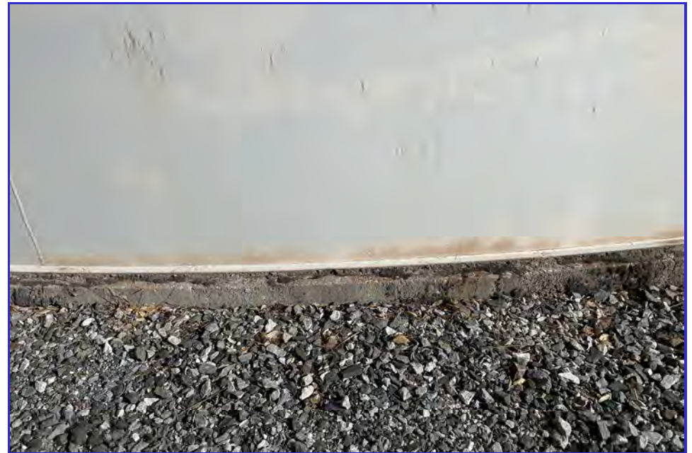
EXTERIOR - CPUD - Mokelumne Reservoir - Maintenance Inspection -159
