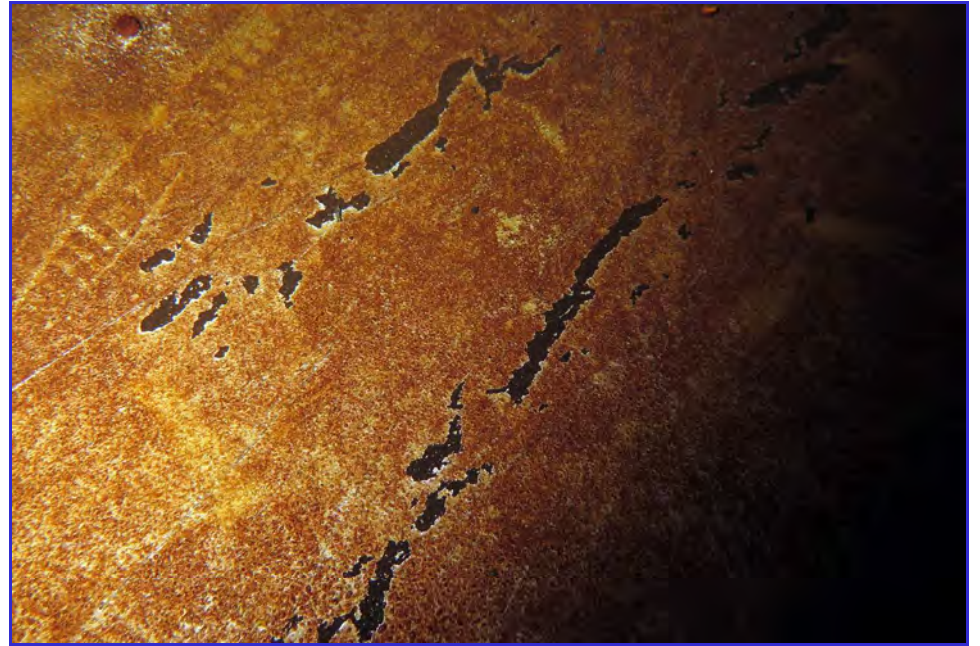
INTERIOR - Calaveras Public Utility District - Clear Well Tank - Maintenance Inspection -137
