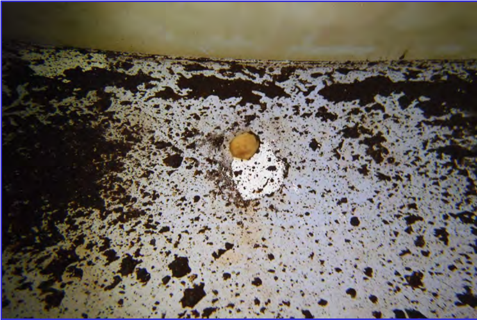
INTERIOR - CPUD - Mokelumne Hill Reservoir - Maintenance Inspection -068
