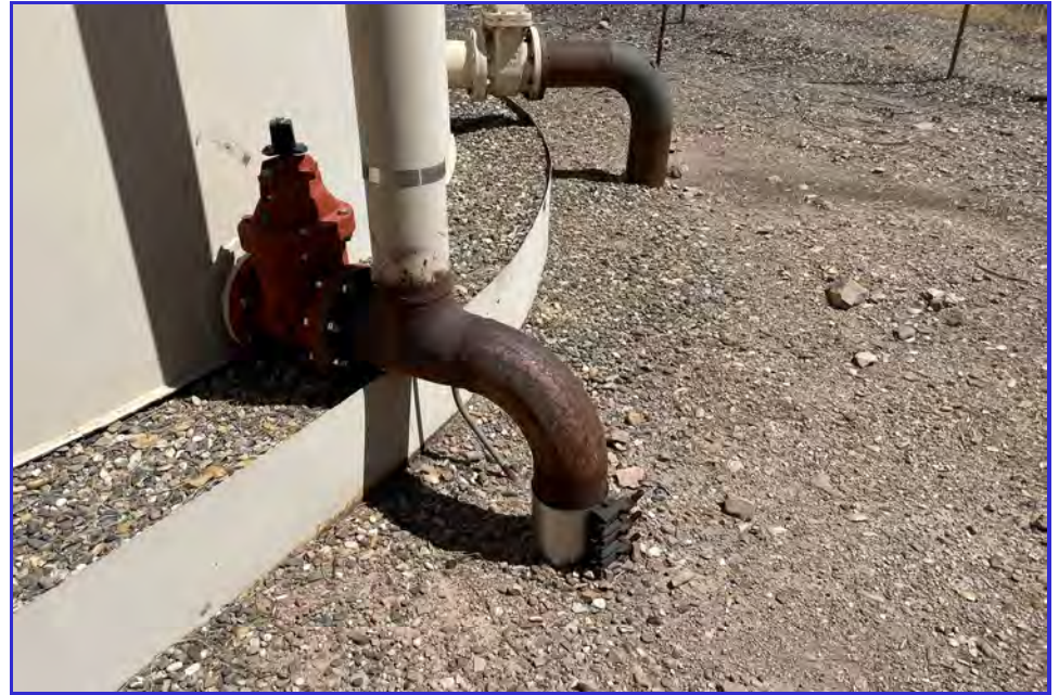
EXTERIOR - CPUD - Golden Hills - Maintenance Inspection -041
