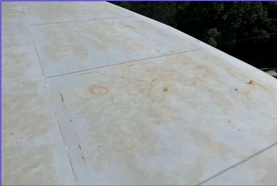
EXTERIOR - CPUD - San Andreas Reservoir - Maintenance Inspection -096
