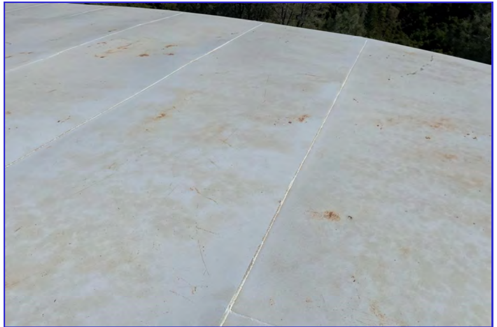
EXTERIOR - CPUD - San Andreas Reservoir - Maintenance Inspection -091
