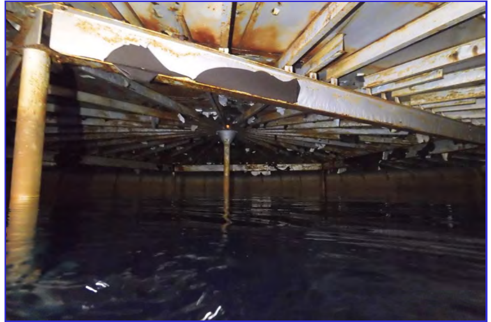
INTERIOR - CPUD - San Andaras Reservoir - Maintenance Inspection -009
