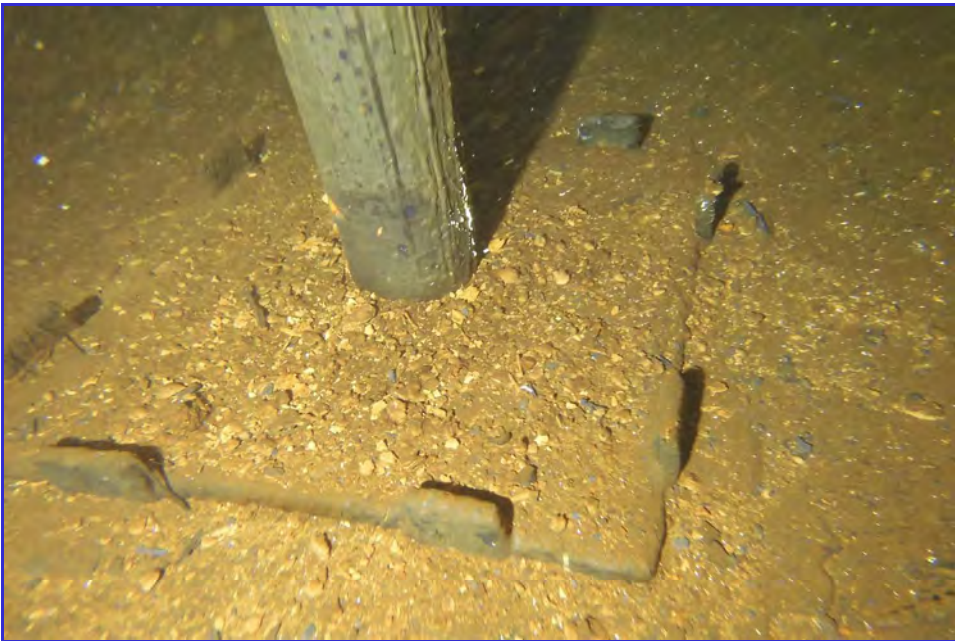
INTERIOR - CPUD - Paloma Reservoir - Maintenance Inspection -126
