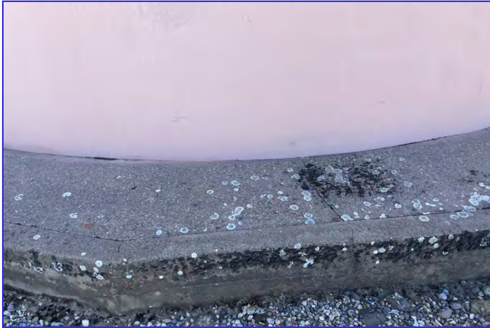
EXTERIOR - CPUD - Paloma Reservoir - Maintenance Inspection -080
