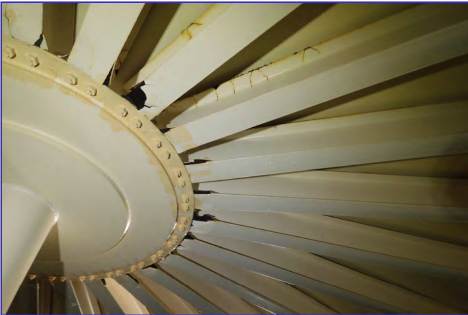
INTERIOR - CPUD - Railroad Flat Reservoir - Maintenance Inspection -038
