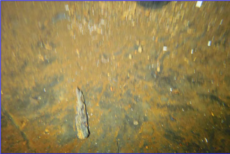
INTERIOR - CPUD - Paloma Reservoir - Maintenance Inspection -112
