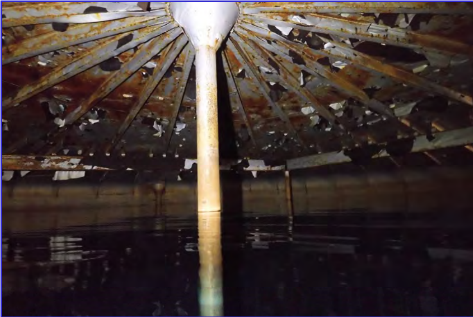
INTERIOR - CPUD - San Andaras Reservoir - Maintenance Inspection -084
