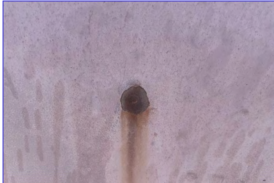
EXTERIOR - CPUD - Paloma Reservoir - Maintenance Inspection -085
