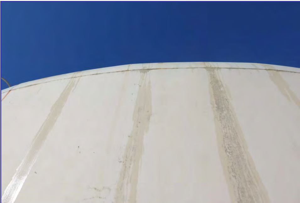
EXTERIOR - Calaveras Public Utility District - Clear Well Tank - Maintenance Inspection -122
