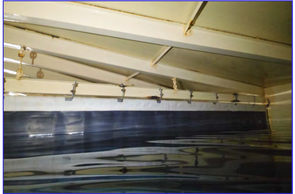
INTERIOR - CPUD - Railroad Flat Reservoir - Maintenance Inspection -049
