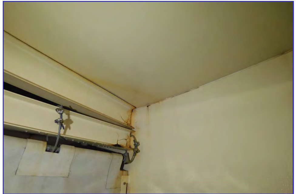
INTERIOR - CPUD - Railroad Flat Reservoir - Maintenance Inspection -027
