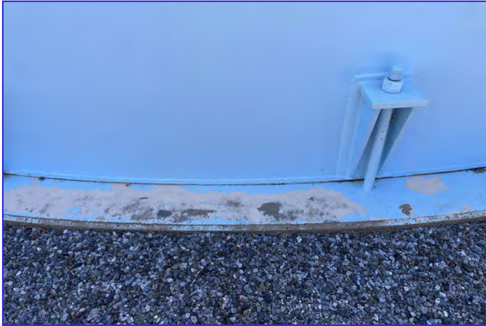
EXTERIOR - CPUD - Railroad Flat Reservoir - Maintenance Inspection -072
