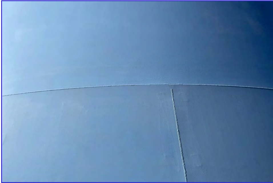
EXTERIOR - CPUD - Railroad Flat Reservoir - Maintenance Inspection -092
