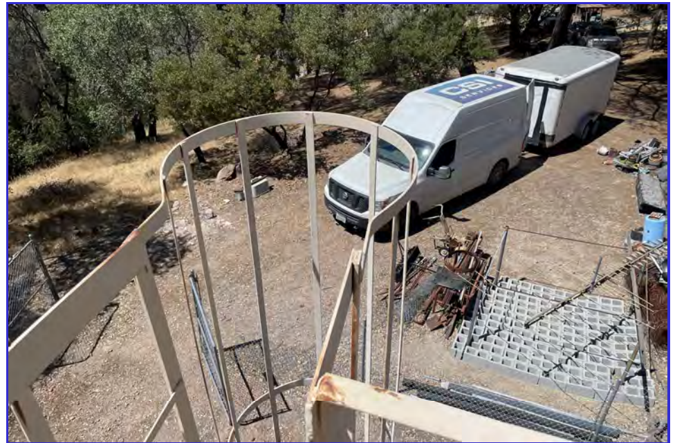
EXTERIOR - CPUD - Golden Hills - Maintenance Inspection -019
