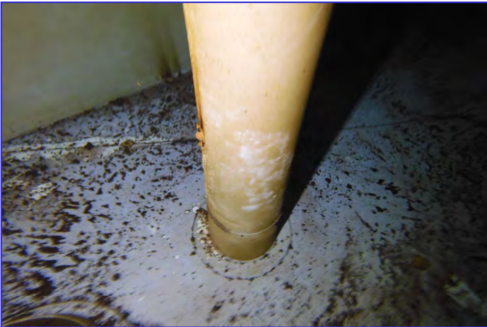
INTERIOR - CPUD - Mokelumne Hill Reservoir - Maintenance Inspection -110
