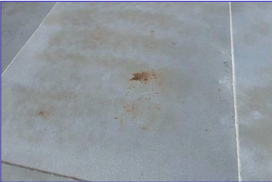
EXTERIOR - CPUD - San Andreas Reservoir - Maintenance Inspection -010
