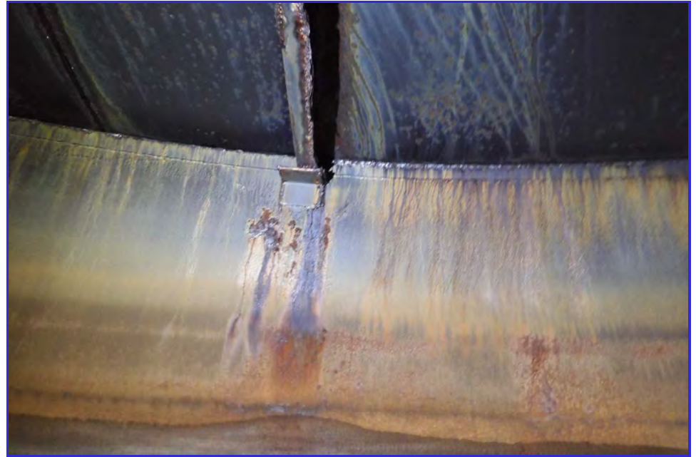
INTERIOR - CPUD - Paloma Reservoir - Maintenance Inspection -009
