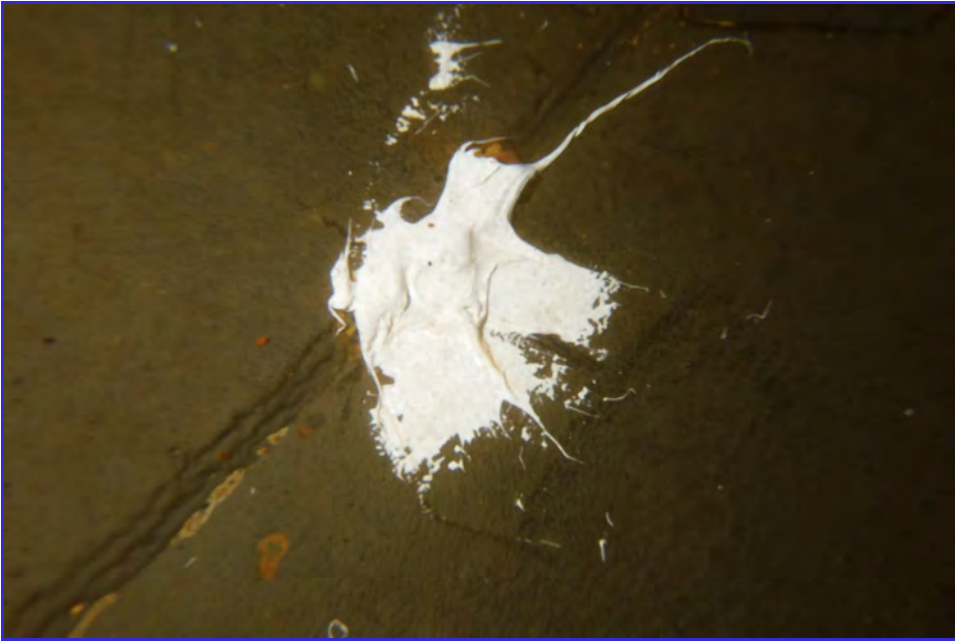
INTERIOR - CPUD - Golden Hills - Maintenance Inspection -120
