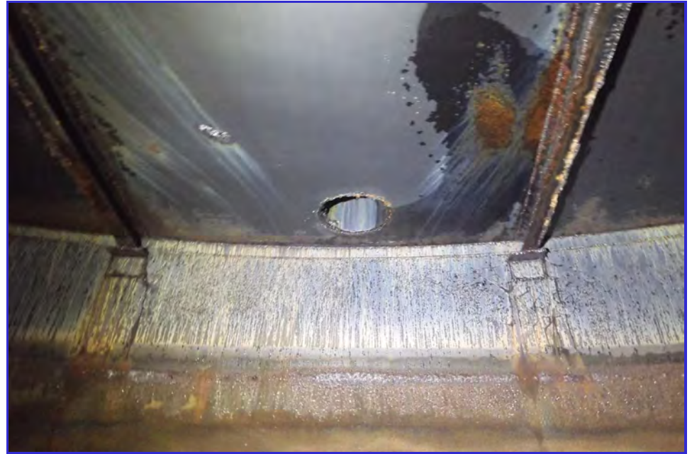
INTERIOR - CPUD - Paloma Reservoir - Maintenance Inspection -021
