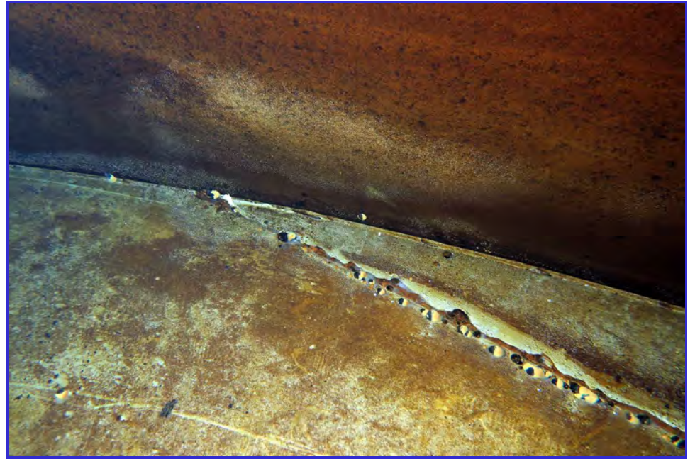
INTERIOR - Calaveras Public Utility District - Clear Well Tank - Maintenance Inspection -081
