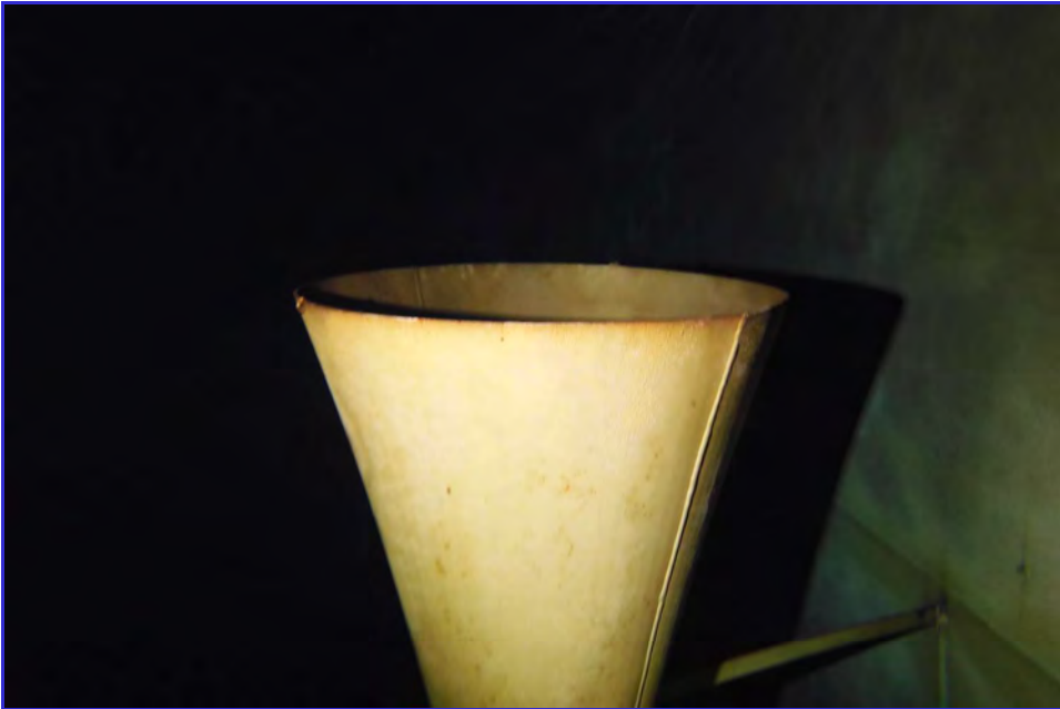
INTERIOR - CPUD - Mokelumne Hill Reservoir - Maintenance Inspection -060
