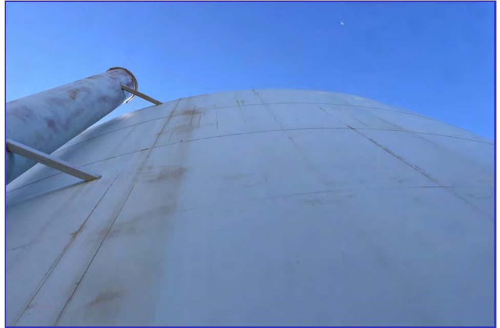
EXTERIOR - CPUD - Mokelumne Reservoir - Maintenance Inspection -129
