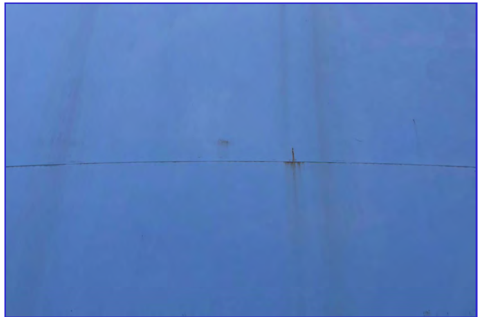
EXTERIOR - CPUD - Mokelumne Reservoir - Maintenance Inspection -123
