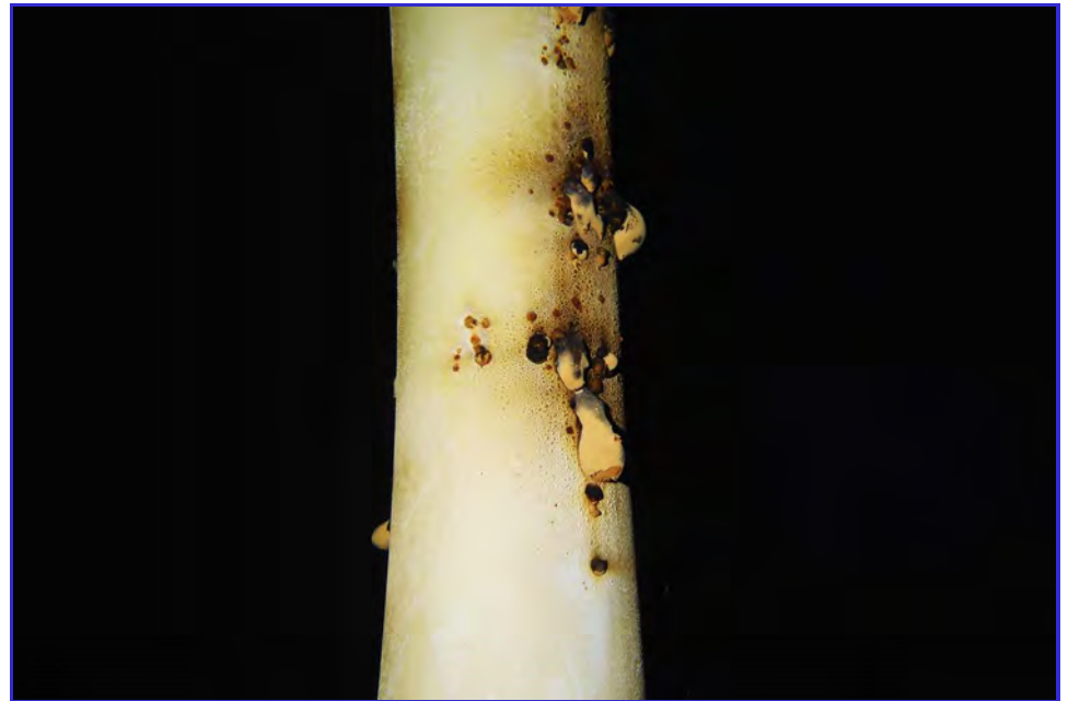
INTERIOR - CPUD - Mokelumne Hill Reservoir - Maintenance Inspection -115
