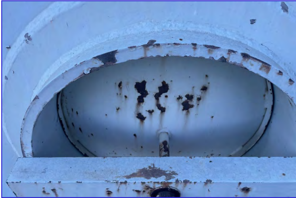
EXTERIOR - CPUD - San Andreas Reservoir - Maintenance Inspection -192
