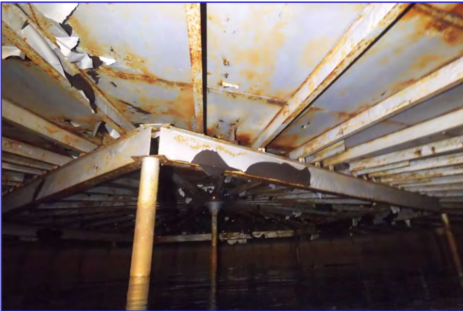
INTERIOR - CPUD - San Andaras Reservoir - Maintenance Inspection -006
