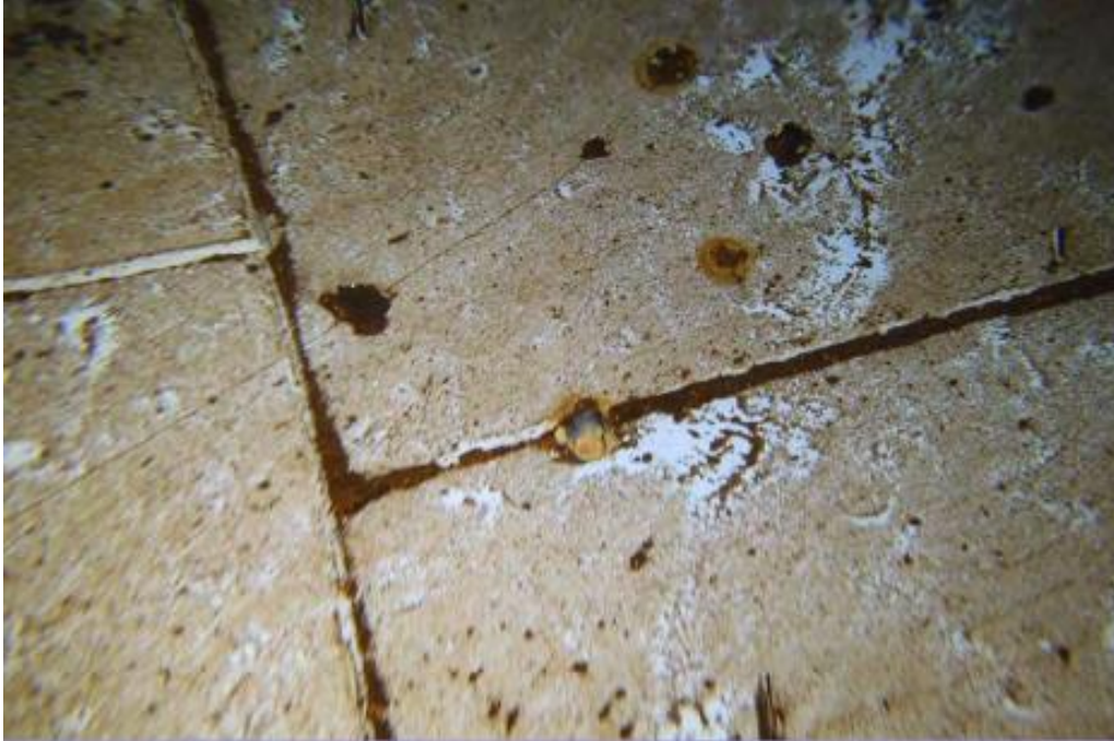
Figure 9-4. Example of Interior Mokelumne Hill Tank Floor
