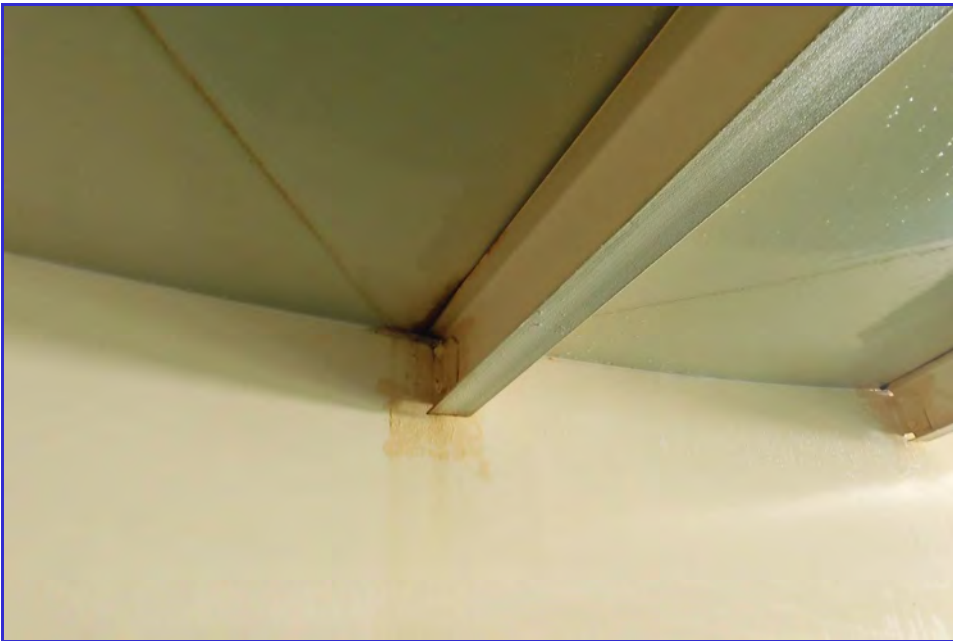
INTERIOR - CPUD - Railroad Flat Reservoir - Maintenance Inspection -022
