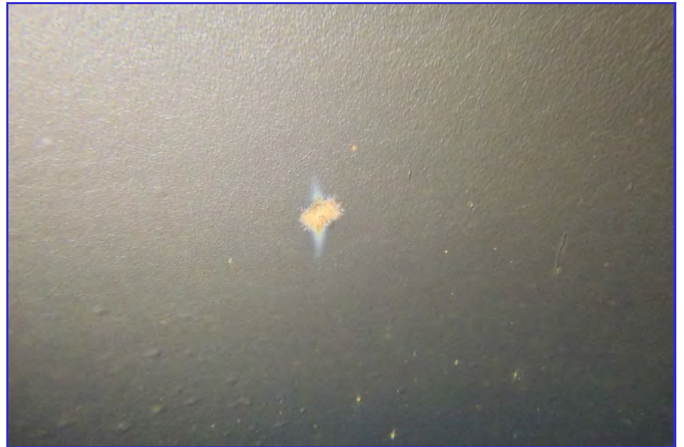
INTERIOR - CPUD - Paloma Reservoir - Maintenance Inspection -055
