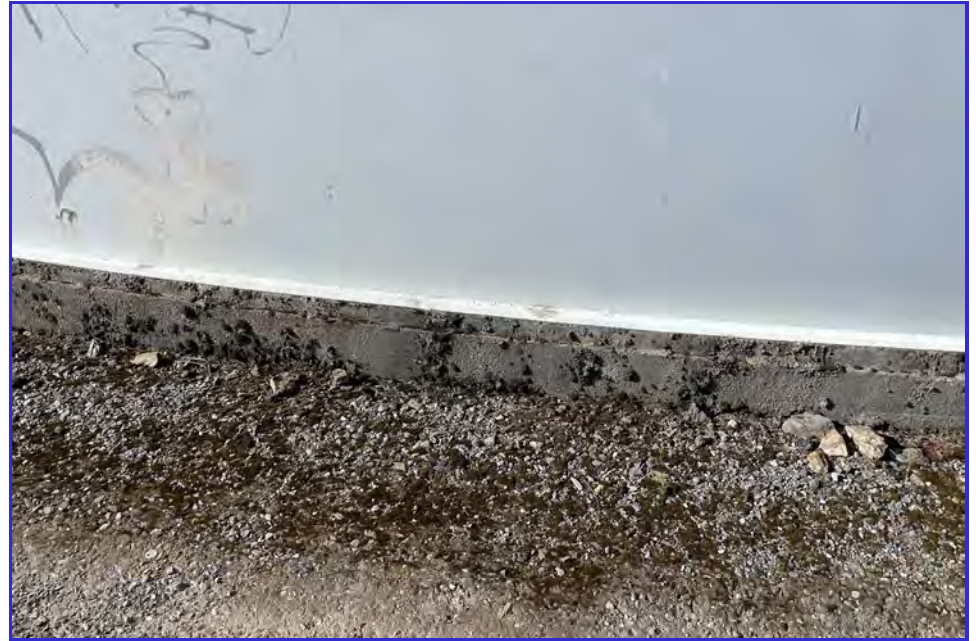
EXTERIOR - CPUD - San Andreas Reservoir - Maintenance Inspection -121
