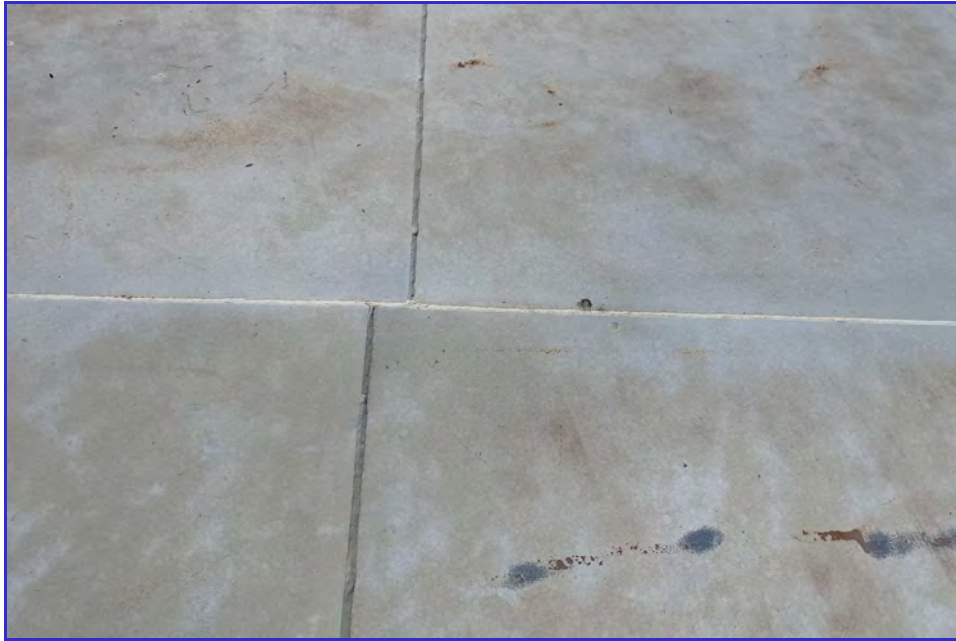
EXTERIOR - CPUD - San Andreas Reservoir - Maintenance Inspection -028
