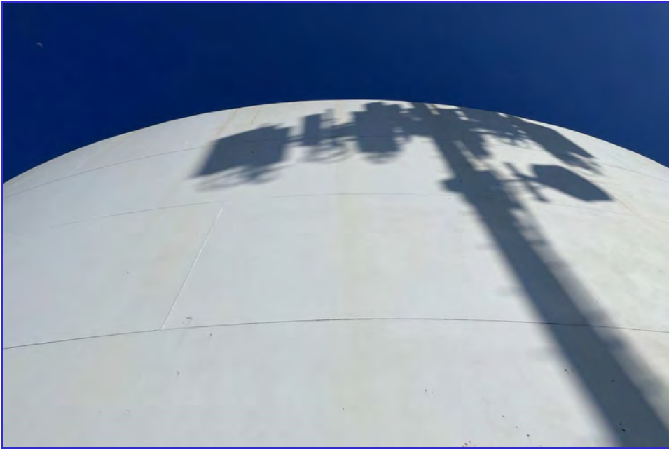
EXTERIOR - CPUD - San Andreas Reservoir - Maintenance Inspection -148
