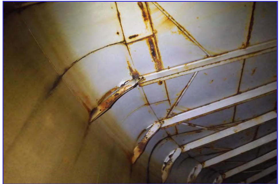
INTERIOR - CPUD - Mokelumne Hill Reservoir - Maintenance Inspection -059
