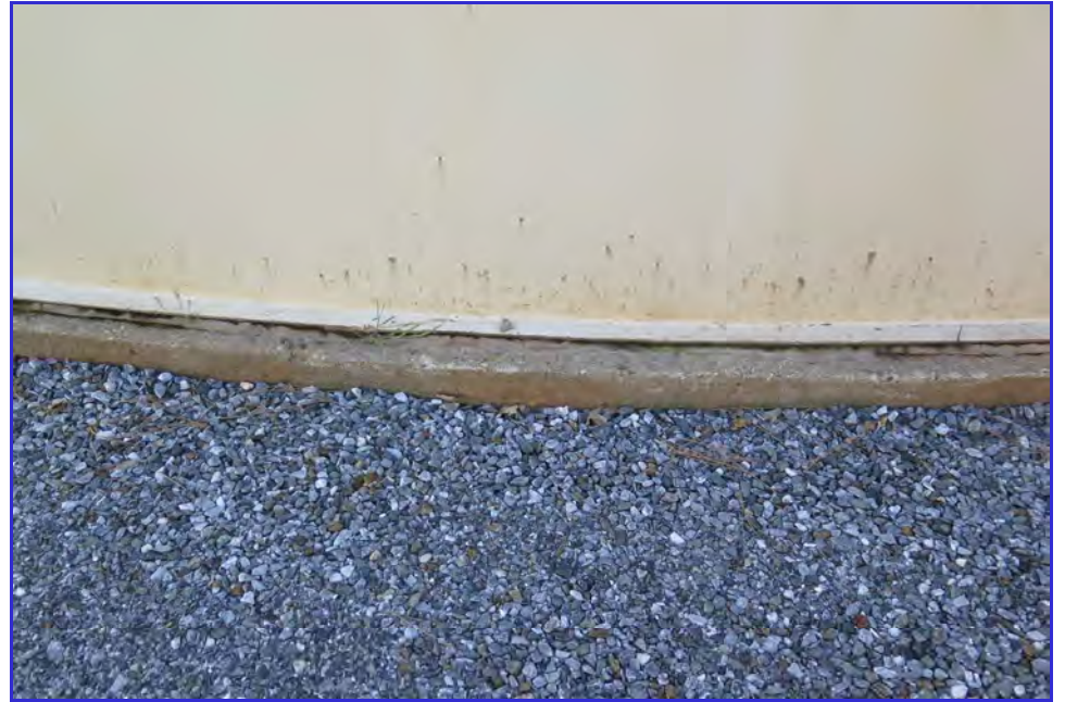
EXTERIOR - Calaveras Public Utility District - Clear Well Tank - Maintenance Inspection -101
