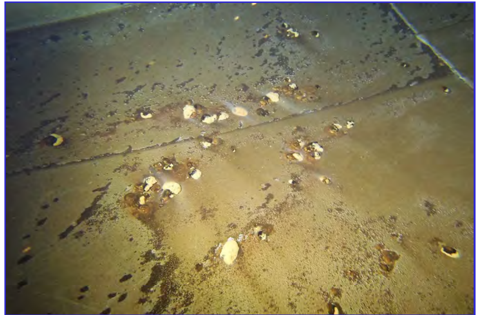
INTERIOR - CPUD - San Andaras Reservoir - Maintenance Inspection -211
