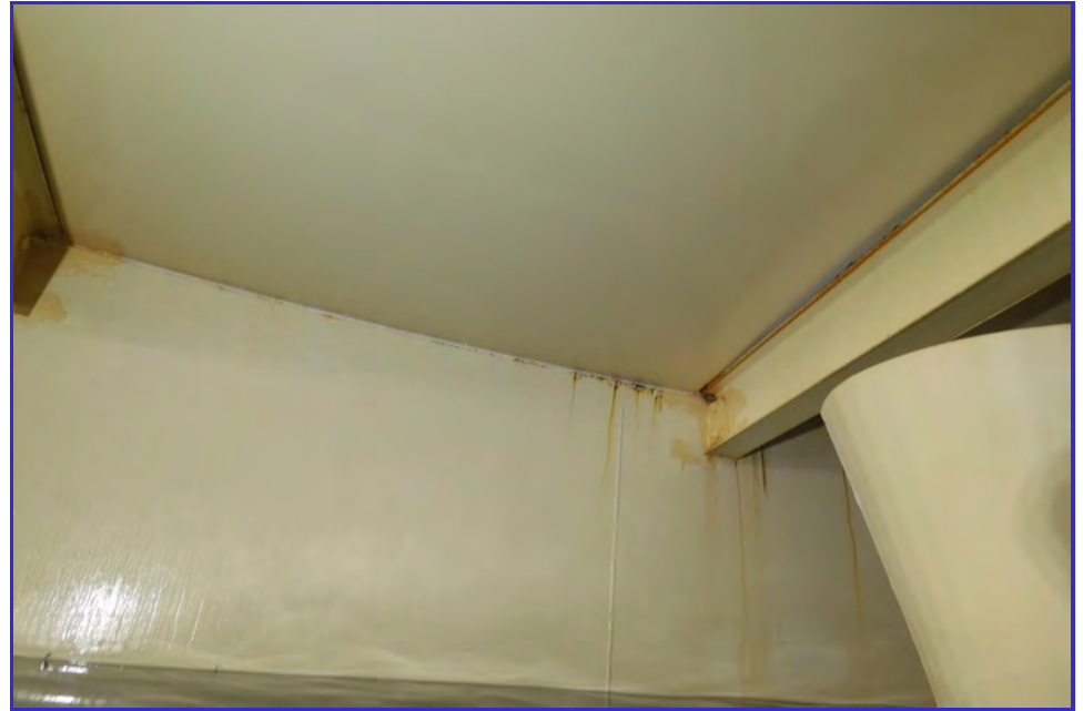
INTERIOR - CPUD - Railroad Flat Reservoir - Maintenance Inspection -013
