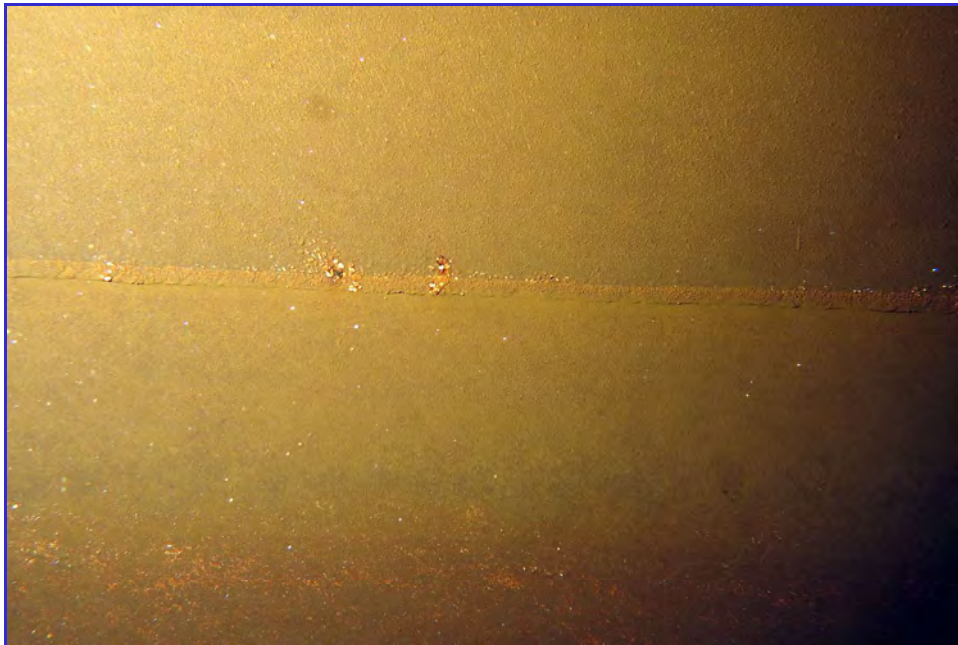
INTERIOR - Calaveras Public Utility District - Clear Well Tank - Maintenance Inspection -090
