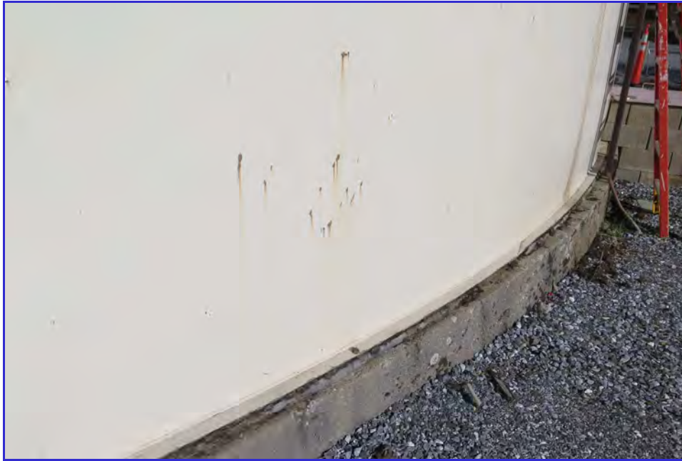
EXTERIOR - Calaveras Public Utility District - Clear Well Tank - Maintenance Inspection -060
