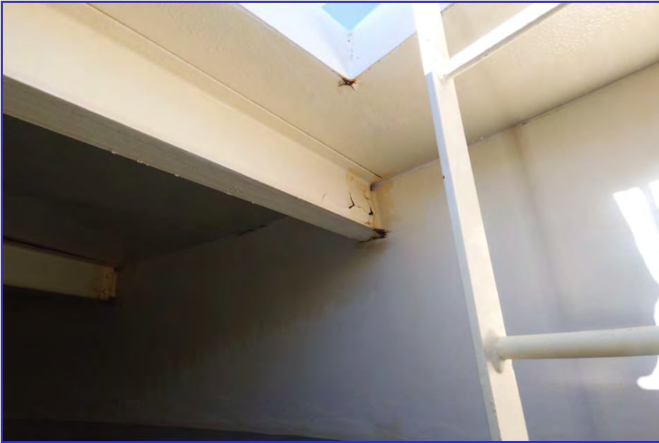
INTERIOR - CPUD - Railroad Flat Reservoir - Maintenance Inspection
