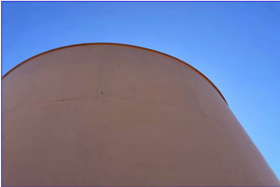
EXTERIOR - CPUD - Paloma Reservoir - Maintenance Inspection -038
