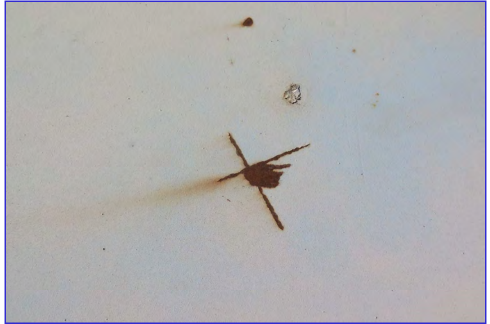
EXTERIOR - Calaveras Public Utility District - Clear Well Tank - Maintenance Inspection -053
