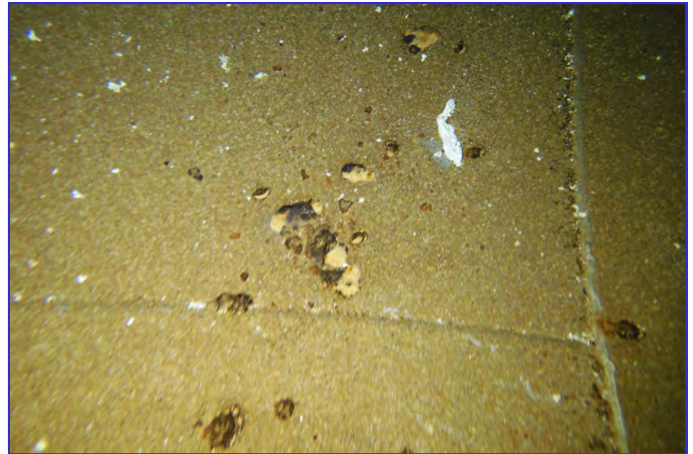
INTERIOR - CPUD - San Andaras Reservoir - Maintenance Inspection -175
