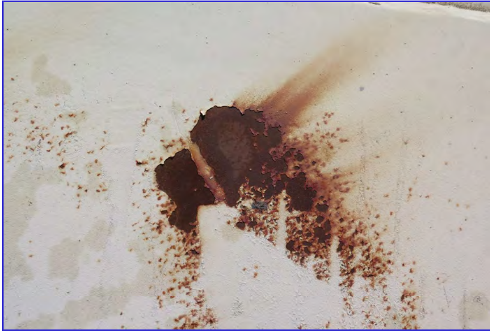
EXTERIOR - Calaveras Public Utility District - Clear Well Tank - Maintenance Inspection -032
