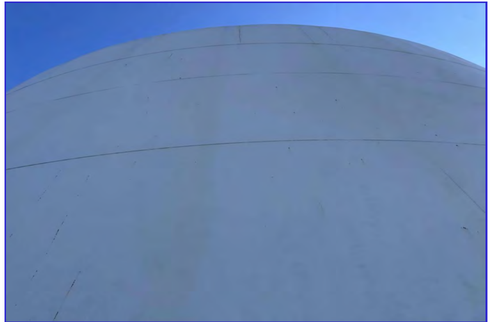
EXTERIOR - CPUD - San Andreas Reservoir - Maintenance Inspection -179
