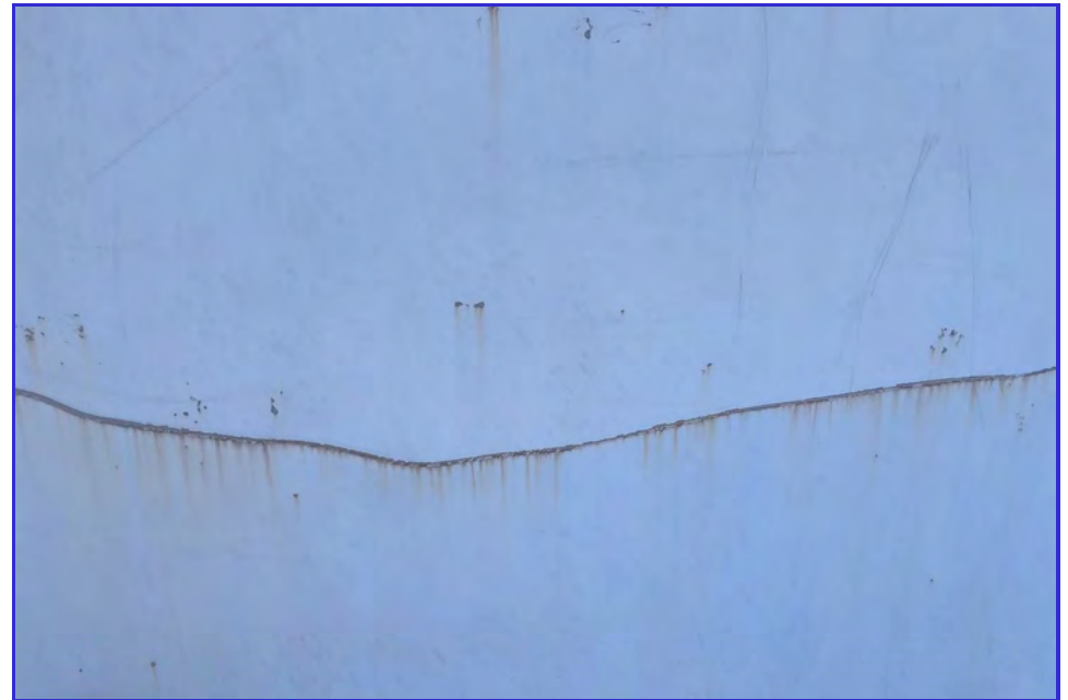
EXTERIOR - CPUD - San Andreas Reservoir - Maintenance Inspection -107
