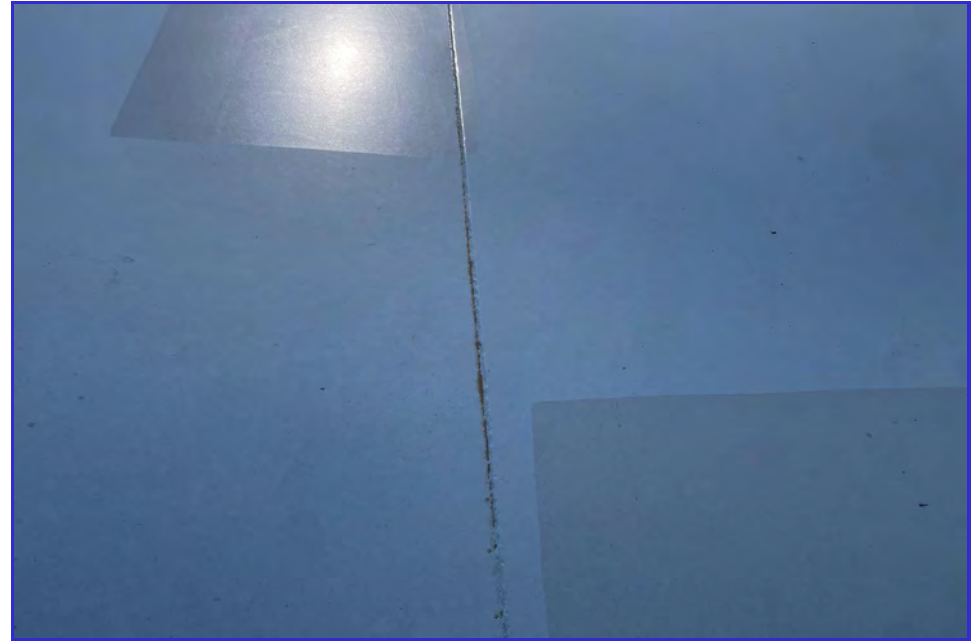
EXTERIOR - CPUD - Railroad Flat Reservoir - Maintenance Inspection -025
