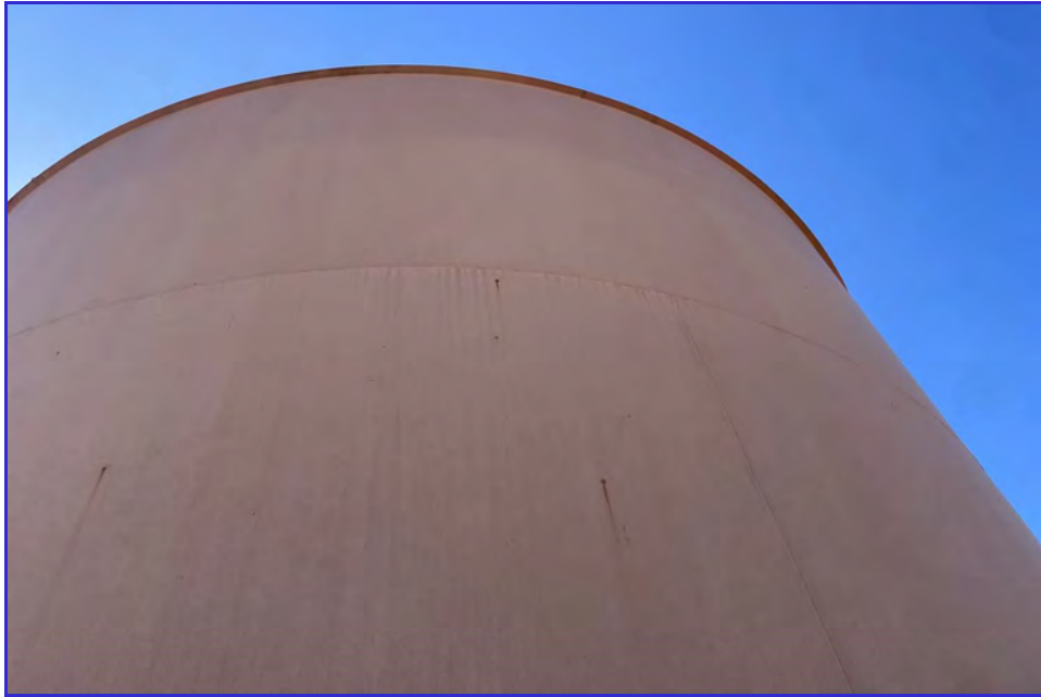
EXTERIOR - CPUD - Paloma Reservoir - Maintenance Inspection -036
