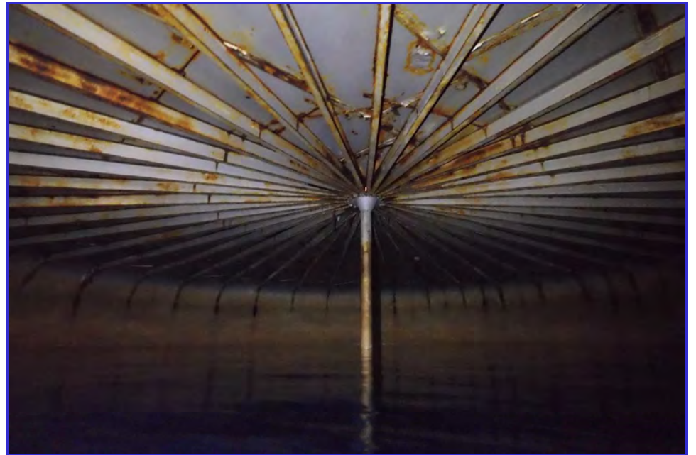
INTERIOR - CPUD - Mokelumne Hill Reservoir - Maintenance Inspection -007
