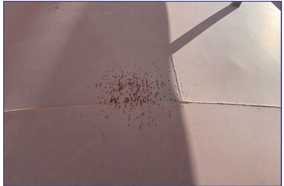
EXTERIOR - CPUD - Paloma Reservoir - Maintenance Inspection -047
