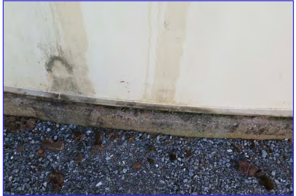
EXTERIOR - Calaveras Public Utility District - Clear Well Tank - Maintenance Inspection -113
