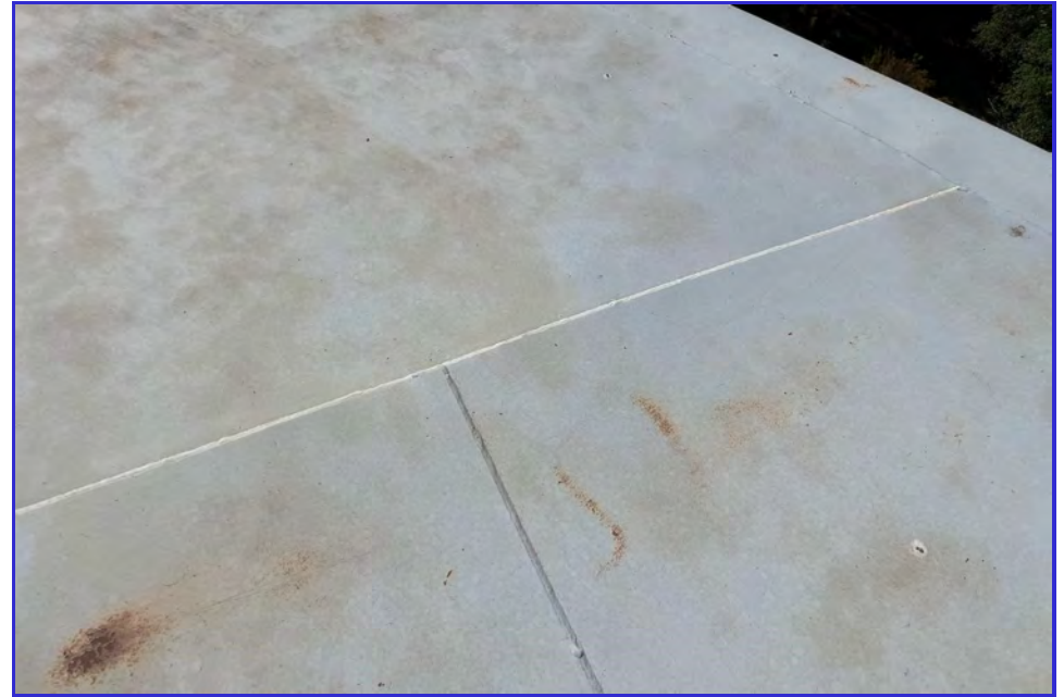
EXTERIOR - CPUD - San Andreas Reservoir - Maintenance Inspection -041
