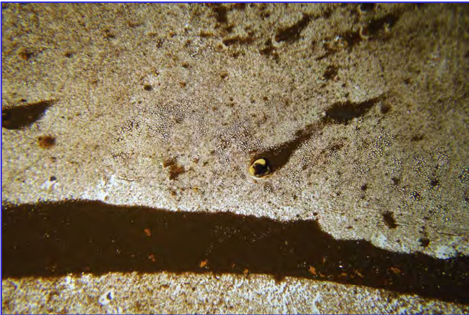
INTERIOR - CPUD - Mokelumne Hill Reservoir - Maintenance Inspection -150
