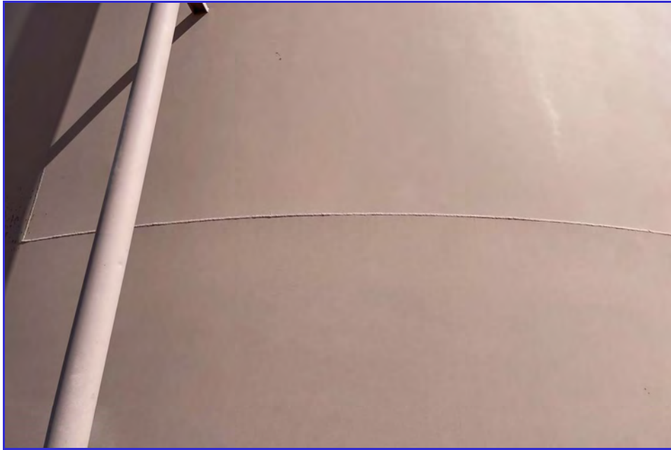
EXTERIOR - CPUD - Paloma Reservoir - Maintenance Inspection -076
