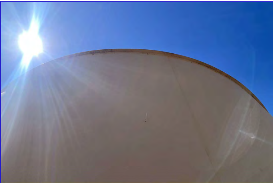
EXTERIOR - CPUD - Golden Hills - Maintenance Inspection -050
