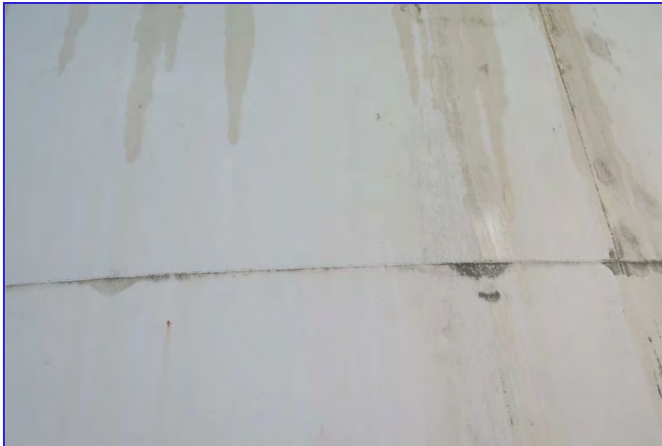
EXTERIOR - Calaveras Public Utility District - Clear Well Tank - Maintenance Inspection -114
