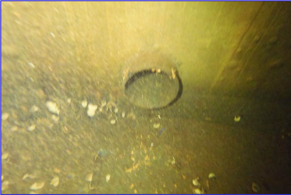
INTERIOR - CPUD - Golden Hills - Maintenance Inspection -080
