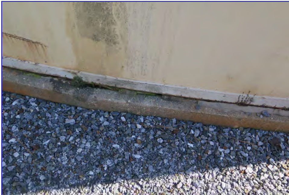
EXTERIOR - Calaveras Public Utility District - Clear Well Tank - Maintenance Inspection -086
