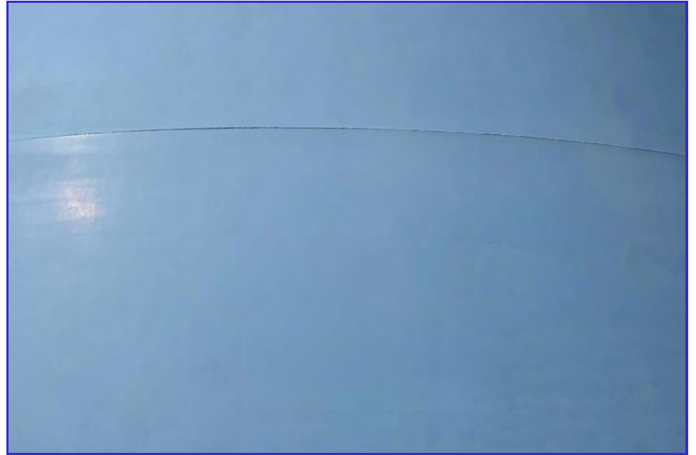
EXTERIOR - CPUD - Railroad Flat Reservoir - Maintenance Inspection -049
