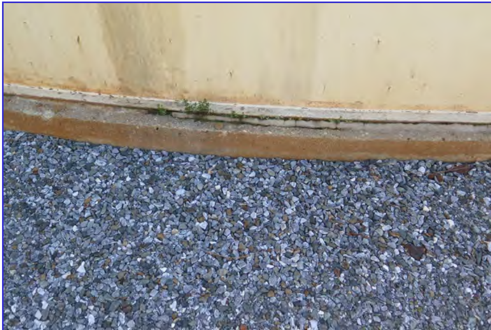
EXTERIOR - Calaveras Public Utility District - Clear Well Tank - Maintenance Inspection -090
