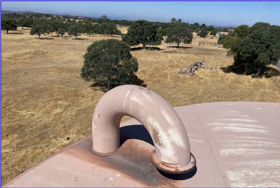
EXTERIOR - CPUD - Paloma Reservoir - Maintenance Inspection -028
