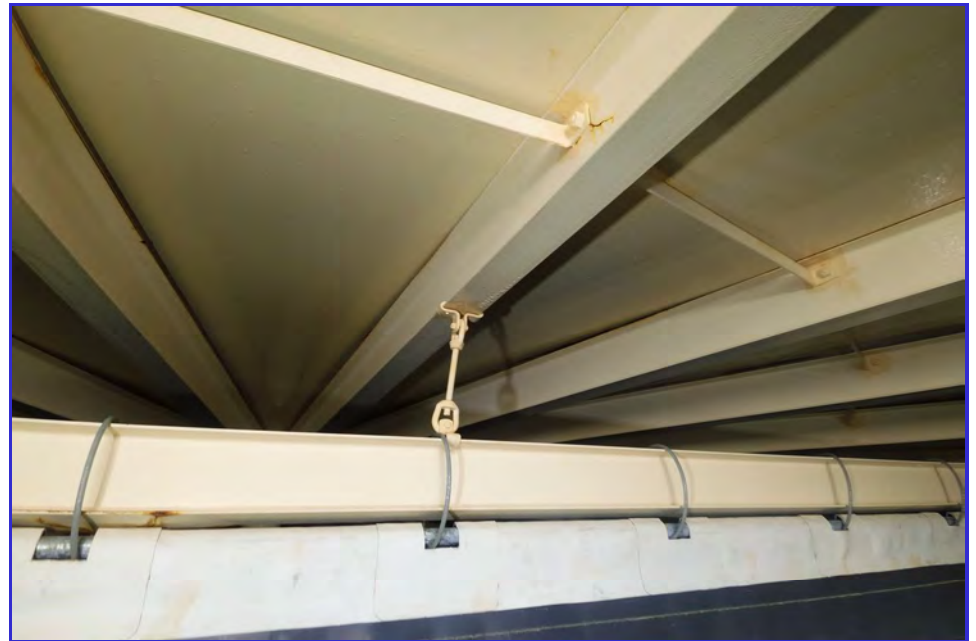
INTERIOR - CPUD - Railroad Flat Reservoir - Maintenance Inspection -007
