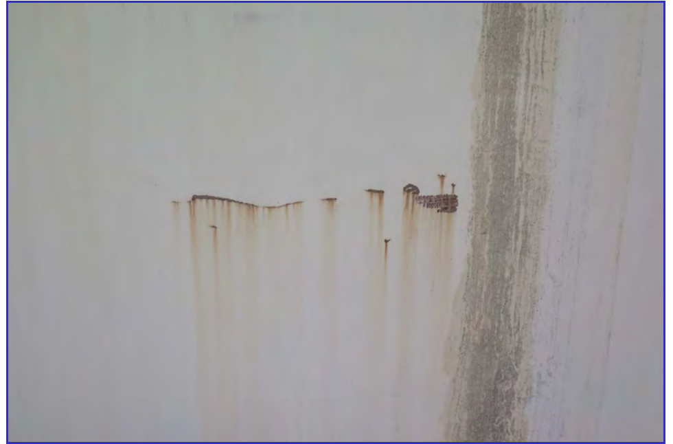
EXTERIOR - Calaveras Public Utility District - Clear Well Tank - Maintenance Inspection -089
