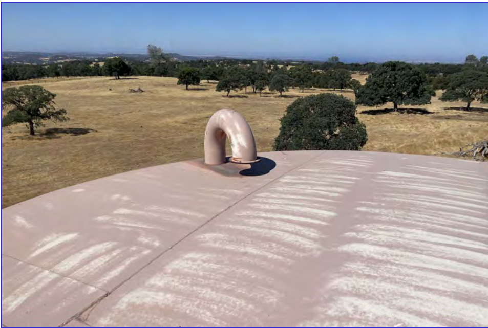
EXTERIOR - CPUD - Paloma Reservoir - Maintenance Inspection -010
