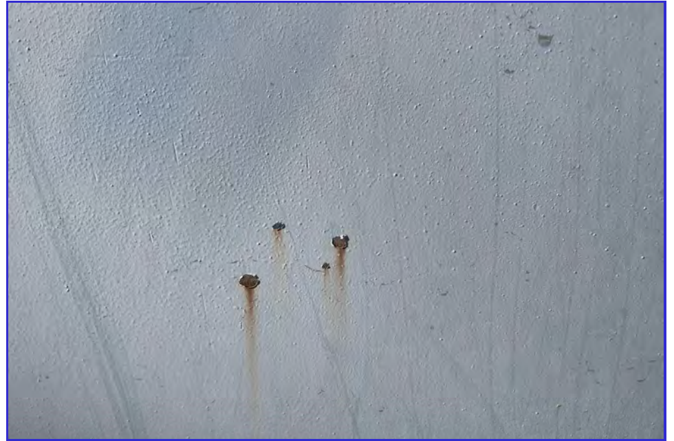
EXTERIOR - CPUD - Mokelumne Reservoir - Maintenance Inspection -085
