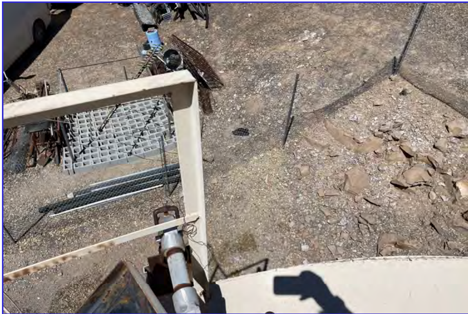
EXTERIOR - CPUD - Golden Hills - Maintenance Inspection -018
