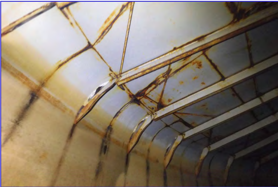
INTERIOR - CPUD - Mokelumne Hill Reservoir - Maintenance Inspection -002
