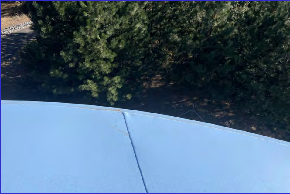
EXTERIOR - CPUD - Railroad Flat Reservoir - Maintenance Inspection -012
