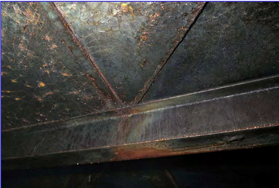
INTERIOR - Calaveras Public Utility District - Clear Well Tank - Maintenance Inspection -050
