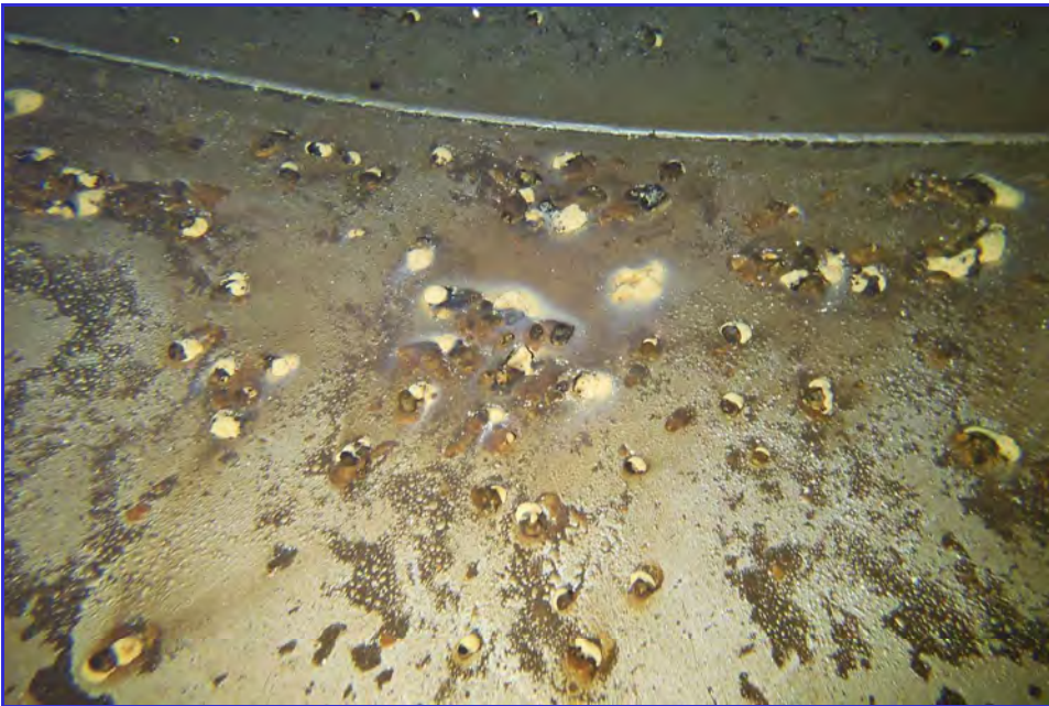
INTERIOR - CPUD - San Andaras Reservoir - Maintenance Inspection -182
