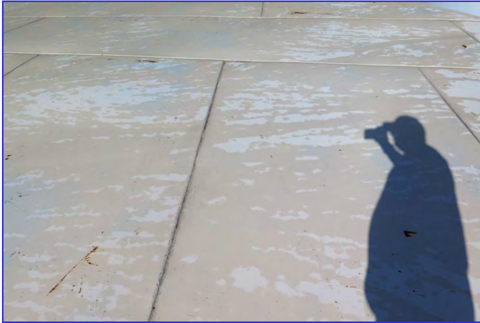
EXTERIOR - Calaveras Public Utility District - Clear Well Tank - Maintenance Inspection -008
