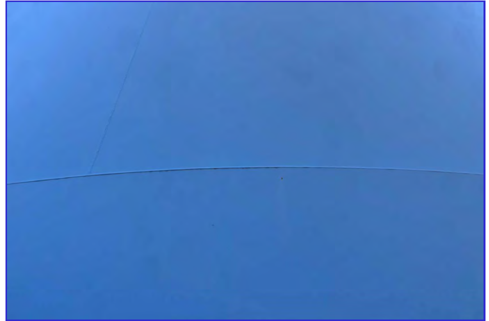
EXTERIOR - CPUD - Railroad Flat Reservoir - Maintenance Inspection -061
