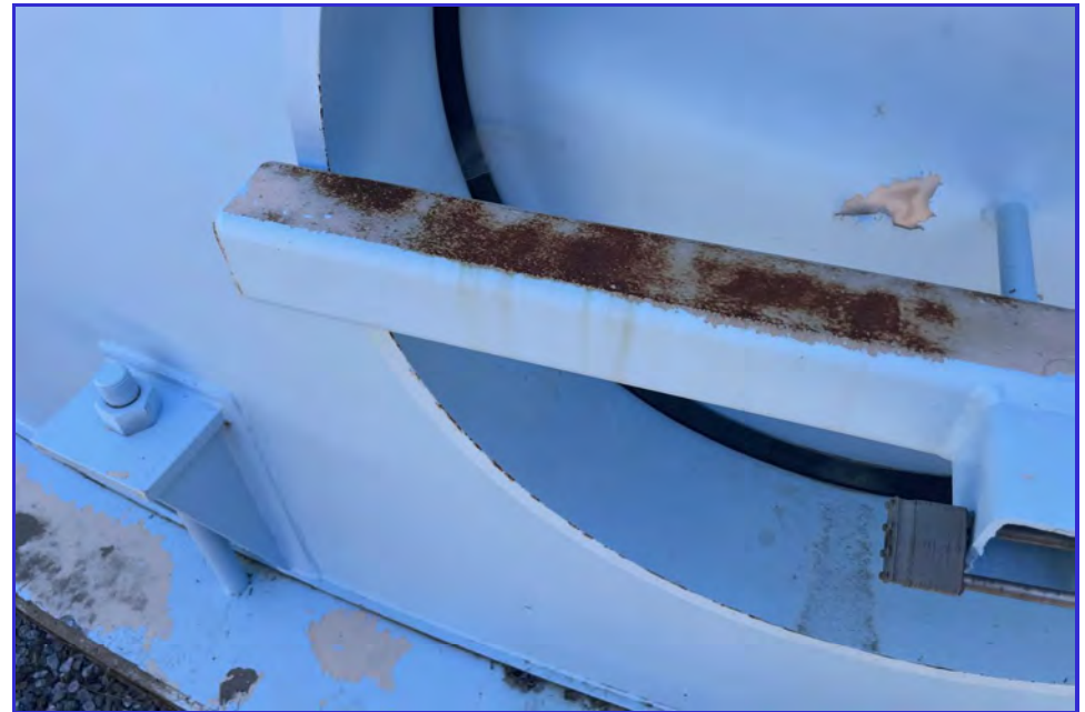
EXTERIOR - CPUD - Railroad Flat Reservoir - Maintenance Inspection -075
