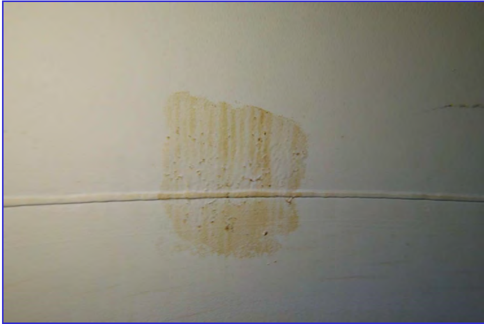
INTERIOR - CPUD - Railroad Flat Reservoir - Maintenance Inspection -068
