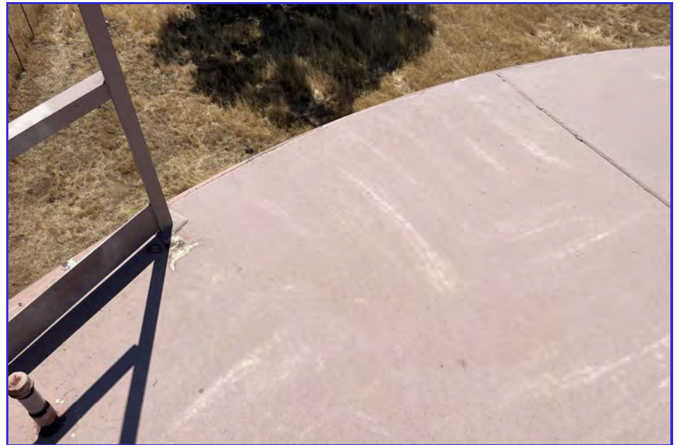
EXTERIOR - CPUD - Paloma Reservoir - Maintenance Inspection -007
