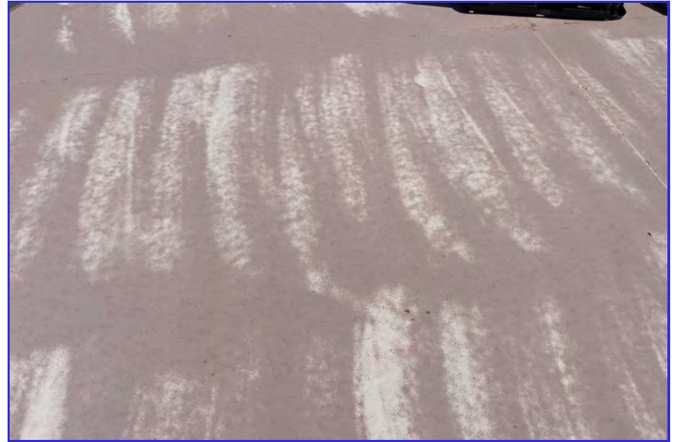
EXTERIOR - CPUD - Paloma Reservoir - Maintenance Inspection -013
