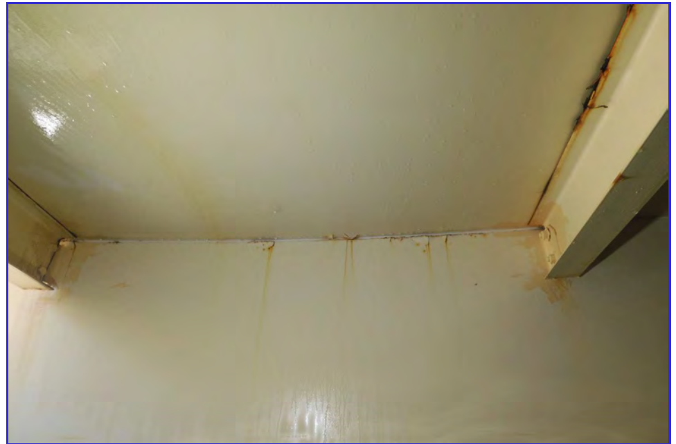
INTERIOR - CPUD - Railroad Flat Reservoir - Maintenance Inspection -011
