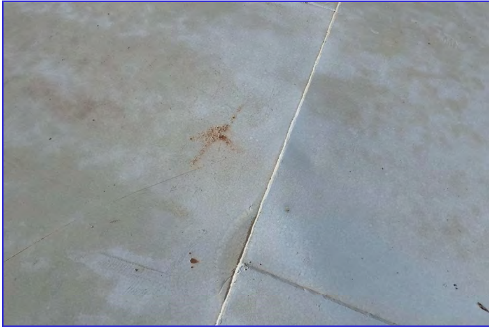
EXTERIOR - CPUD - San Andreas Reservoir - Maintenance Inspection -072
