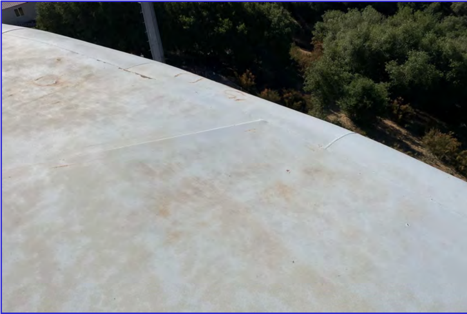
EXTERIOR - CPUD - San Andreas Reservoir - Maintenance Inspection -040
