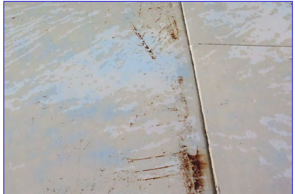
EXTERIOR - Calaveras Public Utility District - Clear Well Tank - Maintenance Inspection -019
