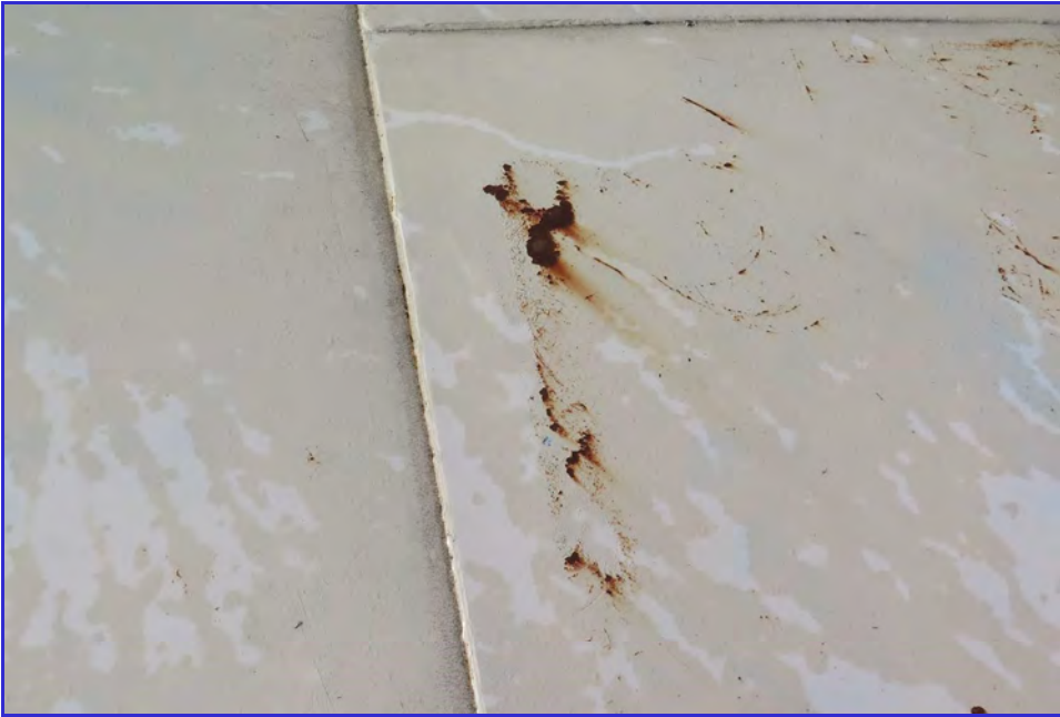
EXTERIOR - Calaveras Public Utility District - Clear Well Tank - Maintenance Inspection -012
