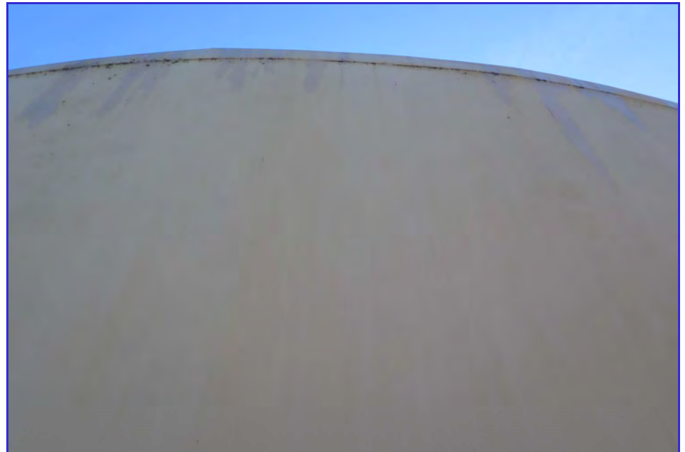
EXTERIOR - Calaveras Public Utility District - Clear Well Tank - Maintenance Inspection -099
