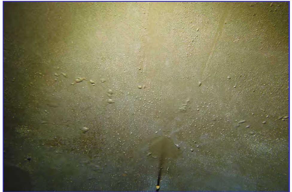
INTERIOR - CPUD - San Andaras Reservoir - Maintenance Inspection -139
