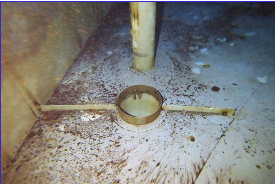
INTERIOR - CPUD - Mokelumne Hill Reservoir - Maintenance Inspection -106
