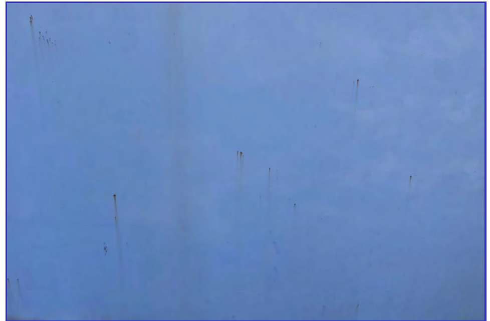
EXTERIOR - CPUD - Mokelumne Reservoir - Maintenance Inspection -115
