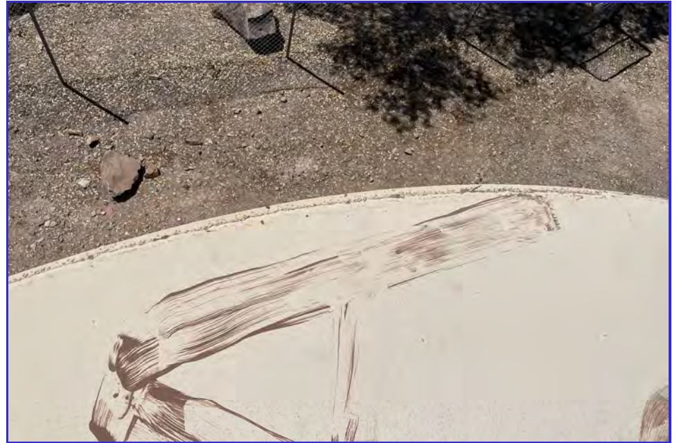
EXTERIOR - CPUD - Golden Hills - Maintenance Inspection -015
