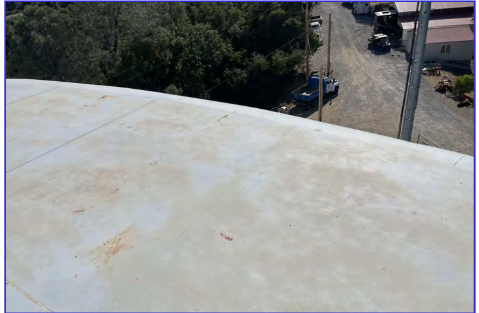
EXTERIOR - CPUD - San Andreas Reservoir - Maintenance Inspection -097
