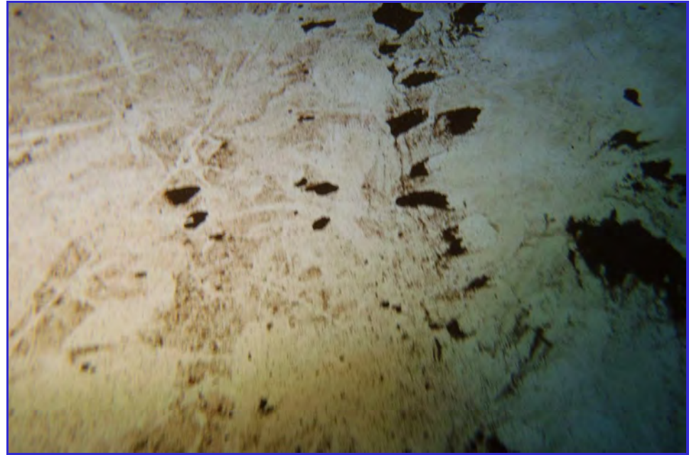
INTERIOR - CPUD - Railroad Flat Reservoir - Maintenance Inspection -165
