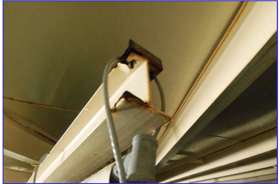
INTERIOR - CPUD - Railroad Flat Reservoir - Maintenance Inspection -025
