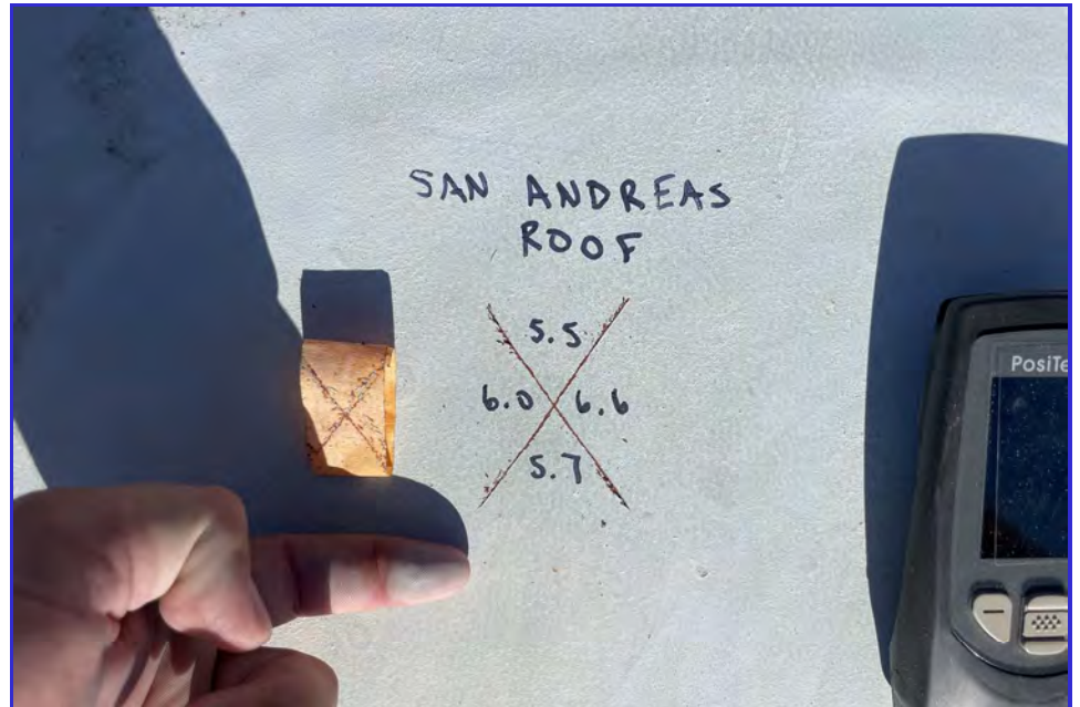
EXTERIOR - CPUD - San Andreas Reservoir - Maintenance Inspection -099
