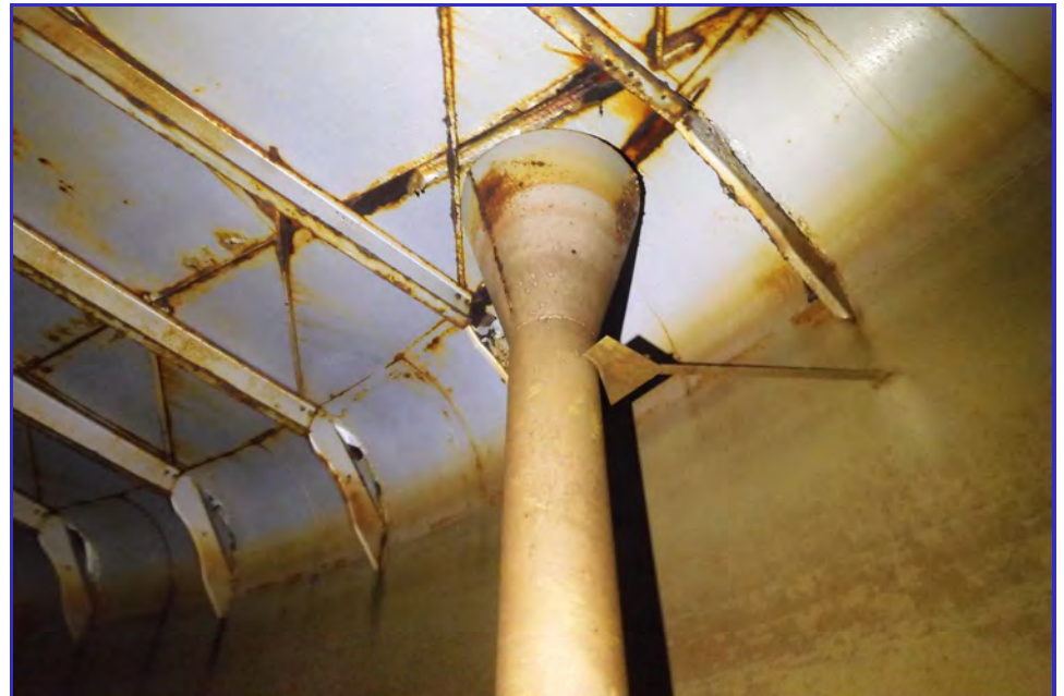
INTERIOR - CPUD - Mokelumne Hill Reservoir - Maintenance Inspection -011
