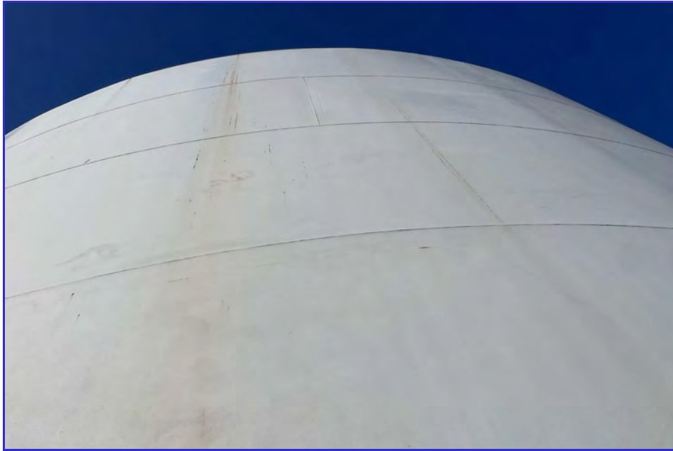
EXTERIOR - CPUD - Mokelumne Reservoir - Maintenance Inspection -088
