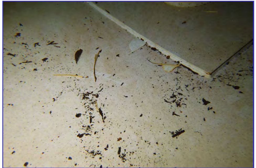
INTERIOR - CPUD - Railroad Flat Reservoir - Maintenance Inspection -135
