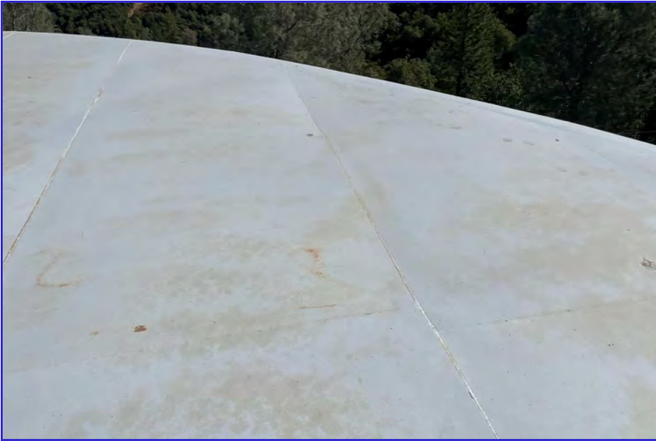
EXTERIOR - CPUD - San Andreas Reservoir - Maintenance Inspection -092
