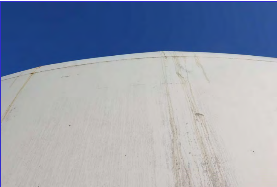
EXTERIOR - Calaveras Public Utility District - Clear Well Tank - Maintenance Inspection -074
