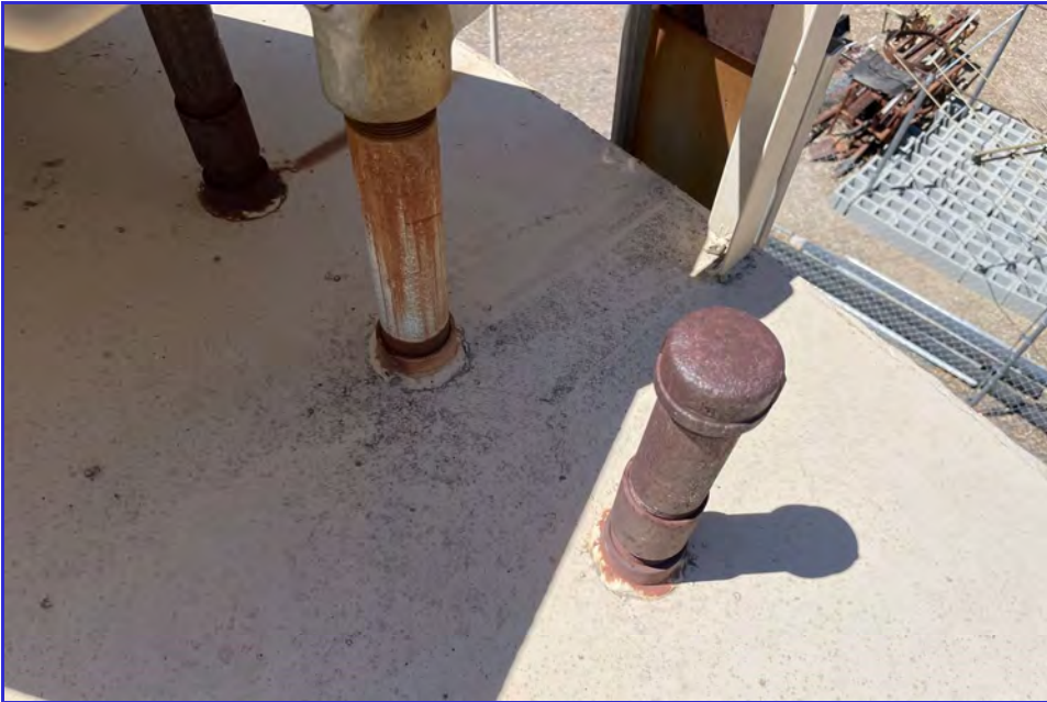
EXTERIOR - CPUD - Golden Hills - Maintenance Inspection -028
