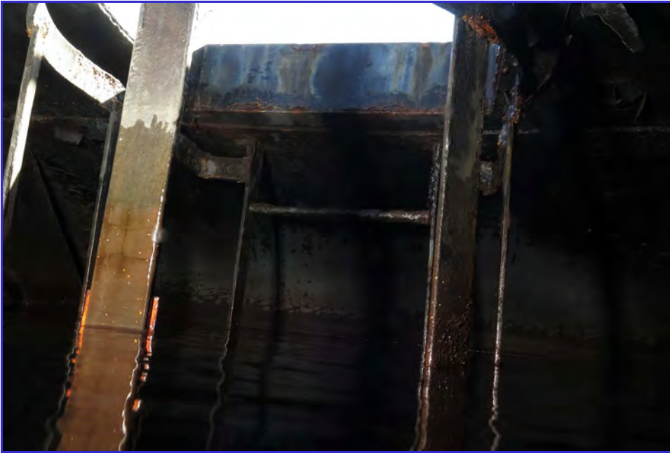
INTERIOR - Calaveras Public Utility District - Clear Well Tank - Maintenance Inspection
