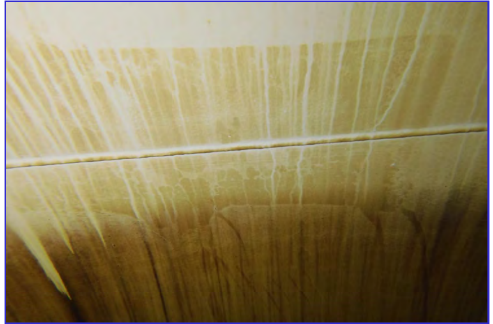
INTERIOR - CPUD - Railroad Flat Reservoir - Maintenance Inspection -077
