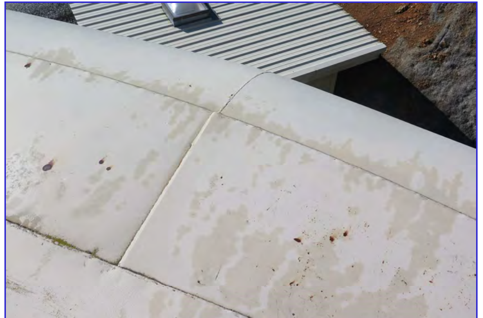
EXTERIOR - Calaveras Public Utility District - Clear Well Tank - Maintenance Inspection -027
