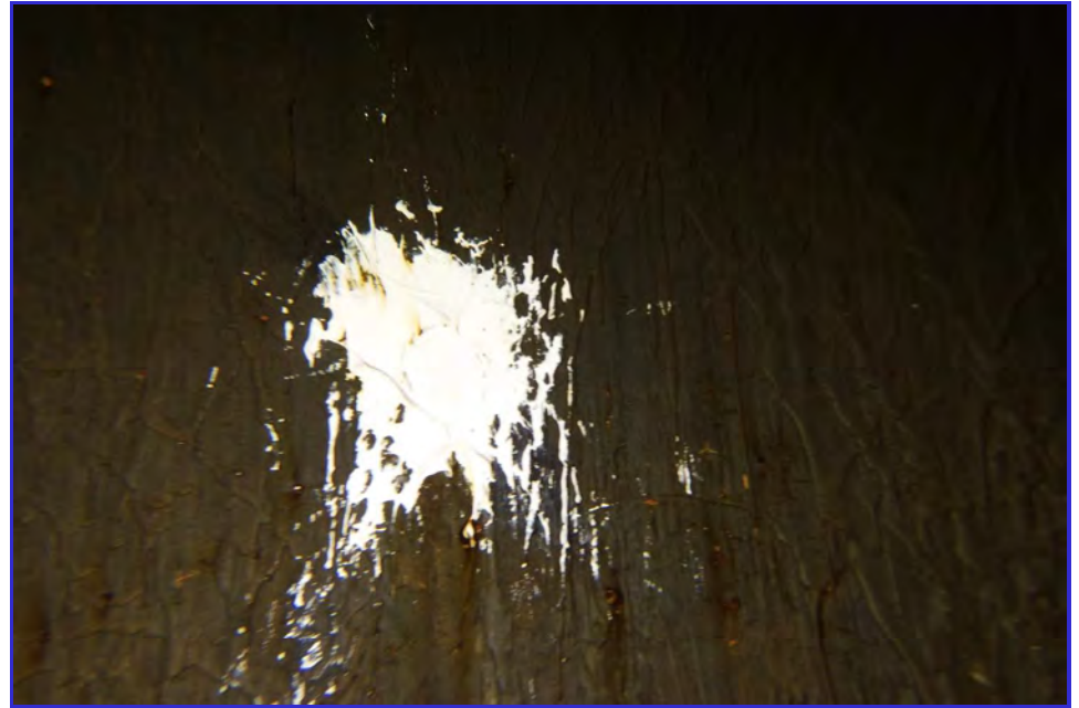
INTERIOR - CPUD - Paloma Reservoir - Maintenance Inspection -101
