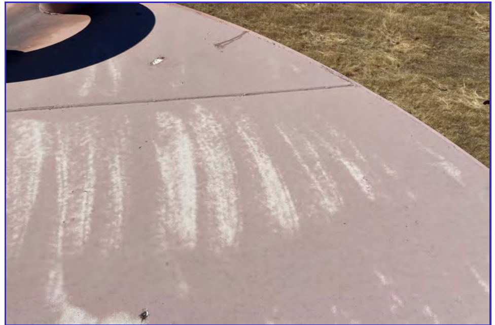
EXTERIOR - CPUD - Paloma Reservoir - Maintenance Inspection -019
