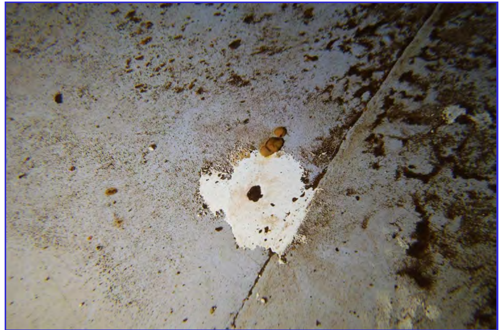
INTERIOR - CPUD - Mokelumne Hill Reservoir - Maintenance Inspection -159
