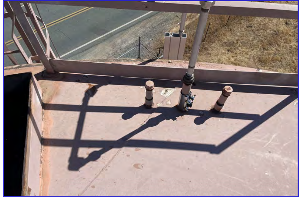
EXTERIOR - CPUD - Paloma Reservoir - Maintenance Inspection -005
