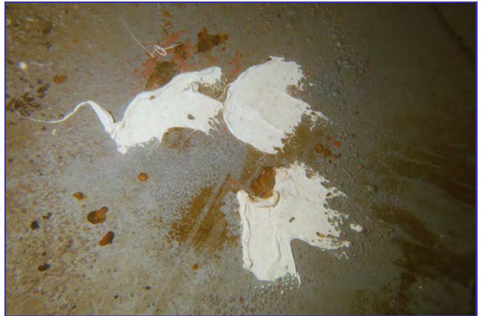
INTERIOR - CPUD - San Andaras Reservoir - Maintenance Inspection -251
