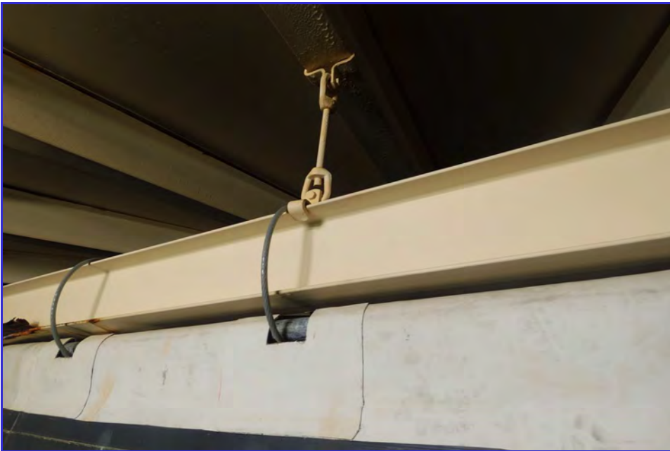
INTERIOR - CPUD - Railroad Flat Reservoir - Maintenance Inspection -018
