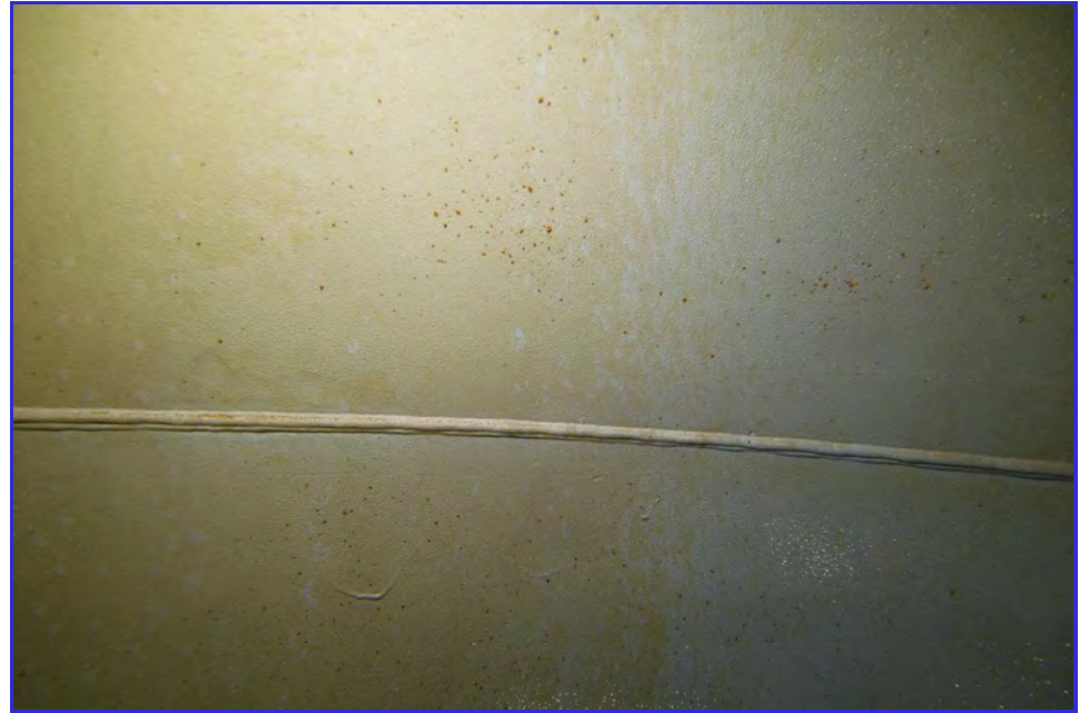
INTERIOR - CPUD - Mokelumne Hill Reservoir - Maintenance Inspection -105
