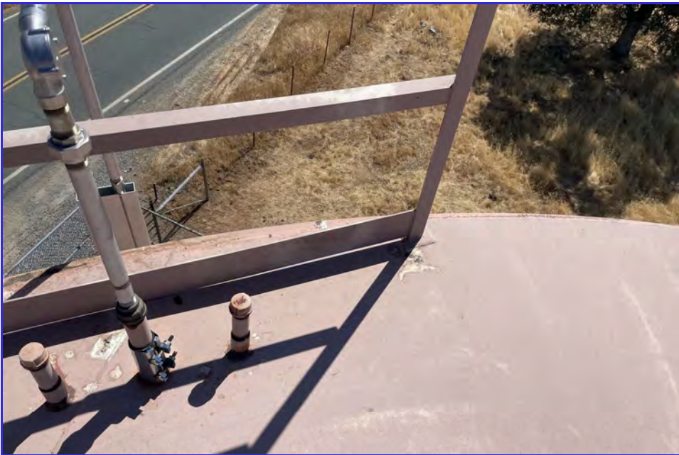
EXTERIOR - CPUD - Paloma Reservoir - Maintenance Inspection -002
