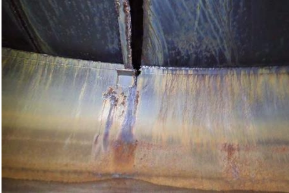
Figure 9-7. Example of Paloma Tank Interior Roof
