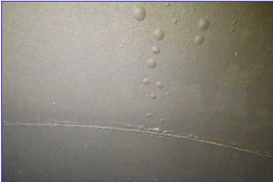
INTERIOR - CPUD - Paloma Reservoir - Maintenance Inspection -050
