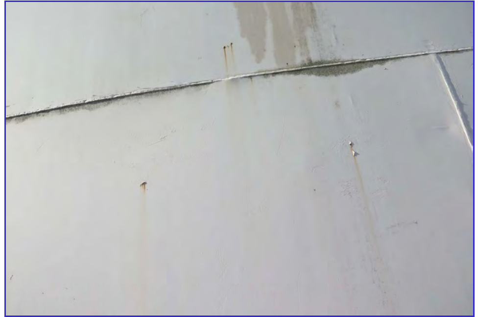
EXTERIOR - Calaveras Public Utility District - Clear Well Tank - Maintenance Inspection -117
