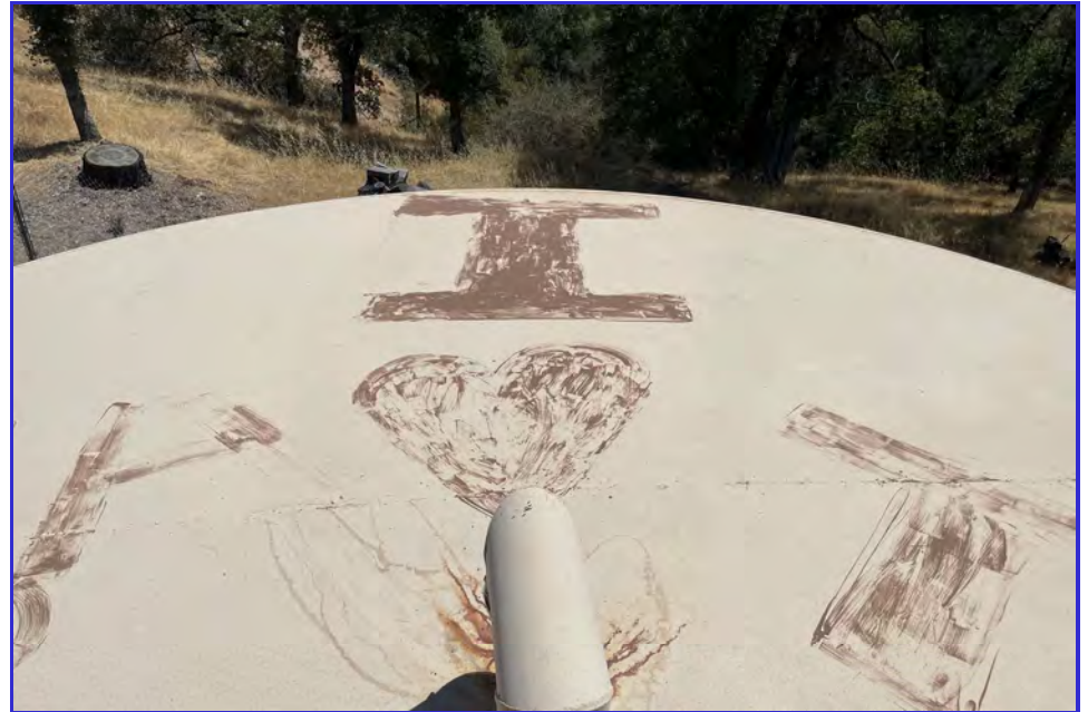
EXTERIOR - CPUD - Golden Hills - Maintenance Inspection -017
