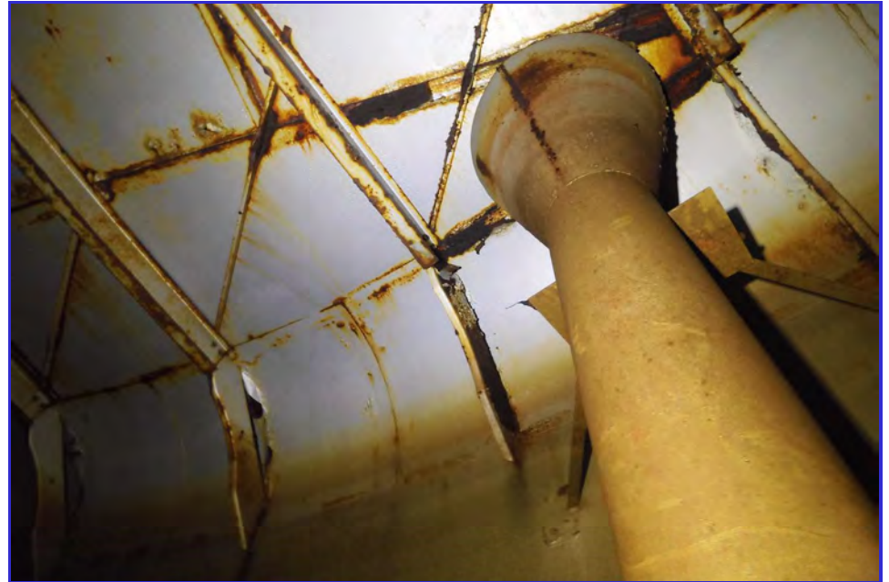
INTERIOR - CPUD - Mokelumne Hill Reservoir - Maintenance Inspection -013
