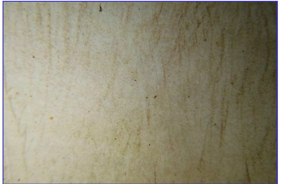
INTERIOR - CPUD - Railroad Flat Reservoir - Maintenance Inspection -111
