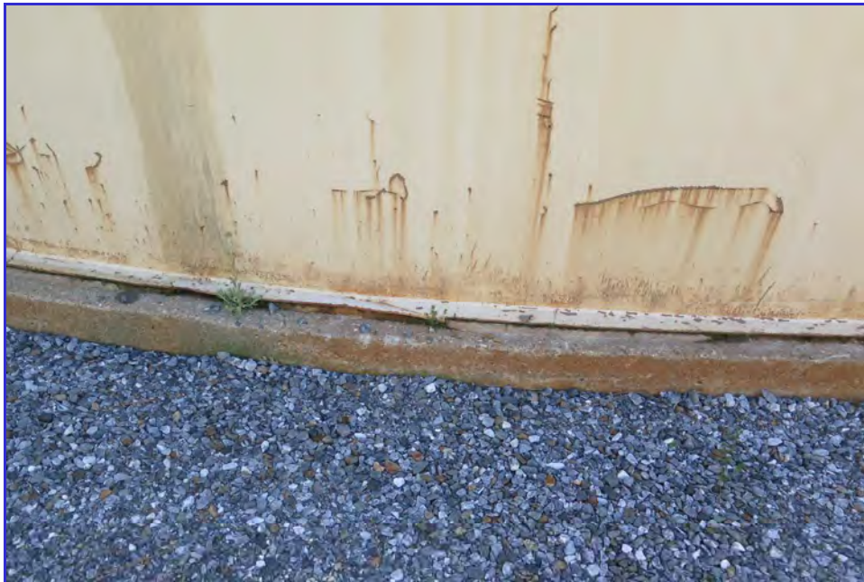
EXTERIOR - Calaveras Public Utility District - Clear Well Tank - Maintenance Inspection -094
