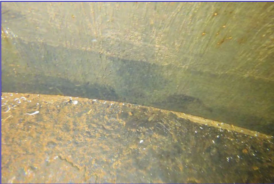
INTERIOR - CPUD - Paloma Reservoir - Maintenance Inspection -102
