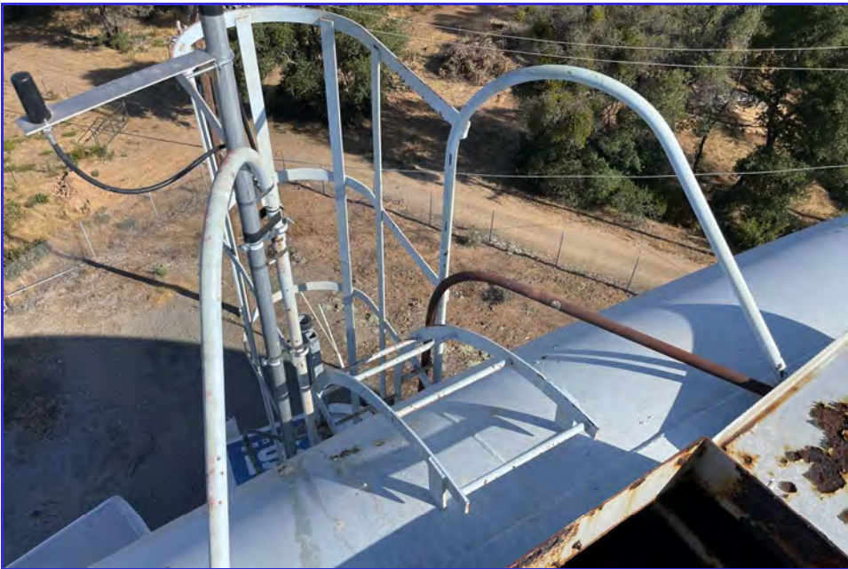
EXTERIOR - CPUD - San Andreas Reservoir - Maintenance Inspection -002
