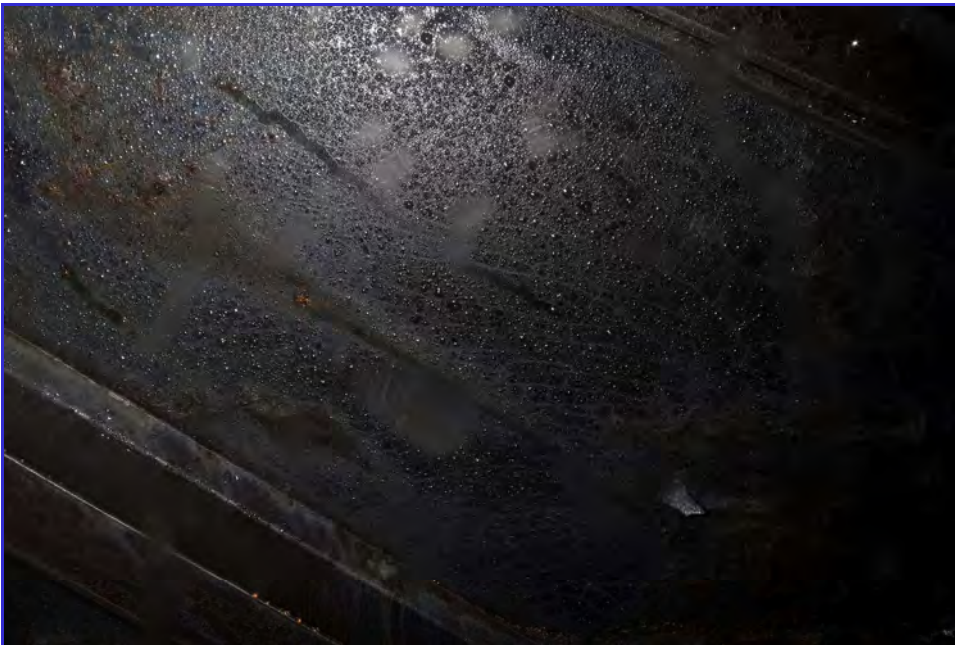
INTERIOR - Calaveras Public Utility District - Clear Well Tank - Maintenance Inspection -010
