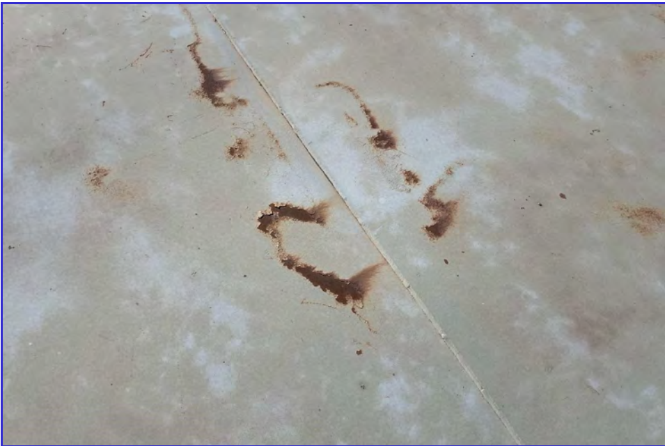
EXTERIOR - CPUD - San Andreas Reservoir - Maintenance Inspection -082
