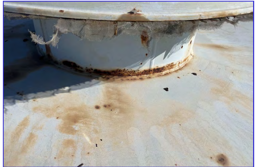
EXTERIOR - CPUD - San Andreas Reservoir - Maintenance Inspection -087
