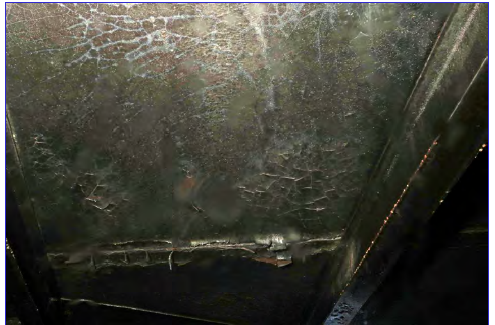
INTERIOR - Calaveras Public Utility District - Clear Well Tank - Maintenance Inspection -007
