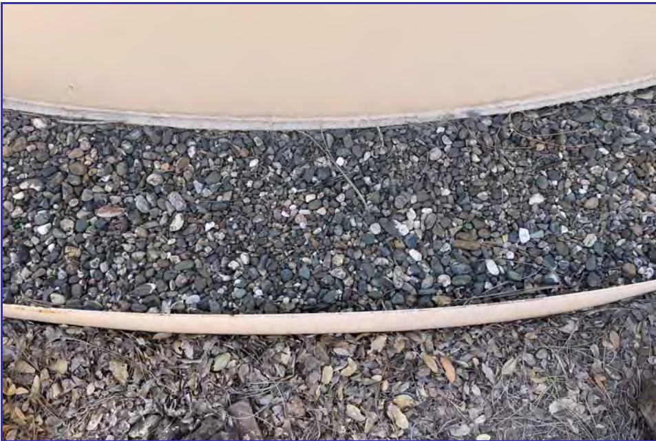
EXTERIOR - CPUD - Golden Hills - Maintenance Inspection -054
