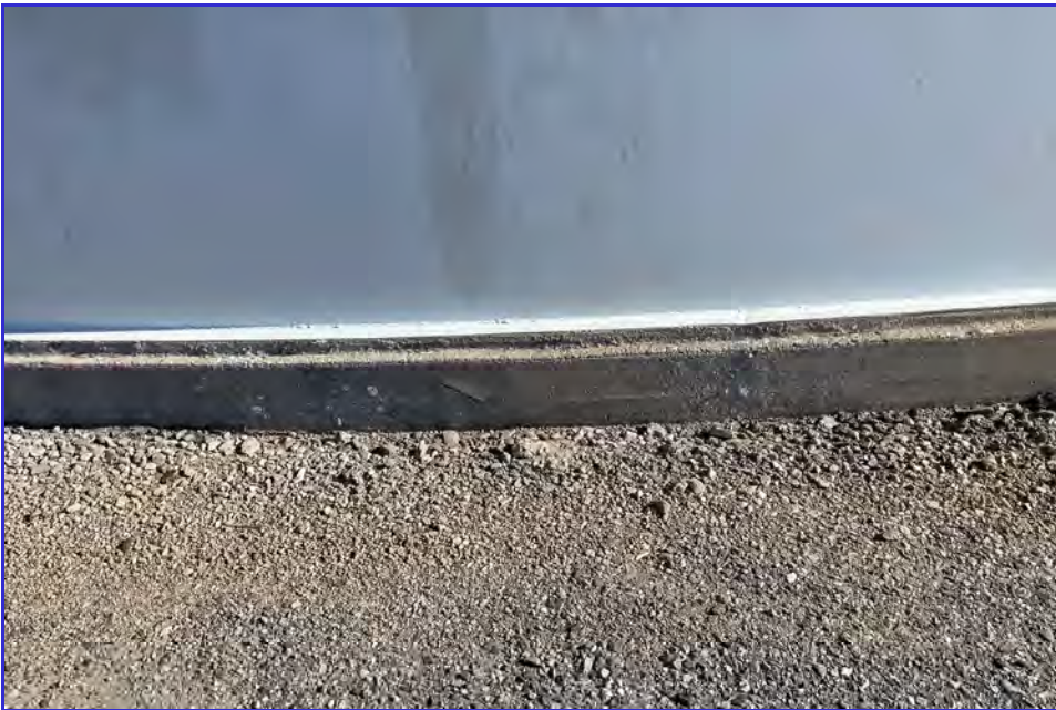
EXTERIOR - CPUD - San Andreas Reservoir - Maintenance Inspection -182
