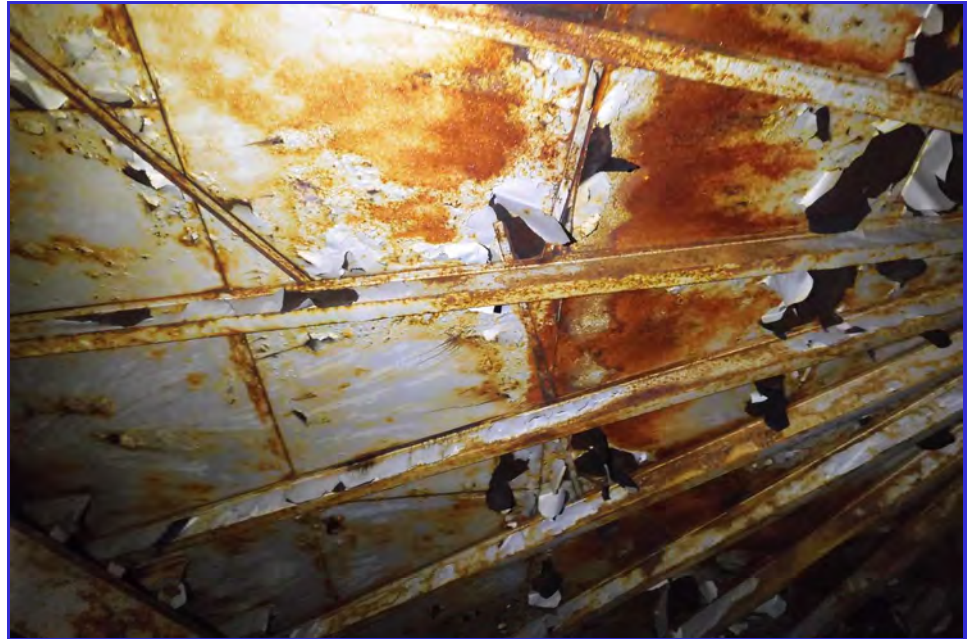
INTERIOR - CPUD - San Andaras Reservoir - Maintenance Inspection -077
