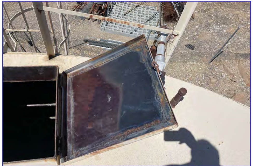
EXTERIOR - CPUD - Golden Hills - Maintenance Inspection -023
