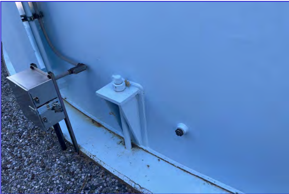
EXTERIOR - CPUD - Railroad Flat Reservoir - Maintenance Inspection -066
