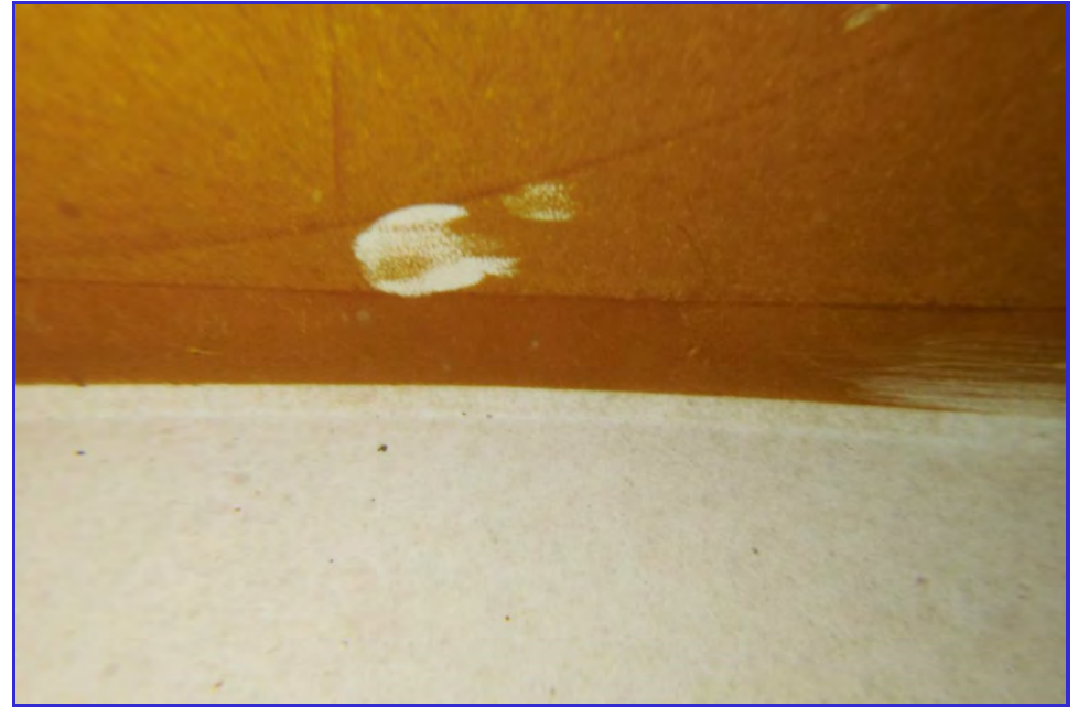
INTERIOR - CPUD - Railroad Flat Reservoir - Maintenance Inspection -113
