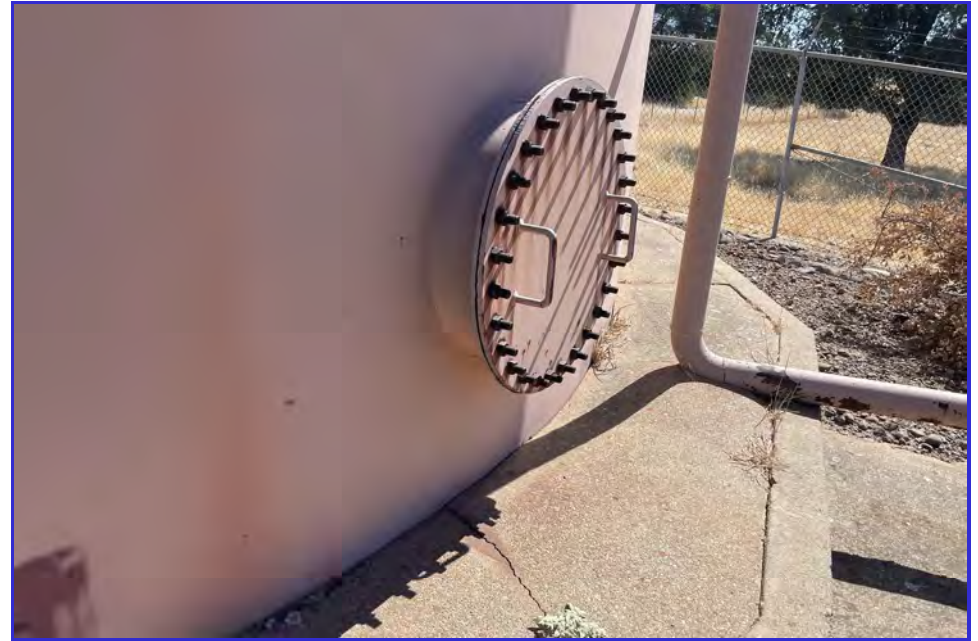
EXTERIOR - CPUD - Paloma Reservoir - Maintenance Inspection -045
