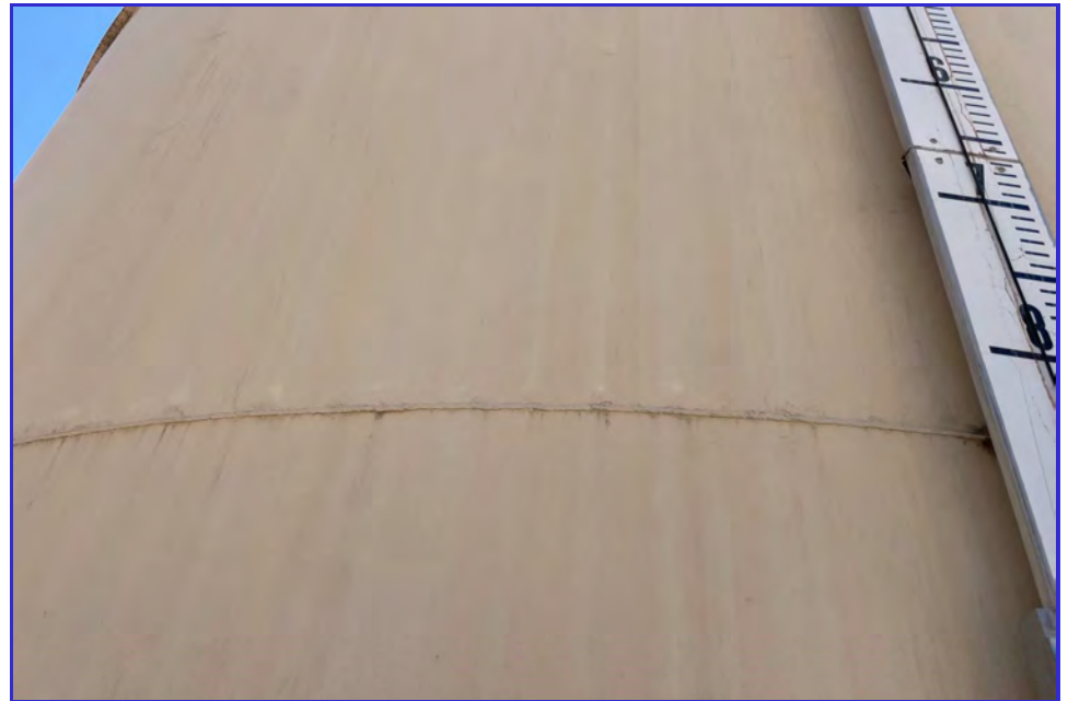
EXTERIOR - CPUD - Golden Hills - Maintenance Inspection -059
