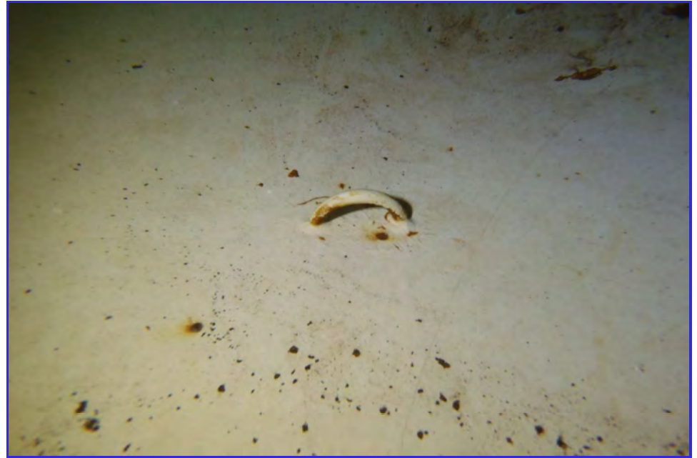
INTERIOR - CPUD - Railroad Flat Reservoir - Maintenance Inspection -161
