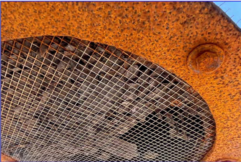
EXTERIOR - CPUD - Paloma Reservoir - Maintenance Inspection -030
