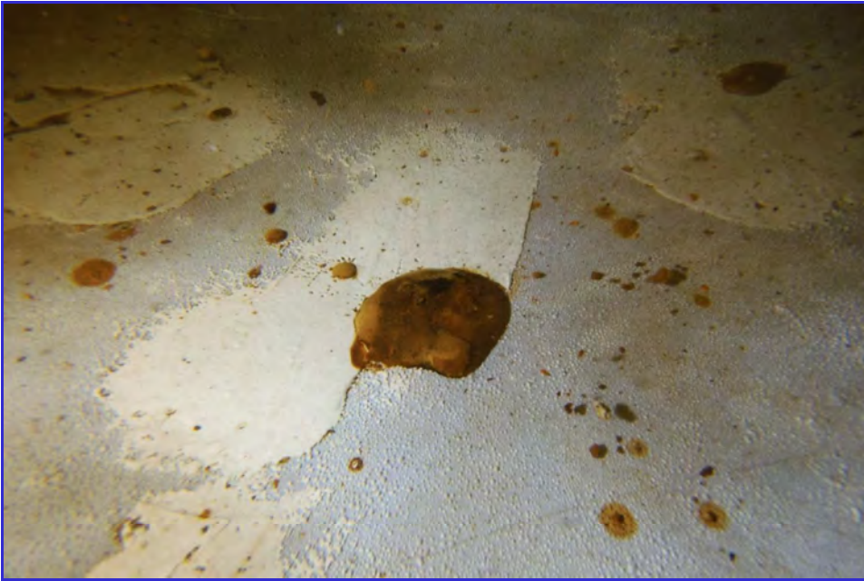
INTERIOR - CPUD - Mokelumne Hill Reservoir - Maintenance Inspection -152
