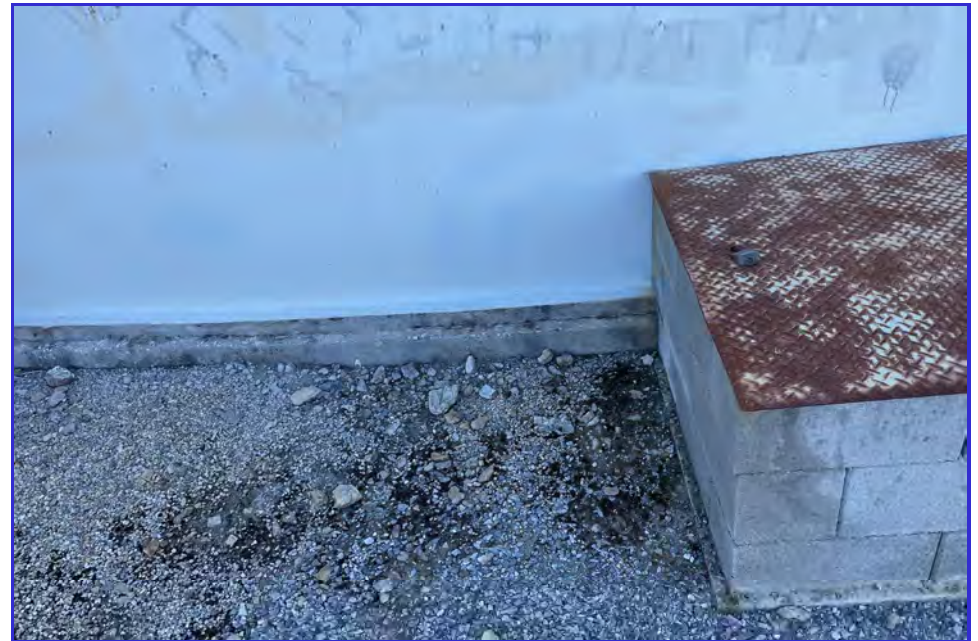
EXTERIOR - CPUD - San Andreas Reservoir - Maintenance Inspection -175
