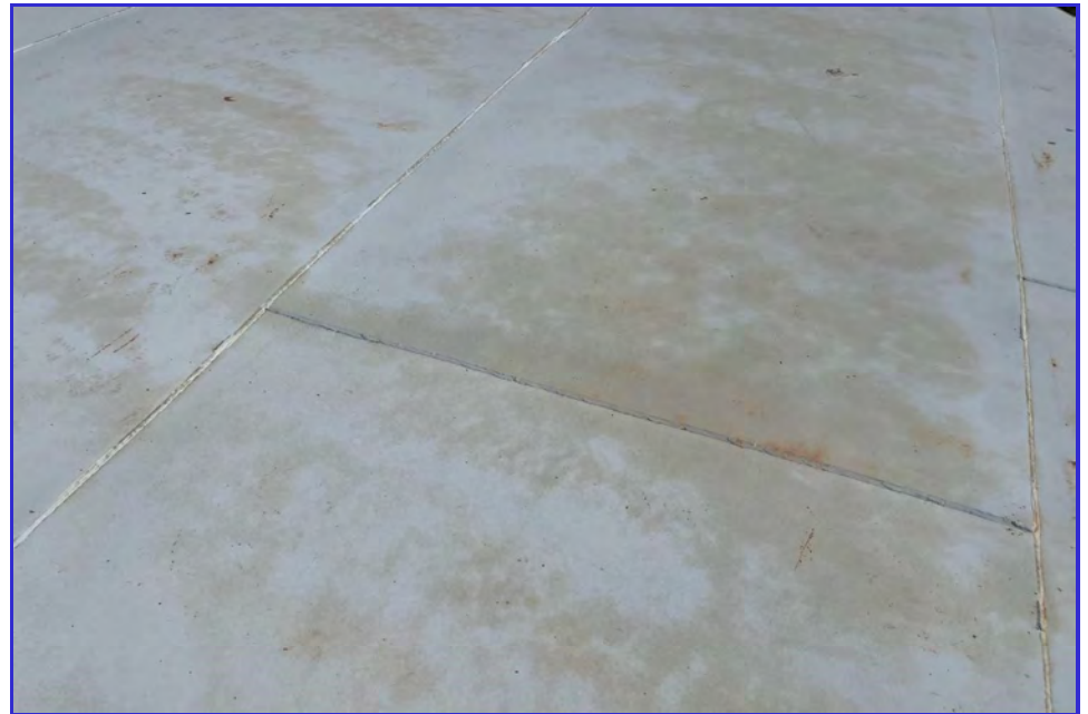
EXTERIOR - CPUD - San Andreas Reservoir - Maintenance Inspection -055
