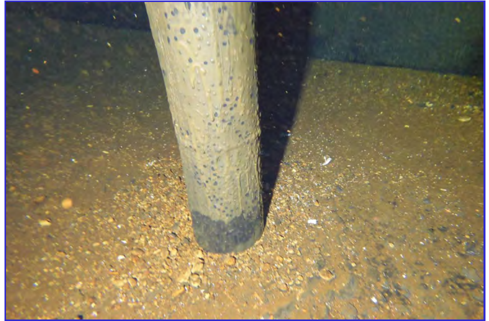
INTERIOR - CPUD - Paloma Reservoir - Maintenance Inspection -113
