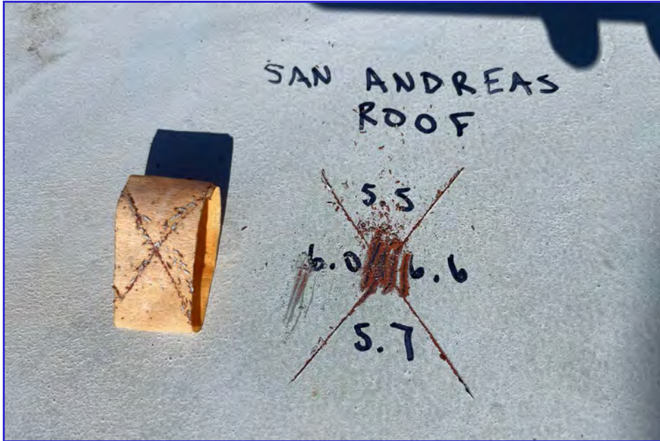
EXTERIOR - CPUD - San Andreas Reservoir - Maintenance Inspection -100
