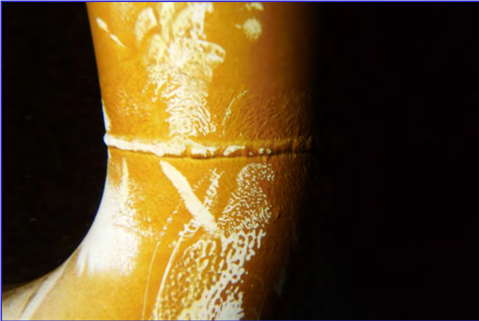
INTERIOR - CPUD - Railroad Flat Reservoir - Maintenance Inspection -168
