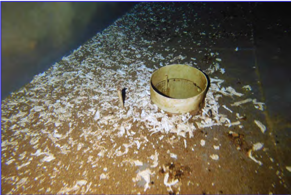
INTERIOR - CPUD - San Andaras Reservoir - Maintenance Inspection -206
