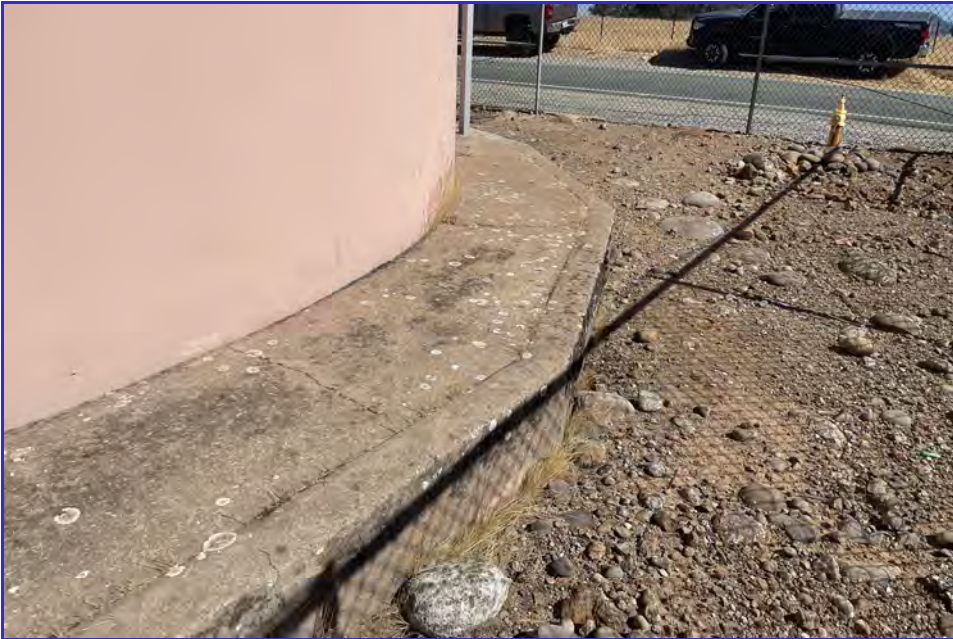
EXTERIOR - CPUD - Paloma Reservoir - Maintenance Inspection -052
