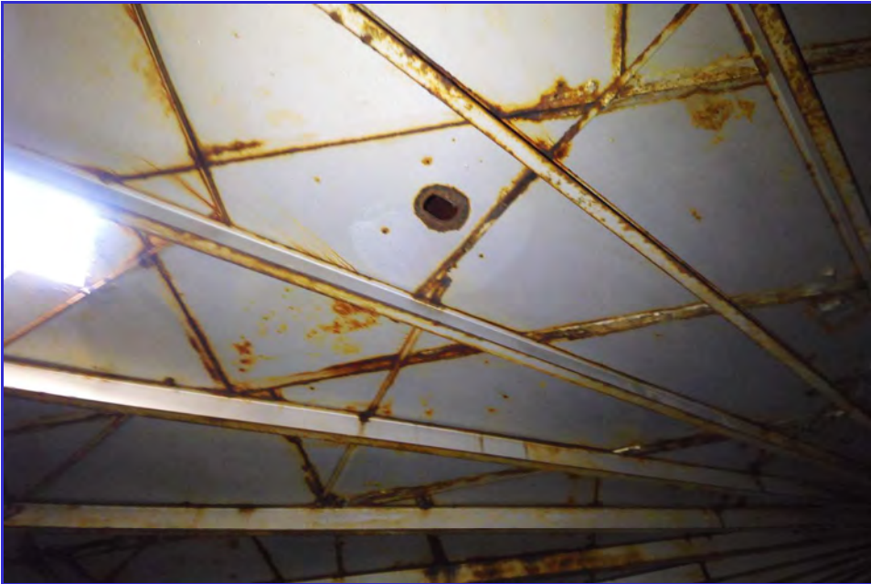
INTERIOR - CPUD - Mokelumne Hill Reservoir - Maintenance Inspection -008
