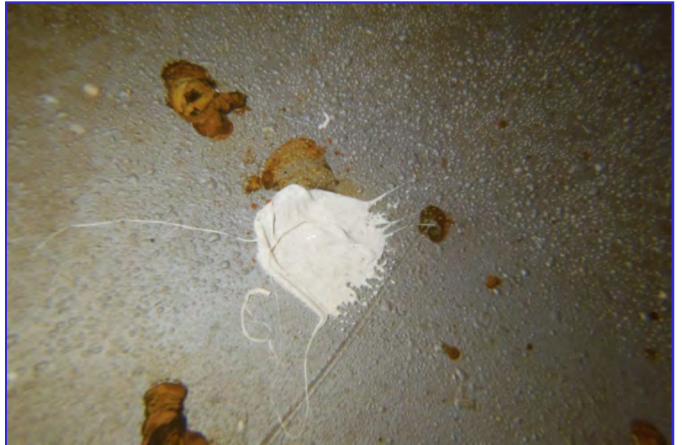
INTERIOR - CPUD - San Andaras Reservoir - Maintenance Inspection -245
