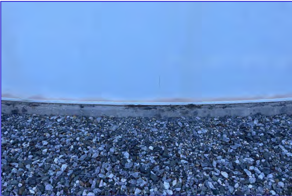
EXTERIOR - CPUD - Mokelumne Reservoir - Maintenance Inspection -150
