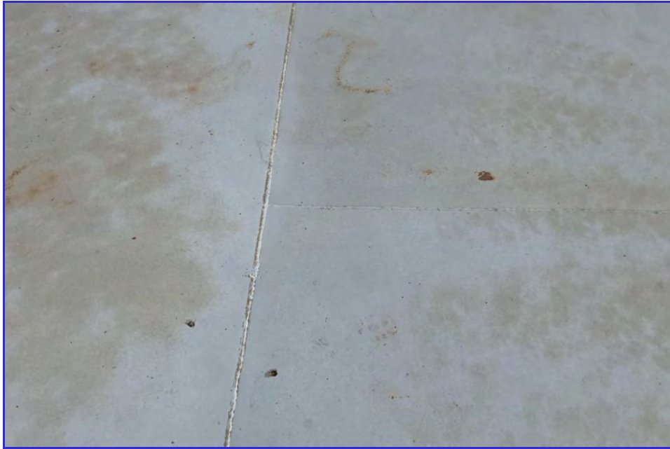
EXTERIOR - CPUD - San Andreas Reservoir - Maintenance Inspection -056
