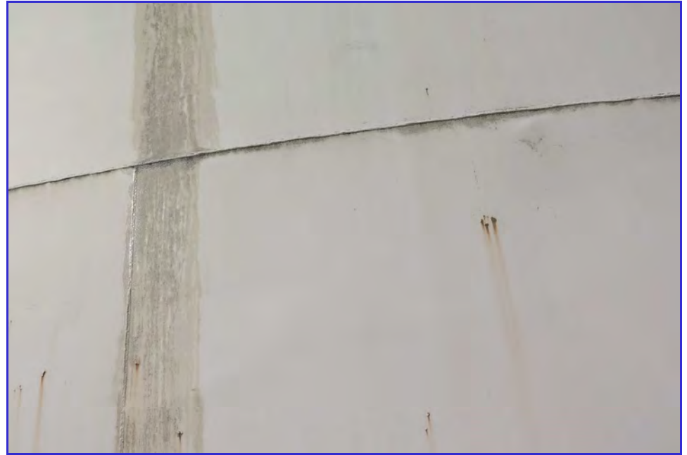
EXTERIOR - Calaveras Public Utility District - Clear Well Tank - Maintenance Inspection -121
