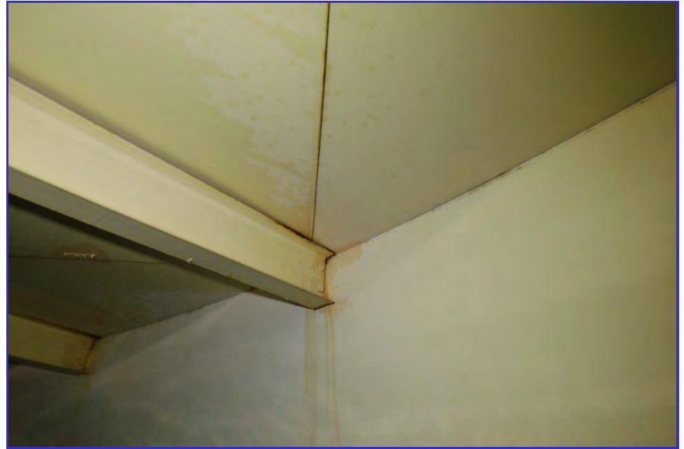
INTERIOR - CPUD - Railroad Flat Reservoir - Maintenance Inspection -057
