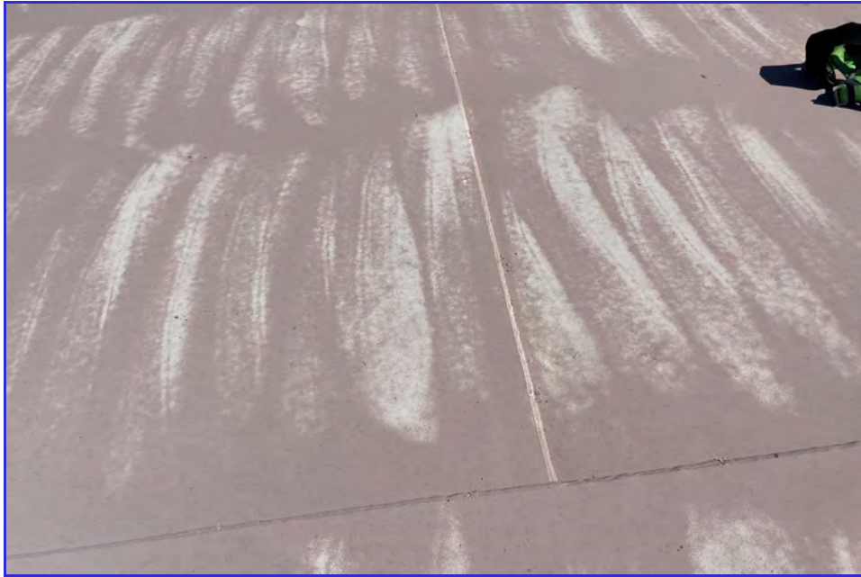
EXTERIOR - CPUD - Paloma Reservoir - Maintenance Inspection -032
