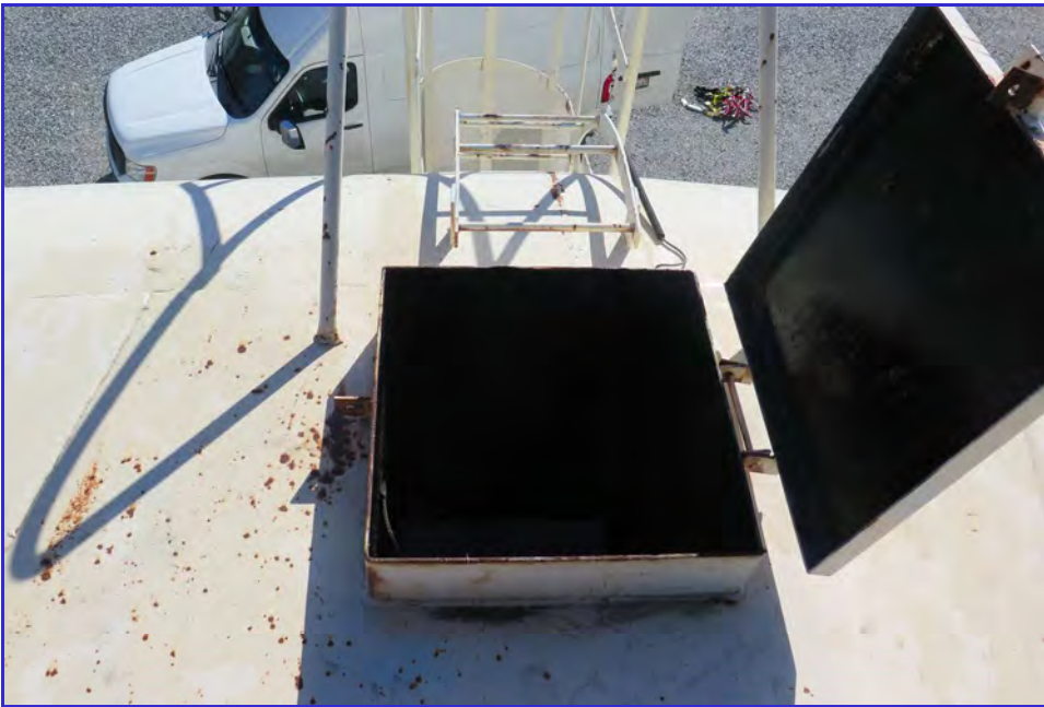
EXTERIOR - Calaveras Public Utility District - Clear Well Tank - Maintenance Inspection -002
