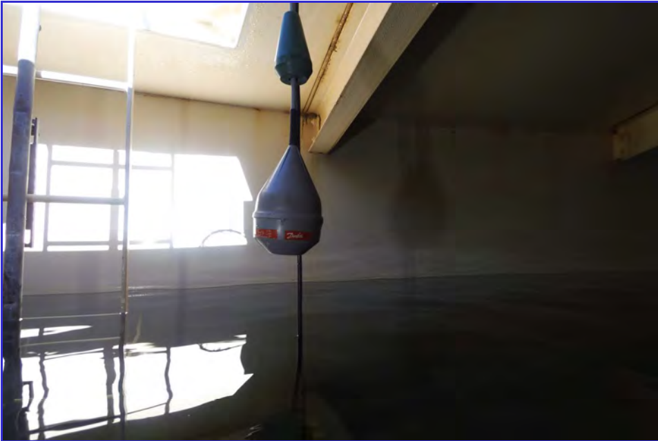
INTERIOR - CPUD - Railroad Flat Reservoir - Maintenance Inspection -004
