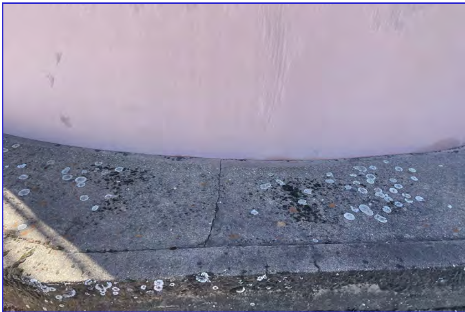
EXTERIOR - CPUD - Paloma Reservoir - Maintenance Inspection -086
