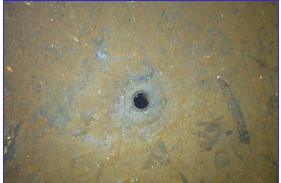
INTERIOR - CPUD - Paloma Reservoir - Maintenance Inspection -085
