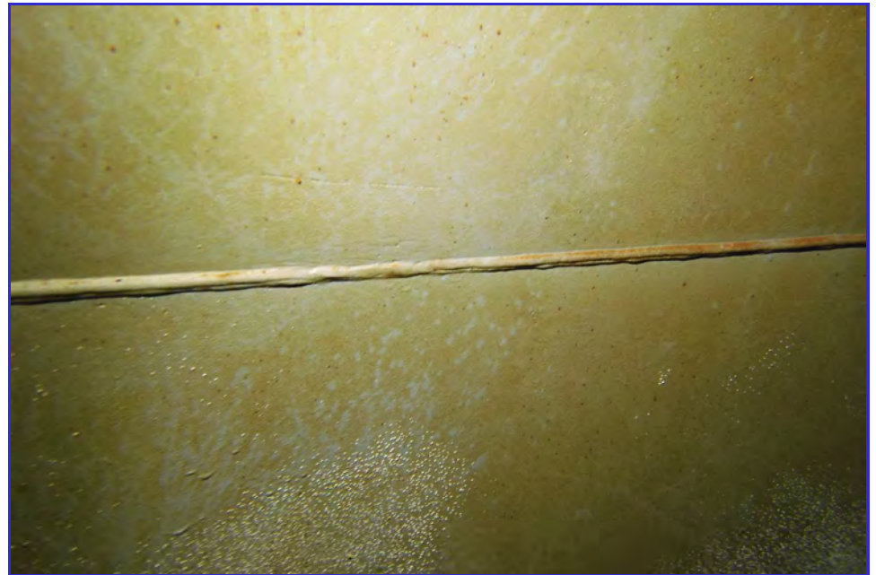
INTERIOR - CPUD - Mokelumne Hill Reservoir - Maintenance Inspection -091
