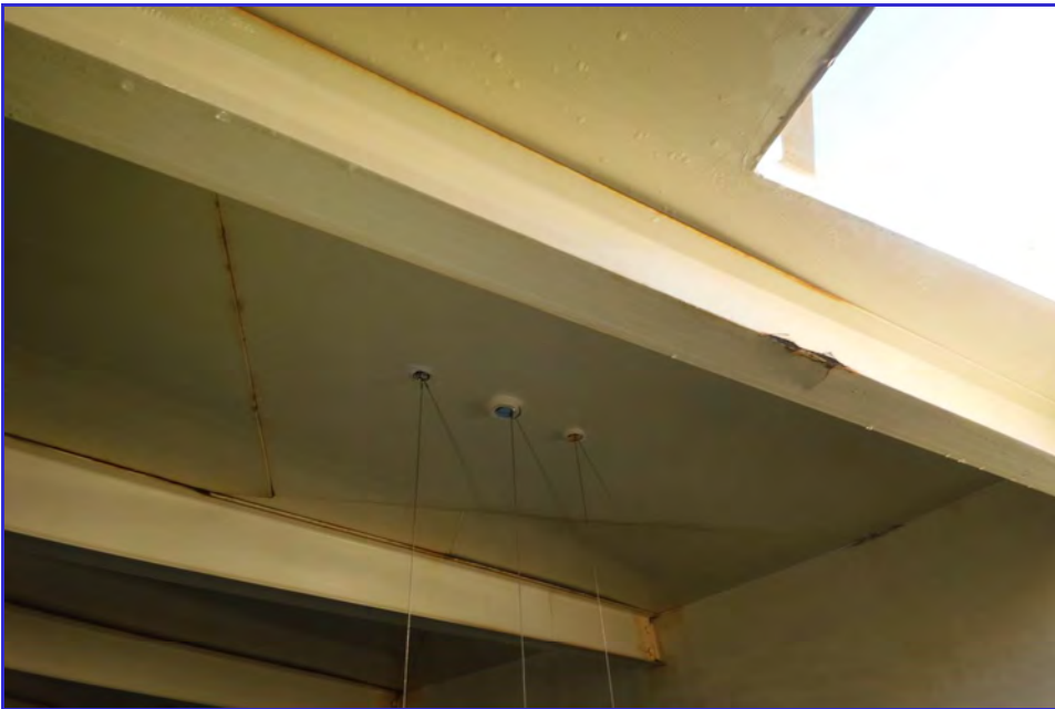
INTERIOR - CPUD - Railroad Flat Reservoir - Maintenance Inspection -006
