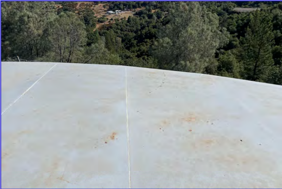
EXTERIOR - CPUD - San Andreas Reservoir - Maintenance Inspection -060
