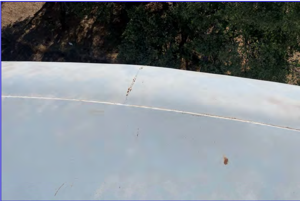
EXTERIOR - CPUD - Mokelumne Reservoir - Maintenance Inspection -054
