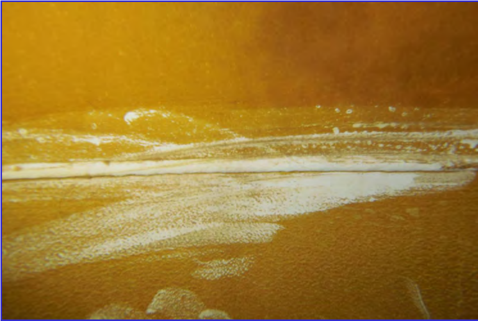
INTERIOR - CPUD - Railroad Flat Reservoir - Maintenance Inspection -100
