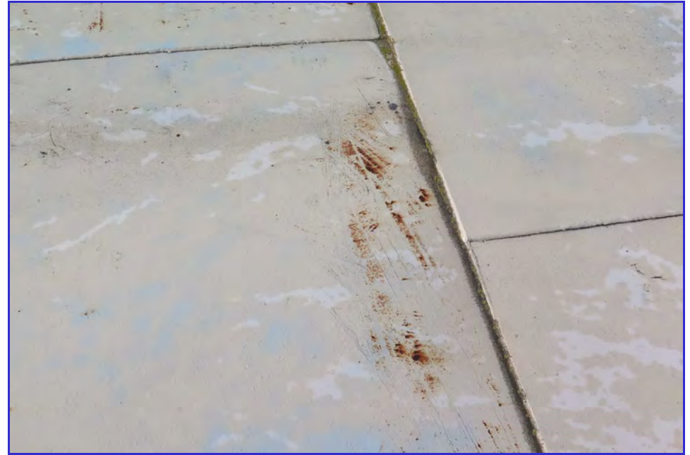
EXTERIOR - Calaveras Public Utility District - Clear Well Tank - Maintenance Inspection -017
