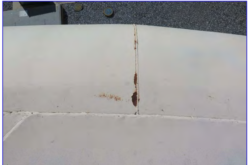
EXTERIOR - Calaveras Public Utility District - Clear Well Tank - Maintenance Inspection -035
