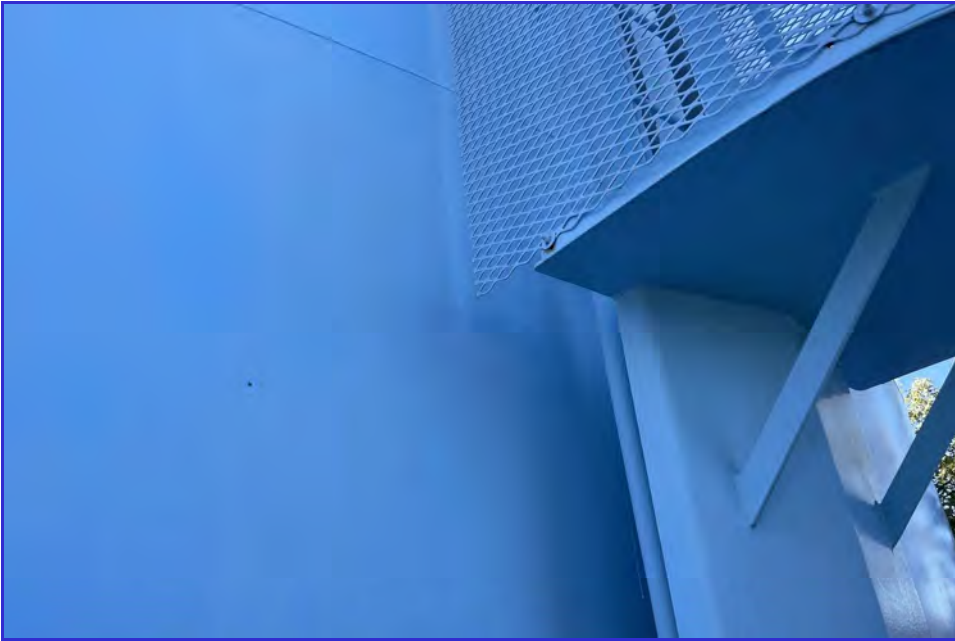
EXTERIOR - CPUD - Railroad Flat Reservoir - Maintenance Inspection -064
