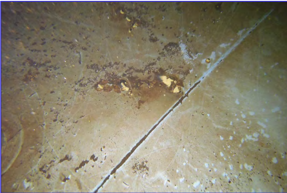
INTERIOR - CPUD - San Andaras Reservoir - Maintenance Inspection -190
