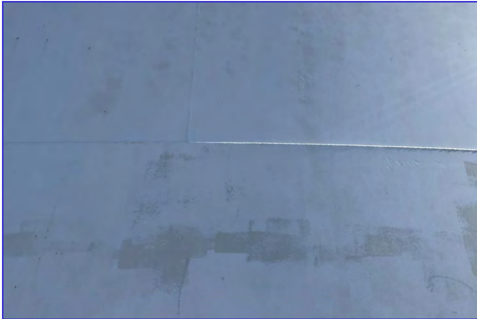
EXTERIOR - CPUD - San Andreas Reservoir - Maintenance Inspection -156
