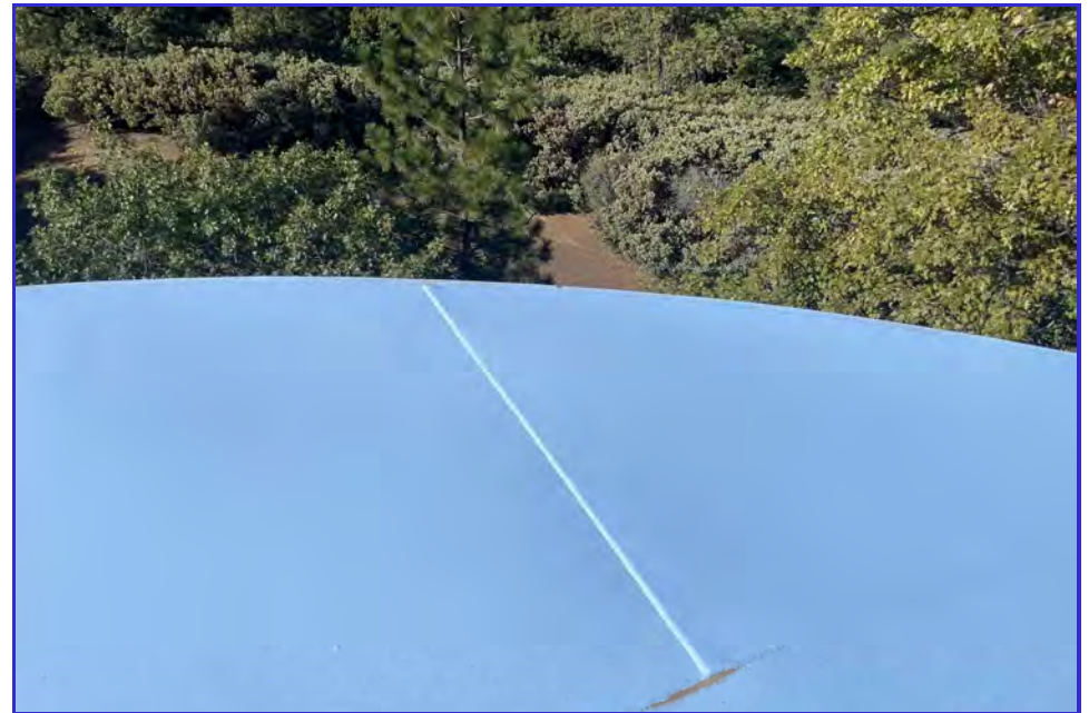
EXTERIOR - CPUD - Railroad Flat Reservoir - Maintenance Inspection -031
