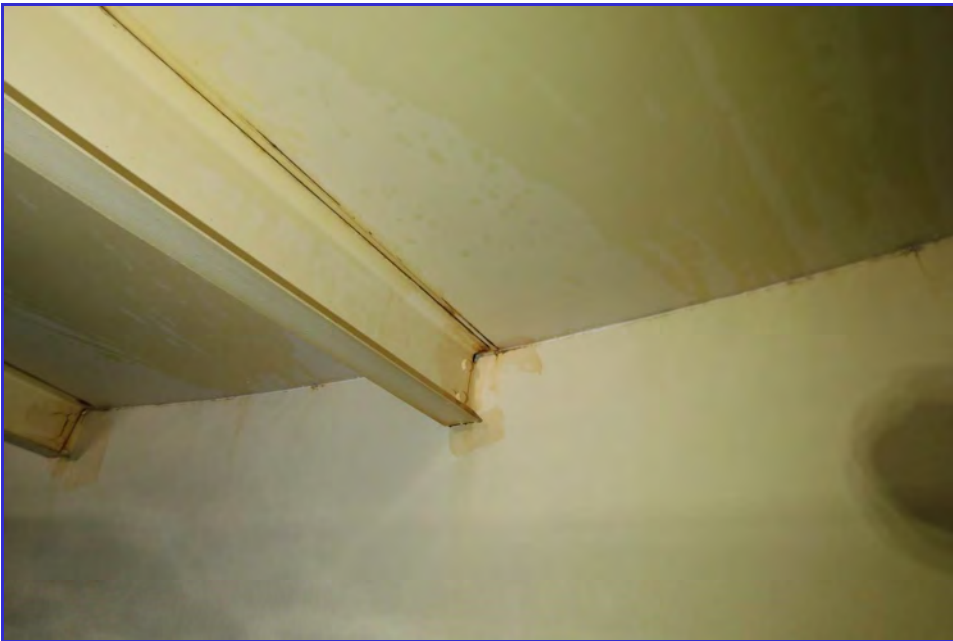
INTERIOR - CPUD - Railroad Flat Reservoir - Maintenance Inspection -062
