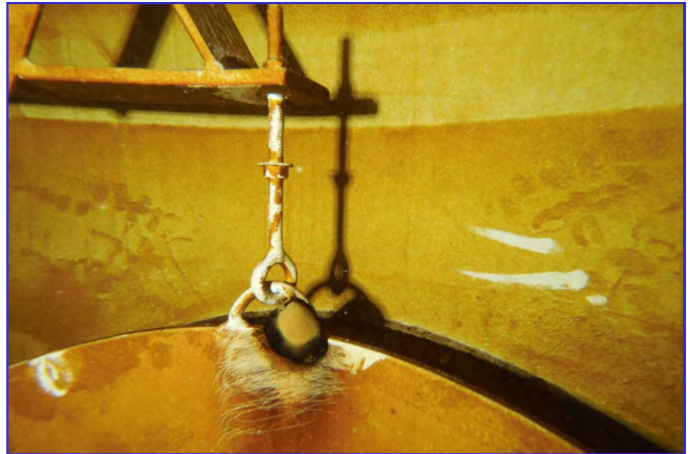
INTERIOR - CPUD - Railroad Flat Reservoir - Maintenance Inspection -119
