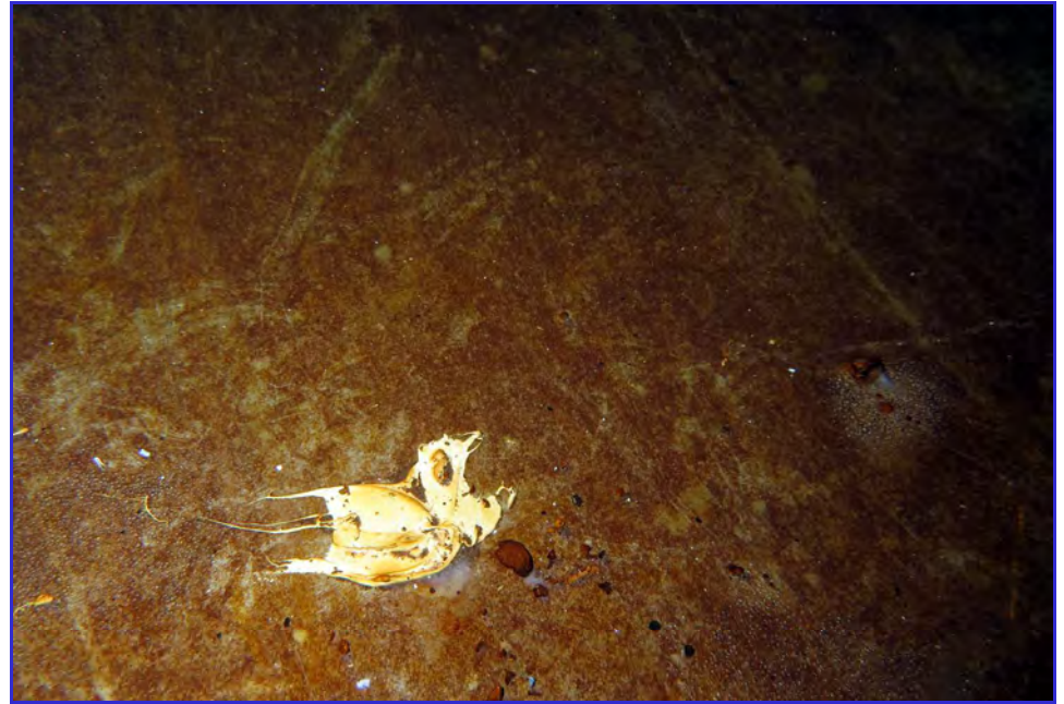
INTERIOR - Calaveras Public Utility District - Clear Well Tank - Maintenance Inspection -129
