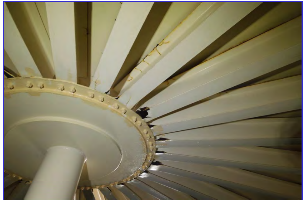
INTERIOR - CPUD - Railroad Flat Reservoir - Maintenance Inspection -039
