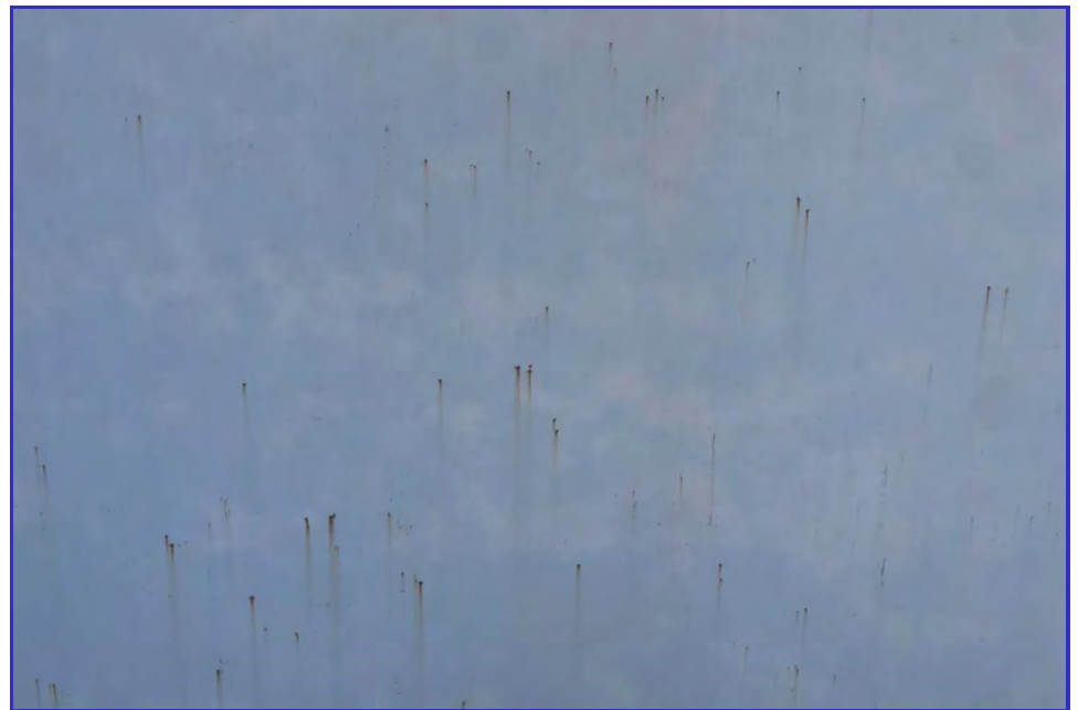
EXTERIOR - CPUD - Mokelumne Reservoir - Maintenance Inspection -111
