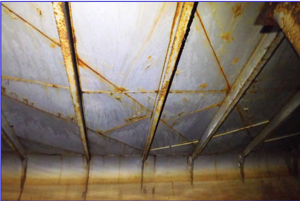
INTERIOR - CPUD - San Andaras Reservoir - Maintenance Inspection -062
