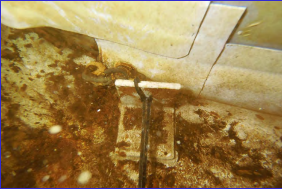
INTERIOR - CPUD - Railroad Flat Reservoir - Maintenance Inspection -140
