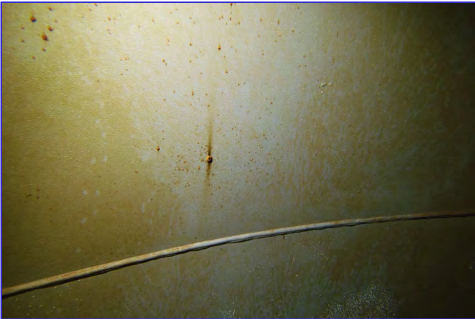
INTERIOR - CPUD - Mokelumne Hill Reservoir - Maintenance Inspection -090
