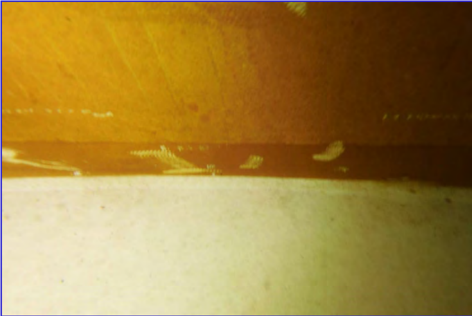
INTERIOR - CPUD - Railroad Flat Reservoir - Maintenance Inspection -116
