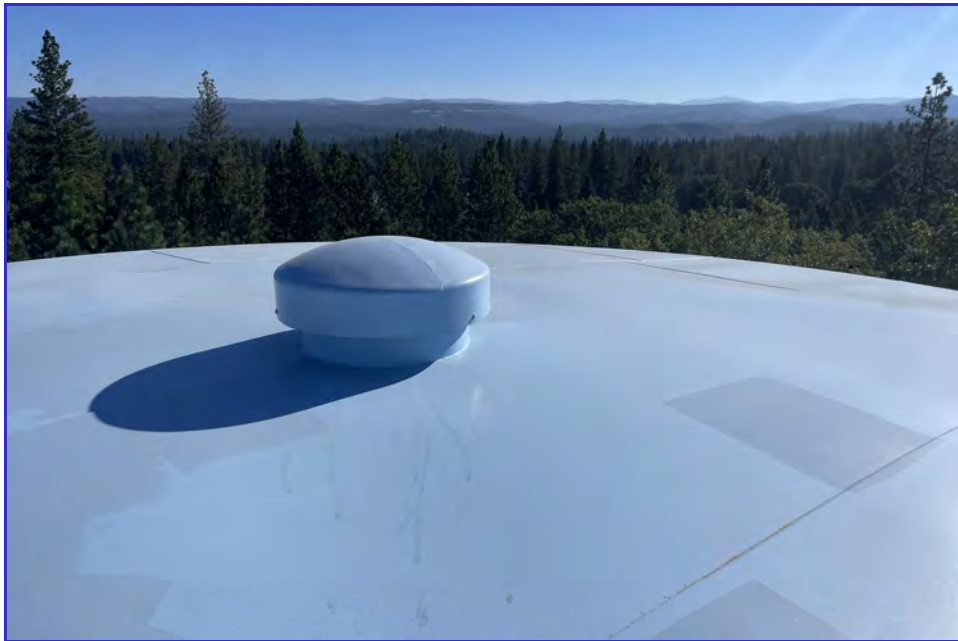
EXTERIOR - CPUD - Railroad Flat Reservoir - Maintenance Inspection -026
