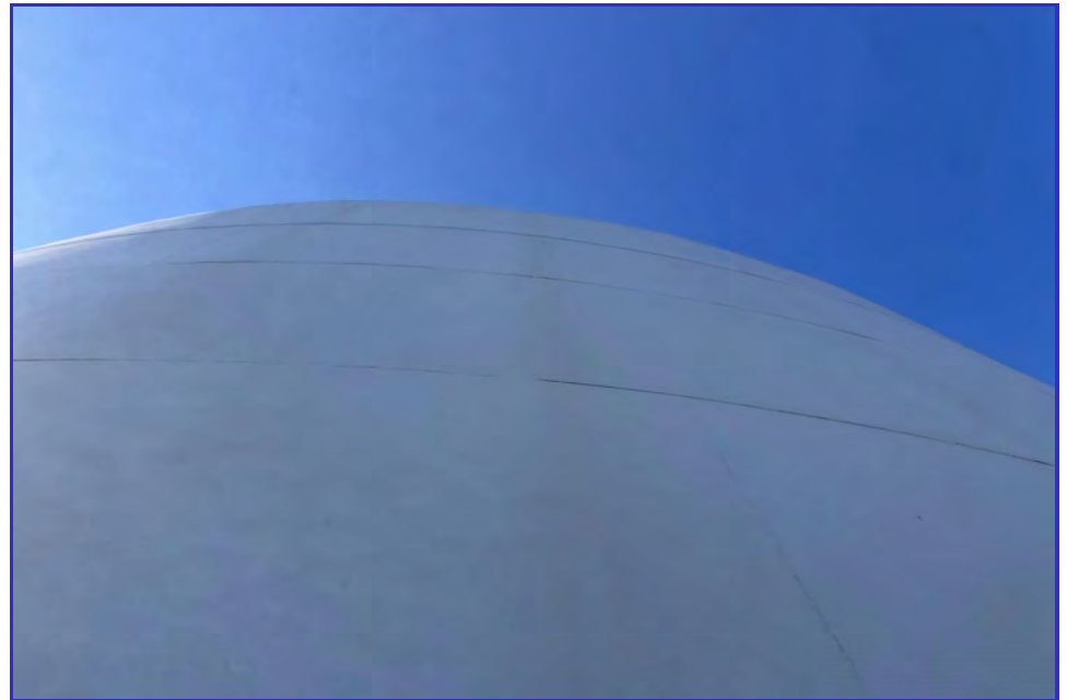
EXTERIOR - CPUD - San Andreas Reservoir - Maintenance Inspection -187
