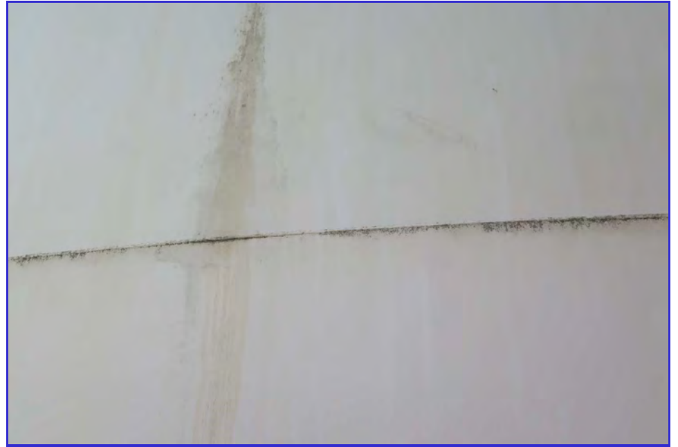
EXTERIOR - Calaveras Public Utility District - Clear Well Tank - Maintenance Inspection -105
