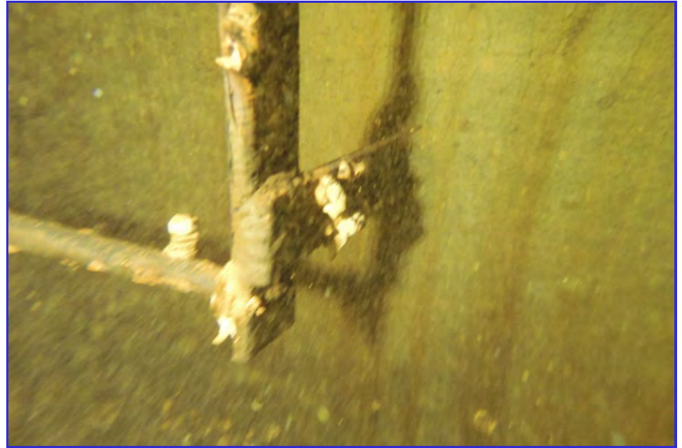
INTERIOR - CPUD - Golden Hills - Maintenance Inspection -109
