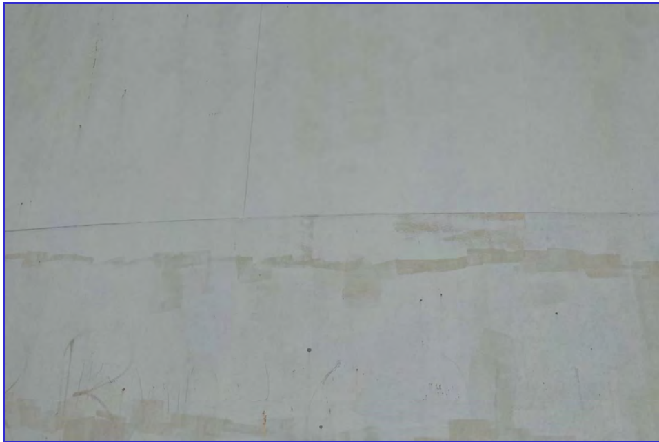
EXTERIOR - CPUD - San Andreas Reservoir - Maintenance Inspection -134
