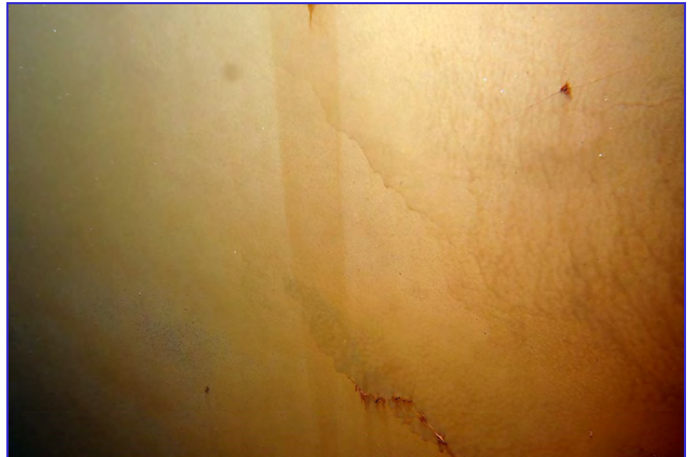
INTERIOR - Calaveras Public Utility District - Clear Well Tank - Maintenance Inspection -059
