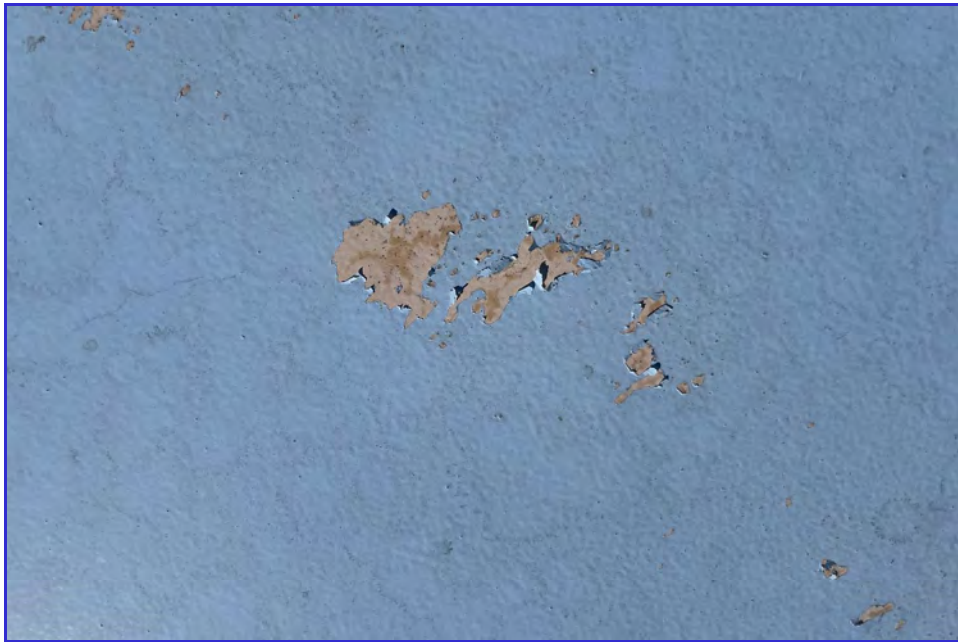
EXTERIOR - CPUD - Railroad Flat Reservoir - Maintenance Inspection -042
