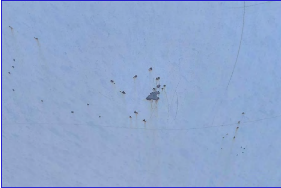
EXTERIOR - CPUD - San Andreas Reservoir - Maintenance Inspection -108
