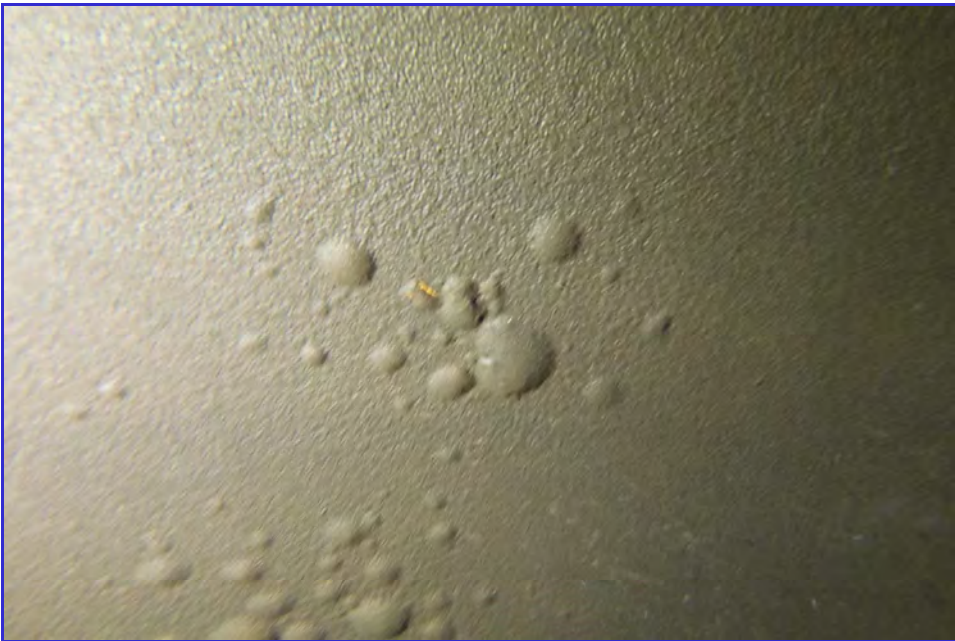
INTERIOR - CPUD - Paloma Reservoir - Maintenance Inspection -046
