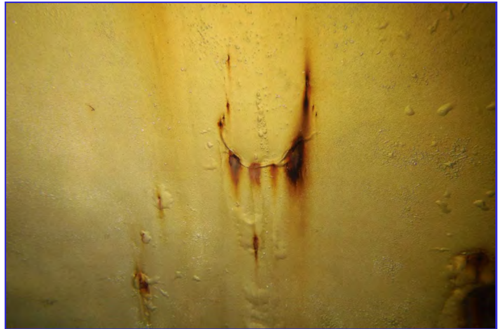
INTERIOR - CPUD - San Andaras Reservoir - Maintenance Inspection -107
