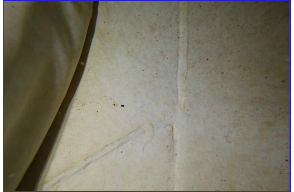
INTERIOR - CPUD - Railroad Flat Reservoir - Maintenance Inspection -109
