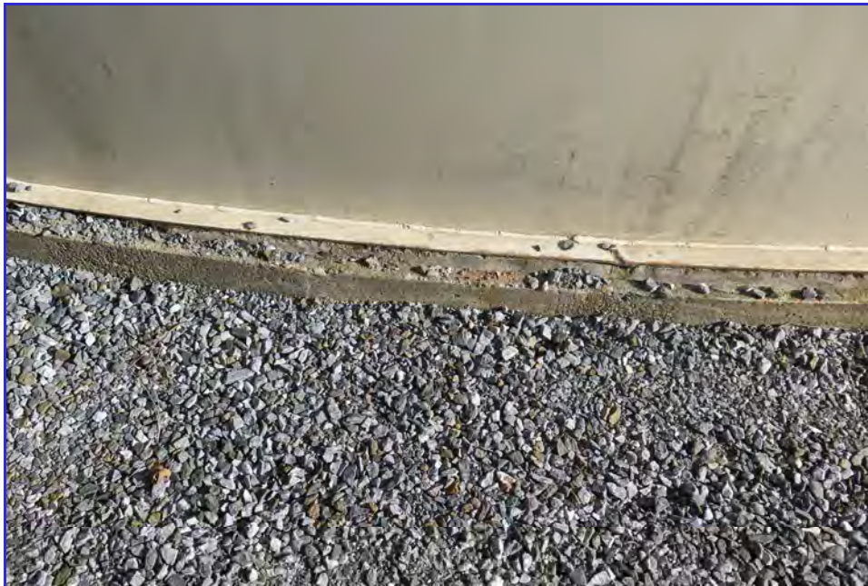
EXTERIOR - Calaveras Public Utility District - Clear Well Tank - Maintenance Inspection -078
