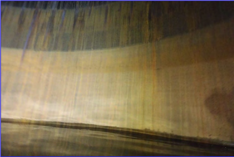
INTERIOR - CPUD - Golden Hills - Maintenance Inspection -028
