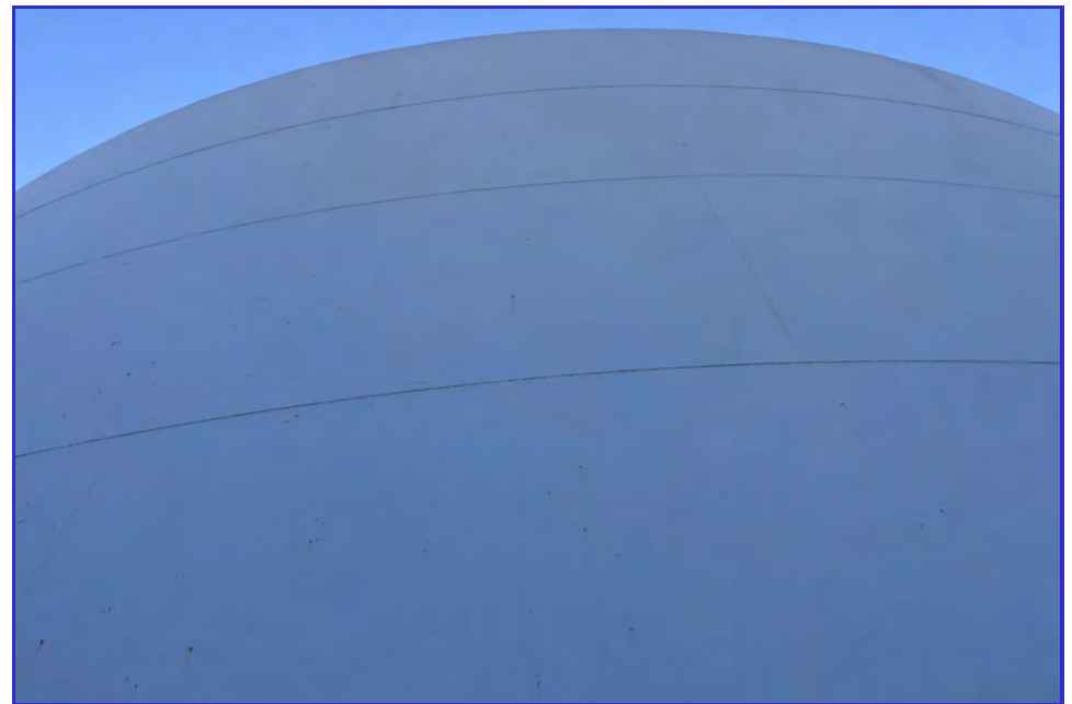
EXTERIOR - CPUD - San Andreas Reservoir - Maintenance Inspection -171
