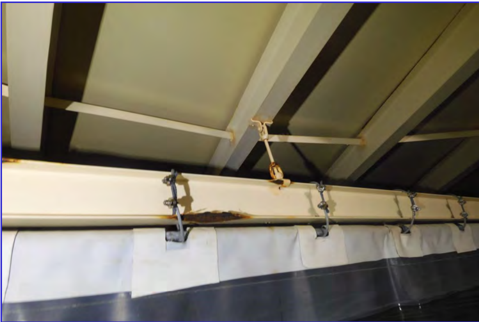
INTERIOR - CPUD - Railroad Flat Reservoir - Maintenance Inspection -042
