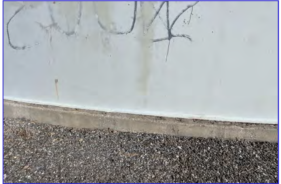
EXTERIOR - CPUD - San Andreas Reservoir - Maintenance Inspection -149
