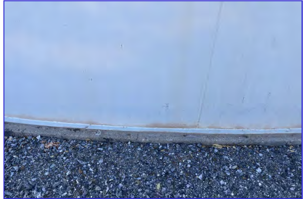
EXTERIOR - CPUD - Mokelumne Reservoir - Maintenance Inspection -113
