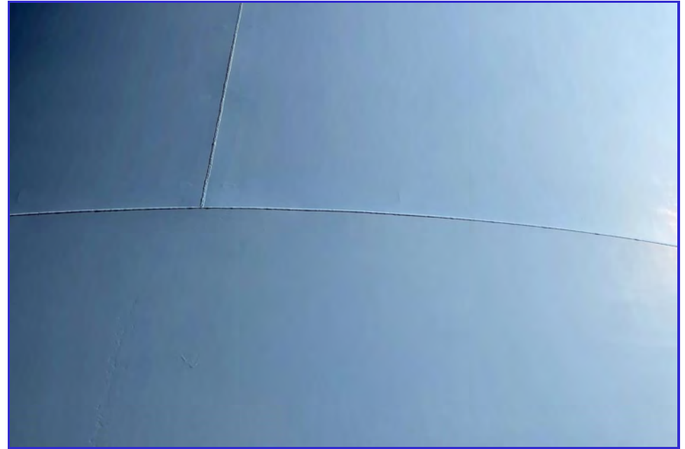
EXTERIOR - CPUD - Railroad Flat Reservoir - Maintenance Inspection -057
