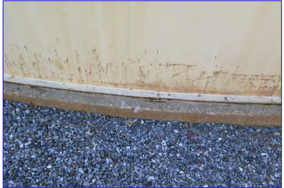
EXTERIOR - Calaveras Public Utility District - Clear Well Tank - Maintenance Inspection -097
