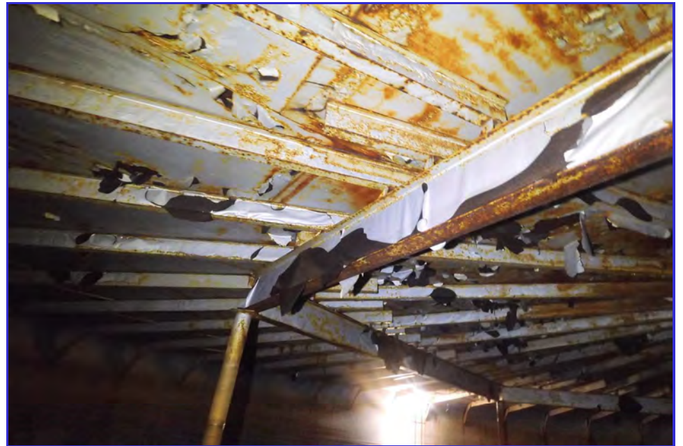
INTERIOR - CPUD - San Andaras Reservoir - Maintenance Inspection -051
