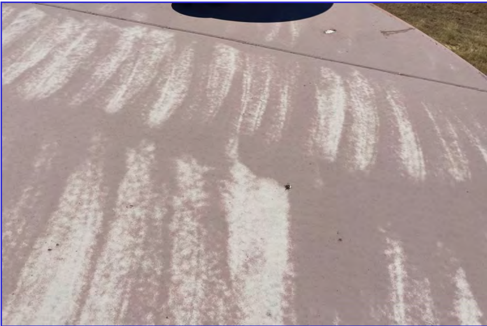
EXTERIOR - CPUD - Paloma Reservoir - Maintenance Inspection -018
