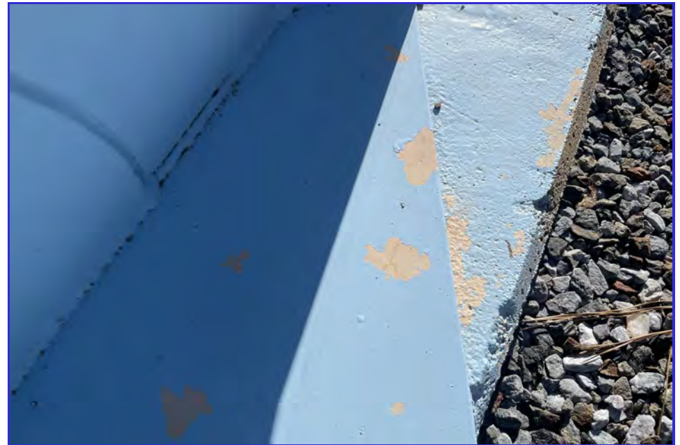
EXTERIOR - CPUD - Railroad Flat Reservoir - Maintenance Inspection -079
