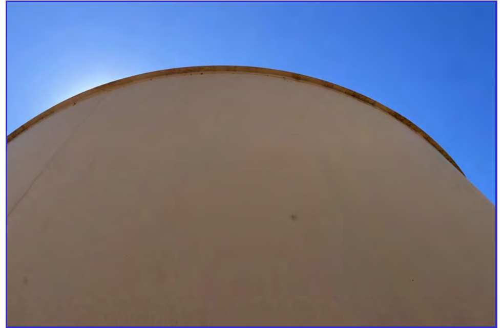
EXTERIOR - CPUD - Golden Hills - Maintenance Inspection -053
