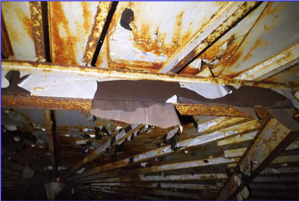
INTERIOR - CPUD - San Andaras Reservoir - Maintenance Inspection -056
