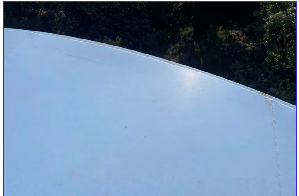
EXTERIOR - CPUD - Railroad Flat Reservoir - Maintenance Inspection -019
