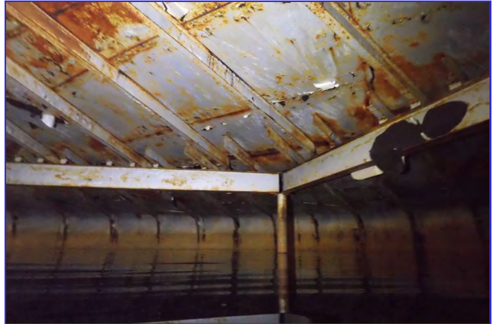
INTERIOR - CPUD - San Andaras Reservoir - Maintenance Inspection -081
