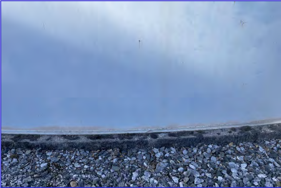
EXTERIOR - CPUD - Mokelumne Reservoir - Maintenance Inspection -080
