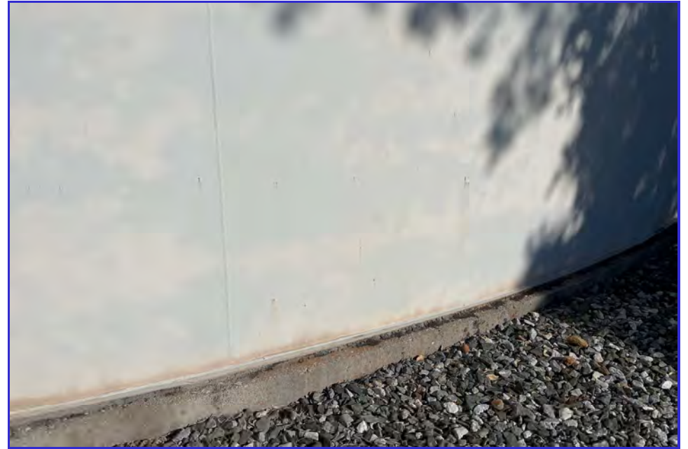
EXTERIOR - CPUD - Mokelumne Reservoir - Maintenance Inspection -161
