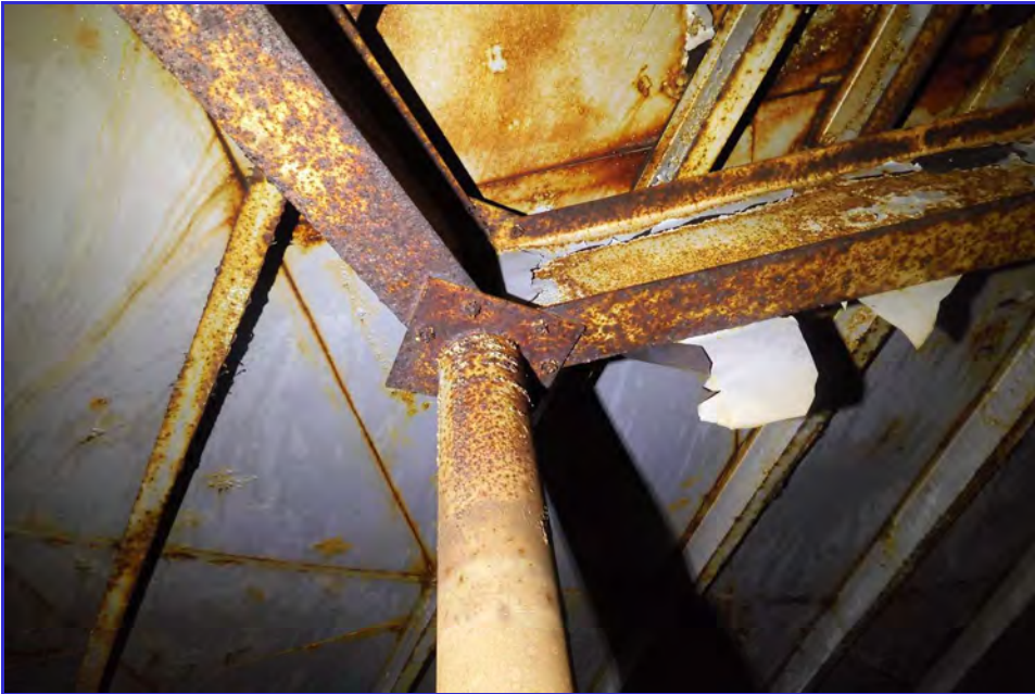
INTERIOR - CPUD - San Andaras Reservoir - Maintenance Inspection -060
