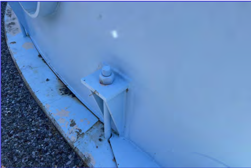
EXTERIOR - CPUD - Railroad Flat Reservoir - Maintenance Inspection -078
