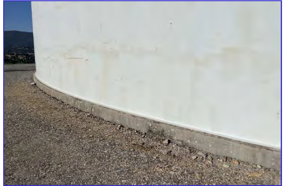
EXTERIOR - CPUD - San Andreas Reservoir - Maintenance Inspection -133
