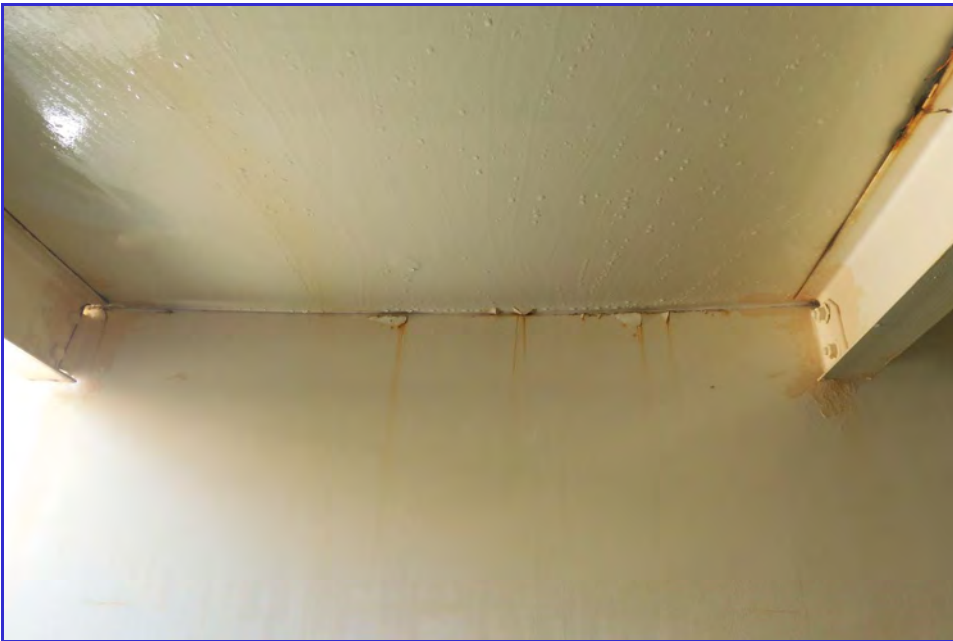
INTERIOR - CPUD - Railroad Flat Reservoir - Maintenance Inspection -010
