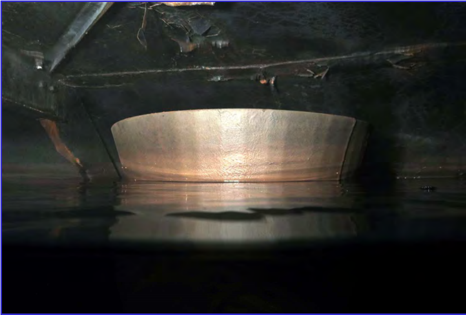
INTERIOR - Calaveras Public Utility District - Clear Well Tank - Maintenance Inspection -056
