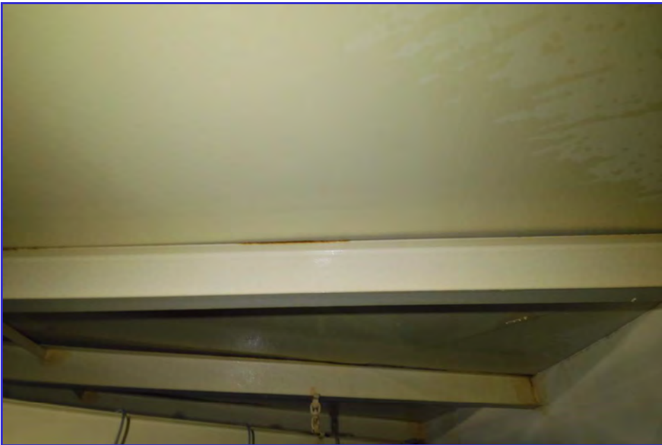
INTERIOR - CPUD - Railroad Flat Reservoir - Maintenance Inspection -058
