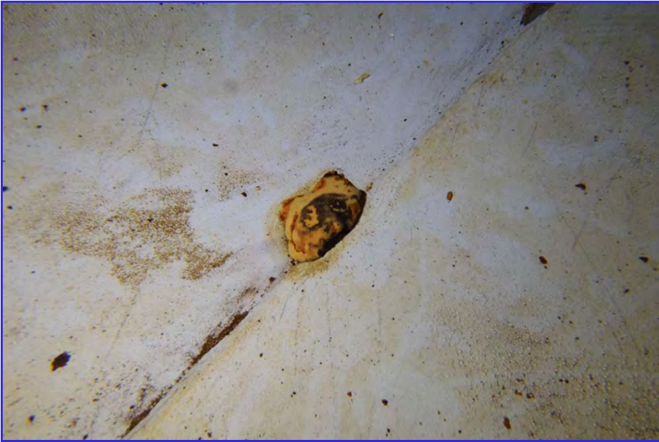
INTERIOR - CPUD - Mokelumne Hill Reservoir - Maintenance Inspection -164
