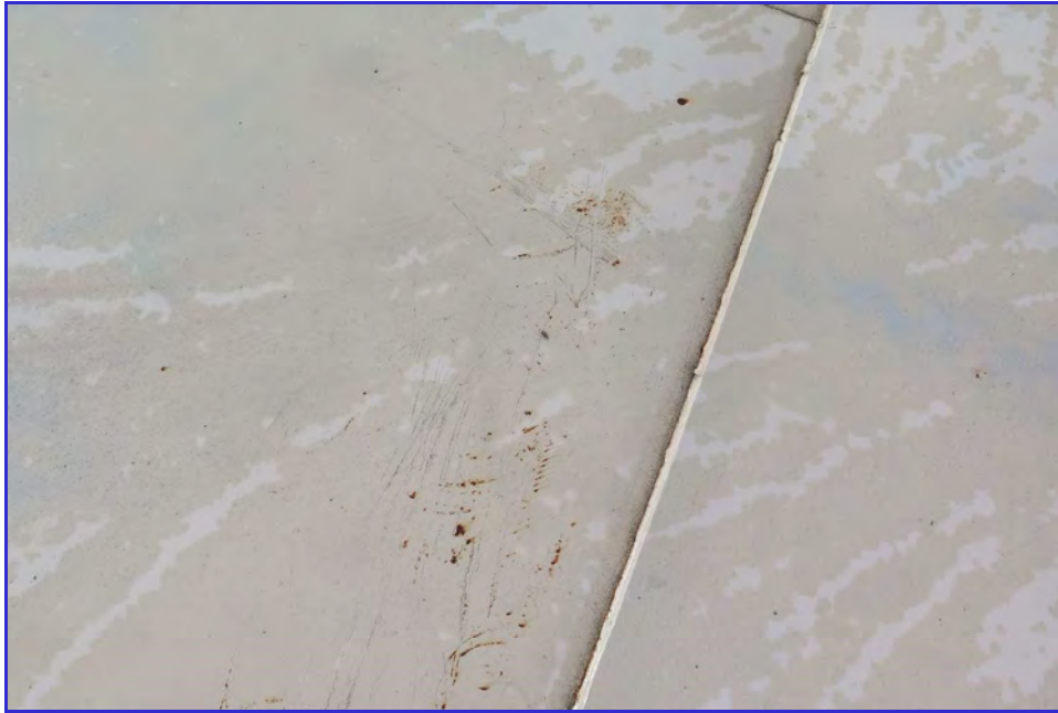
EXTERIOR - Calaveras Public Utility District - Clear Well Tank - Maintenance Inspection -024
