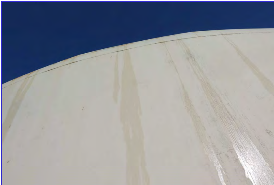
EXTERIOR - Calaveras Public Utility District - Clear Well Tank - Maintenance Inspection -066
