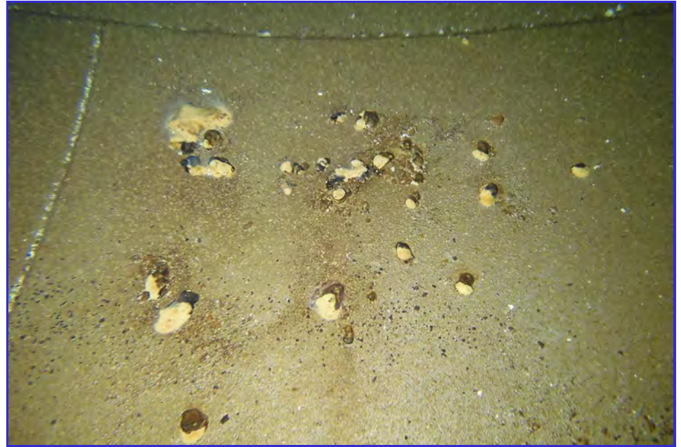
INTERIOR - CPUD - San Andaras Reservoir - Maintenance Inspection -205
