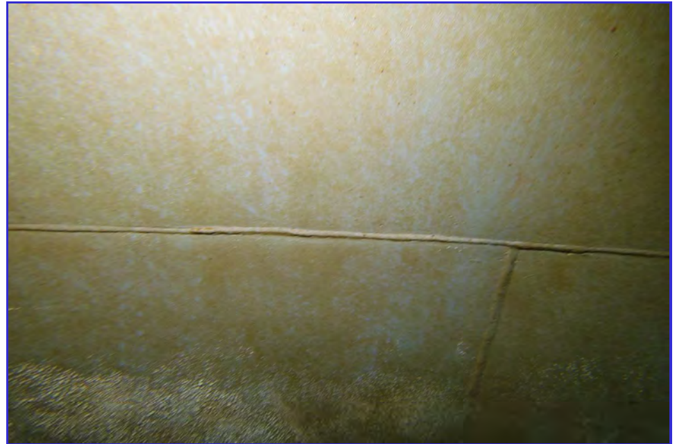
INTERIOR - CPUD - Mokelumne Hill Reservoir - Maintenance Inspection -081
