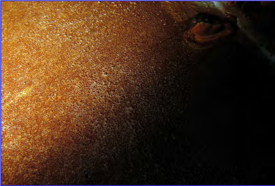
INTERIOR - Calaveras Public Utility District - Clear Well Tank - Maintenance Inspection -136
