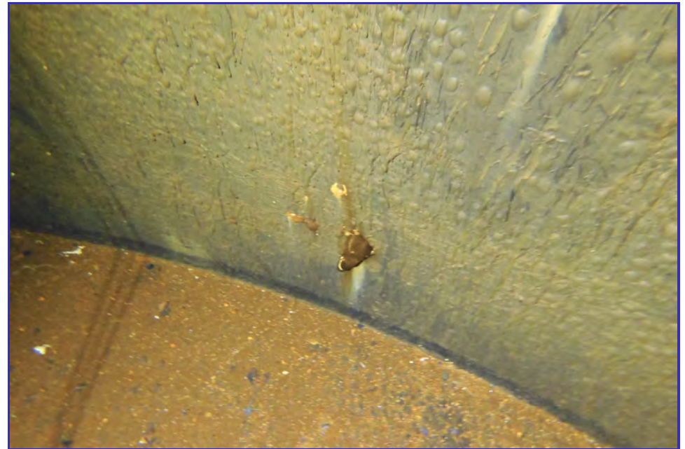
INTERIOR - CPUD - Paloma Reservoir - Maintenance Inspection -107
