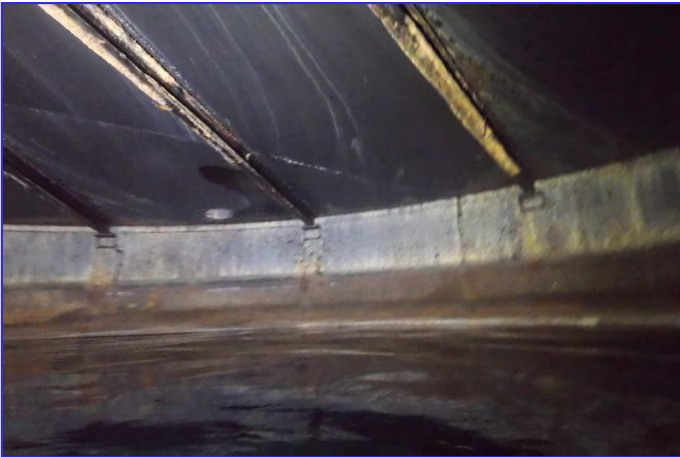
INTERIOR - CPUD - Paloma Reservoir - Maintenance Inspection -030
