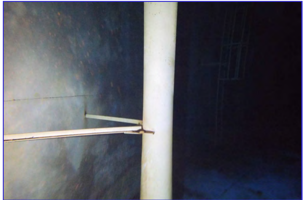
INTERIOR - CPUD - Mokelumne Hill Reservoir - Maintenance Inspection -107
