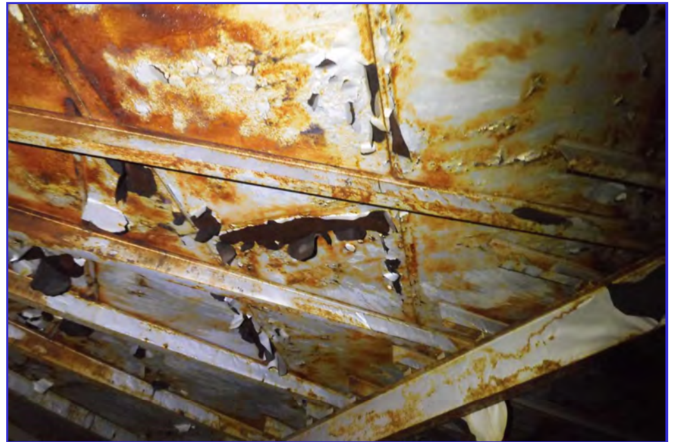
INTERIOR - CPUD - San Andaras Reservoir - Maintenance Inspection -075
