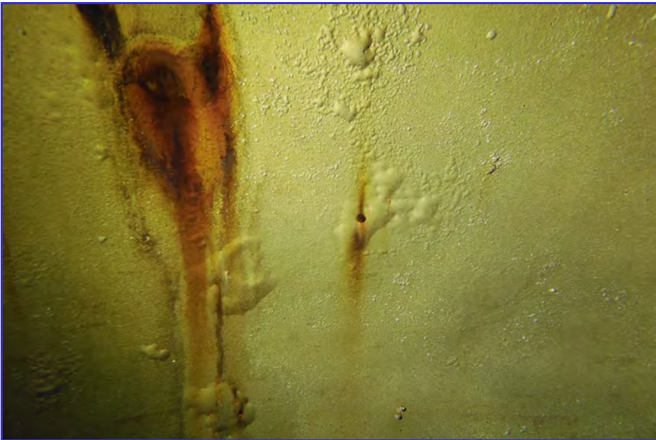
INTERIOR - CPUD - San Andaras Reservoir - Maintenance Inspection -102
