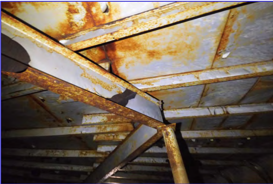
INTERIOR - CPUD - San Andaras Reservoir - Maintenance Inspection -090
