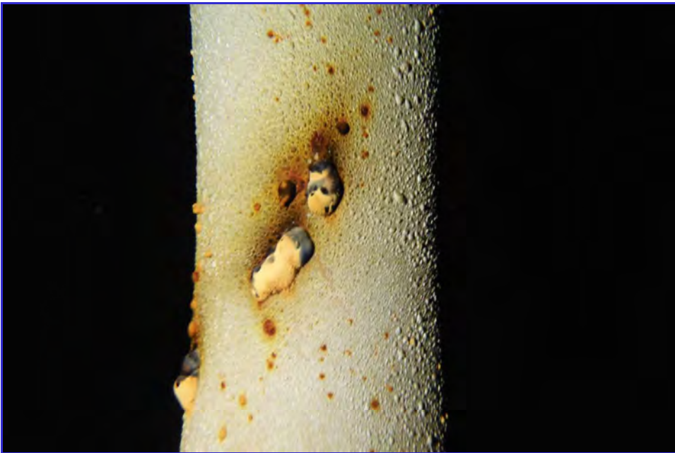
INTERIOR - CPUD - San Andaras Reservoir - Maintenance Inspection -158
