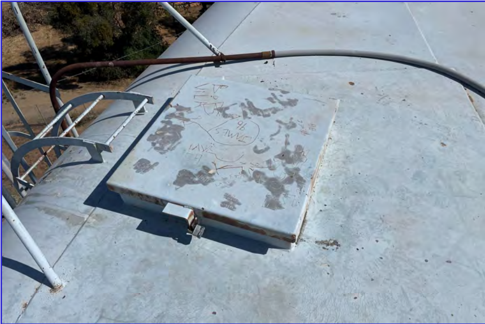
EXTERIOR - CPUD - San Andreas Reservoir - Maintenance Inspection
