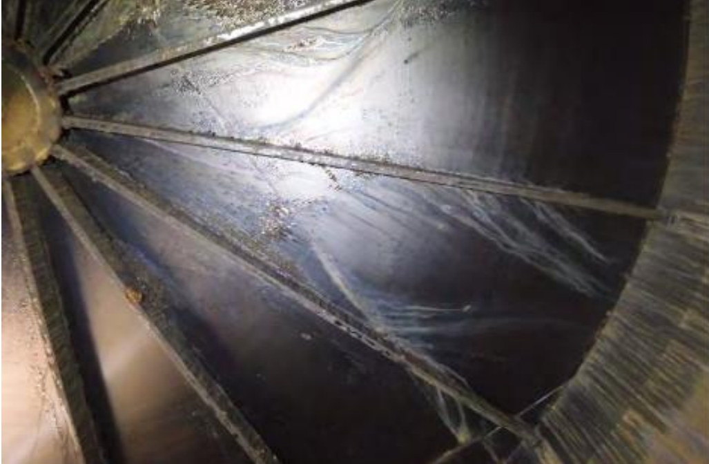
Figure 9-11. Example of Golden Hills Tank Interior Roof
