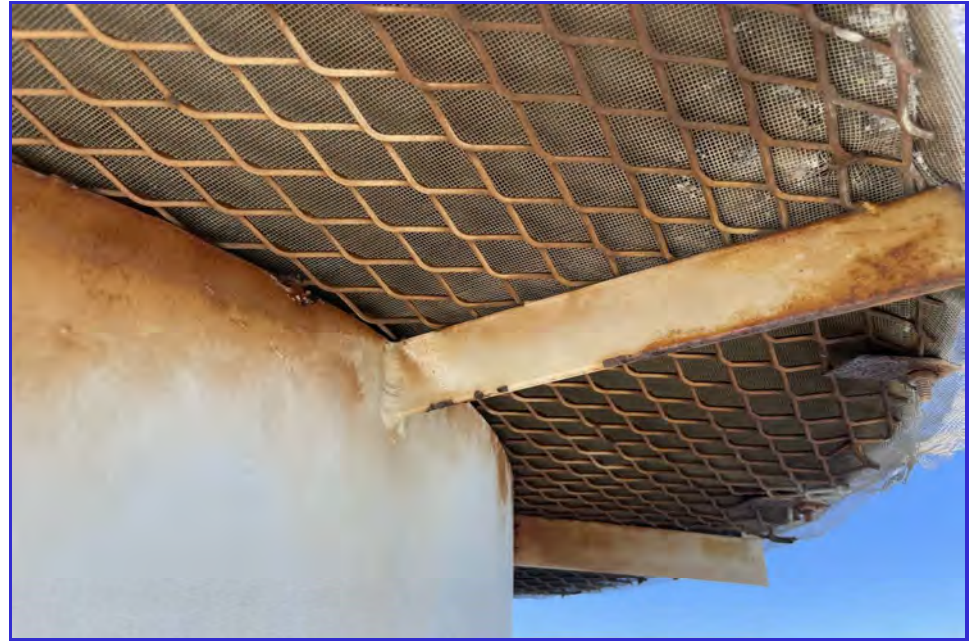
EXTERIOR - CPUD - Mokelumne Reservoir - Maintenance Inspection -029
