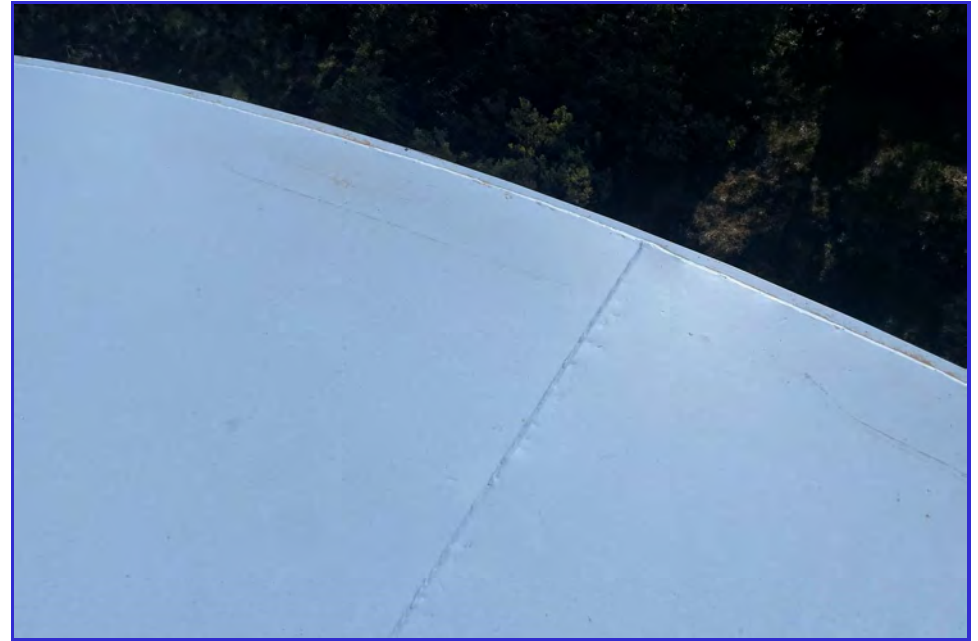
EXTERIOR - CPUD - Railroad Flat Reservoir - Maintenance Inspection -017
