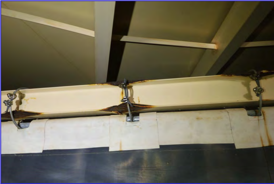
INTERIOR - CPUD - Railroad Flat Reservoir - Maintenance Inspection -044
