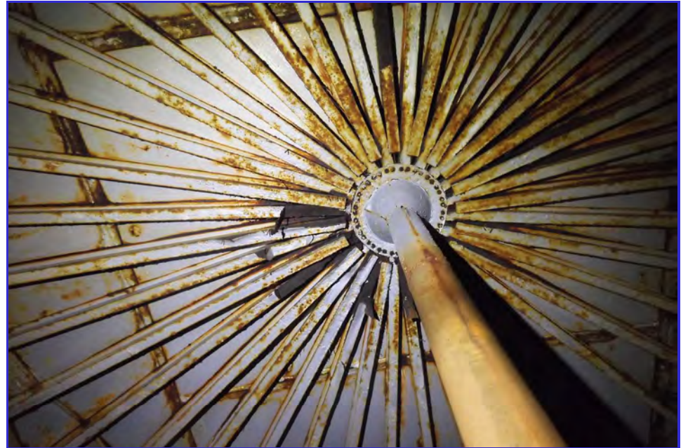
INTERIOR - CPUD - Mokelumne Hill Reservoir - Maintenance Inspection -049
