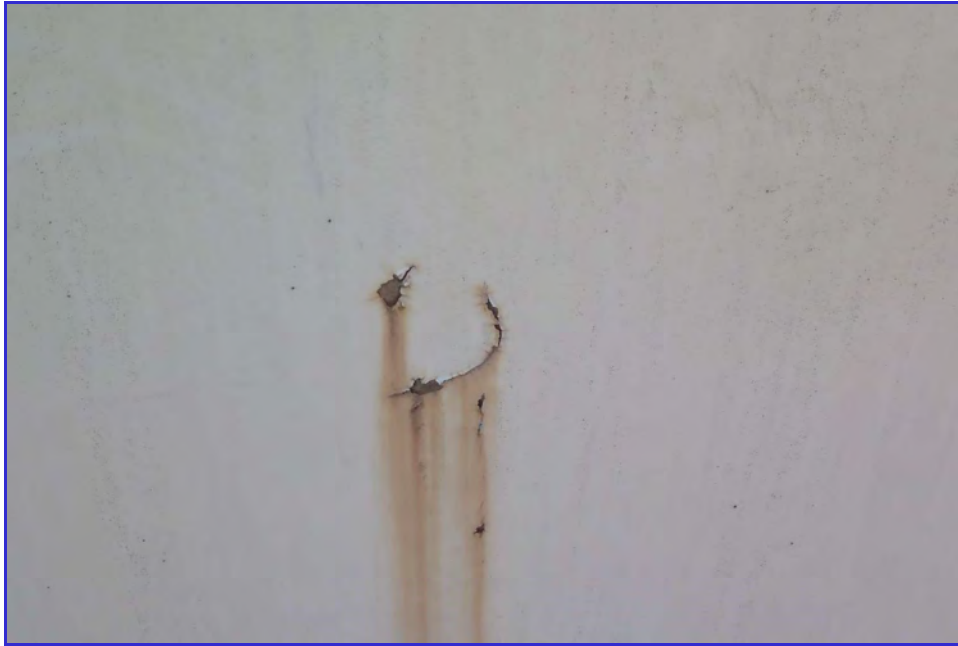
EXTERIOR - Calaveras Public Utility District - Clear Well Tank - Maintenance Inspection -084
