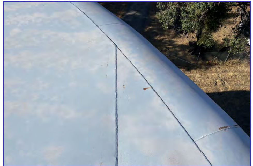
EXTERIOR - CPUD - Mokelumne Reservoir - Maintenance Inspection -071
