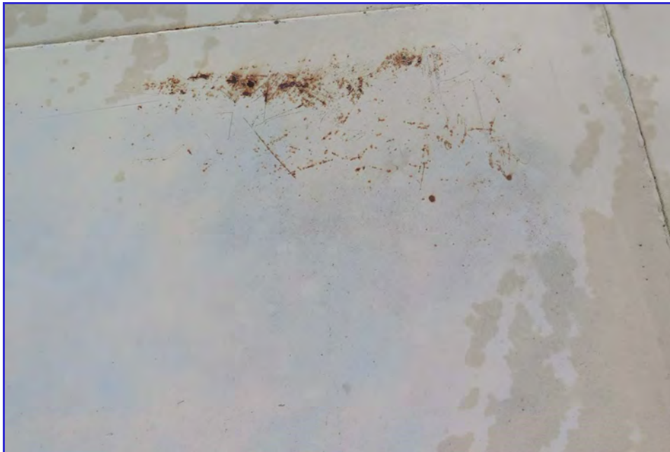
EXTERIOR - Calaveras Public Utility District - Clear Well Tank - Maintenance Inspection -038
