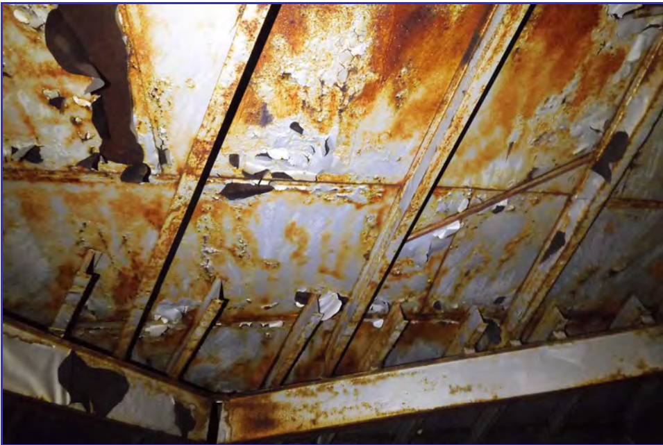
INTERIOR - CPUD - San Andaras Reservoir - Maintenance Inspection -078
