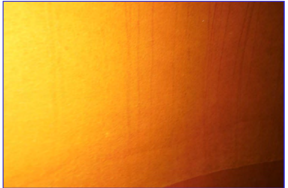
INTERIOR - CPUD - Railroad Flat Reservoir - Maintenance Inspection -091
