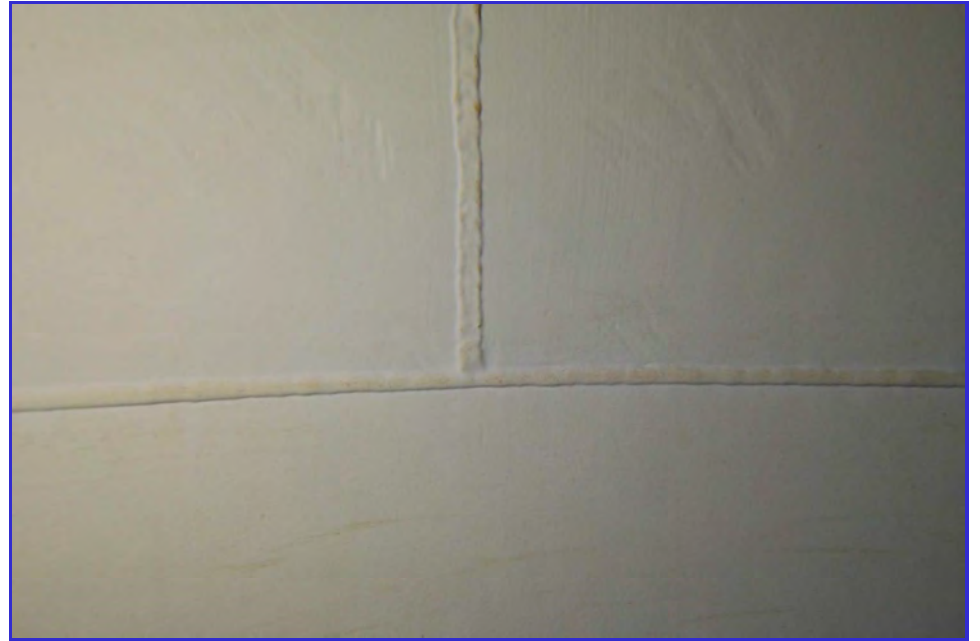
INTERIOR - CPUD - Railroad Flat Reservoir - Maintenance Inspection -069
