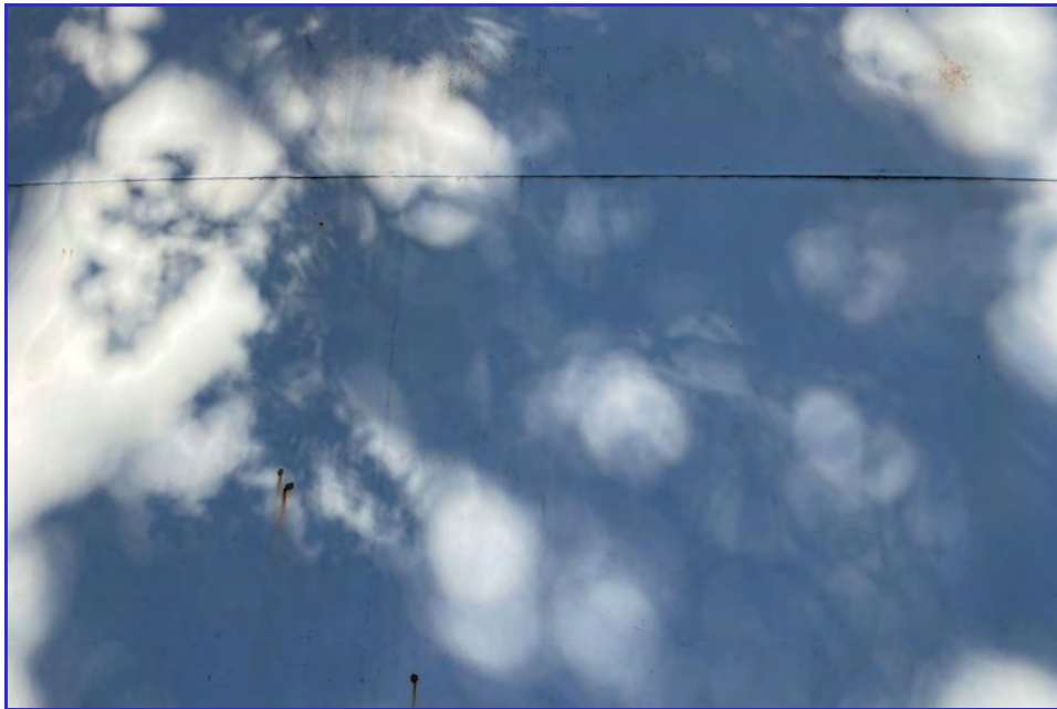
EXTERIOR - CPUD - Mokelumne Reservoir - Maintenance Inspection -166
