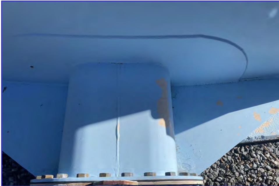
EXTERIOR - CPUD - Railroad Flat Reservoir - Maintenance Inspection -080
