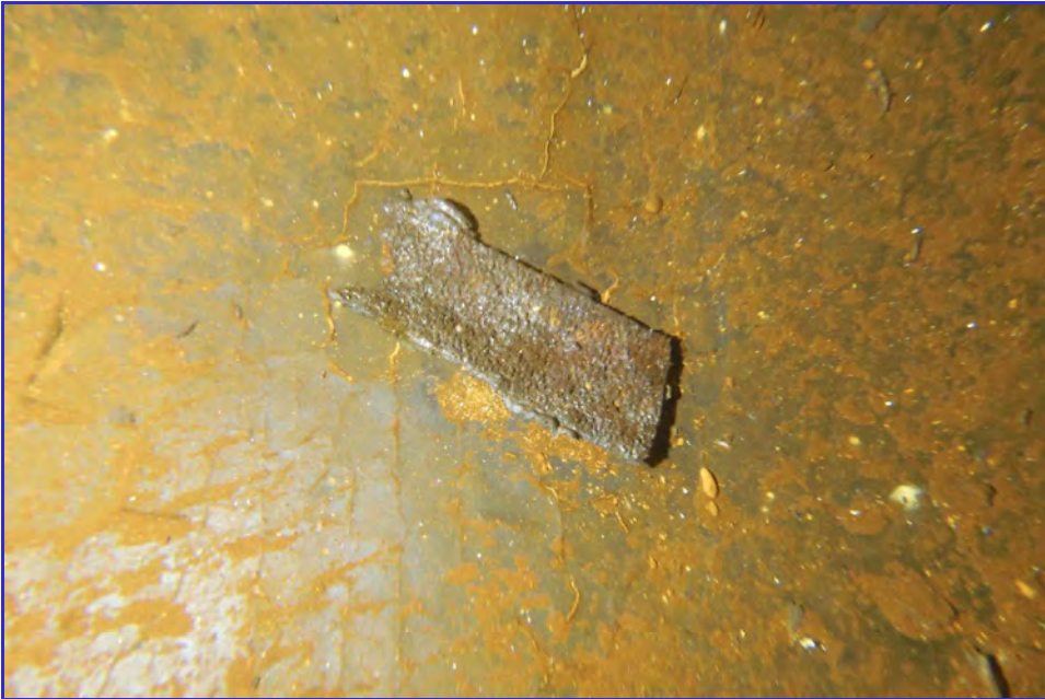
INTERIOR - CPUD - Paloma Reservoir - Maintenance Inspection -124
