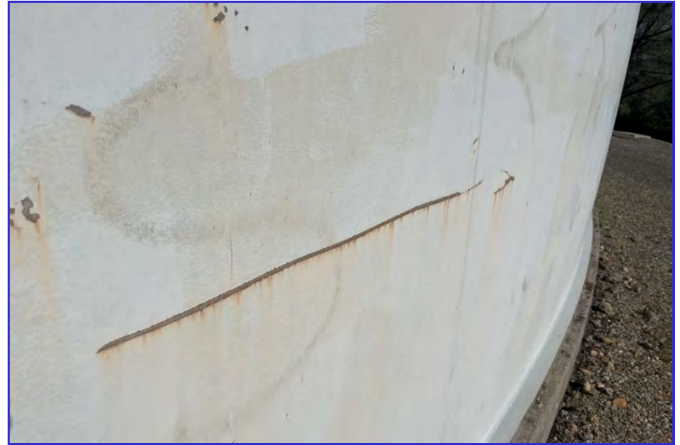
EXTERIOR - CPUD - San Andreas Reservoir - Maintenance Inspection -137
