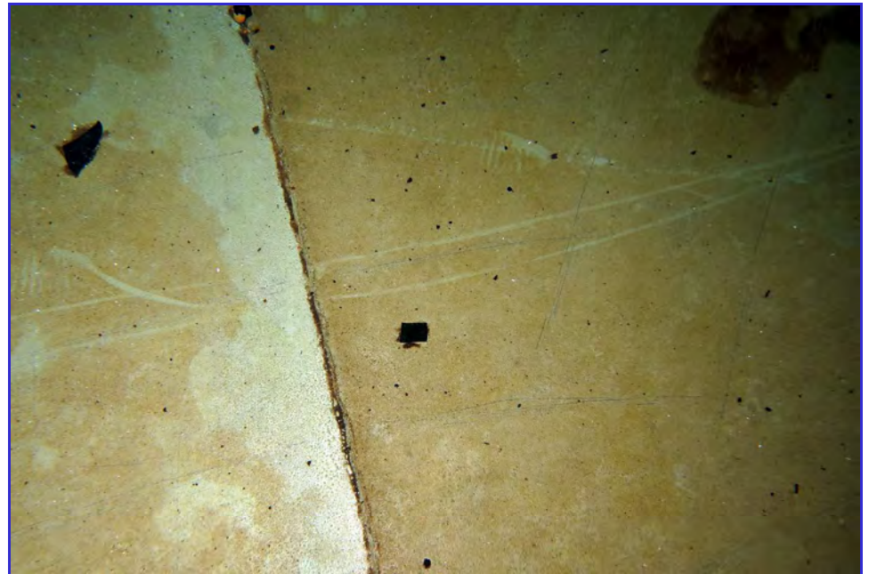
INTERIOR - Calaveras Public Utility District - Clear Well Tank - Maintenance Inspection -111
