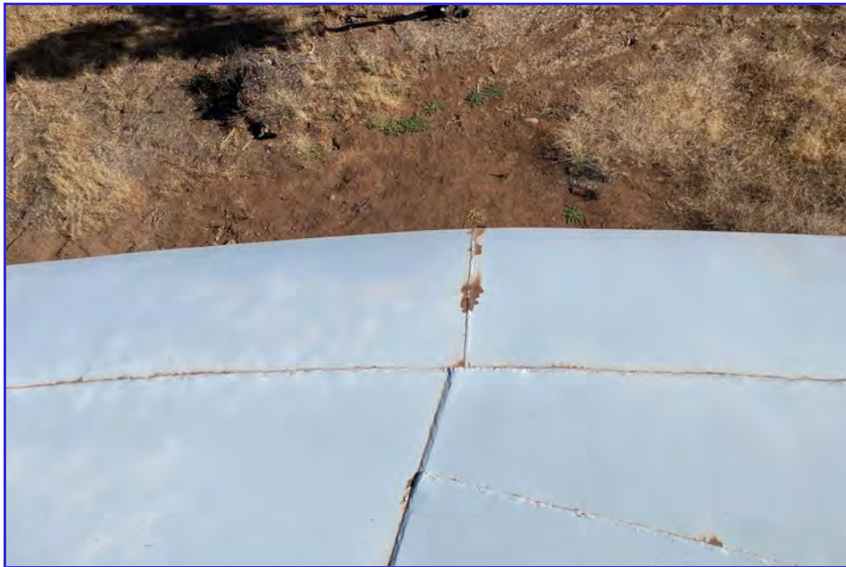
EXTERIOR - CPUD - Mokelumne Reservoir - Maintenance Inspection -034
