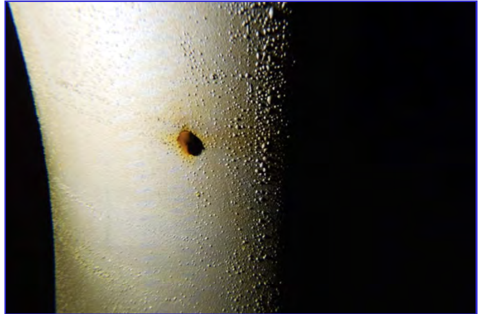
INTERIOR - CPUD - San Andaras Reservoir - Maintenance Inspection -153
