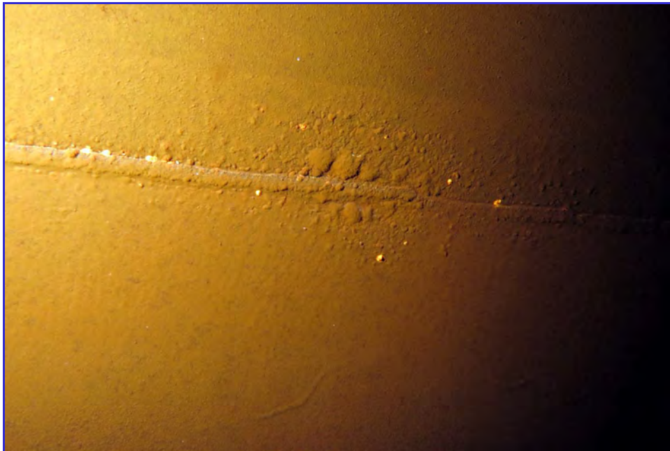
INTERIOR - Calaveras Public Utility District - Clear Well Tank - Maintenance Inspection -070
