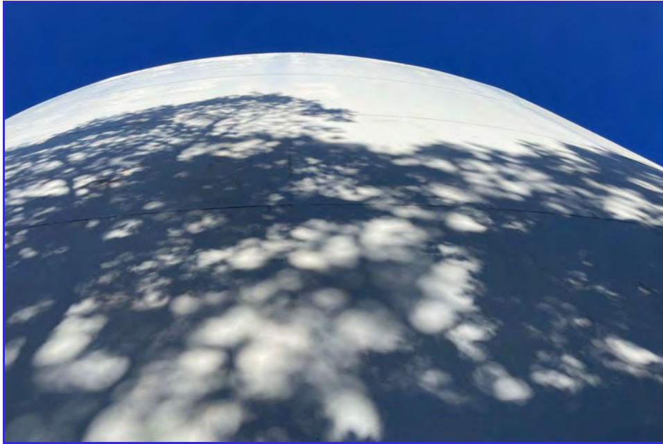
EXTERIOR - CPUD - Mokelumne Reservoir - Maintenance Inspection -164
