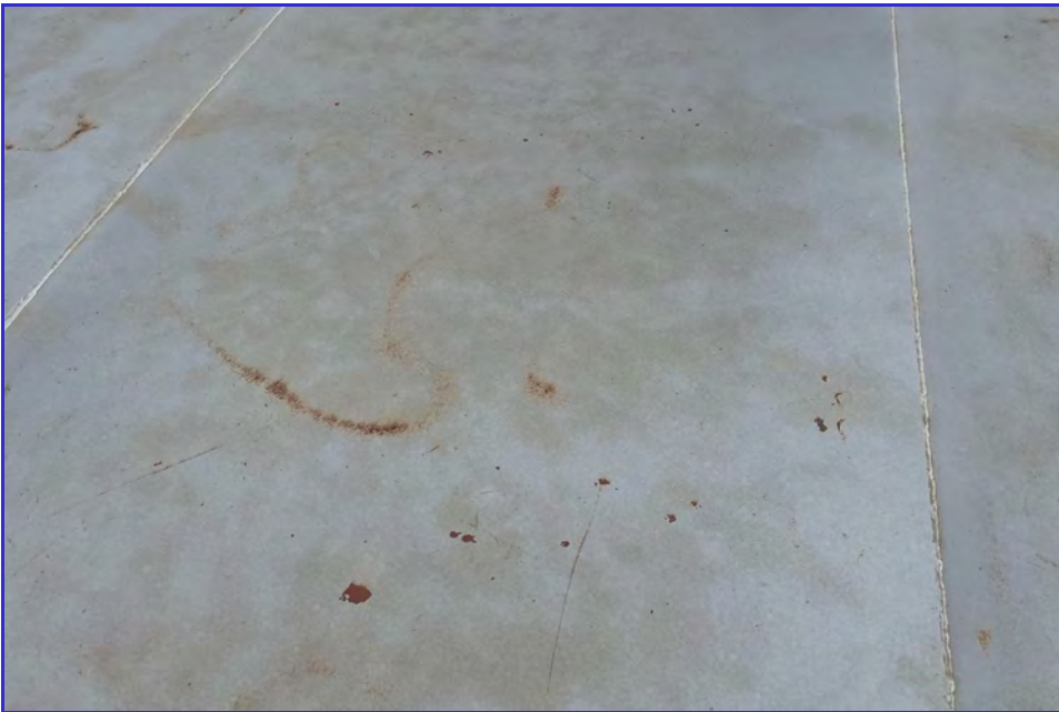
EXTERIOR - CPUD - San Andreas Reservoir - Maintenance Inspection -062
