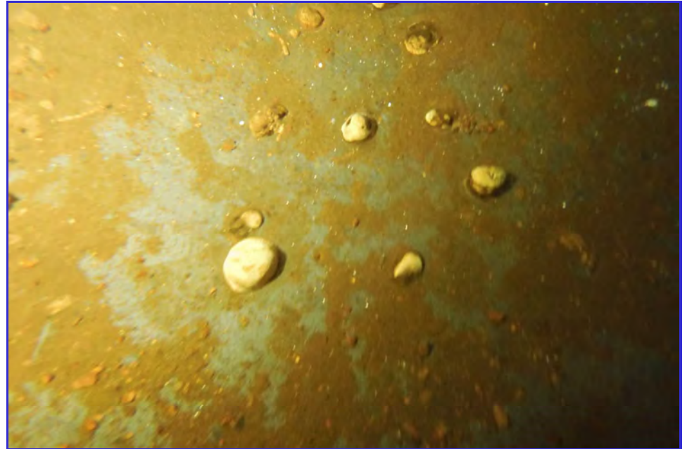
INTERIOR - CPUD - Golden Hills - Maintenance Inspection -101
