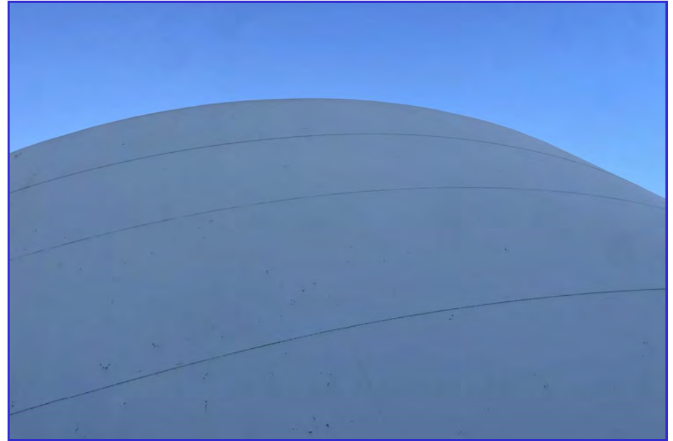
EXTERIOR - CPUD - San Andreas Reservoir - Maintenance Inspection -173
