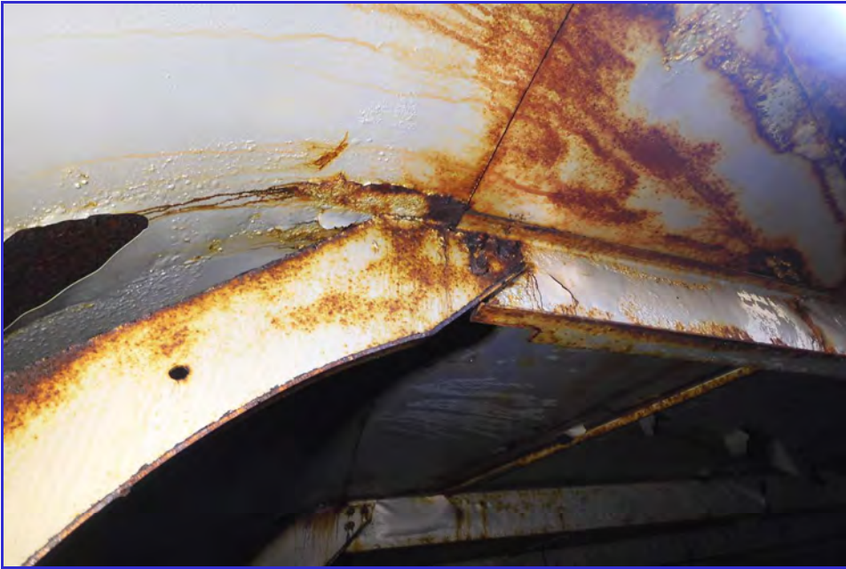
INTERIOR - CPUD - San Andreas Reservoir - Maintenance Inspection
