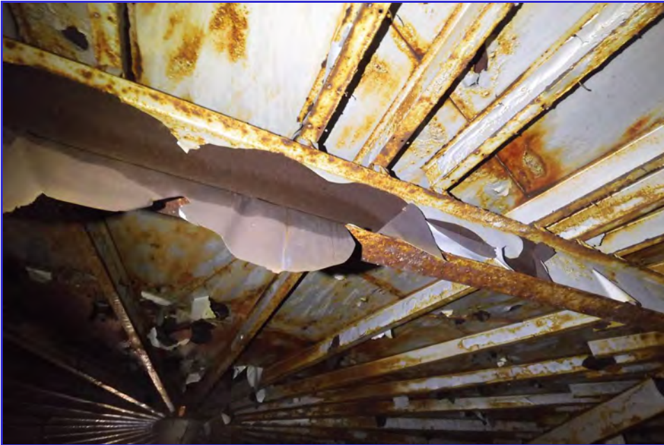
INTERIOR - CPUD - San Andaras Reservoir - Maintenance Inspection -068
