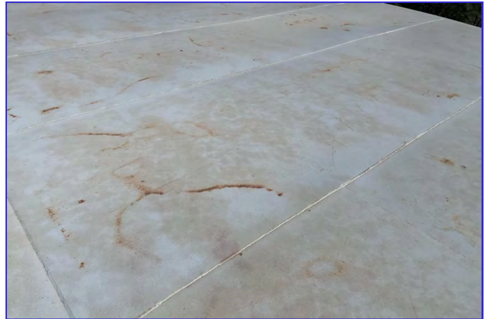
EXTERIOR - CPUD - San Andreas Reservoir - Maintenance Inspection -059
