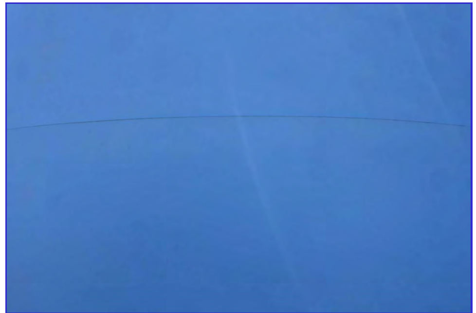
EXTERIOR - CPUD - Railroad Flat Reservoir - Maintenance Inspection -047
