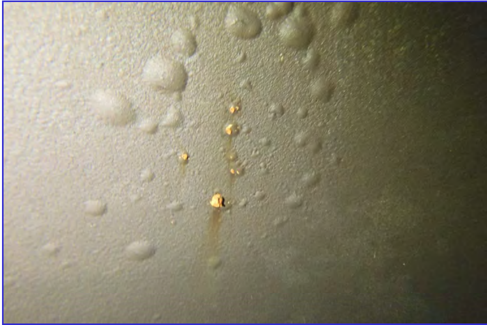
INTERIOR - CPUD - Paloma Reservoir - Maintenance Inspection -048
