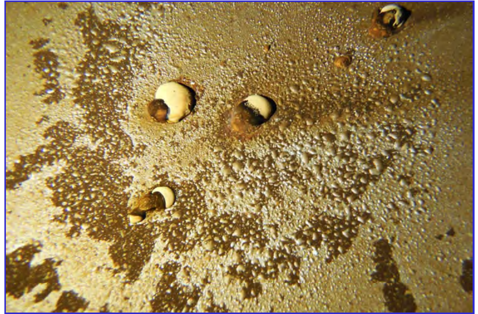
INTERIOR - CPUD - San Andaras Reservoir - Maintenance Inspection -209
