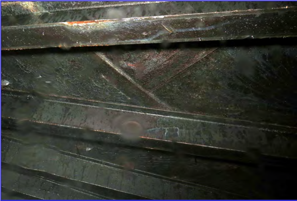
INTERIOR - Calaveras Public Utility District - Clear Well Tank - Maintenance Inspection -024
