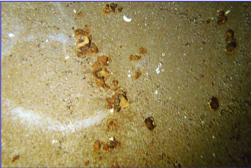
INTERIOR - CPUD - San Andaras Reservoir - Maintenance Inspection -178
