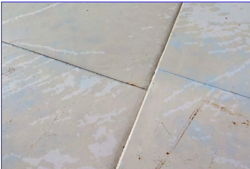
EXTERIOR - Calaveras Public Utility District - Clear Well Tank - Maintenance Inspection -022
