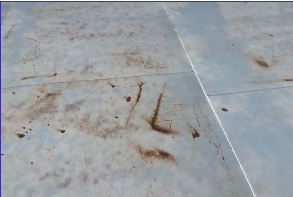
EXTERIOR - CPUD - Mokelumne Reservoir - Maintenance Inspection -018
