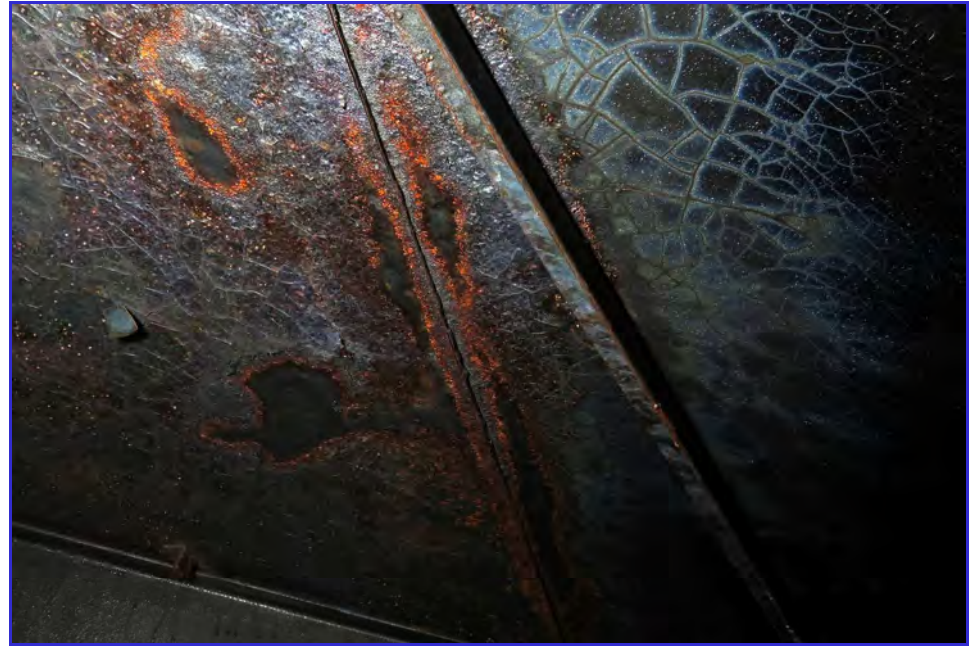
INTERIOR - Calaveras Public Utility District - Clear Well Tank - Maintenance Inspection -041
