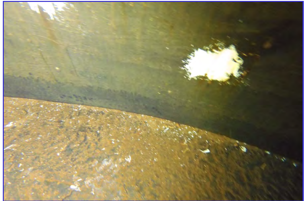
INTERIOR - CPUD - Paloma Reservoir - Maintenance Inspection -103
