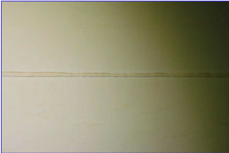
INTERIOR - CPUD - Railroad Flat Reservoir - Maintenance Inspection -070
