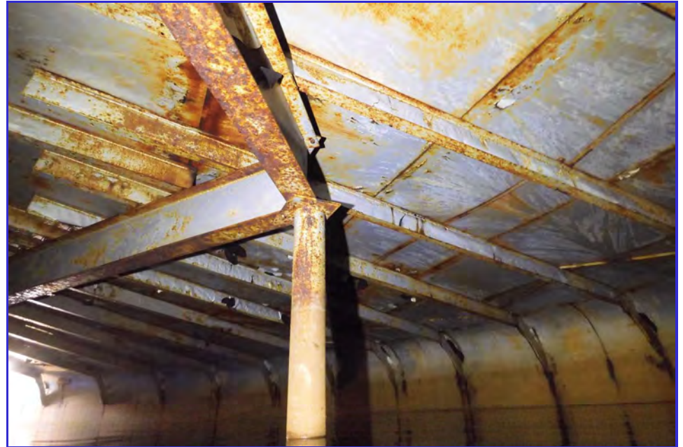
INTERIOR - CPUD - San Andaras Reservoir - Maintenance Inspection -089
