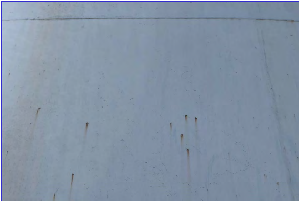
EXTERIOR - CPUD - Mokelumne Reservoir - Maintenance Inspection -134
