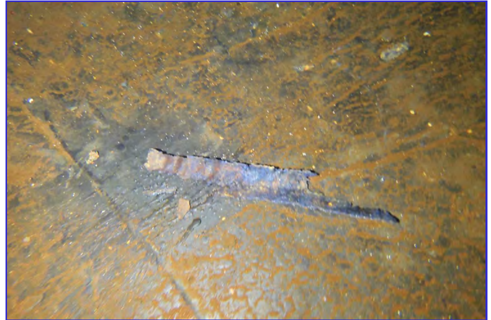
INTERIOR - CPUD - Paloma Reservoir - Maintenance Inspection -109
