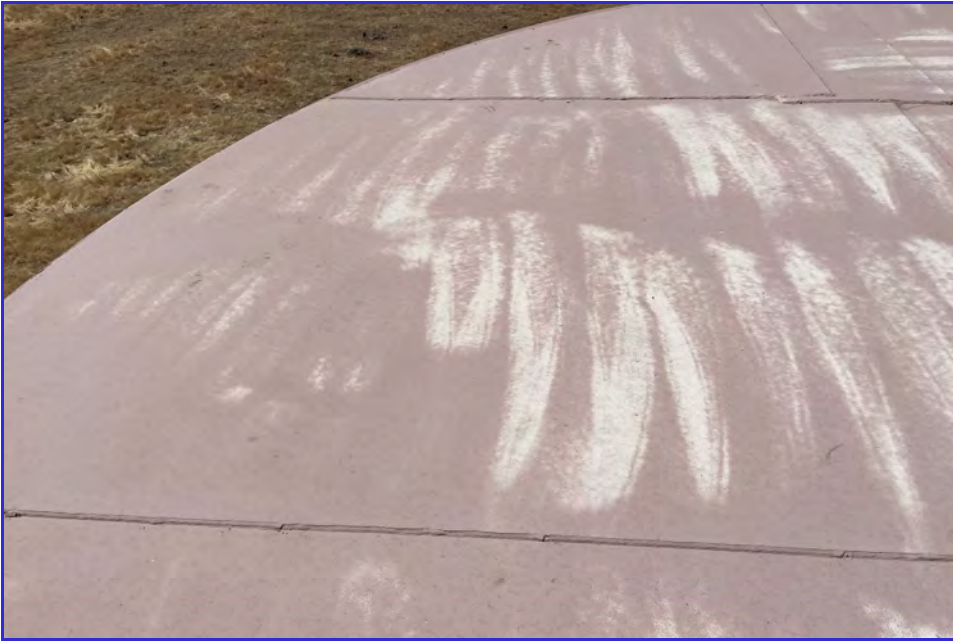
EXTERIOR - CPUD - Paloma Reservoir - Maintenance Inspection -008
