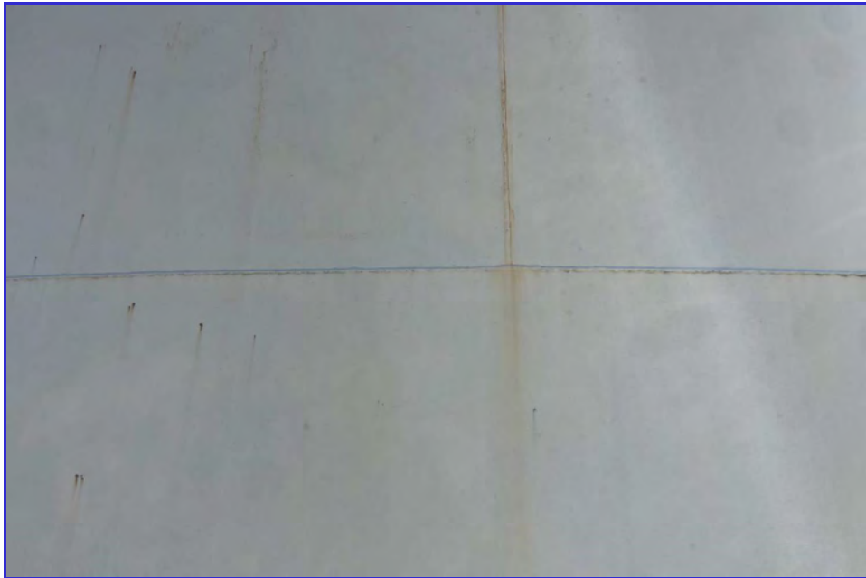
EXTERIOR - CPUD - Mokelumne Reservoir - Maintenance Inspection -108
