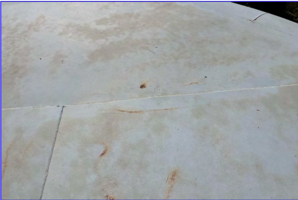
EXTERIOR - CPUD - San Andreas Reservoir - Maintenance Inspection -038
