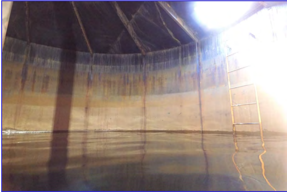
INTERIOR - CPUD - Golden Hills - Maintenance Inspection -012
