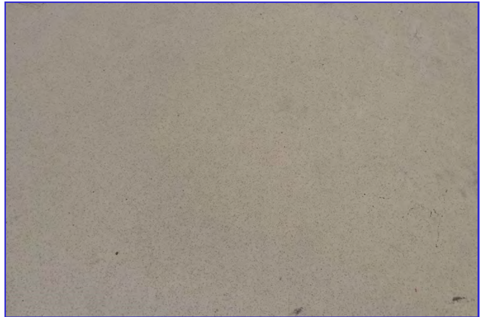
EXTERIOR - CPUD - Golden Hills - Maintenance Inspection -011
