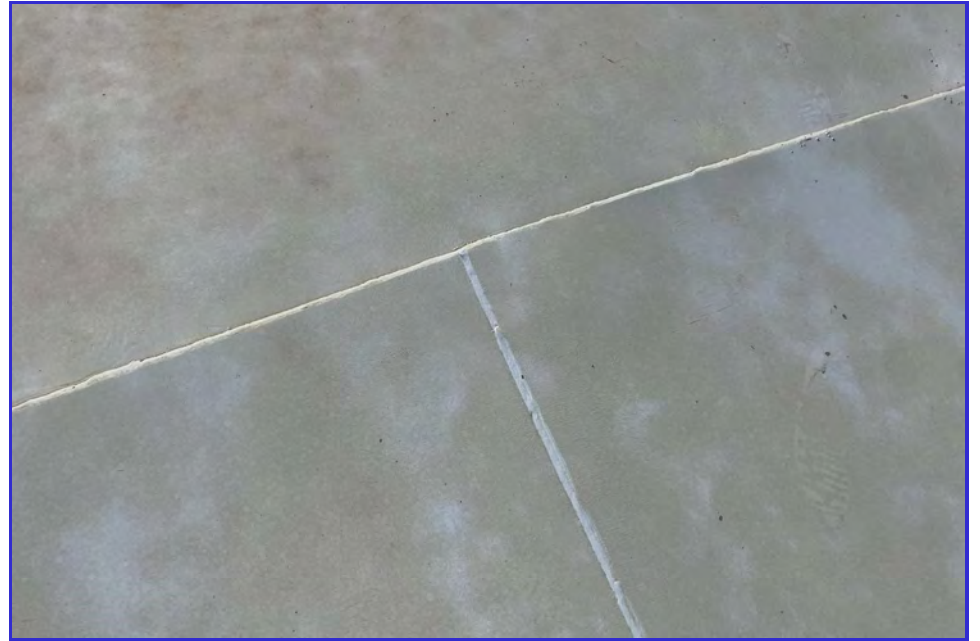
EXTERIOR - CPUD - San Andreas Reservoir - Maintenance Inspection -073
