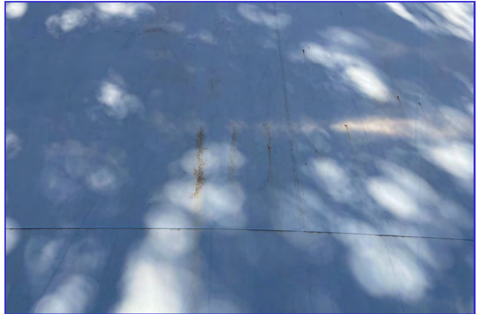
EXTERIOR - CPUD - Mokelumne Reservoir - Maintenance Inspection -169
