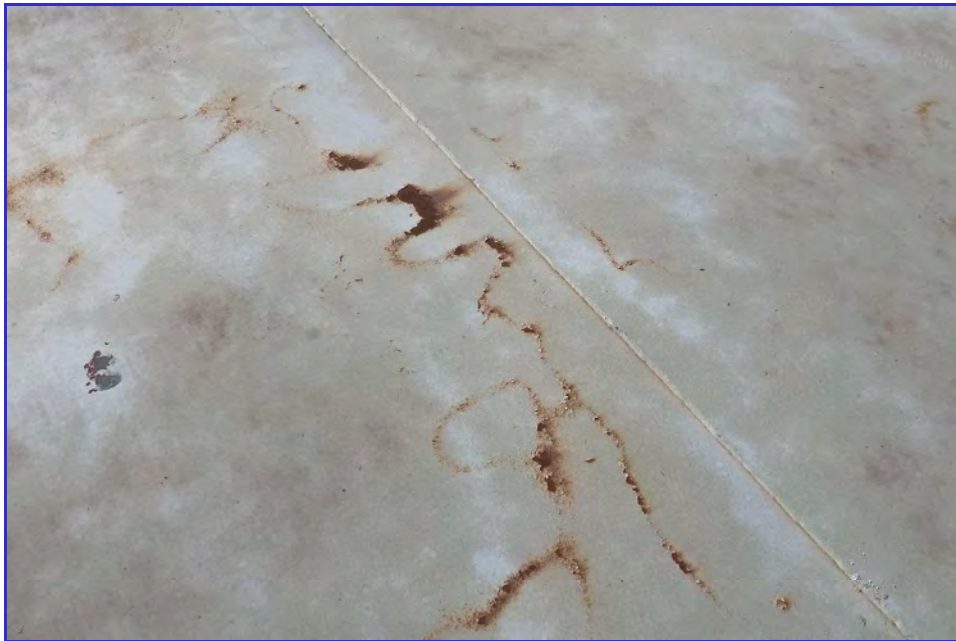
EXTERIOR - CPUD - San Andreas Reservoir - Maintenance Inspection -022
