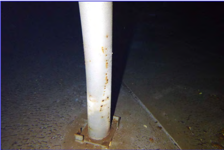
INTERIOR - CPUD - San Andaras Reservoir - Maintenance Inspection -146
