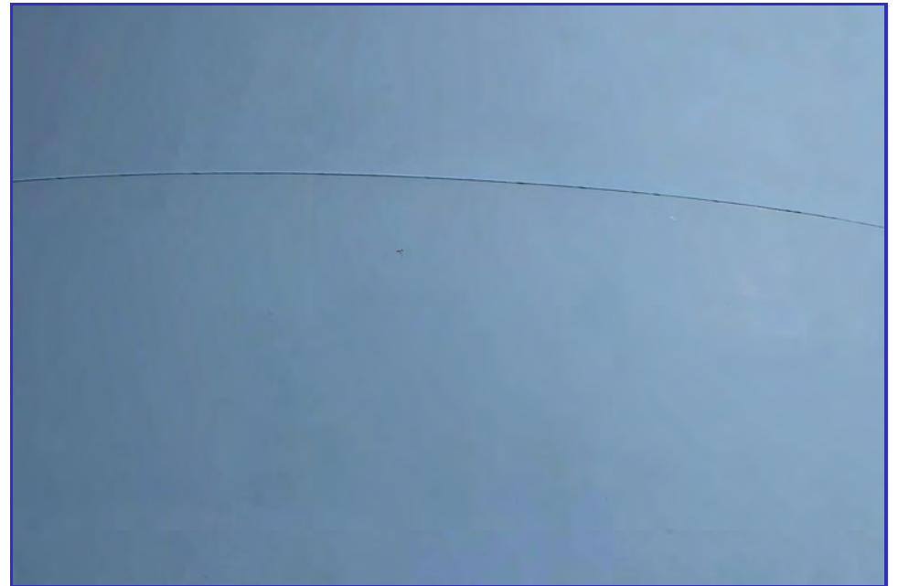
EXTERIOR - CPUD - Railroad Flat Reservoir - Maintenance Inspection -055
