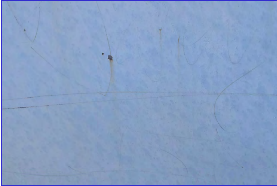
EXTERIOR - CPUD - San Andreas Reservoir - Maintenance Inspection -116
