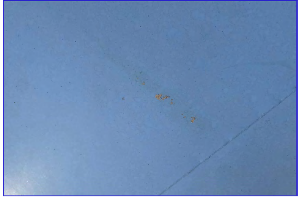
EXTERIOR - CPUD - Railroad Flat Reservoir - Maintenance Inspection -041
