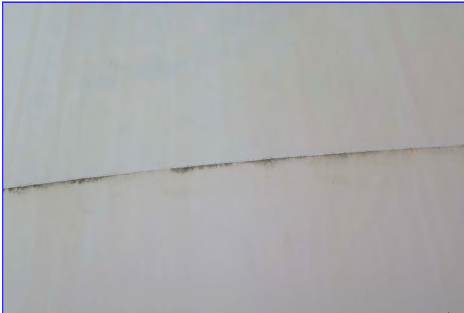
EXTERIOR - Calaveras Public Utility District - Clear Well Tank - Maintenance Inspection -102
