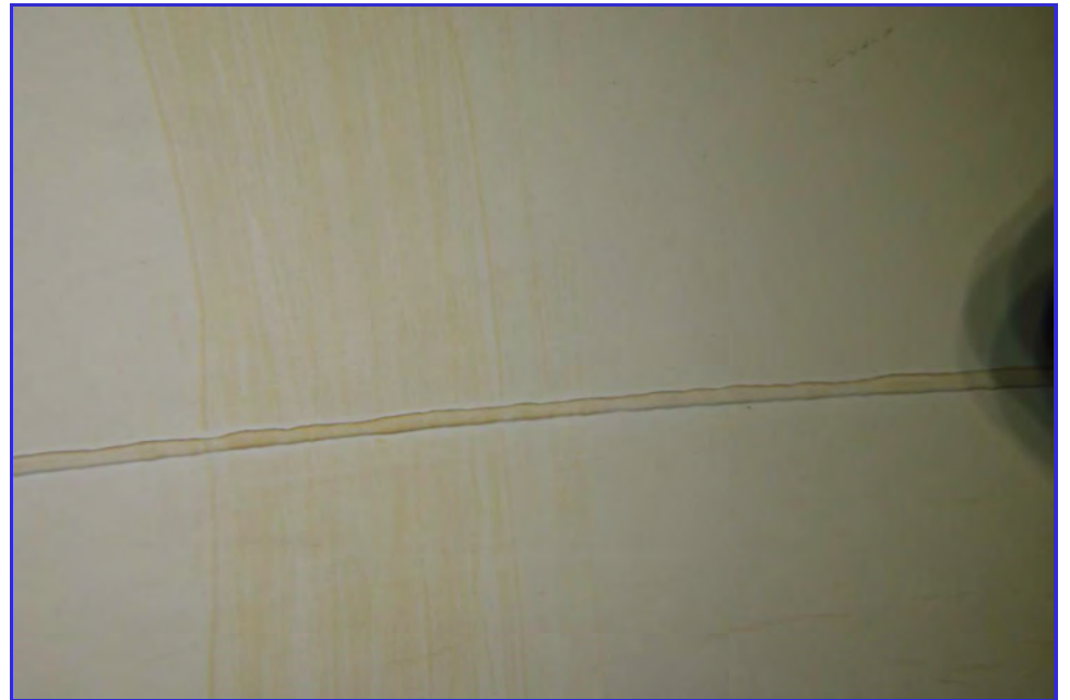
INTERIOR - CPUD - Railroad Flat Reservoir - Maintenance Inspection -071
