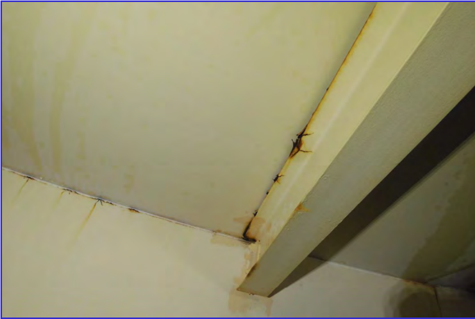
INTERIOR - CPUD - Railroad Flat Reservoir - Maintenance Inspection -064
