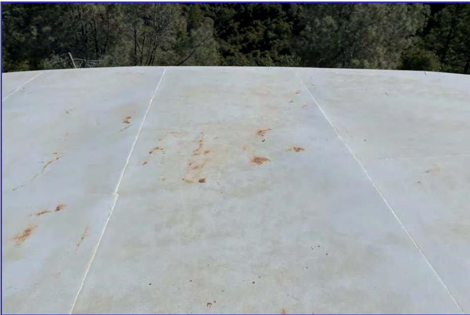
EXTERIOR - CPUD - San Andreas Reservoir - Maintenance Inspection -090
