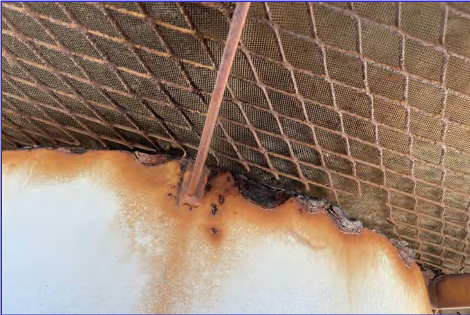
EXTERIOR - CPUD - San Andreas Reservoir - Maintenance Inspection -088
