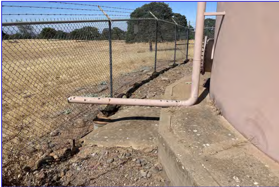
EXTERIOR - CPUD - Paloma Reservoir - Maintenance Inspection -050
