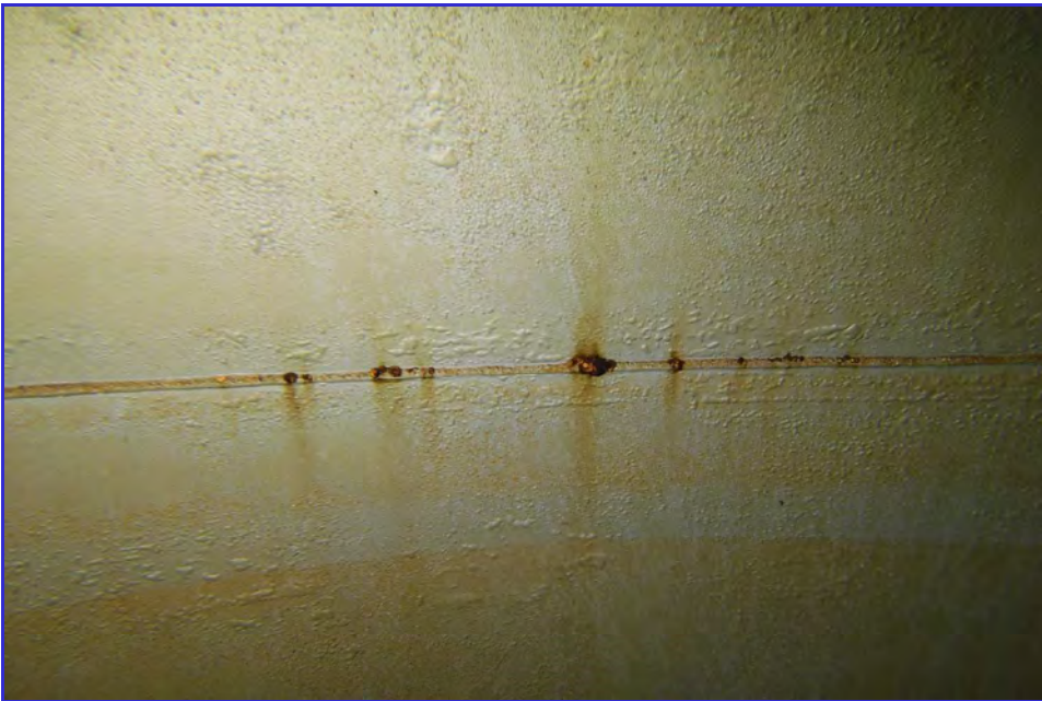
INTERIOR - CPUD - San Andaras Reservoir - Maintenance Inspection -114
