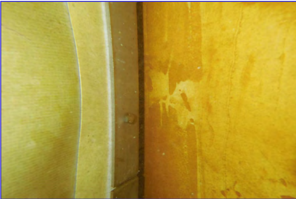
INTERIOR - CPUD - Railroad Flat Reservoir - Maintenance Inspection -142
