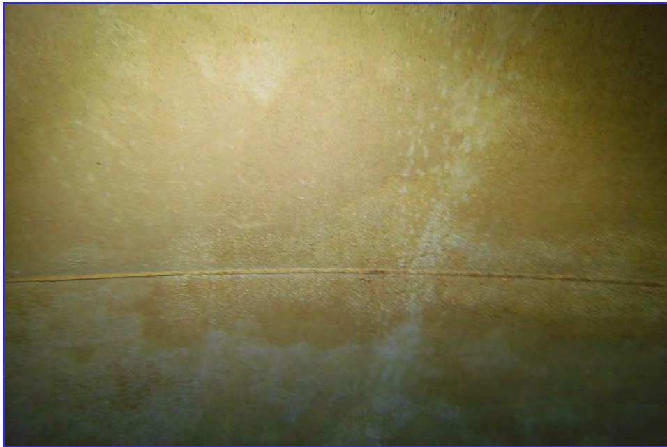
INTERIOR - CPUD - San Andaras Reservoir - Maintenance Inspection -118
