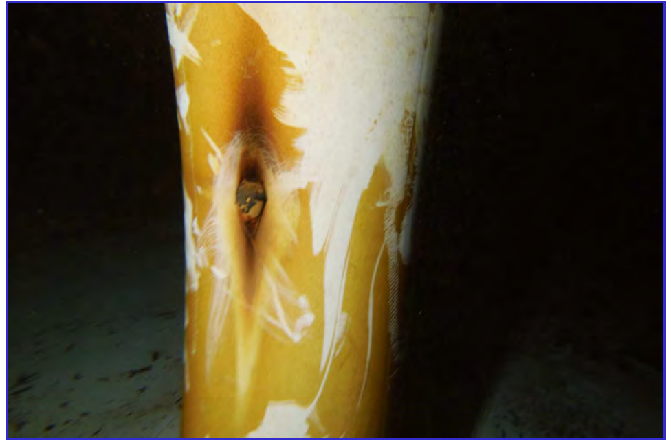
INTERIOR - CPUD - Railroad Flat Reservoir - Maintenance Inspection -137
