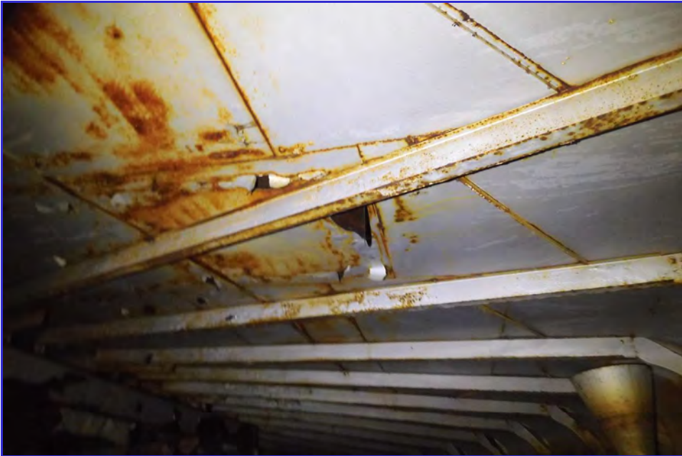
INTERIOR - CPUD - San Andaras Reservoir - Maintenance Inspection -036
