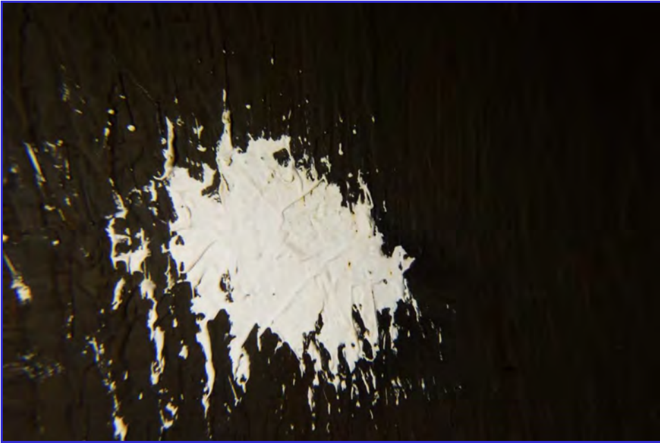
INTERIOR - CPUD - Paloma Reservoir - Maintenance Inspection -100
