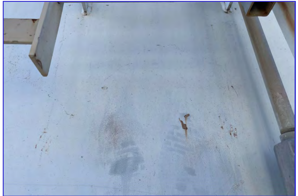
EXTERIOR - CPUD - Mokelumne Reservoir - Maintenance Inspection -131
