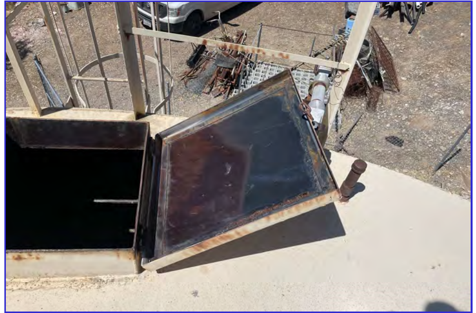
EXTERIOR - CPUD - Golden Hills - Maintenance Inspection -021
