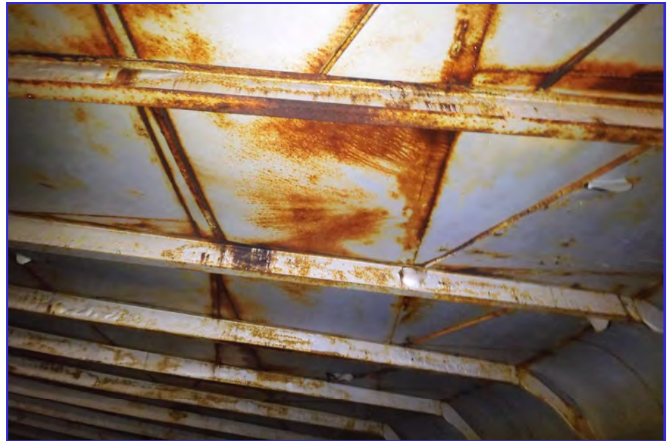
INTERIOR - CPUD - San Andaras Reservoir - Maintenance Inspection -011
