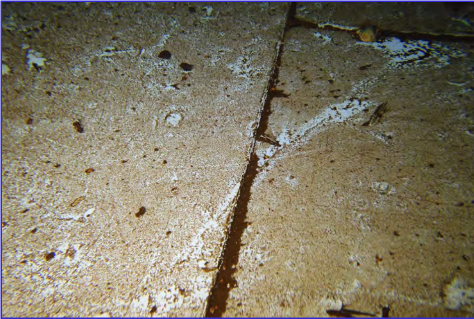
INTERIOR - CPUD - Mokelumne Hill Reservoir - Maintenance Inspection -136
