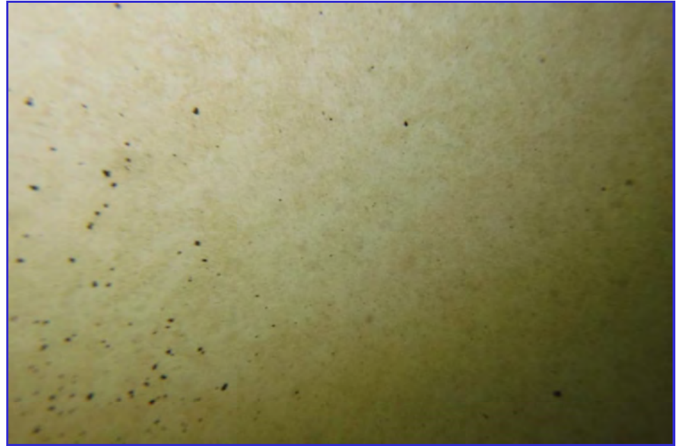
INTERIOR - CPUD - Railroad Flat Reservoir - Maintenance Inspection -129
