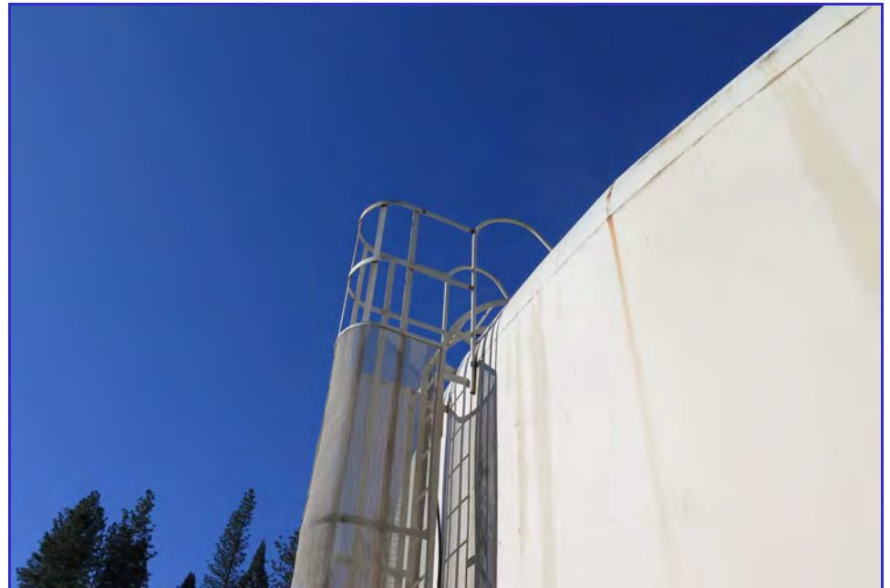
EXTERIOR - Calaveras Public Utility District - Clear Well Tank - Maintenance Inspection -123
