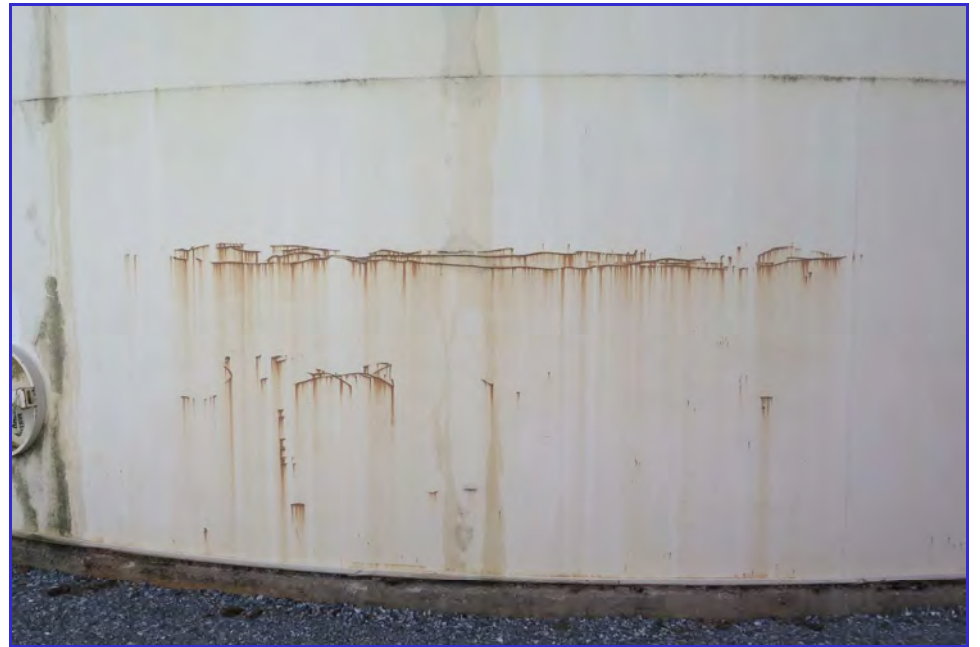
EXTERIOR - Calaveras Public Utility District - Clear Well Tank - Maintenance Inspection -107
