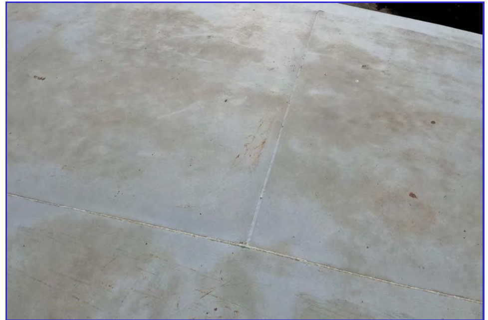
EXTERIOR - CPUD - San Andreas Reservoir - Maintenance Inspection -051
