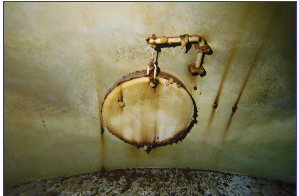
INTERIOR - CPUD - Mokelumne Hill Reservoir - Maintenance Inspection -127
