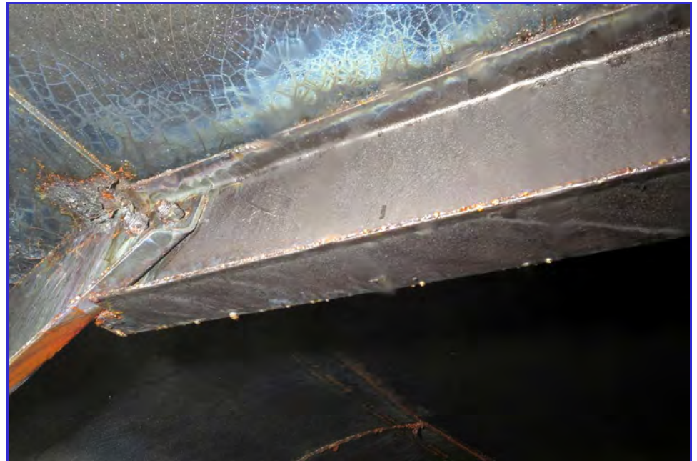
INTERIOR - Calaveras Public Utility District - Clear Well Tank - Maintenance Inspection -043
