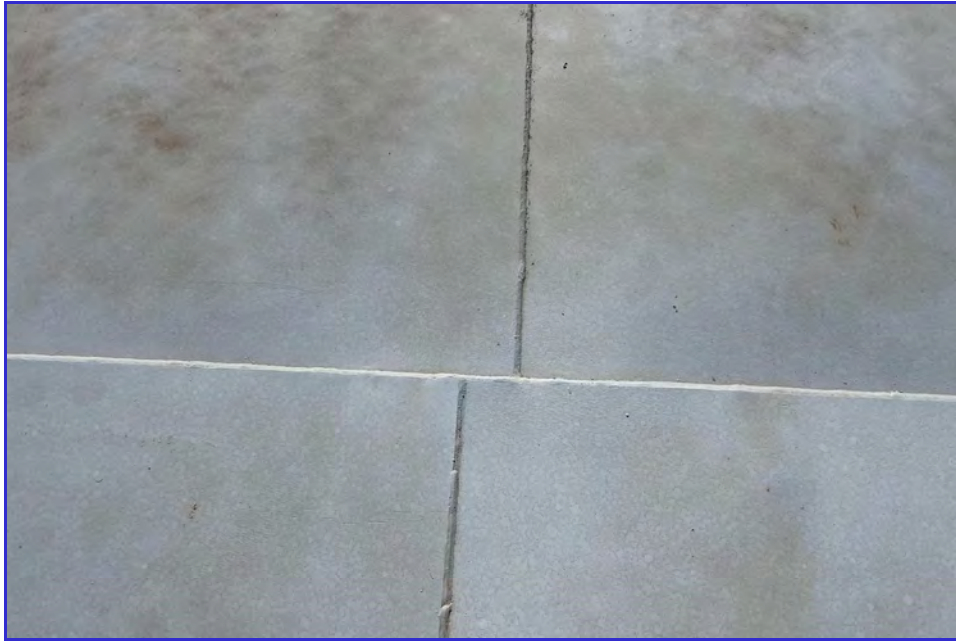
EXTERIOR - CPUD - San Andreas Reservoir - Maintenance Inspection -012
