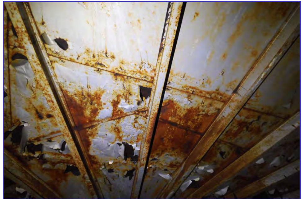
INTERIOR - CPUD - San Andaras Reservoir - Maintenance Inspection -087
