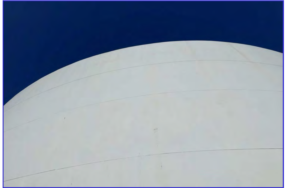
EXTERIOR - CPUD - San Andreas Reservoir - Maintenance Inspection -185
