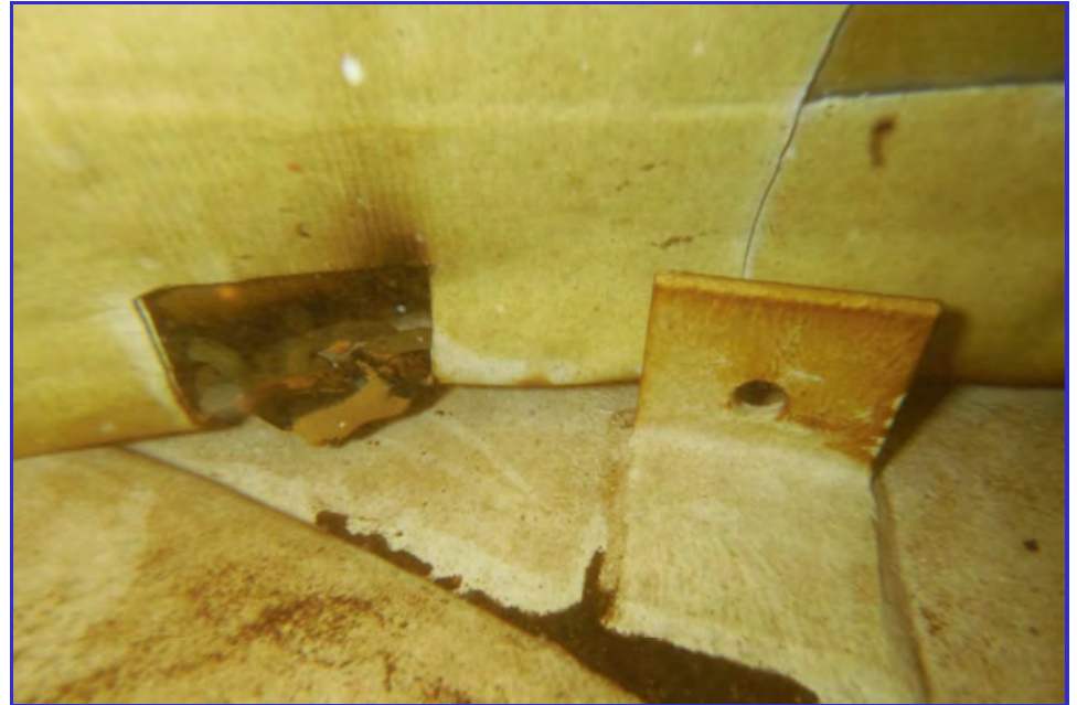
INTERIOR - CPUD - Railroad Flat Reservoir - Maintenance Inspection -145
