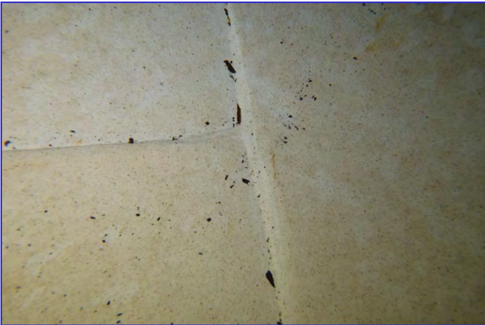
INTERIOR - CPUD - Railroad Flat Reservoir - Maintenance Inspection -134
