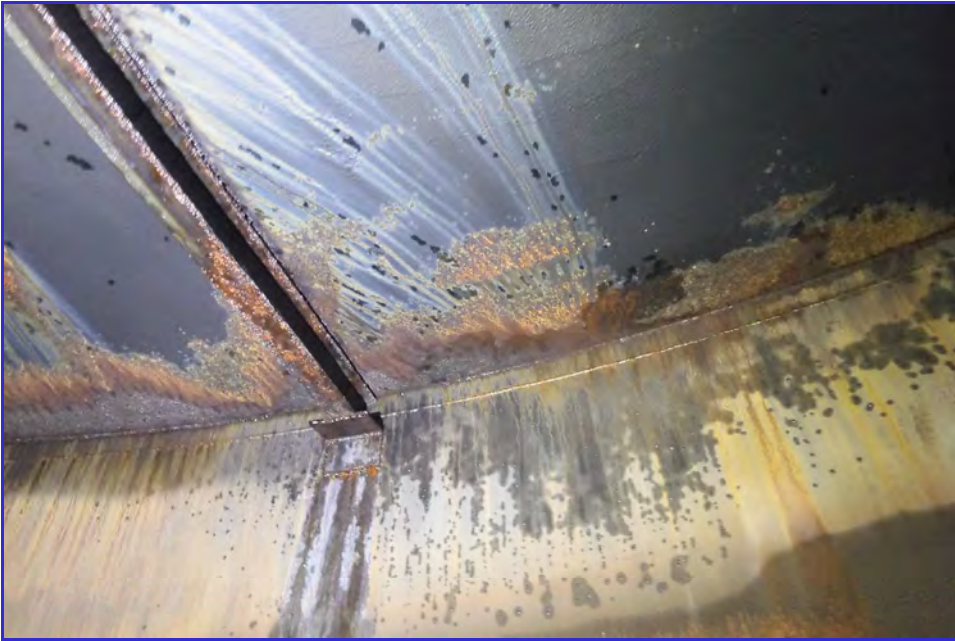
INTERIOR - CPUD - Paloma Reservoir - Maintenance Inspection -044
