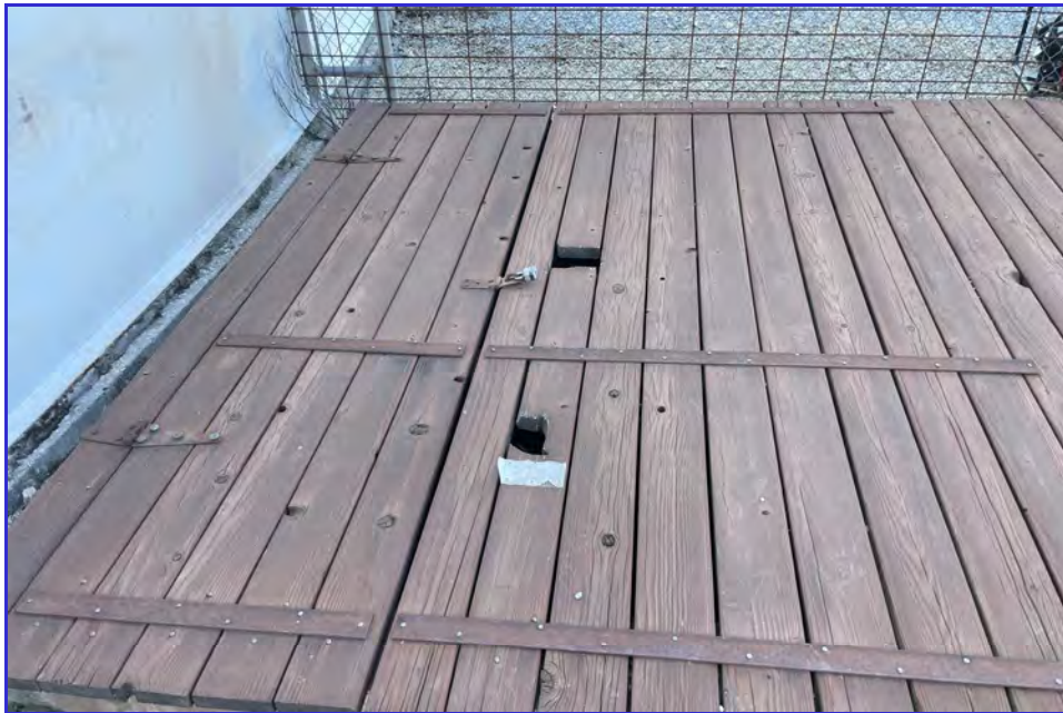
EXTERIOR - CPUD - San Andreas Reservoir - Maintenance Inspection -174
