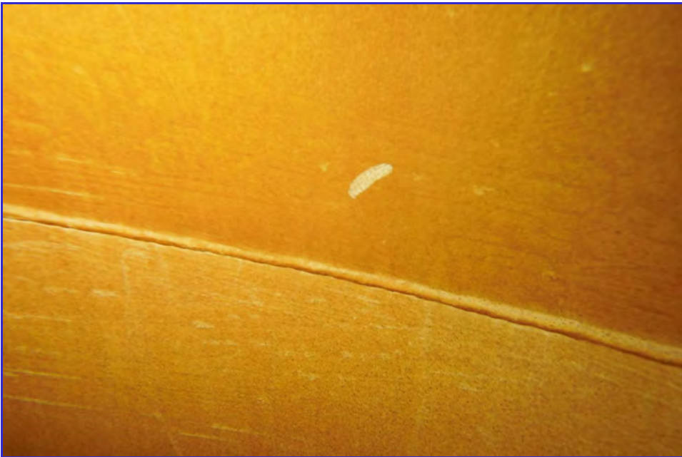
INTERIOR - CPUD - Railroad Flat Reservoir - Maintenance Inspection -082
