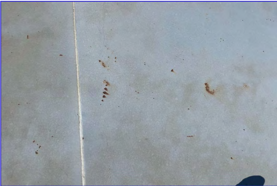
EXTERIOR - CPUD - San Andreas Reservoir - Maintenance Inspection -070
