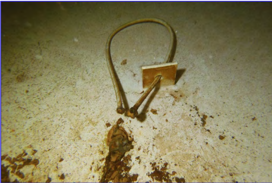
INTERIOR - CPUD - Railroad Flat Reservoir - Maintenance Inspection -118
