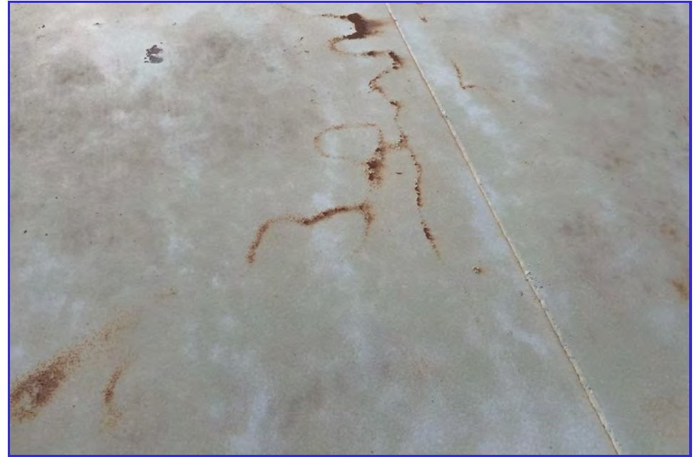
EXTERIOR - CPUD - San Andreas Reservoir - Maintenance Inspection -021
