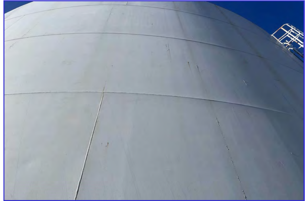
EXTERIOR - CPUD - Mokelumne Reservoir - Maintenance Inspection -177
