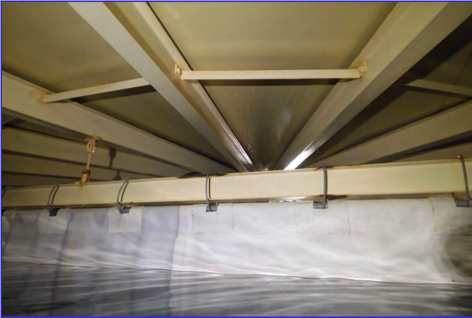
INTERIOR - CPUD - Railroad Flat Reservoir - Maintenance Inspection -060
