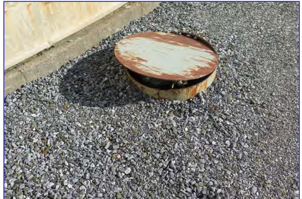
EXTERIOR - Calaveras Public Utility District - Clear Well Tank - Maintenance Inspection -071
