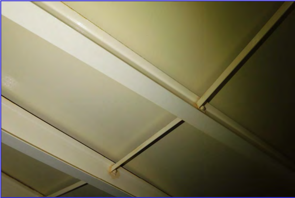
INTERIOR - CPUD - Railroad Flat Reservoir - Maintenance Inspection -048
