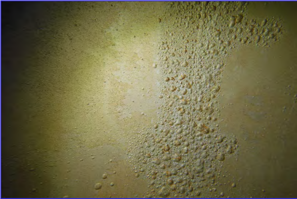
INTERIOR - CPUD - San Andaras Reservoir - Maintenance Inspection -120
