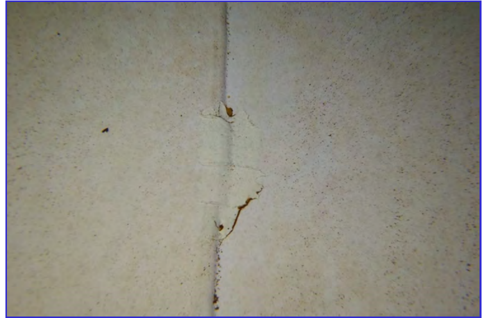
INTERIOR - CPUD - Railroad Flat Reservoir - Maintenance Inspection -153
