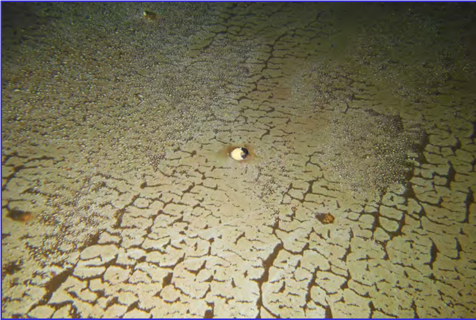
INTERIOR - CPUD - San Andaras Reservoir - Maintenance Inspection -228
