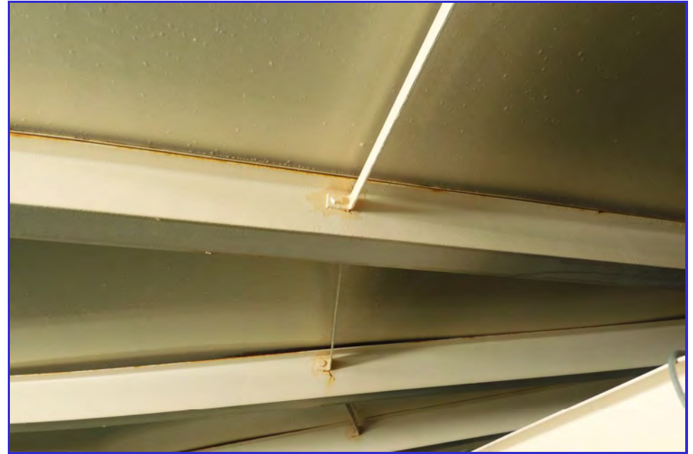
INTERIOR - CPUD - Railroad Flat Reservoir - Maintenance Inspection -017
