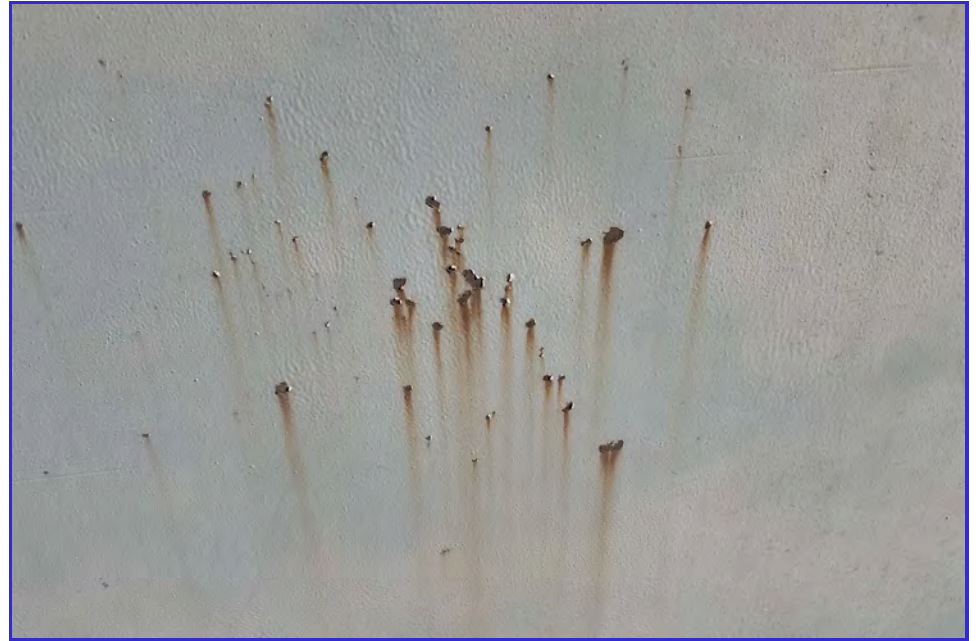
EXTERIOR - CPUD - Mokelumne Reservoir - Maintenance Inspection -105
