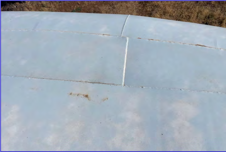
EXTERIOR - CPUD - Mokelumne Reservoir - Maintenance Inspection -004
