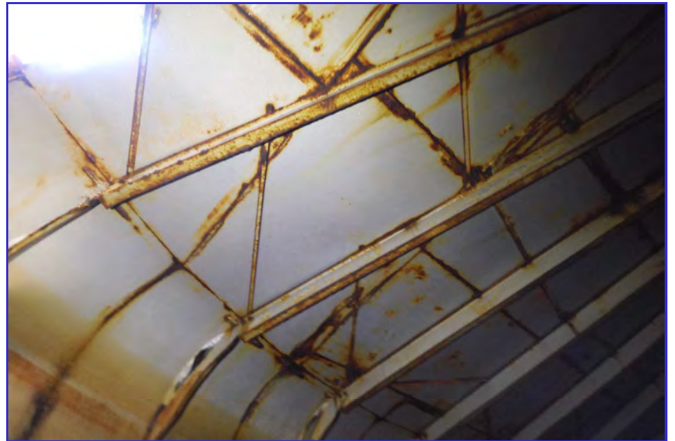
INTERIOR - CPUD - Mokelumne Hill Reservoir - Maintenance Inspection -003
