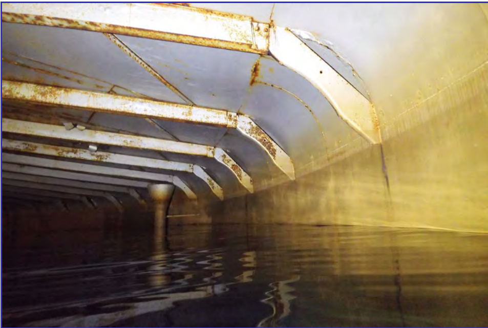
INTERIOR - CPUD - San Andaras Reservoir - Maintenance Inspection -030
