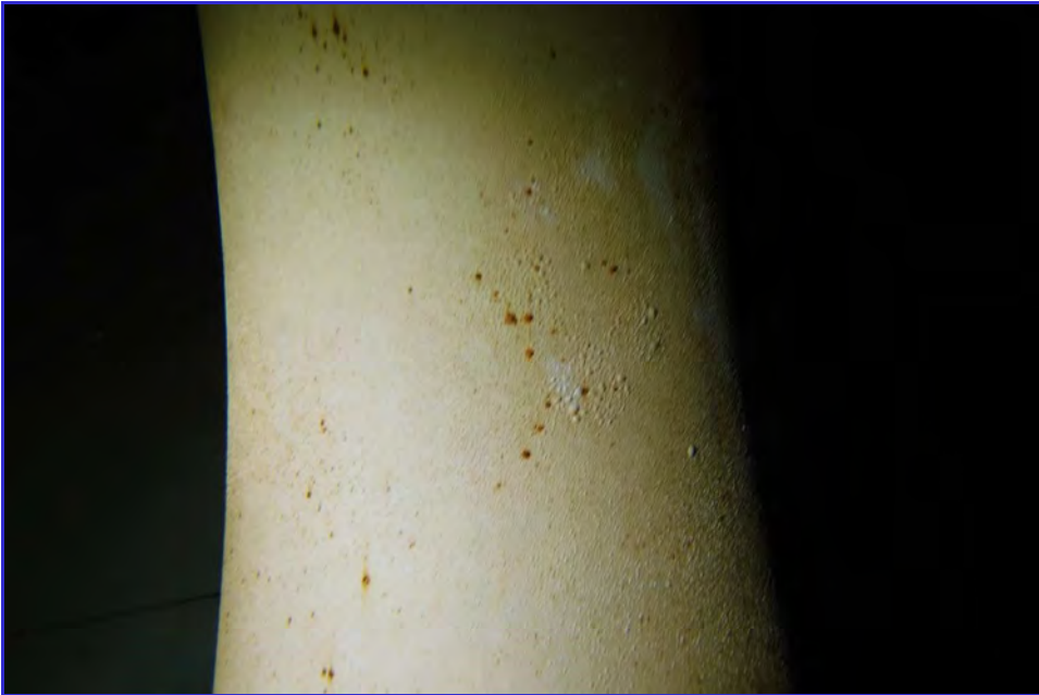
INTERIOR - CPUD - Mokelumne Hill Reservoir - Maintenance Inspection -112
