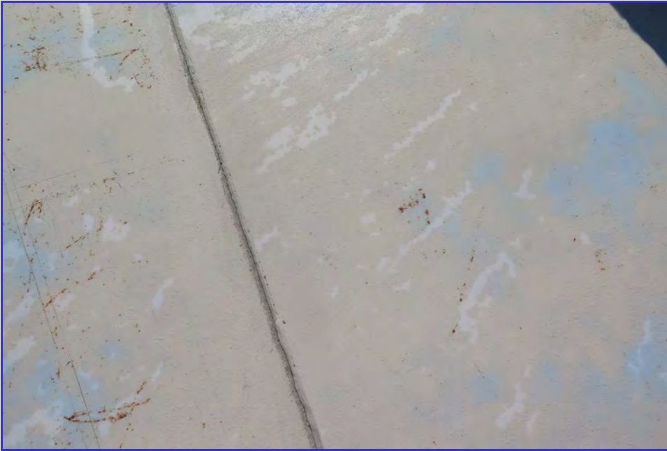
EXTERIOR - Calaveras Public Utility District - Clear Well Tank - Maintenance Inspection -048
