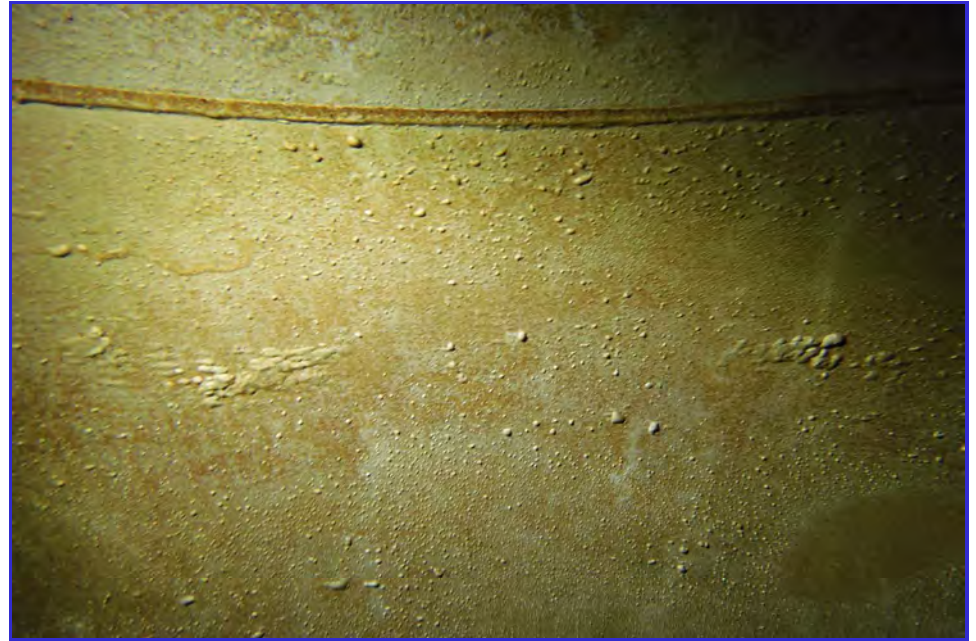
INTERIOR - CPUD - San Andaras Reservoir - Maintenance Inspection -141
