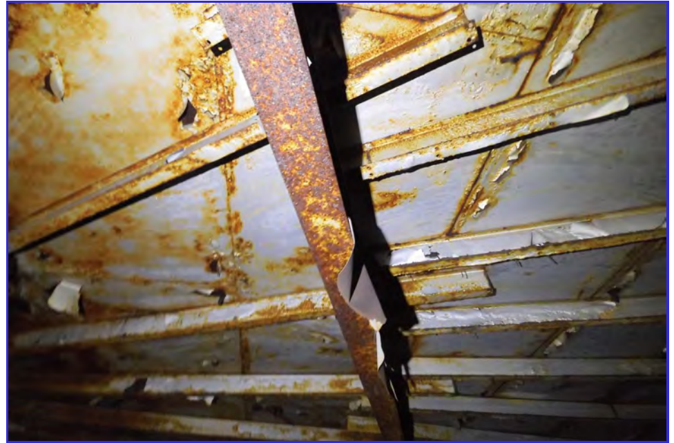
INTERIOR - CPUD - San Andaras Reservoir - Maintenance Inspection -065
