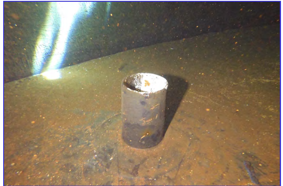
INTERIOR - CPUD - Paloma Reservoir - Maintenance Inspection -139
