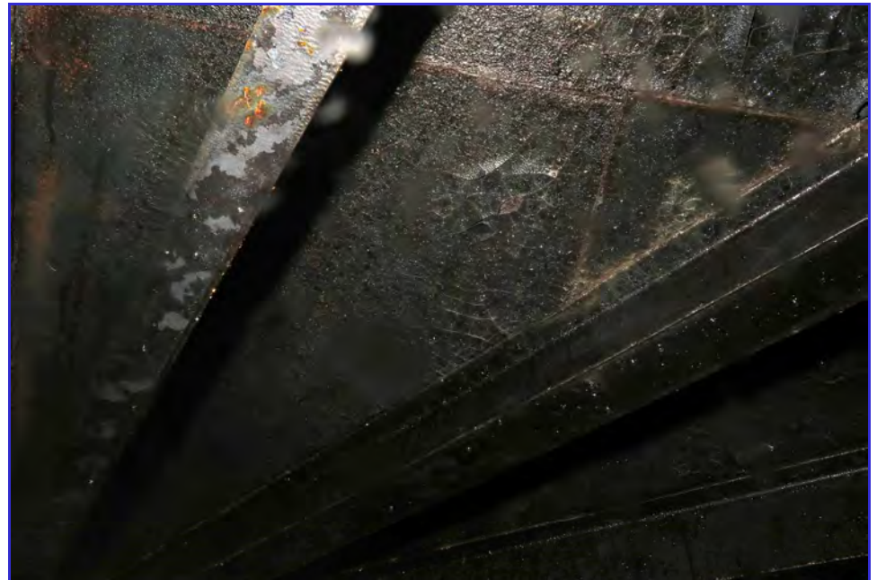
INTERIOR - Calaveras Public Utility District - Clear Well Tank - Maintenance Inspection -023
