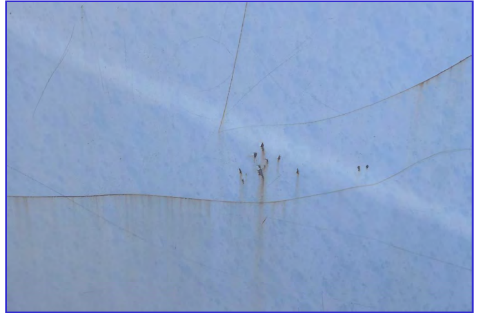
EXTERIOR - CPUD - San Andreas Reservoir - Maintenance Inspection -113
