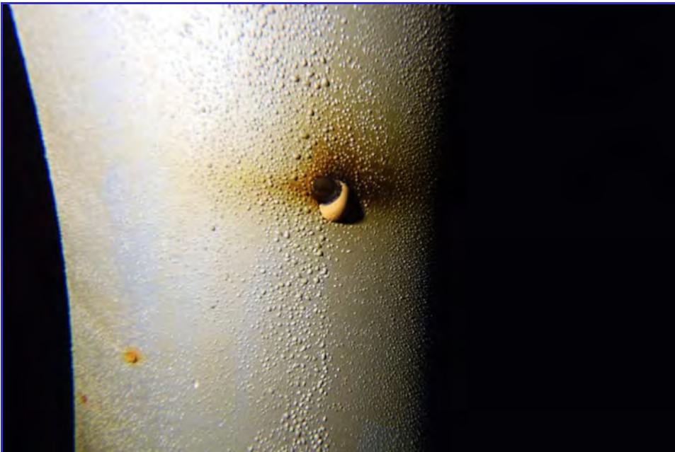
INTERIOR - CPUD - San Andaras Reservoir - Maintenance Inspection -154
