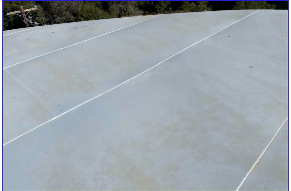
EXTERIOR - CPUD - San Andreas Reservoir - Maintenance Inspection -089
