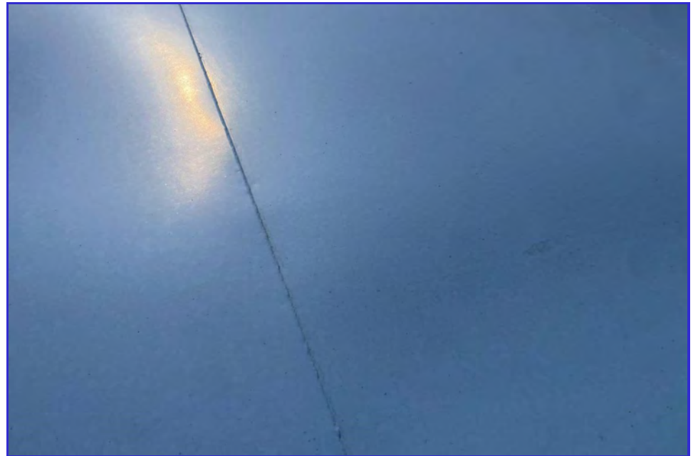
EXTERIOR - CPUD - Railroad Flat Reservoir - Maintenance Inspection -039
