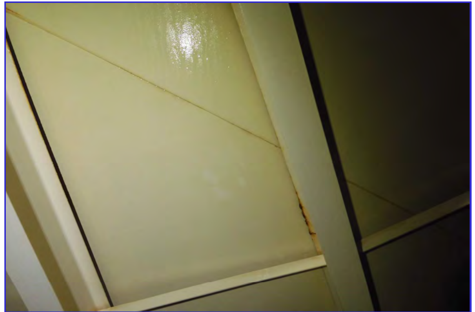
INTERIOR - CPUD - Railroad Flat Reservoir - Maintenance Inspection -047
