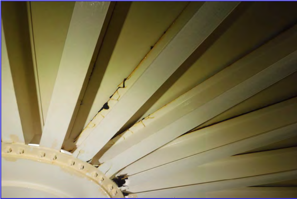
INTERIOR - CPUD - Railroad Flat Reservoir - Maintenance Inspection -040
