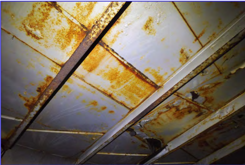
INTERIOR - CPUD - San Andaras Reservoir - Maintenance Inspection -050
