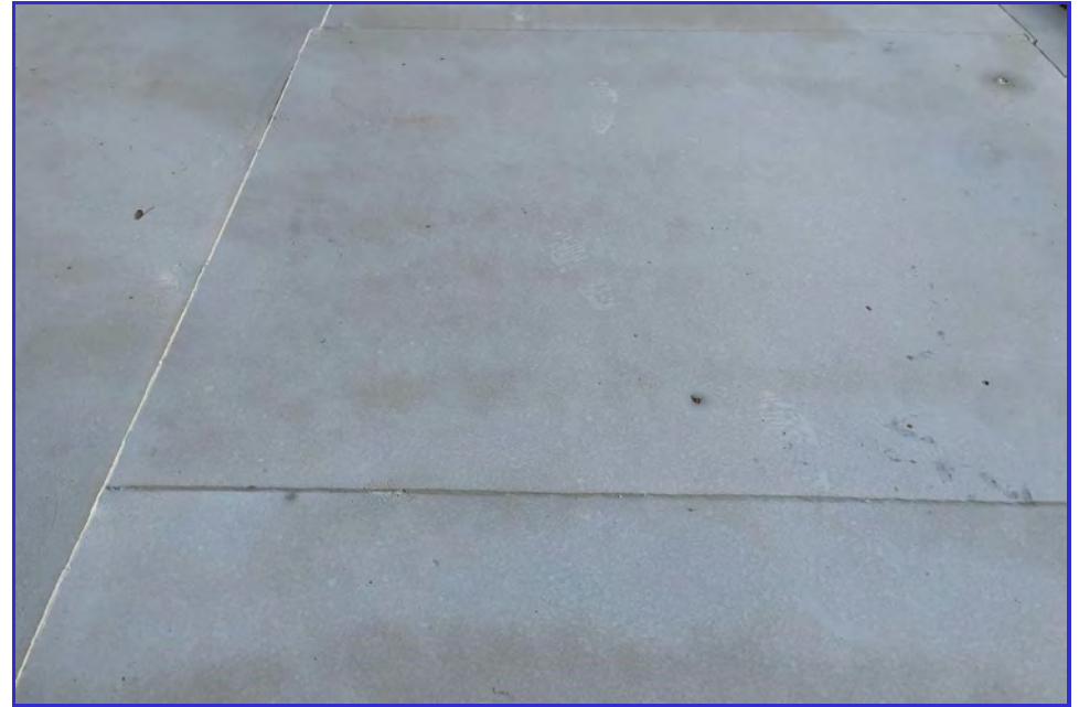
EXTERIOR - CPUD - San Andreas Reservoir - Maintenance Inspection -005
