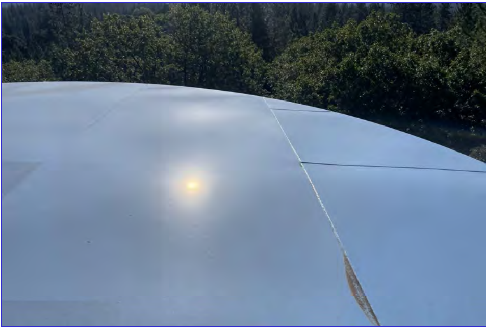
EXTERIOR - CPUD - Railroad Flat Reservoir - Maintenance Inspection -034
