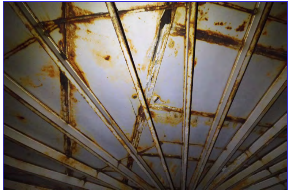
INTERIOR - CPUD - Mokelumne Hill Reservoir - Maintenance Inspection -055
