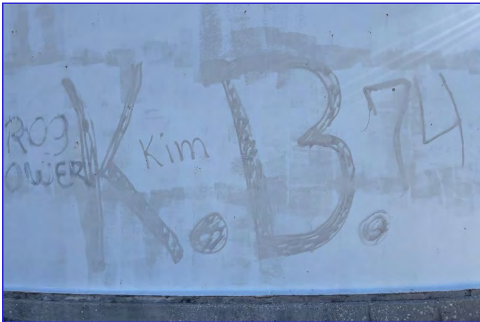
EXTERIOR - CPUD - San Andreas Reservoir - Maintenance Inspection -158
