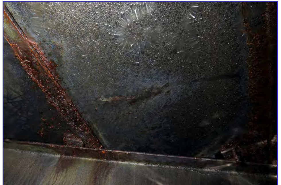
INTERIOR - Calaveras Public Utility District - Clear Well Tank - Maintenance Inspection -003
