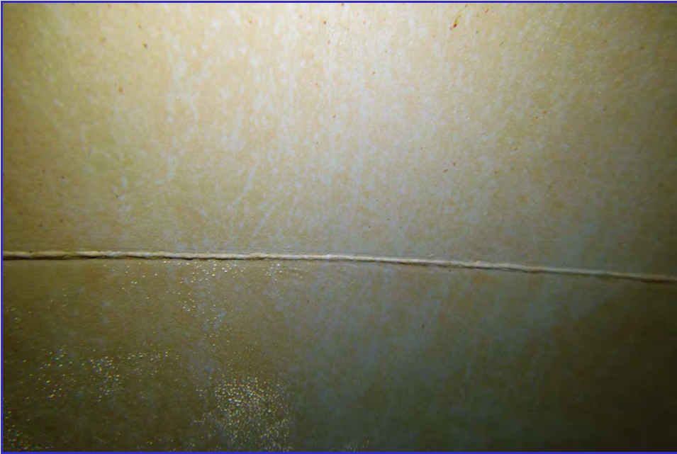
INTERIOR - CPUD - Mokelumne Hill Reservoir - Maintenance Inspection -084
