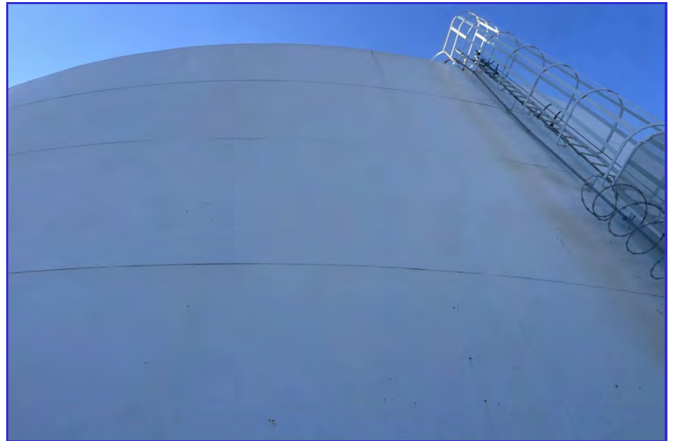
EXTERIOR - CPUD - San Andreas Reservoir - Maintenance Inspection -191
