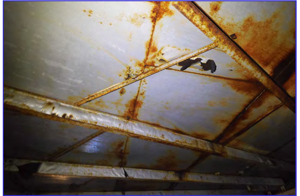
INTERIOR - CPUD - San Andaras Reservoir - Maintenance Inspection -021
