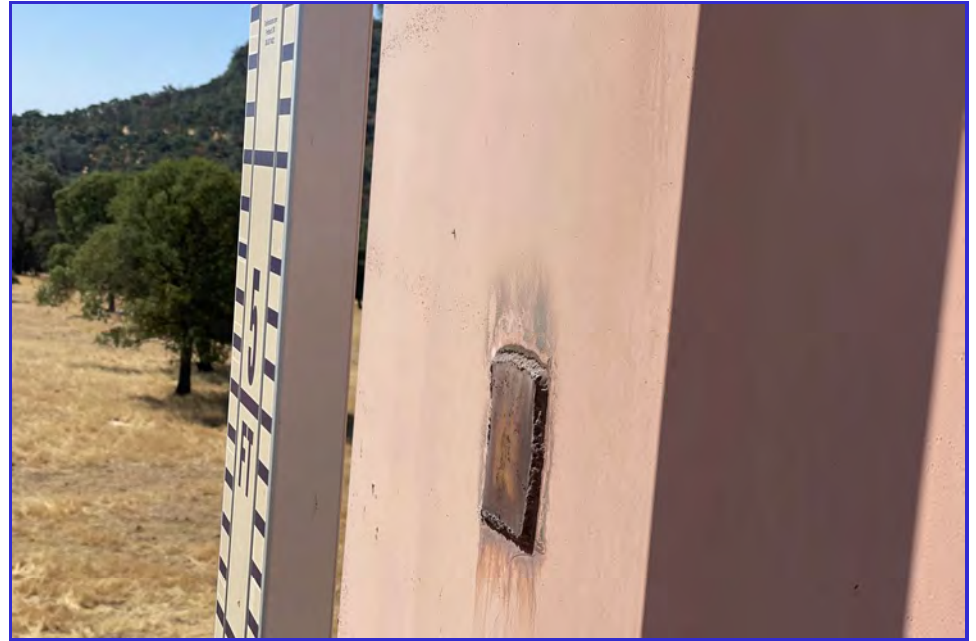
EXTERIOR - CPUD - Paloma Reservoir - Maintenance Inspection -057
