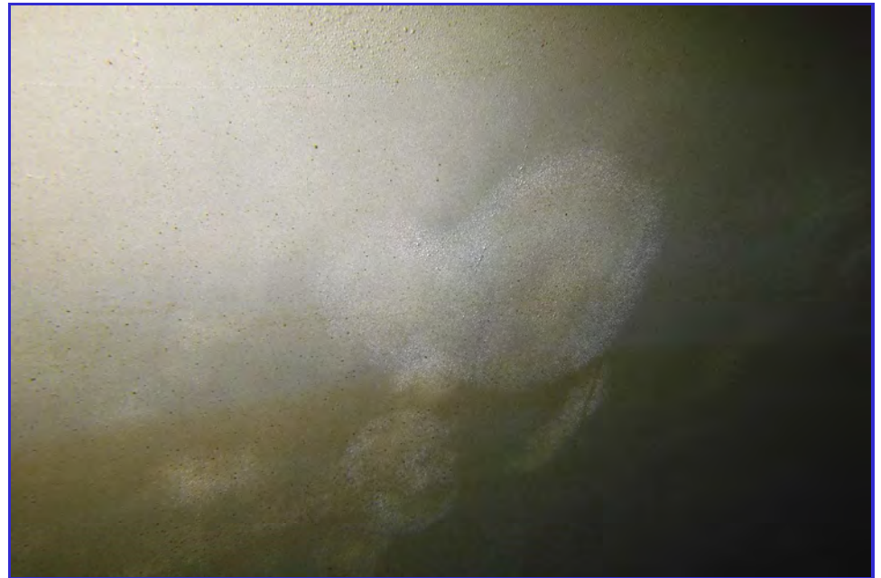
INTERIOR - CPUD - San Andaras Reservoir - Maintenance Inspection -111
