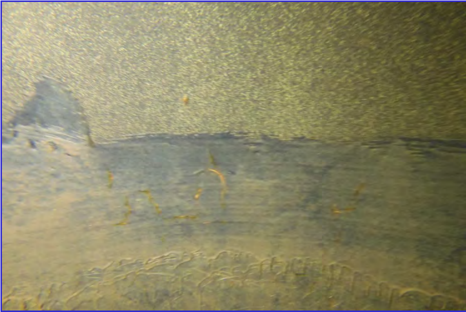
INTERIOR - CPUD - Paloma Reservoir - Maintenance Inspection -068
