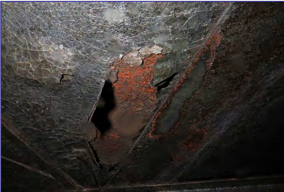
INTERIOR - Calaveras Public Utility District - Clear Well Tank - Maintenance Inspection -030
