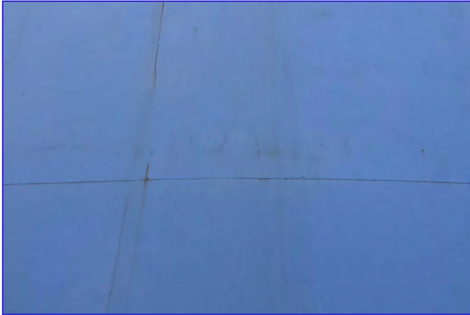
EXTERIOR - CPUD - Mokelumne Reservoir - Maintenance Inspection -124
