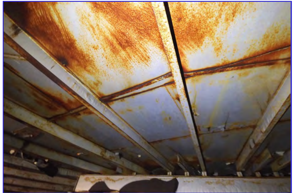
INTERIOR - CPUD - San Andreas Reservoir - Maintenance Inspection -015
