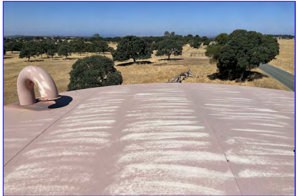
EXTERIOR - CPUD - Paloma Reservoir - Maintenance Inspection -011
