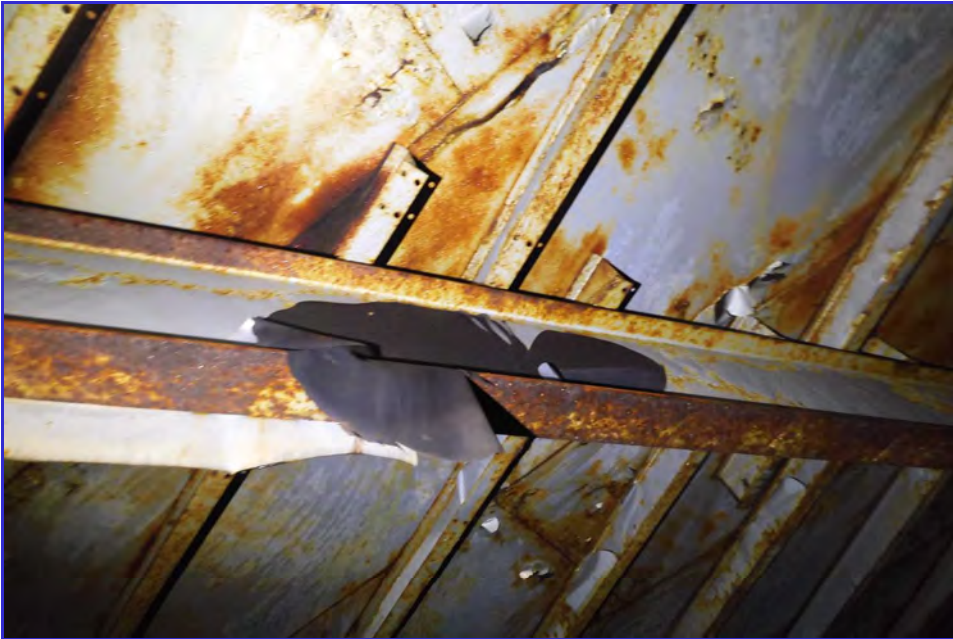
INTERIOR - CPUD - San Andaras Reservoir - Maintenance Inspection -088
