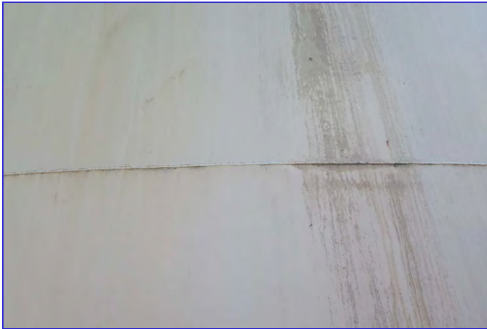
EXTERIOR - Calaveras Public Utility District - Clear Well Tank - Maintenance Inspection -082
