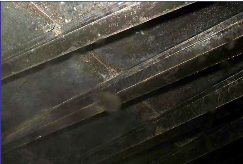
INTERIOR - Calaveras Public Utility District - Clear Well Tank - Maintenance Inspection -014
