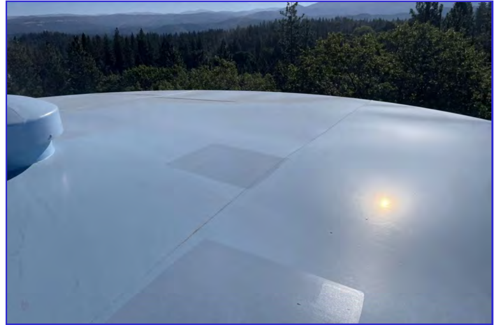
EXTERIOR - CPUD - Railroad Flat Reservoir - Maintenance Inspection -033
