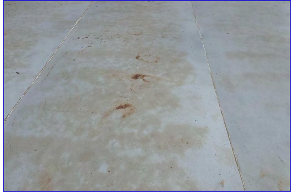
EXTERIOR - CPUD - San Andreas Reservoir - Maintenance Inspection -057
