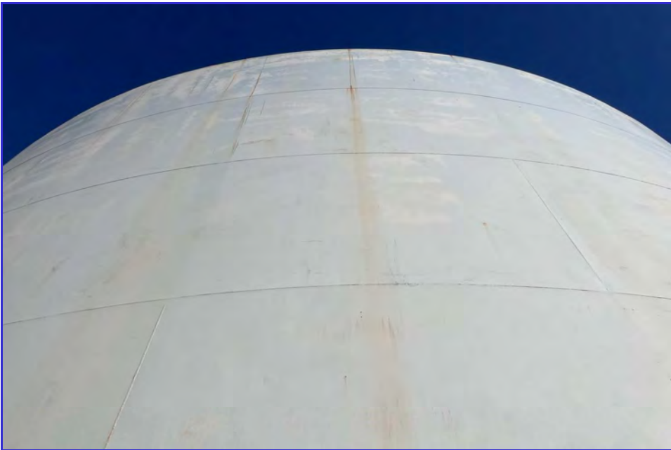
EXTERIOR - CPUD - Mokelumne Reservoir - Maintenance Inspection -102
