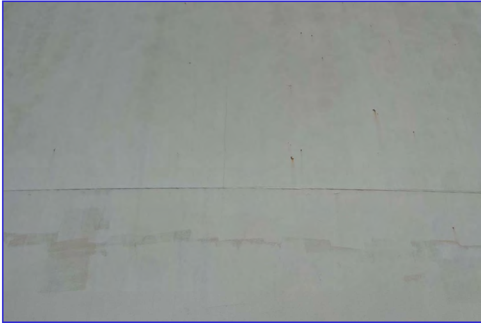
EXTERIOR - CPUD - San Andreas Reservoir - Maintenance Inspection -140
