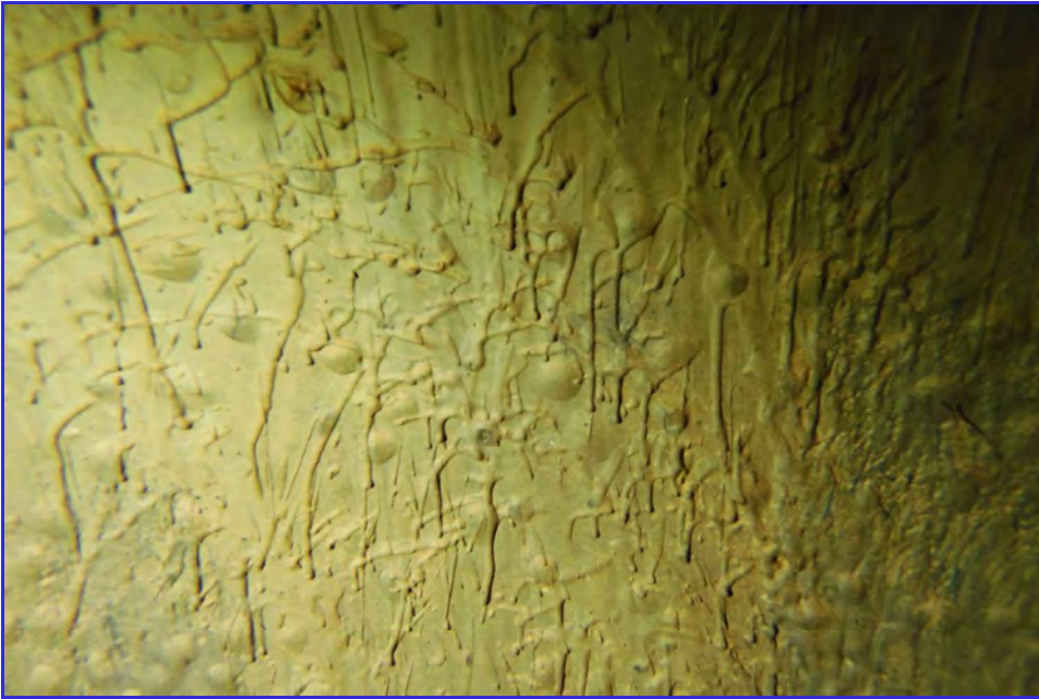
INTERIOR - CPUD - Paloma Reservoir - Maintenance Inspection -096
