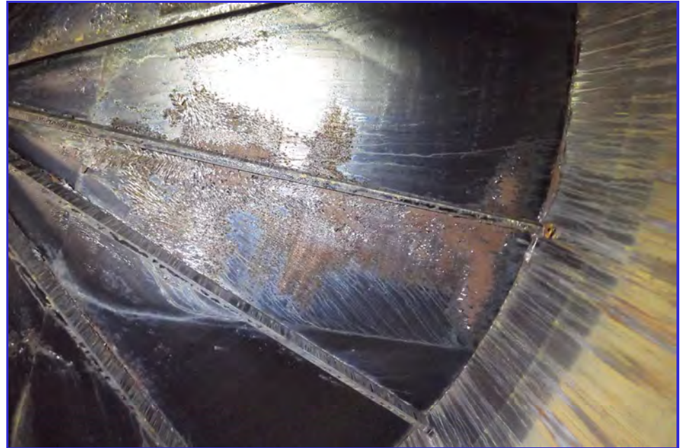
INTERIOR - CPUD - Golden Hills - Maintenance Inspection -025
