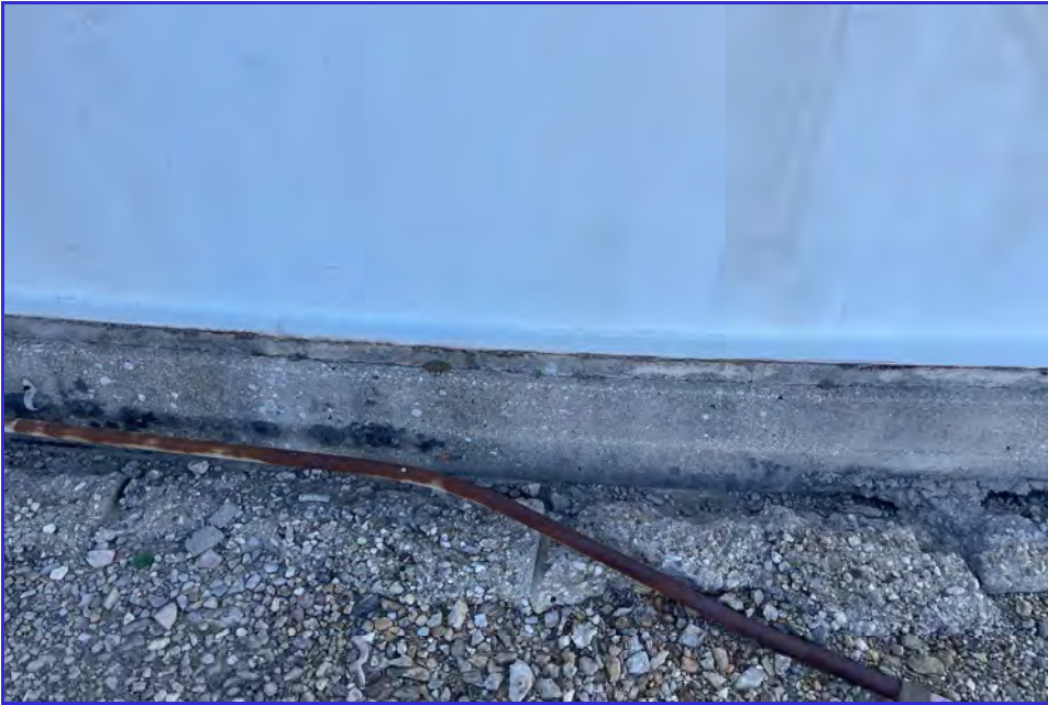
EXTERIOR - CPUD - San Andreas Reservoir - Maintenance Inspection -160
