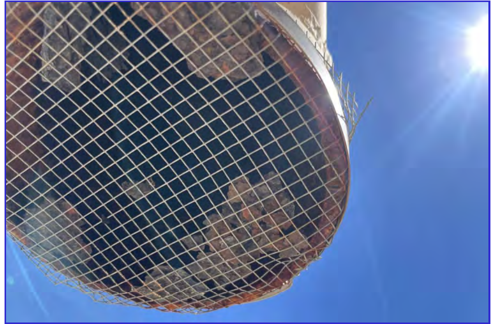
EXTERIOR - CPUD - Golden Hills - Maintenance Inspection -013
