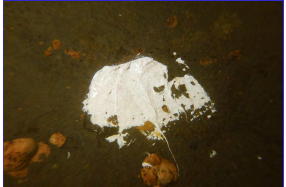
INTERIOR - CPUD - Golden Hills - Maintenance Inspection -125
