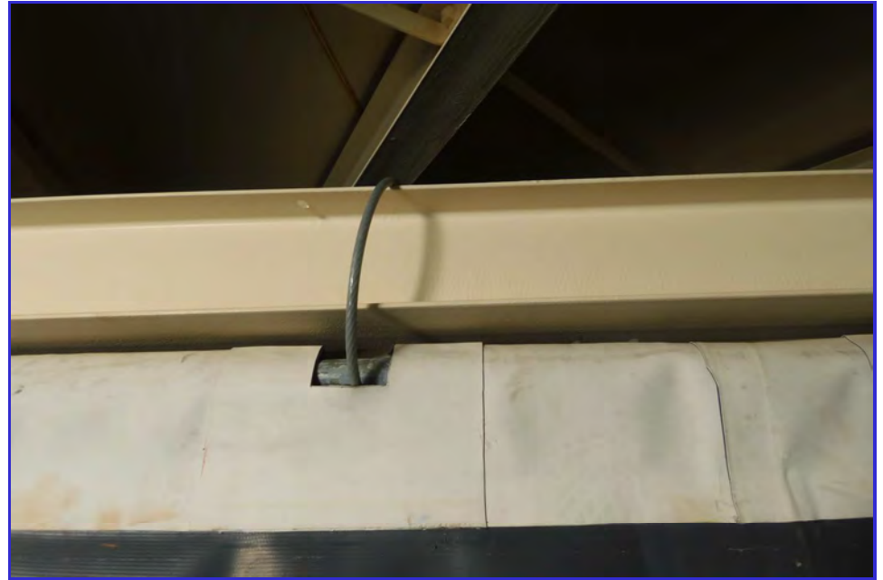
INTERIOR - CPUD - Railroad Flat Reservoir - Maintenance Inspection -021
