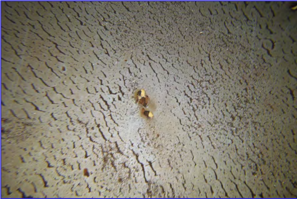
INTERIOR - CPUD - San Andaras Reservoir - Maintenance Inspection -200
