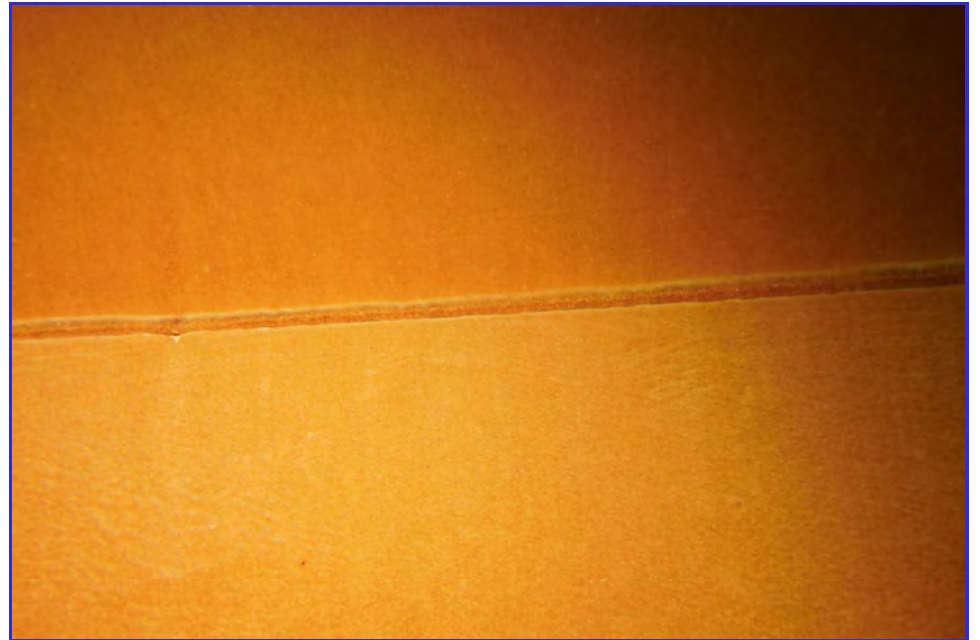
INTERIOR - CPUD - Railroad Flat Reservoir - Maintenance Inspection -097
