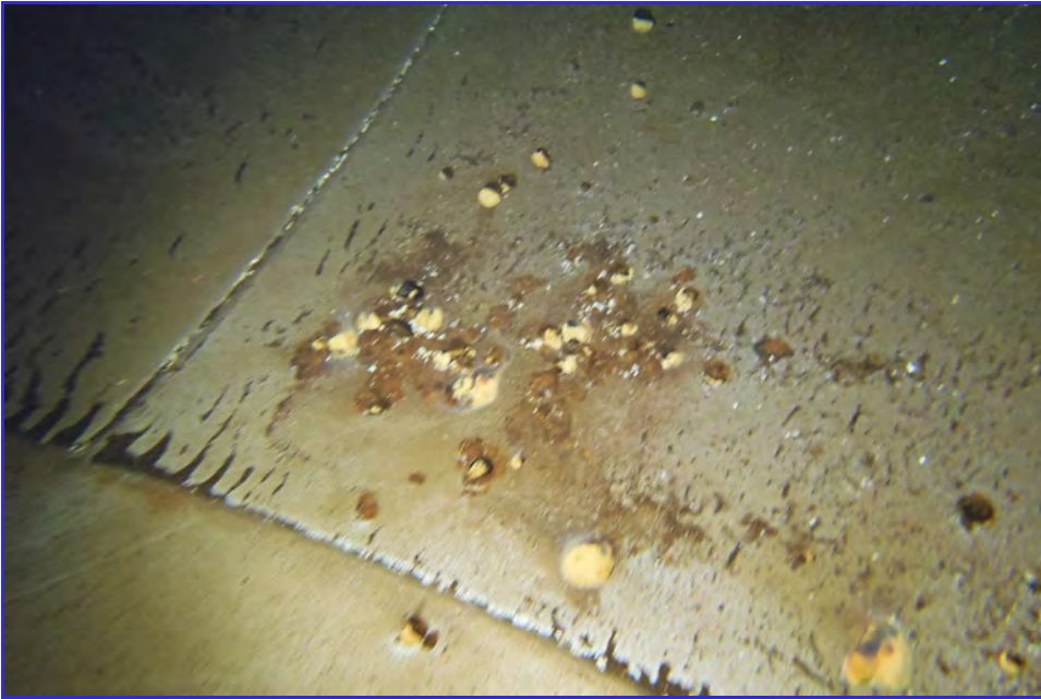
INTERIOR - CPUD - San Andaras Reservoir - Maintenance Inspection -204
