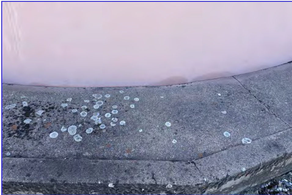
EXTERIOR - CPUD - Paloma Reservoir - Maintenance Inspection -082
