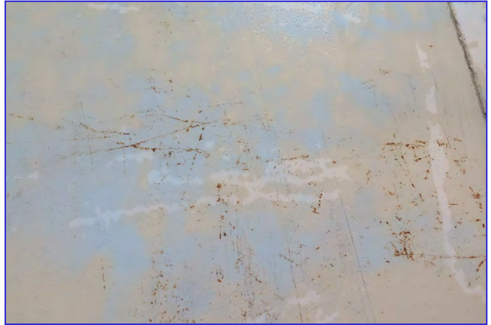
EXTERIOR - Calaveras Public Utility District - Clear Well Tank - Maintenance Inspection -049
