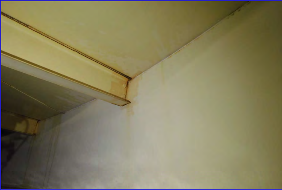
INTERIOR - CPUD - Railroad Flat Reservoir - Maintenance Inspection -056
