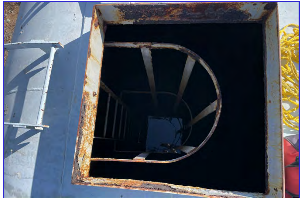
EXTERIOR - CPUD - San Andreas Reservoir - Maintenance Inspection -003
