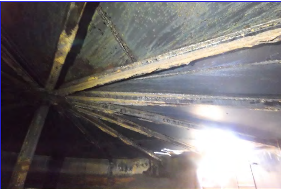
INTERIOR - CPUD - Paloma Reservoir - Maintenance Inspection -014
