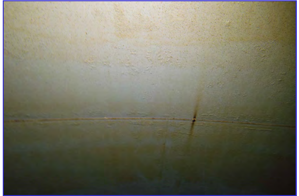
INTERIOR - CPUD - San Andaras Reservoir - Maintenance Inspection -113
