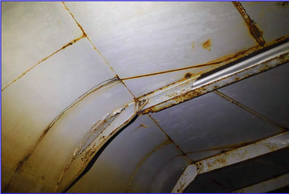
INTERIOR - CPUD - San Anderas Reservoir - Maintenance Inspection -040
