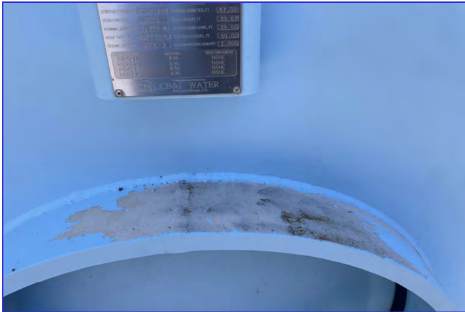
EXTERIOR - CPUD - Railroad Flat Reservoir - Maintenance Inspection -074
