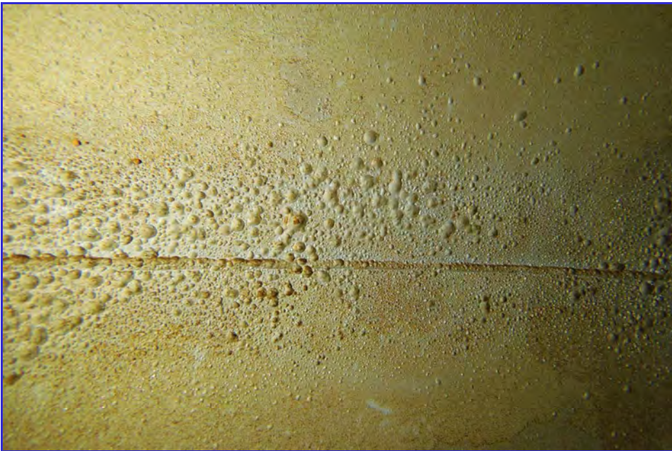
INTERIOR - CPUD - San Andaras Reservoir - Maintenance Inspection -130
