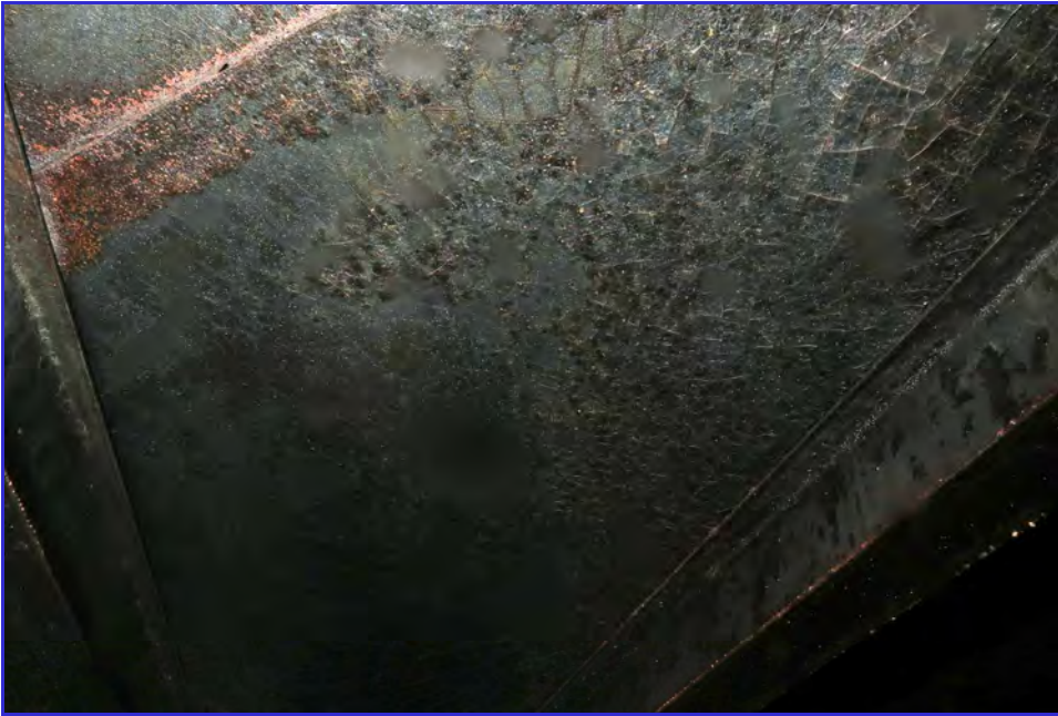
INTERIOR - Calaveras Public Utility District - Clear Well Tank - Maintenance Inspection -028
