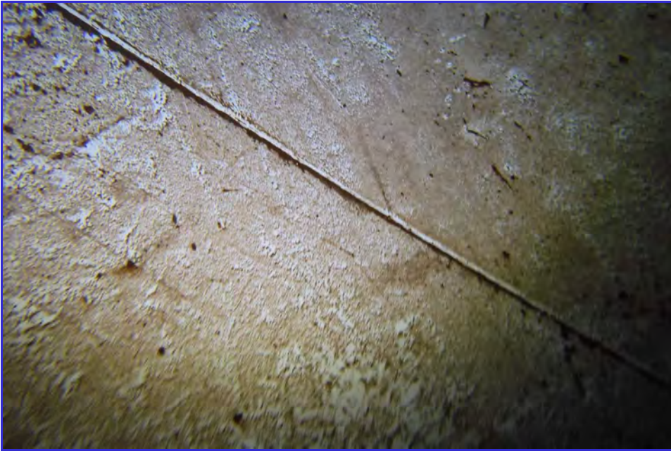
INTERIOR - CPUD - Mokelumne Hill Reservoir - Maintenance Inspection -128
