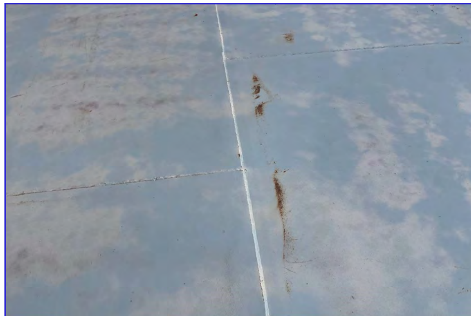
EXTERIOR - CPUD - Mokelumne Reservoir - Maintenance Inspection -011
