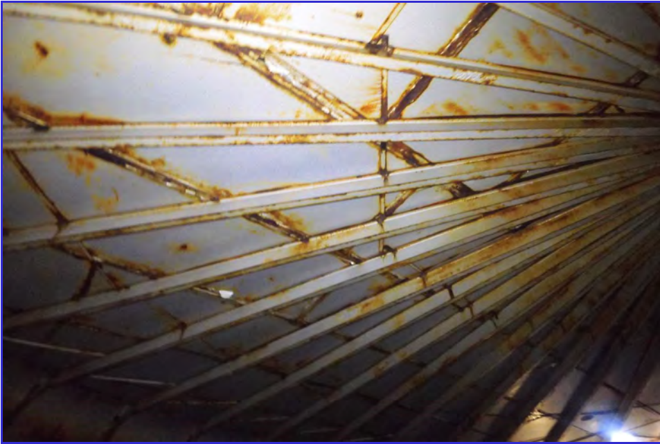
INTERIOR - CPUD - Mokelumne Hill Reservoir - Maintenance Inspection -028
