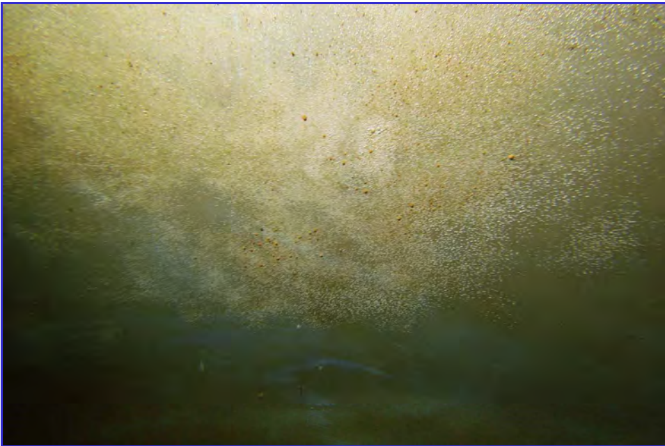
INTERIOR - CPUD - Mokelumne Hill Reservoir - Maintenance Inspection -102
