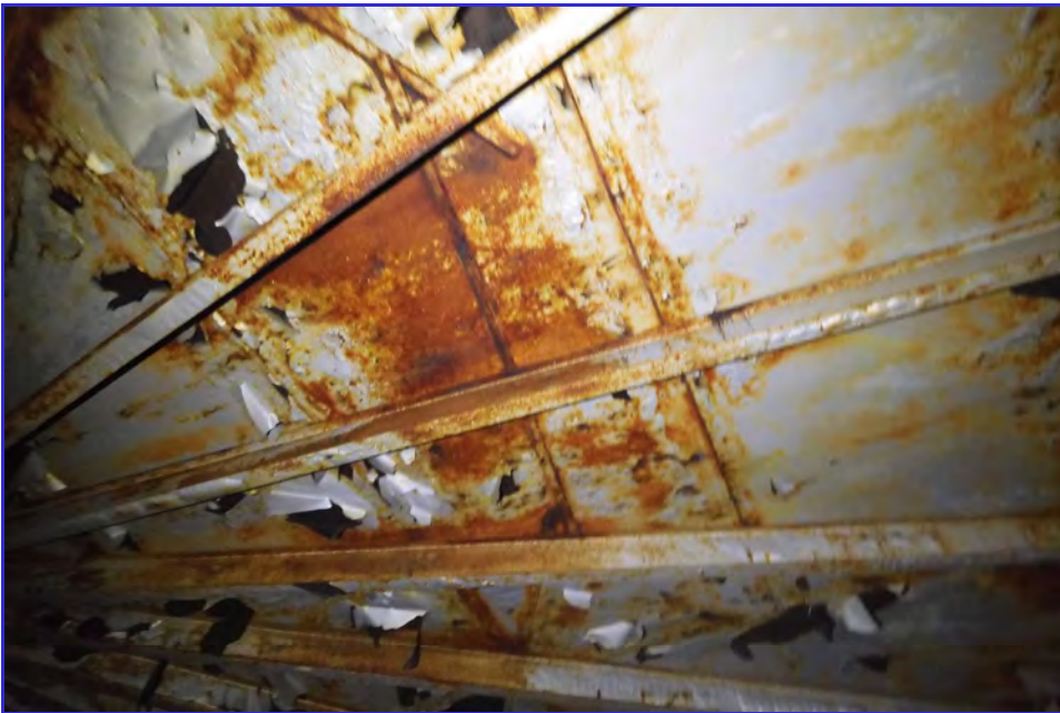
INTERIOR - CPUD - San Andaras Reservoir - Maintenance Inspection -086
