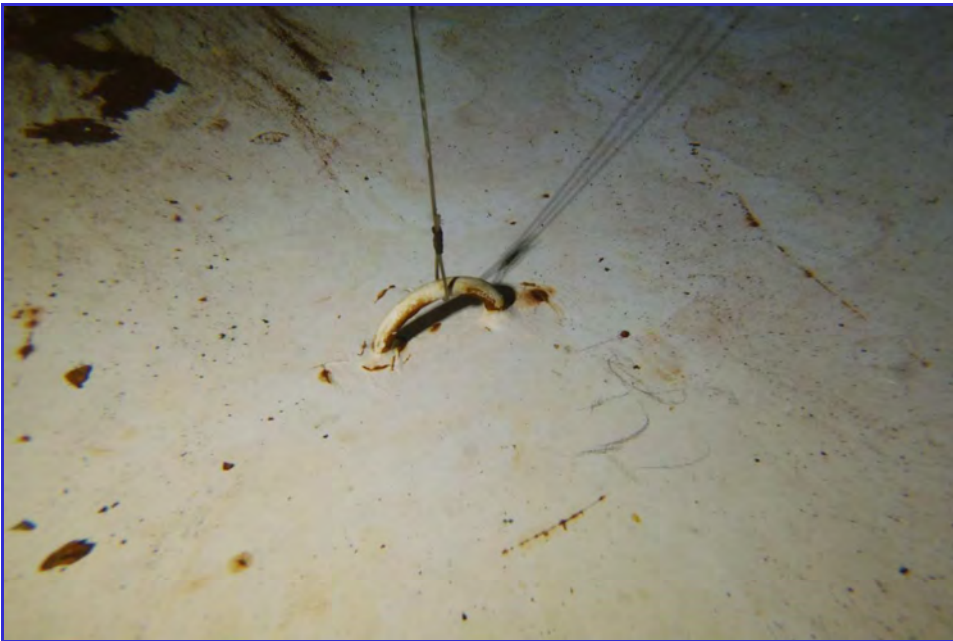
INTERIOR - CPUD - Railroad Flat Reservoir - Maintenance Inspection -162
