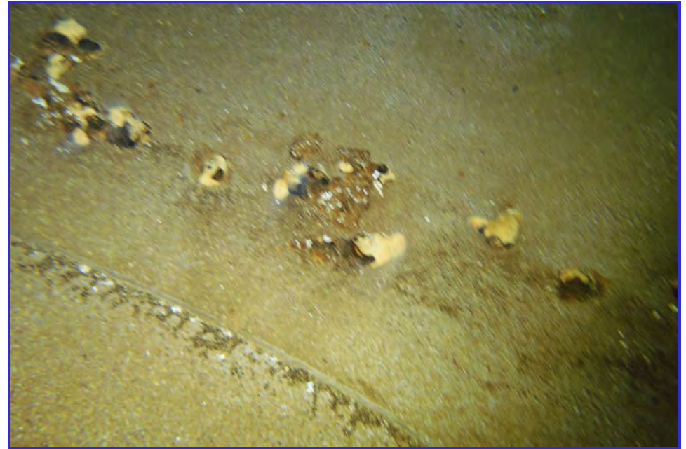
INTERIOR - CPUD - San Andaras Reservoir - Maintenance Inspection -173
