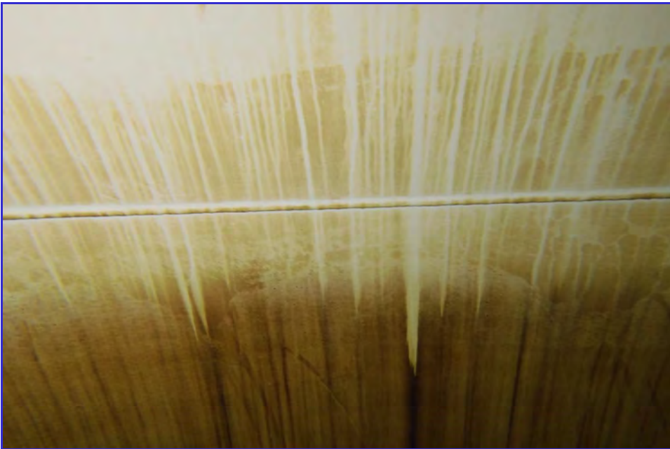
INTERIOR - CPUD - Railroad Flat Reservoir - Maintenance Inspection -078
