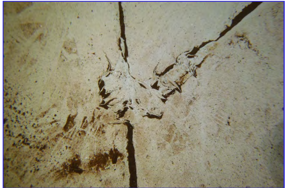
INTERIOR - CPUD - Railroad Flat Reservoir - Maintenance Inspection -159
