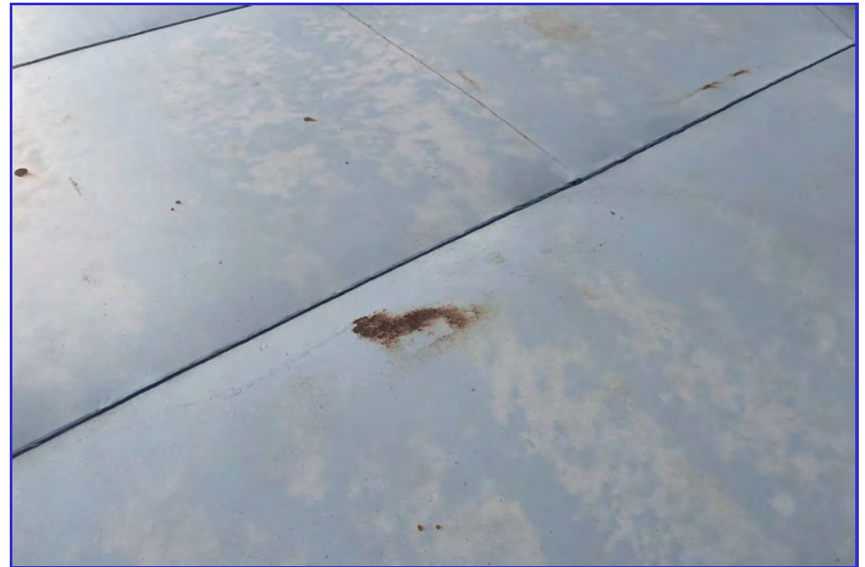
EXTERIOR - CPUD - Mokelumne Reservoir - Maintenance Inspection -039
