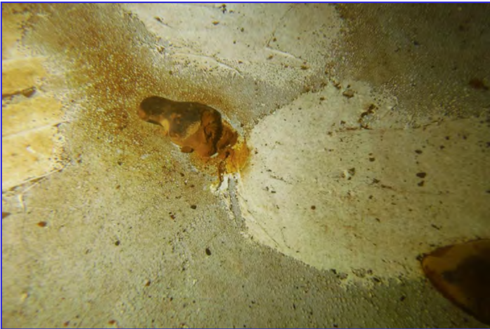
INTERIOR - CPUD - Mokelumne Hill Reservoir - Maintenance Inspection -154
