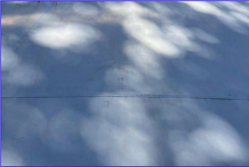
EXTERIOR - CPUD - Mokelumne Reservoir - Maintenance Inspection -172
