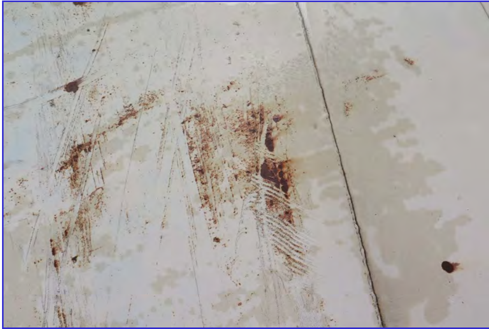
EXTERIOR - Calaveras Public Utility District - Clear Well Tank - Maintenance Inspection -028
