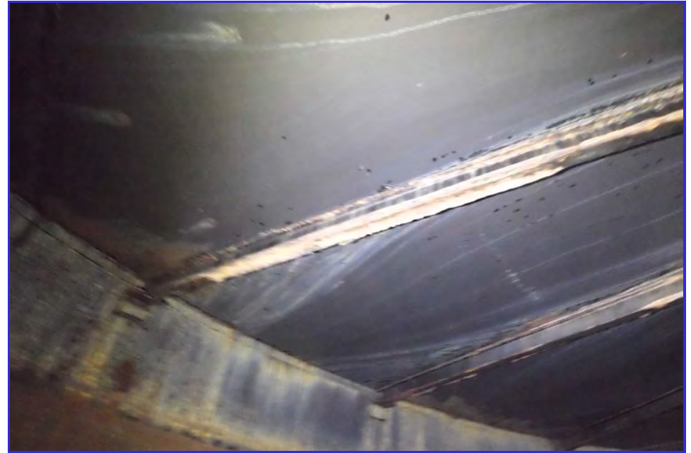
INTERIOR - CPUD - Paloma Reservoir - Maintenance Inspection -025
