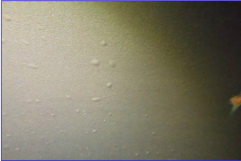
INTERIOR - CPUD - Paloma Reservoir - Maintenance Inspection -056
