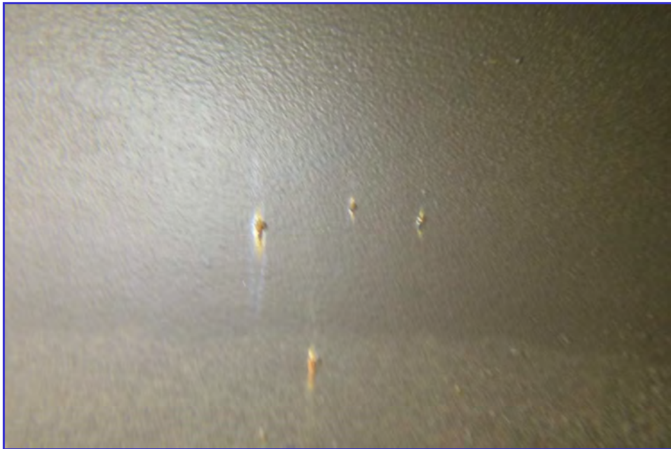
INTERIOR - CPUD - Paloma Reservoir - Maintenance Inspection -062
