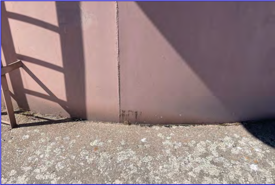
EXTERIOR - CPUD - Paloma Reservoir - Maintenance Inspection -064
