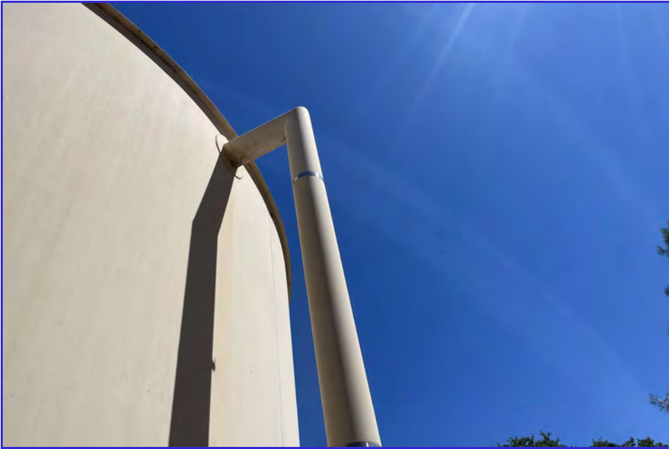
EXTERIOR - CPUD - Golden Hills - Maintenance Inspection -036
