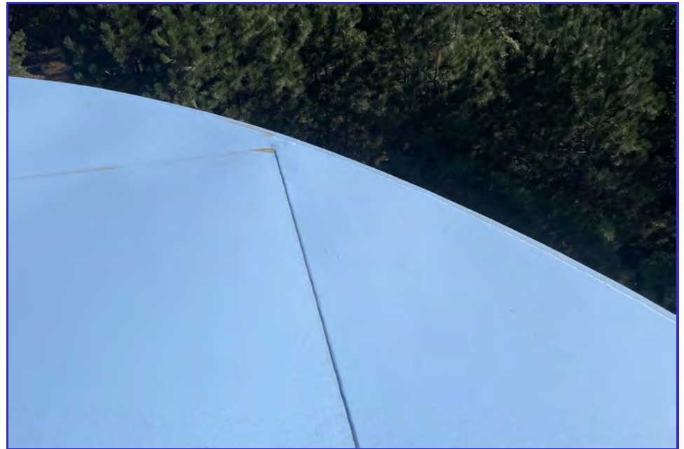
EXTERIOR - CPUD - Railroad Flat Reservoir - Maintenance Inspection -015
