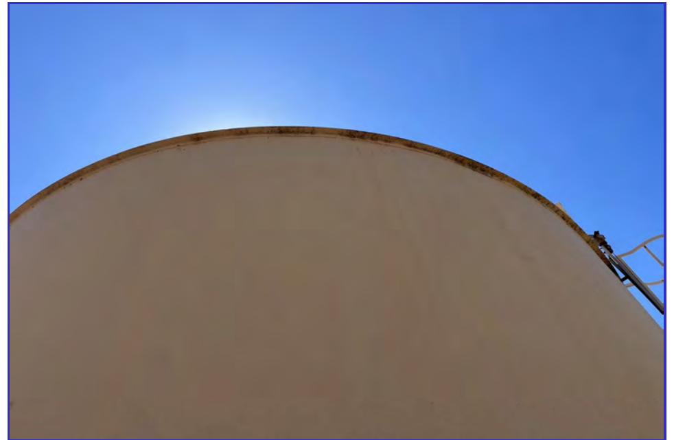
EXTERIOR - CPUD - Golden Hills - Maintenance Inspection -055
