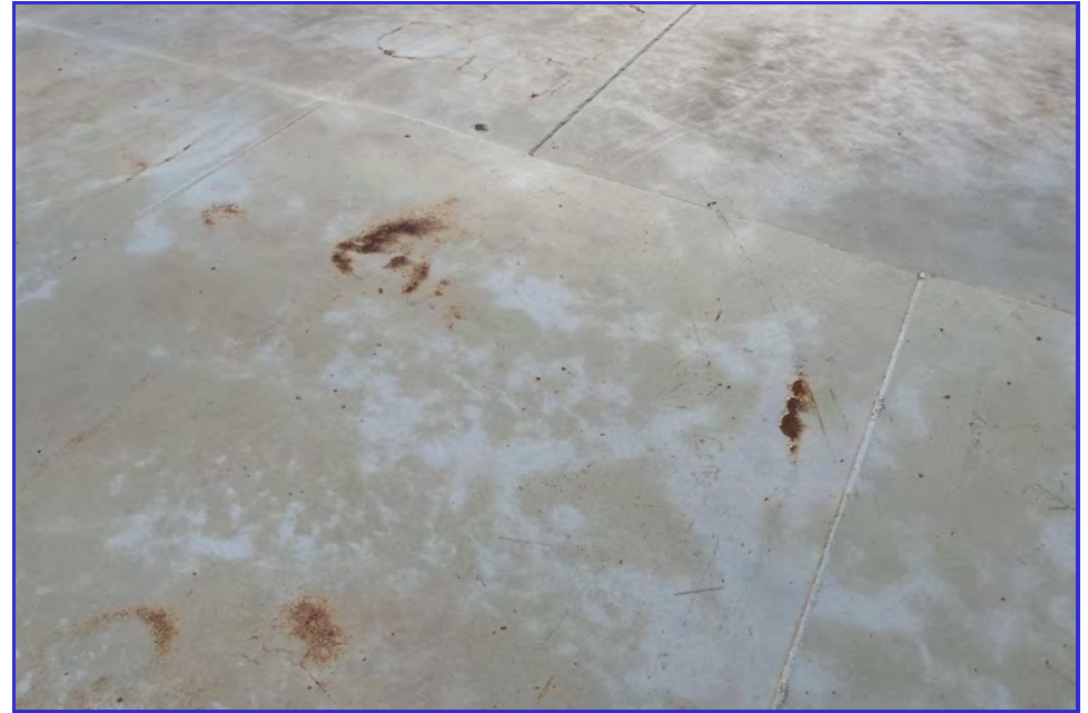
EXTERIOR - CPUD - San Andreas Reservoir - Maintenance Inspection -085
