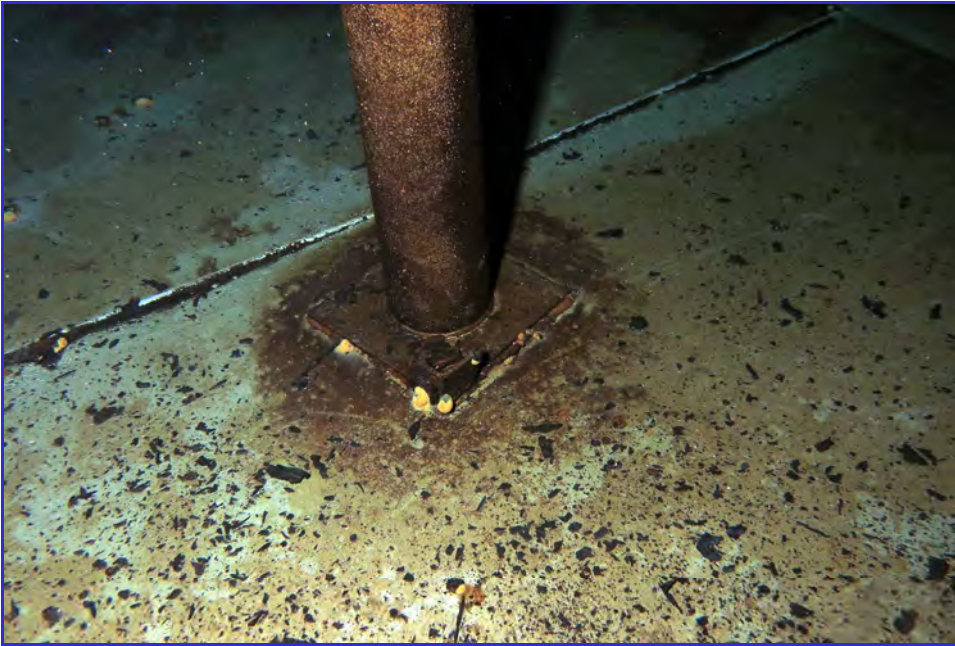
INTERIOR - Calaveras Public Utility District - Clear Well Tank - Maintenance Inspection -108
