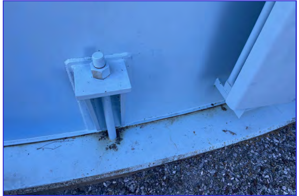
EXTERIOR - CPUD - Railroad Flat Reservoir - Maintenance Inspection -065
