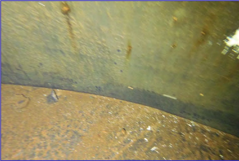
INTERIOR - CPUD - Paloma Reservoir - Maintenance Inspection -104
