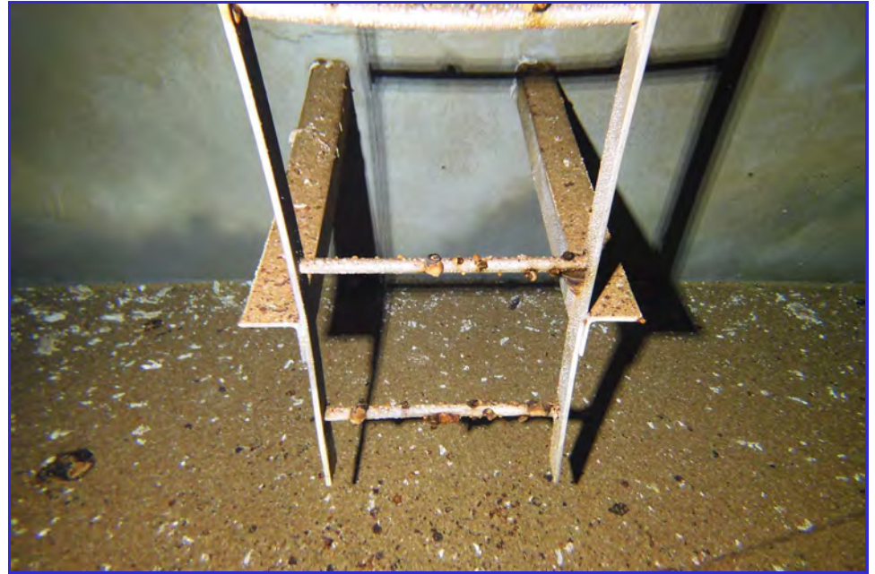
INTERIOR - CPUD - San Anderas Reservoir - Maintenance Inspection -165
