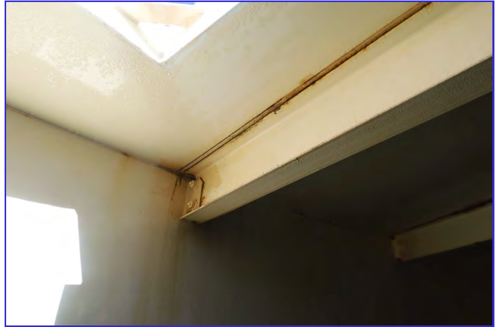
INTERIOR - CPUD - Railroad Flat Reservoir - Maintenance Inspection -001
