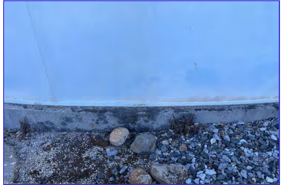
EXTERIOR - CPUD - Mokelumne Reservoir - Maintenance Inspection -145
