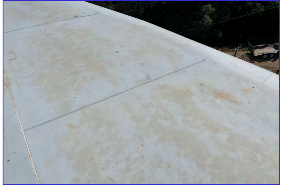
EXTERIOR - CPUD - San Andreas Reservoir - Maintenance Inspection -093
