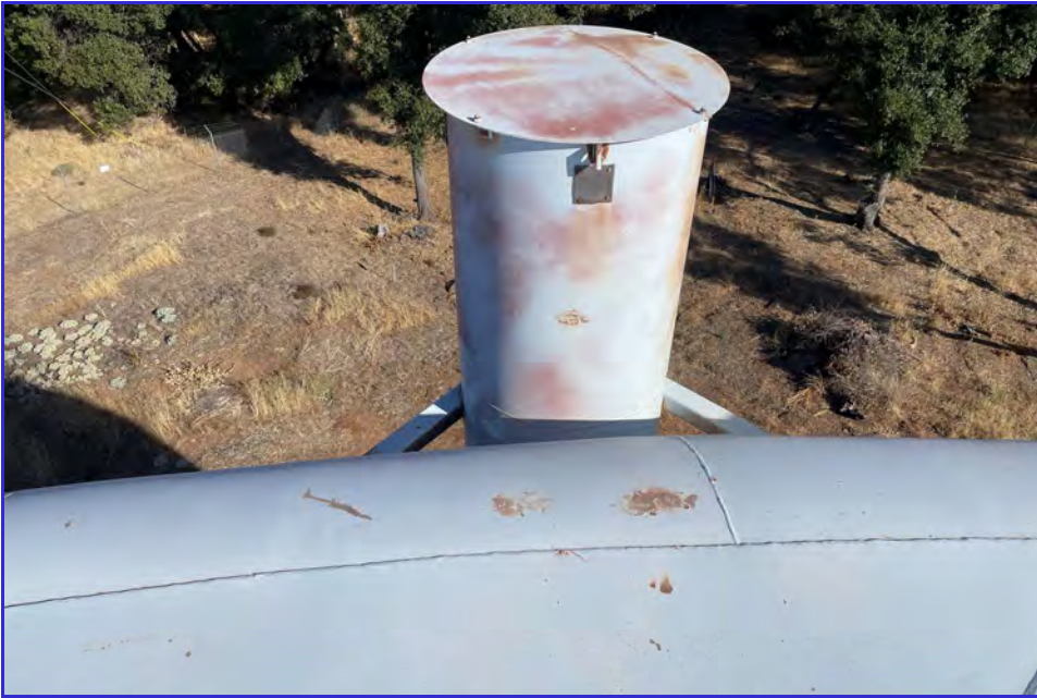
EXTERIOR - CPUD - Mokelumne Reservoir - Maintenance Inspection -076
