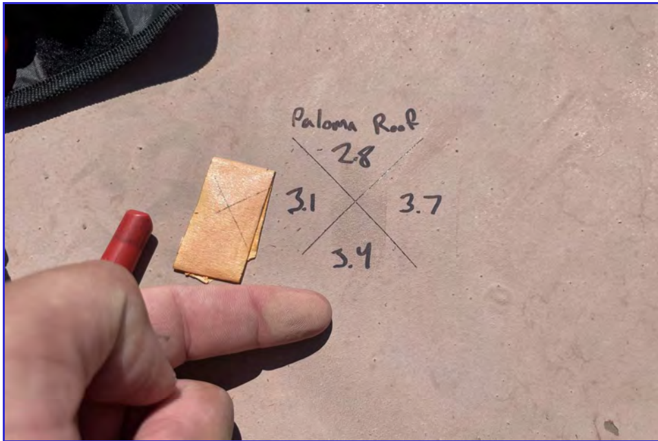
EXTERIOR - CPUD - Paloma Reservoir - Maintenance Inspection -034
