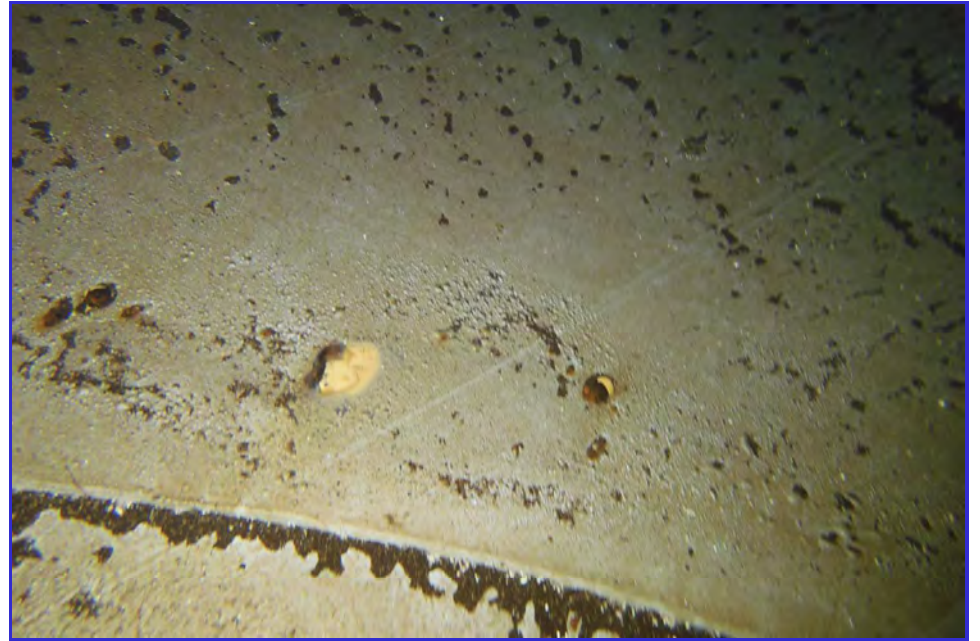
INTERIOR - CPUD - San Andaras Reservoir - Maintenance Inspection -181
