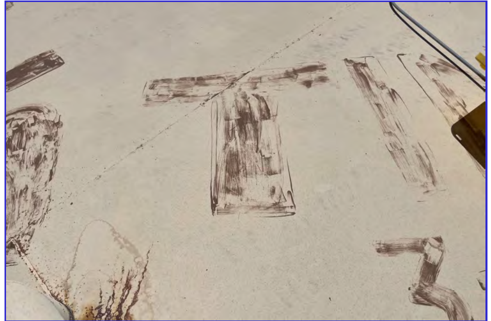
EXTERIOR - CPUD - Golden Hills - Maintenance Inspection -001
