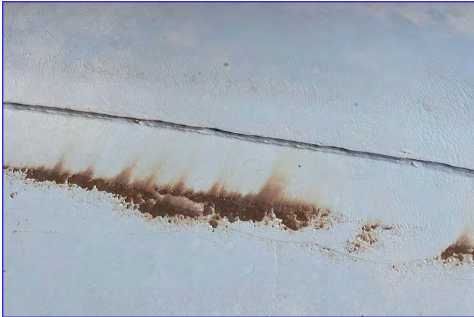
EXTERIOR - CPUD - Mokelumne Reservoir - Maintenance Inspection -040
