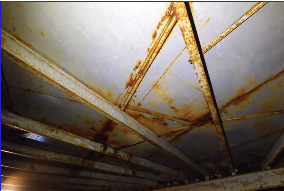
INTERIOR - CPUD - San Andaras Reservoir - Maintenance Inspection -026
