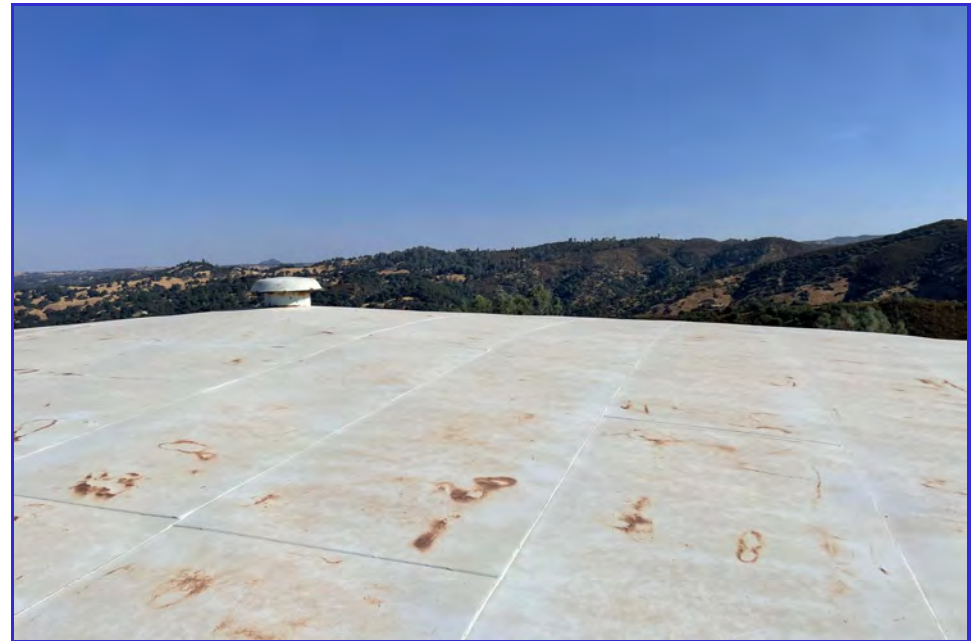
EXTERIOR - CPUD - San Andreas Reservoir - Maintenance Inspection -031
