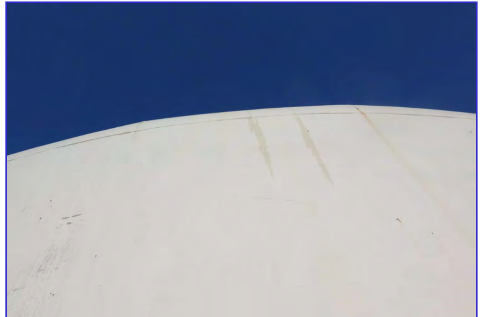
EXTERIOR - Calaveras Public Utility District - Clear Well Tank - Maintenance Inspection -063
