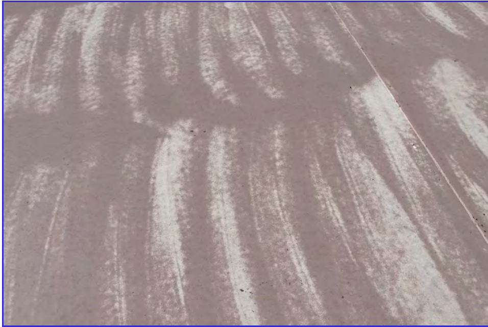
EXTERIOR - CPUD - Paloma Reservoir - Maintenance Inspection -012
