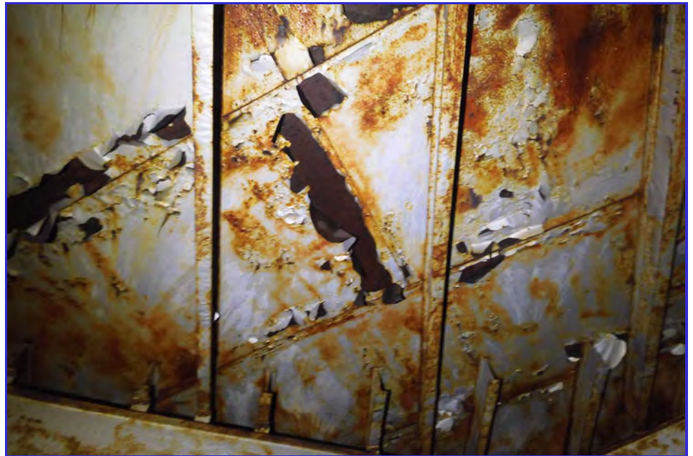
INTERIOR - CPUD - San Andaras Reservoir - Maintenance Inspection -079
