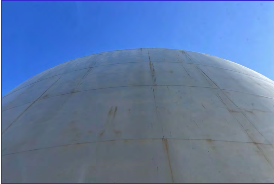
EXTERIOR - CPUD - Mokelumne Reservoir - Maintenance Inspection -156
