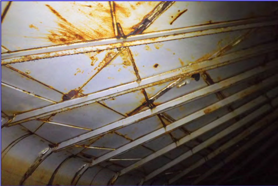
INTERIOR - CPUD - Mokelumne Hill Reservoir - Maintenance Inspection -036
