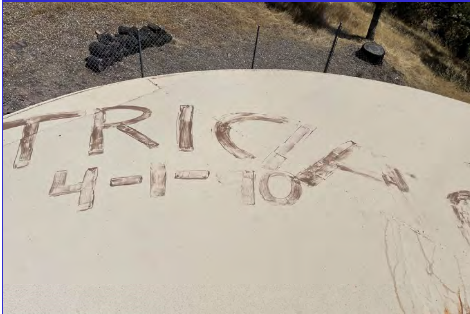
EXTERIOR - CPUD - Golden Hills - Maintenance Inspection -016
