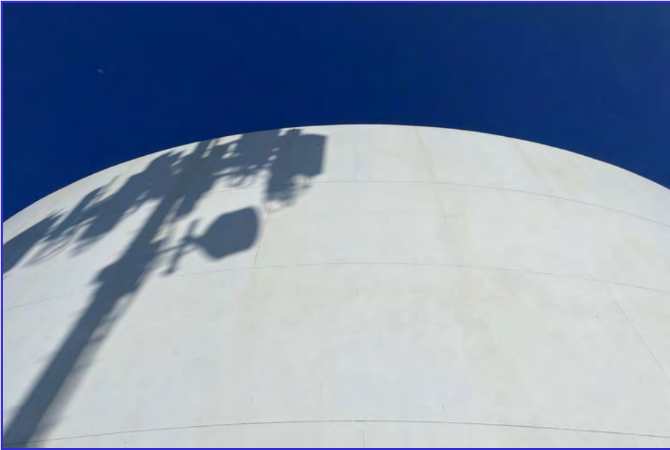
EXTERIOR - CPUD - San Andreas Reservoir - Maintenance Inspection -144
