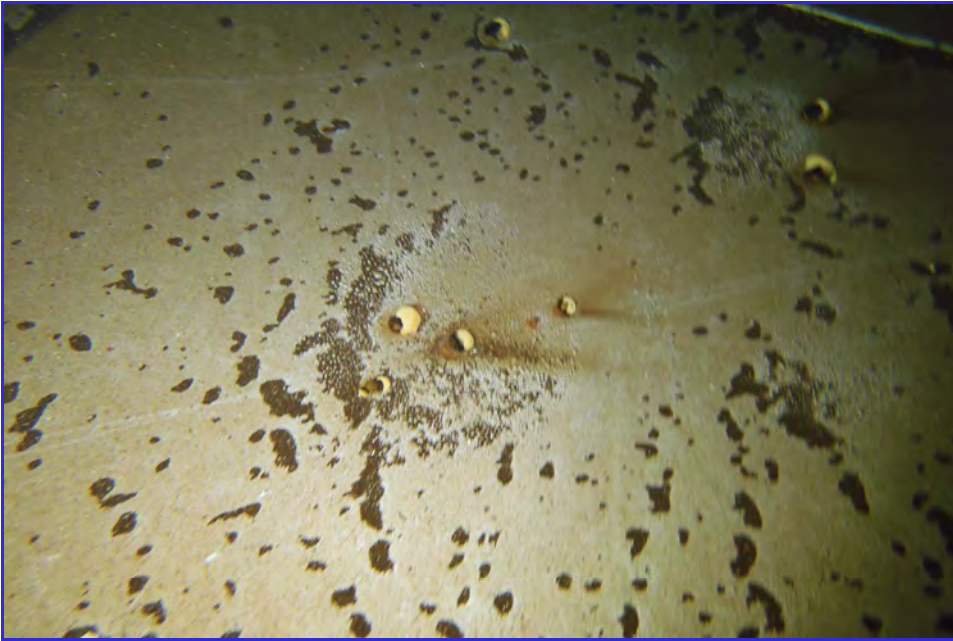
INTERIOR - CPUD - San Andaras Reservoir - Maintenance Inspection -208
