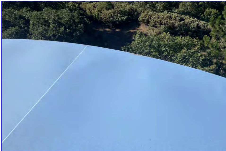
EXTERIOR - CPUD - Railroad Flat Reservoir - Maintenance Inspection -030
