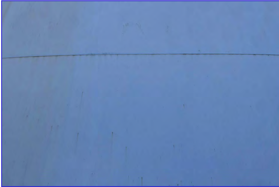
EXTERIOR - CPUD - Mokelumne Reservoir - Maintenance Inspection -128
