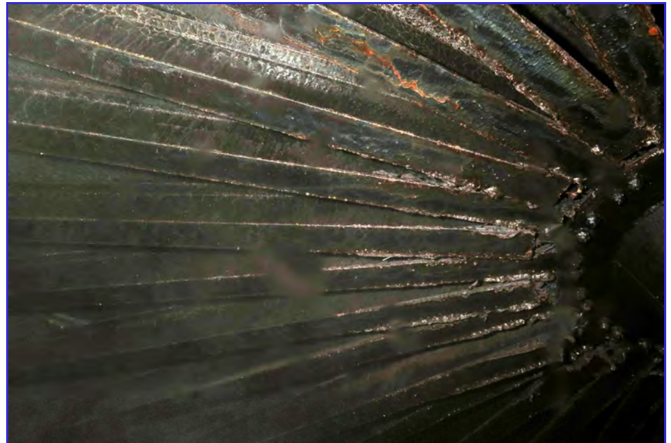
INTERIOR - Calaveras Public Utility District - Clear Well Tank - Maintenance Inspection -015
