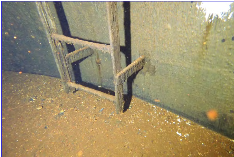
INTERIOR - CPUD - Paloma Reservoir - Maintenance Inspection -110
