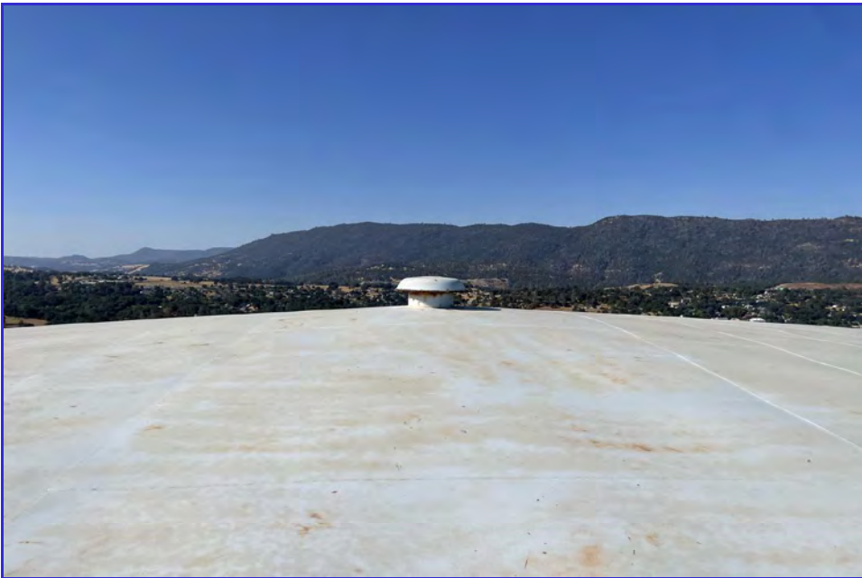
EXTERIOR - CPUD - San Andreas Reservoir - Maintenance Inspection -066
