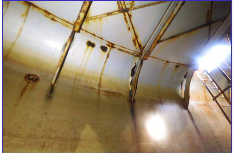
INTERIOR - CPUD - Mokelumne Hill Reservoir - Maintenance Inspection -009
