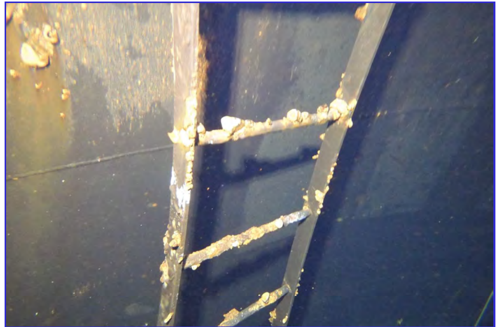
INTERIOR - CPUD - Paloma Reservoir - Maintenance Inspection -119
