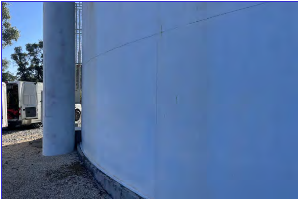
EXTERIOR - CPUD - Mokelumne Reservoir - Maintenance Inspection -146
