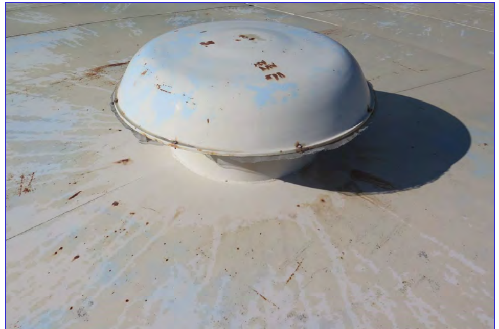
EXTERIOR - Calaveras Public Utility District - Clear Well Tank - Maintenance Inspection -051
