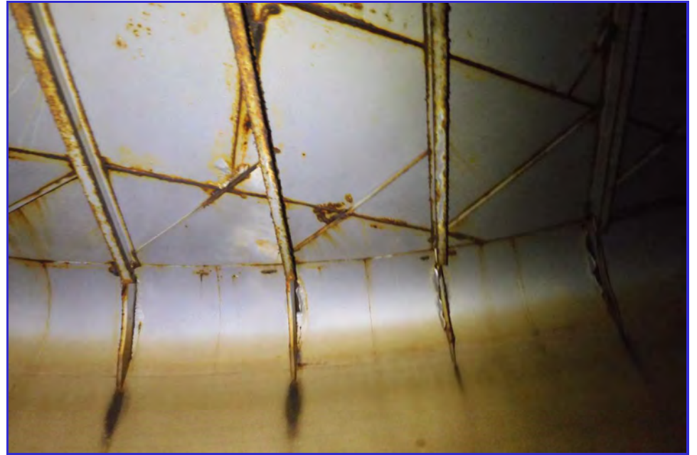
INTERIOR - CPUD - Mokelumne Hill Reservoir - Maintenance Inspection -041
