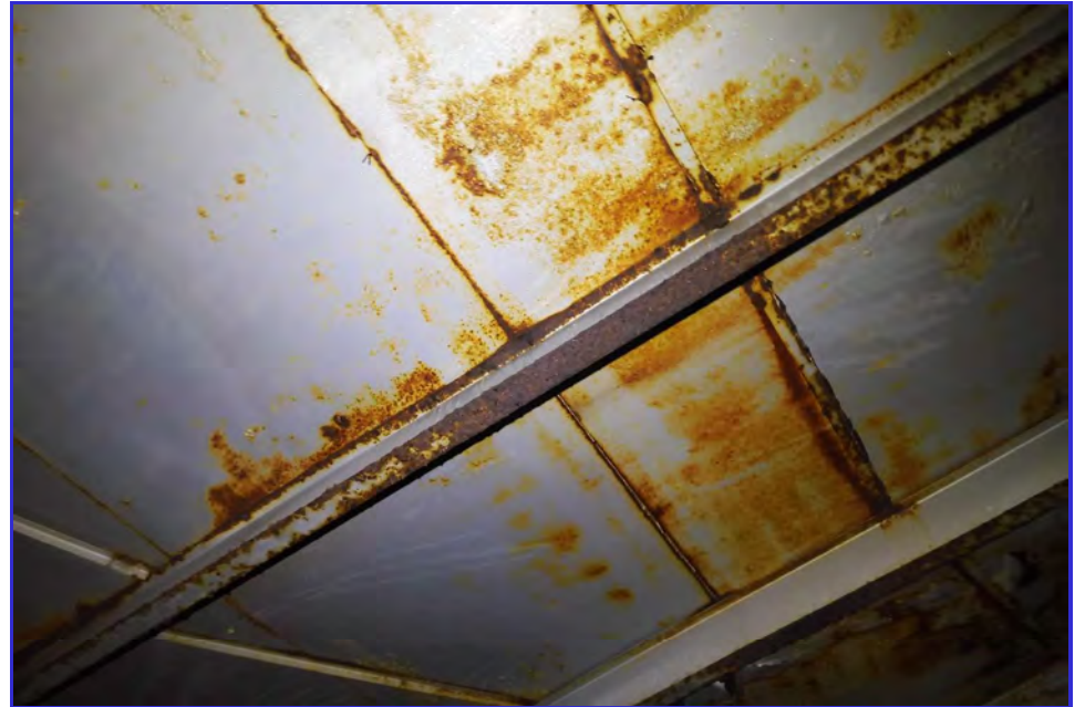
INTERIOR - CPUD - San Andaras Reservoir - Maintenance Inspection -049
