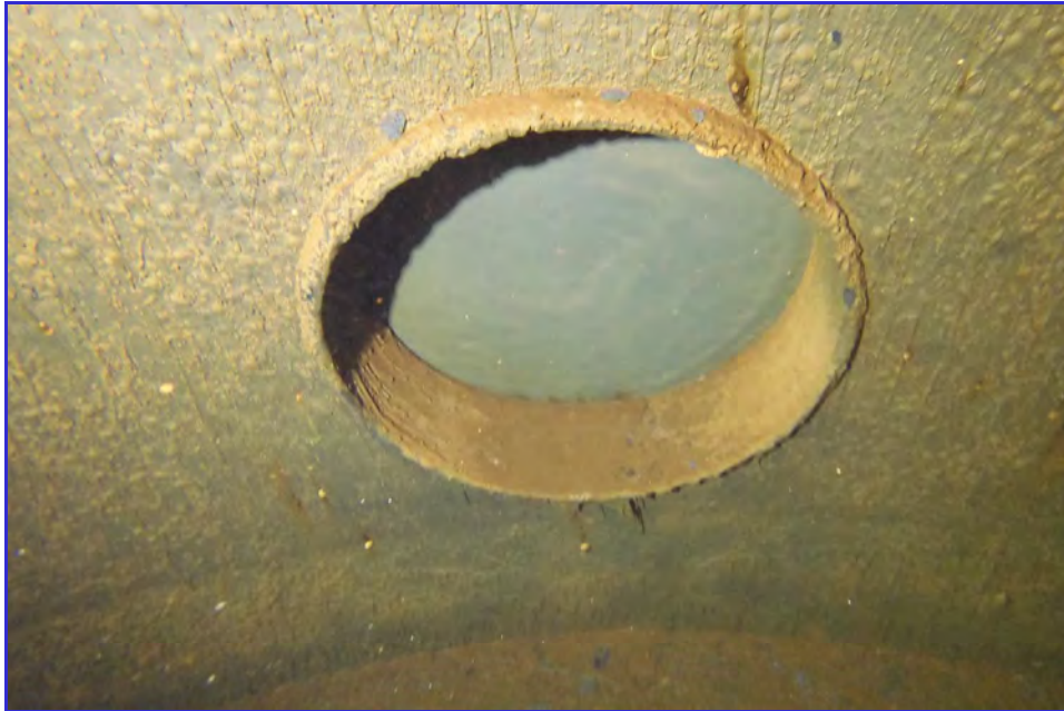
INTERIOR - CPUD - Paloma Reservoir - Maintenance Inspection -084
