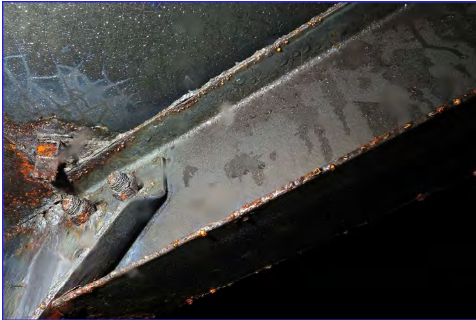
INTERIOR - Calaveras Public Utility District - Clear Well Tank - Maintenance Inspection -036
