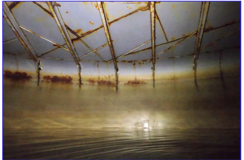
INTERIOR - CPUD - Mokelumne Hill Reservoir - Maintenance Inspection -019
