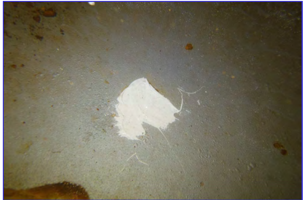
INTERIOR - CPUD - San Andaras Reservoir - Maintenance Inspection -243
