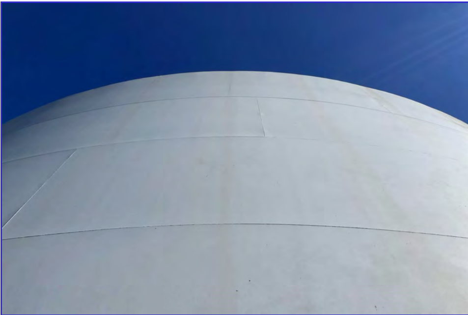
EXTERIOR - CPUD - San Andreas Reservoir - Maintenance Inspection -154
