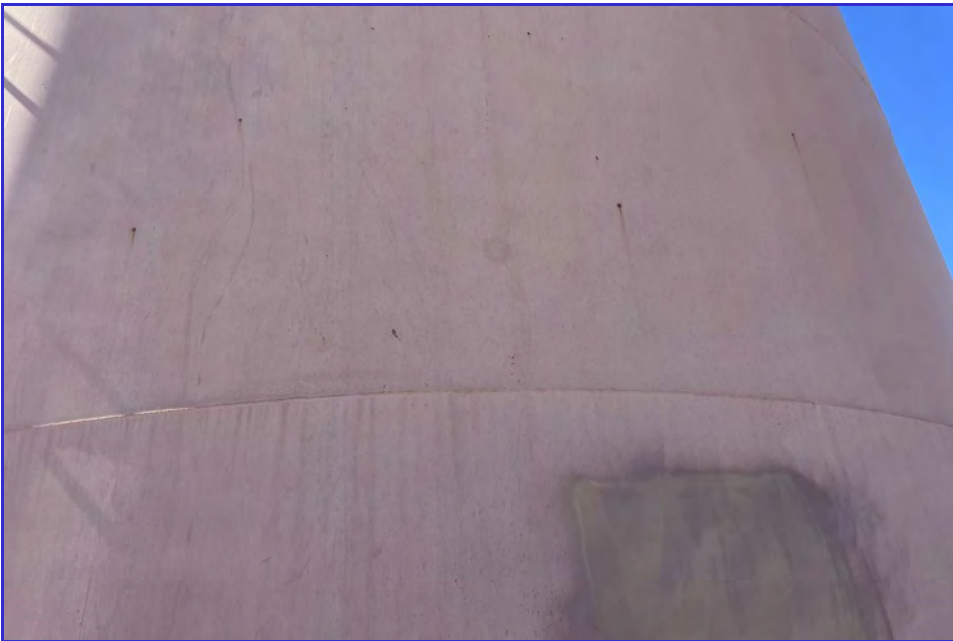
EXTERIOR - CPUD - Paloma Reservoir - Maintenance Inspection -066
