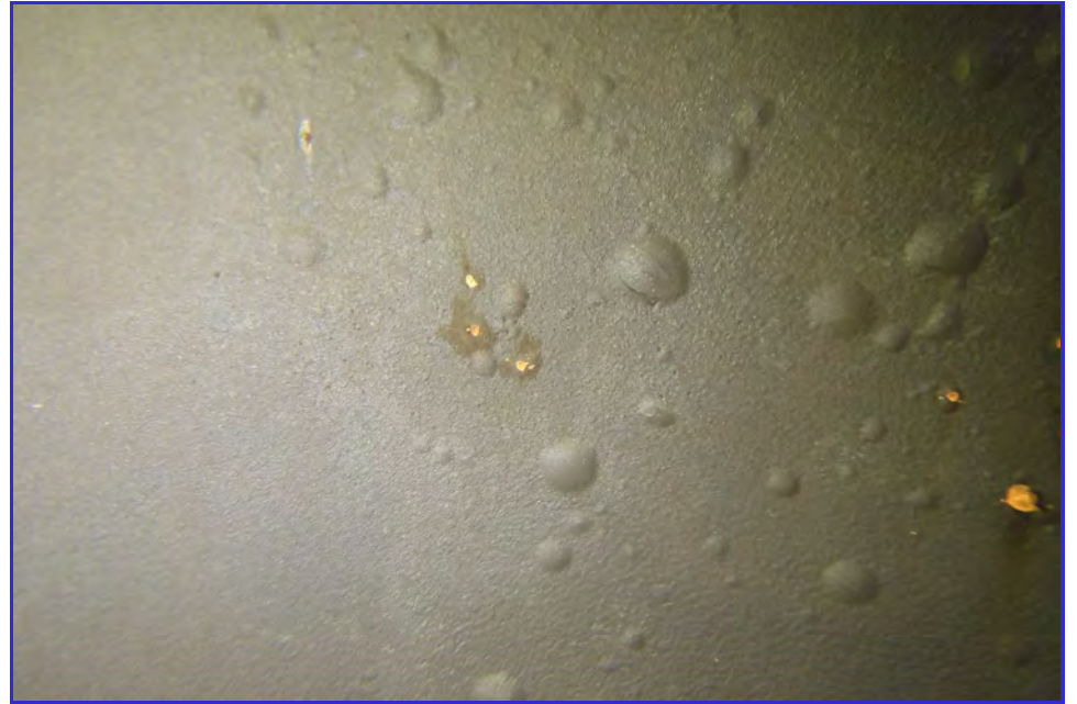
INTERIOR - CPUD - Paloma Reservoir - Maintenance Inspection -049
