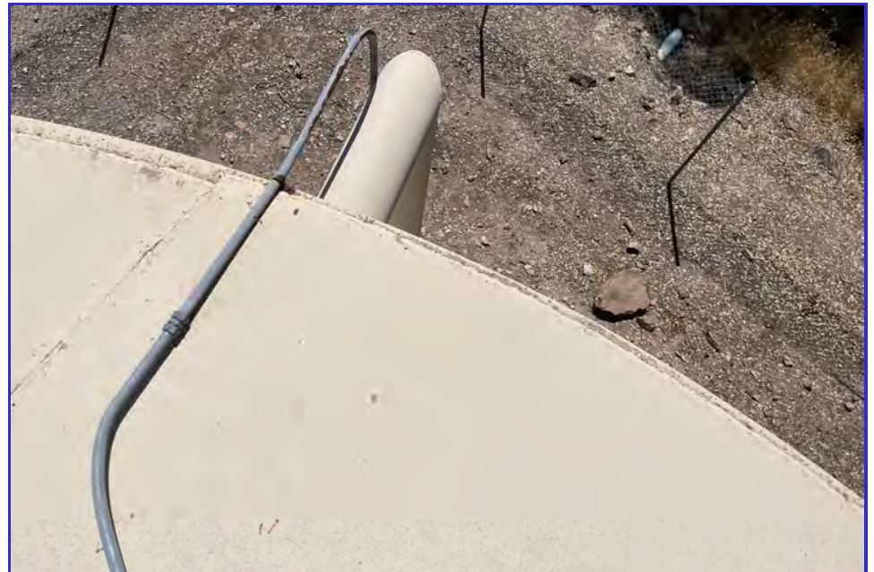
EXTERIOR - CPUD - Golden Hills - Maintenance Inspection -003
