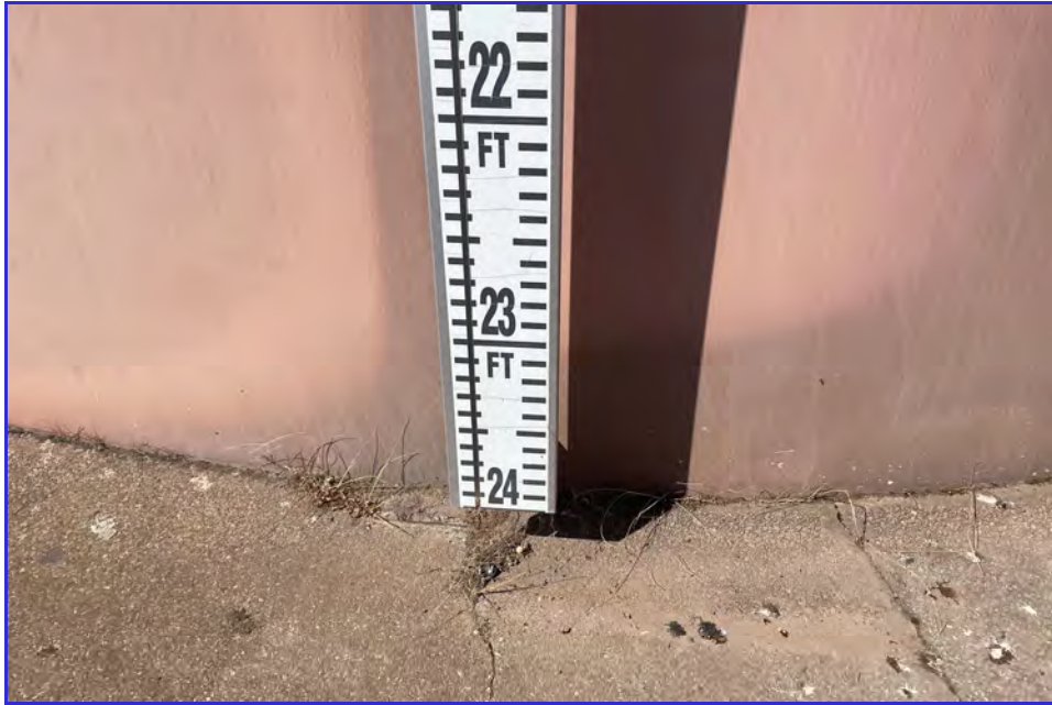
EXTERIOR - CPUD - Paloma Reservoir - Maintenance Inspection -056
