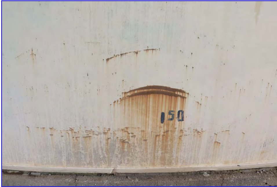
EXTERIOR - Calaveras Public Utility District - Clear Well Tank - Maintenance Inspection -068
