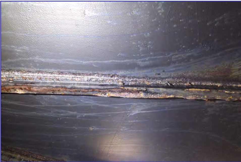
INTERIOR - CPUD - Paloma Reservoir - Maintenance Inspection -006
