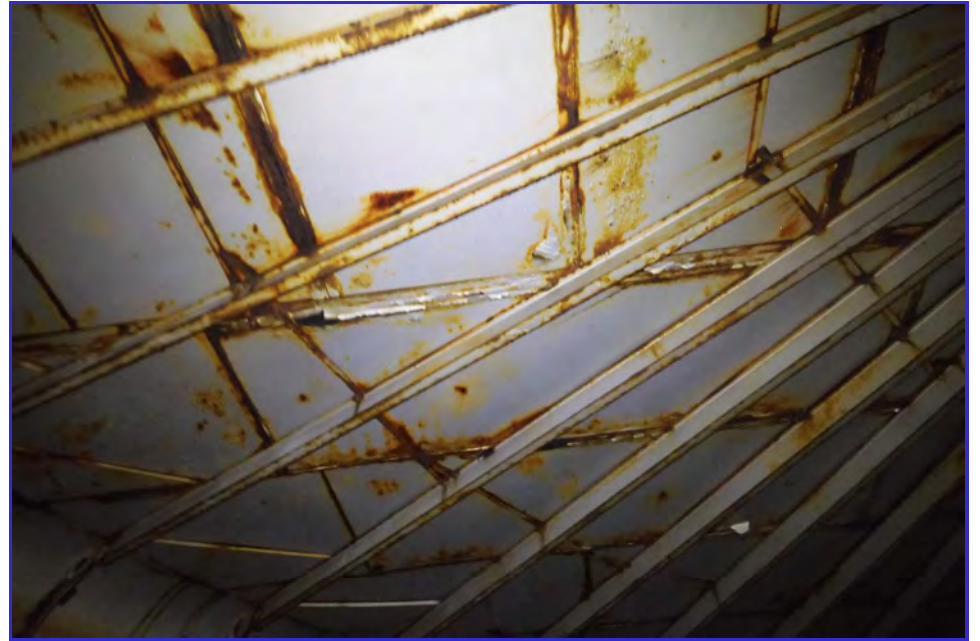
INTERIOR - CPUD - Mokelumne Hill Reservoir - Maintenance Inspection -029
