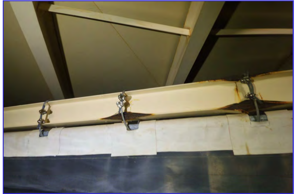
INTERIOR - CPUD - Railroad Flat Reservoir - Maintenance Inspection -045
