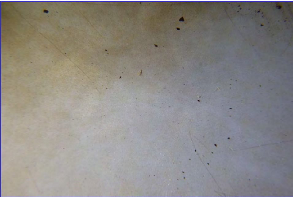
INTERIOR - CPUD - Mokelumne Hill Reservoir - Maintenance Inspection -134
