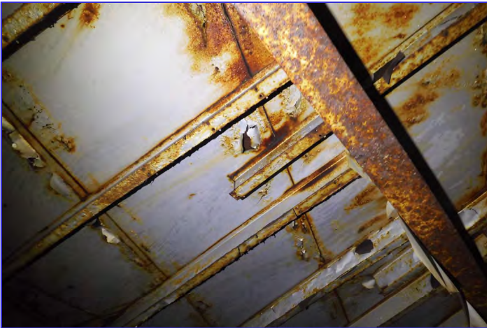
INTERIOR - CPUD - San Andaras Reservoir - Maintenance Inspection -070
