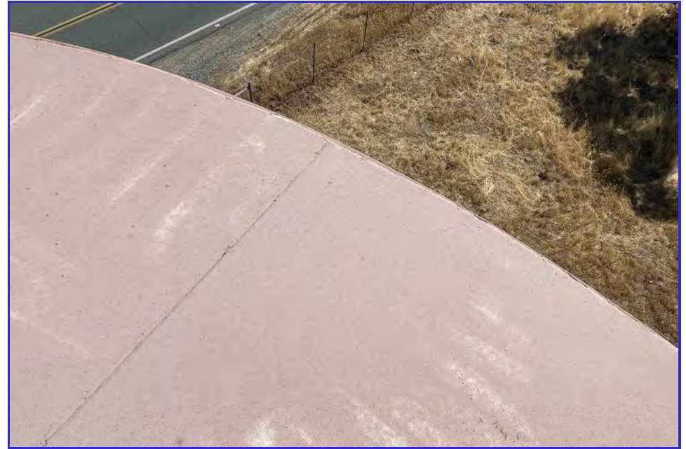
EXTERIOR - CPUD - Paloma Reservoir - Maintenance Inspection -021
