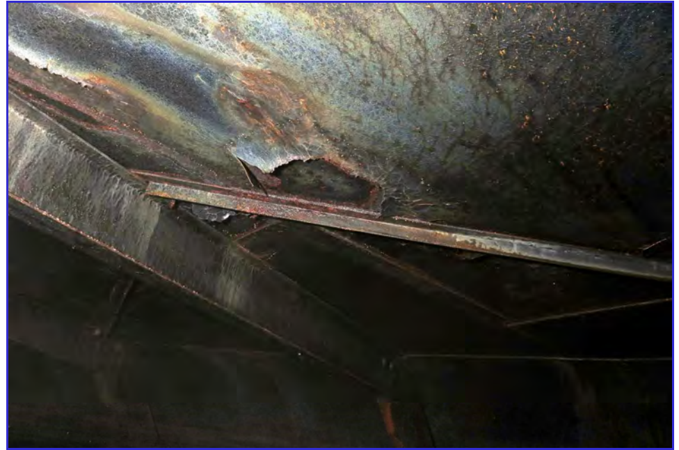
INTERIOR - Calaveras Public Utility District - Clear Well Tank - Maintenance Inspection -053
