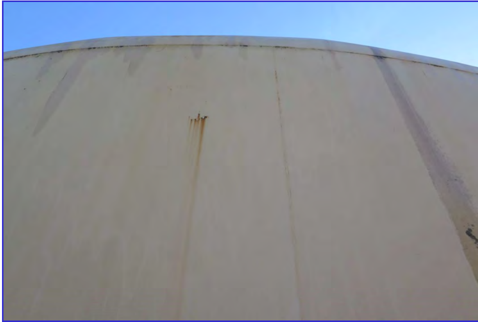
EXTERIOR - Calaveras Public Utility District - Clear Well Tank - Maintenance Inspection -096
