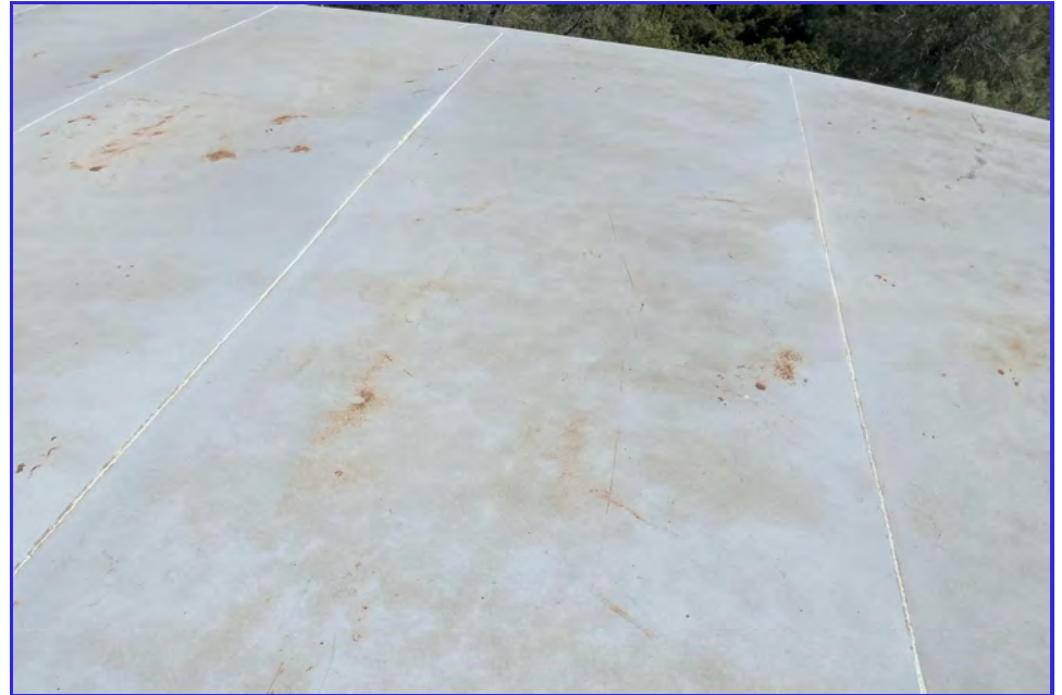
EXTERIOR - CPUD - San Andreas Reservoir - Maintenance Inspection -061
