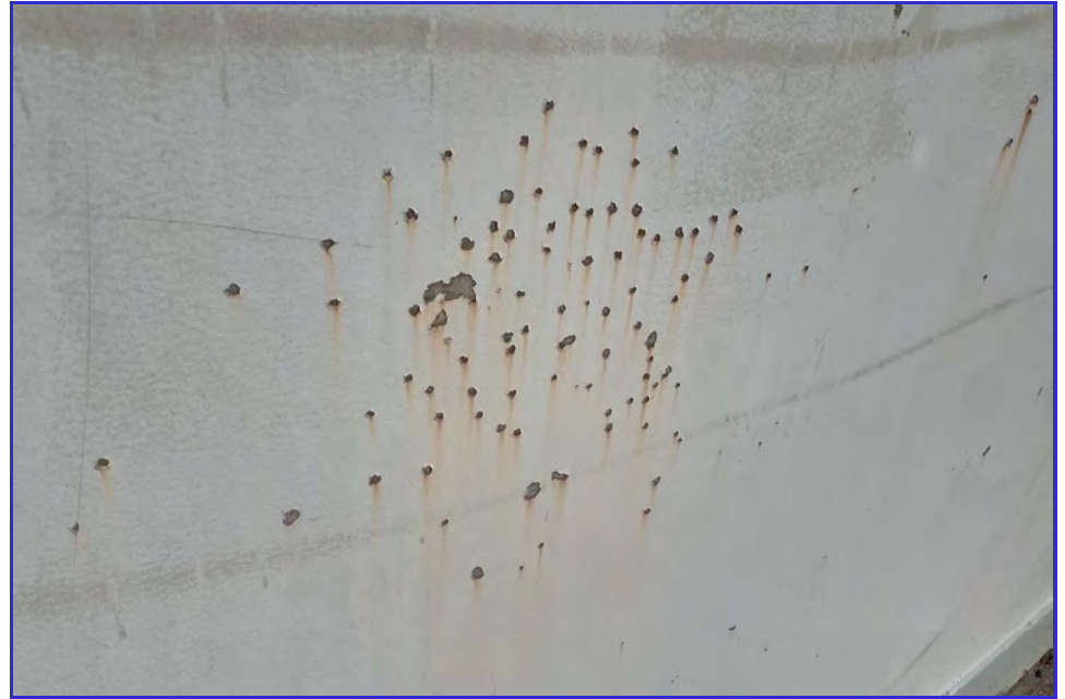
EXTERIOR - CPUD - San Andreas Reservoir - Maintenance Inspection -145
