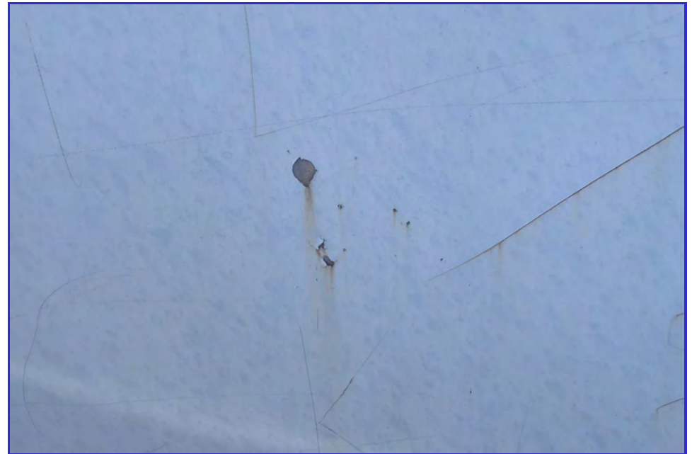
EXTERIOR - CPUD - San Andreas Reservoir - Maintenance Inspection -111
