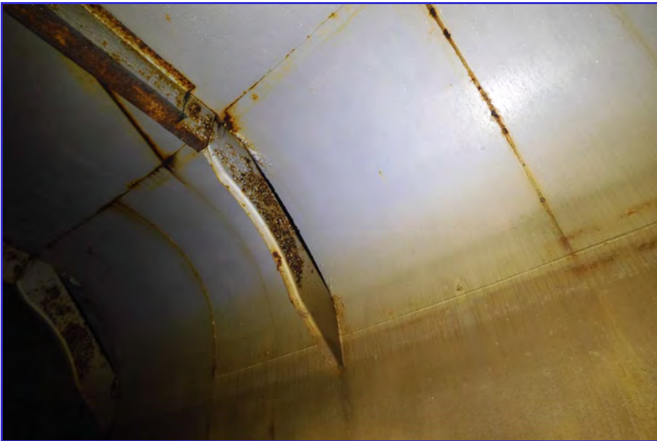
INTERIOR - CPUD - San Andaras Reservoir - Maintenance Inspection -034
