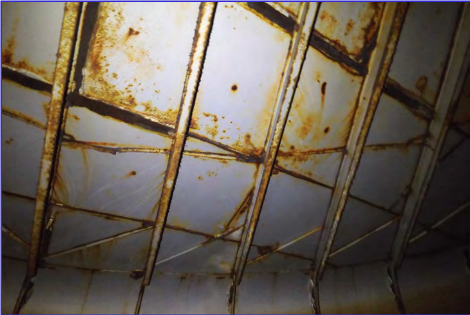
INTERIOR - CPUD - Mokelumne Hill Reservoir - Maintenance Inspection -044
