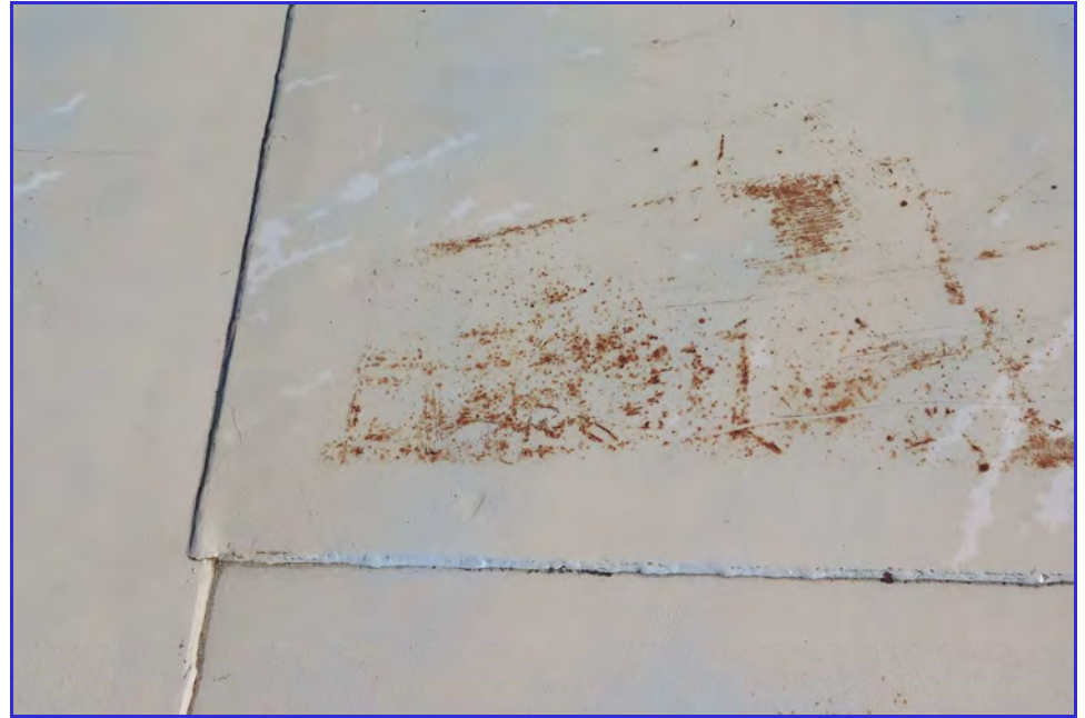
EXTERIOR - Calaveras Public Utility District - Clear Well Tank - Maintenance Inspection -045
