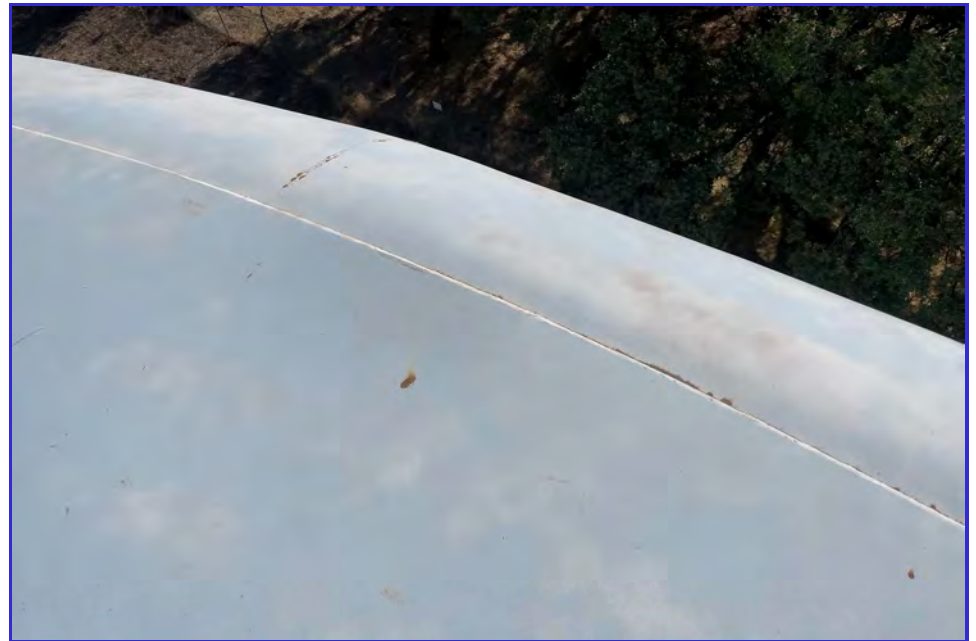
EXTERIOR - CPUD - Mokelumne Reservoir - Maintenance Inspection -055
