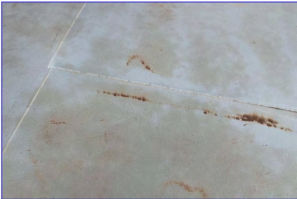
EXTERIOR - CPUD - San Andreas Reservoir - Maintenance Inspection -026
