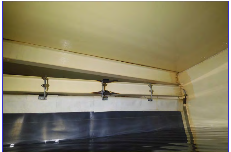
INTERIOR - CPUD - Railroad Flat Reservoir - Maintenance Inspection -051
