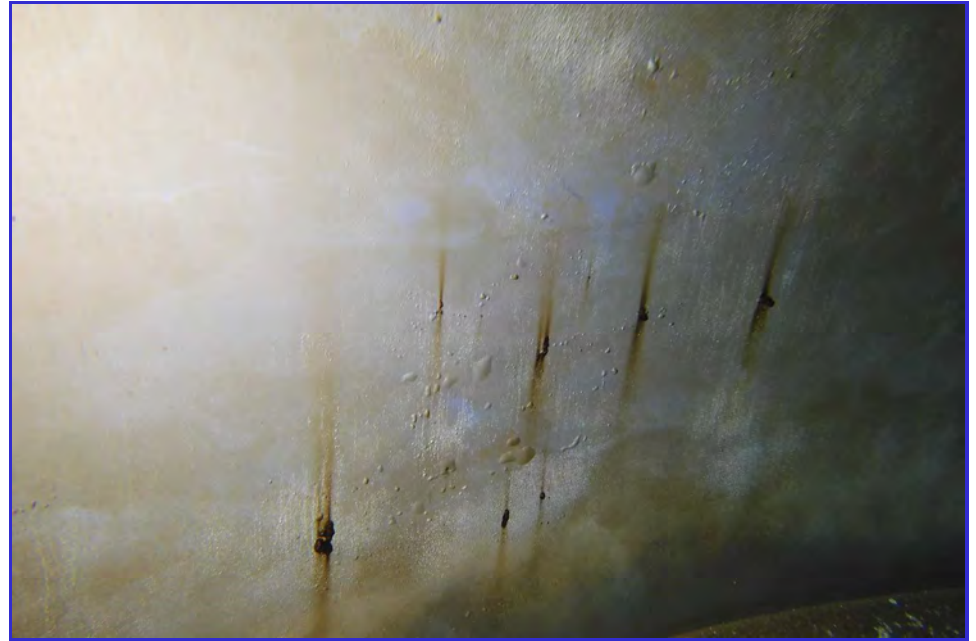
INTERIOR - CPUD - San Andaras Reservoir - Maintenance Inspection -161
