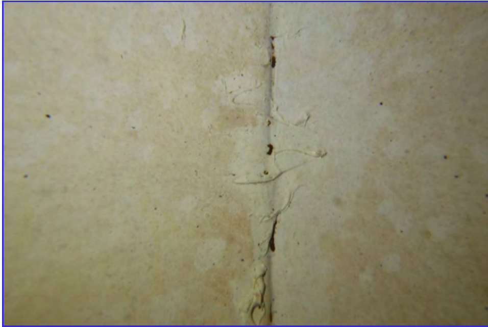
INTERIOR - CPUD - Railroad Flat Reservoir - Maintenance Inspection -152
