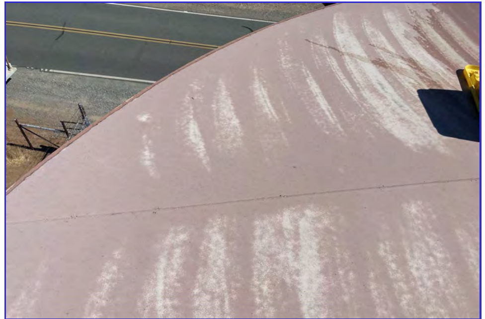
EXTERIOR - CPUD - Paloma Reservoir - Maintenance Inspection -031
