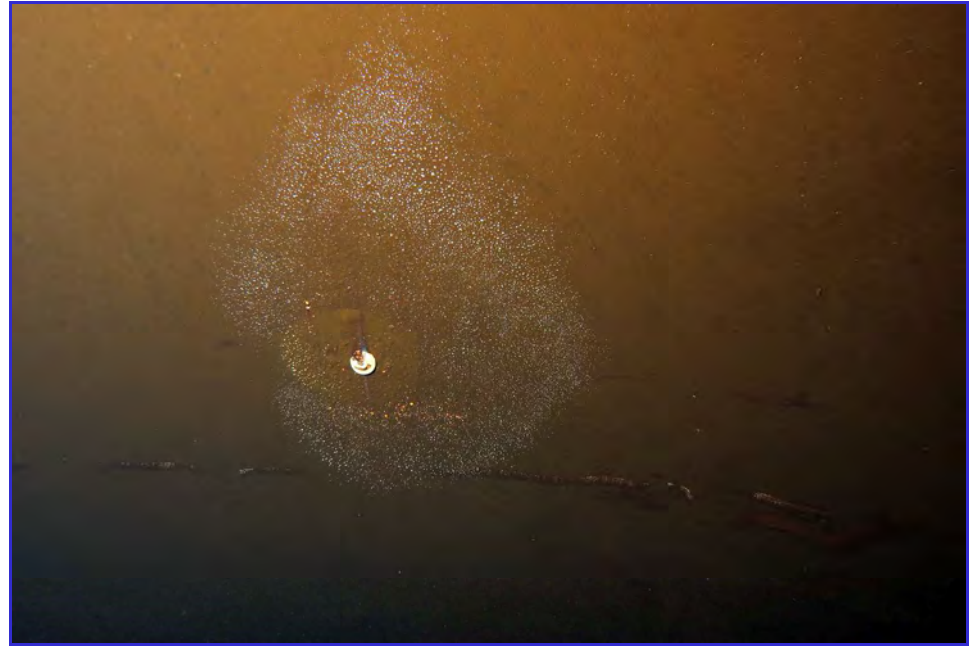
INTERIOR - Calaveras Public Utility District - Clear Well Tank - Maintenance Inspection -097
