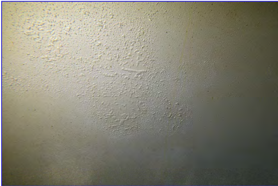
INTERIOR - CPUD - San Andaras Reservoir - Maintenance Inspection -110
