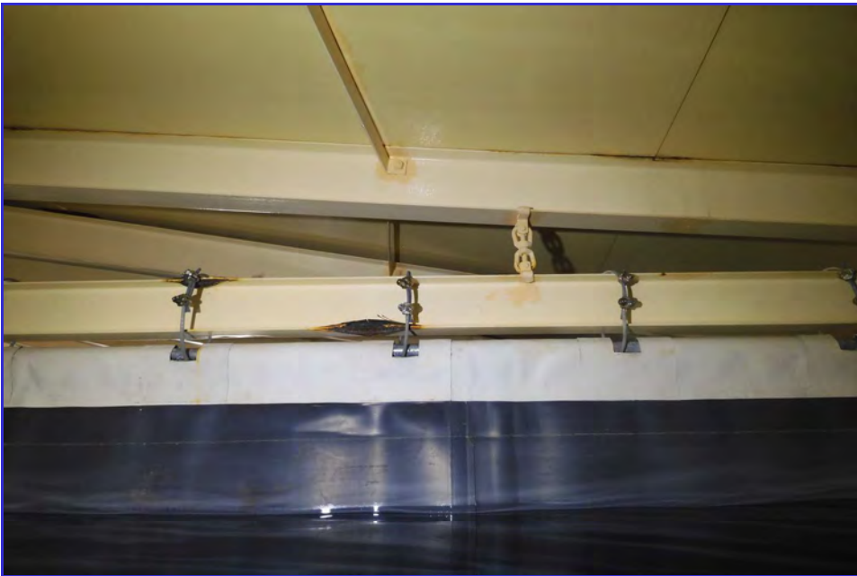
INTERIOR - CPUD - Railroad Flat Reservoir - Maintenance Inspection -050
