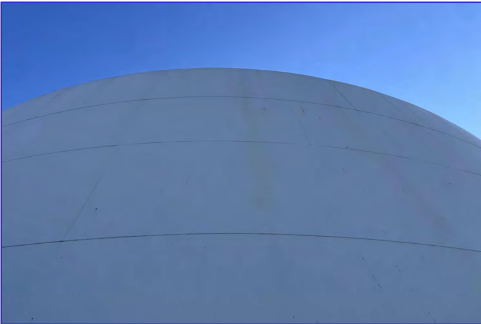
EXTERIOR - CPUD - San Andreas Reservoir - Maintenance Inspection -178
