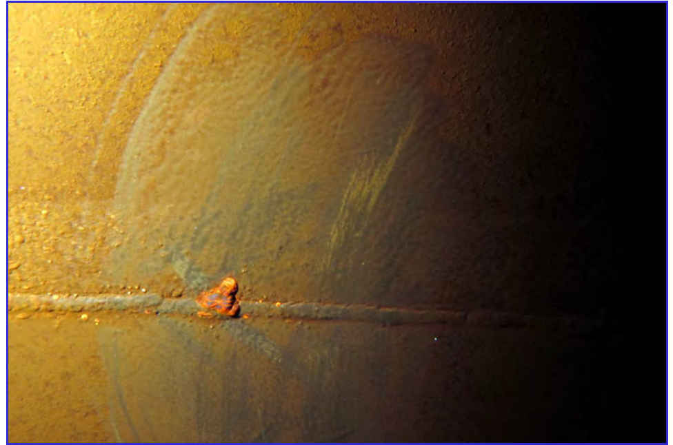
INTERIOR - Calaveras Public Utility District - Clear Well Tank - Maintenance Inspection -073
