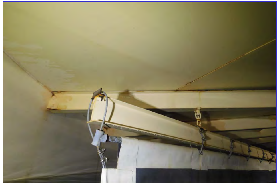
INTERIOR - CPUD - Railroad Flat Reservoir - Maintenance Inspection -055
