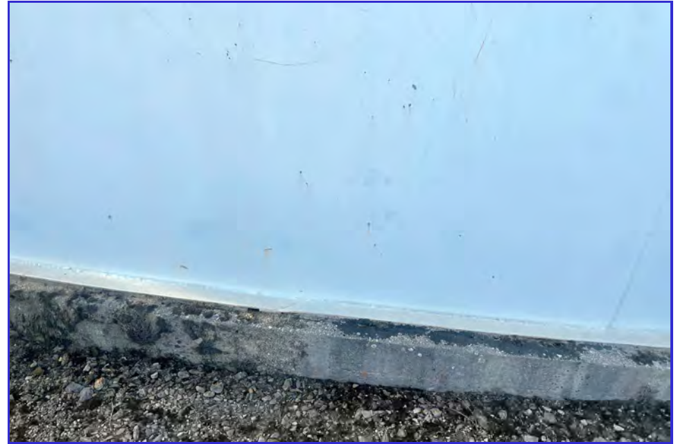
EXTERIOR - CPUD - San Andreas Reservoir - Maintenance Inspection -105
