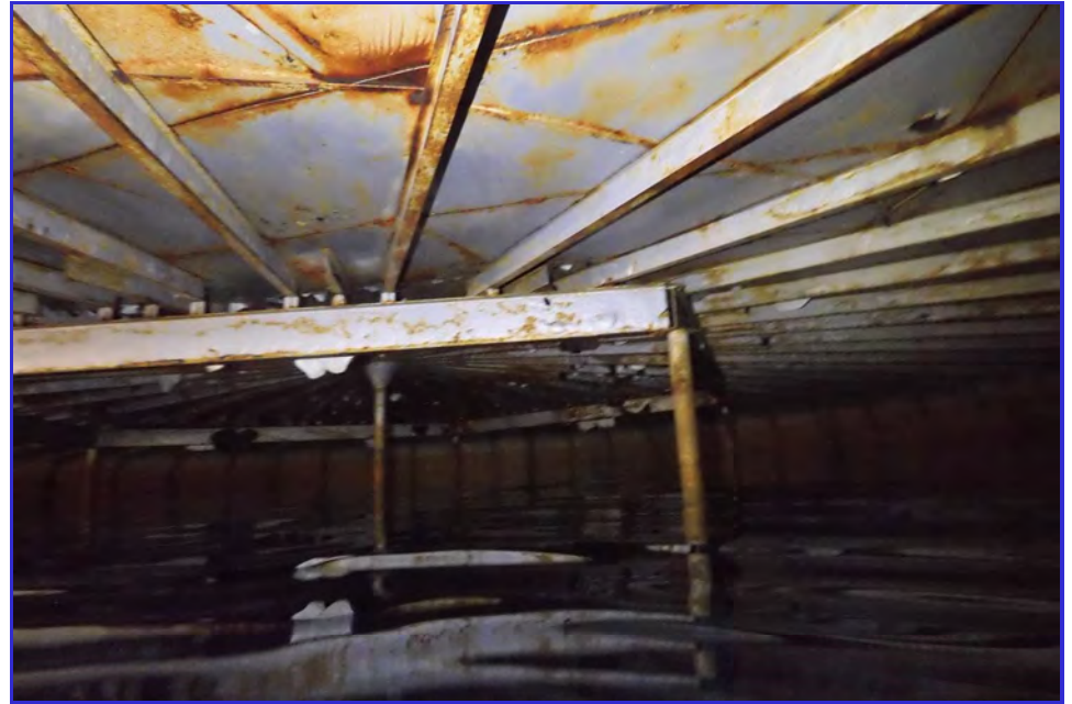
INTERIOR - CPUD - San Andaras Reservoir - Maintenance Inspection -025
