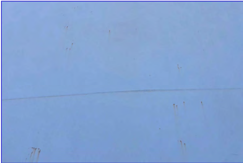
EXTERIOR - CPUD - San Andreas Reservoir - Maintenance Inspection -106
