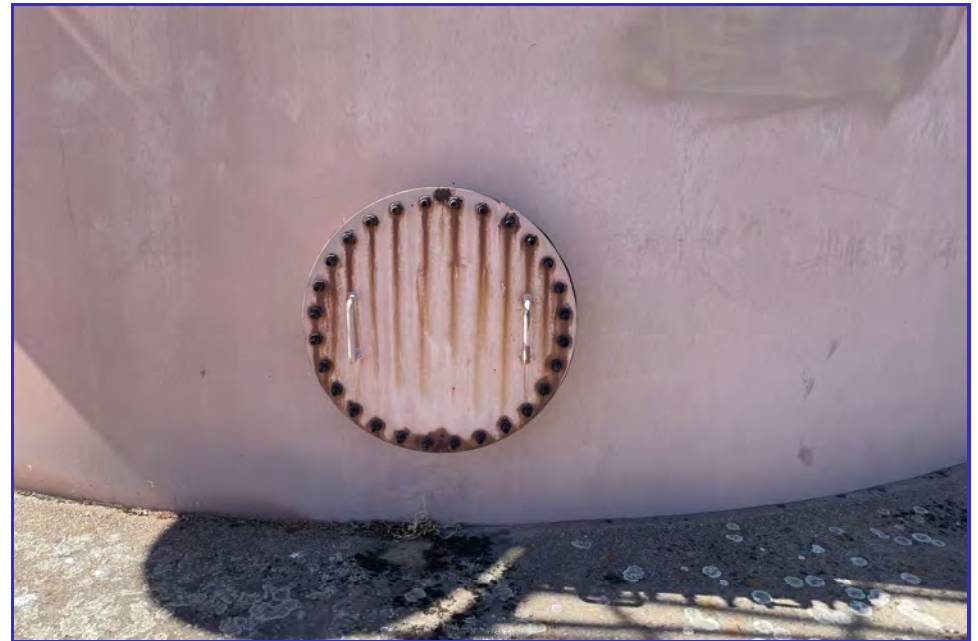
EXTERIOR - CPUD - Paloma Reservoir - Maintenance Inspection -067
