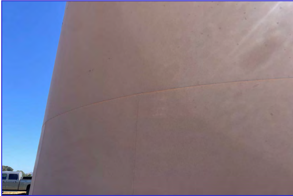
EXTERIOR - CPUD - Paloma Reservoir - Maintenance Inspection -040
