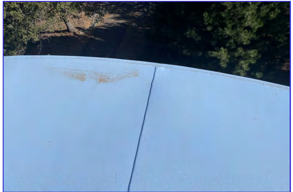
EXTERIOR - CPUD - Railroad Flat Reservoir - Maintenance Inspection -011
