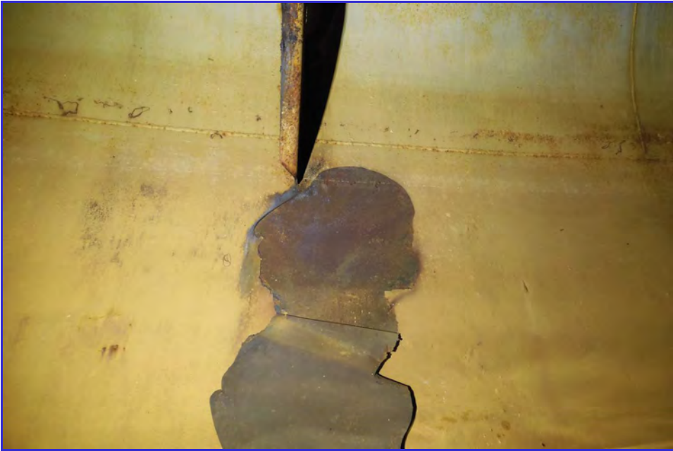
INTERIOR - CPUD - San Andaras Reservoir - Maintenance Inspection -100
