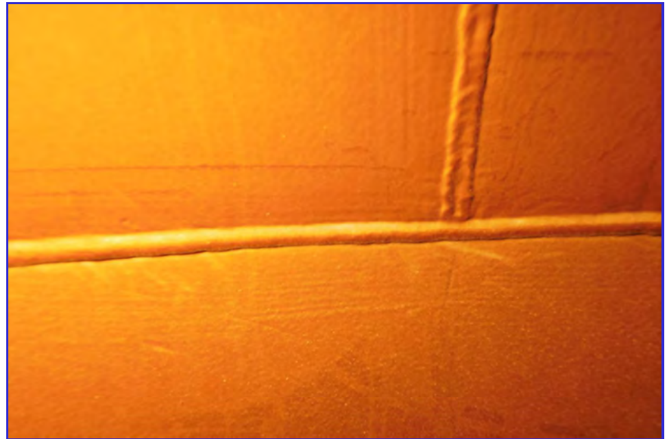
INTERIOR - CPUD - Railroad Flat Reservoir - Maintenance Inspection -103
