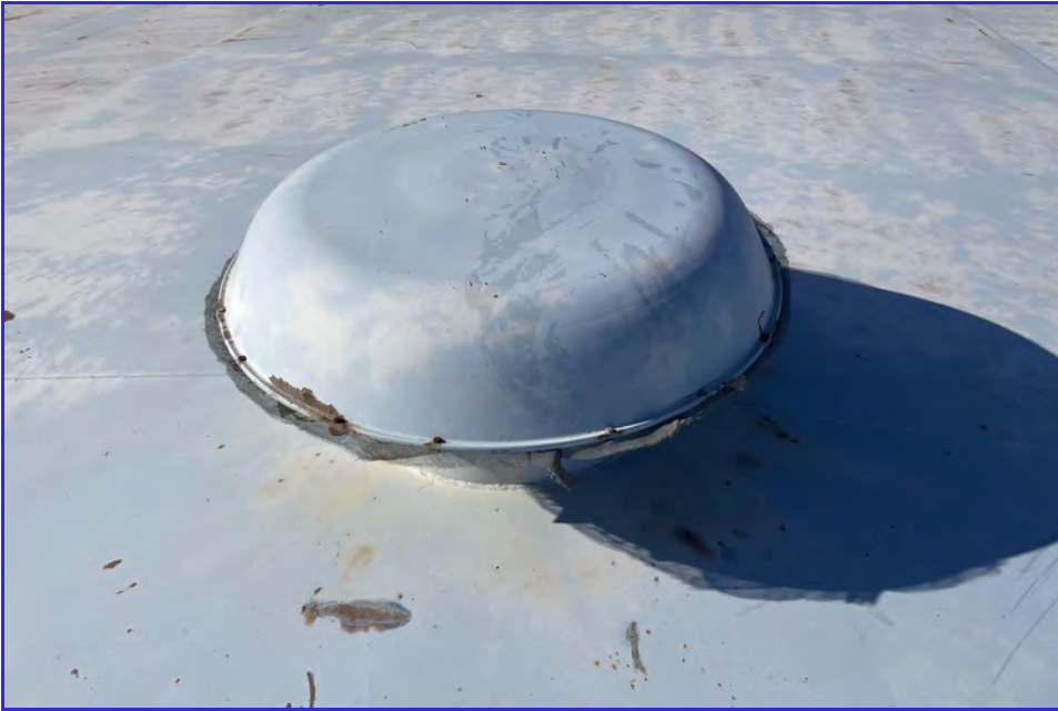
EXTERIOR - CPUD - Mokelumne Reservoir - Maintenance Inspection -028
