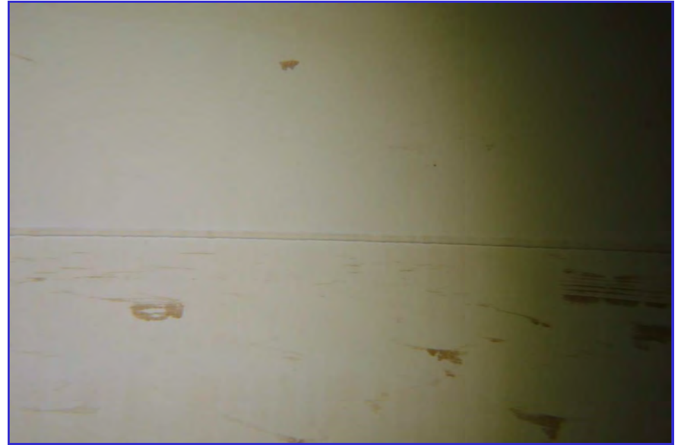
INTERIOR - CPUD - Railroad Flat Reservoir - Maintenance Inspection -073
