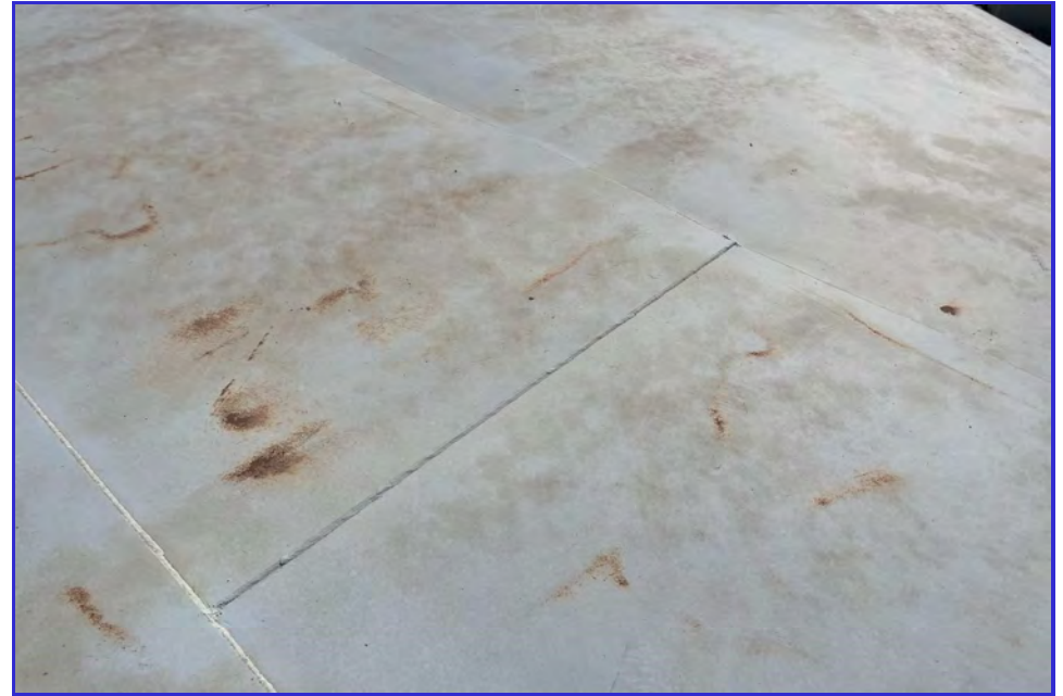
EXTERIOR - CPUD - San Andreas Reservoir - Maintenance Inspection -033
