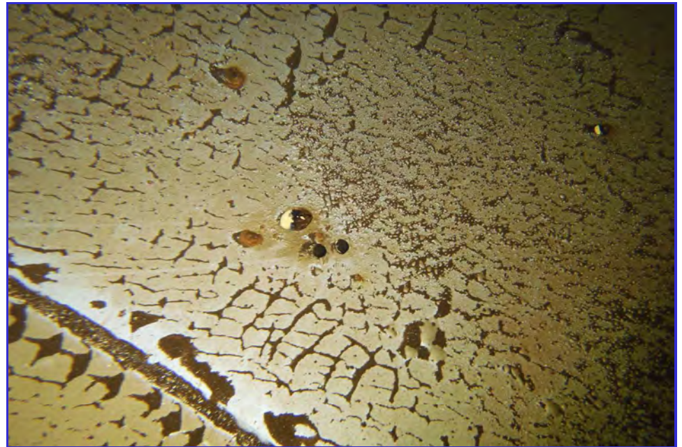
INTERIOR - CPUD - San Andaras Reservoir - Maintenance Inspection -227
