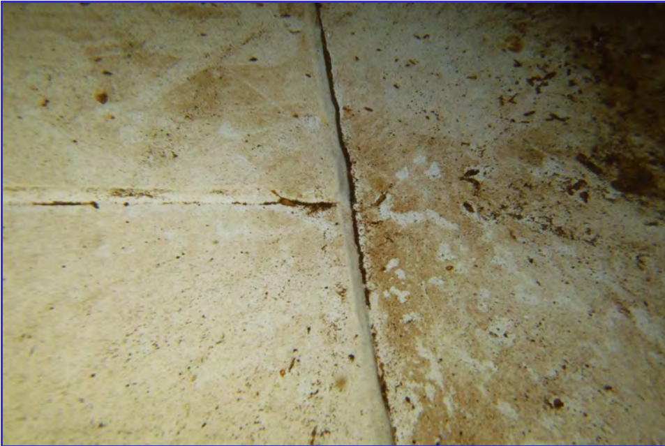
INTERIOR - CPUD - Railroad Flat Reservoir - Maintenance Inspection -156
