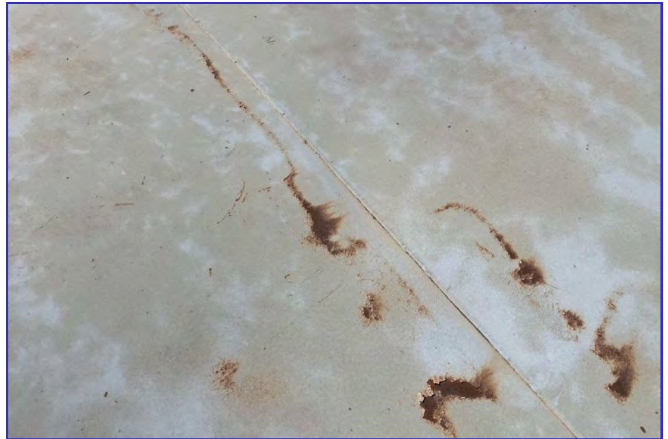
EXTERIOR - CPUD - San Andreas Reservoir - Maintenance Inspection -083
