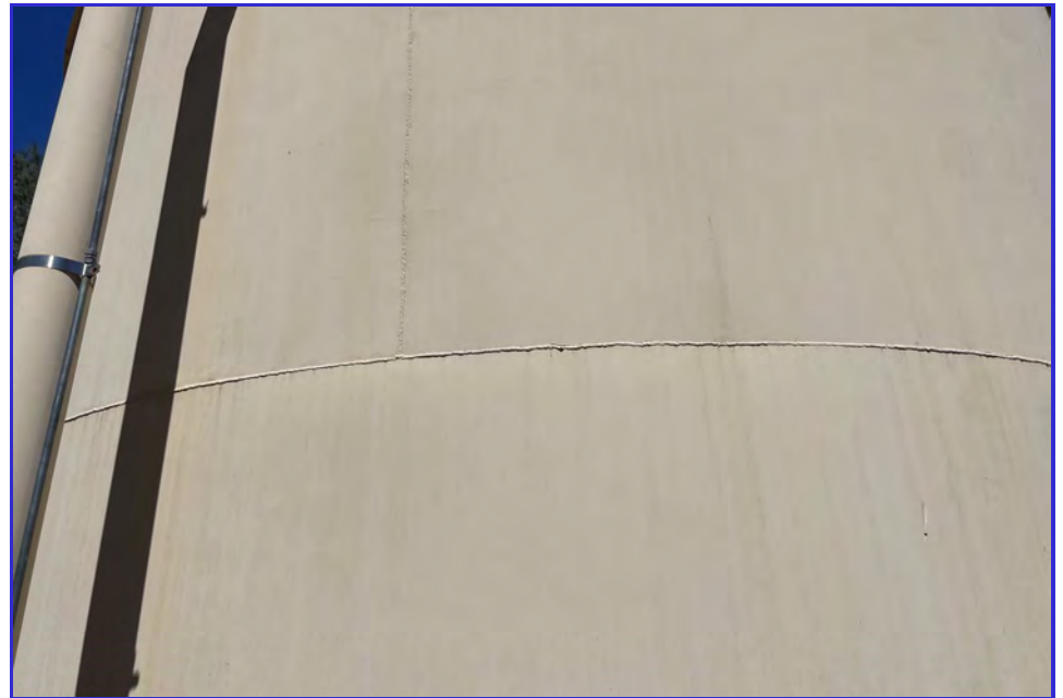
EXTERIOR - CPUD - Golden Hills - Maintenance Inspection -035
