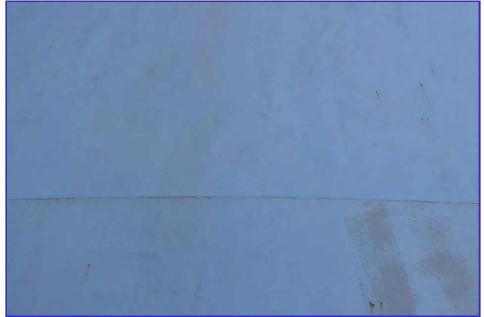
EXTERIOR - CPUD - San Andreas Reservoir - Maintenance Inspection -161
