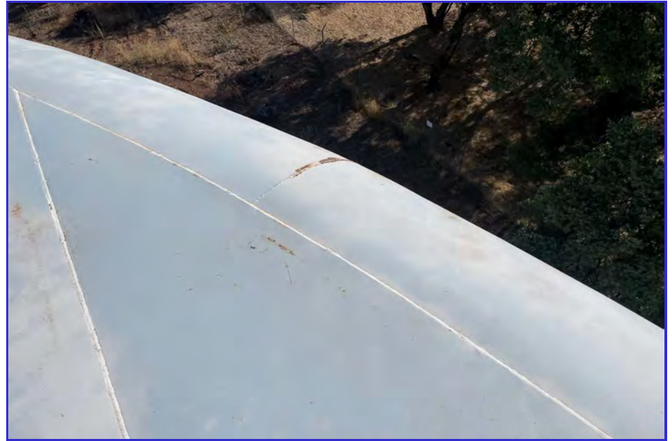
EXTERIOR - CPUD - Mokelumne Reservoir - Maintenance Inspection -053
