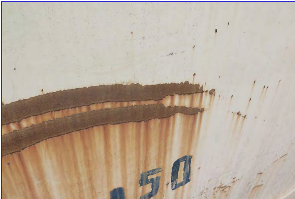
EXTERIOR - Calaveras Public Utility District - Clear Well Tank - Maintenance Inspection -070
