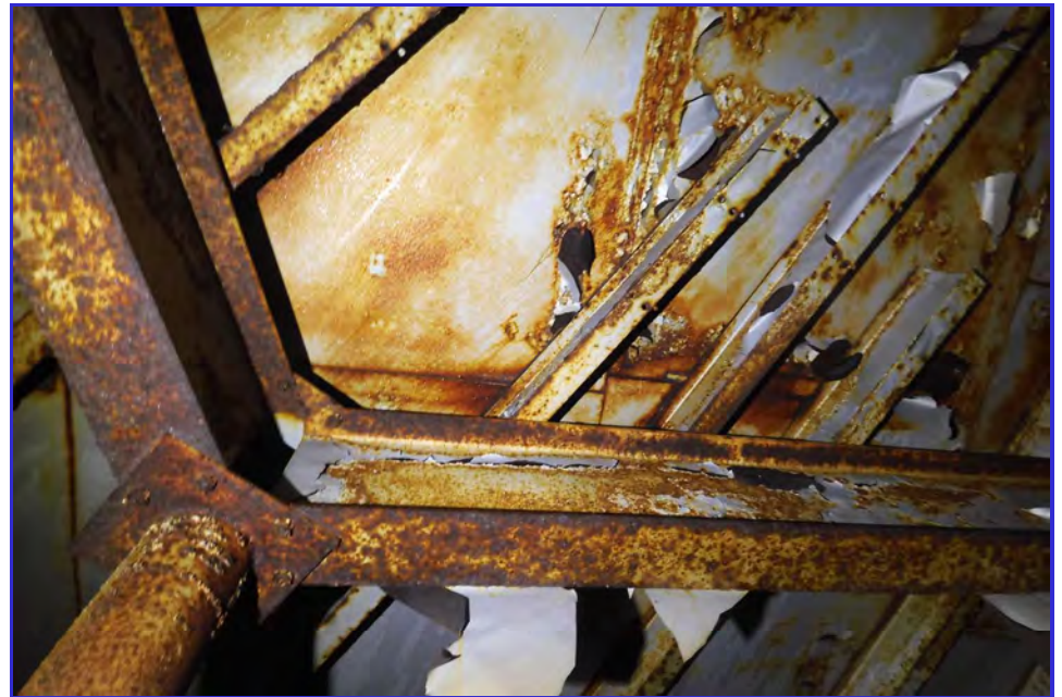
INTERIOR - CPUD - San Andaras Reservoir - Maintenance Inspection -059
