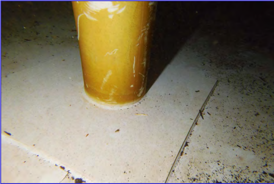
INTERIOR - CPUD - Railroad Flat Reservoir - Maintenance Inspection -136
