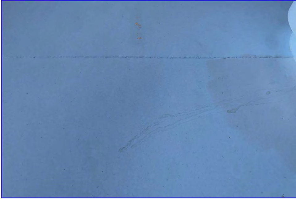
EXTERIOR - CPUD - Railroad Flat Reservoir - Maintenance Inspection -040
