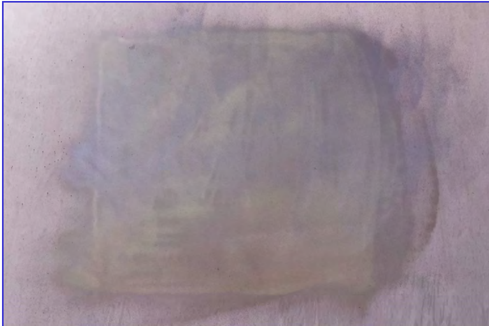
EXTERIOR - CPUD - Paloma Reservoir - Maintenance Inspection -084
