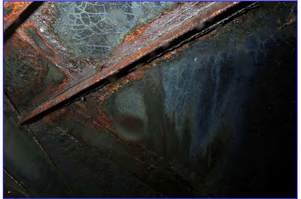
INTERIOR - Calaveras Public Utility District - Clear Well Tank - Maintenance Inspection -033
