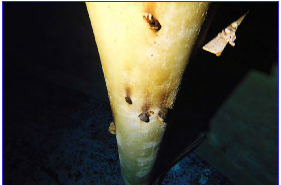
INTERIOR - CPUD - Mokelumne Hill Reservoir - Maintenance Inspection -063
