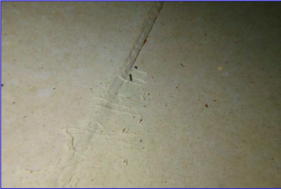
INTERIOR - CPUD - Railroad Flat Reservoir - Maintenance Inspection -148
