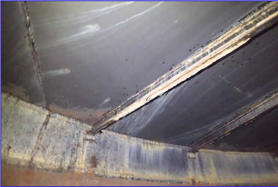
INTERIOR - CPUD - Paloma Reservoir - Maintenance Inspection -024
