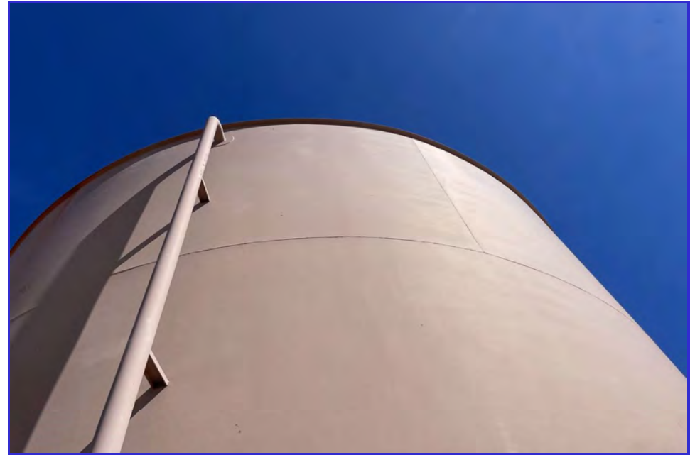
EXTERIOR - CPUD - Paloma Reservoir - Maintenance Inspection -077
