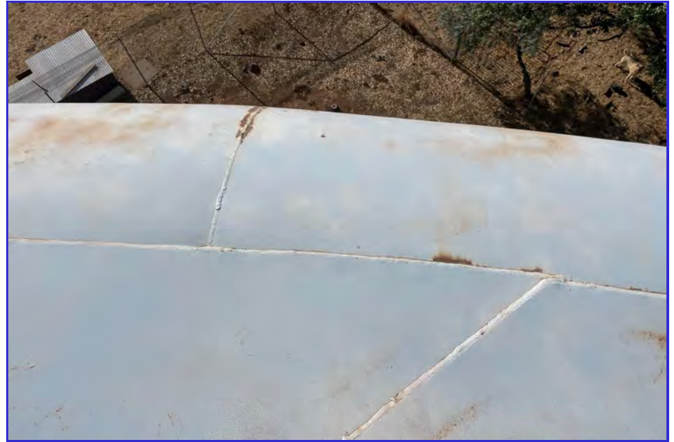
EXTERIOR - CPUD - Mokelumne Reservoir - Maintenance Inspection -061
