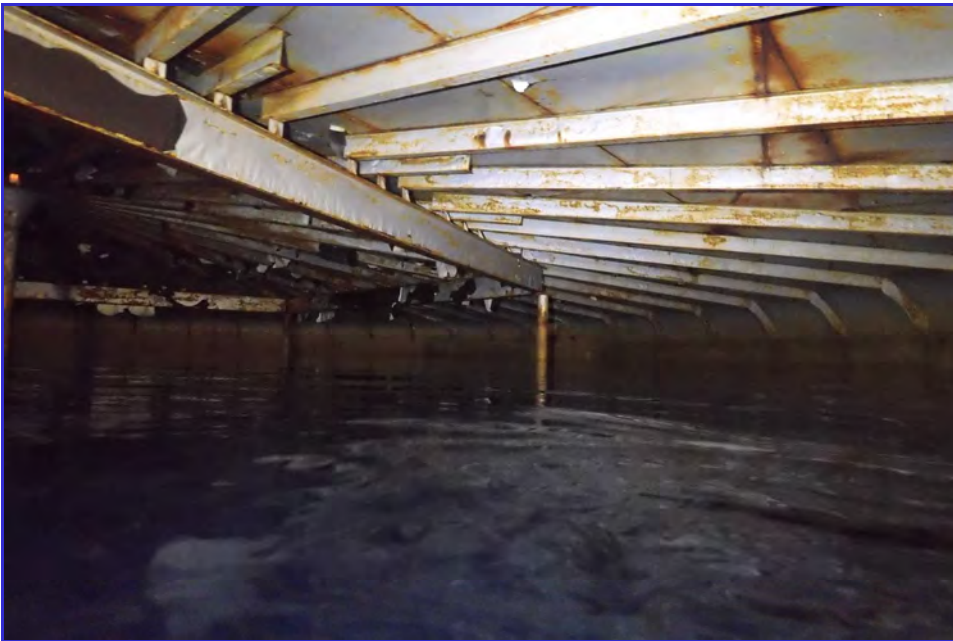
INTERIOR - CPUD - San Andaras Reservoir - Maintenance Inspection -010
