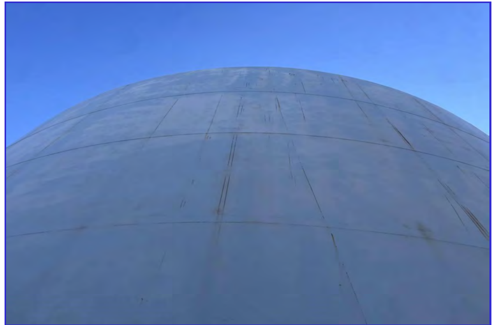
EXTERIOR - CPUD - Mokelumne Reservoir - Maintenance Inspection -151
