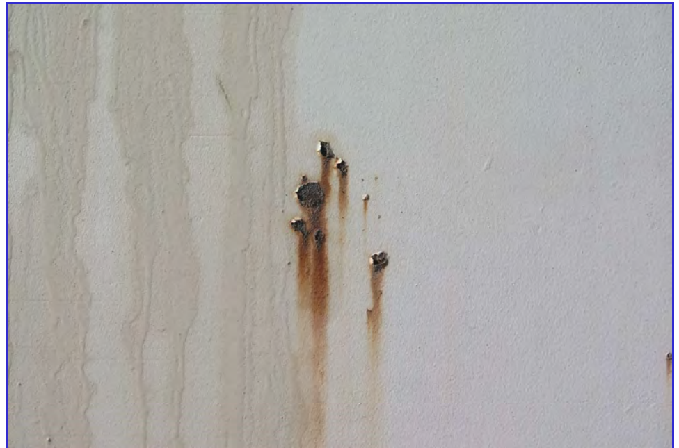
EXTERIOR - Calaveras Public Utility District - Clear Well Tank - Maintenance Inspection -119
