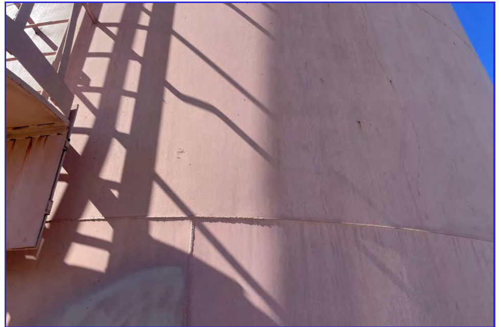
EXTERIOR - CPUD - Paloma Reservoir - Maintenance Inspection -063
