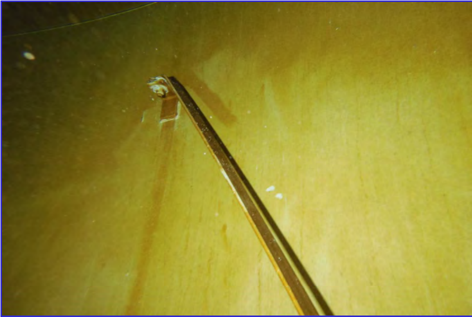
INTERIOR - CPUD - Railroad Flat Reservoir - Maintenance Inspection -120
