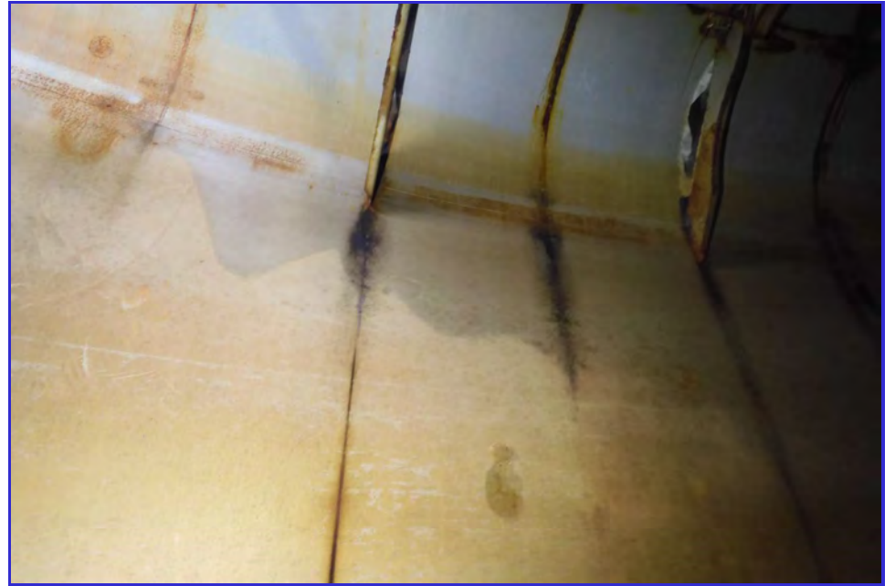
INTERIOR - CPUD - Mokelumne Hill Reservoir - Maintenance Inspection -001
