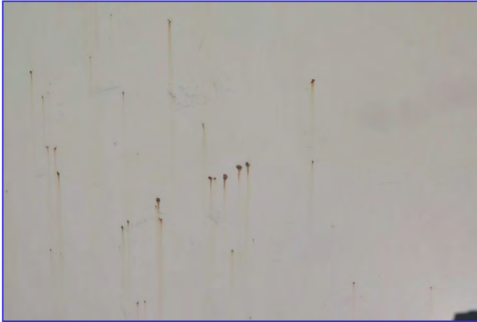
EXTERIOR - Calaveras Public Utility District - Clear Well Tank - Maintenance Inspection -056
