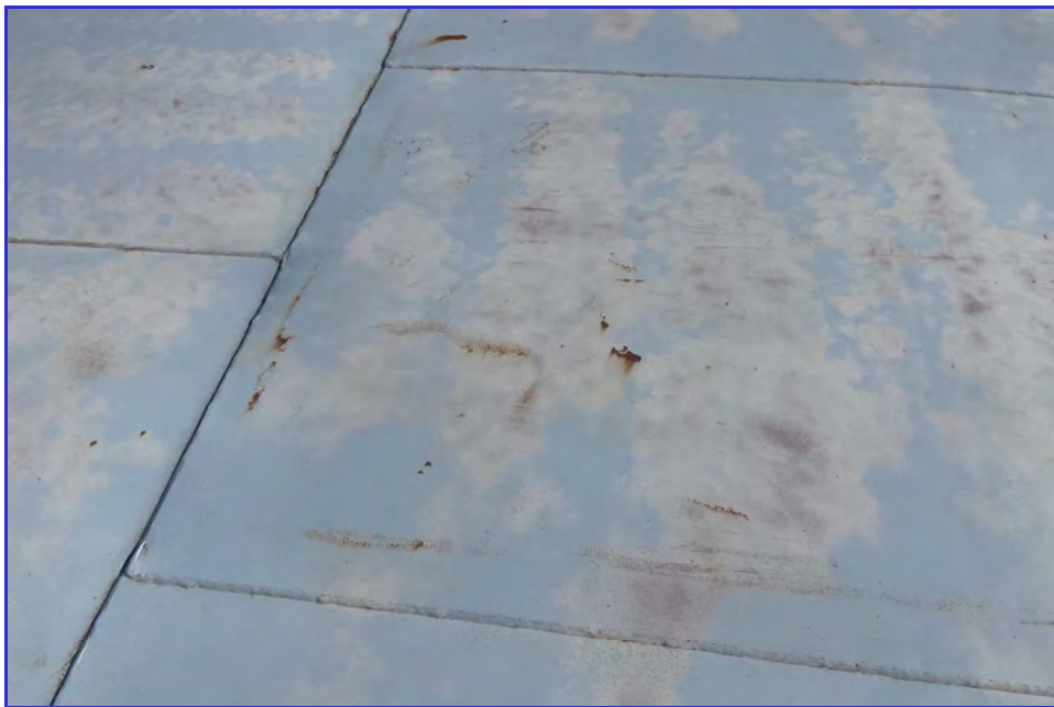
EXTERIOR - CPUD - Mokelumne Reservoir - Maintenance Inspection -042
