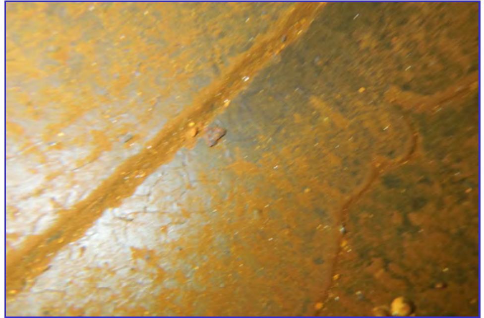
INTERIOR - CPUD - Paloma Reservoir - Maintenance Inspection -145
