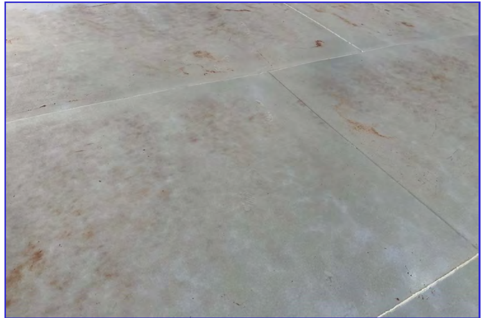
EXTERIOR - CPUD - San Andreas Reservoir - Maintenance Inspection -075
