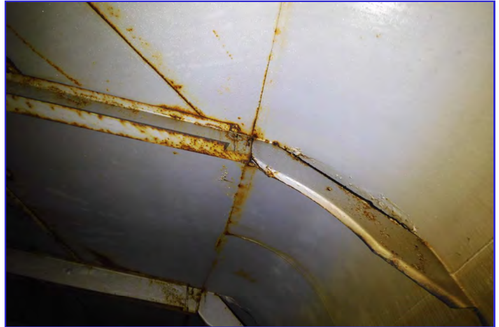
INTERIOR - CPUD - San Andaras Reservoir - Maintenance Inspection -029
