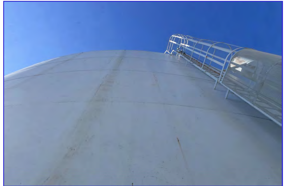
EXTERIOR - CPUD - Mokelumne Reservoir - Maintenance Inspection -135
