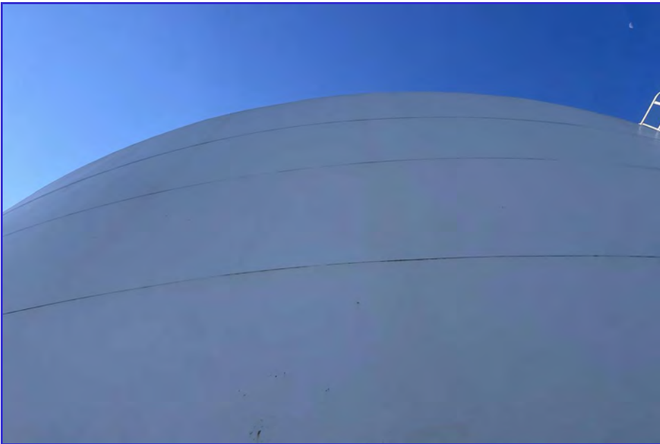
EXTERIOR - CPUD - San Andreas Reservoir - Maintenance Inspection -190
