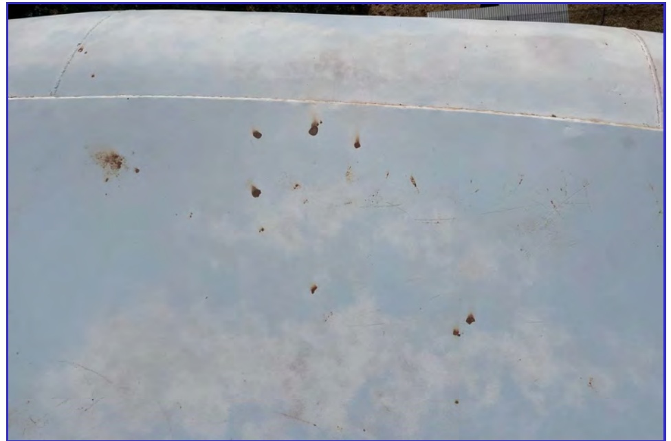
EXTERIOR - CPUD - Mokelumne Reservoir - Maintenance Inspection -059
