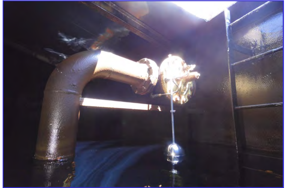
INTERIOR - CPUD - Paloma Reservoir - Maintenance Inspection -001
