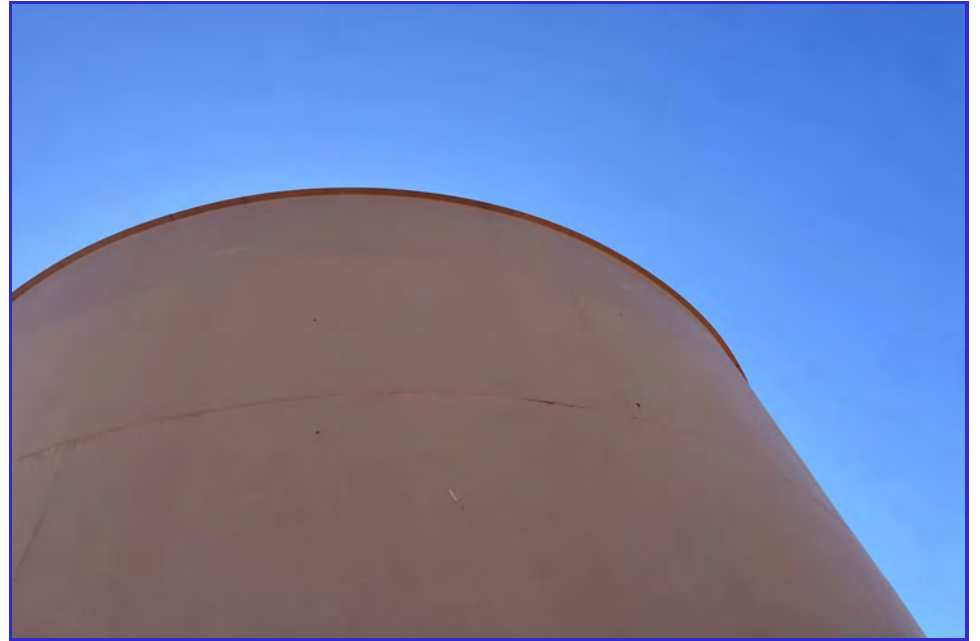
EXTERIOR - CPUD - Paloma Reservoir - Maintenance Inspection -037
