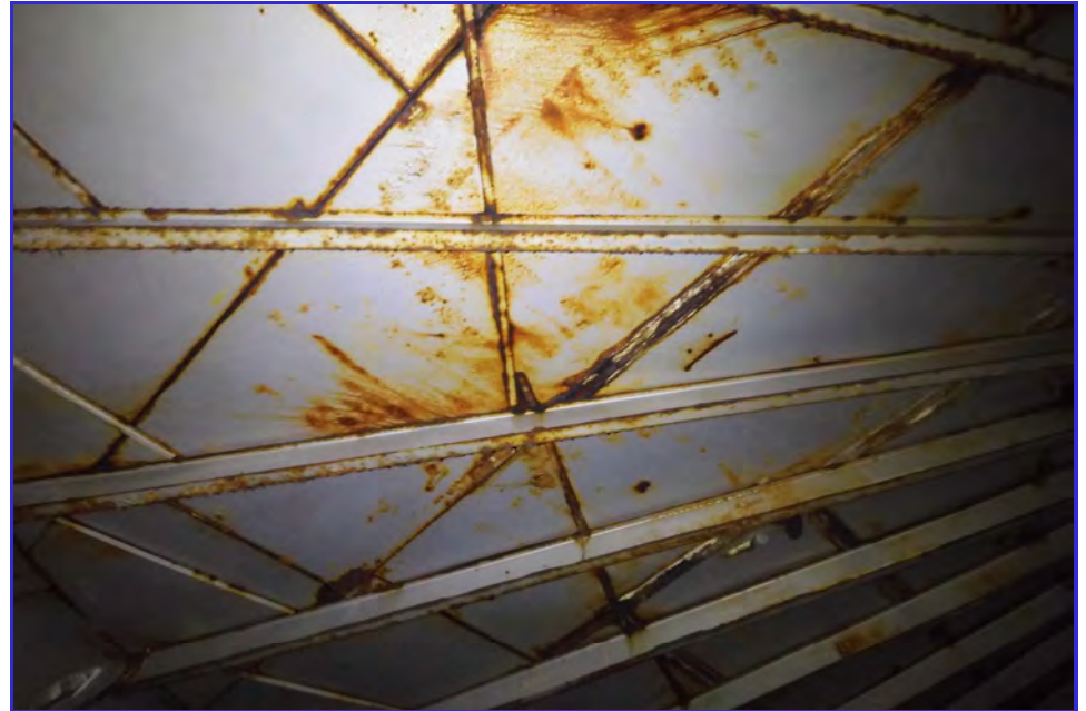
INTERIOR - CPUD - Mokelumne Hill Reservoir - Maintenance Inspection -037
