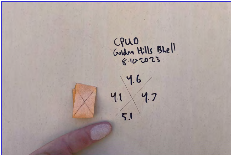
EXTERIOR - CPUD - Golden Hills - Maintenance Inspection -066
