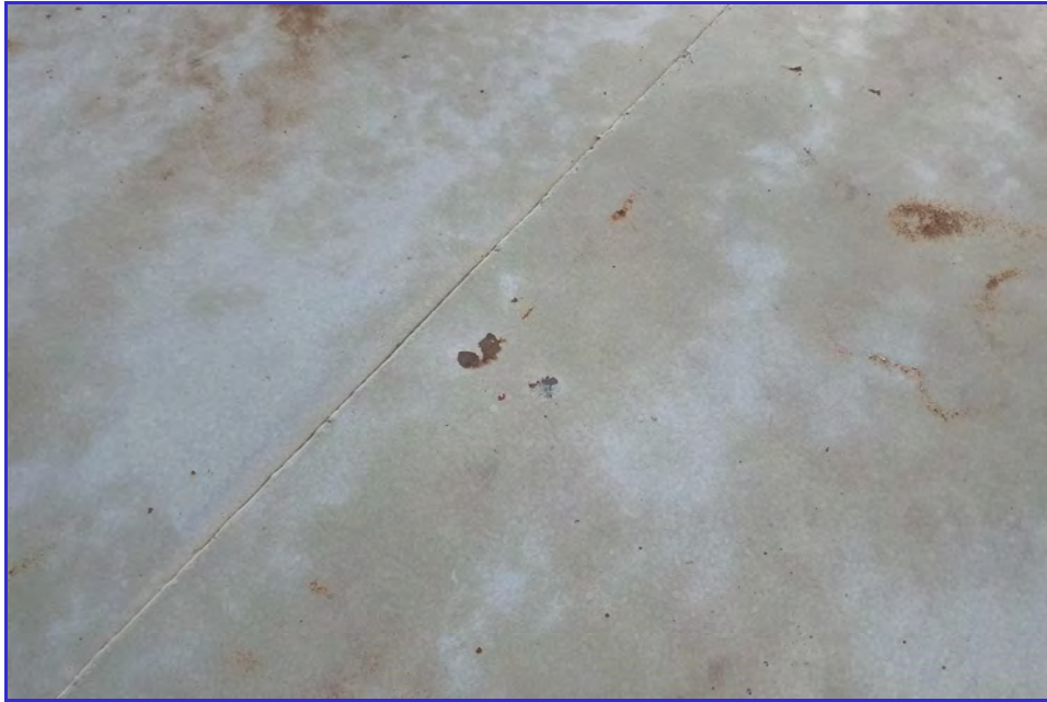
EXTERIOR - CPUD - San Andreas Reservoir - Maintenance Inspection -020
