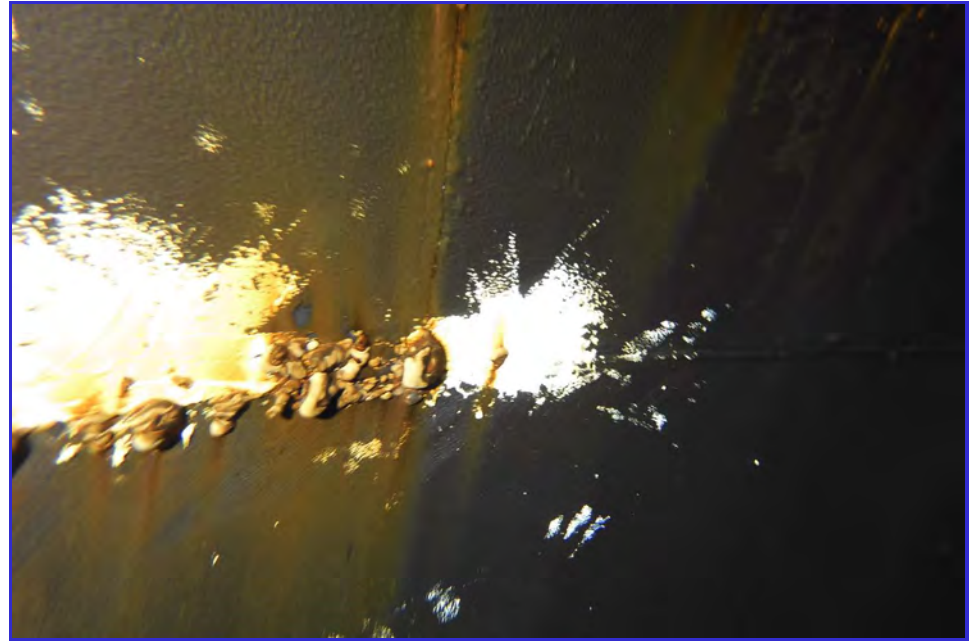
INTERIOR - CPUD - Paloma Reservoir - Maintenance Inspection -053
