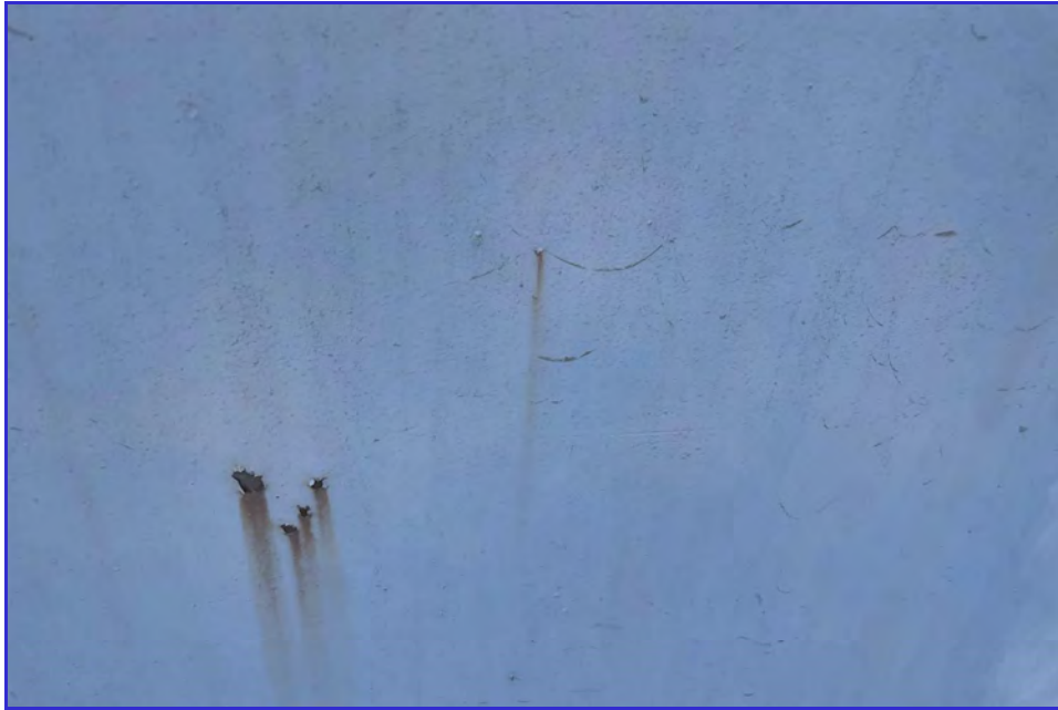
EXTERIOR - CPUD - Mokelumne Reservoir - Maintenance Inspection -096
