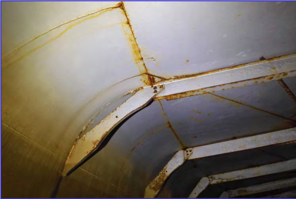
INTERIOR - CPUD - San Andaras Reservoir - Maintenance Inspection -032
