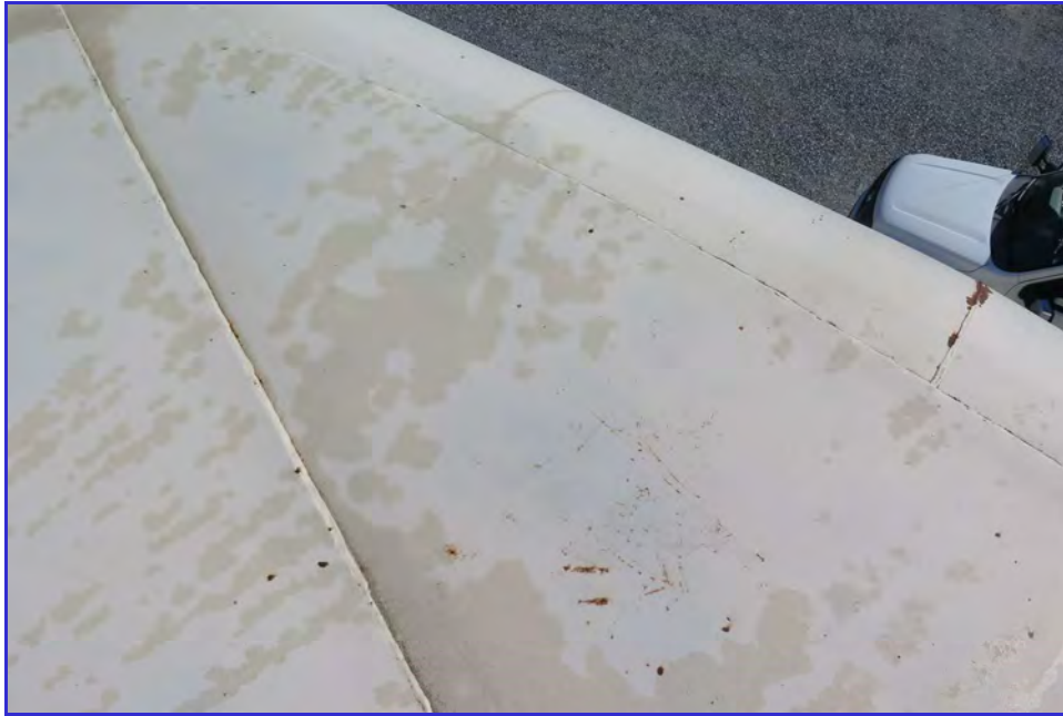
EXTERIOR - Calaveras Public Utility District - Clear Well Tank - Maintenance Inspection -004
