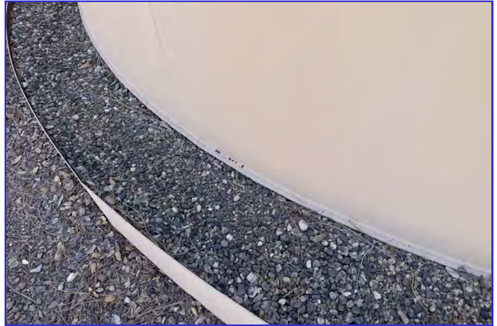
EXTERIOR - CPUD - Golden Hills - Maintenance Inspection -057
