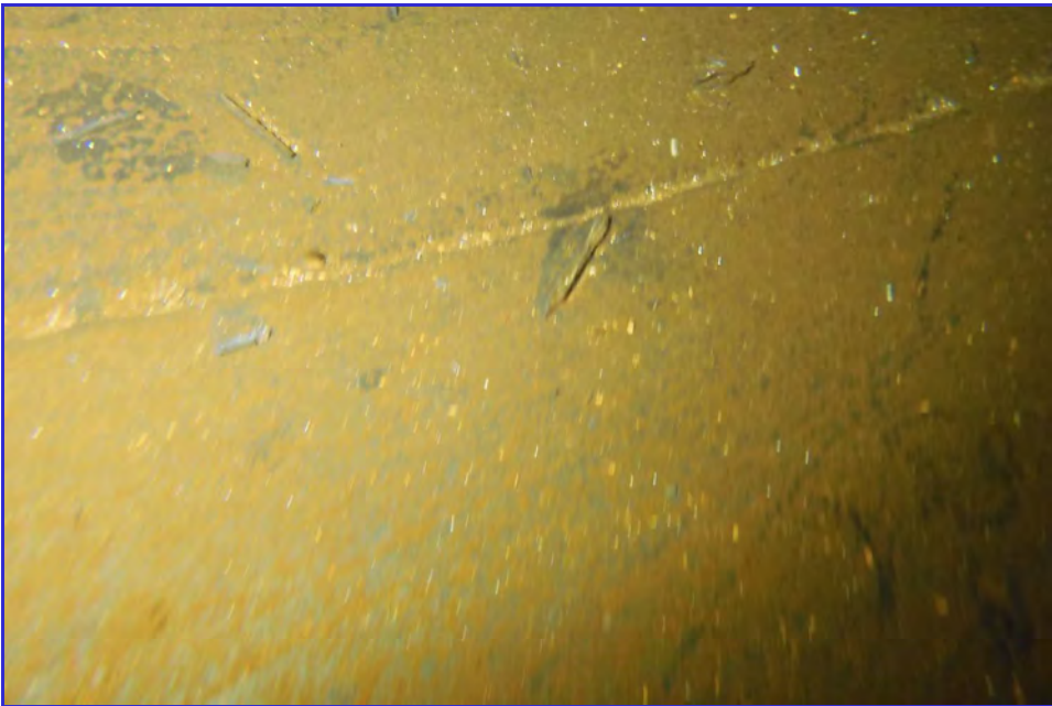
INTERIOR - CPUD - Paloma Reservoir - Maintenance Inspection -130
