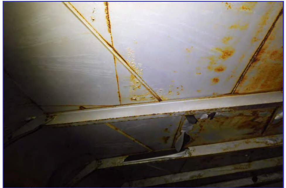
INTERIOR - CPUD - San Anderas Reservoir - Maintenance Inspection -043
