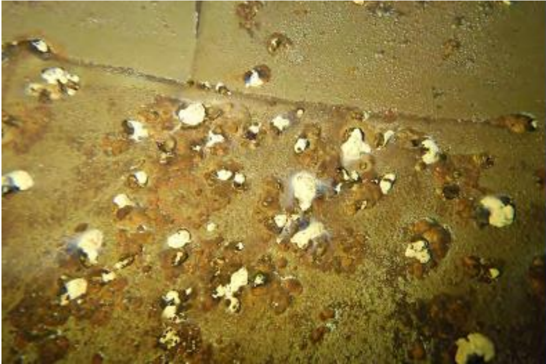
Figure 9-14. Example of San Andreas Tank Interior Floor
