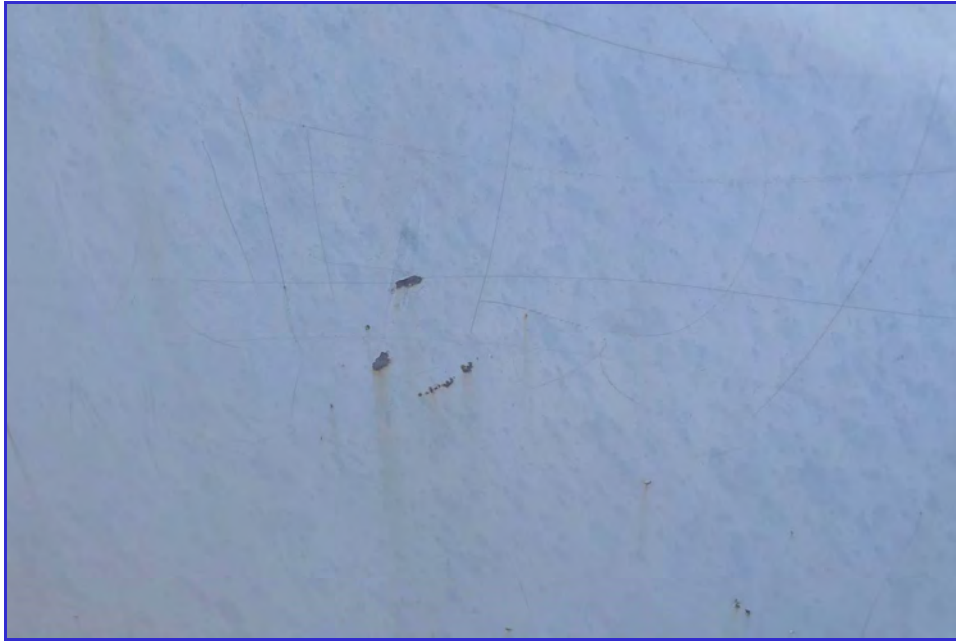
EXTERIOR - CPUD - San Andreas Reservoir - Maintenance Inspection -112
