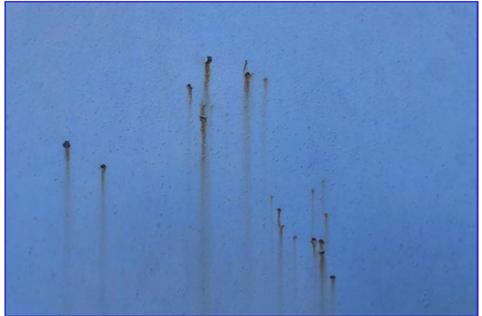
EXTERIOR - CPUD - Mokelumne Reservoir - Maintenance Inspection -121
