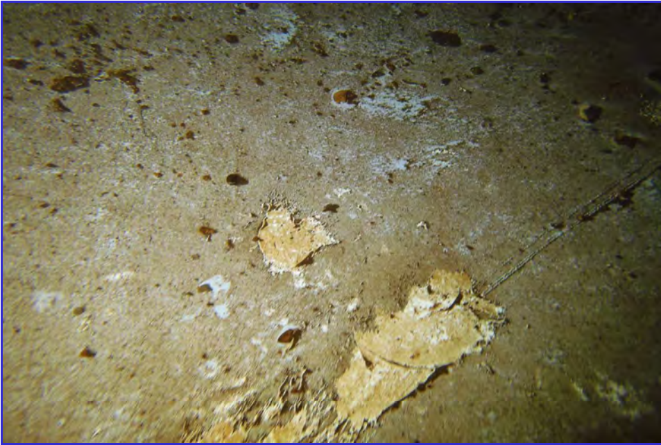
INTERIOR - CPUD - Mokelumne Hill Reservoir - Maintenance Inspection -156
