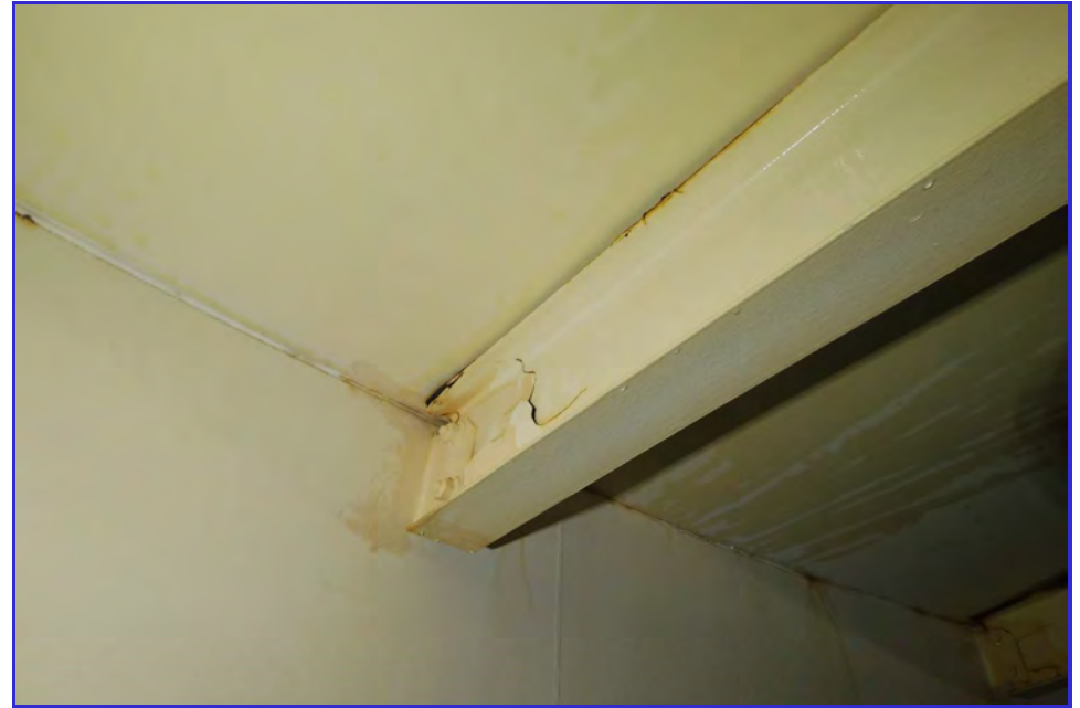
INTERIOR - CPUD - Railroad Flat Reservoir - Maintenance Inspection -065
