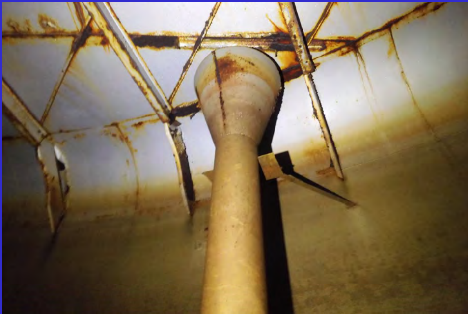
INTERIOR - CPUD - Mokelumne Hill Reservoir - Maintenance Inspection -012
