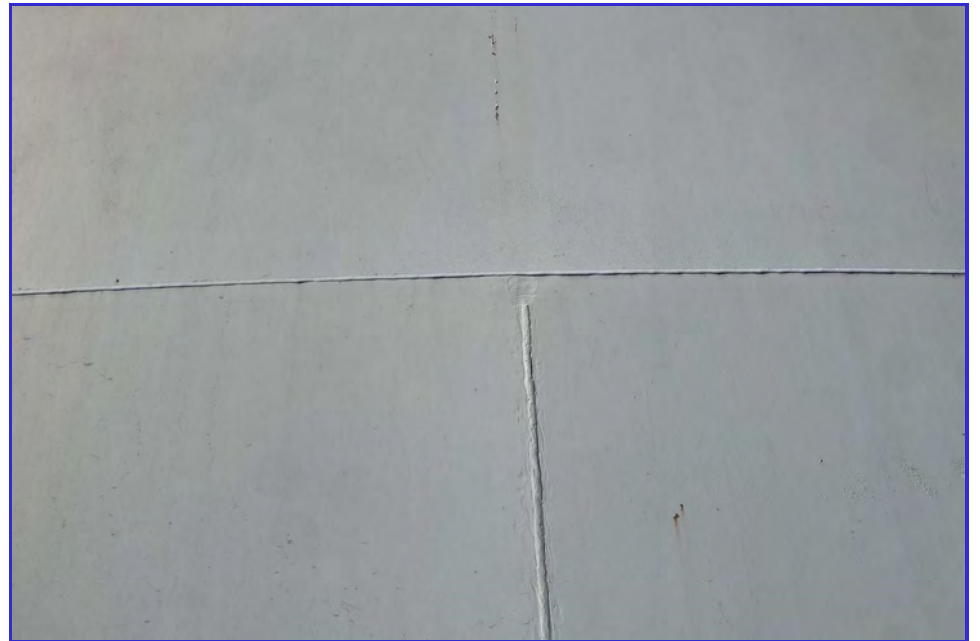
EXTERIOR - CPUD - Mokelumne Reservoir - Maintenance Inspection -087
