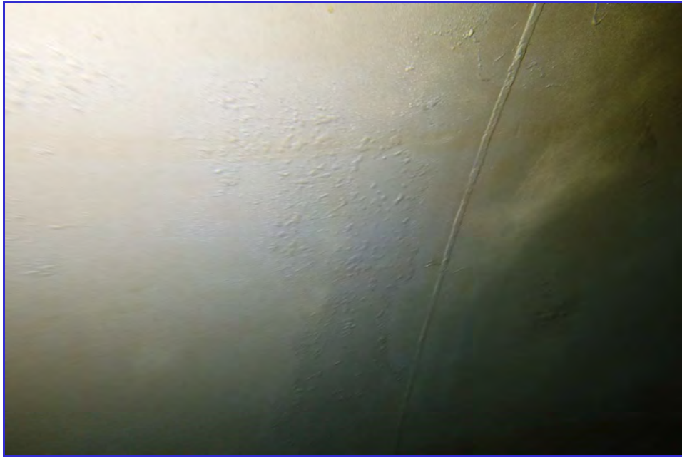
INTERIOR - CPUD - San Andaras Reservoir - Maintenance Inspection -108
