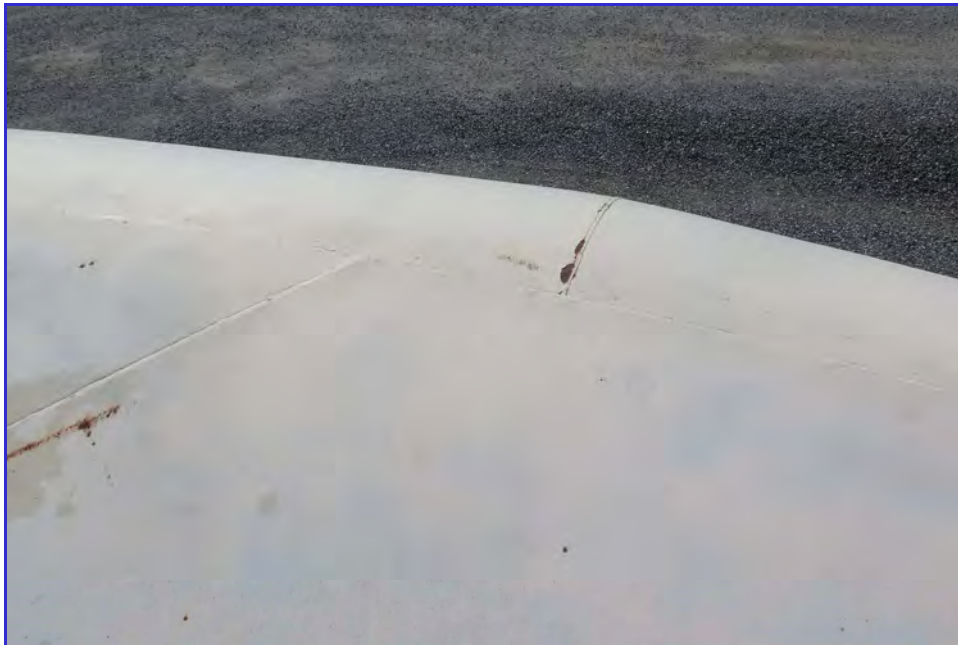
EXTERIOR - Calaveras Public Utility District - Clear Well Tank - Maintenance Inspection -034
