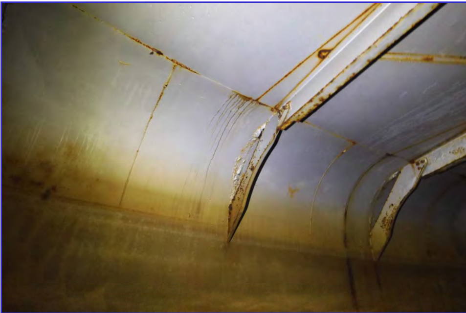
INTERIOR - CPUD - San Anderas Reservoir - Maintenance Inspection -042
