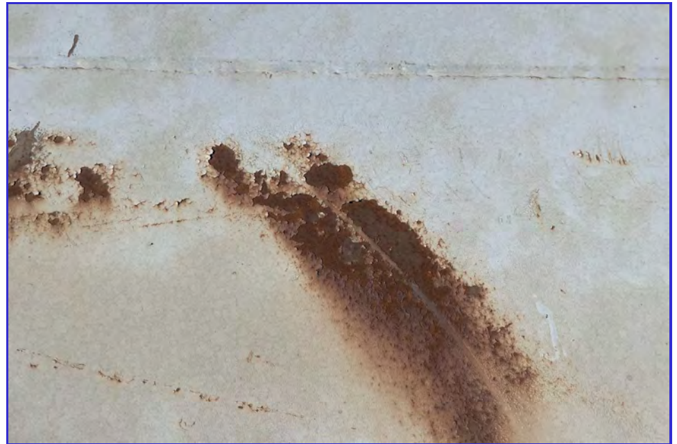
EXTERIOR - CPUD - San Andreas Reservoir - Maintenance Inspection -067
