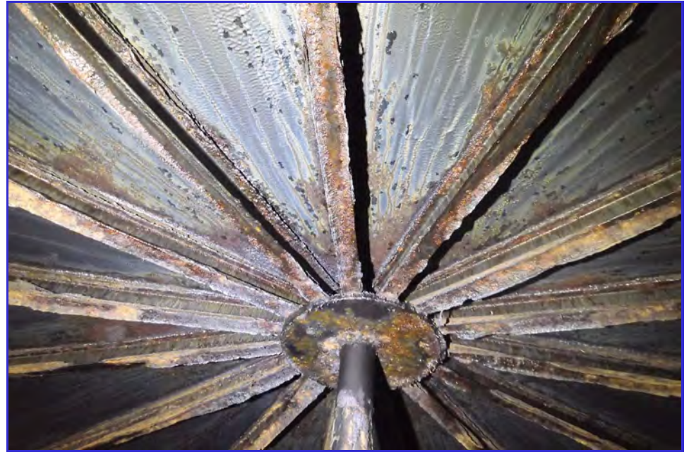
INTERIOR - CPUD - Paloma Reservoir - Maintenance Inspection -033
