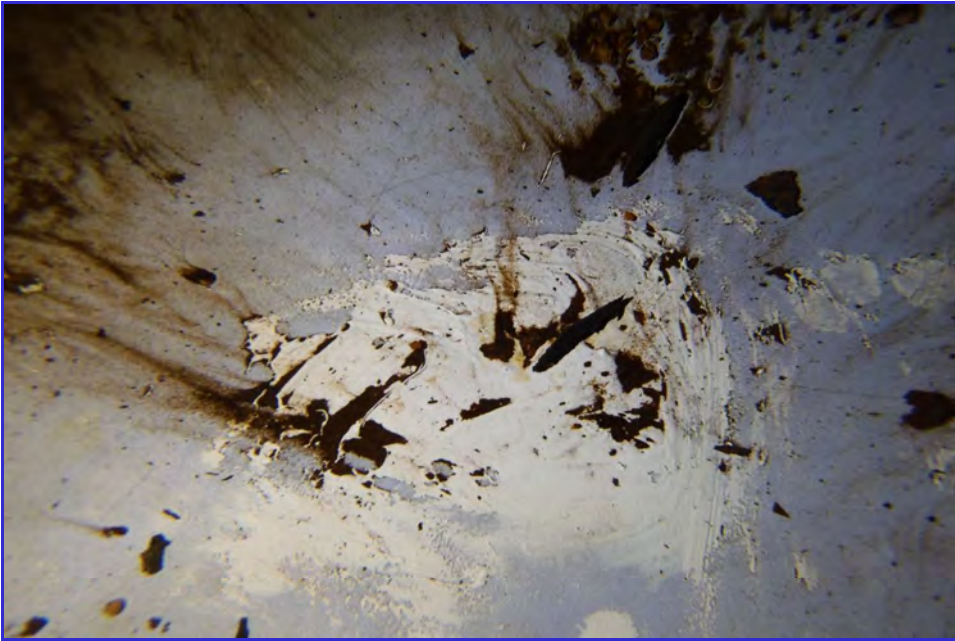
INTERIOR - CPUD - Mokelumne Hill Reservoir - Maintenance Inspection -132
