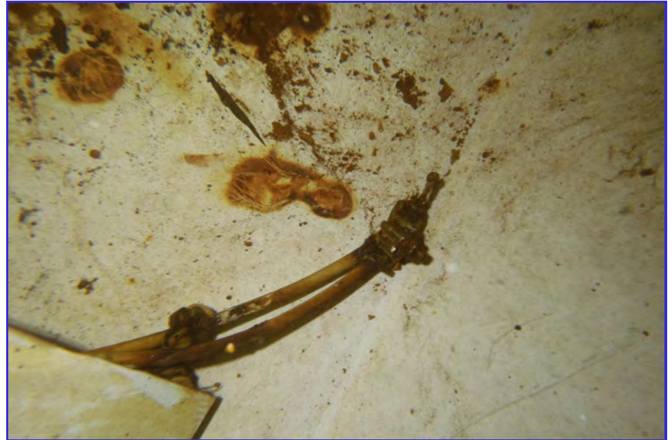
INTERIOR - CPUD - Railroad Flat Reservoir - Maintenance Inspection -117
