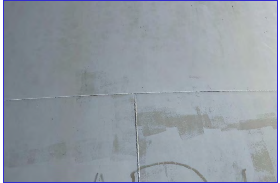
EXTERIOR - CPUD - San Andreas Reservoir - Maintenance Inspection -153
