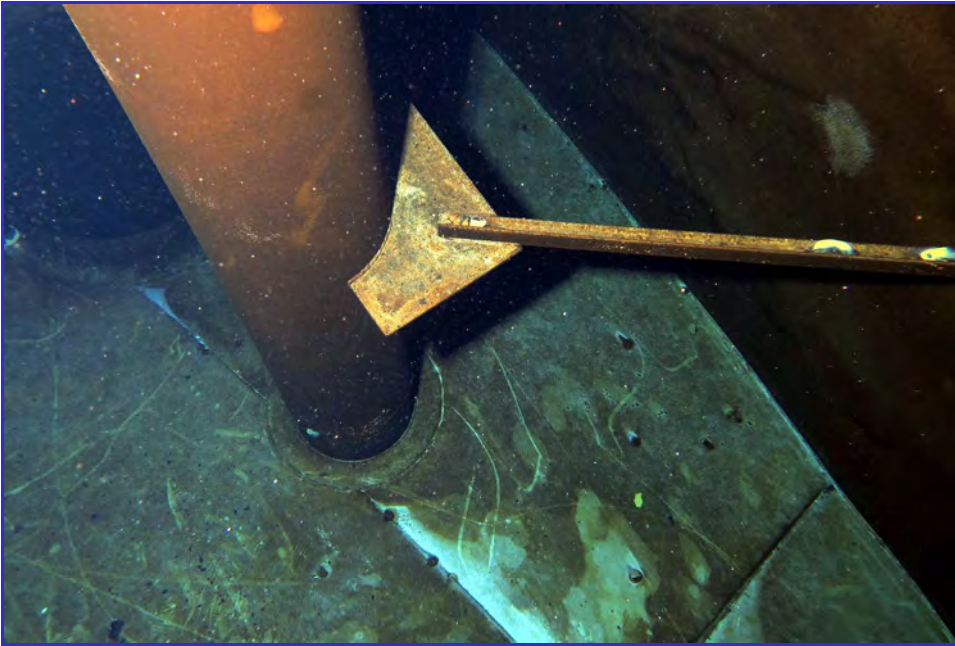
INTERIOR - Calaveras Public Utility District - Clear Well Tank - Maintenance Inspection -060
