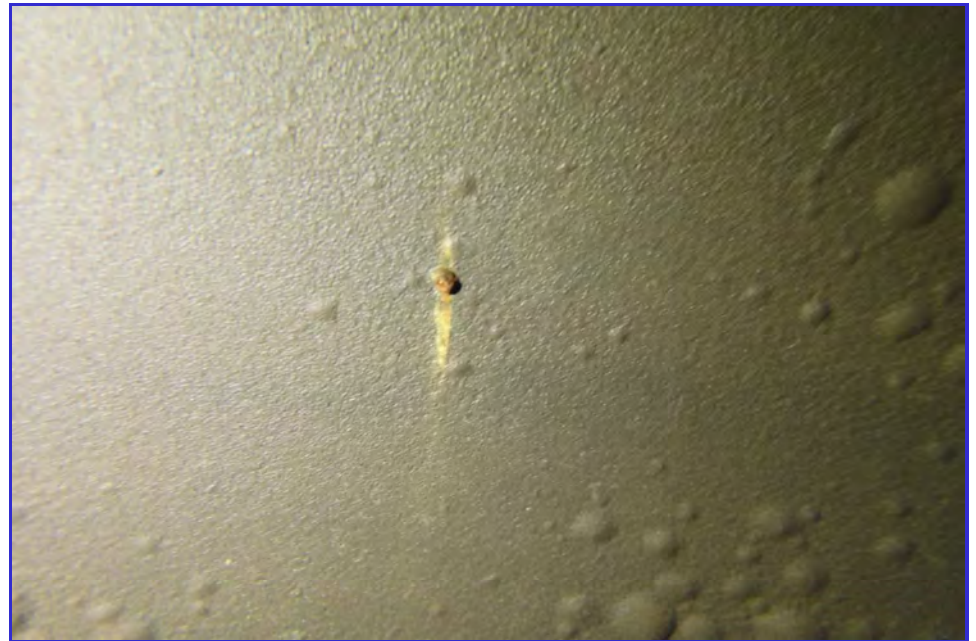
INTERIOR - CPUD - Paloma Reservoir - Maintenance Inspection -047
