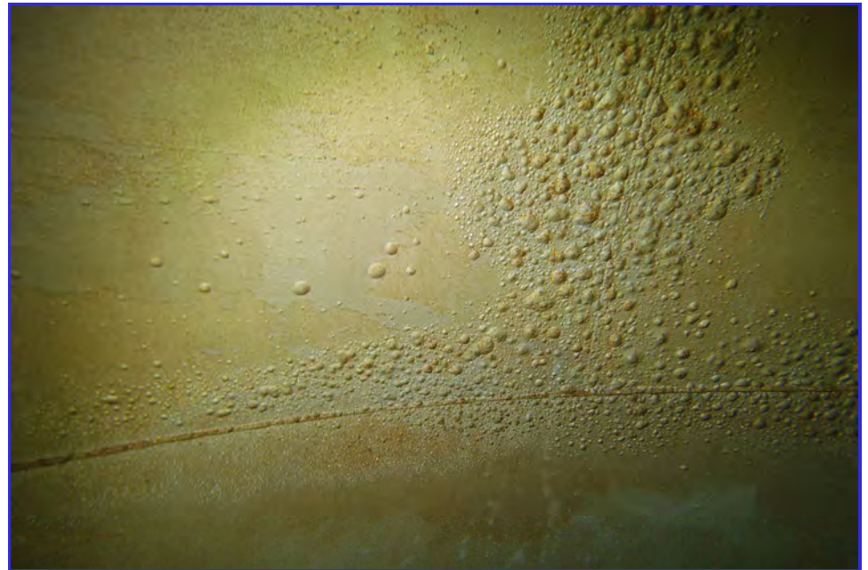
INTERIOR - CPUD - San Andaras Reservoir - Maintenance Inspection -119
