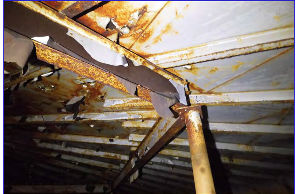
INTERIOR - CPUD - San Andaras Reservoir - Maintenance Inspection -057
