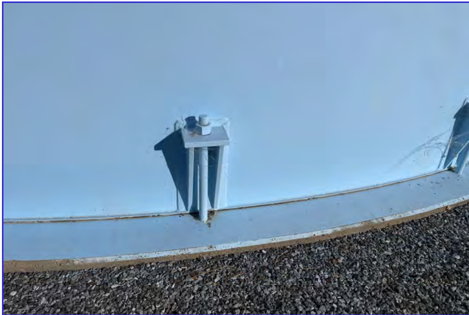
EXTERIOR - CPUD - Railroad Flat Reservoir - Maintenance Inspection -086
