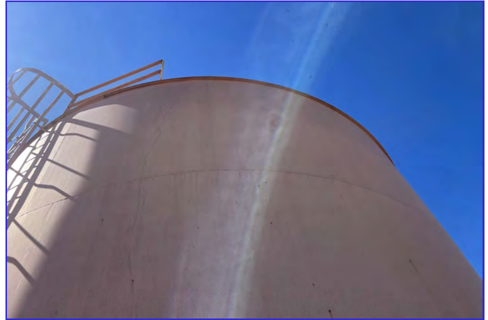
EXTERIOR - CPUD - Paloma Reservoir - Maintenance Inspection -065
