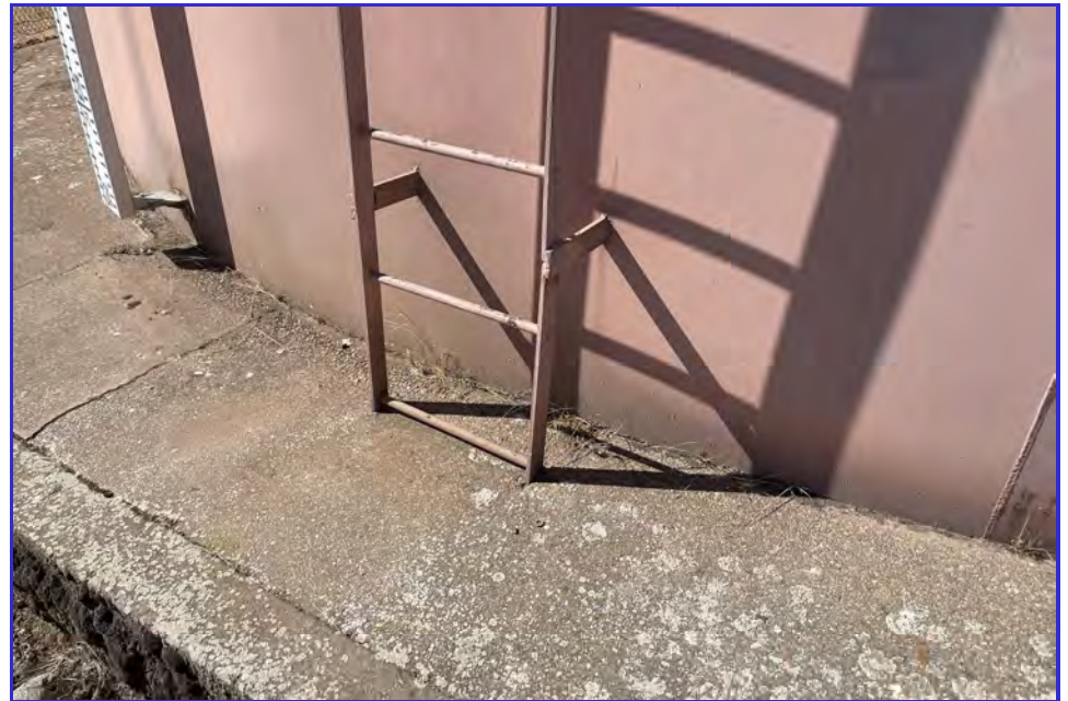
EXTERIOR - CPUD - Paloma Reservoir - Maintenance Inspection -059
