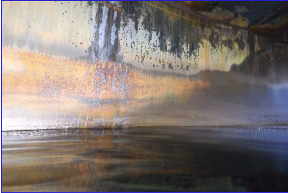
INTERIOR - CPUD - Paloma Reservoir - Maintenance Inspection -040
