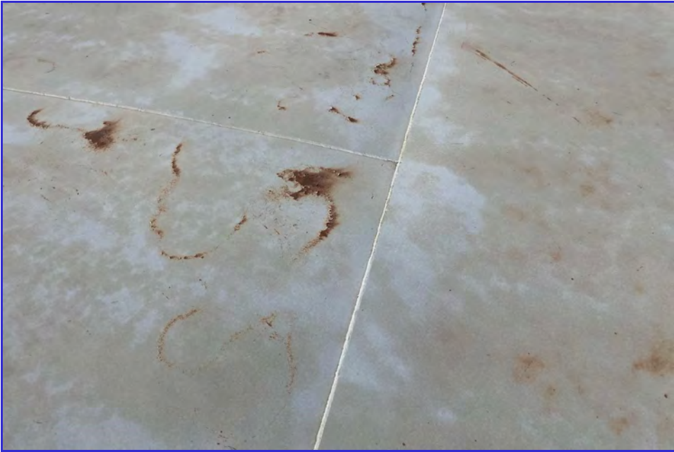
EXTERIOR - CPUD - San Andreas Reservoir - Maintenance Inspection -080
