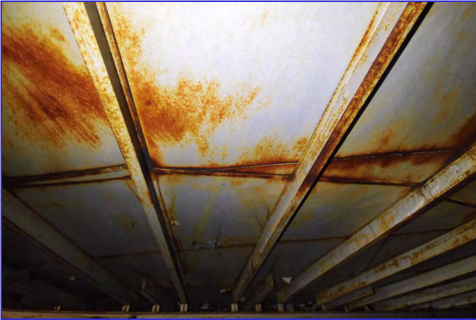
INTERIOR - CPUD - San Andaras Reservoir - Maintenance Inspection -016
