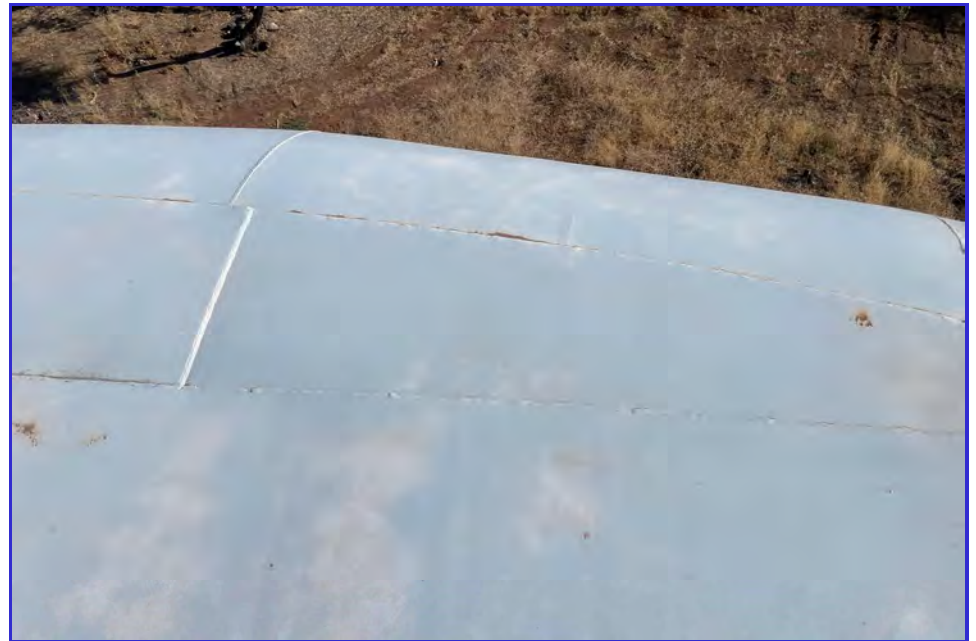
EXTERIOR - CPUD - Mokelumne Reservoir - Maintenance Inspection -003
