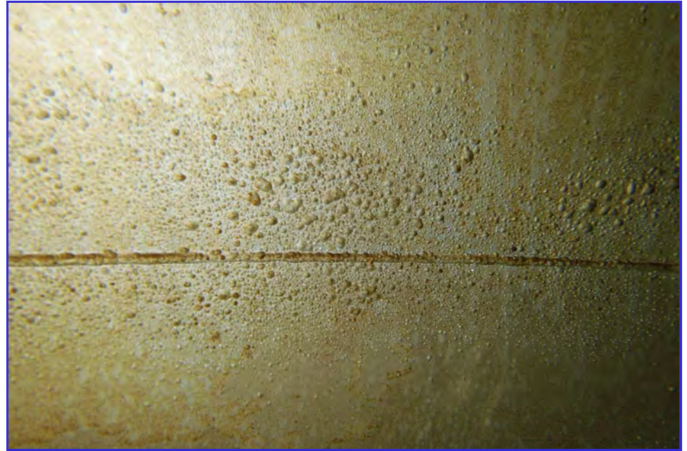
INTERIOR - CPUD - San Andaras Reservoir - Maintenance Inspection -129
