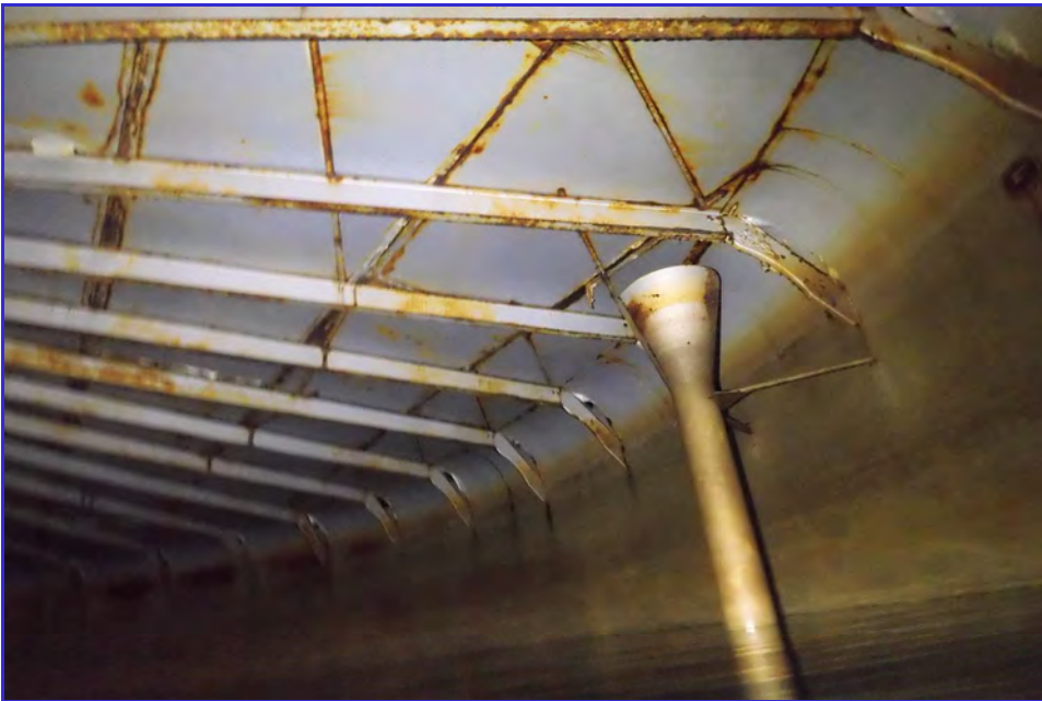
INTERIOR - CPUD - Mokelumne Hill Reservoir - Maintenance Inspection -006
