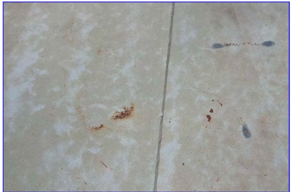
EXTERIOR - CPUD - San Andreas Reservoir - Maintenance Inspection -027
