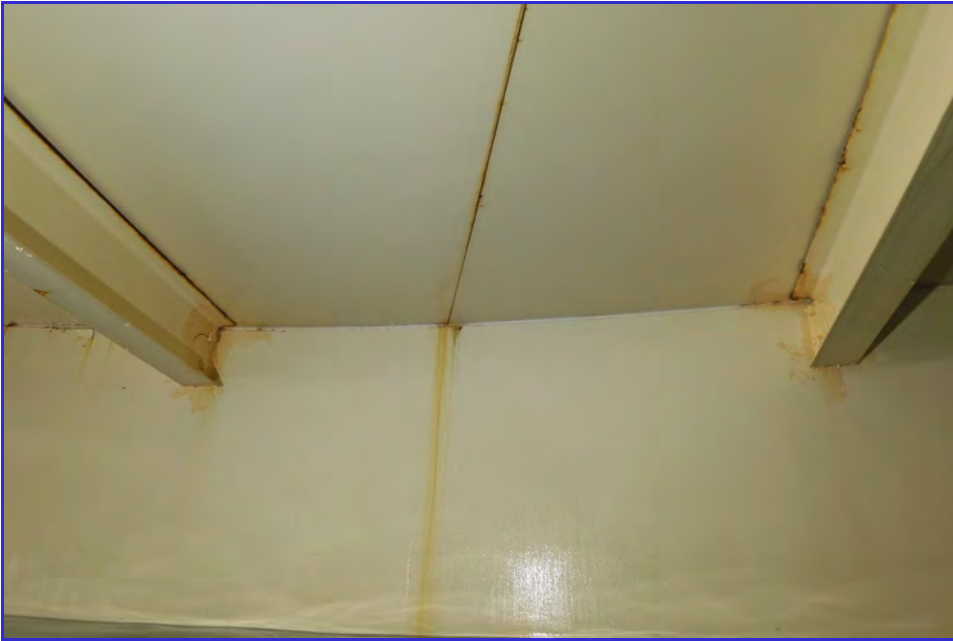
INTERIOR - CPUD - Railroad Flat Reservoir - Maintenance Inspection -012
