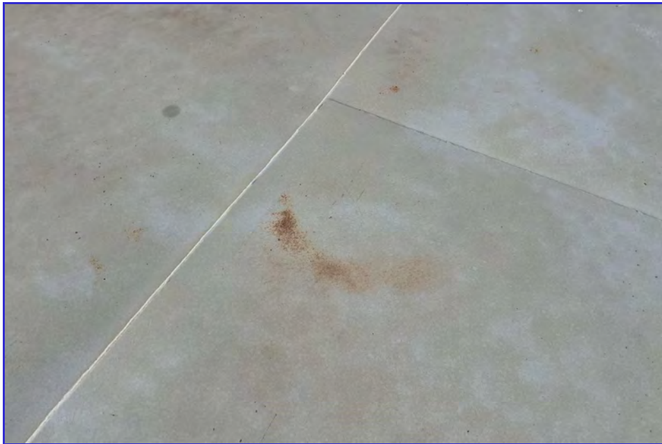
EXTERIOR - CPUD - San Andreas Reservoir - Maintenance Inspection -014
