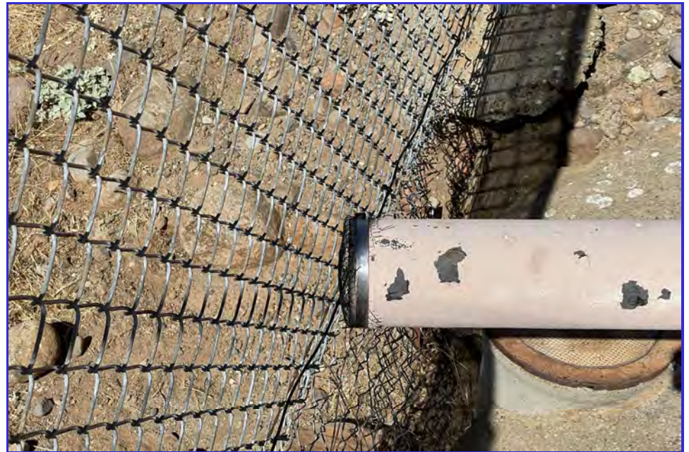
EXTERIOR - CPUD - Paloma Reservoir - Maintenance Inspection -051
