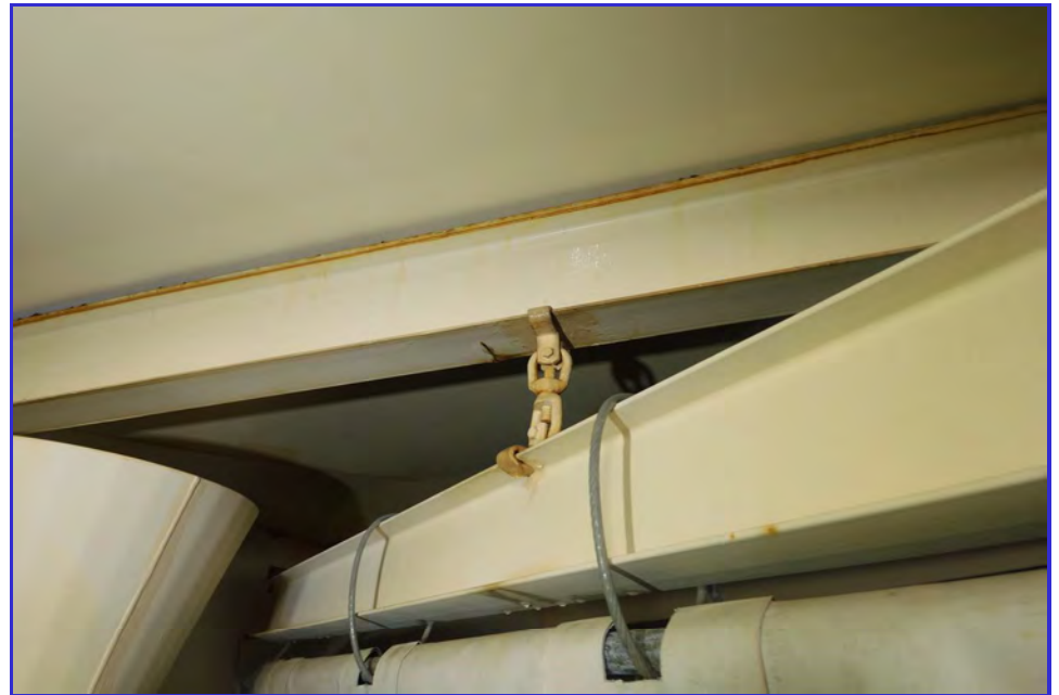
INTERIOR - CPUD - Railroad Flat Reservoir - Maintenance Inspection -015
