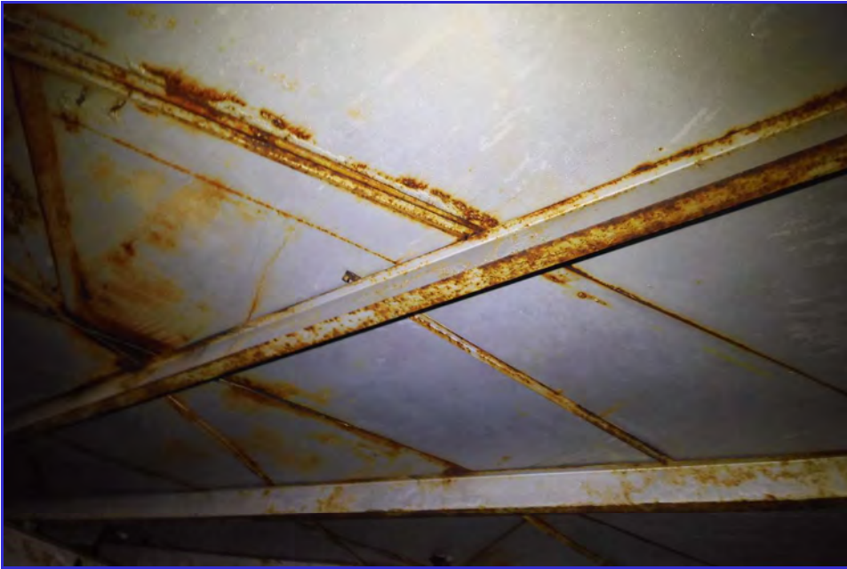
INTERIOR - CPUD - San Andaras Reservoir - Maintenance Inspection -024
