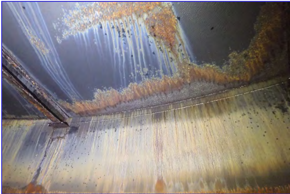
INTERIOR - CPUD - Paloma Reservoir - Maintenance Inspection -042
