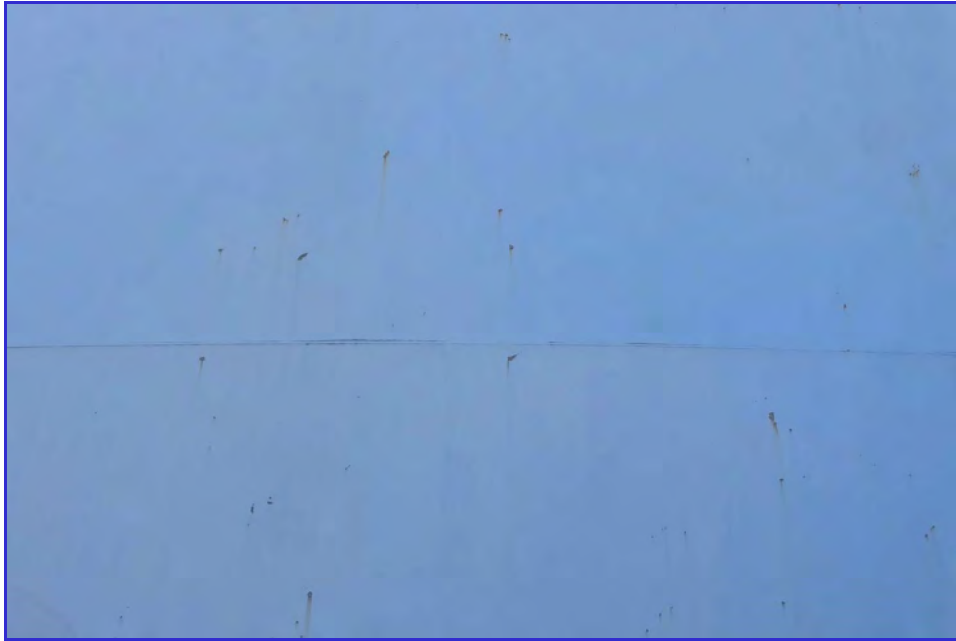
EXTERIOR - CPUD - San Andreas Reservoir - Maintenance Inspection -104
