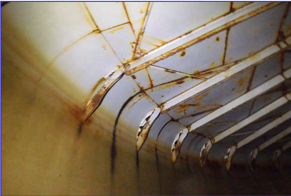
INTERIOR - CPUD - Mokelumne Hill Reservoir - Maintenance Inspection -058
