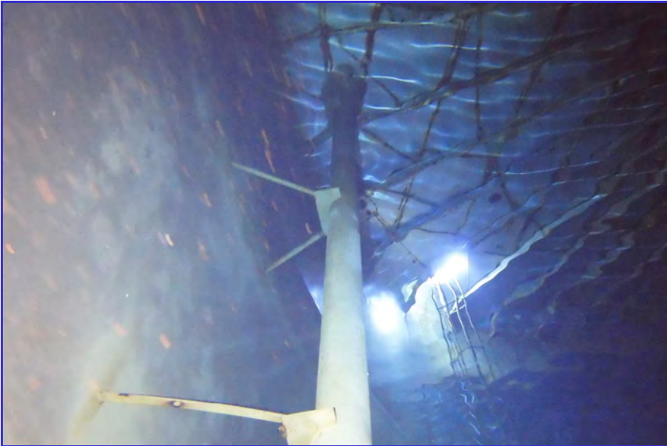
INTERIOR - CPUD - Mokelumne Hill Reservoir - Maintenance Inspection -108
