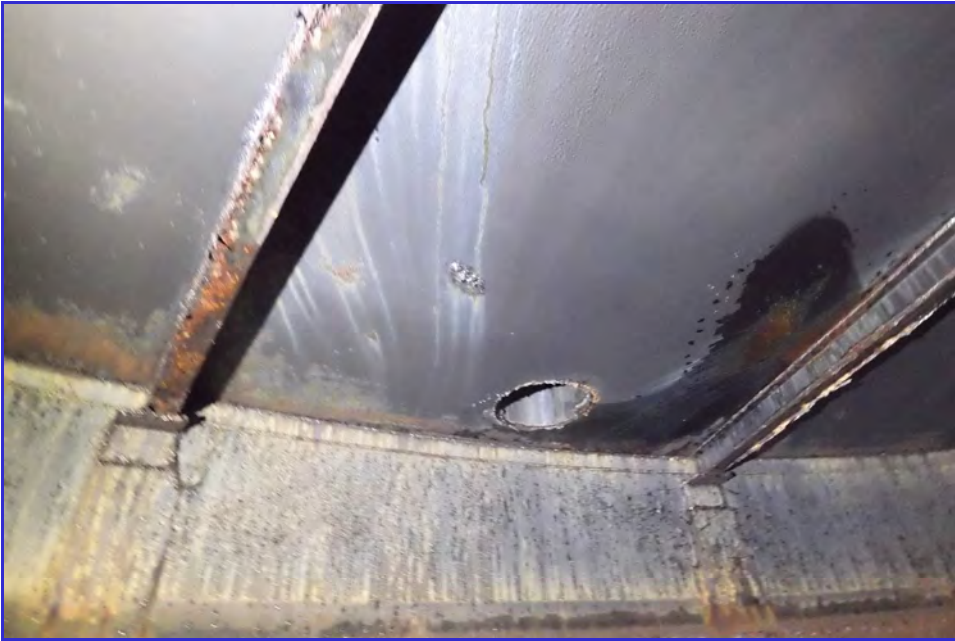
INTERIOR - CPUD - Paloma Reservoir - Maintenance Inspection -020
