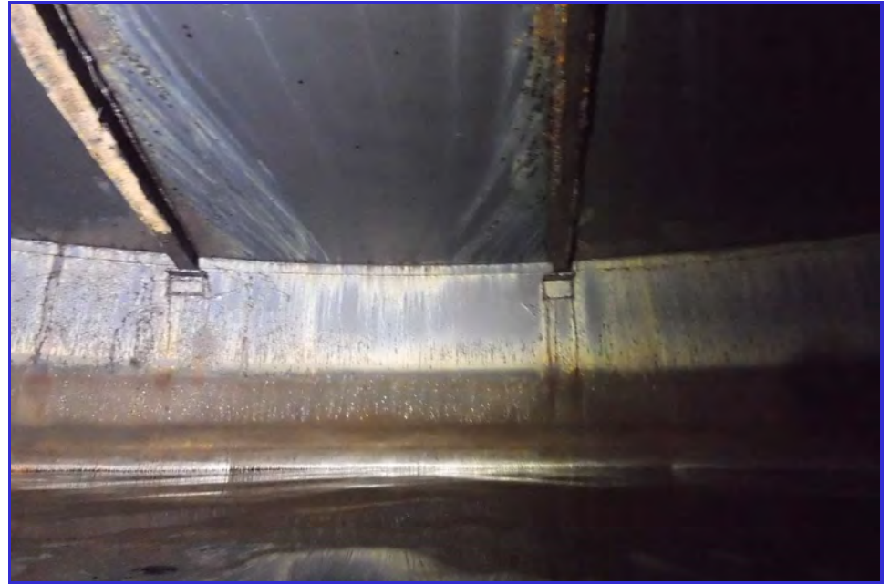
INTERIOR - CPUD - Paloma Reservoir - Maintenance Inspection -029
