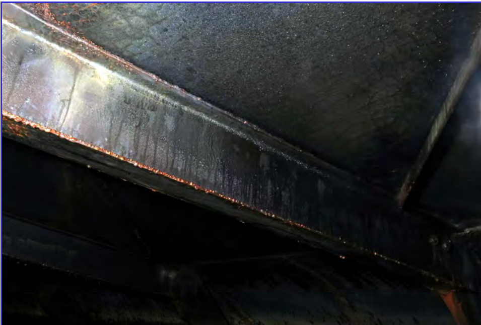
INTERIOR - Calaveras Public Utility District - Clear Well Tank - Maintenance Inspection -002
