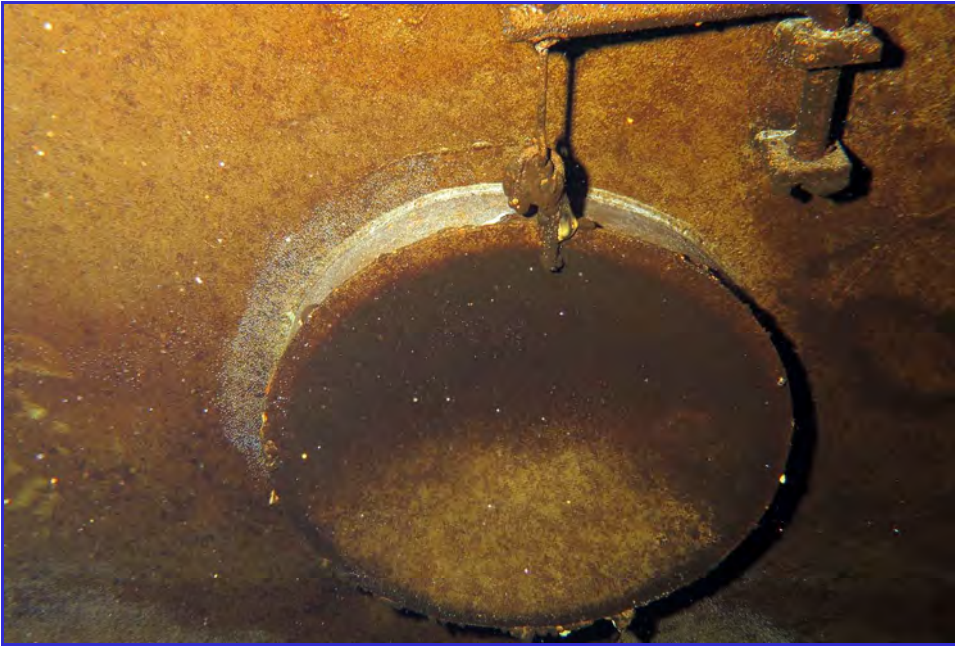
INTERIOR - Calaveras Public Utility District - Clear Well Tank - Maintenance Inspection -064
