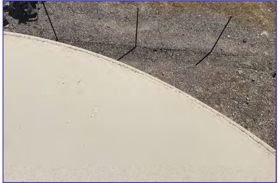
EXTERIOR - CPUD - Golden Hills - Maintenance Inspection -005
