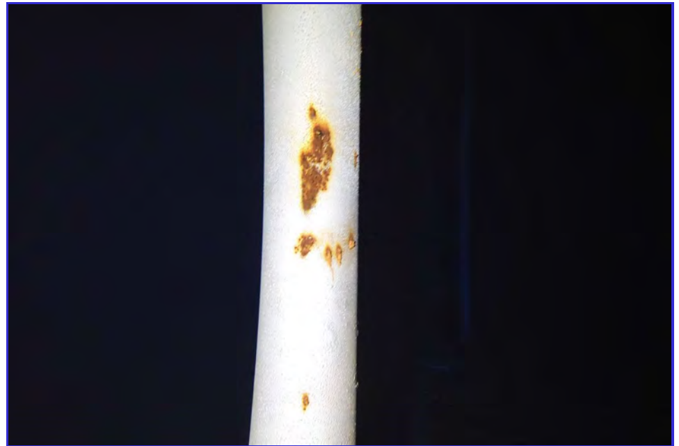
INTERIOR - CPUD - San Andaras Reservoir - Maintenance Inspection -147
