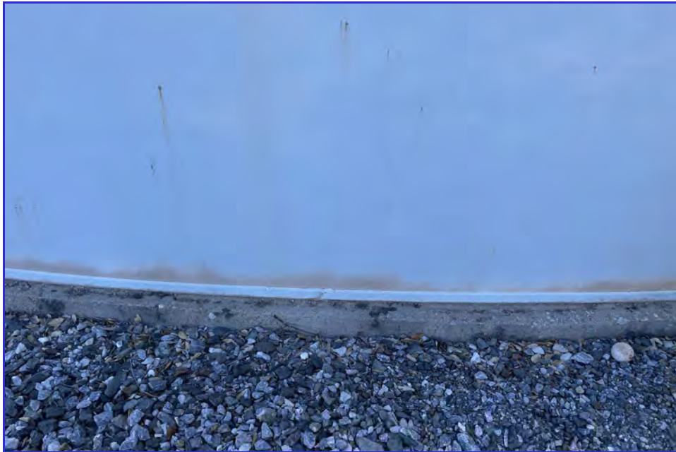
EXTERIOR - CPUD - Mokelumne Reservoir - Maintenance Inspection -116
