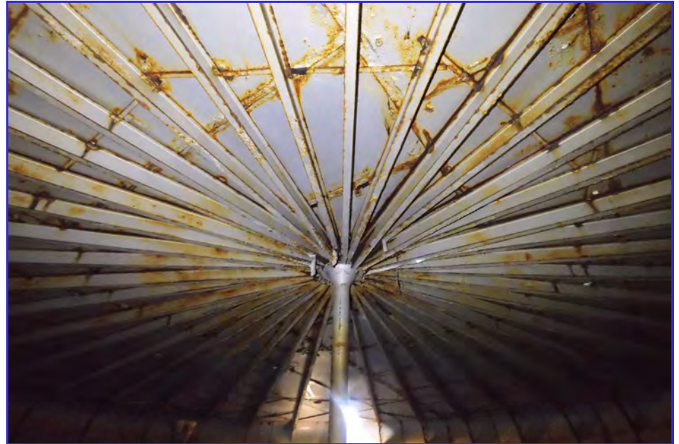
INTERIOR - CPUD - Mokelumne Hill Reservoir - Maintenance Inspection -033
