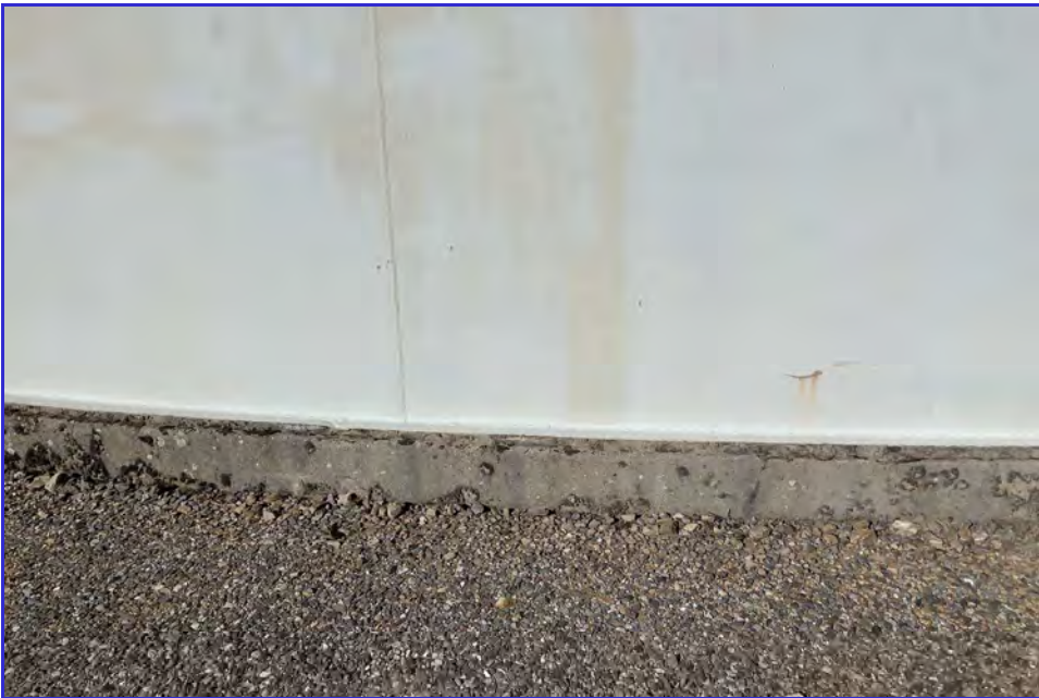
EXTERIOR - CPUD - San Andreas Reservoir - Maintenance Inspection -130
