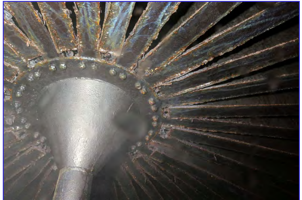
INTERIOR - Calaveras Public Utility District - Clear Well Tank - Maintenance Inspection -019
