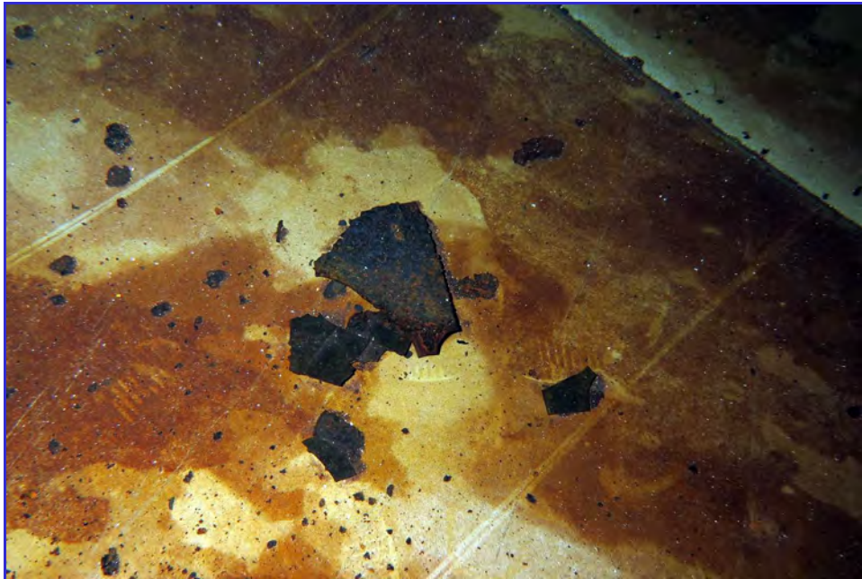
INTERIOR - Calaveras Public Utility District - Clear Well Tank - Maintenance Inspection -104
