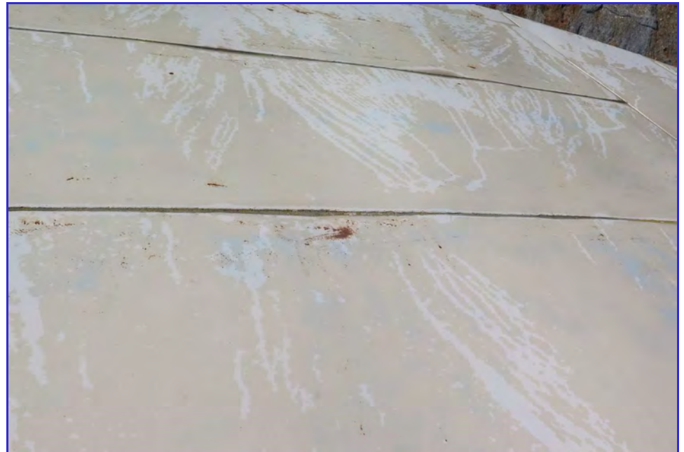
EXTERIOR - Calaveras Public Utility District - Clear Well Tank - Maintenance Inspection -043
