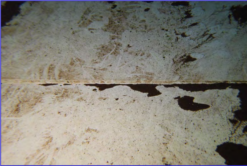
INTERIOR - CPUD - Railroad Flat Reservoir - Maintenance Inspection -164
