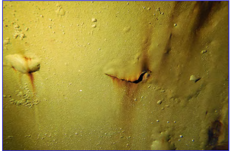
INTERIOR - CPUD - San Andaras Reservoir - Maintenance Inspection -105
