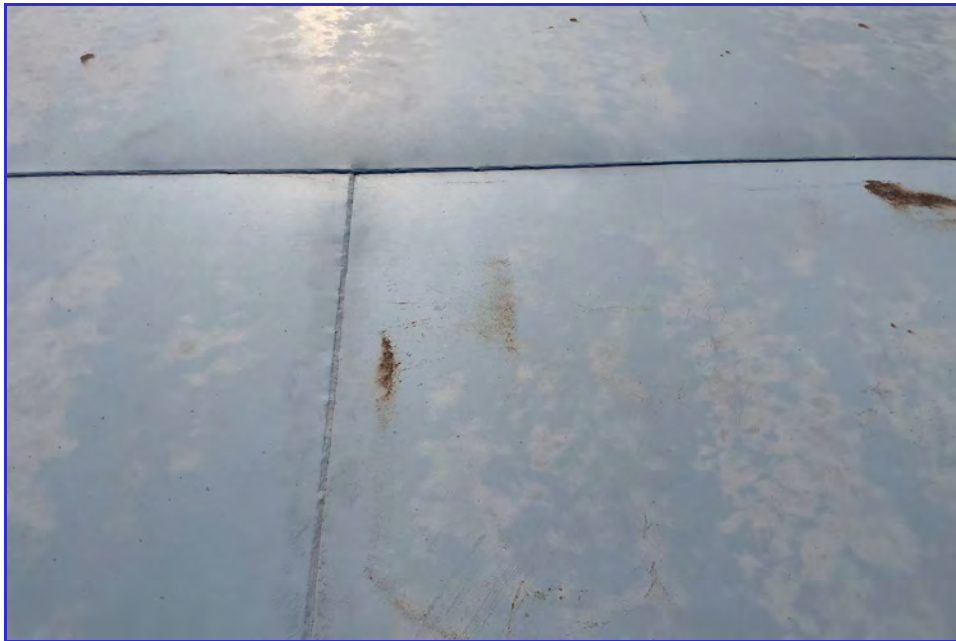
EXTERIOR - CPUD - Mokelumne Reservoir - Maintenance Inspection -038
