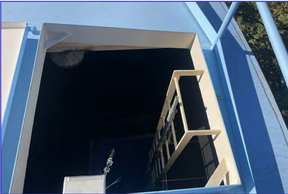
EXTERIOR - CPUD - Railroad Flat Reservoir - Maintenance Inspection -006
