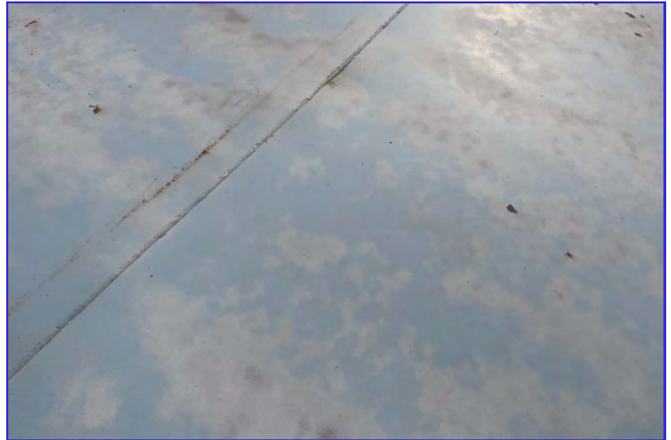
EXTERIOR - CPUD - Mokelumne Reservoir - Maintenance Inspection -041
