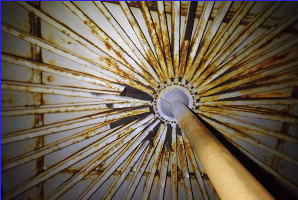
INTERIOR - CPUD - Mokelumne Hill Reservoir - Maintenance Inspection -048
