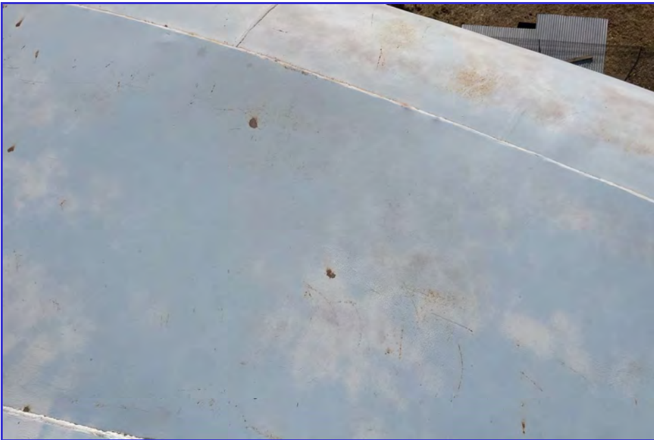
EXTERIOR - CPUD - Mokelumne Reservoir - Maintenance Inspection -046
