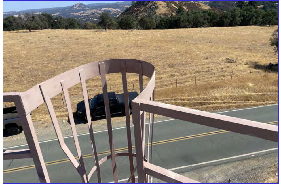
EXTERIOR - CPUD - Paloma Reservoir - Maintenance Inspection -001
