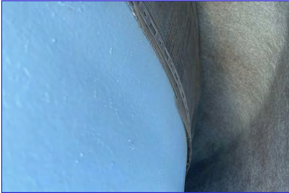
EXTERIOR - CPUD - Railroad Flat Reservoir - Maintenance Inspection -028
