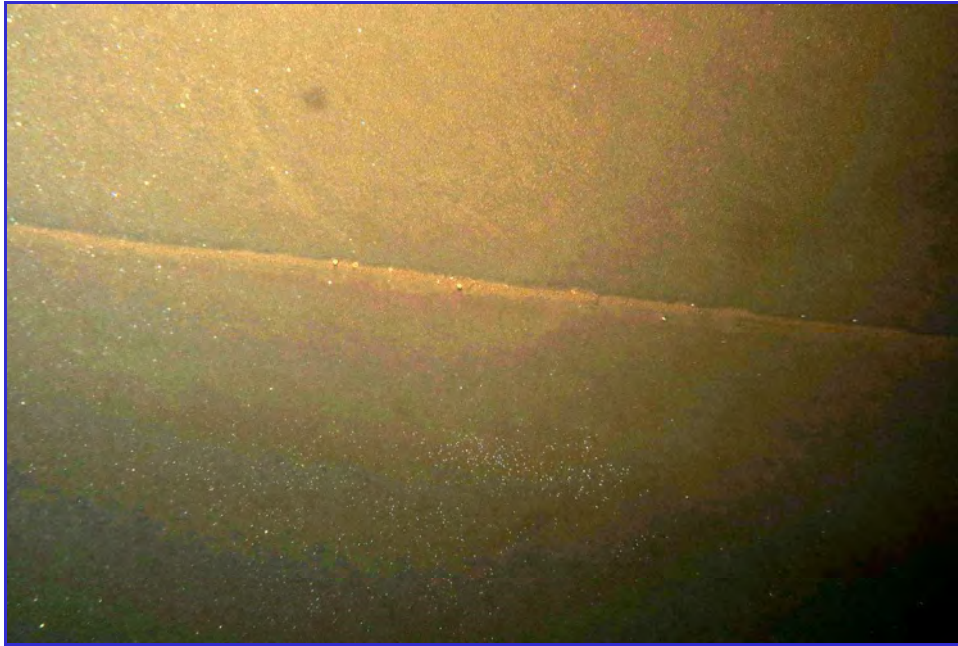
INTERIOR - Calaveras Public Utility District - Clear Well Tank - Maintenance Inspection -096
