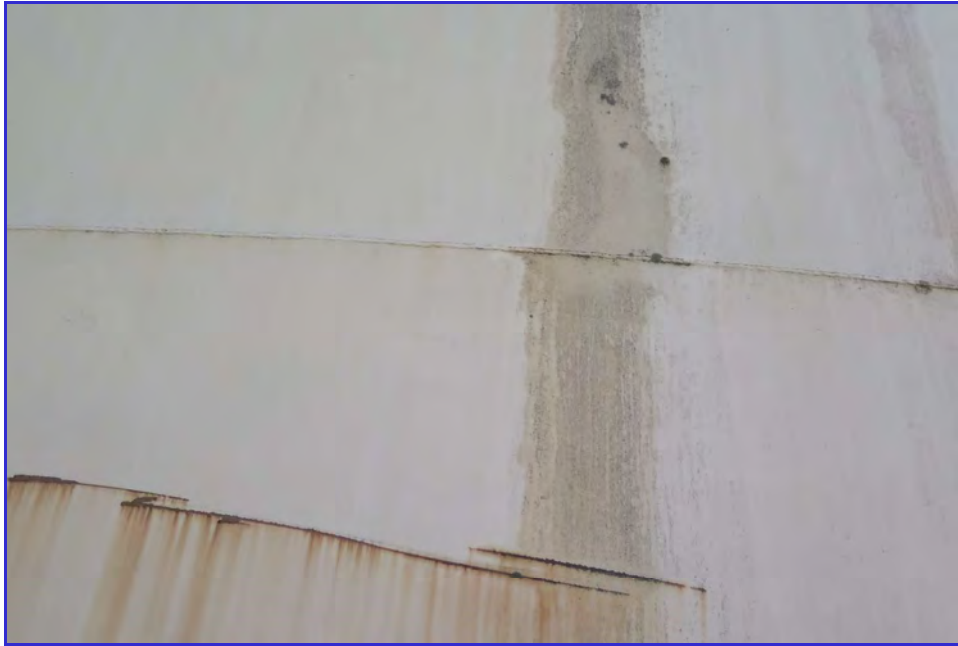
EXTERIOR - Calaveras Public Utility District - Clear Well Tank - Maintenance Inspection -092
