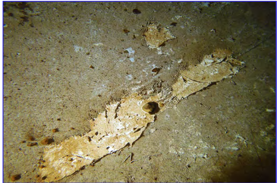
INTERIOR - CPUD - Mokelumne Hill Reservoir - Maintenance Inspection -155
