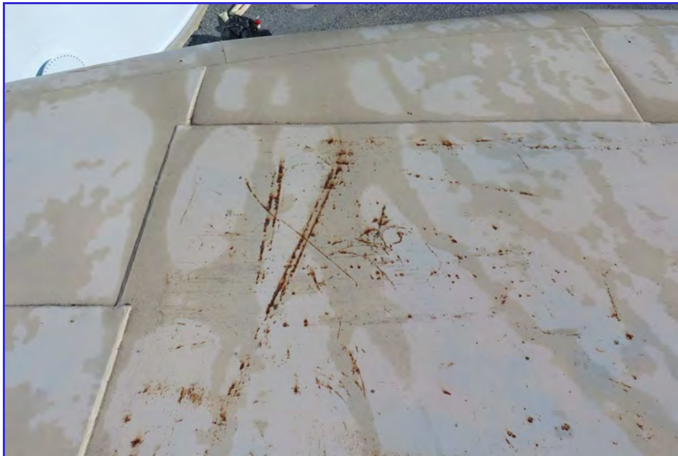
EXTERIOR - Calaveras Public Utility District - Clear Well Tank - Maintenance Inspection -010
