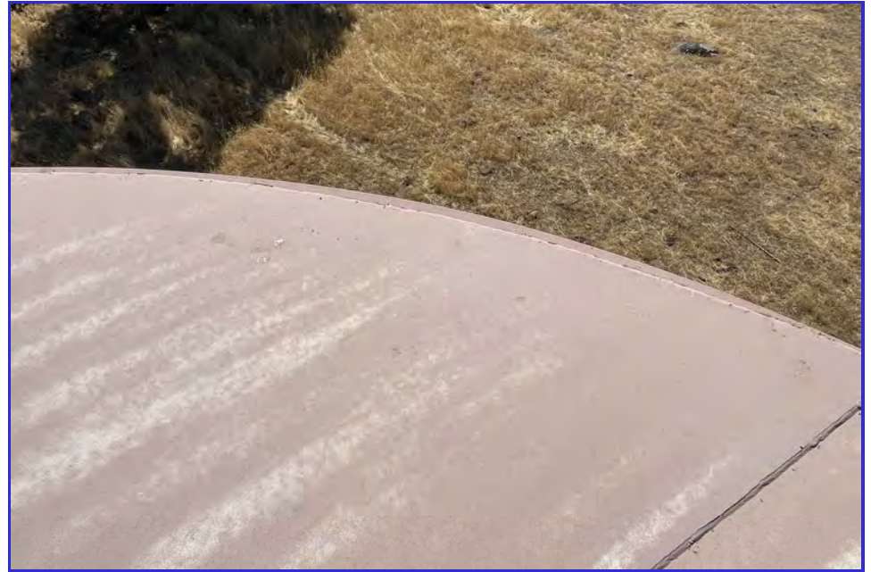
EXTERIOR - CPUD - Paloma Reservoir - Maintenance Inspection -025
