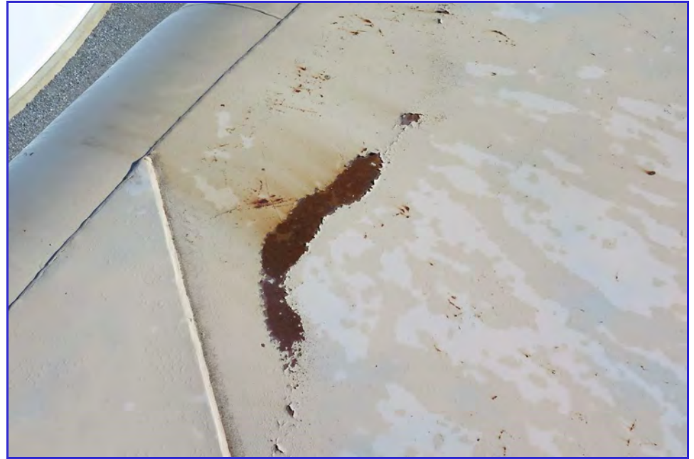
EXTERIOR - Calaveras Public Utility District - Clear Well Tank - Maintenance Inspection -013
