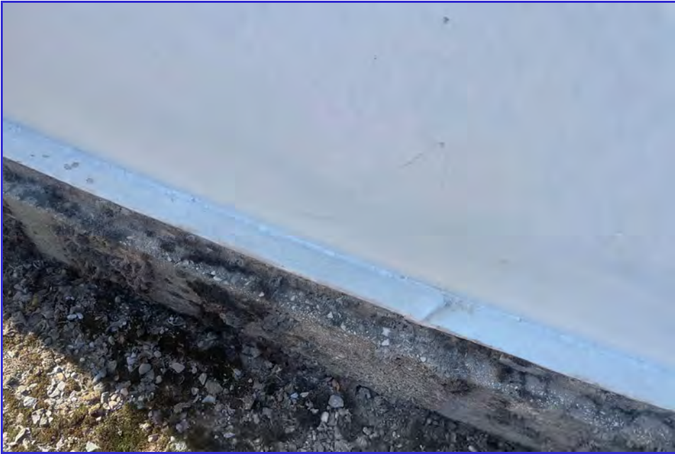
EXTERIOR - CPUD - San Andreas Reservoir - Maintenance Inspection -188
