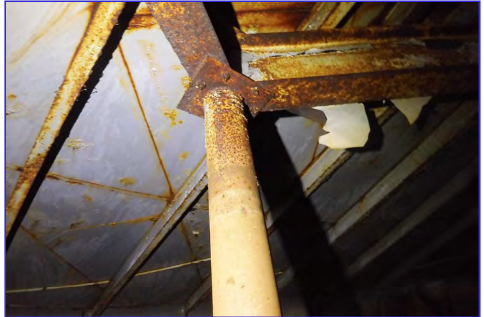
INTERIOR - CPUD - San Andaras Reservoir - Maintenance Inspection -061
