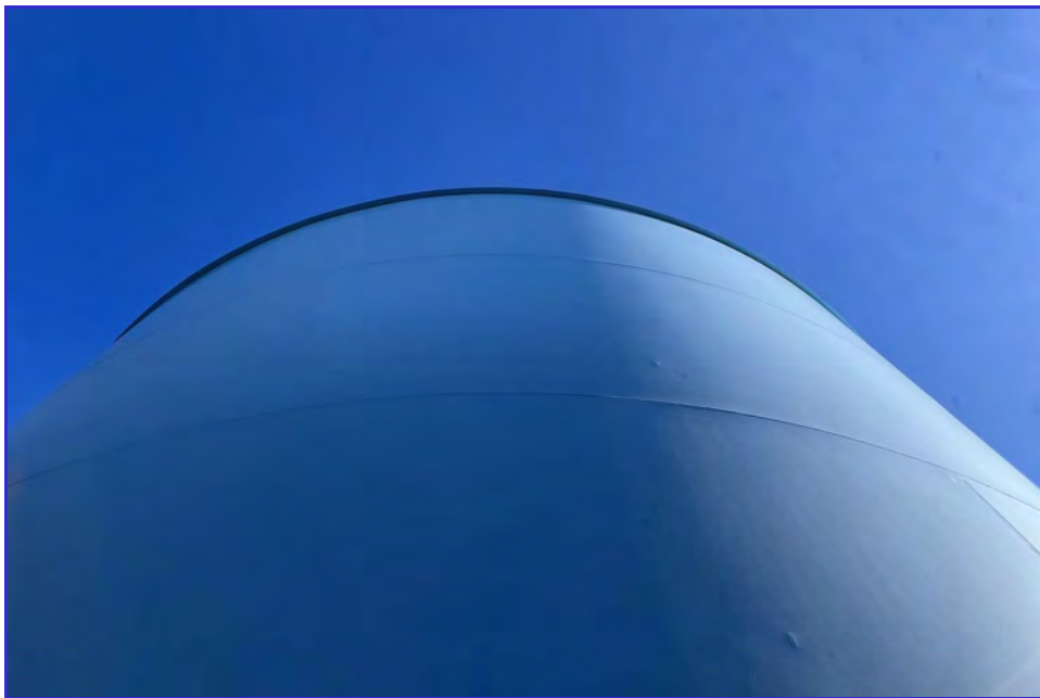
EXTERIOR - CPUD - Railroad Flat Reservoir - Maintenance Inspection -082
