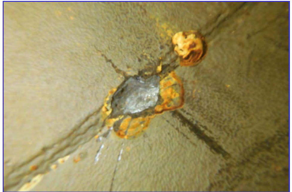
INTERIOR - CPUD - Golden Hills - Maintenance Inspection -119
