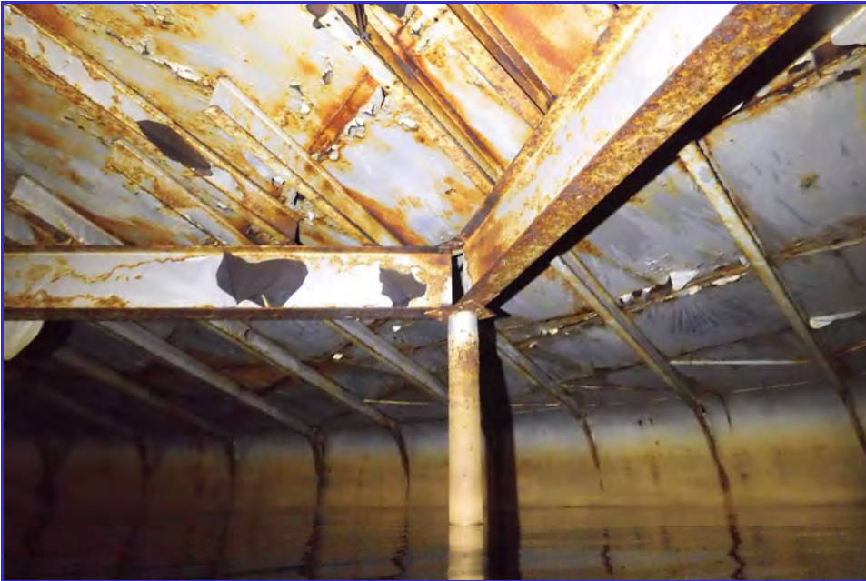
INTERIOR - CPUD - San Andaras Reservoir - Maintenance Inspection -072
