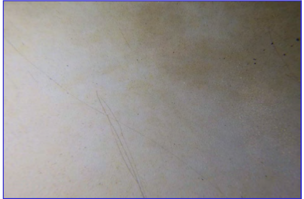
INTERIOR - CPUD - Mokelumne Hill Reservoir - Maintenance Inspection -133
