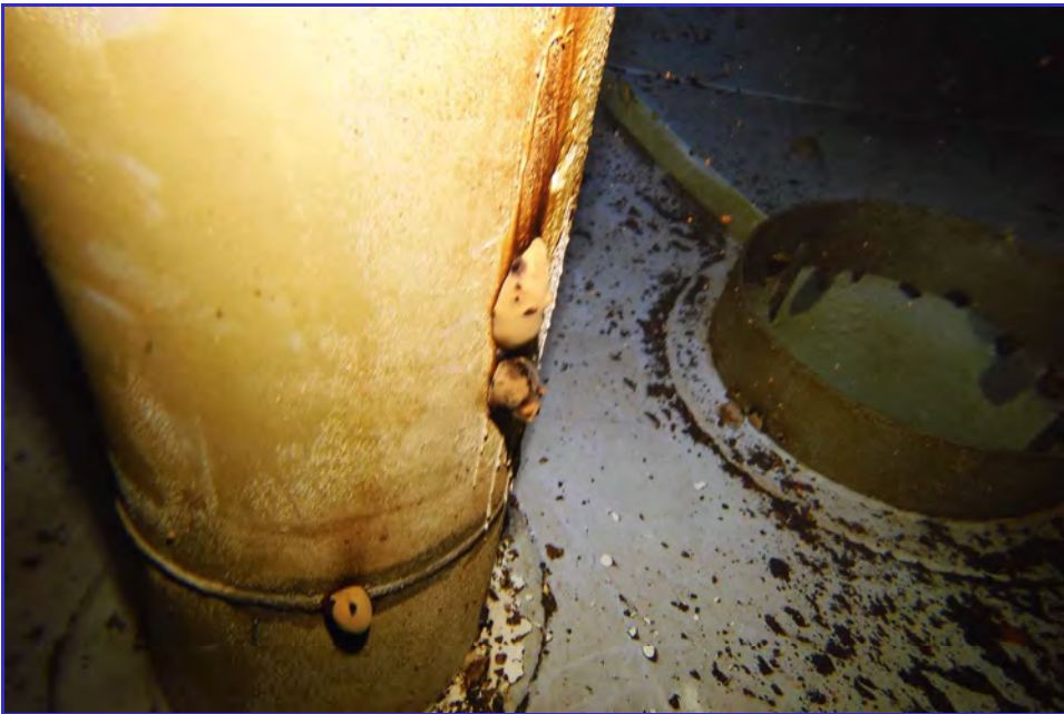
INTERIOR - CPUD - Mokelumne Hill Reservoir - Maintenance Inspection -118
