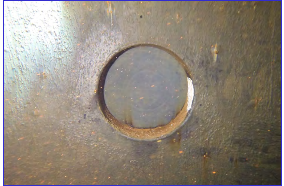
INTERIOR - CPUD - Paloma Reservoir - Maintenance Inspection -141
