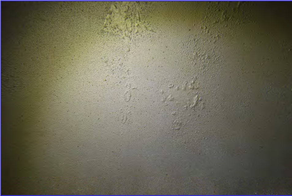
INTERIOR - CPUD - San Andaras Reservoir - Maintenance Inspection -112
