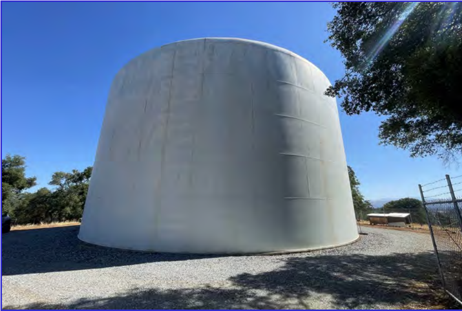
EXTERIOR - CPUD - Mokelumne Reservoir - Maintenance Inspection
