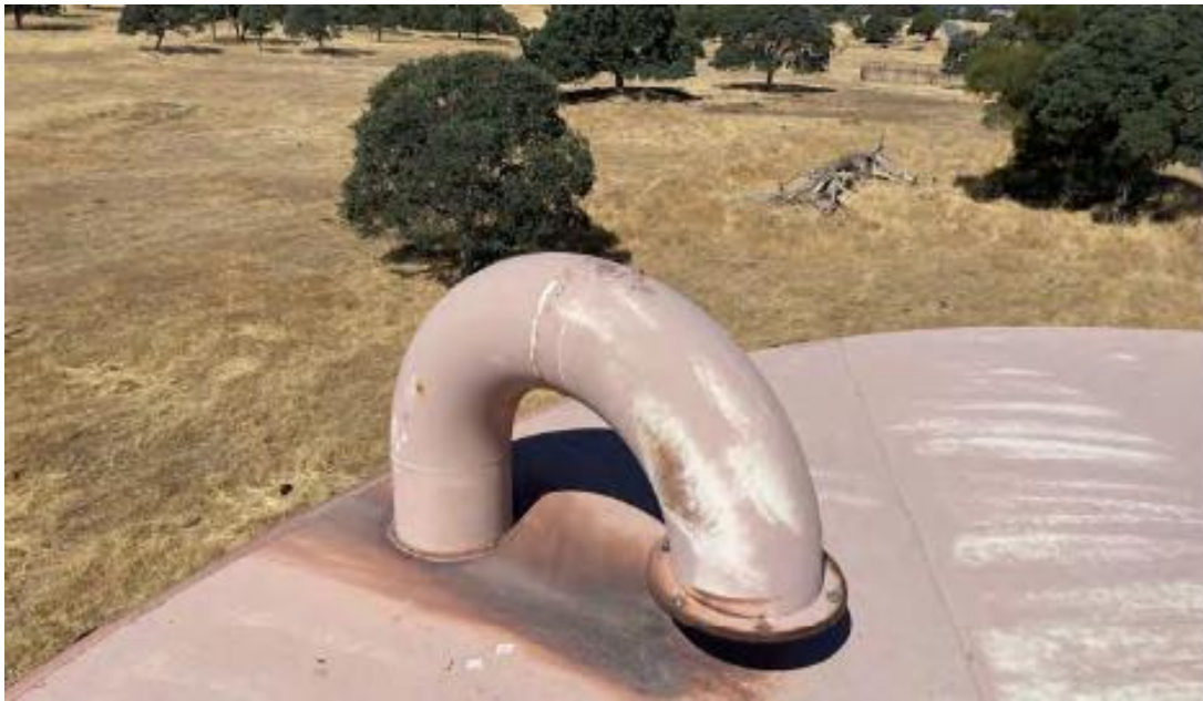
Figure 9-9. Example of Exterior Paloma Tank Roof
