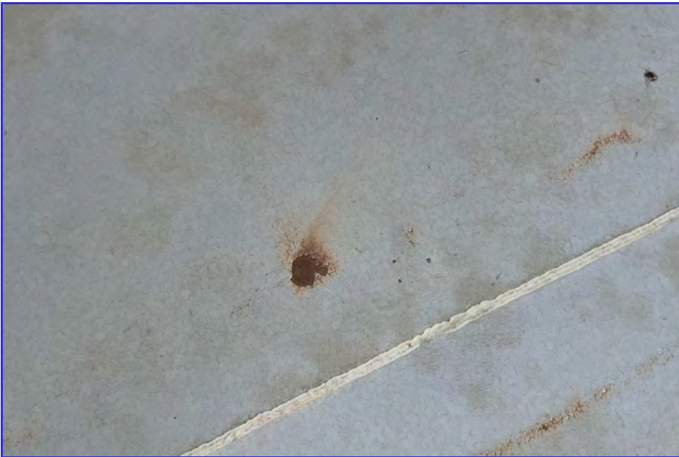
EXTERIOR - CPUD - San Andreas Reservoir - Maintenance Inspection -034
