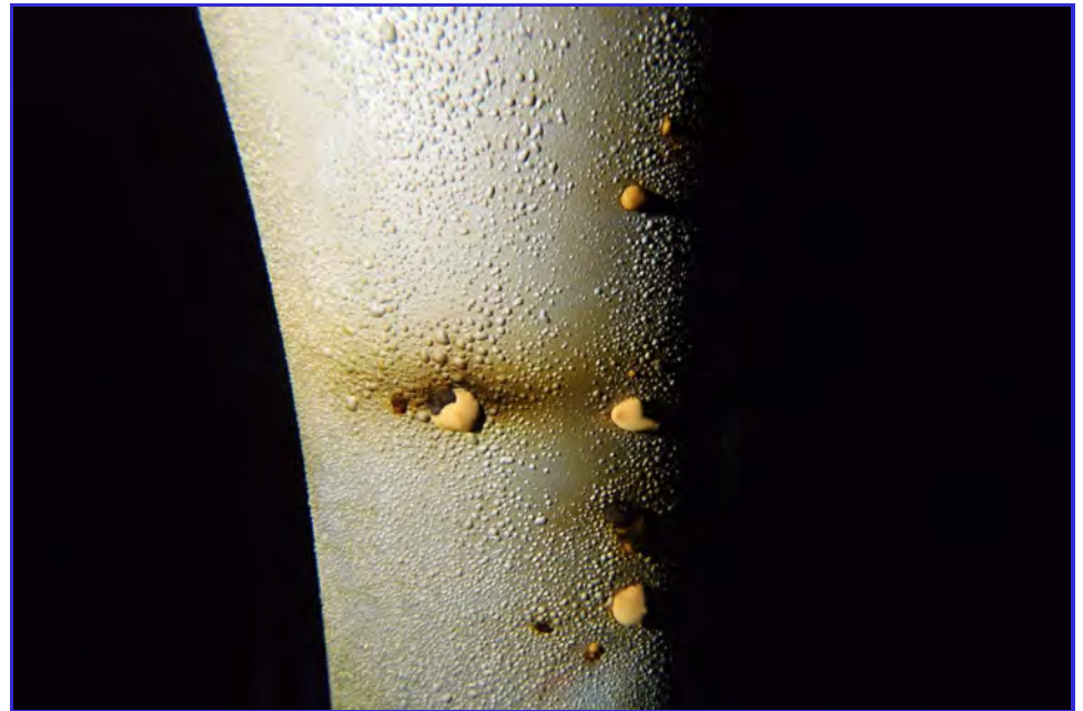
INTERIOR - CPUD - San Andaras Reservoir - Maintenance Inspection -151
