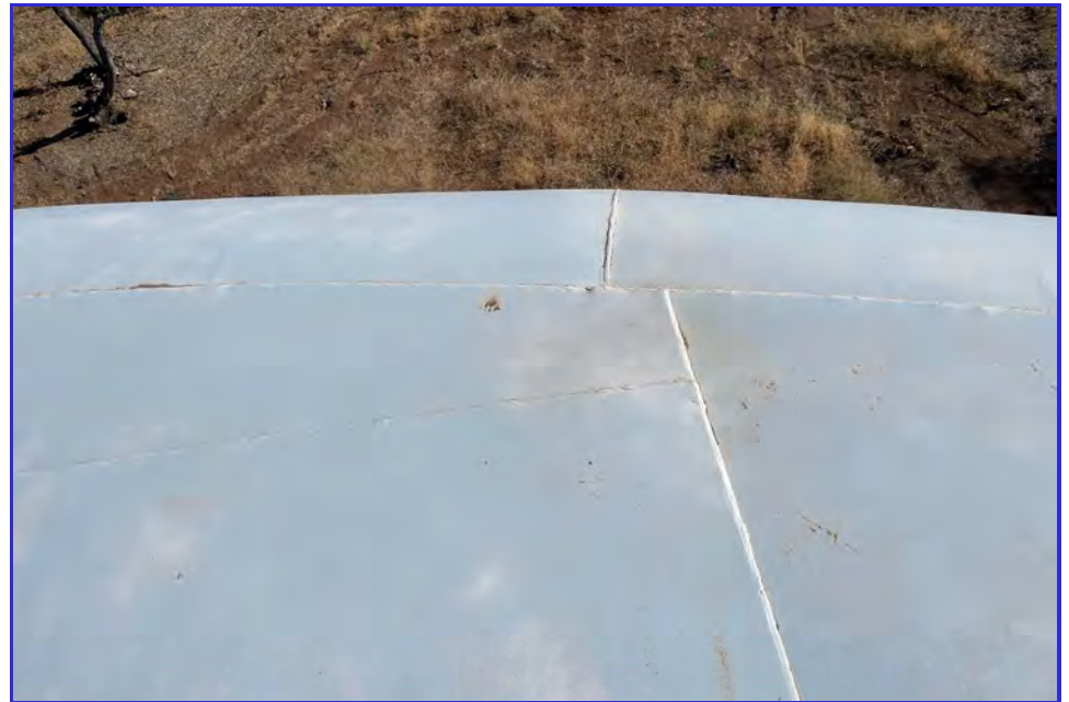
EXTERIOR - CPUD - Mokelumne Reservoir - Maintenance Inspection -047
