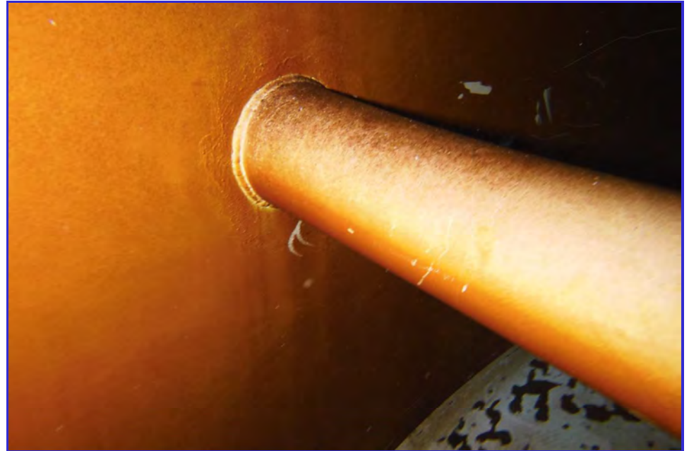
INTERIOR - CPUD - Railroad Flat Reservoir - Maintenance Inspection -169
