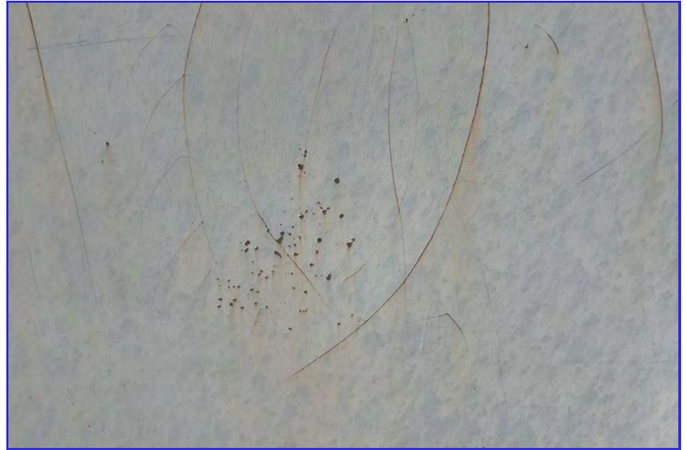
EXTERIOR - CPUD - San Andreas Reservoir - Maintenance Inspection -129
