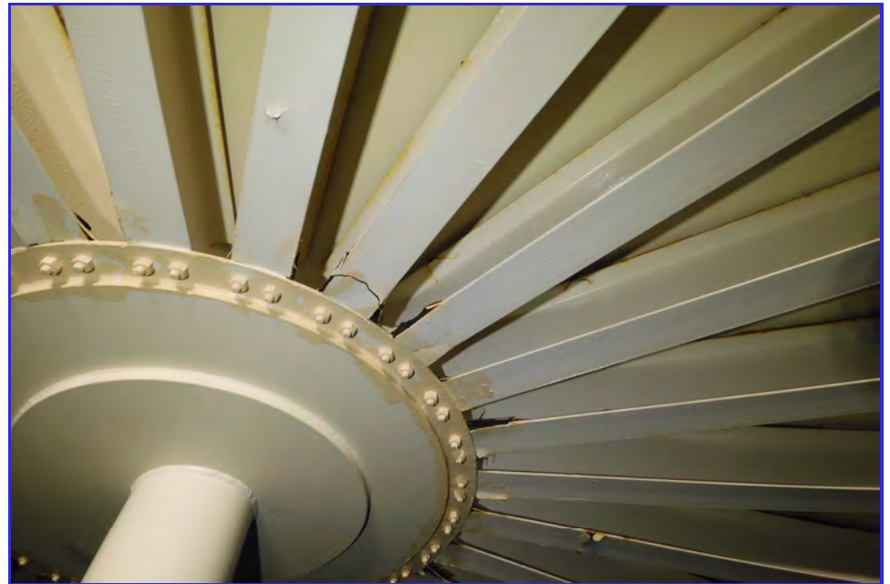
INTERIOR - CPUD - Railroad Flat Reservoir - Maintenance Inspection -035
