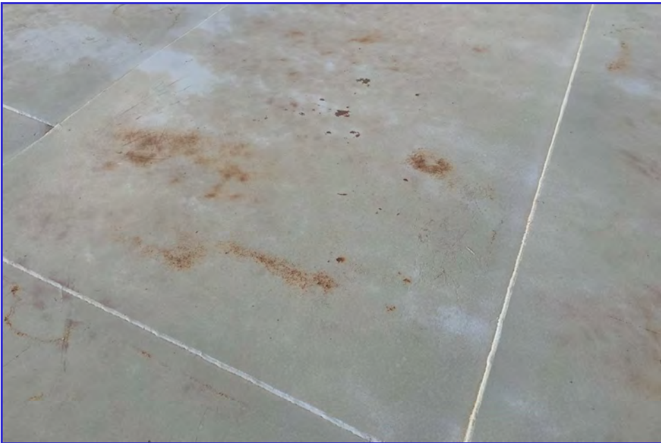
EXTERIOR - CPUD - San Andreas Reservoir - Maintenance Inspection -078
