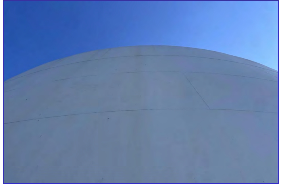
EXTERIOR - CPUD - San Andreas Reservoir - Maintenance Inspection -181
