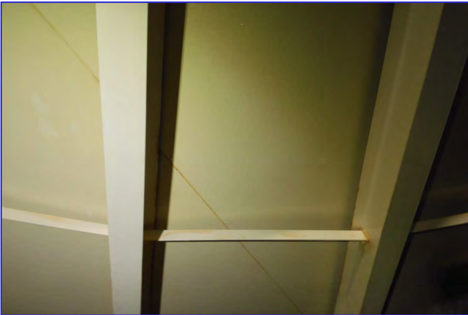
INTERIOR - CPUD - Railroad Flat Reservoir - Maintenance Inspection -046
