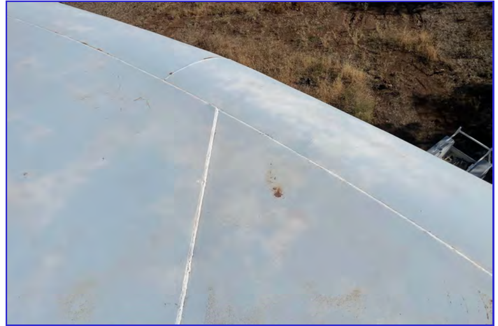
EXTERIOR - CPUD - Mokelumne Reservoir - Maintenance Inspection -049
