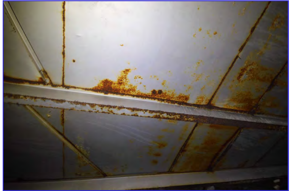
INTERIOR - CPUD - San Andreas Reservoir - Maintenance Inspection -045
