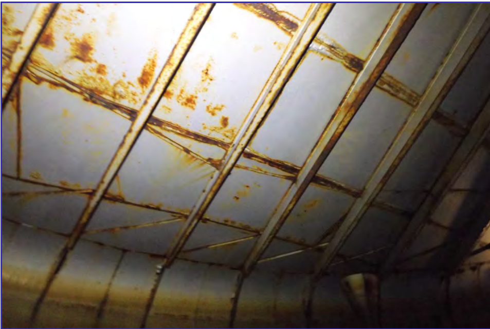
INTERIOR - CPUD - Mokelumne Hill Reservoir - Maintenance Inspection -018
