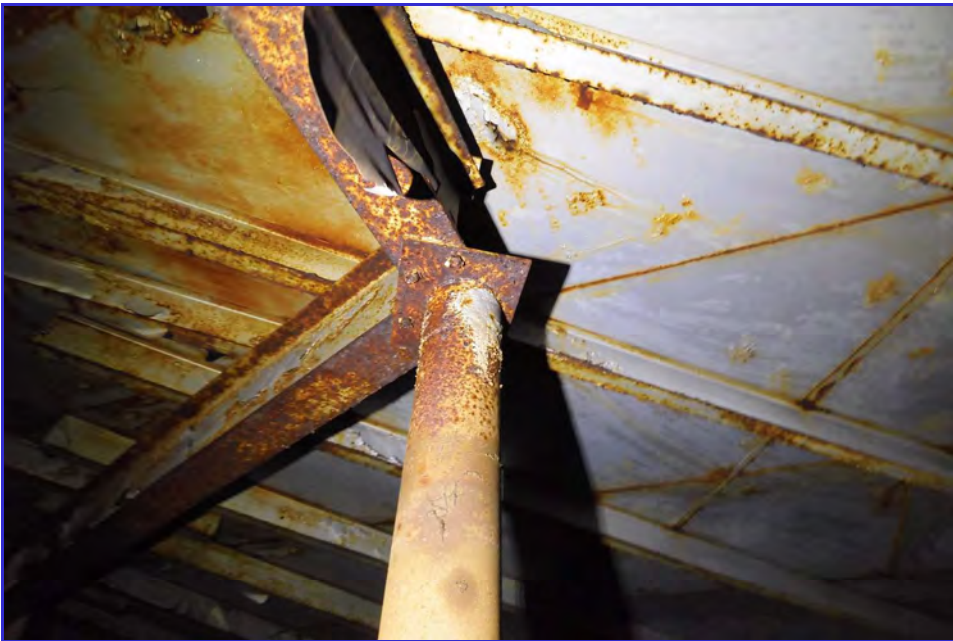
INTERIOR - CPUD - San Andaras Reservoir - Maintenance Inspection -058
