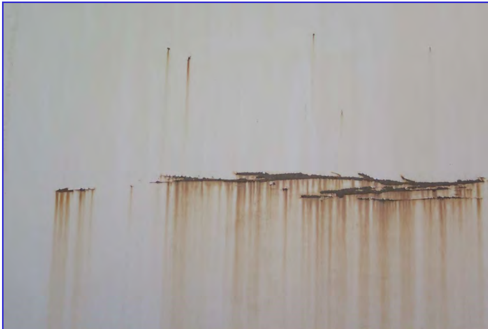
EXTERIOR - Calaveras Public Utility District - Clear Well Tank - Maintenance Inspection -098
