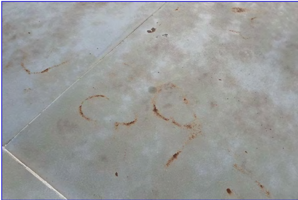
EXTERIOR - CPUD - San Andreas Reservoir - Maintenance Inspection -018
