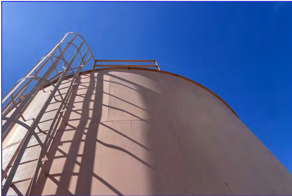
EXTERIOR - CPUD - Paloma Reservoir - Maintenance Inspection -062
