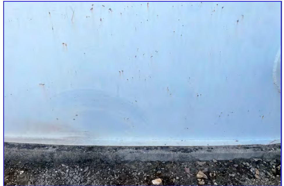
EXTERIOR - CPUD - San Andreas Reservoir - Maintenance Inspection -103
