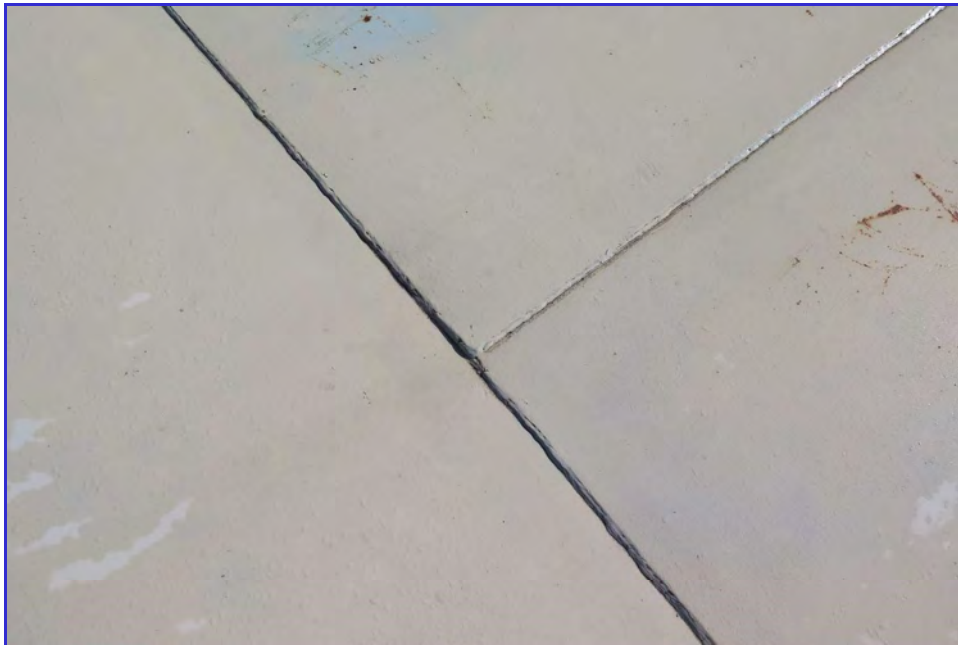
EXTERIOR - Calaveras Public Utility District - Clear Well Tank - Maintenance Inspection -046
