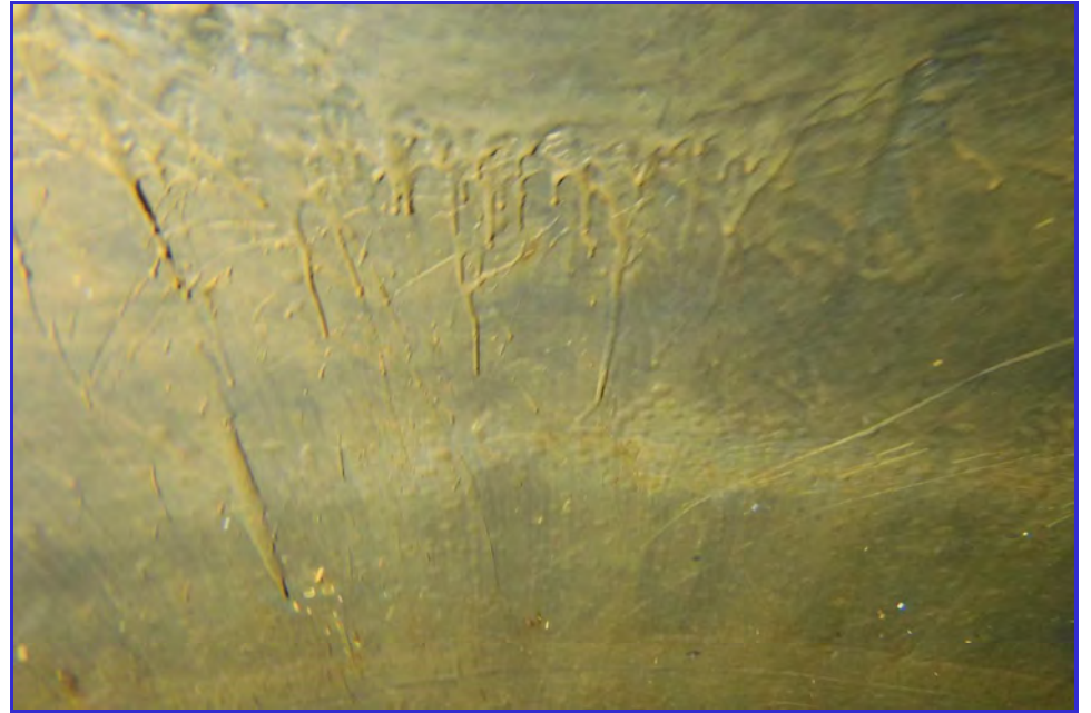
INTERIOR - CPUD - Paloma Reservoir - Maintenance Inspection -073
