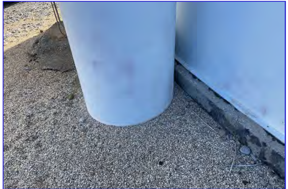
EXTERIOR - CPUD - Mokelumne Reservoir - Maintenance Inspection -143
