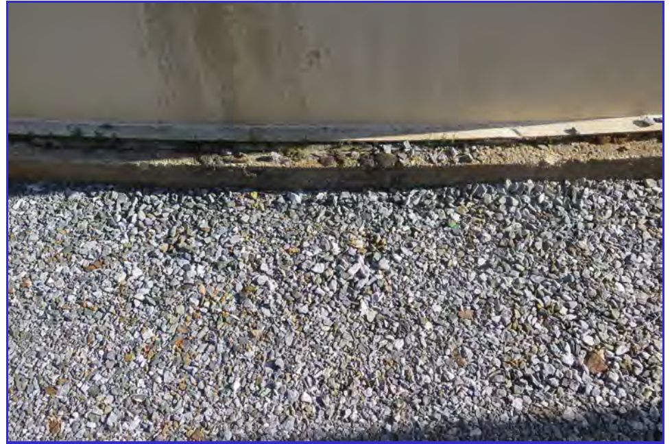
EXTERIOR - Calaveras Public Utility District - Clear Well Tank - Maintenance Inspection -081
