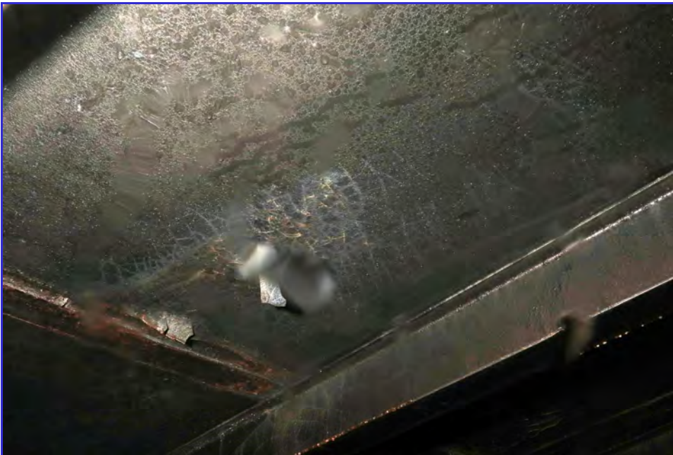
INTERIOR - Calaveras Public Utility District - Clear Well Tank - Maintenance Inspection -006
