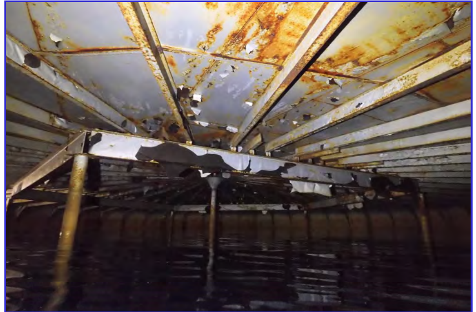
INTERIOR - CPUD - San Andaras Reservoir - Maintenance Inspection -037
