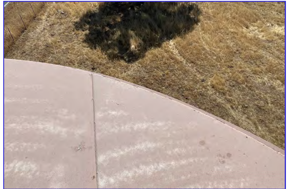
EXTERIOR - CPUD - Paloma Reservoir - Maintenance Inspection -023
