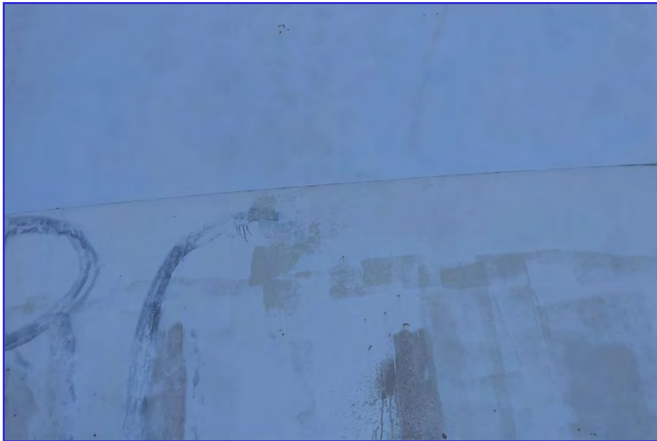
EXTERIOR - CPUD - San Andreas Reservoir - Maintenance Inspection -166
