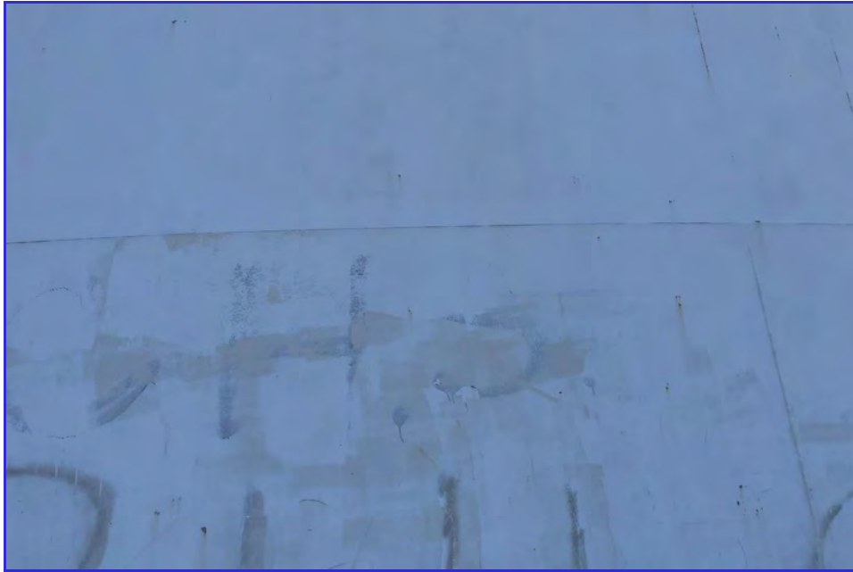
EXTERIOR - CPUD - San Andreas Reservoir - Maintenance Inspection -164
