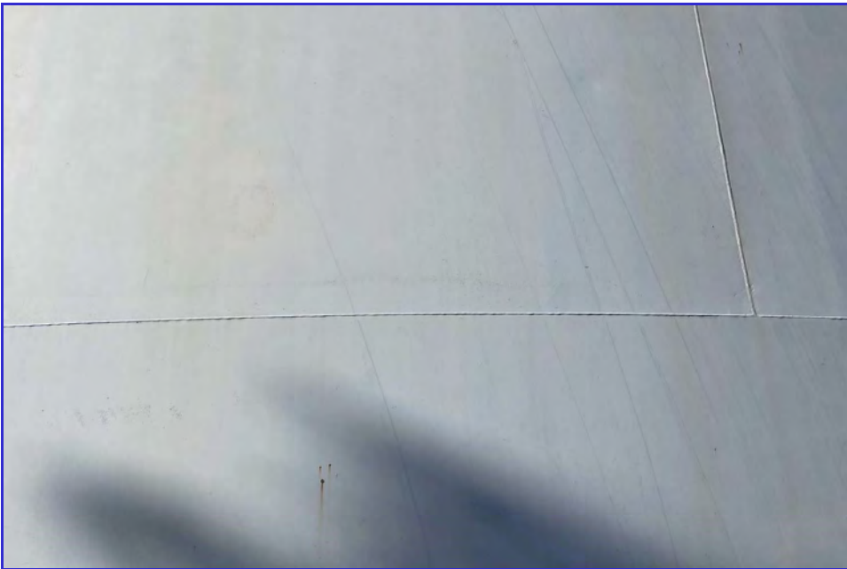
EXTERIOR - CPUD - Mokelumne Reservoir - Maintenance Inspection -082
