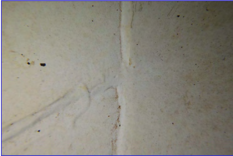
INTERIOR - CPUD - Railroad Flat Reservoir - Maintenance Inspection -108
