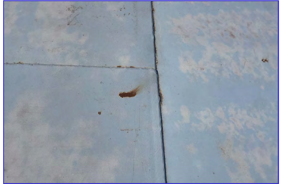
EXTERIOR - CPUD - Mokelumne Reservoir - Maintenance Inspection -021
