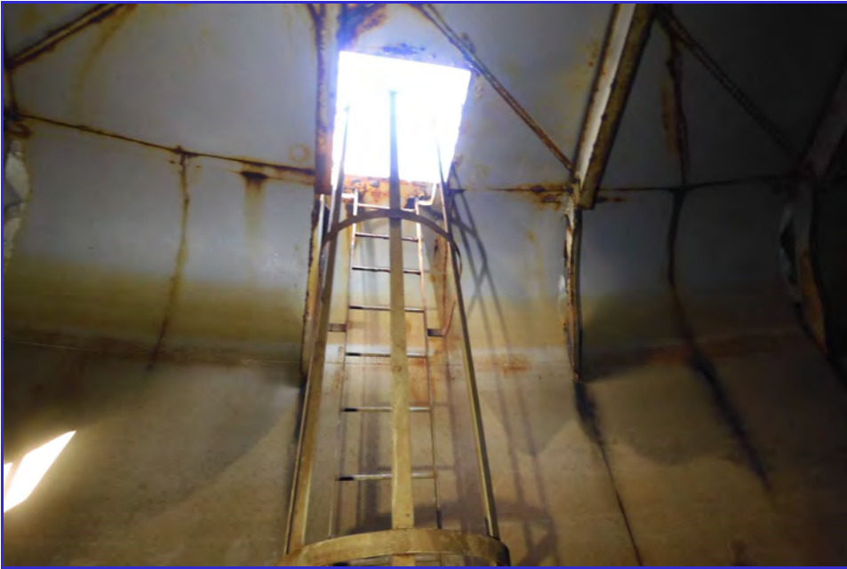
INTERIOR - CPUD - Mokelumne Hill Reservoir - Maintenance Inspection
