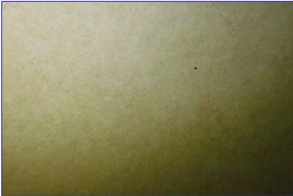
INTERIOR - CPUD - Railroad Flat Reservoir - Maintenance Inspection -130
