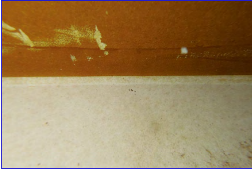
INTERIOR - CPUD - Railroad Flat Reservoir - Maintenance Inspection -112
