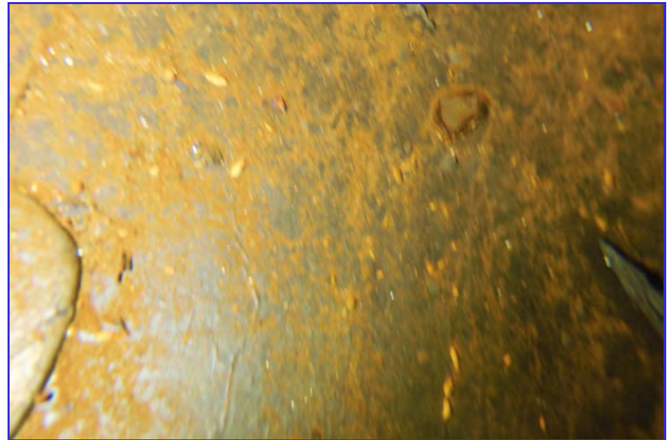
INTERIOR - CPUD - Paloma Reservoir - Maintenance Inspection -143
