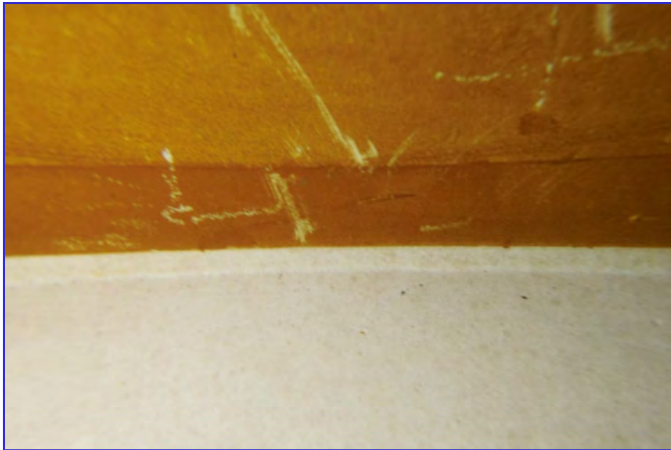
INTERIOR - CPUD - Railroad Flat Reservoir - Maintenance Inspection -114
