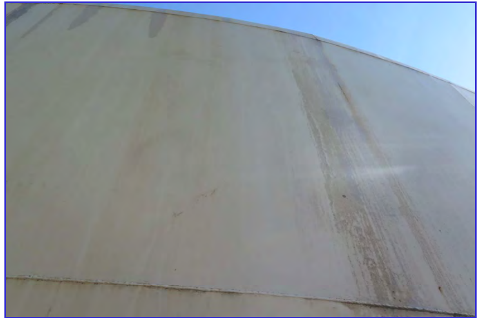
EXTERIOR - Calaveras Public Utility District - Clear Well Tank - Maintenance Inspection -083
