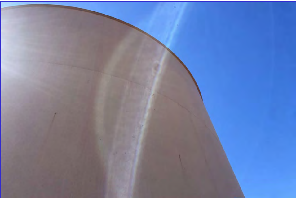
EXTERIOR - CPUD - Paloma Reservoir - Maintenance Inspection -070
