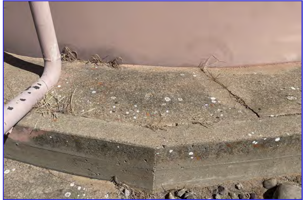
EXTERIOR - CPUD - Paloma Reservoir - Maintenance Inspection -049
