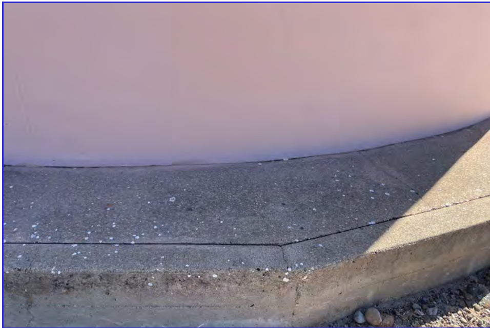
EXTERIOR - CPUD - Paloma Reservoir - Maintenance Inspection -042
