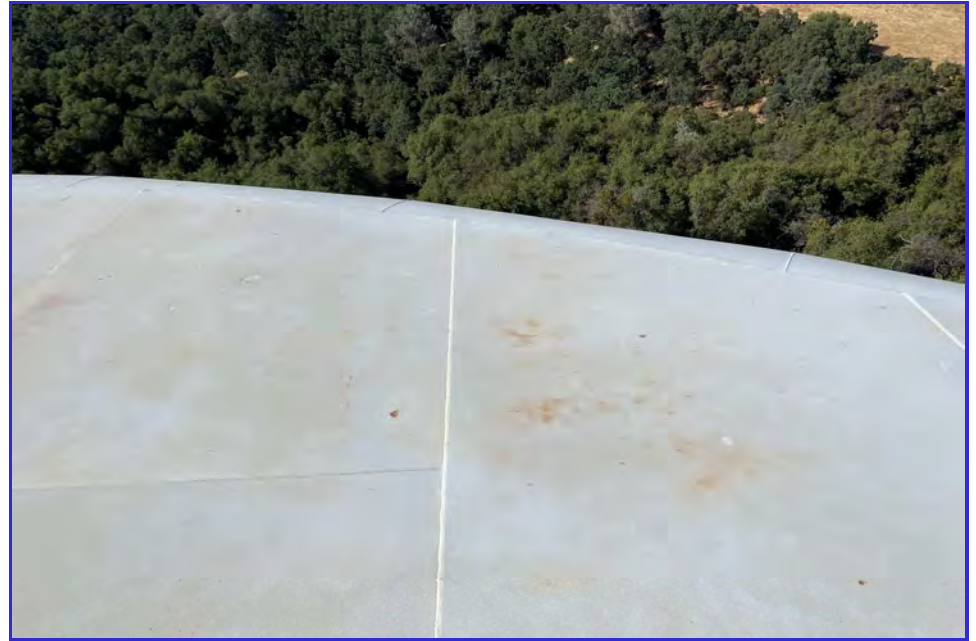
EXTERIOR - CPUD - San Andreas Reservoir - Maintenance Inspection -045
