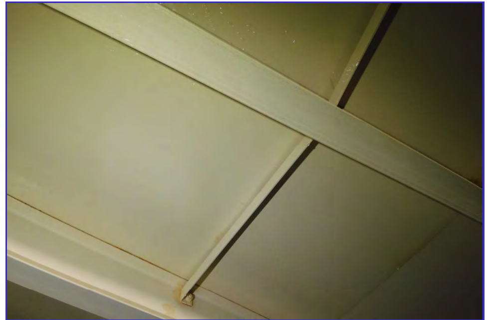
INTERIOR - CPUD - Railroad Flat Reservoir - Maintenance Inspection -031
