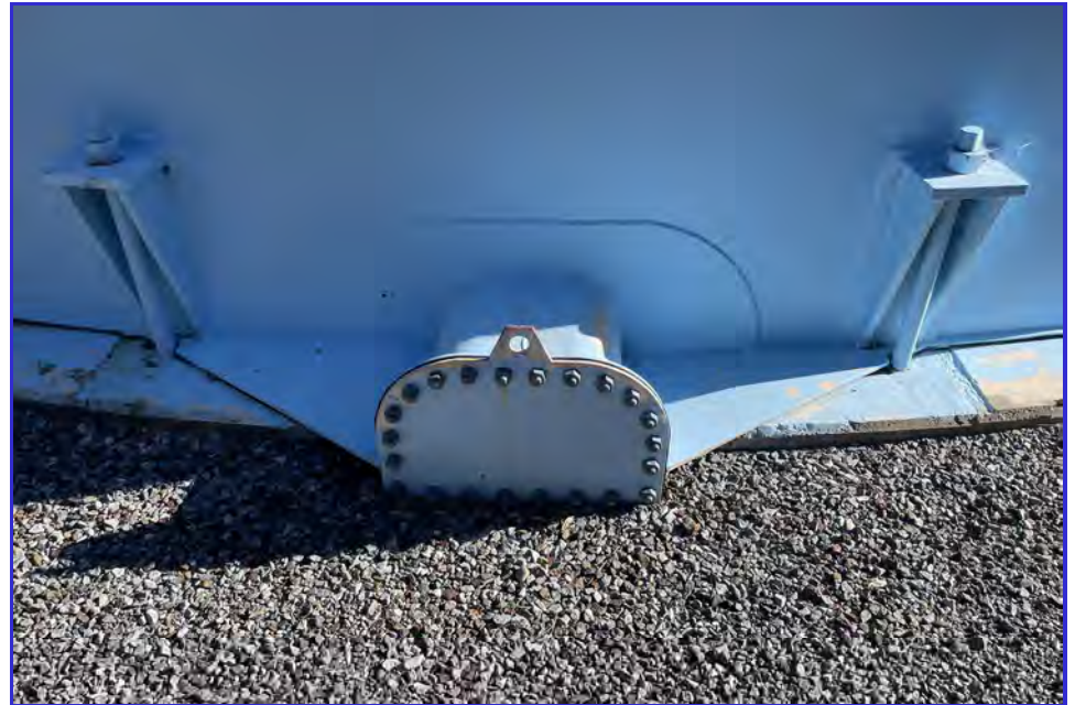
EXTERIOR - CPUD - Railroad Flat Reservoir - Maintenance Inspection -081
