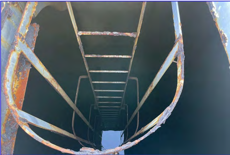
EXTERIOR - CPUD - Mokelumne Reservoir - Maintenance Inspection -002
