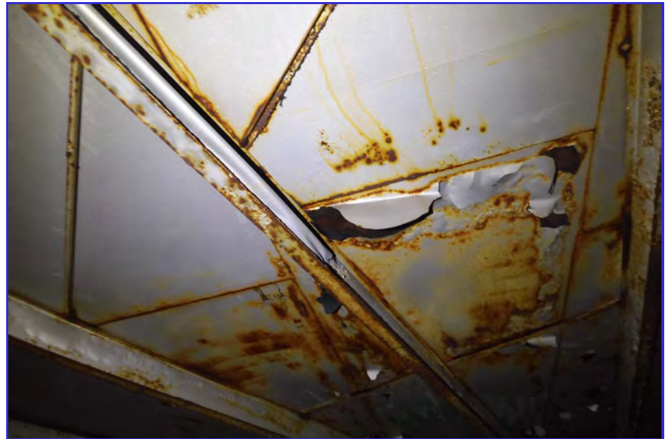
INTERIOR - CPUD - San Andaras Reservoir - Maintenance Inspection -039
