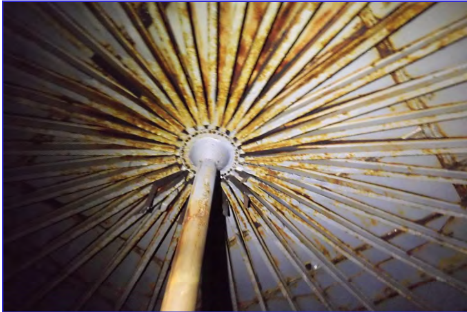
INTERIOR - CPUD - Mokelumne Hill Reservoir - Maintenance Inspection -052
