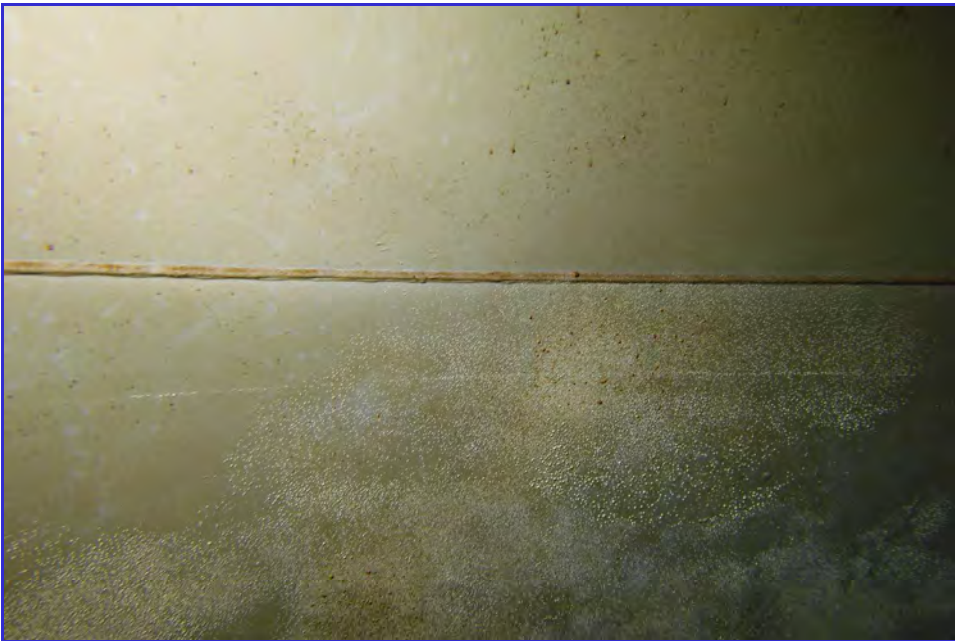
INTERIOR - CPUD - Mokelumne Hill Reservoir - Maintenance Inspection -070
