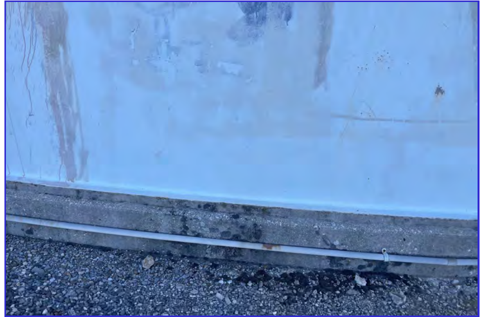
EXTERIOR - CPUD - San Andreas Reservoir - Maintenance Inspection -165
