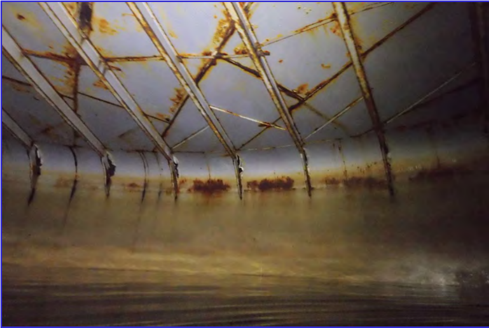
INTERIOR - CPUD - Mokelumne Hill Reservoir - Maintenance Inspection -020
