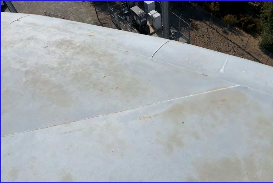
EXTERIOR - CPUD - San Andreas Reservoir - Maintenance Inspection -036
