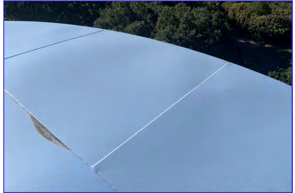
EXTERIOR - CPUD - Railroad Flat Reservoir - Maintenance Inspection -029
