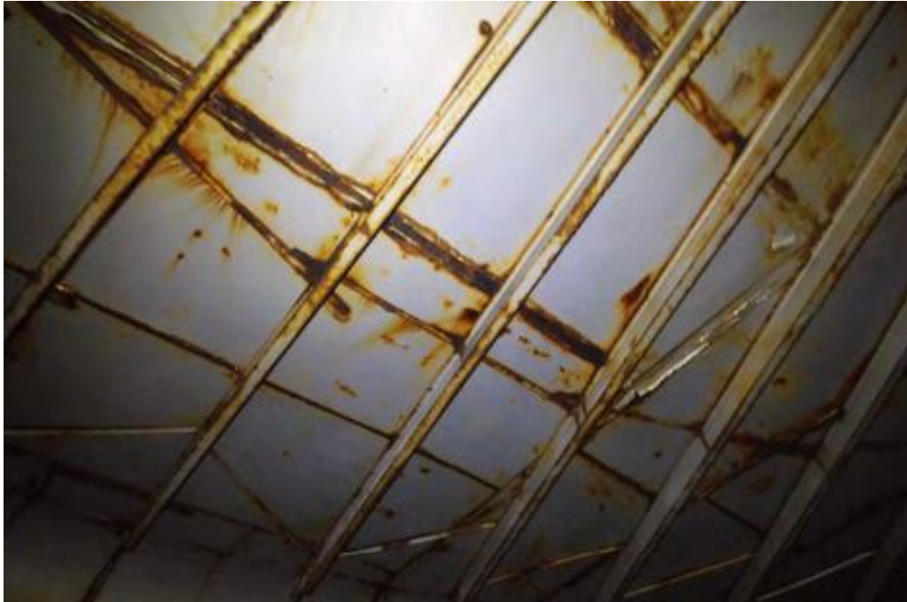
Figure 9-3. Example of Interior Mokelumne Hill Tank Roof
