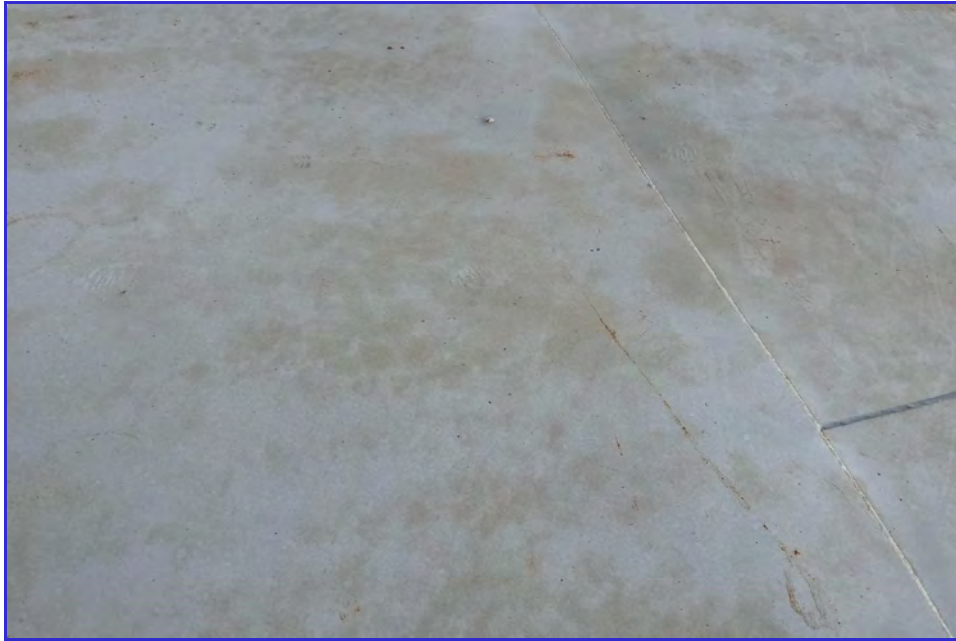
EXTERIOR - CPUD - San Andreas Reservoir - Maintenance Inspection -048
