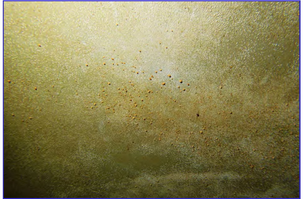
INTERIOR - CPUD - Mokelumne Hill Reservoir - Maintenance Inspection -093
