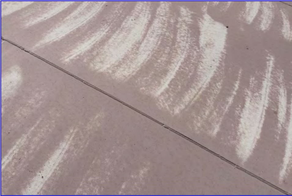
EXTERIOR - CPUD - Paloma Reservoir - Maintenance Inspection -016
