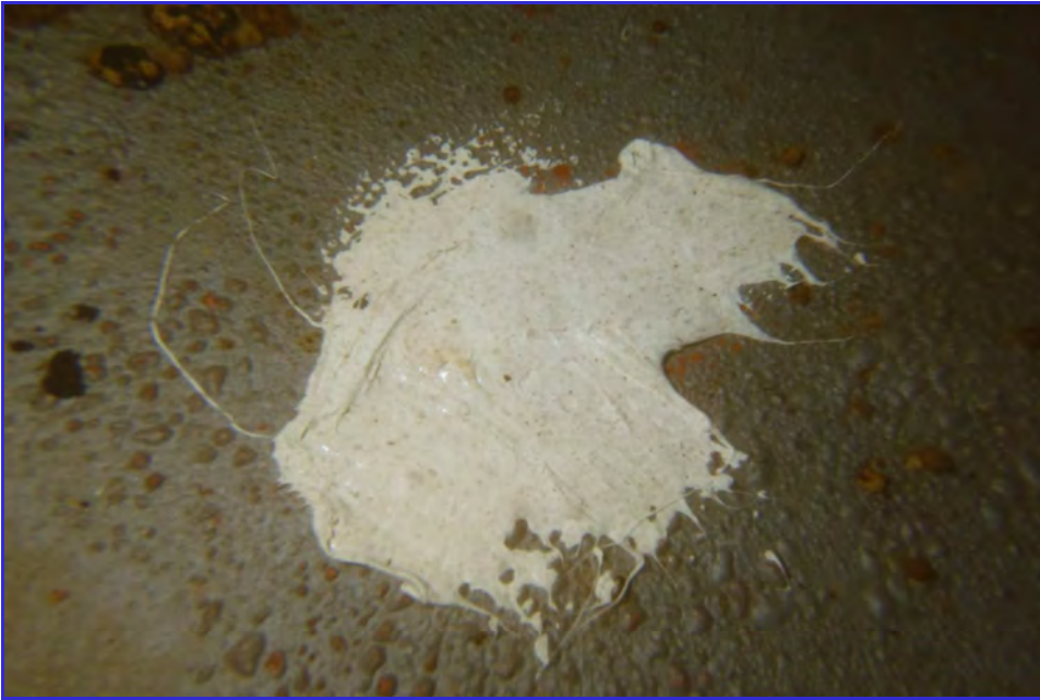
INTERIOR - CPUD - San Andaras Reservoir - Maintenance Inspection -248
