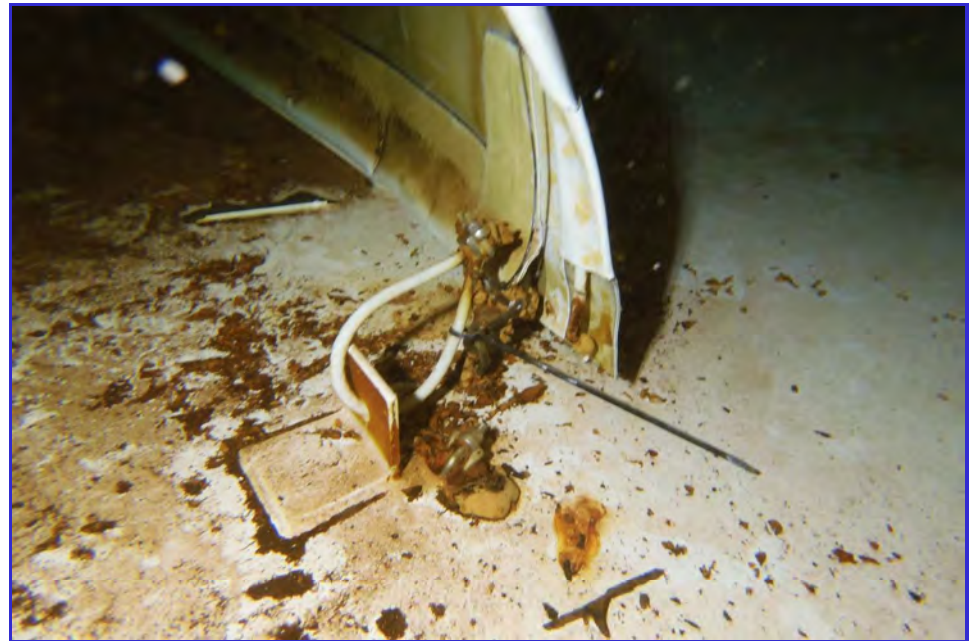
INTERIOR - CPUD - Railroad Flat Reservoir - Maintenance Inspection -139
