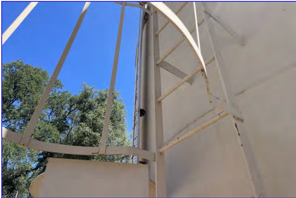
EXTERIOR - CPUD - Golden Hills - Maintenance Inspection -062
