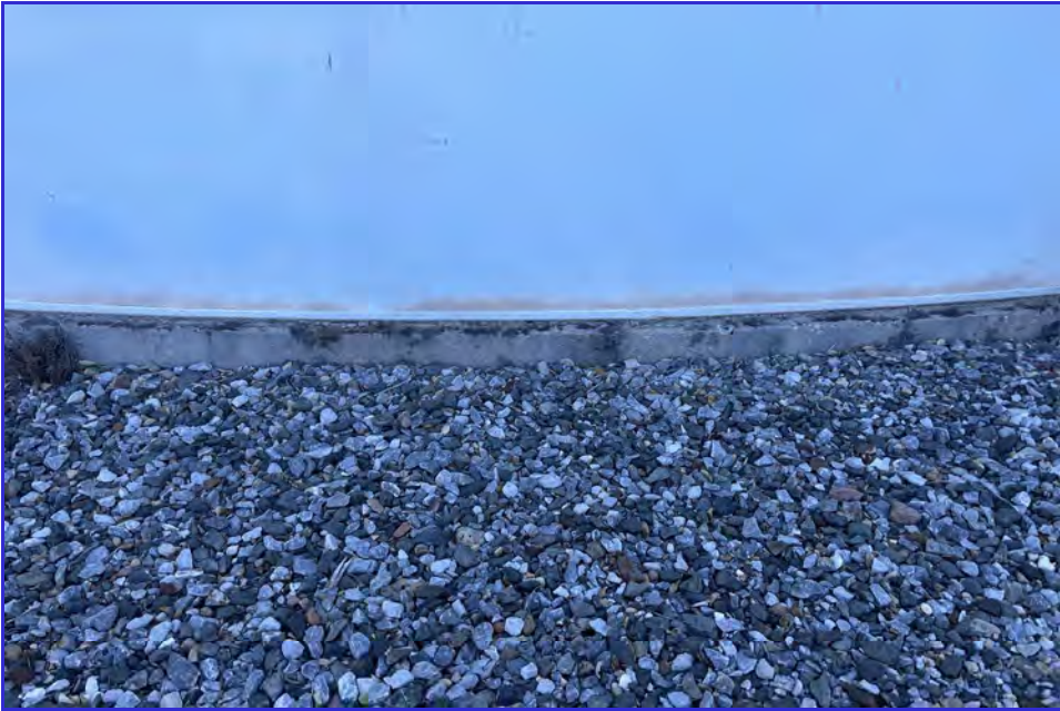
EXTERIOR - CPUD - Mokelumne Reservoir - Maintenance Inspection -148
