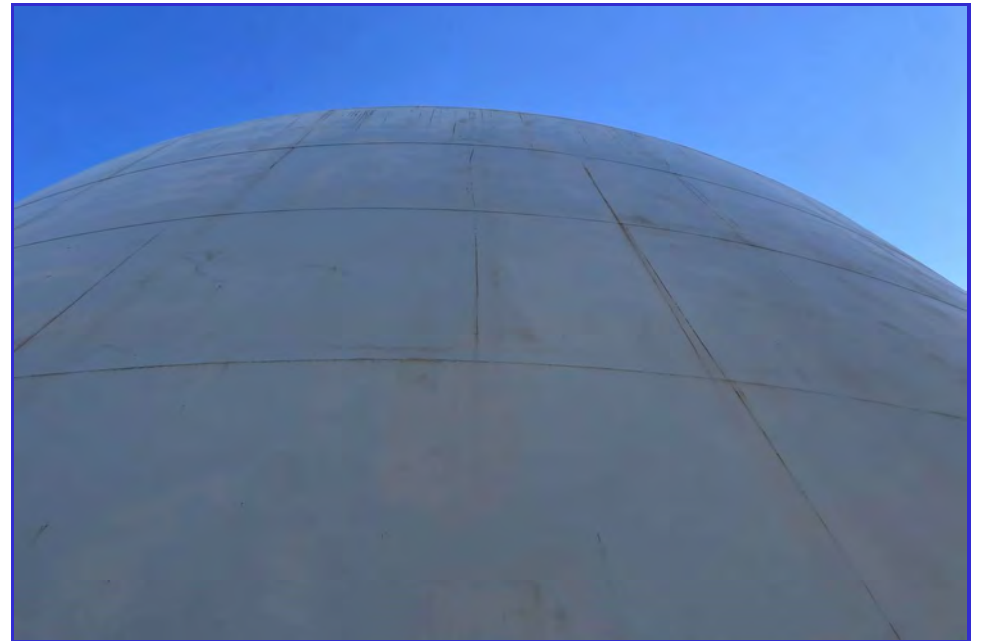
EXTERIOR - CPUD - Mokelumne Reservoir - Maintenance Inspection -155
