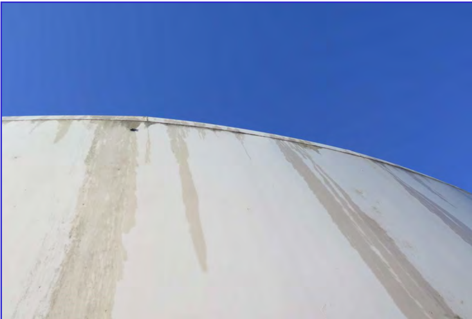
EXTERIOR - Calaveras Public Utility District - Clear Well Tank - Maintenance Inspection -118
