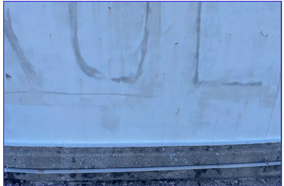
EXTERIOR - CPUD - San Andreas Reservoir - Maintenance Inspection -163
