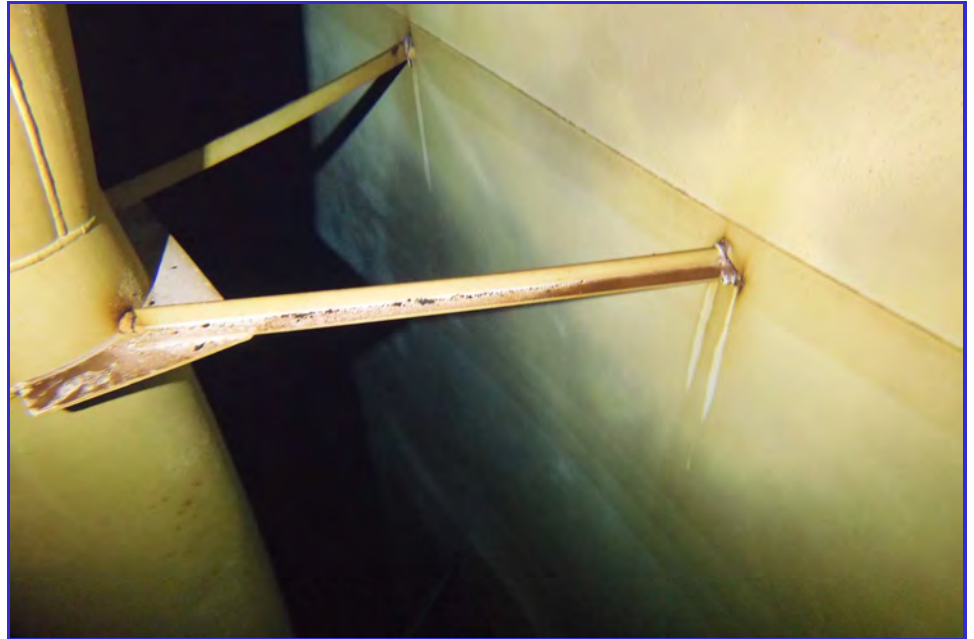
INTERIOR - CPUD - Mokelumne Hill Reservoir - Maintenance Inspection -061
