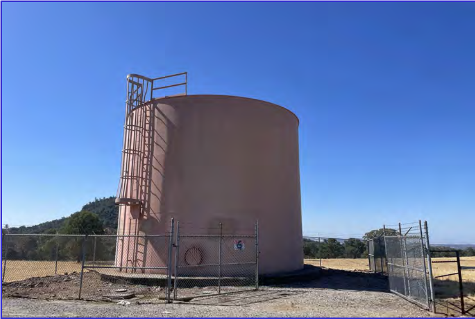
EXTERIOR - CPUD - Paloma Reservoir - Maintenance Inspection
