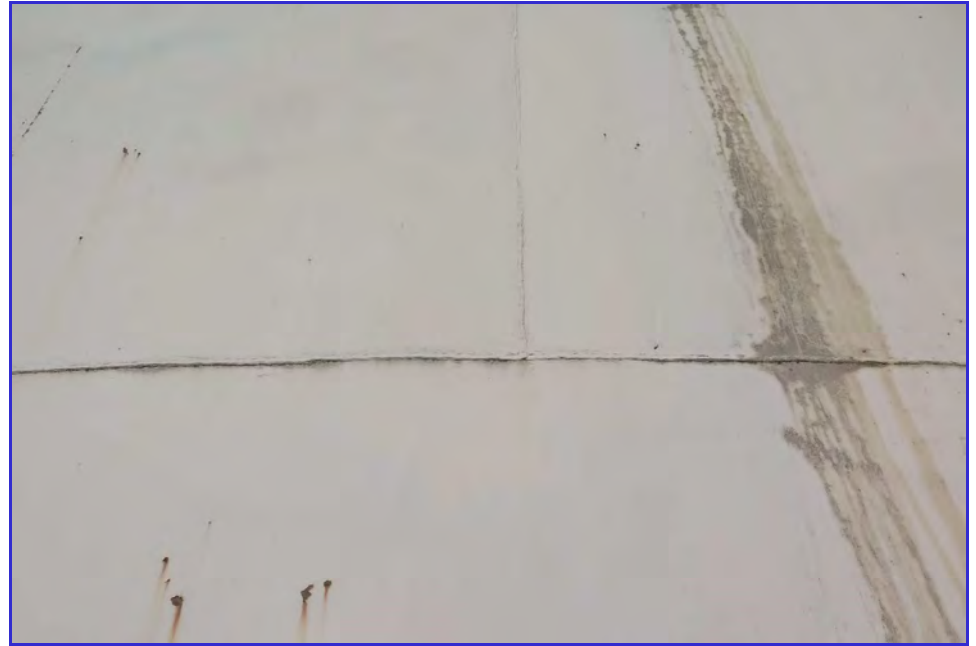
EXTERIOR - Calaveras Public Utility District - Clear Well Tank - Maintenance Inspection -057
