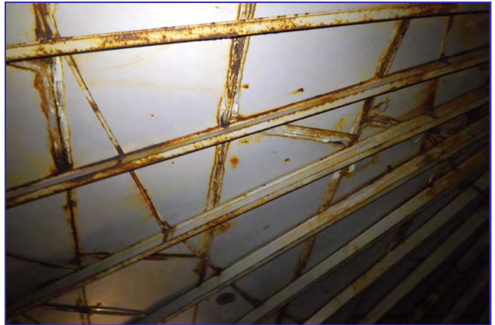
INTERIOR - CPUD - Mokelumne Hill Reservoir - Maintenance Inspection -015
