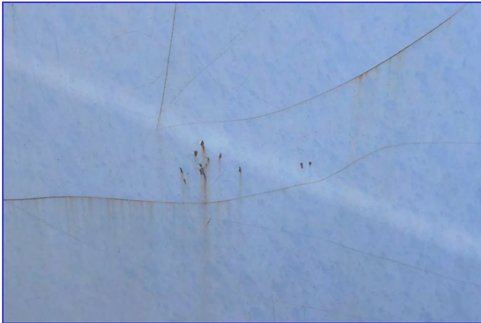
EXTERIOR - CPUD - San Andreas Reservoir - Maintenance Inspection -114
