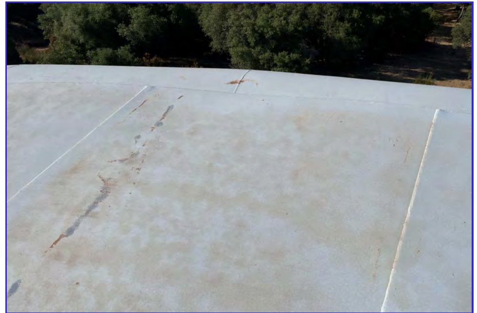
EXTERIOR - CPUD - San Andreas Reservoir - Maintenance Inspection -043
