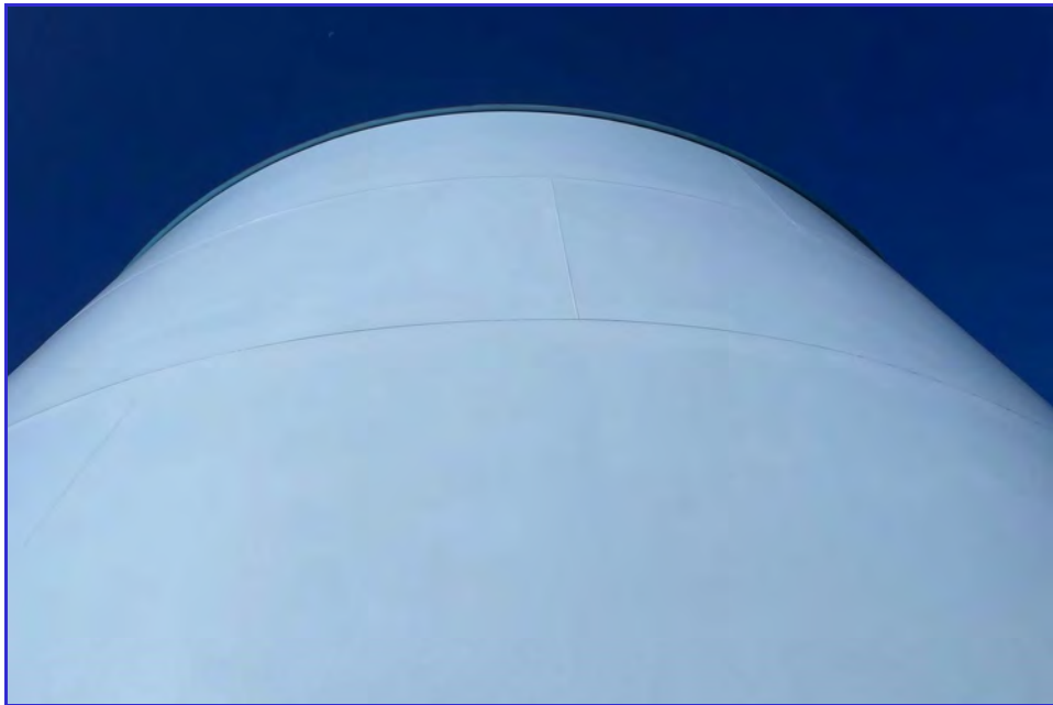
EXTERIOR - CPUD - Railroad Flat Reservoir - Maintenance Inspection -050
