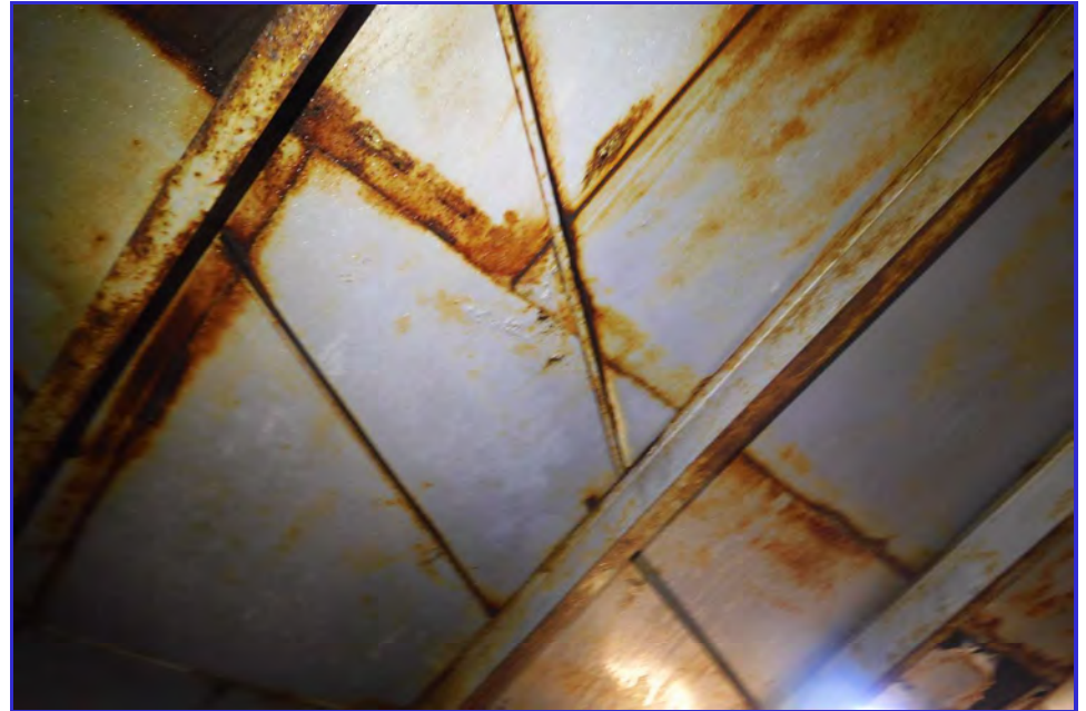
INTERIOR - CPUD - San Andreas Reservoir - Maintenance Inspection -013
