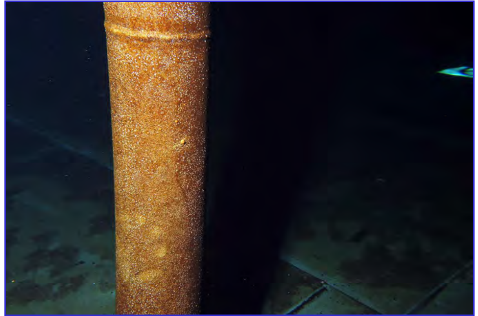
INTERIOR - Calaveras Public Utility District - Clear Well Tank - Maintenance Inspection -109
