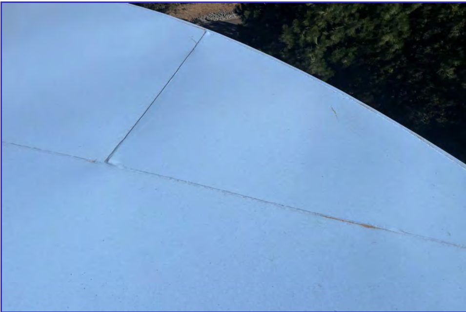
EXTERIOR - CPUD - Railroad Flat Reservoir - Maintenance Inspection -014
