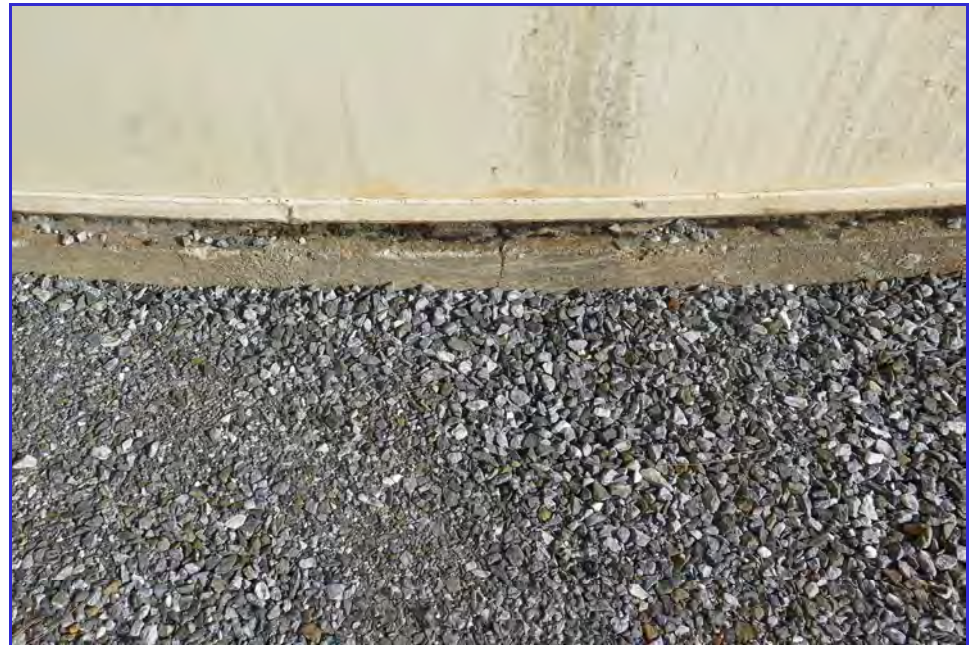
EXTERIOR - Calaveras Public Utility District - Clear Well Tank - Maintenance Inspection -075
