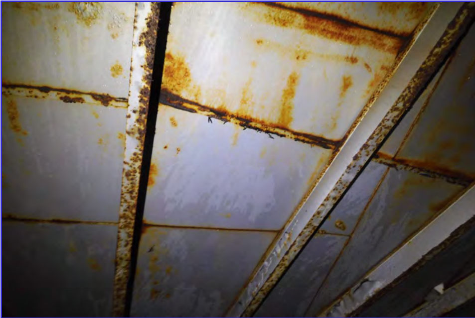
INTERIOR - CPUD - San Andaras Reservoir - Maintenance Inspection -048
