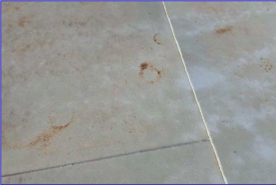
EXTERIOR - CPUD - San Andreas Reservoir - Maintenance Inspection -076
