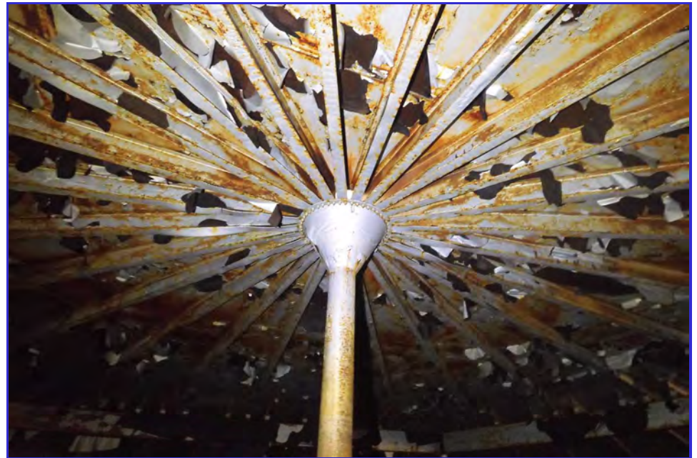
INTERIOR - CPUD - San Andaras Reservoir - Maintenance Inspection -083
