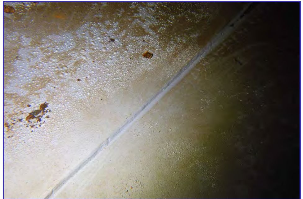
INTERIOR - CPUD - San Andaras Reservoir - Maintenance Inspection -187
