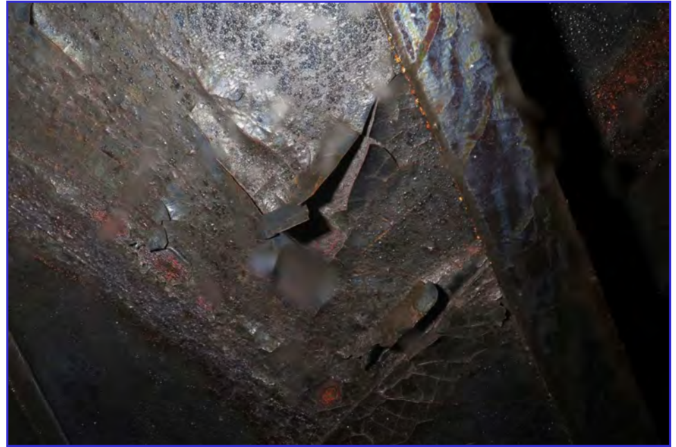
INTERIOR - Calaveras Public Utility District - Clear Well Tank - Maintenance Inspection -009
