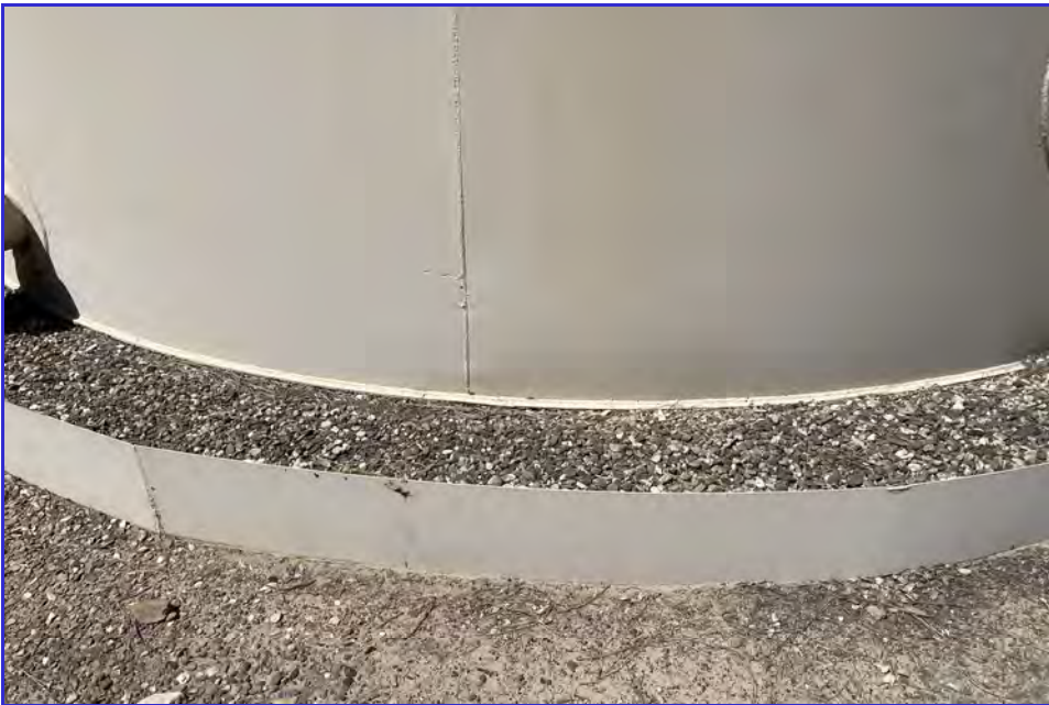
EXTERIOR - CPUD - Golden Hills - Maintenance Inspection -046
