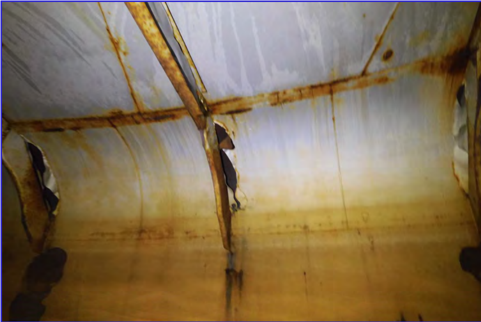
INTERIOR - CPUD - San Andaras Reservoir - Maintenance Inspection -096
