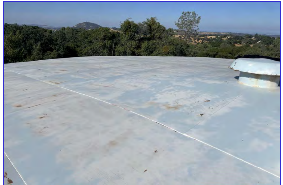
EXTERIOR - CPUD - Mokelumne Reservoir - Maintenance Inspection -015
