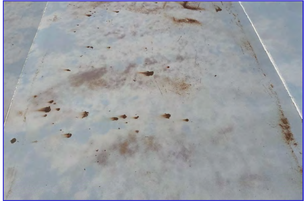
EXTERIOR - CPUD - Mokelumne Reservoir - Maintenance Inspection -017
