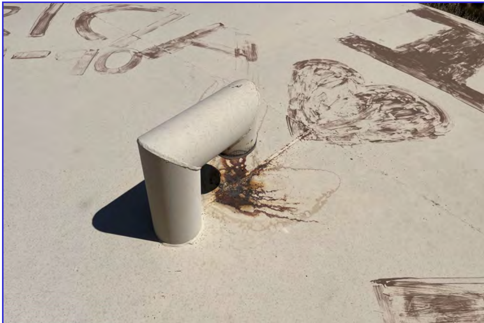
EXTERIOR - CPUD - Golden Hills - Maintenance Inspection -002
