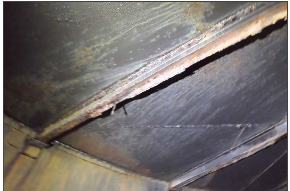
INTERIOR - CPUD - Paloma Reservoir - Maintenance Inspection -011
