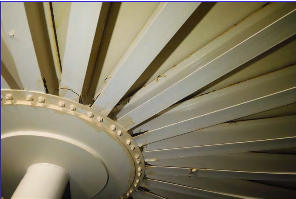
INTERIOR - CPUD - Railroad Flat Reservoir - Maintenance Inspection -034
