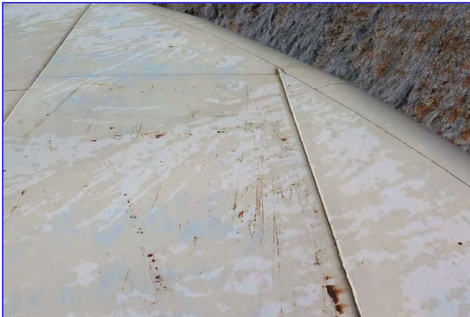
EXTERIOR - Calaveras Public Utility District - Clear Well Tank - Maintenance Inspection -020
