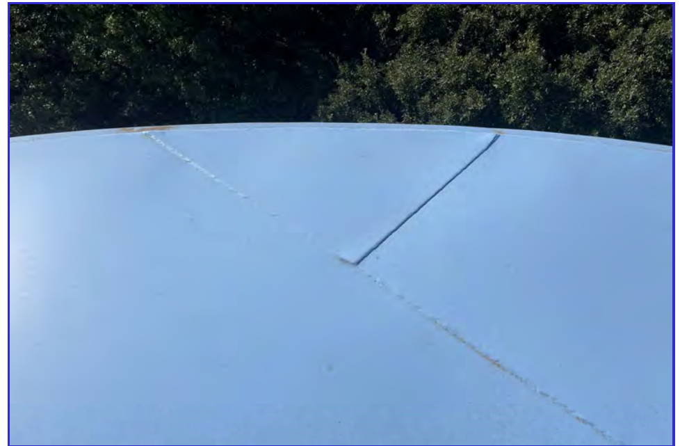
EXTERIOR - CPUD - Railroad Flat Reservoir - Maintenance Inspection -023
