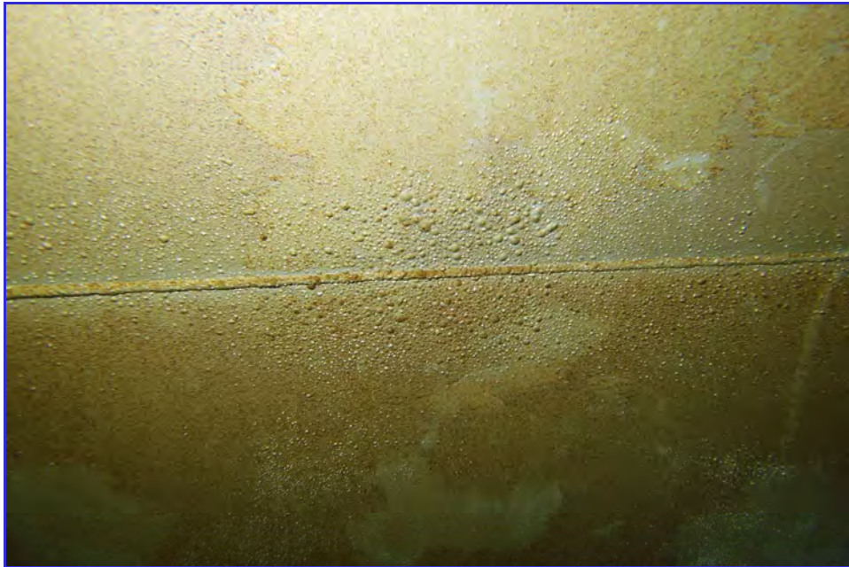
INTERIOR - CPUD - San Anderas Reservoir - Maintenance Inspection -124
