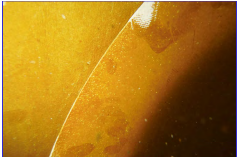
INTERIOR - CPUD - Railroad Flat Reservoir - Maintenance Inspection -123
