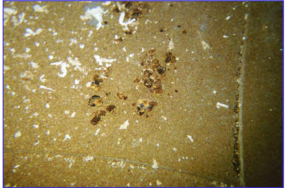
INTERIOR - CPUD - San Andaras Reservoir - Maintenance Inspection -177
