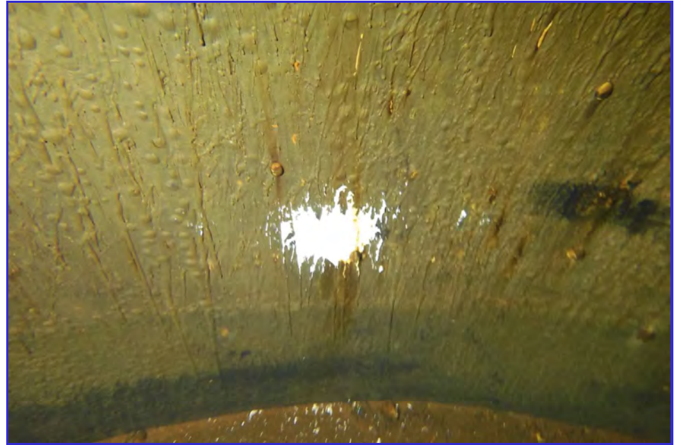
INTERIOR - CPUD - Paloma Reservoir - Maintenance Inspection -097
