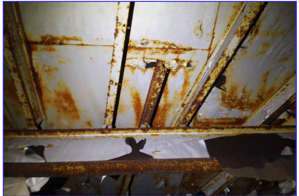
INTERIOR - CPUD - San Andaras Reservoir - Maintenance Inspection -055
