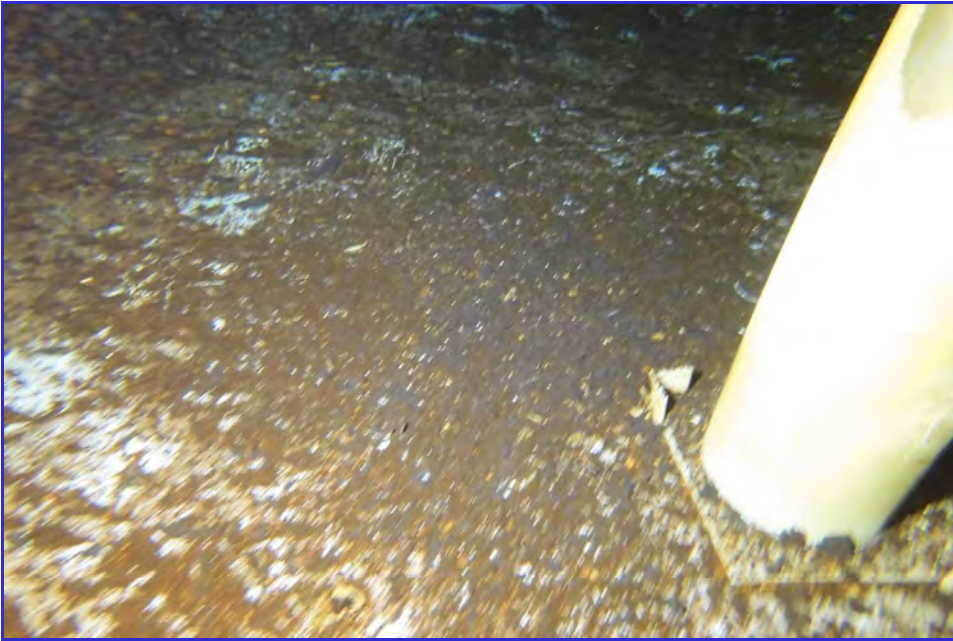
INTERIOR - CPUD - Mokelumne Hill Reservoir - Maintenance Inspection -148
