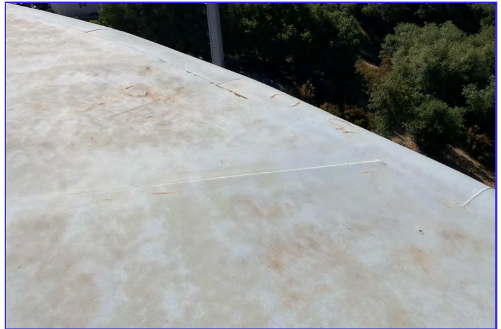
EXTERIOR - CPUD - San Andreas Reservoir - Maintenance Inspection -039
