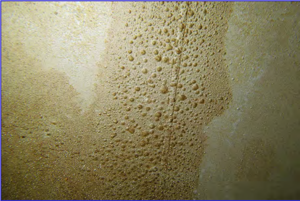
INTERIOR - CPUD - San Andaras Reservoir - Maintenance Inspection -132
