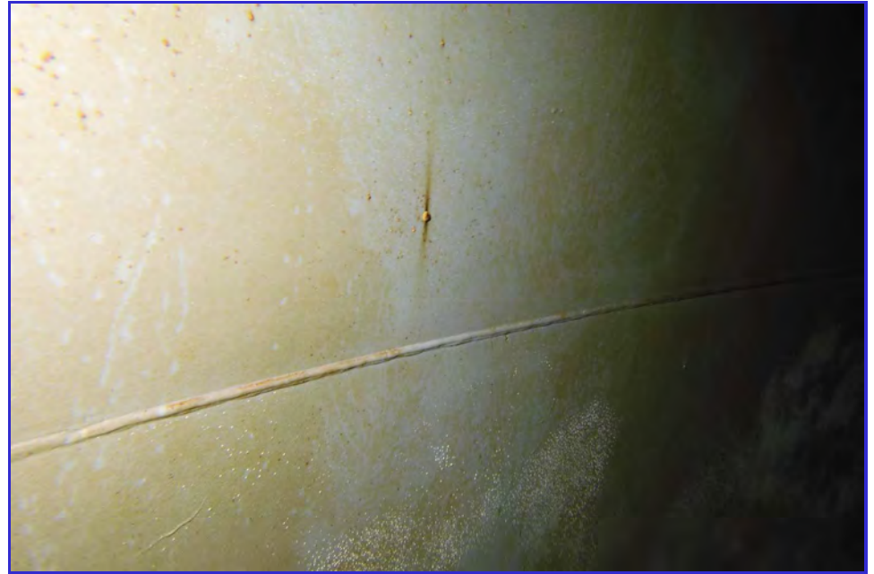
INTERIOR - CPUD - Mokelumne Hill Reservoir - Maintenance Inspection -089
