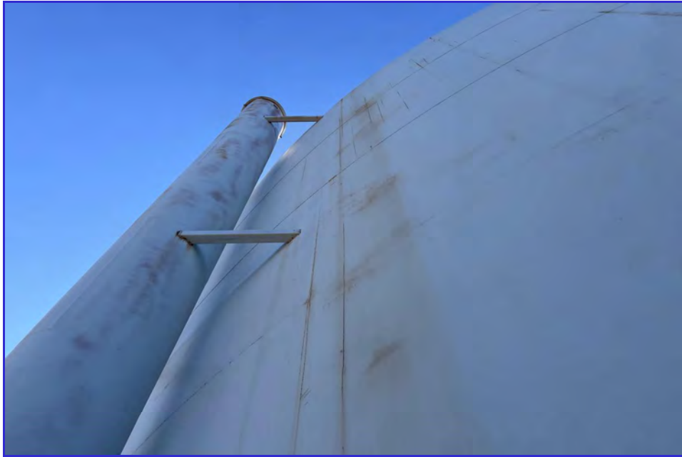
EXTERIOR - CPUD - Mokelumne Reservoir - Maintenance Inspection -144
