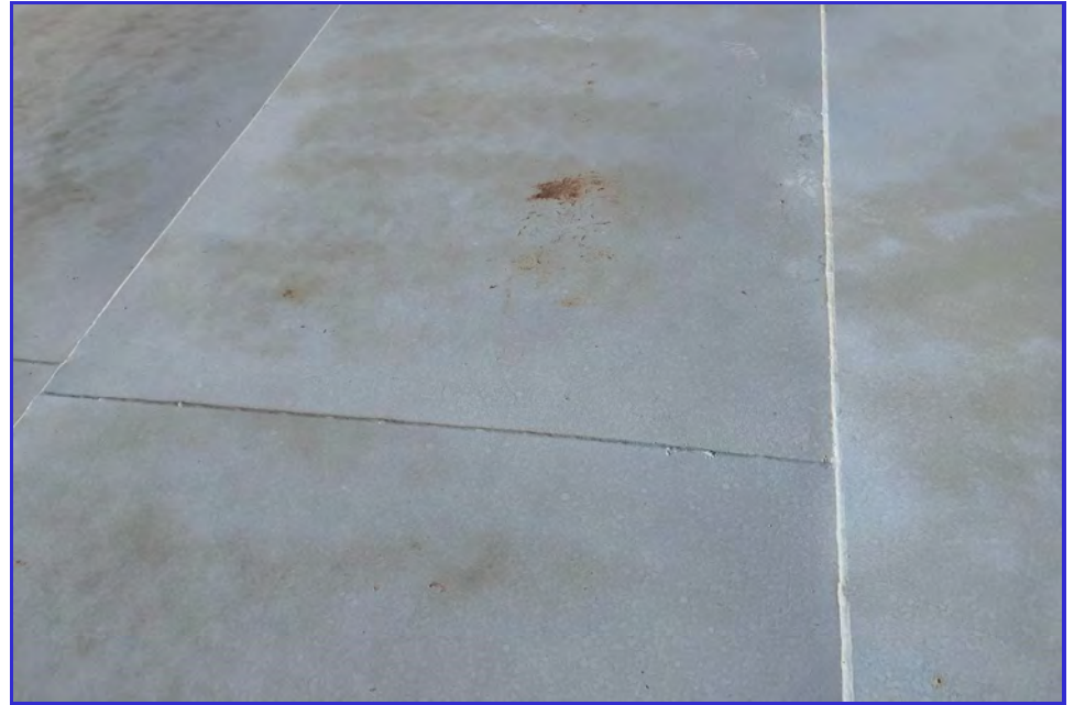
EXTERIOR - CPUD - San Andreas Reservoir - Maintenance Inspection -009
