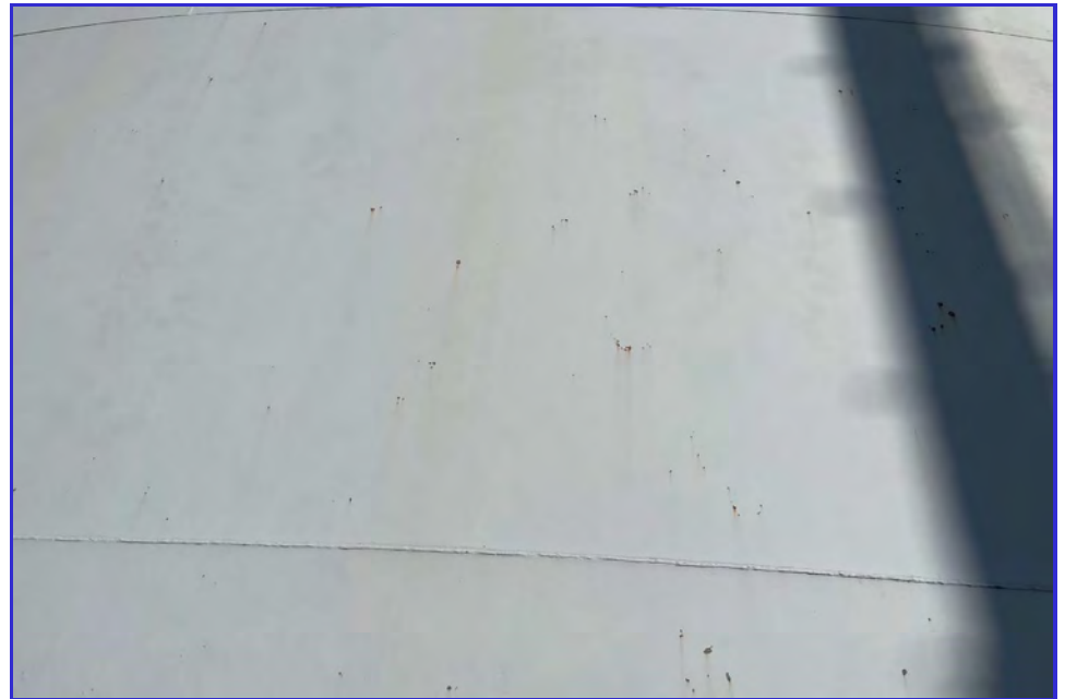
EXTERIOR - CPUD - San Andreas Reservoir - Maintenance Inspection -147
