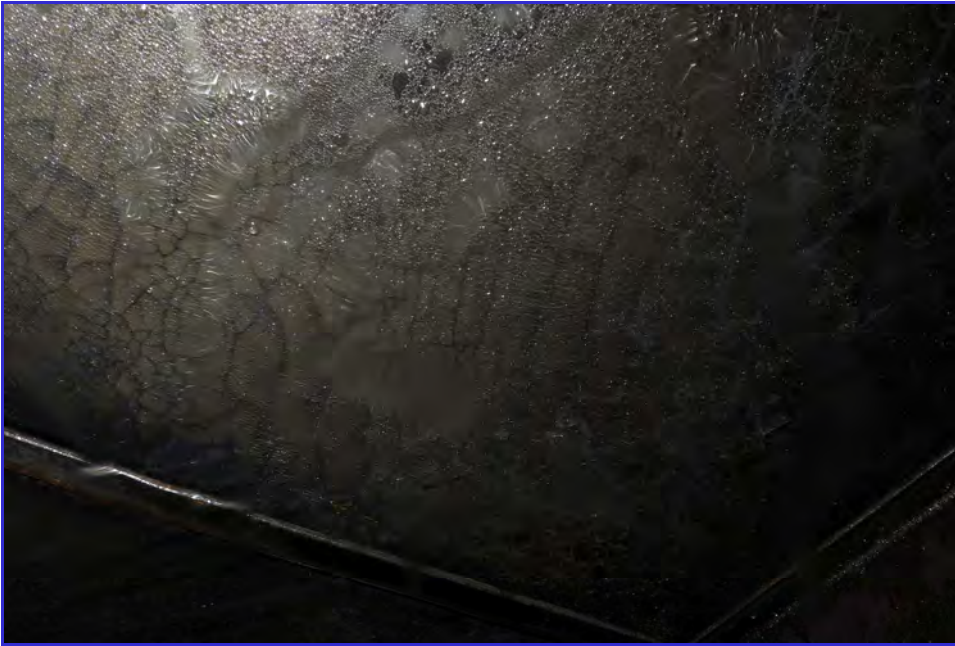
INTERIOR - Calaveras Public Utility District - Clear Well Tank - Maintenance Inspection -004
