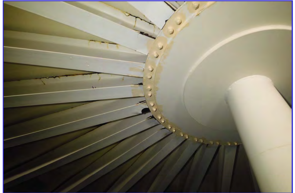
INTERIOR - CPUD - Railroad Flat Reservoir - Maintenance Inspection -037
