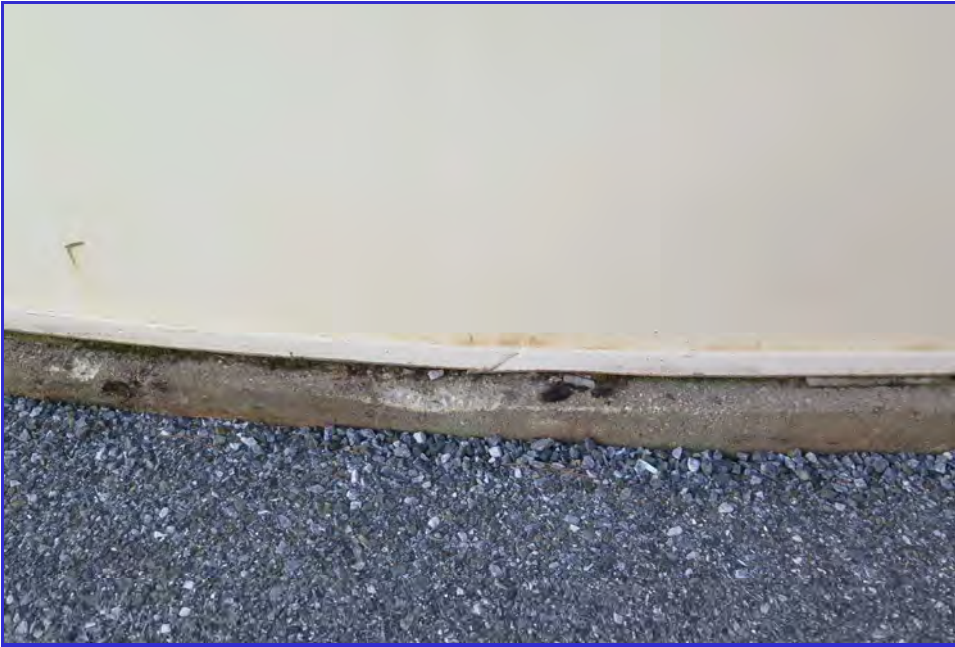
EXTERIOR - Calaveras Public Utility District - Clear Well Tank - Maintenance Inspection -104
