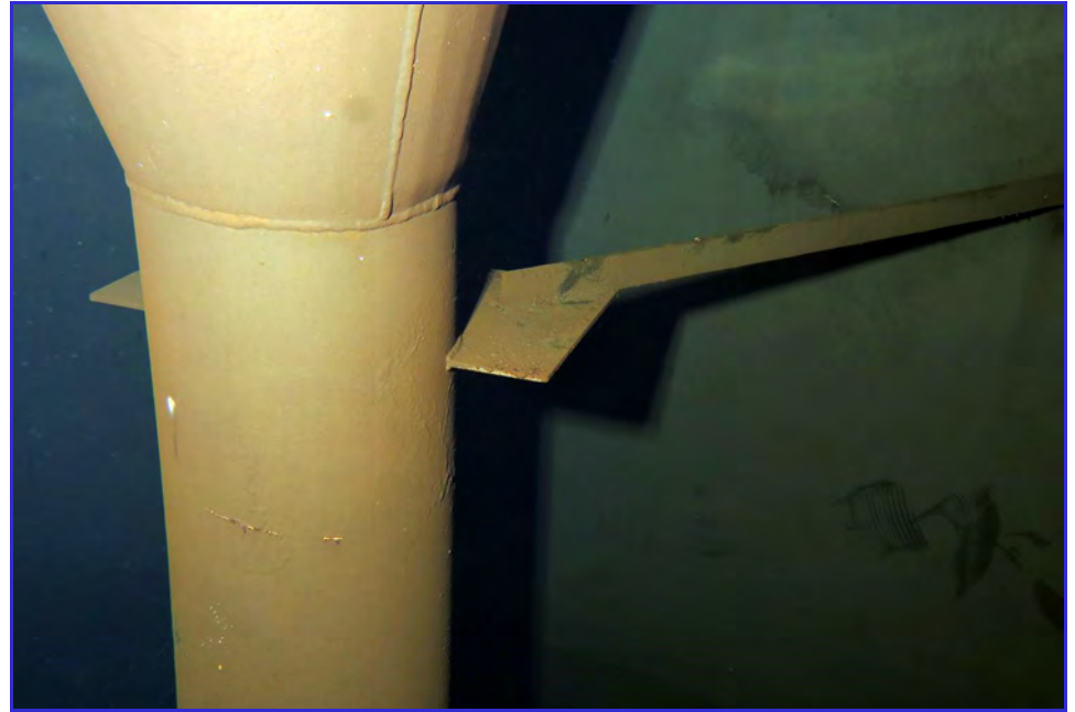
INTERIOR - Calaveras Public Utility District - Clear Well Tank - Maintenance Inspection -057
