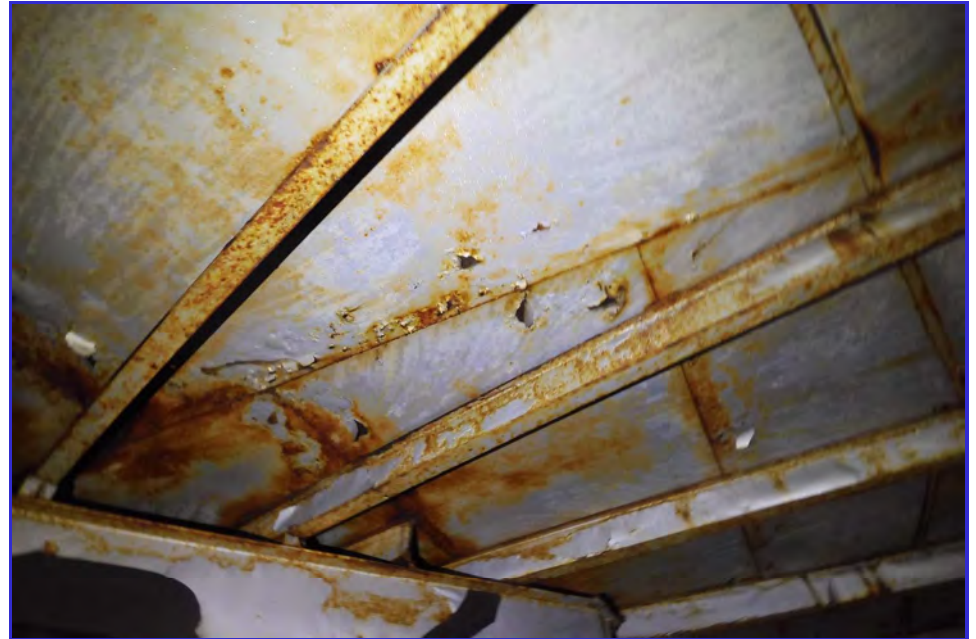
INTERIOR - CPUD - San Andaras Reservoir - Maintenance Inspection -093
