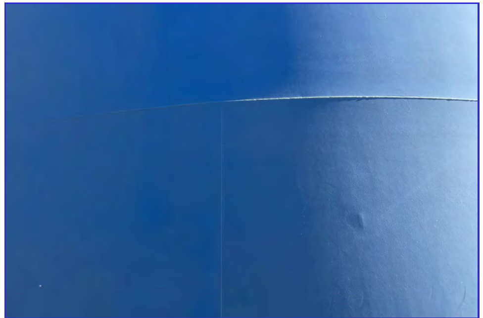
EXTERIOR - CPUD - Railroad Flat Reservoir - Maintenance Inspection -083
