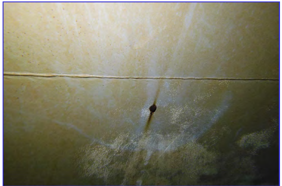
INTERIOR - CPUD - Mokelumne Hill Reservoir - Maintenance Inspection -083
