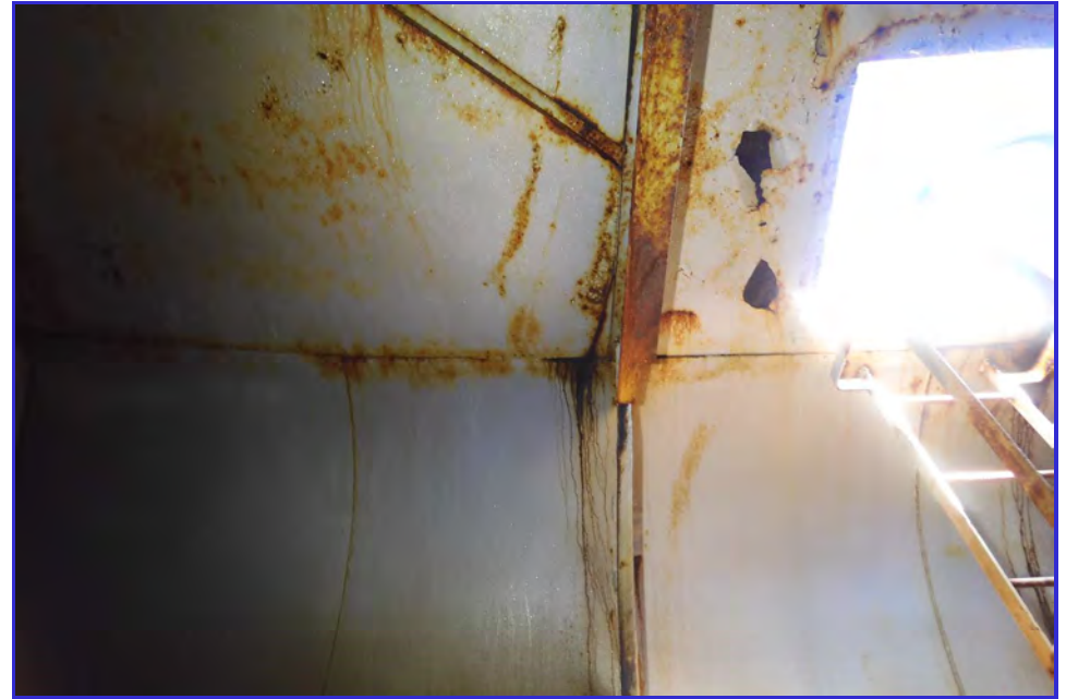
INTERIOR - CPUD - San Andreas Reservoir - Maintenance Inspection -001
