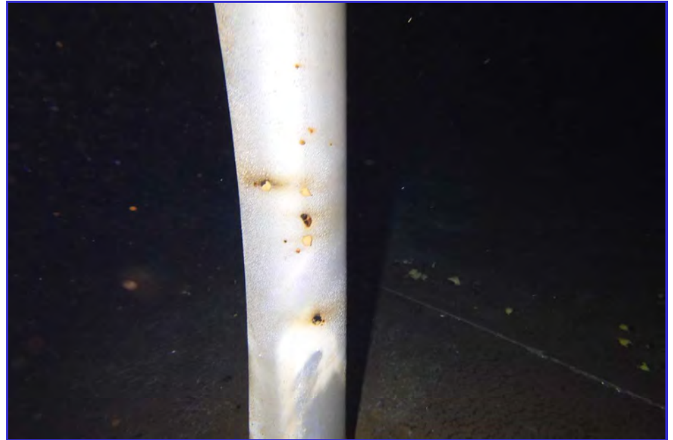
INTERIOR - CPUD - San Andaras Reservoir - Maintenance Inspection -149
