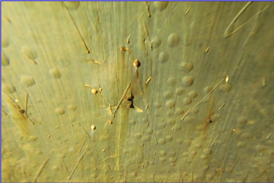
INTERIOR - CPUD - Paloma Reservoir - Maintenance Inspection -076
