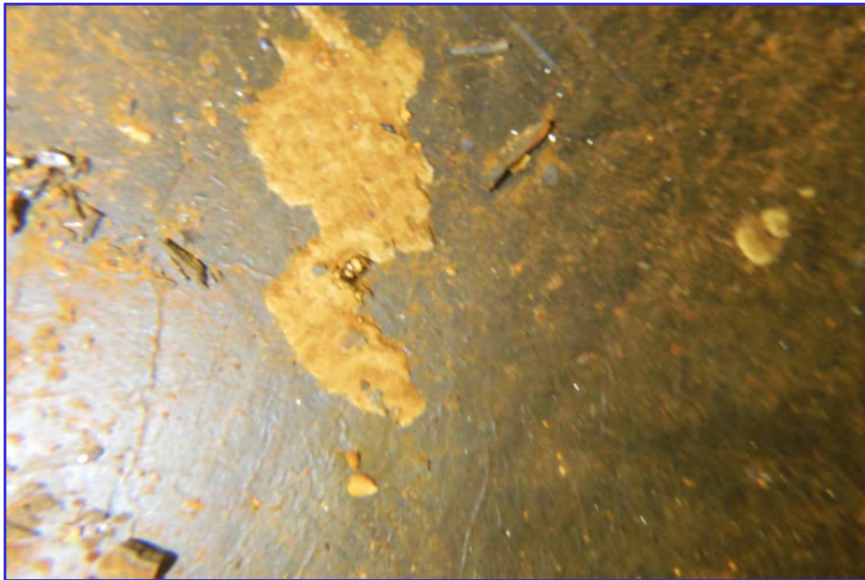
INTERIOR - CPUD - Paloma Reservoir - Maintenance Inspection -142
