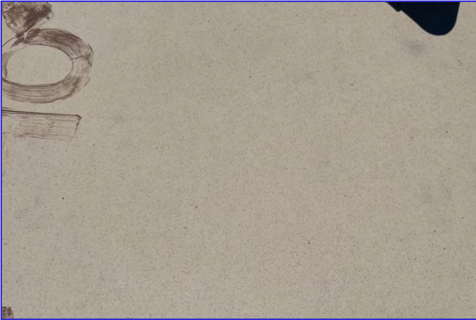
EXTERIOR - CPUD - Golden Hills - Maintenance Inspection -012
