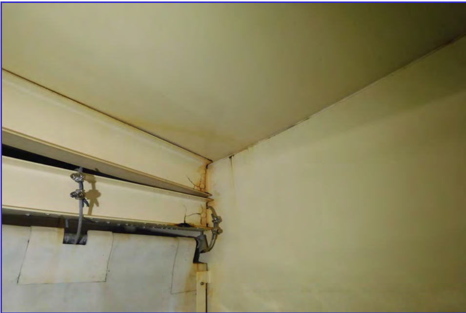
INTERIOR - CPUD - Railroad Flat Reservoir - Maintenance Inspection -026
