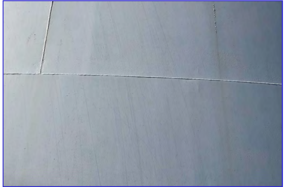
EXTERIOR - CPUD - Mokelumne Reservoir - Maintenance Inspection -081
