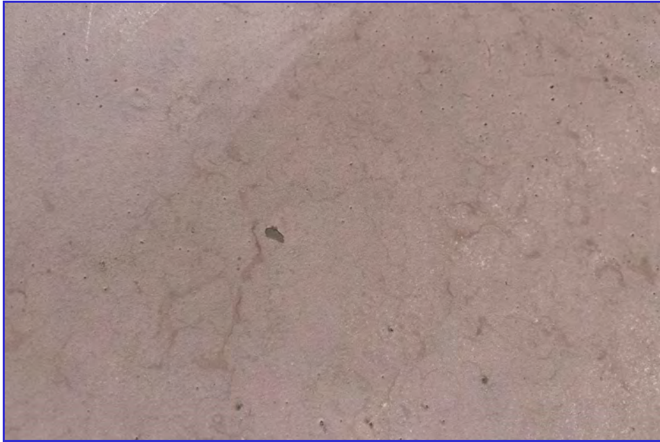
EXTERIOR - CPUD - Paloma Reservoir - Maintenance Inspection -020
