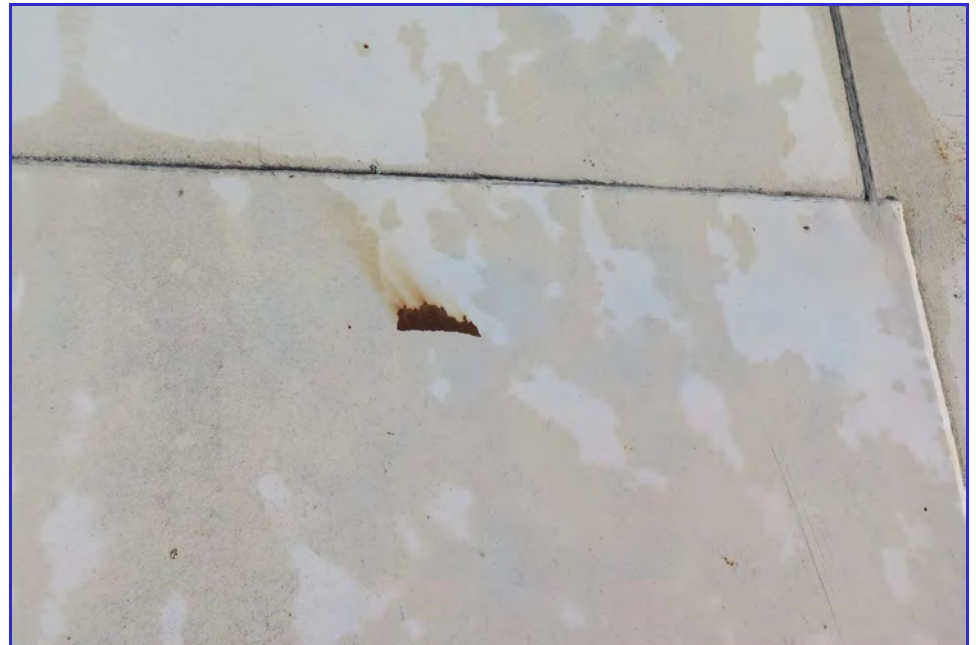
EXTERIOR - Calaveras Public Utility District - Clear Well Tank - Maintenance Inspection -011
