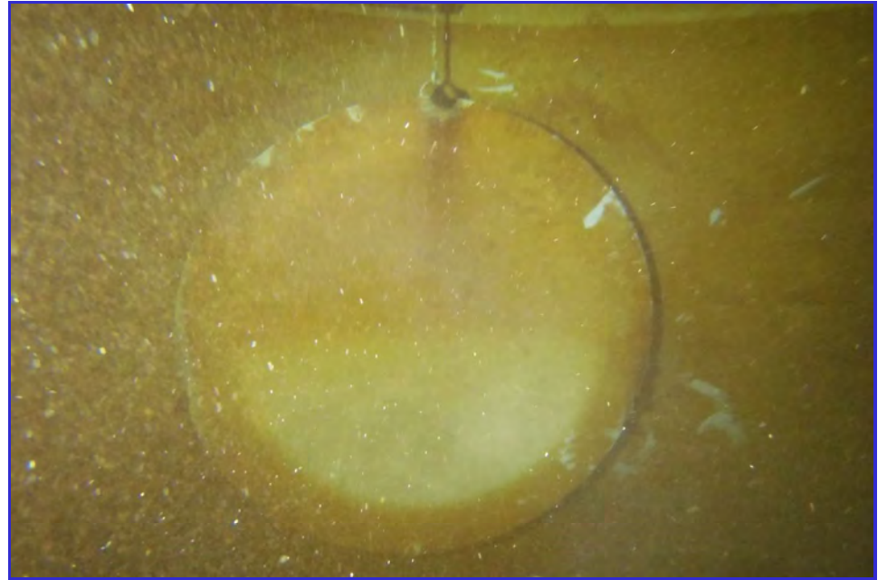
INTERIOR - CPUD - Railroad Flat Reservoir - Maintenance Inspection -121
