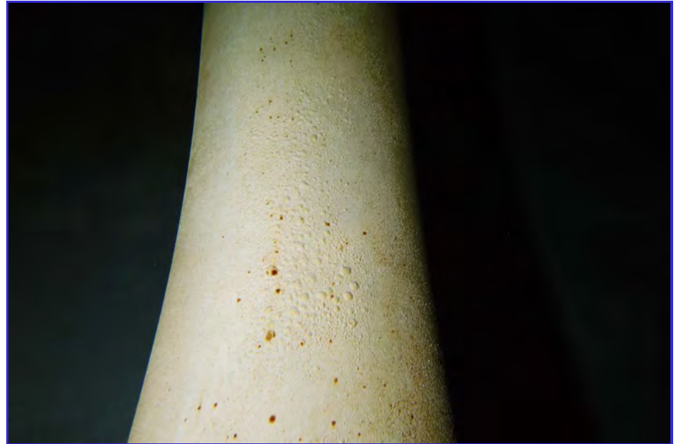
INTERIOR - CPUD - Mokelumne Hill Reservoir - Maintenance Inspection -113
