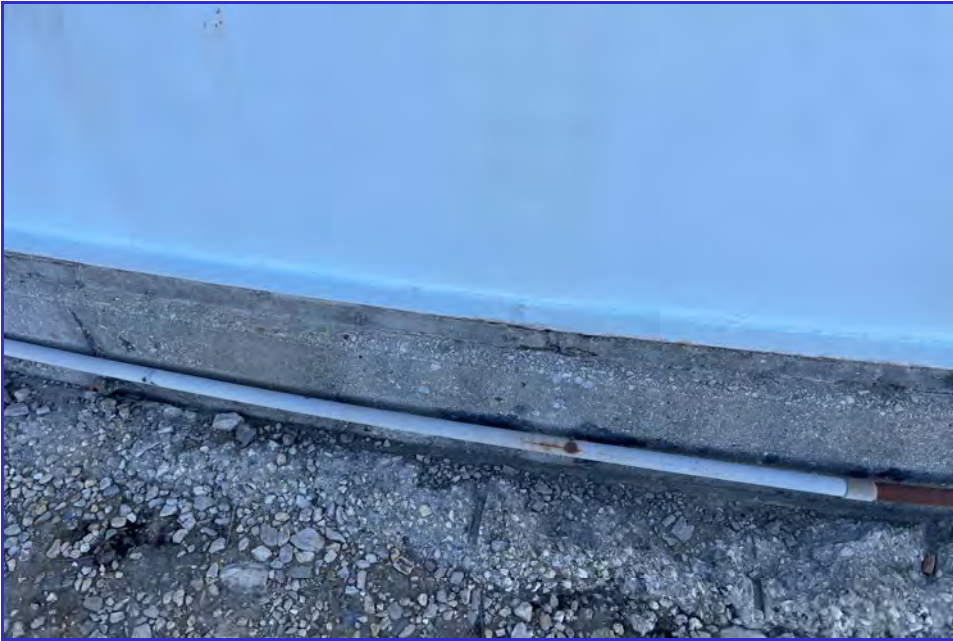
EXTERIOR - CPUD - San Andreas Reservoir - Maintenance Inspection -180
