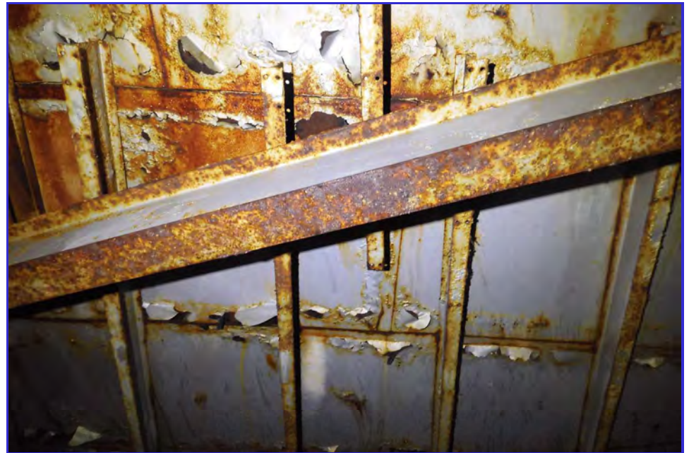
INTERIOR - CPUD - San Andaras Reservoir - Maintenance Inspection -071
