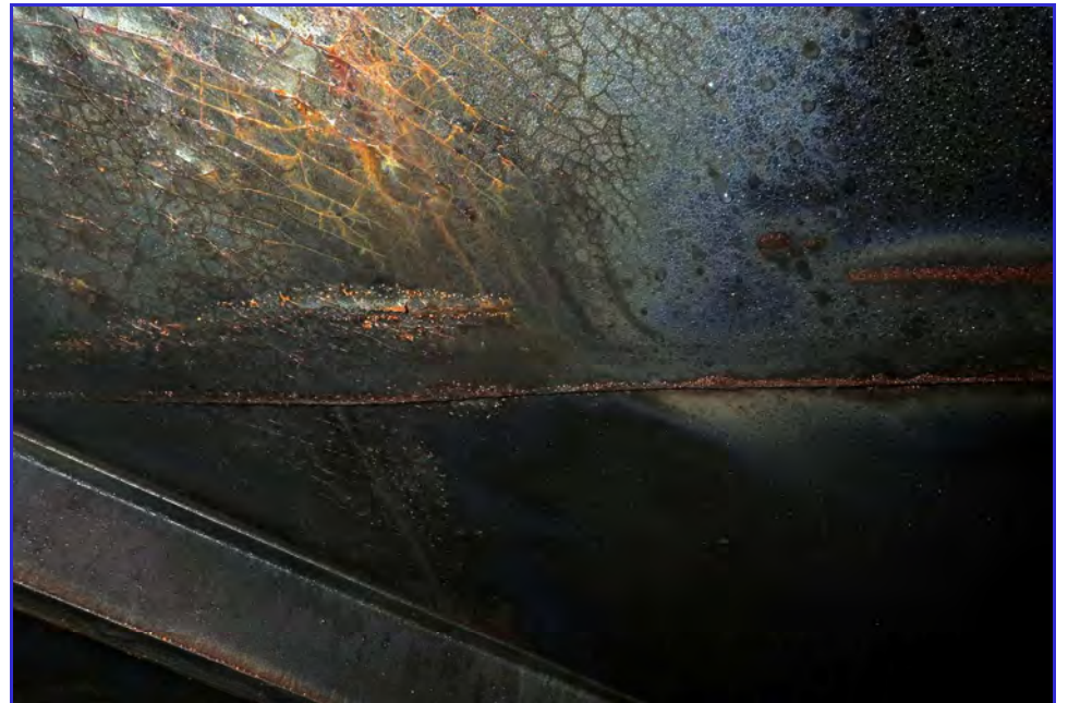
INTERIOR - Calaveras Public Utility District - Clear Well Tank - Maintenance Inspection -051
