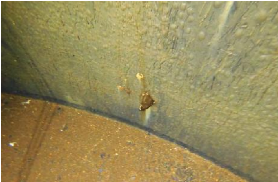
Figure 9-8. Example of Paloma Tank Interior Floor and Shell
