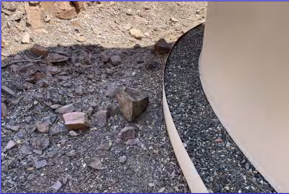
EXTERIOR - CPUD - Golden Hills - Maintenance Inspection -056
