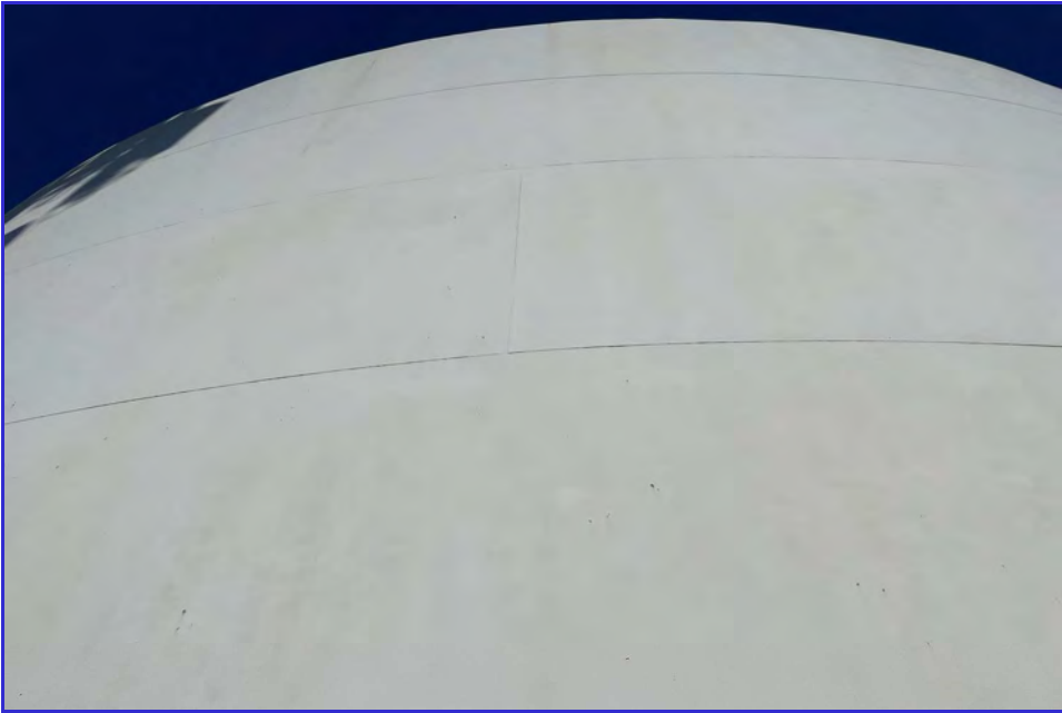
EXTERIOR - CPUD - San Andreas Reservoir - Maintenance Inspection -184
