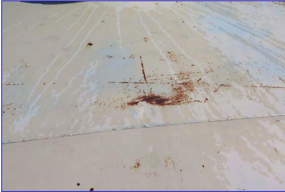
EXTERIOR - Calaveras Public Utility District - Clear Well Tank - Maintenance Inspection -044
