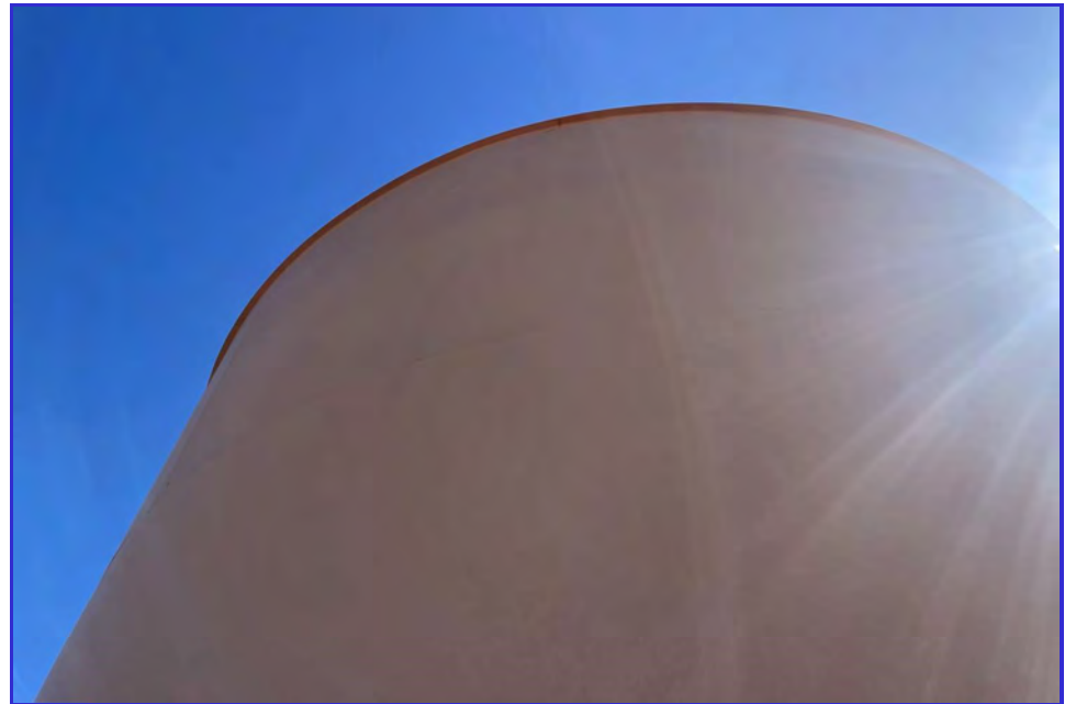
EXTERIOR - CPUD - Paloma Reservoir - Maintenance Inspection -039
