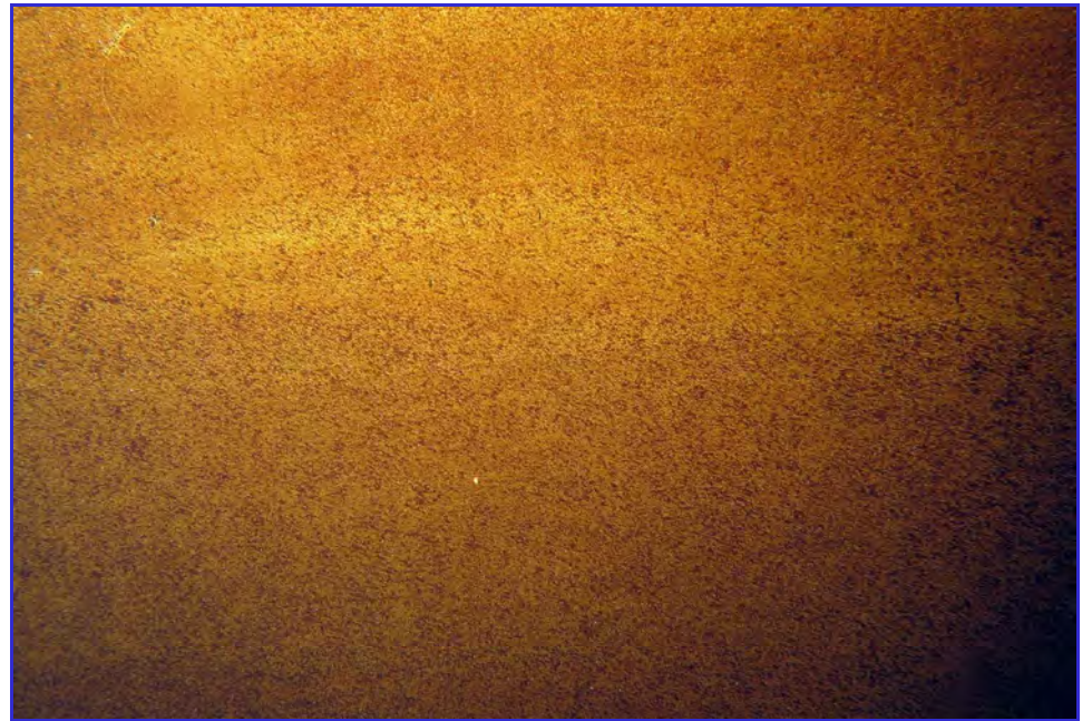
INTERIOR - Calaveras Public Utility District - Clear Well Tank - Maintenance Inspection -083
