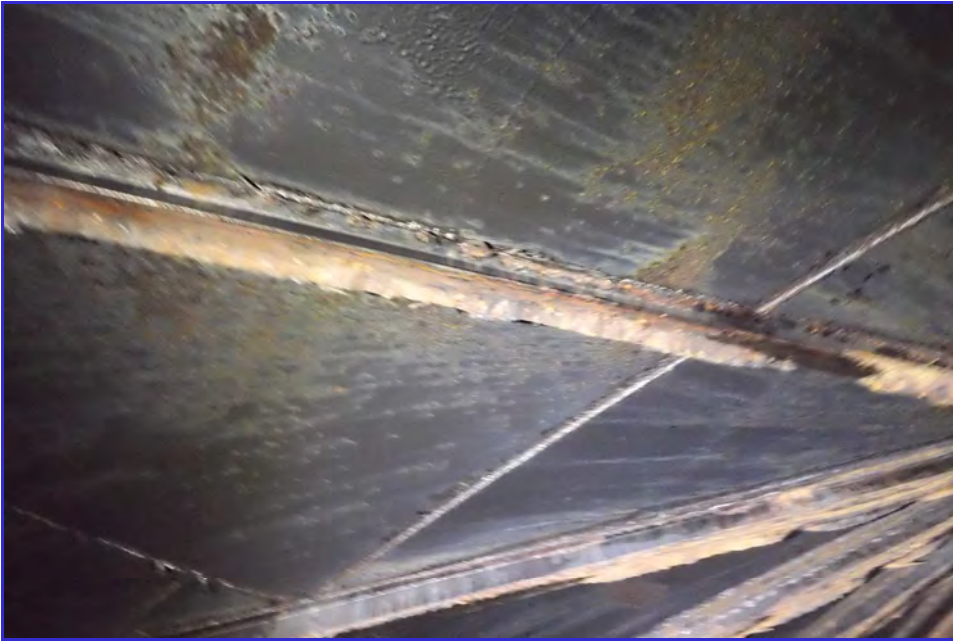
INTERIOR - CPUD - Paloma Reservoir - Maintenance Inspection -012
