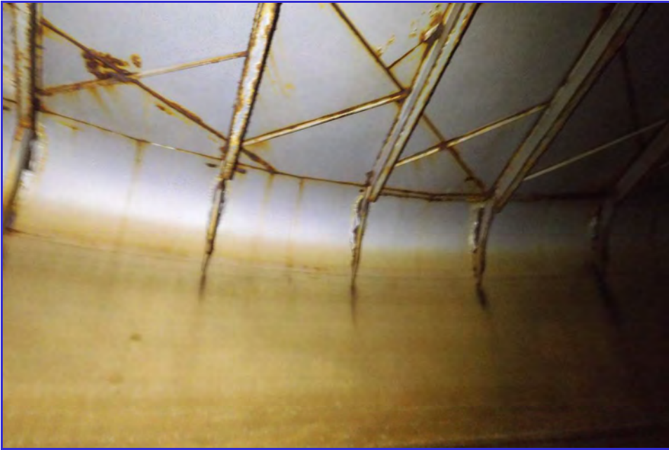
INTERIOR - CPUD - Mokelumne Hill Reservoir - Maintenance Inspection -040
