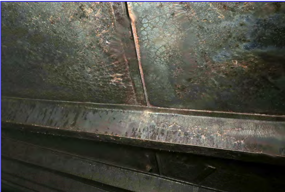
INTERIOR - Calaveras Public Utility District - Clear Well Tank - Maintenance Inspection -046
