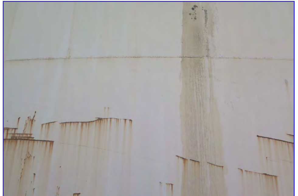
EXTERIOR - Calaveras Public Utility District - Clear Well Tank - Maintenance Inspection -095
