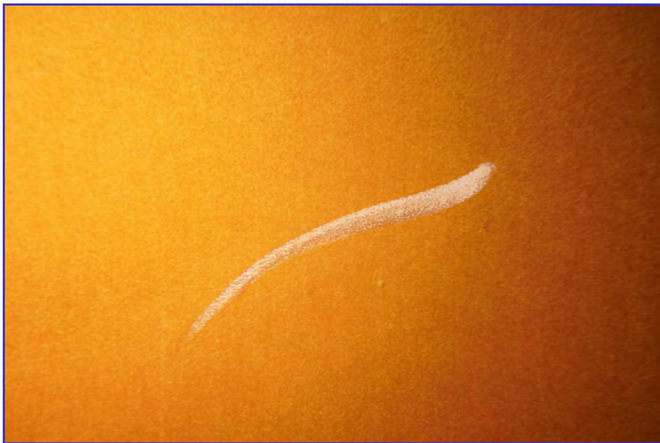
INTERIOR - CPUD - Railroad Flat Reservoir - Maintenance Inspection -098
