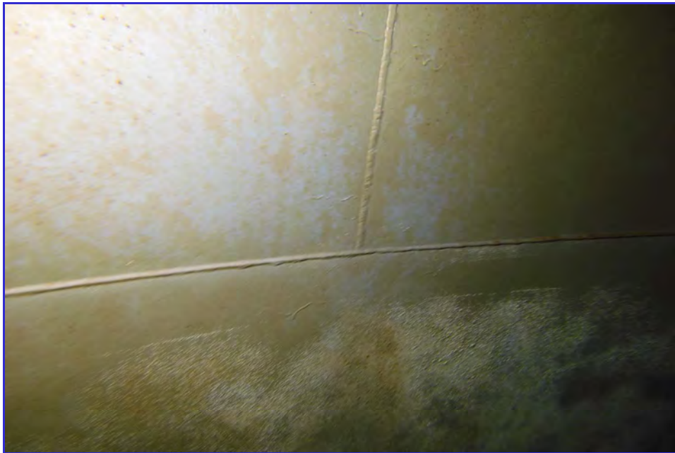
INTERIOR - CPUD - Mokelumne Hill Reservoir - Maintenance Inspection -074
