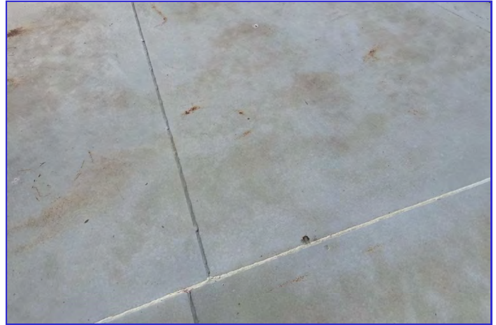
EXTERIOR - CPUD - San Andreas Reservoir - Maintenance Inspection -029
