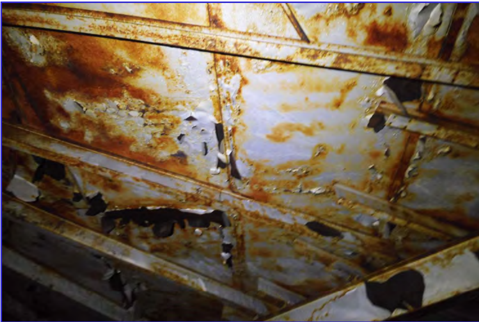
INTERIOR - CPUD - San Andaras Reservoir - Maintenance Inspection -074
