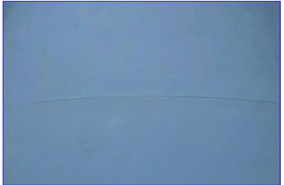
EXTERIOR - CPUD - Railroad Flat Reservoir - Maintenance Inspection -051
