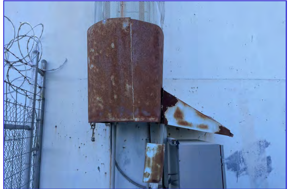
EXTERIOR - CPUD - San Andreas Reservoir - Maintenance Inspection -101
