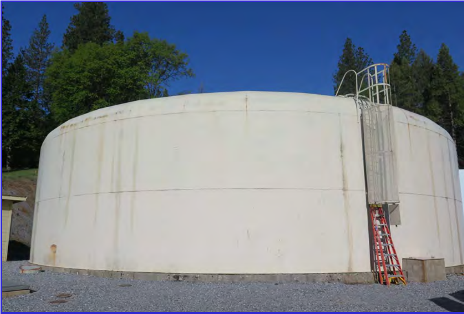
EXTERIOR - Calaveras Public Utility District - Clear Well Tank - Maintenance Inspection
