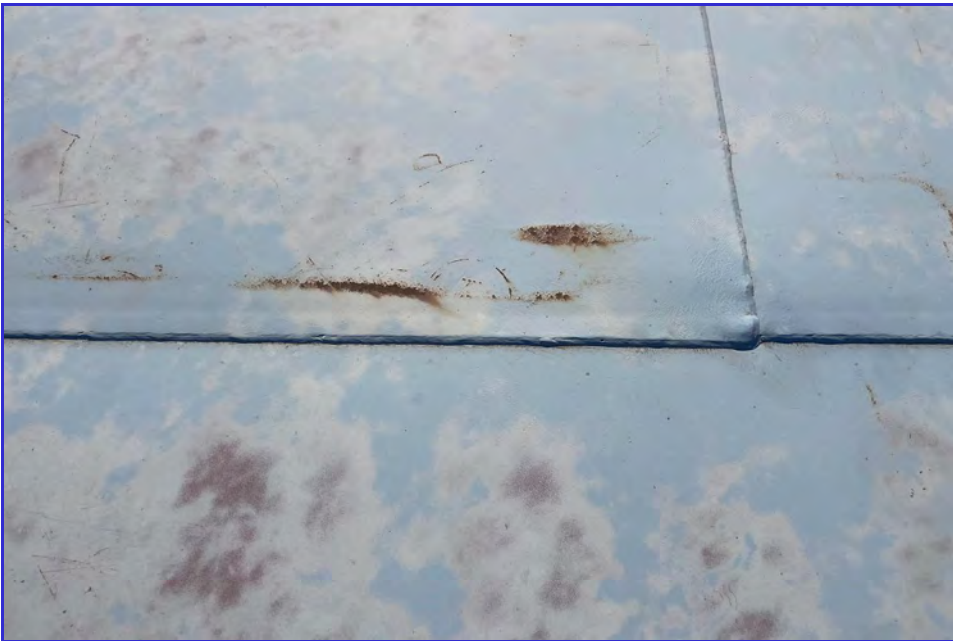
EXTERIOR - CPUD - Mokelumne Reservoir - Maintenance Inspection -022
