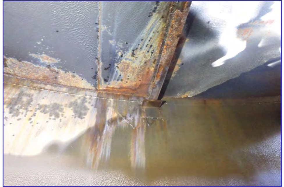
INTERIOR - CPUD - Paloma Reservoir - Maintenance Inspection -045
