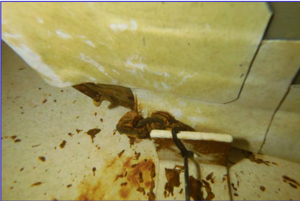
INTERIOR - CPUD - Railroad Flat Reservoir - Maintenance Inspection -146
