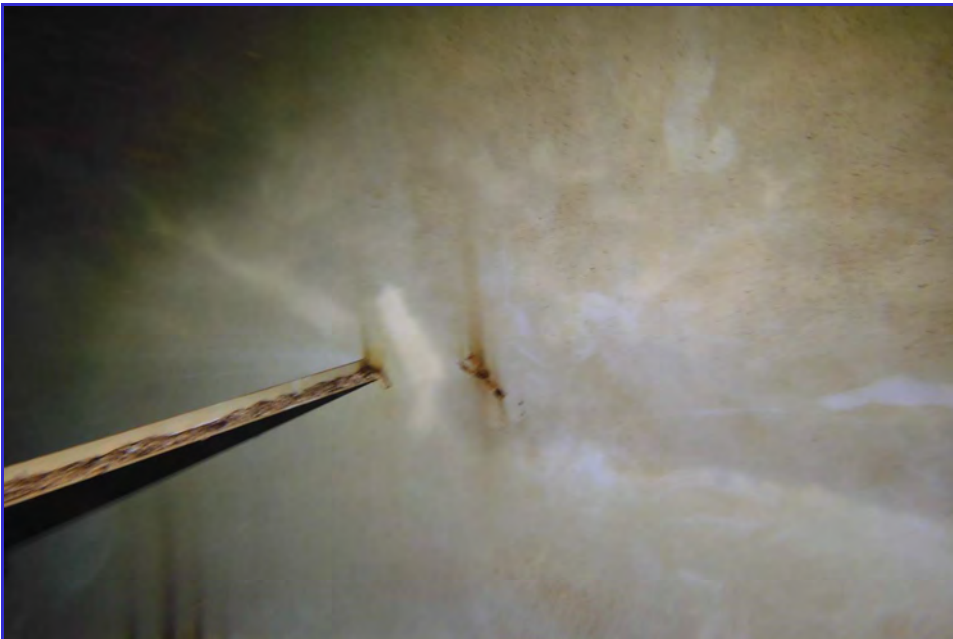
INTERIOR - CPUD - Mokelumne Hill Reservoir - Maintenance Inspection -066
