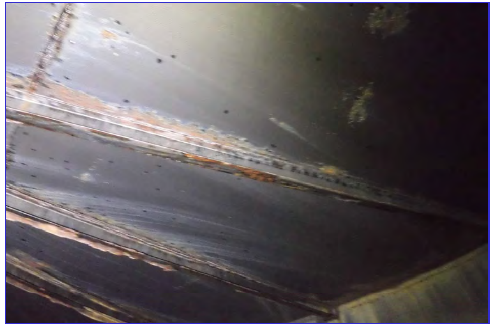
INTERIOR - CPUD - Paloma Reservoir - Maintenance Inspection -035
