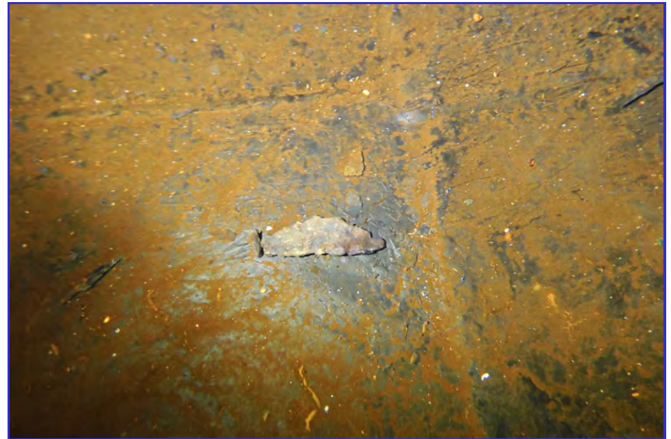
INTERIOR - CPUD - Paloma Reservoir - Maintenance Inspection -111
