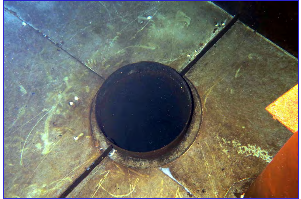
INTERIOR - Calaveras Public Utility District - Clear Well Tank - Maintenance Inspection -061
