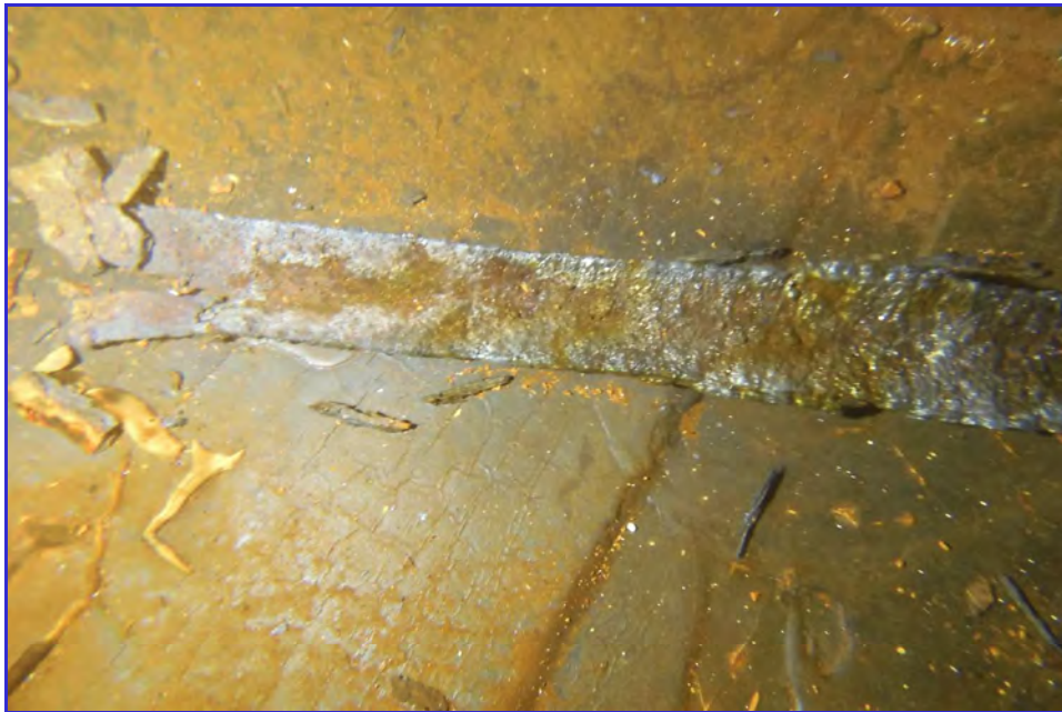
INTERIOR - CPUD - Paloma Reservoir - Maintenance Inspection -122
