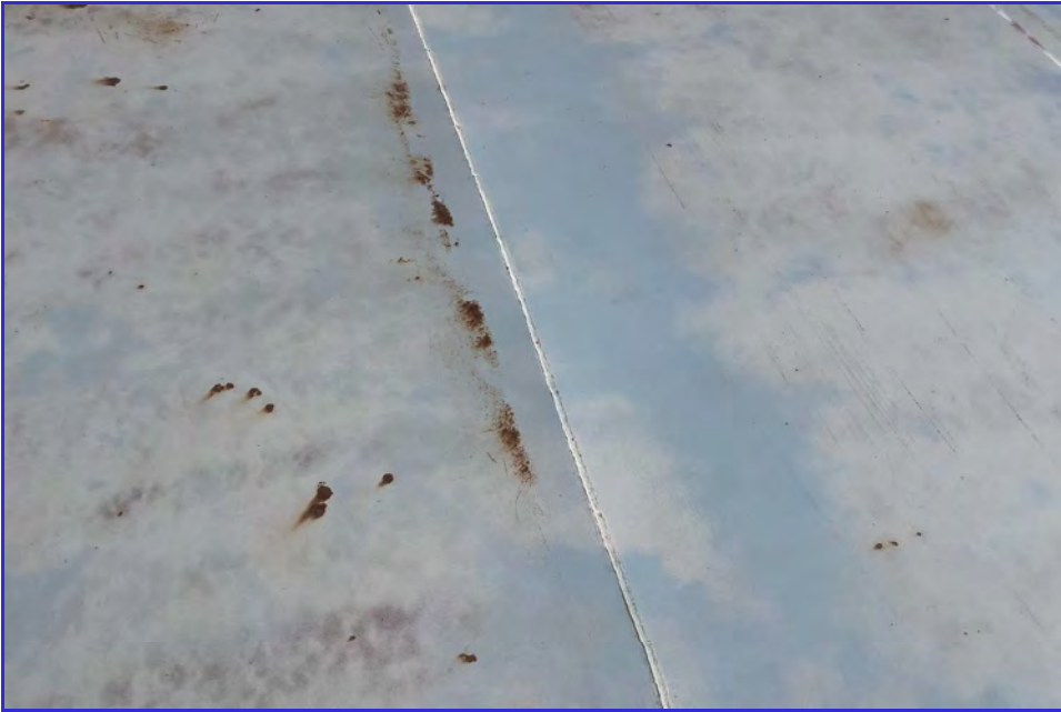
EXTERIOR - CPUD - Mokelumne Reservoir - Maintenance Inspection -016
