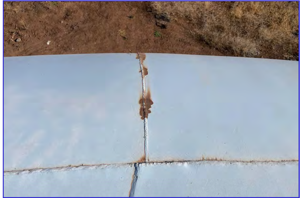
EXTERIOR - CPUD - Mokelumne Reservoir - Maintenance Inspection -005
