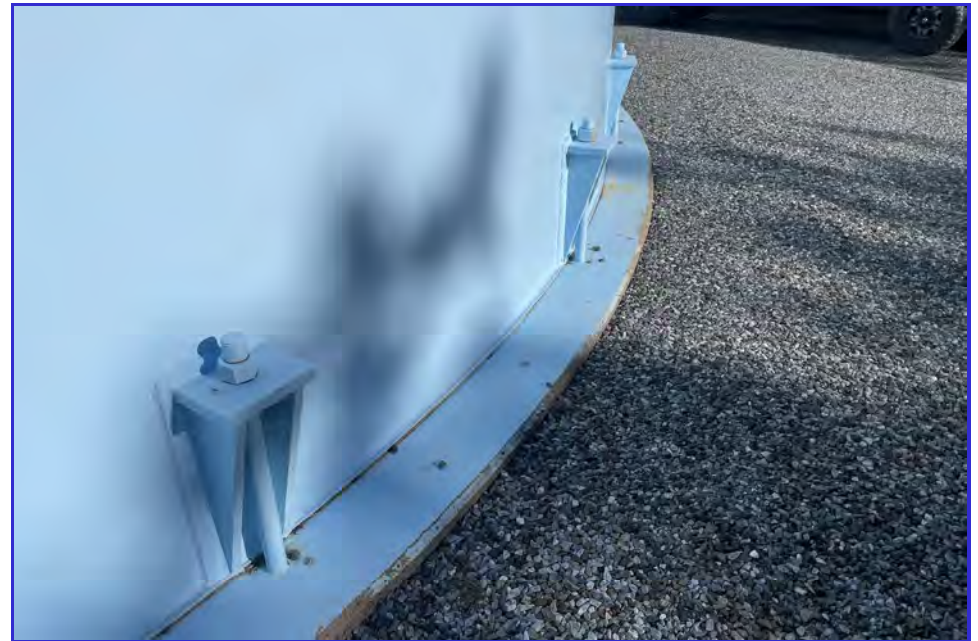
EXTERIOR - CPUD - Railroad Flat Reservoir - Maintenance Inspection -087
