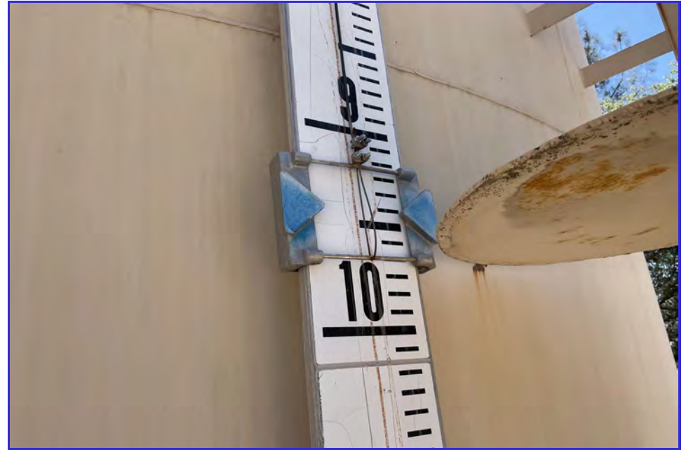
EXTERIOR - CPUD - Golden Hills - Maintenance Inspection -061
