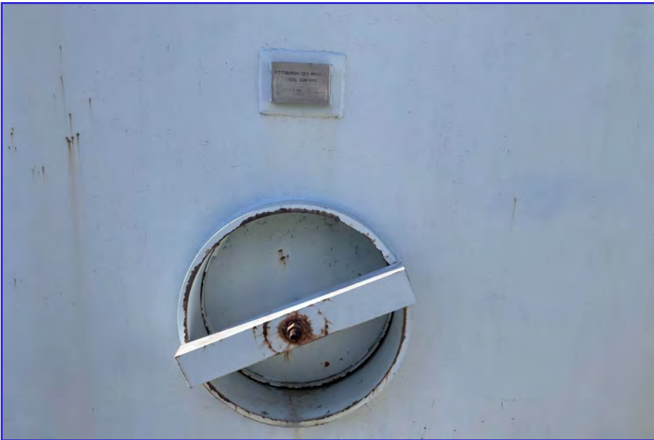
EXTERIOR - CPUD - Mokelumne Reservoir - Maintenance Inspection -178
