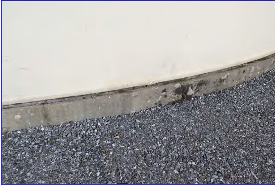
EXTERIOR - Calaveras Public Utility District - Clear Well Tank - Maintenance Inspection -064
