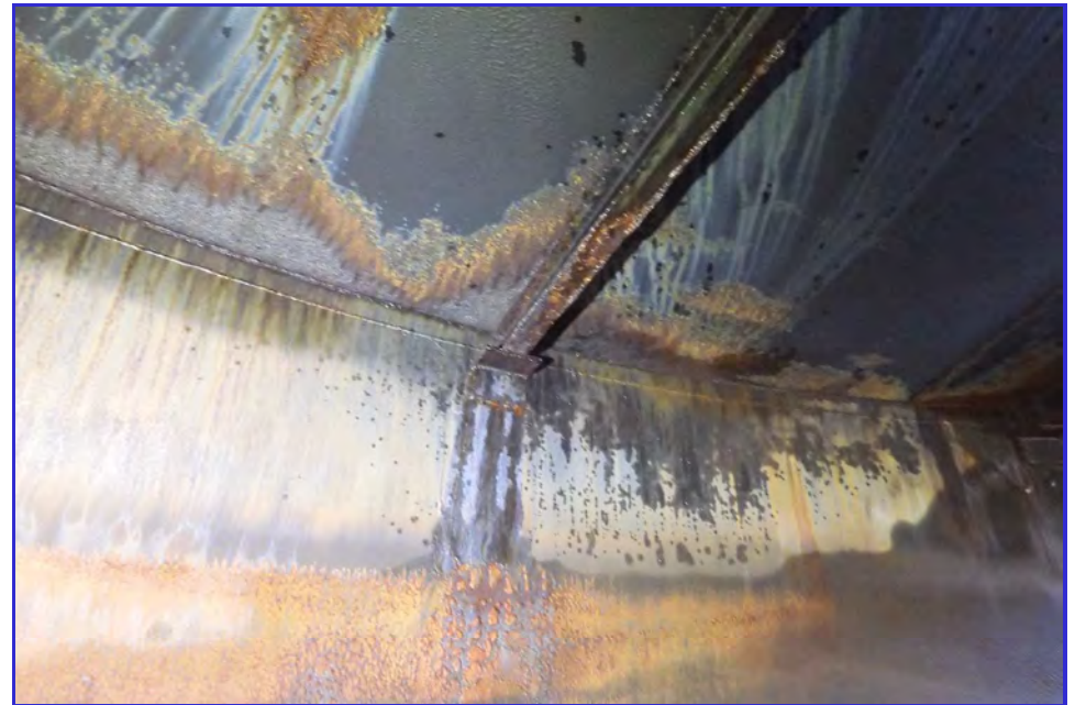
INTERIOR - CPUD - Paloma Reservoir - Maintenance Inspection -039
