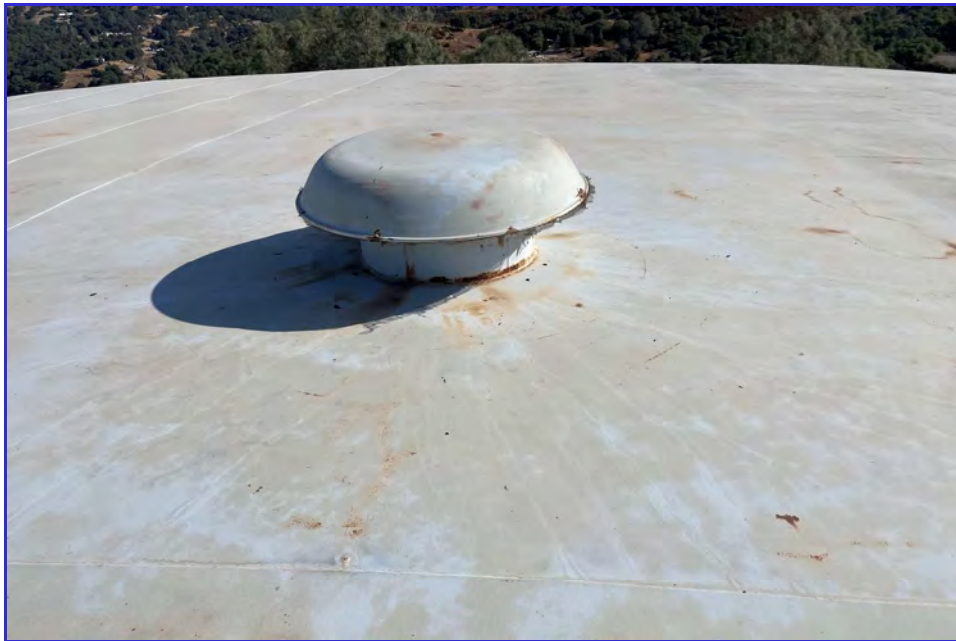
EXTERIOR - CPUD - San Andreas Reservoir - Maintenance Inspection -086
