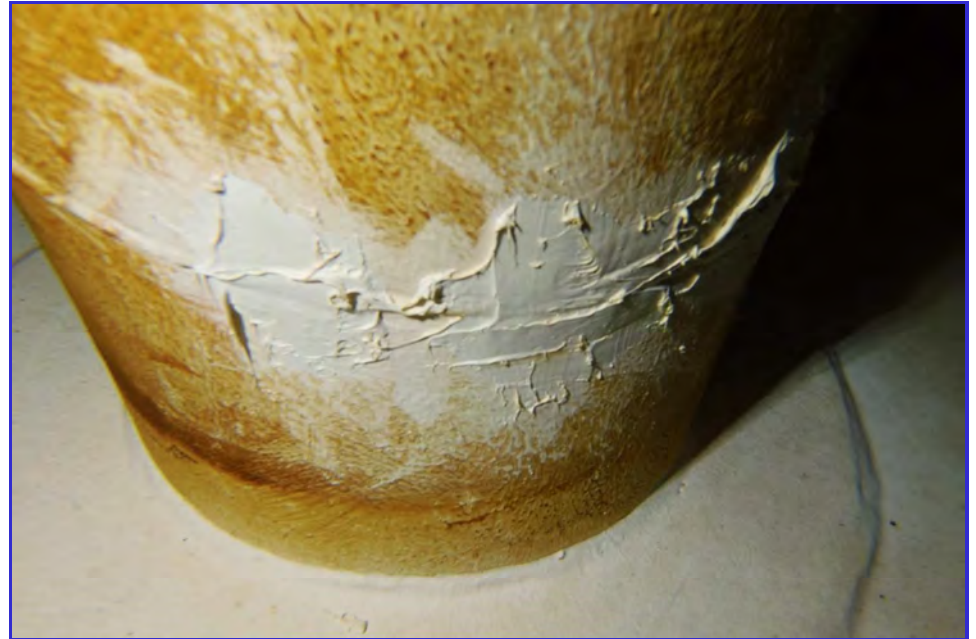
INTERIOR - CPUD - Railroad Flat Reservoir - Maintenance Inspection -105
