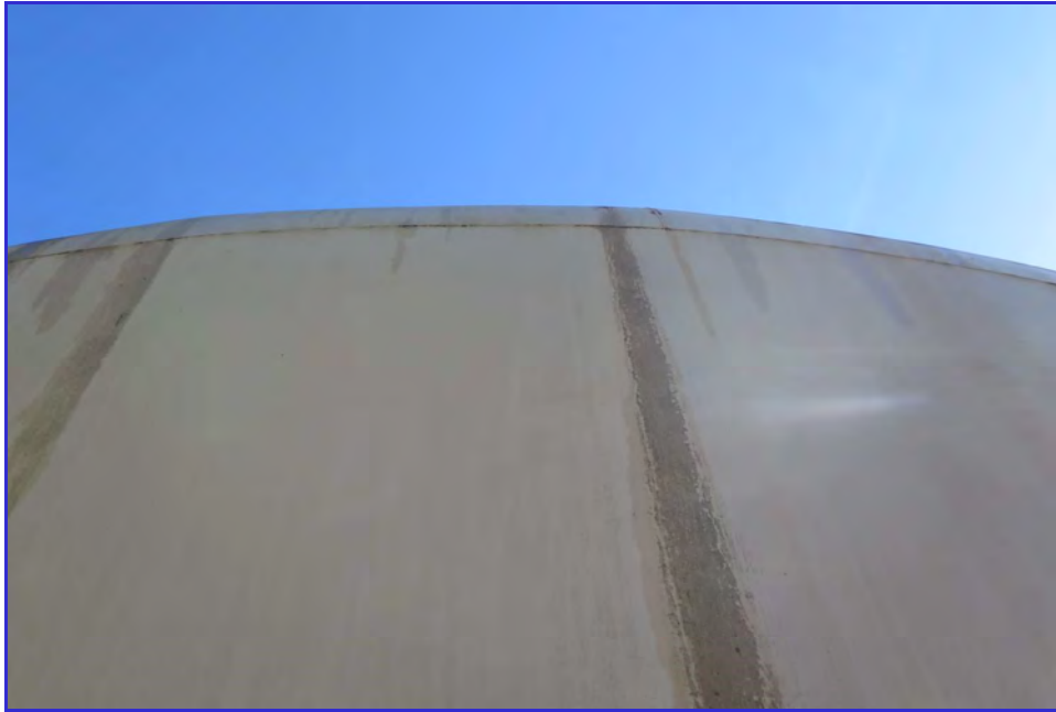
EXTERIOR - Calaveras Public Utility District - Clear Well Tank - Maintenance Inspection -088
