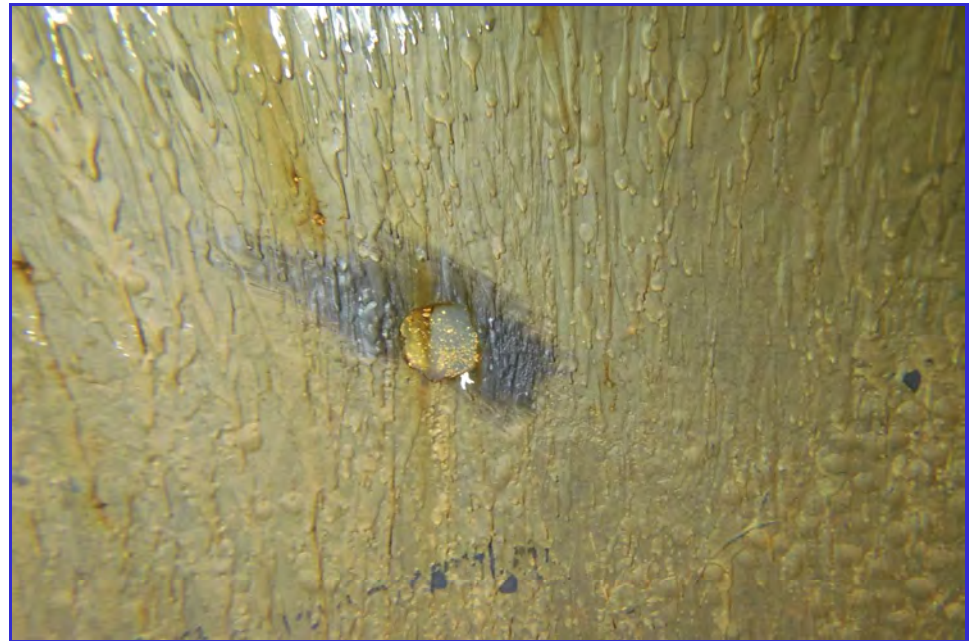
INTERIOR - CPUD - Paloma Reservoir - Maintenance Inspection -099
