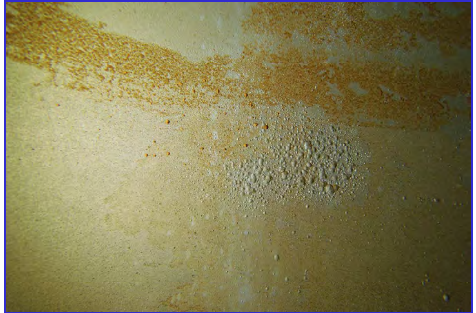
INTERIOR - CPUD - San Andaras Reservoir - Maintenance Inspection -117
