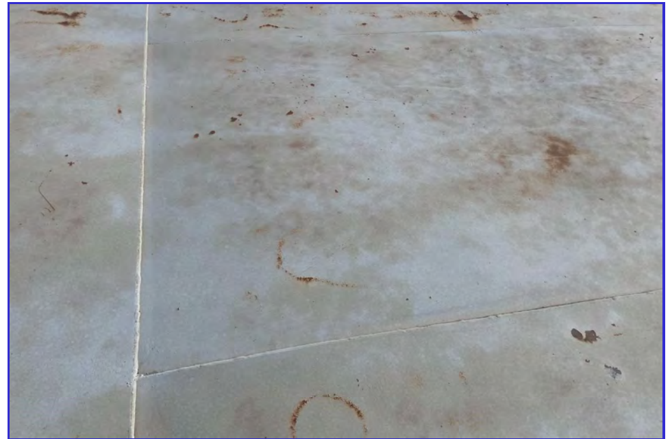
EXTERIOR - CPUD - San Andreas Reservoir - Maintenance Inspection -019
