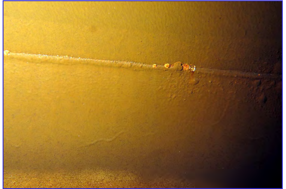
INTERIOR - Calaveras Public Utility District - Clear Well Tank - Maintenance Inspection -069
