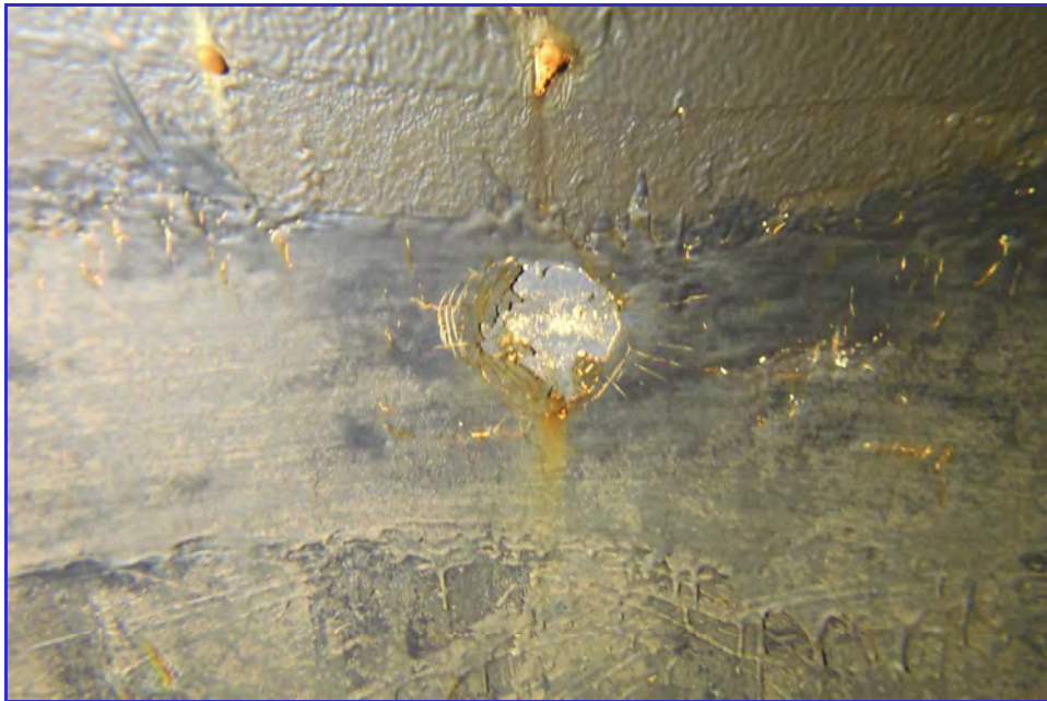
INTERIOR - CPUD - Paloma Reservoir - Maintenance Inspection -058
