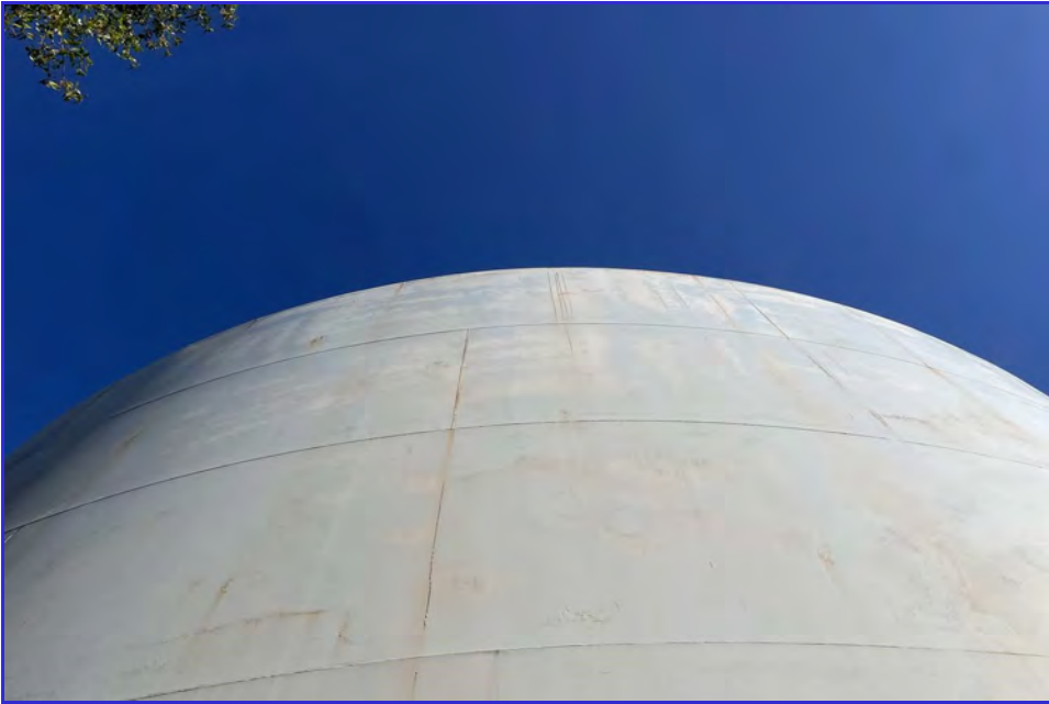
EXTERIOR - CPUD - Mokelumne Reservoir - Maintenance Inspection -104
