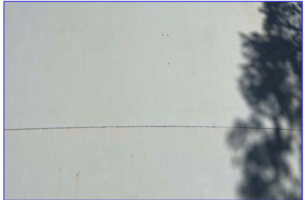
EXTERIOR - CPUD - Mokelumne Reservoir - Maintenance Inspection -099
