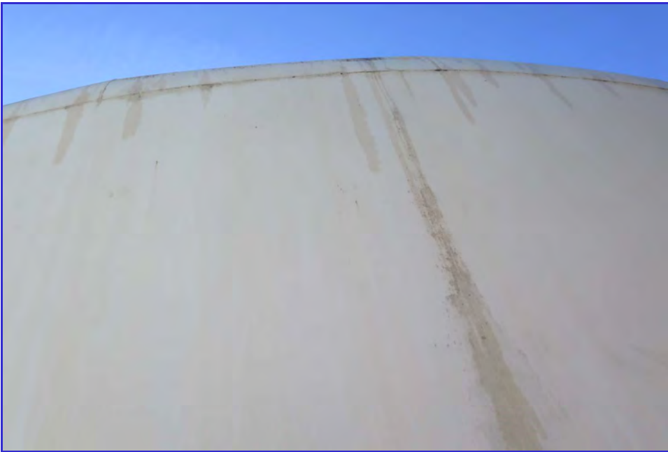
EXTERIOR - Calaveras Public Utility District - Clear Well Tank - Maintenance Inspection -106
