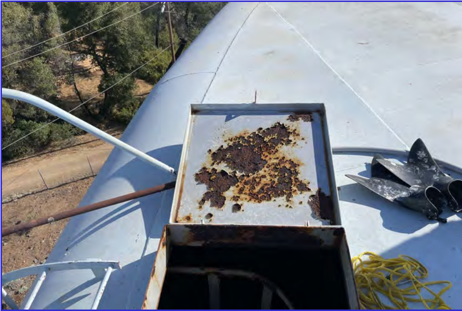
EXTERIOR - CPUD - San Andreas Reservoir - Maintenance Inspection -004
