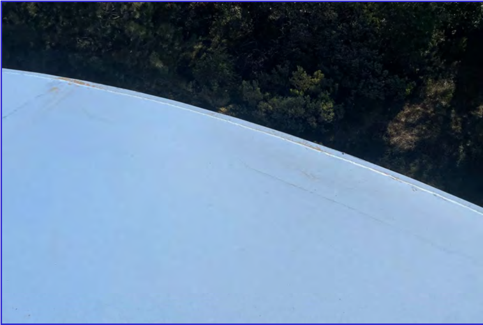
EXTERIOR - CPUD - Railroad Flat Reservoir - Maintenance Inspection -016
