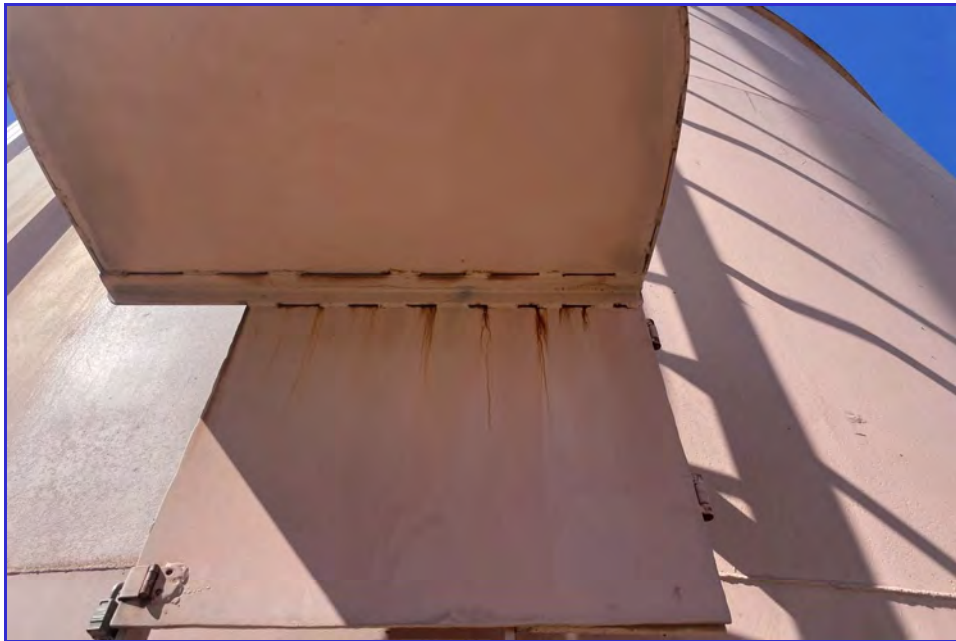
EXTERIOR - CPUD - Paloma Reservoir - Maintenance Inspection -058
