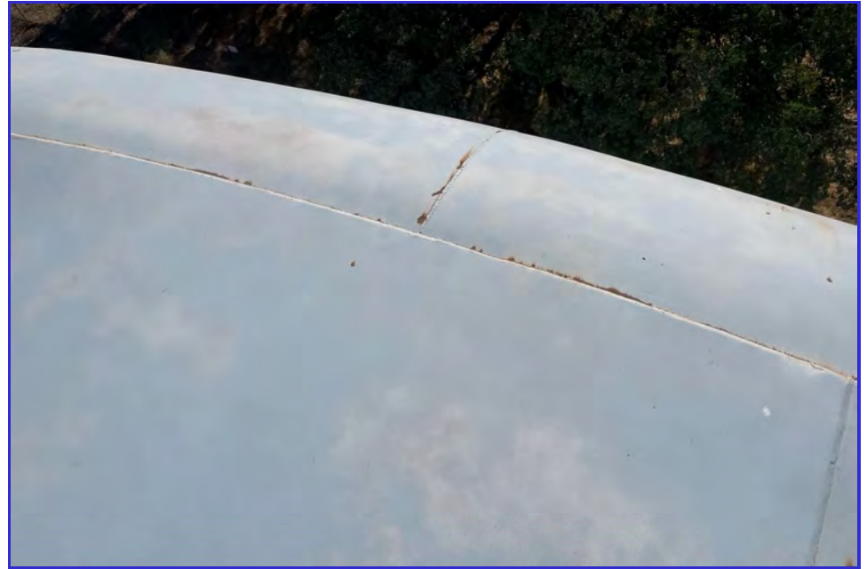
EXTERIOR - CPUD - Mokelumne Reservoir - Maintenance Inspection -057
