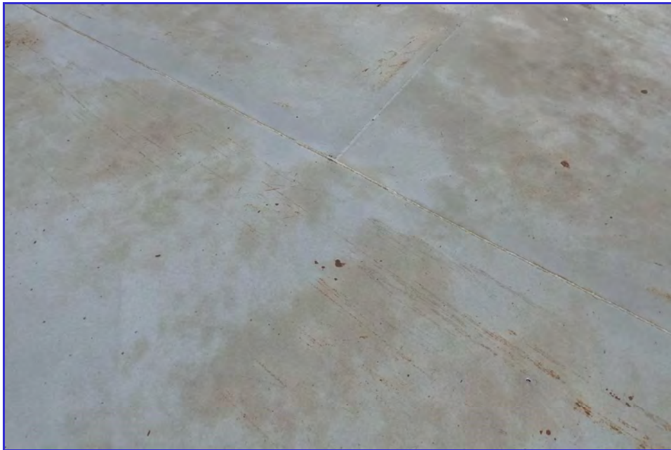
EXTERIOR - CPUD - San Andreas Reservoir - Maintenance Inspection -050
