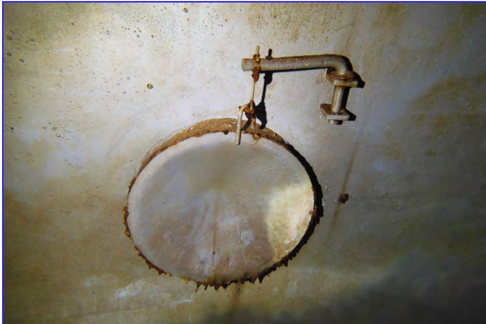
INTERIOR - CPUD - San Andaras Reservoir - Maintenance Inspection -168
