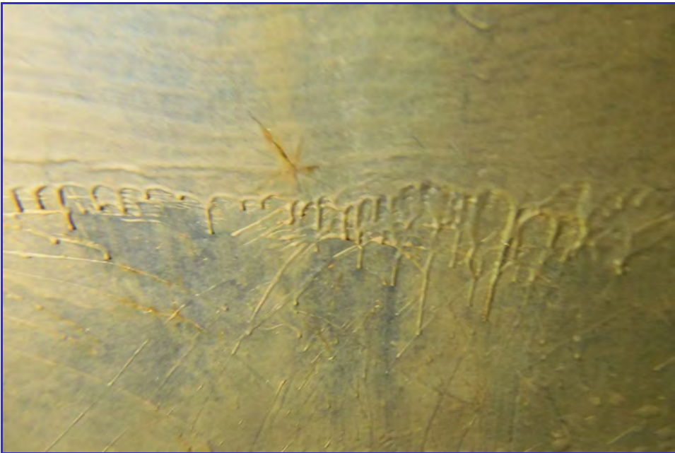
INTERIOR - CPUD - Paloma Reservoir - Maintenance Inspection -070
