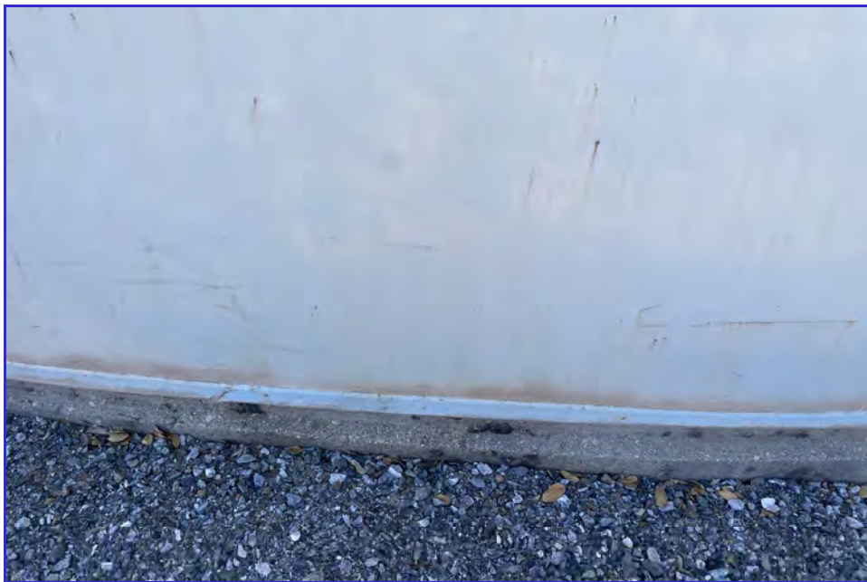
EXTERIOR - CPUD - Mokelumne Reservoir - Maintenance Inspection -110
