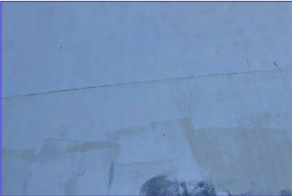
EXTERIOR - CPUD - San Andreas Reservoir - Maintenance Inspection -162
