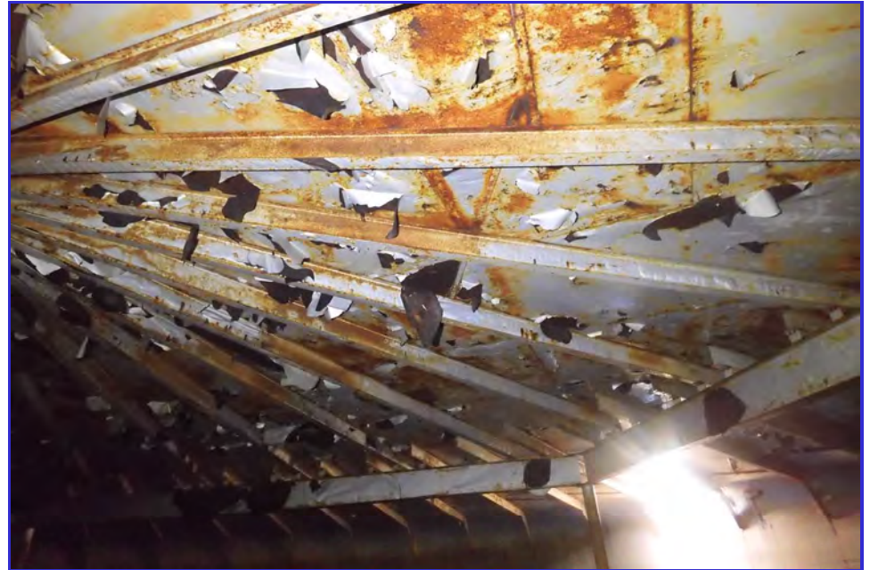
INTERIOR - CPUD - San Andaras Reservoir - Maintenance Inspection -085
