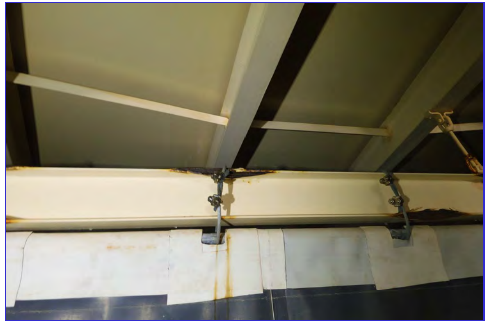
INTERIOR - CPUD - Railroad Flat Reservoir - Maintenance Inspection -043
