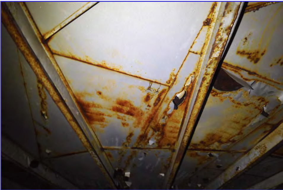
INTERIOR - CPUD - San Andaras Reservoir - Maintenance Inspection -038
