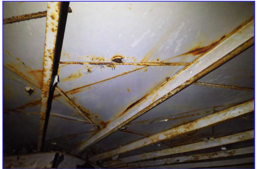
INTERIOR - CPUD - San Andaras Reservoir - Maintenance Inspection -031
