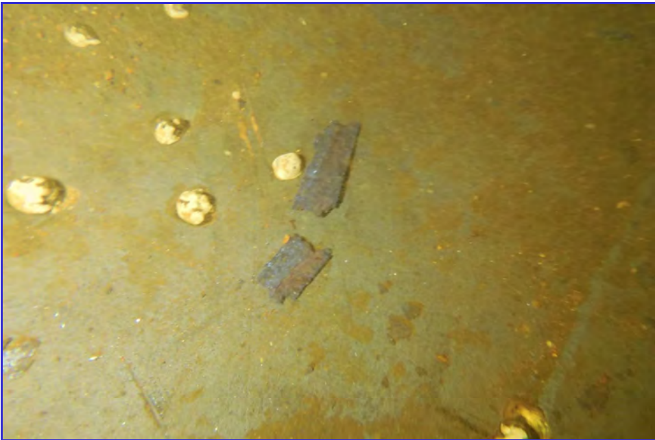
INTERIOR - CPUD - Golden Hills - Maintenance Inspection -042
