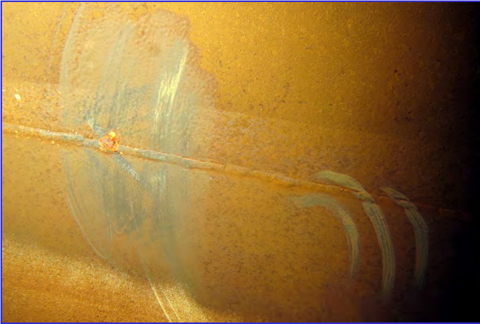
INTERIOR - Calaveras Public Utility District - Clear Well Tank - Maintenance Inspection -072
