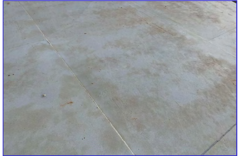
EXTERIOR - CPUD - San Andreas Reservoir - Maintenance Inspection -049
