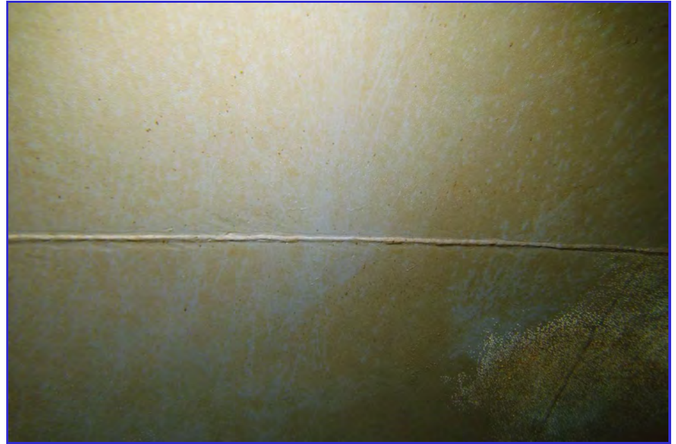
INTERIOR - CPUD - Mokelumne Hill Reservoir - Maintenance Inspection -085
