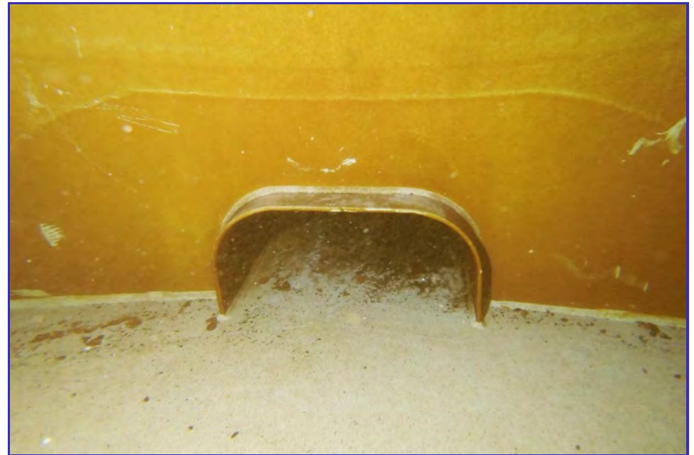
INTERIOR - CPUD - Railroad Flat Reservoir - Maintenance Inspection -087
