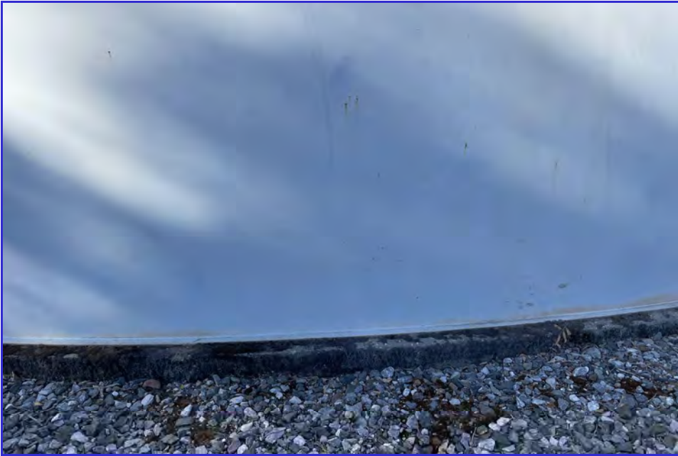
EXTERIOR - CPUD - Mokelumne Reservoir - Maintenance Inspection -176
