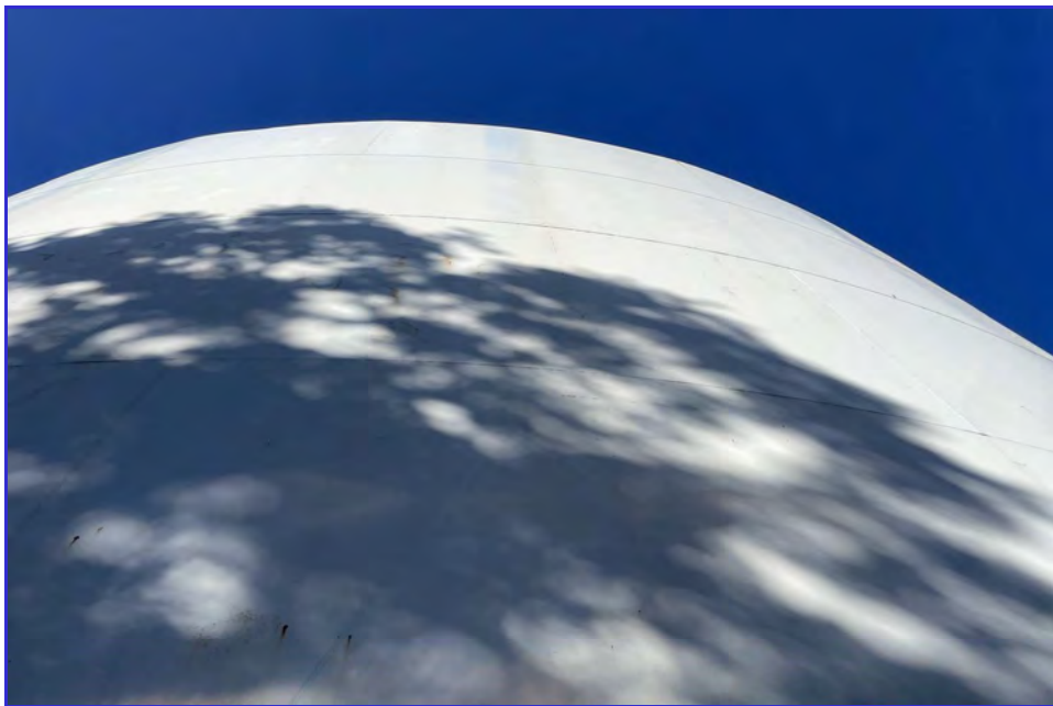
EXTERIOR - CPUD - Mokelumne Reservoir - Maintenance Inspection -094
