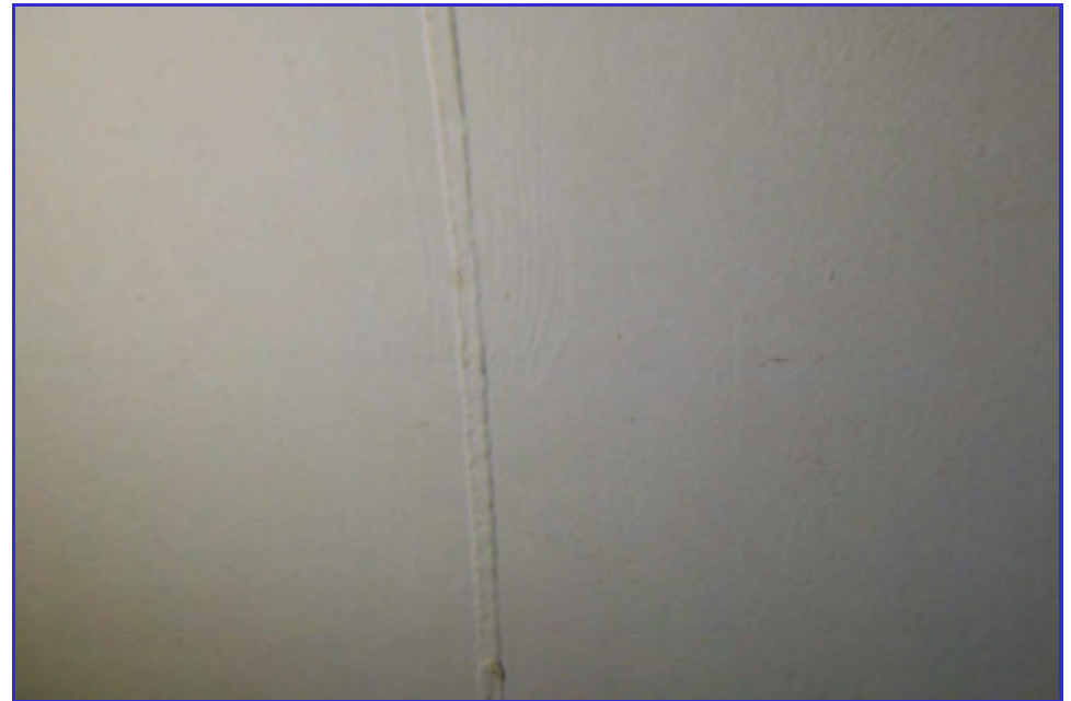
INTERIOR - CPUD - Railroad Flat Reservoir - Maintenance Inspection -067
