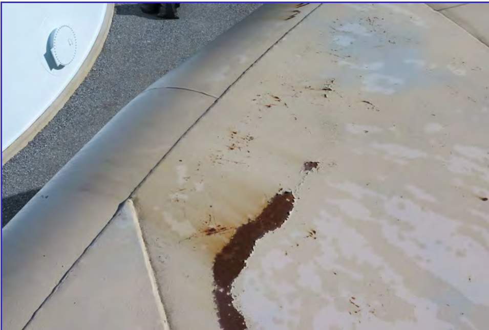
EXTERIOR - Calaveras Public Utility District - Clear Well Tank - Maintenance Inspection -014
