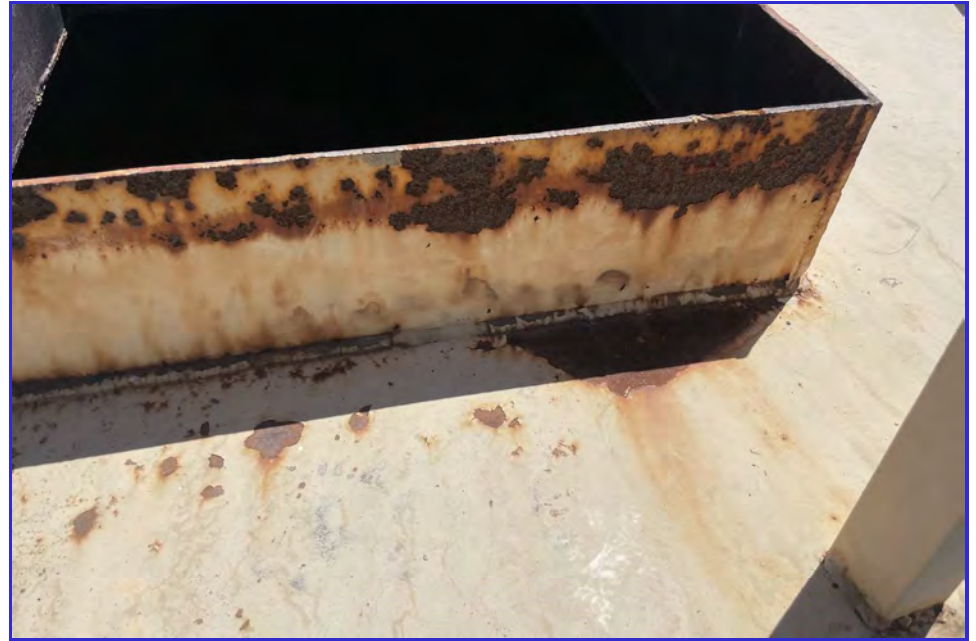
EXTERIOR - CPUD - Golden Hills - Maintenance Inspection -025
