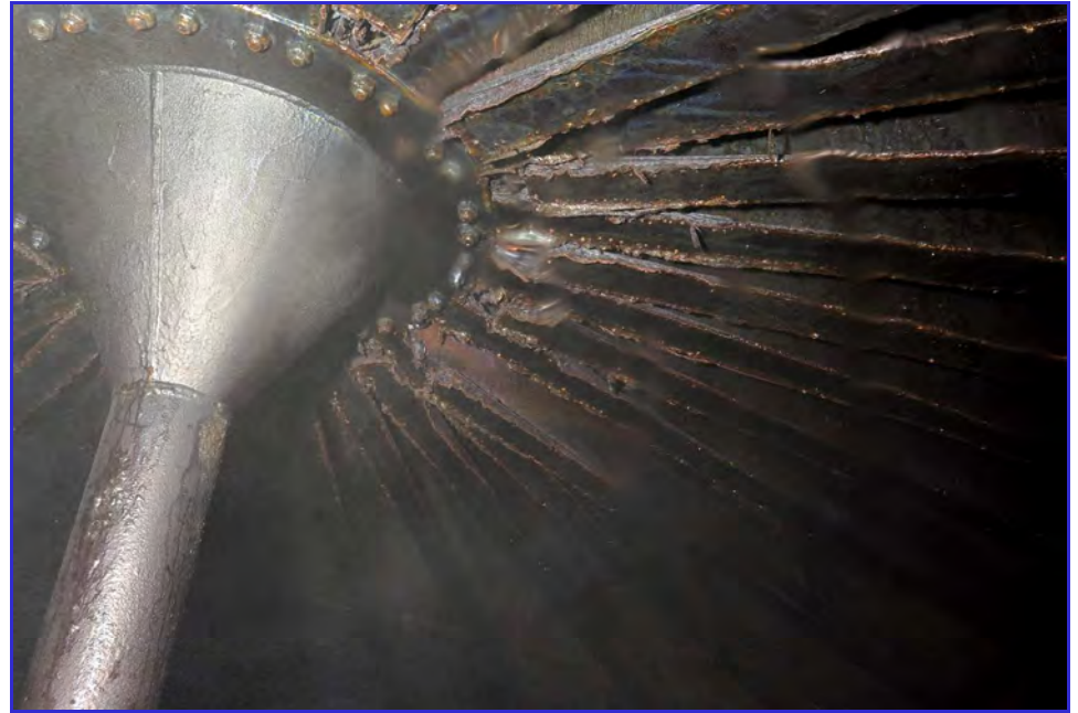
INTERIOR - Calaveras Public Utility District - Clear Well Tank - Maintenance Inspection -021
