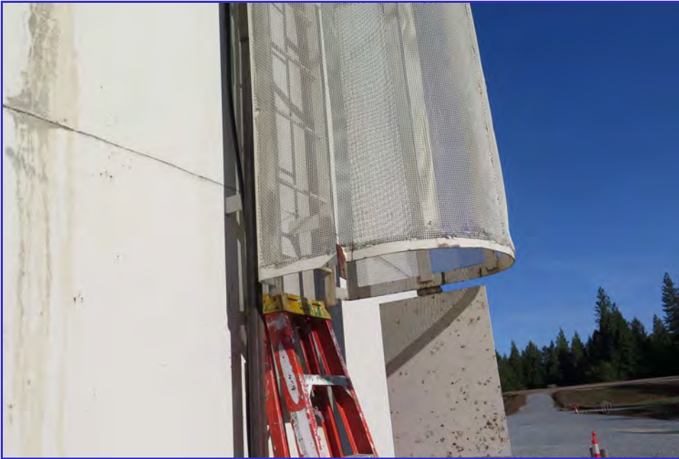
EXTERIOR - Calaveras Public Utility District - Clear Well Tank - Maintenance Inspection -054
