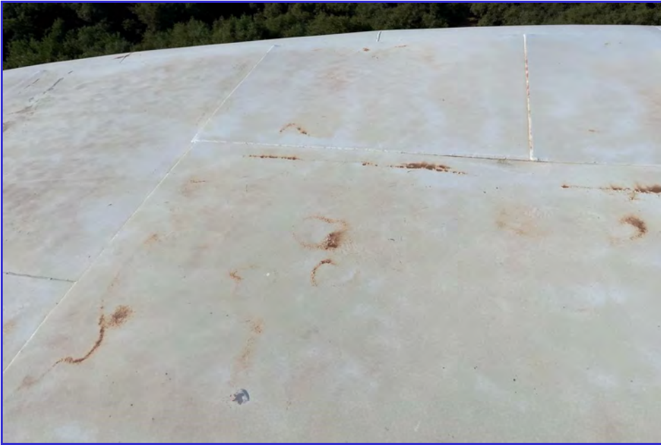
EXTERIOR - CPUD - San Andreas Reservoir - Maintenance Inspection -044
