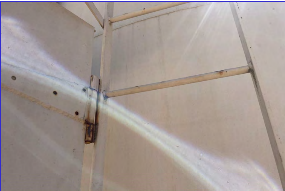
EXTERIOR - CPUD - Golden Hills - Maintenance Inspection -038
