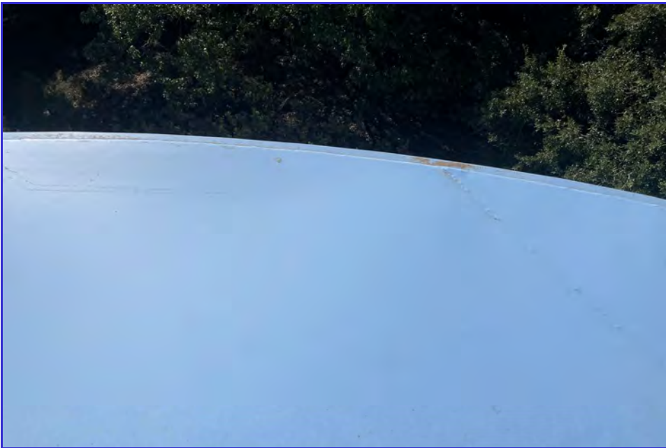
EXTERIOR - CPUD - Railroad Flat Reservoir - Maintenance Inspection -022
