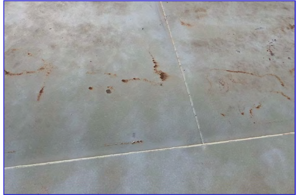
EXTERIOR - CPUD - San Andreas Reservoir - Maintenance Inspection -017
