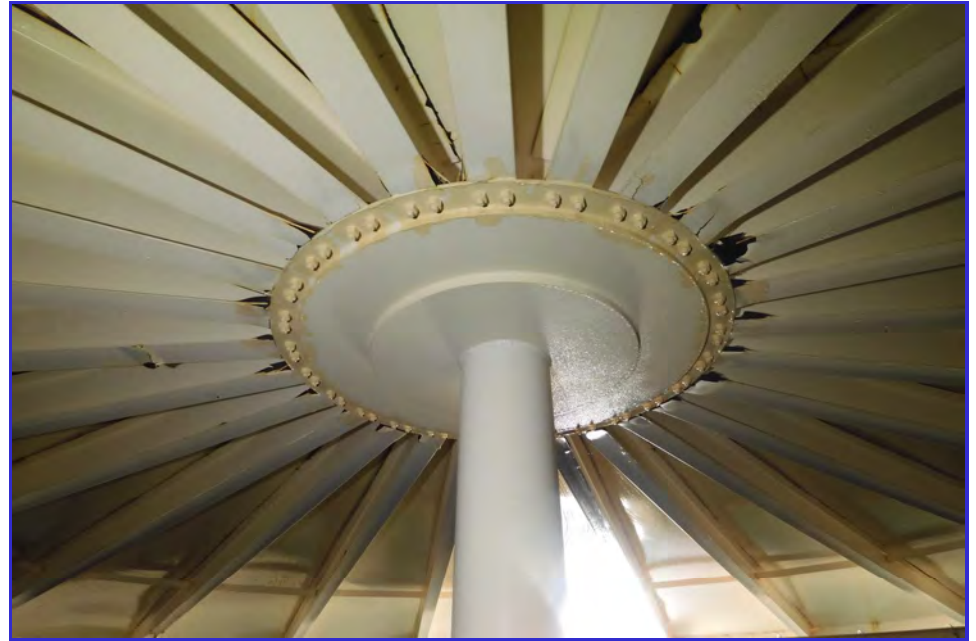
INTERIOR - CPUD - Railroad Flat Reservoir - Maintenance Inspection -041
