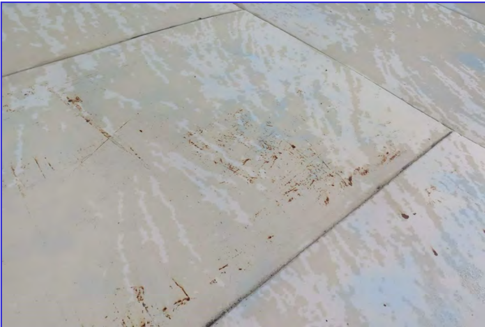
EXTERIOR - Calaveras Public Utility District - Clear Well Tank - Maintenance Inspection -050
