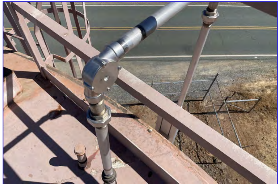
EXTERIOR - CPUD - Paloma Reservoir - Maintenance Inspection -003
