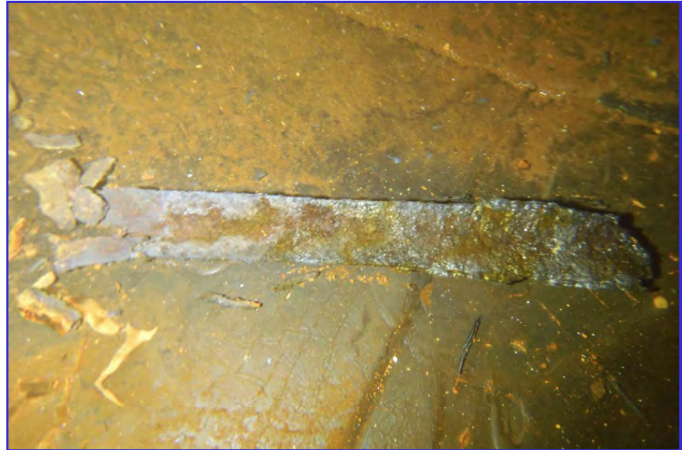
INTERIOR - CPUD - Paloma Reservoir - Maintenance Inspection -121
