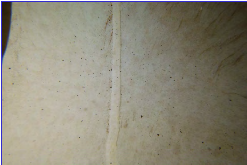
INTERIOR - CPUD - Railroad Flat Reservoir - Maintenance Inspection -110
