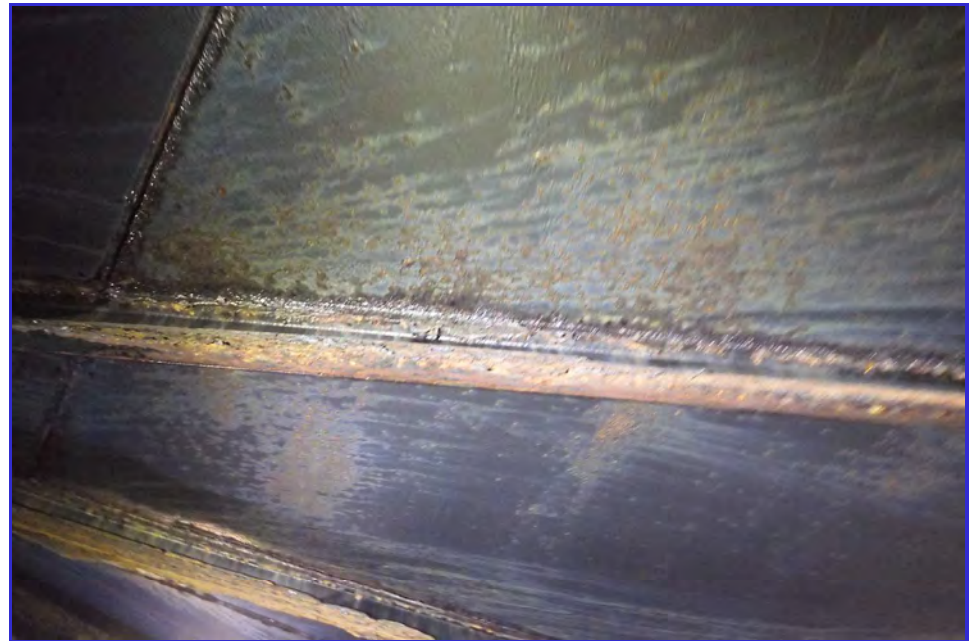
INTERIOR - CPUD - Paloma Reservoir - Maintenance Inspection -015
