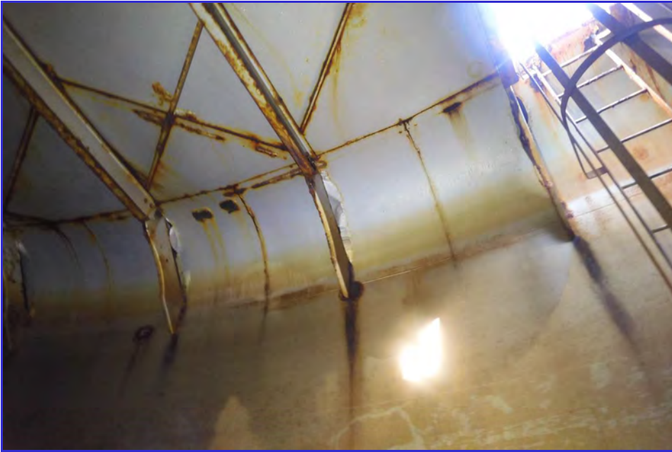
INTERIOR - CPUD - Mokelumne Hill Reservoir - Maintenance Inspection -004
