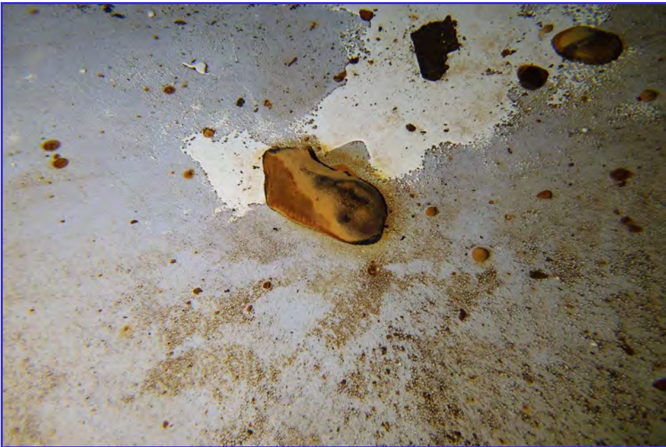
INTERIOR - CPUD - Mokelumne Hill Reservoir - Maintenance Inspection -166
