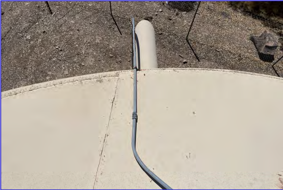
EXTERIOR - CPUD - Golden Hills - Maintenance Inspection -014
