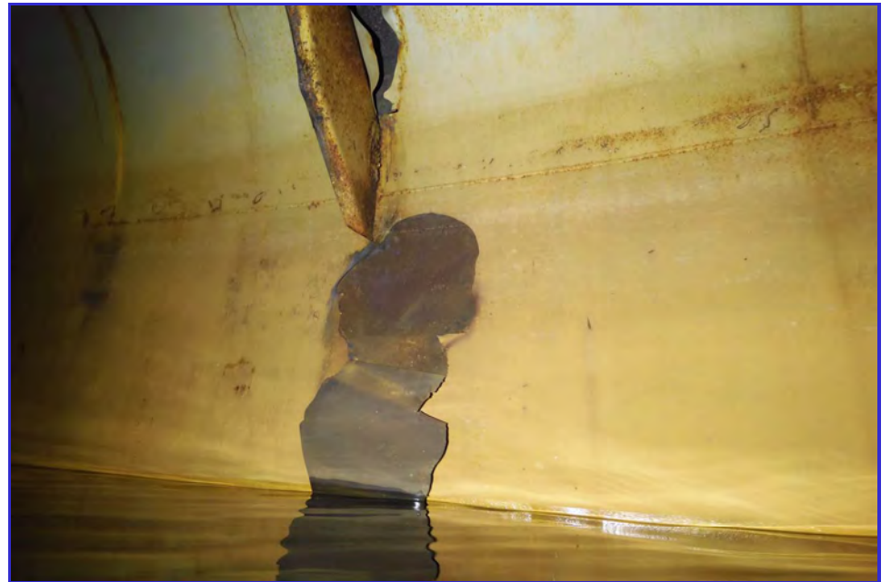
INTERIOR - CPUD - San Andaras Reservoir - Maintenance Inspection -099
