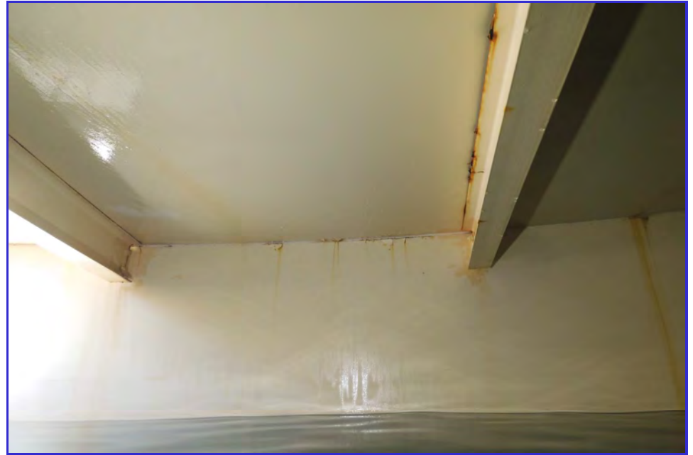
INTERIOR - CPUD - Railroad Flat Reservoir - Maintenance Inspection -009
