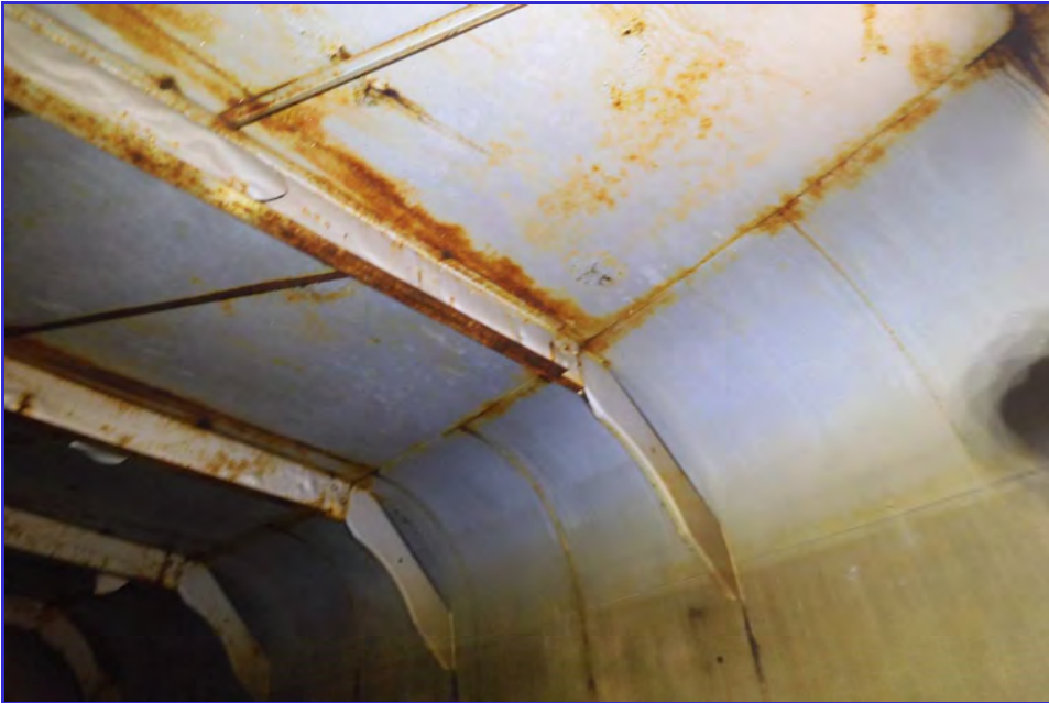
INTERIOR - CPUD - San Andaras Reservoir - Maintenance Inspection -004
