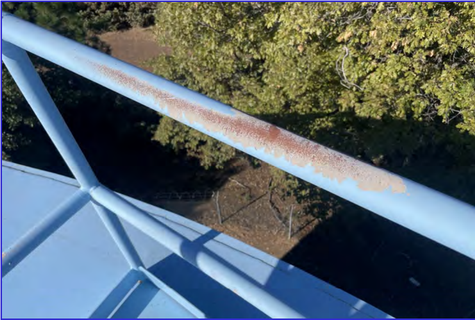
EXTERIOR - CPUD - Railroad Flat Reservoir - Maintenance Inspection -004
