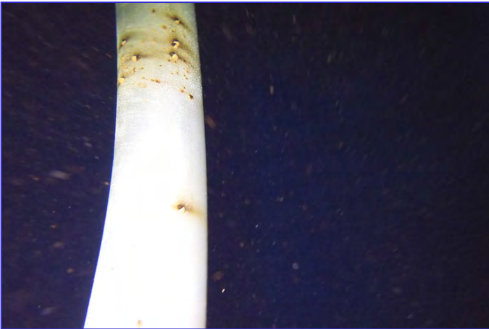
INTERIOR - CPUD - San Andaras Reservoir - Maintenance Inspection -150
