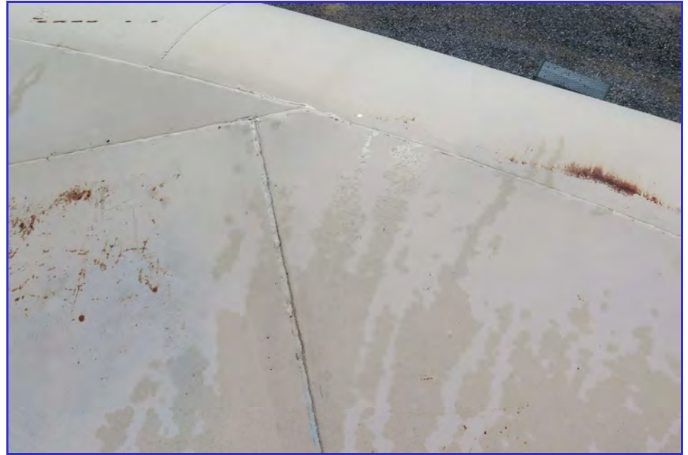
EXTERIOR - Calaveras Public Utility District - Clear Well Tank - Maintenance Inspection -037
