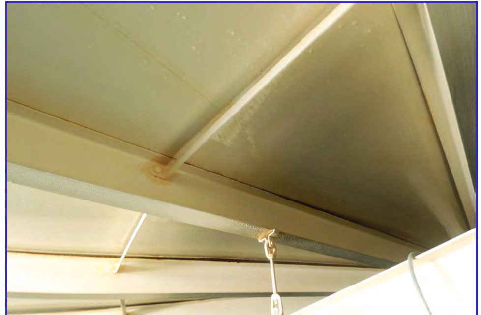
INTERIOR - CPUD - Railroad Flat Reservoir - Maintenance Inspection -019
