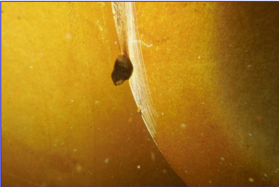
INTERIOR - CPUD - Railroad Flat Reservoir - Maintenance Inspection -122
