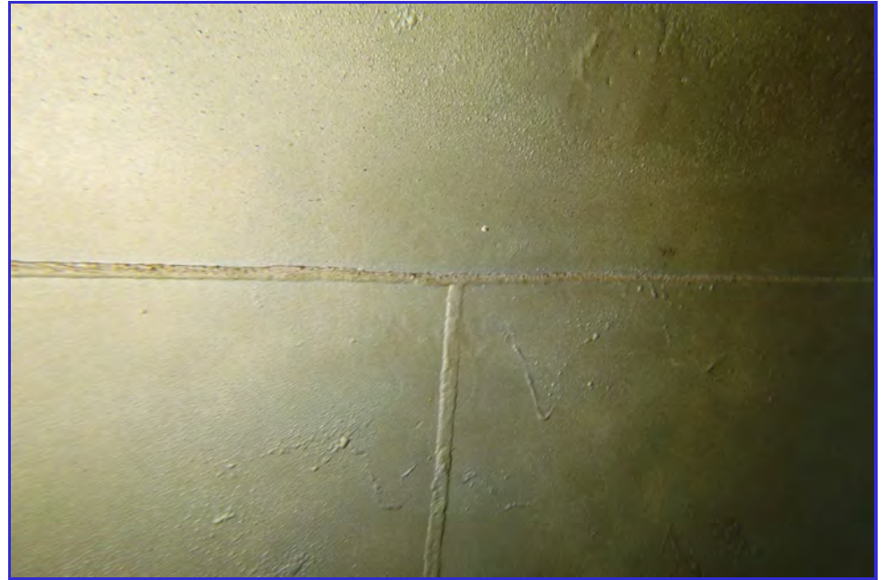
INTERIOR - CPUD - San Andaras Reservoir - Maintenance Inspection -109
