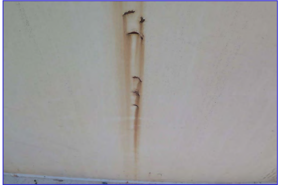
EXTERIOR - Calaveras Public Utility District - Clear Well Tank - Maintenance Inspection -085
