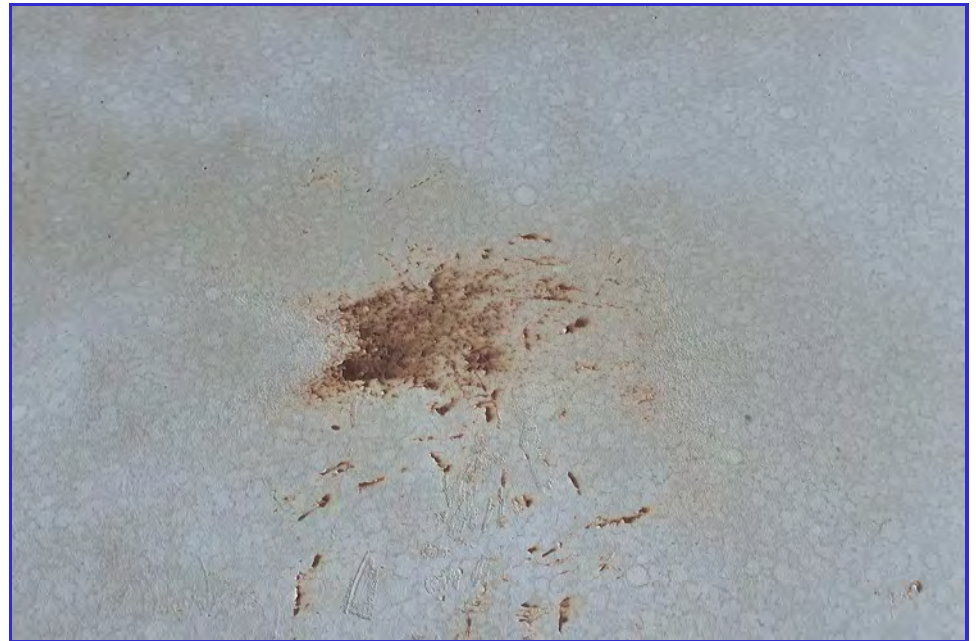
EXTERIOR - CPUD - San Andreas Reservoir - Maintenance Inspection -011
