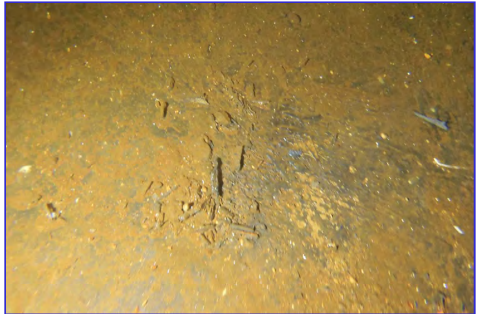
INTERIOR - CPUD - Paloma Reservoir - Maintenance Inspection -123
