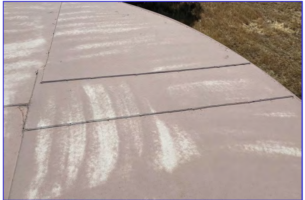
EXTERIOR - CPUD - Paloma Reservoir - Maintenance Inspection -027
