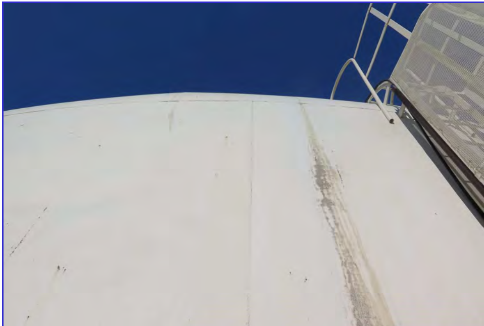
EXTERIOR - Calaveras Public Utility District - Clear Well Tank - Maintenance Inspection -058
