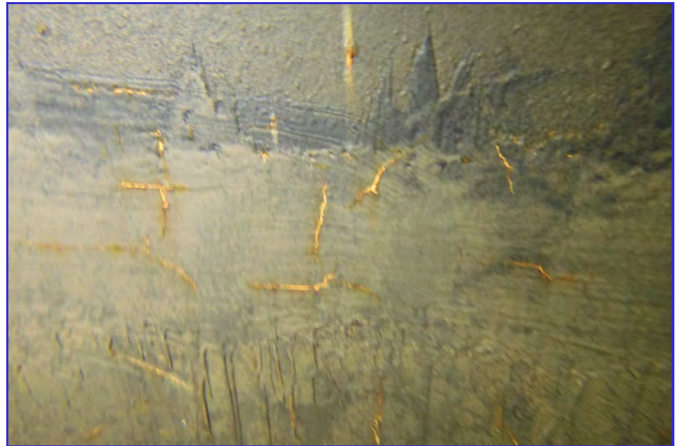
INTERIOR - CPUD - Paloma Reservoir - Maintenance Inspection -063
