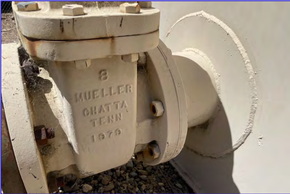
EXTERIOR - CPUD - Golden Hills - Maintenance Inspection -044
