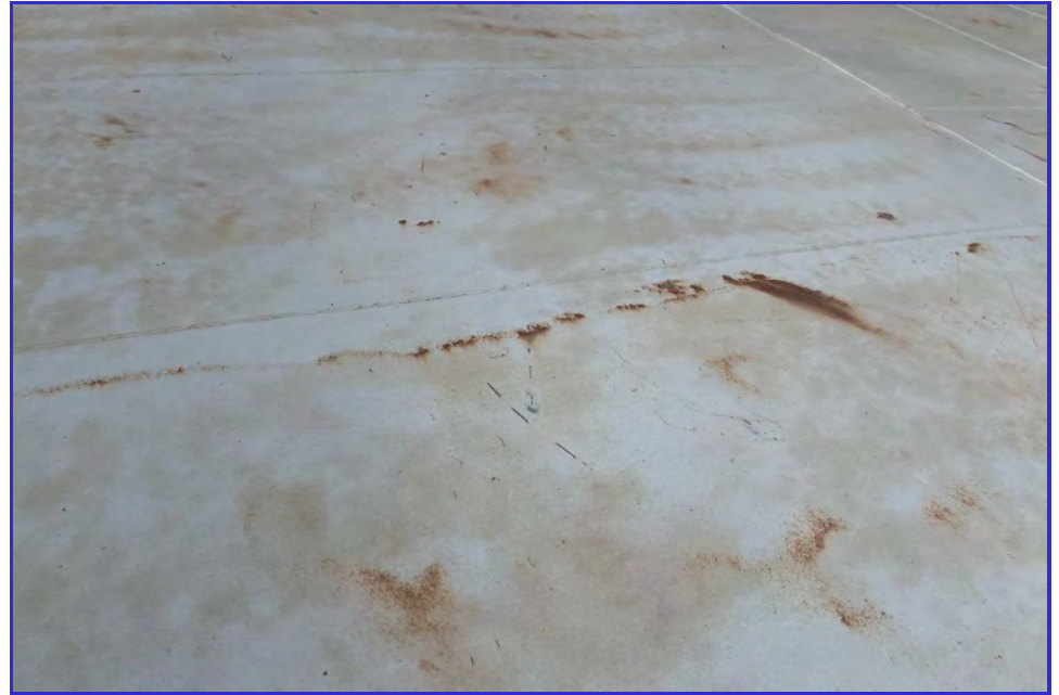
EXTERIOR - CPUD - San Andreas Reservoir - Maintenance Inspection -065
