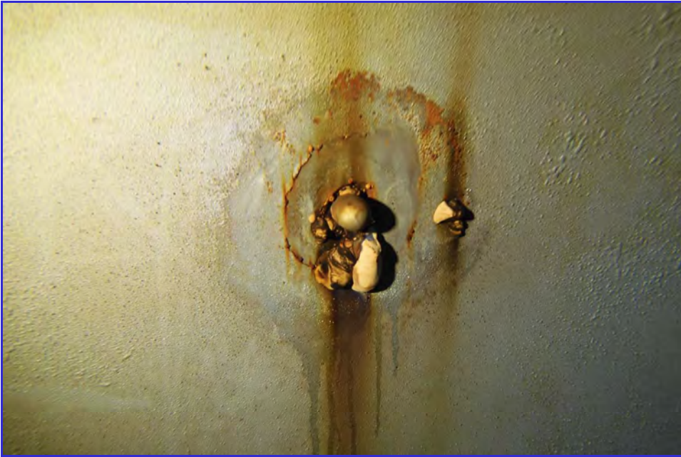
INTERIOR - CPUD - San Andaras Reservoir - Maintenance Inspection -160
