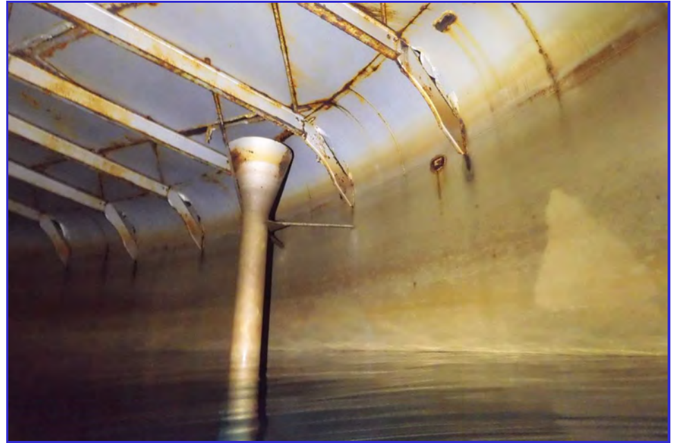
INTERIOR - CPUD - Mokelumne Hill Reservoir - Maintenance Inspection -005
