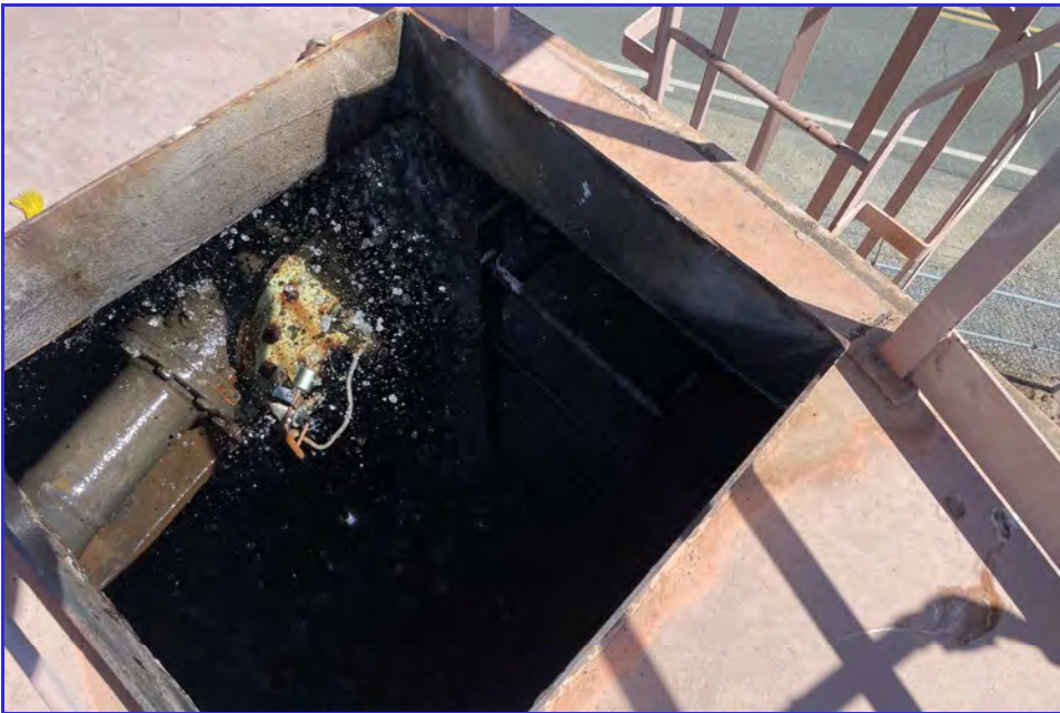
EXTERIOR - CPUD - Paloma Reservoir - Maintenance Inspection -006
