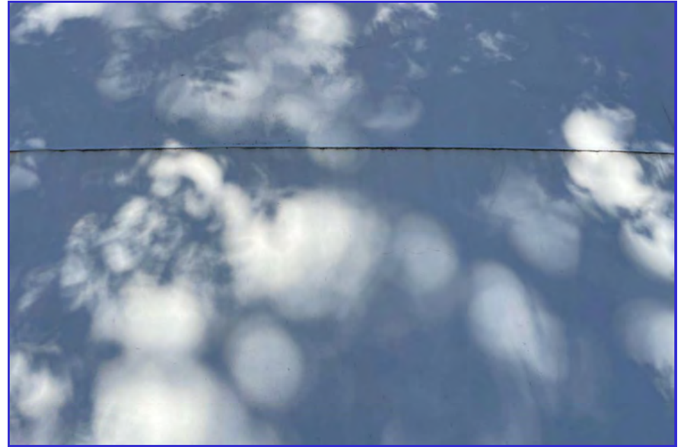
EXTERIOR - CPUD - Mokelumne Reservoir - Maintenance Inspection -165
