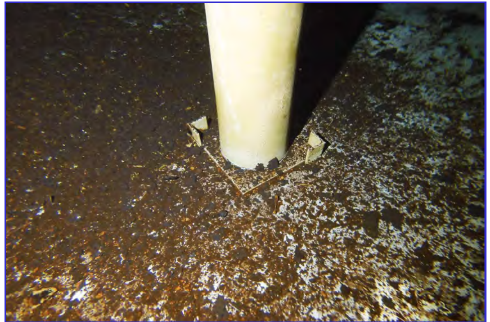
INTERIOR - CPUD - Mokelumne Hill Reservoir - Maintenance Inspection -147
