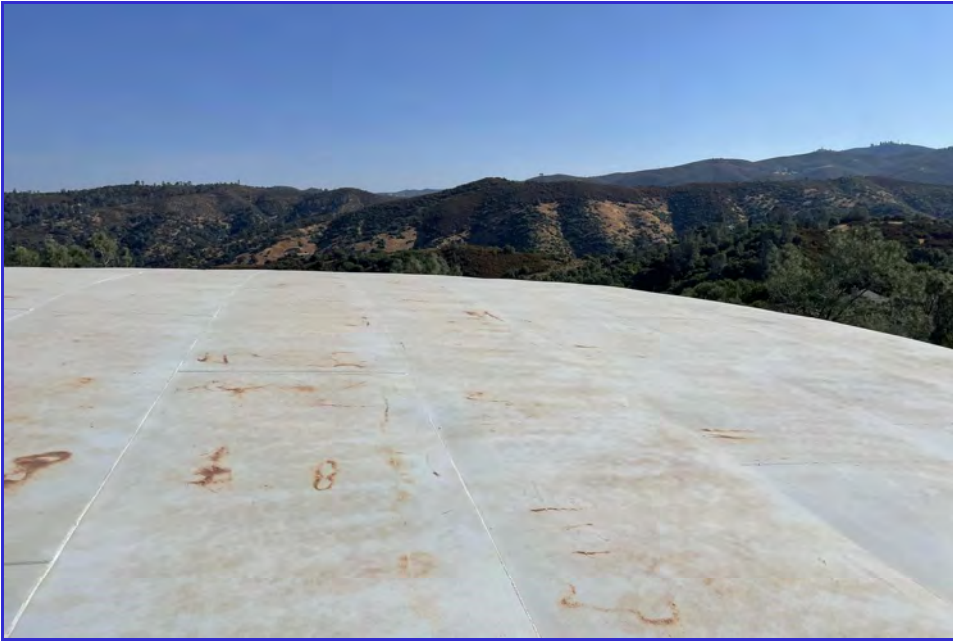
EXTERIOR - CPUD - San Andreas Reservoir - Maintenance Inspection -032
