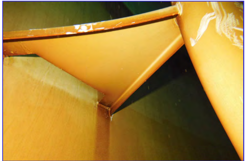
INTERIOR - CPUD - Railroad Flat Reservoir - Maintenance Inspection -171
