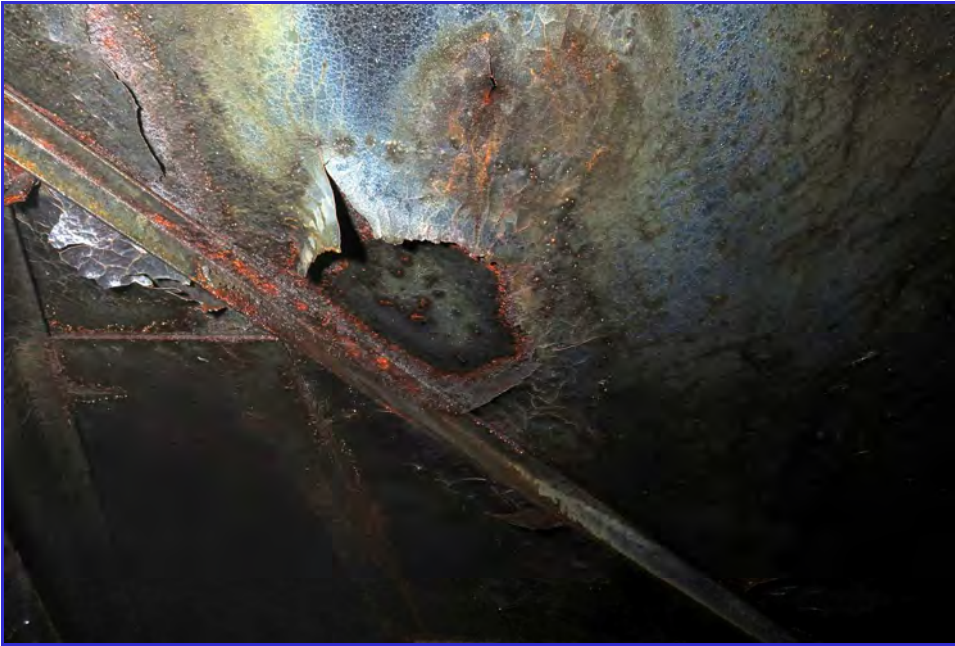
INTERIOR - Calaveras Public Utility District - Clear Well Tank - Maintenance Inspection -052
