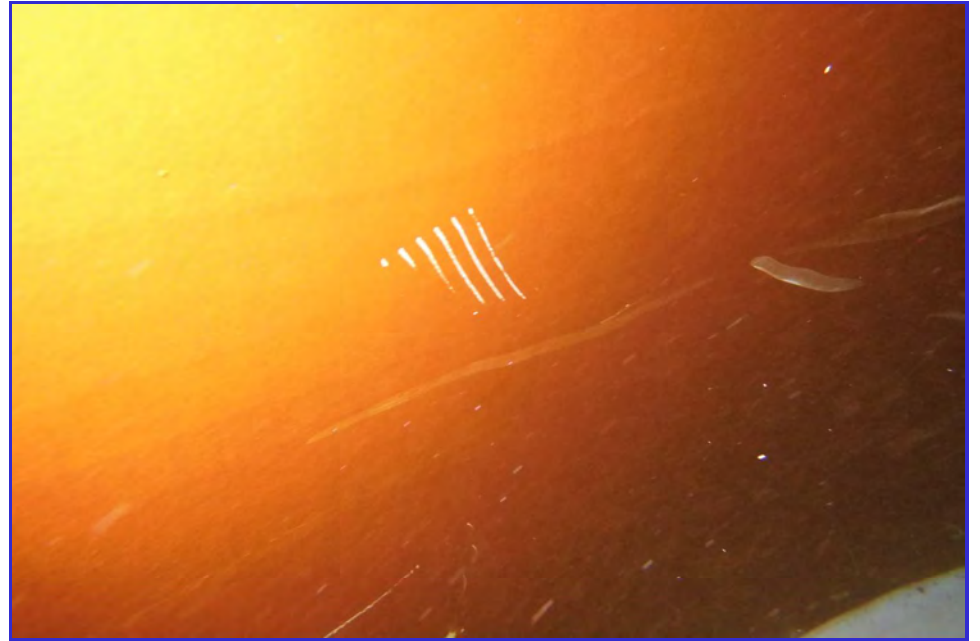
INTERIOR - CPUD - Railroad Flat Reservoir - Maintenance Inspection -089
