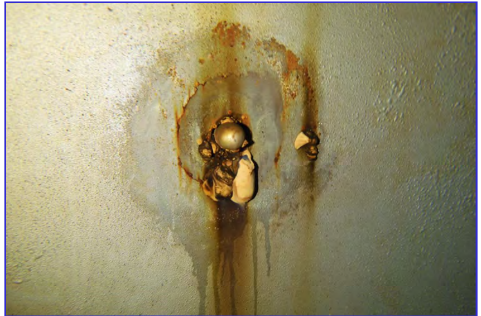
INTERIOR - CPUD - San Andaras Reservoir - Maintenance Inspection -159
