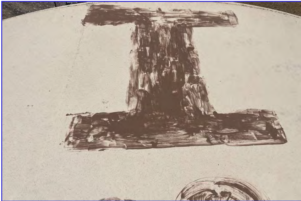
EXTERIOR - CPUD - Golden Hills - Maintenance Inspection -006
