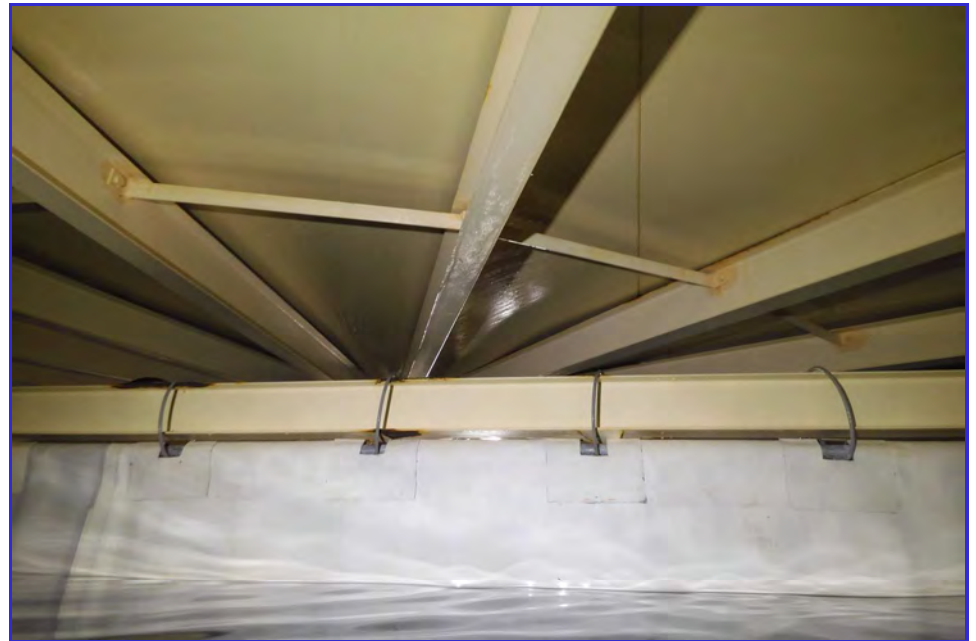
INTERIOR - CPUD - Railroad Flat Reservoir - Maintenance Inspection -059
