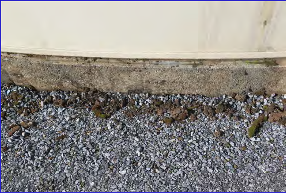
EXTERIOR - Calaveras Public Utility District - Clear Well Tank - Maintenance Inspection -120
