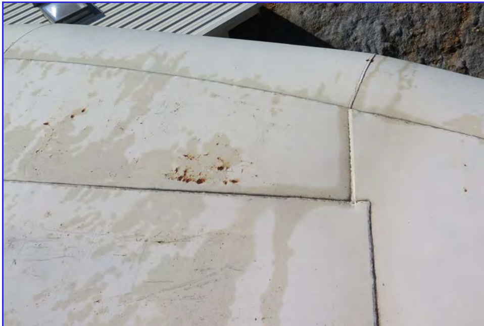
EXTERIOR - Calaveras Public Utility District - Clear Well Tank - Maintenance Inspection -026
