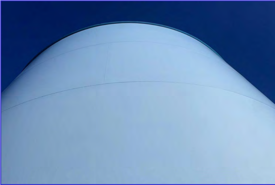
EXTERIOR - CPUD - Railroad Flat Reservoir - Maintenance Inspection -056
