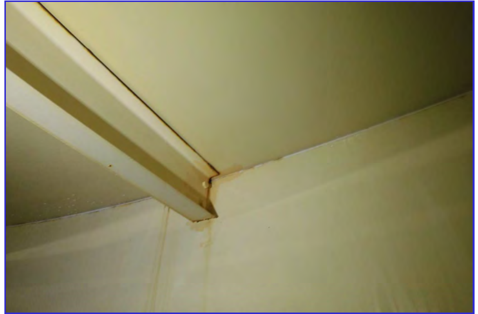
INTERIOR - CPUD - Railroad Flat Reservoir - Maintenance Inspection -053
