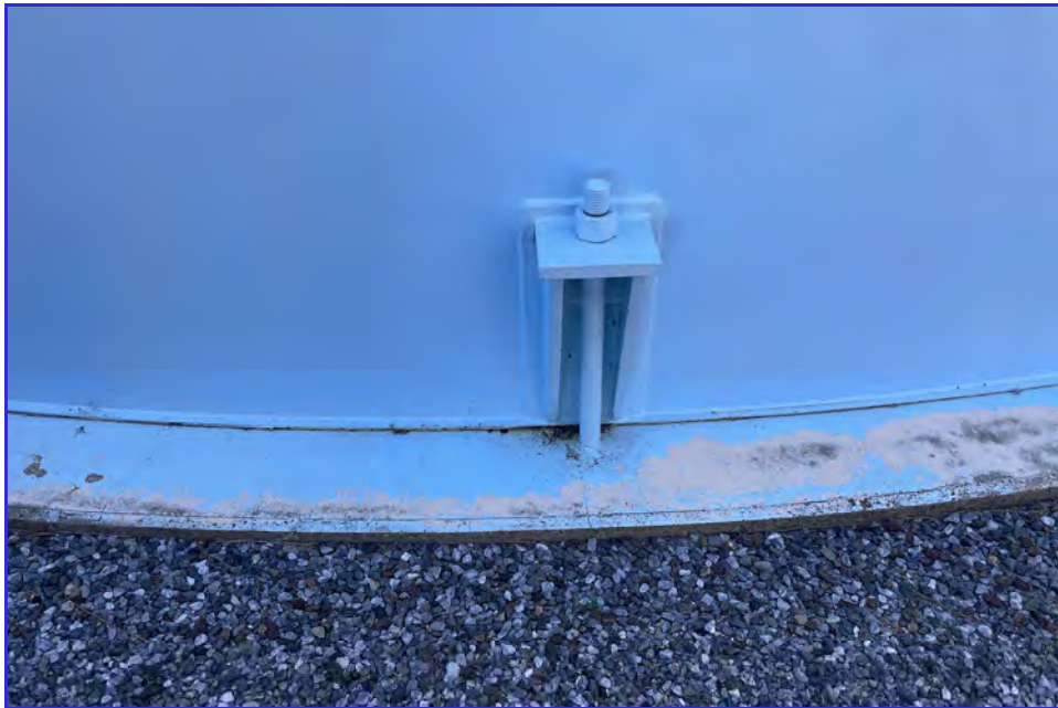
EXTERIOR - CPUD - Railroad Flat Reservoir - Maintenance Inspection -070
