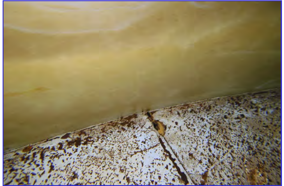
INTERIOR - CPUD - Mokelumne Hill Reservoir - Maintenance Inspection -101
