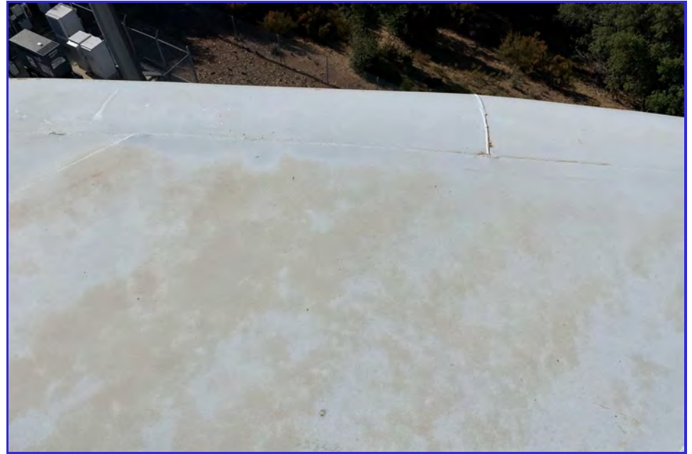
EXTERIOR - CPUD - San Andreas Reservoir - Maintenance Inspection -037
