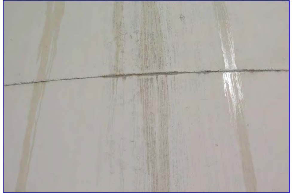
EXTERIOR - Calaveras Public Utility District - Clear Well Tank - Maintenance Inspection -065
