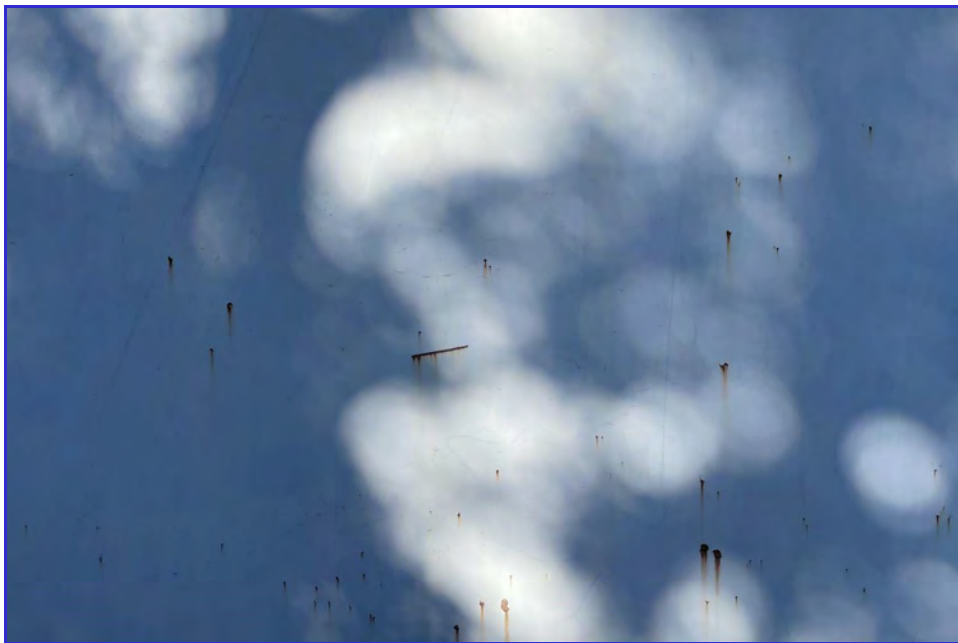
EXTERIOR - CPUD - Mokelumne Reservoir - Maintenance Inspection -170
