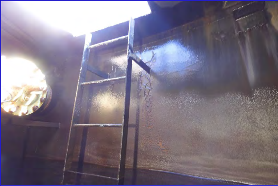
INTERIOR - CPUD - Paloma Reservoir - Maintenance Inspection
