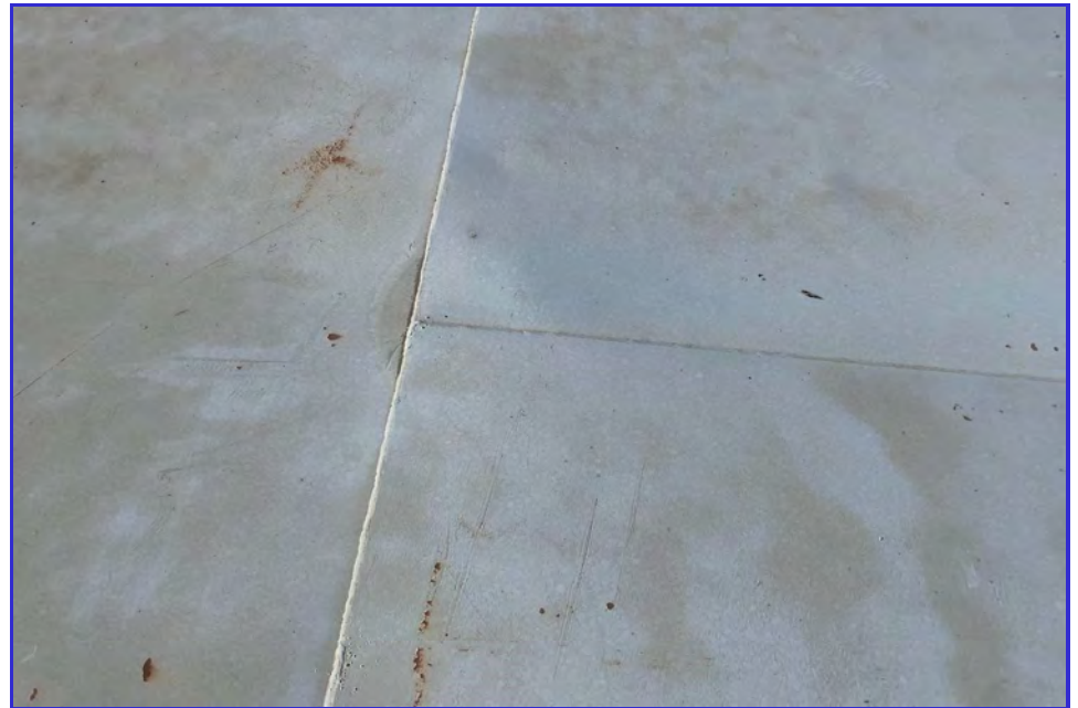
EXTERIOR - CPUD - San Andreas Reservoir - Maintenance Inspection -071
