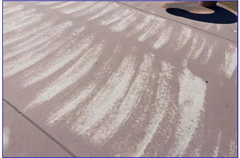
EXTERIOR - CPUD - Paloma Reservoir - Maintenance Inspection -017
