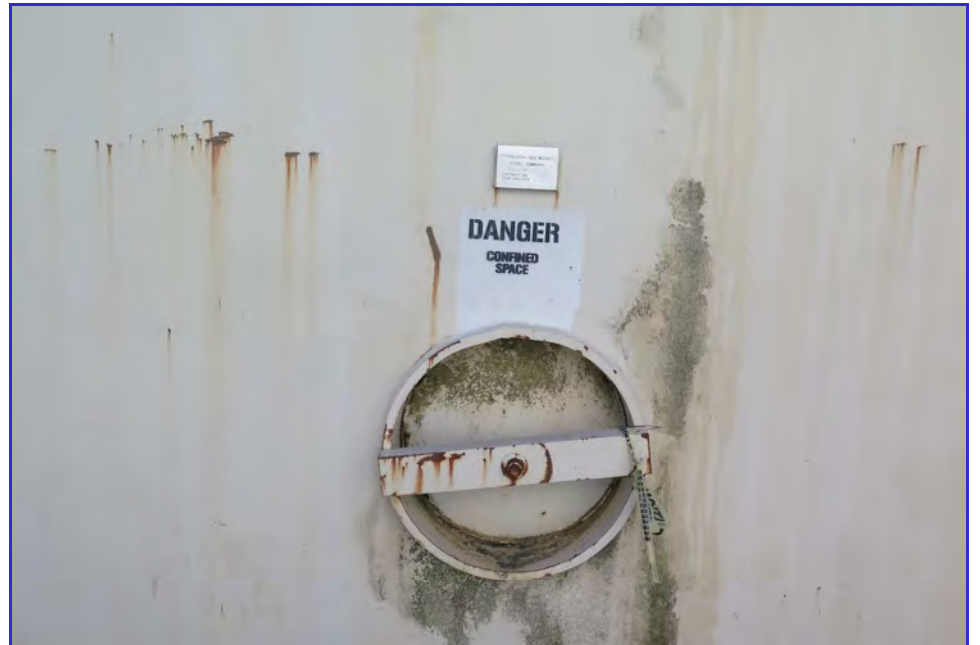
EXTERIOR - Calaveras Public Utility District - Clear Well Tank - Maintenance Inspection -111
