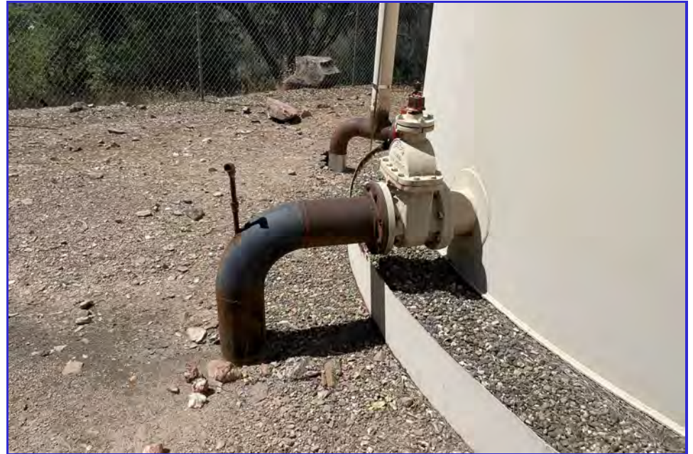
EXTERIOR - CPUD - Golden Hills - Maintenance Inspection -045
