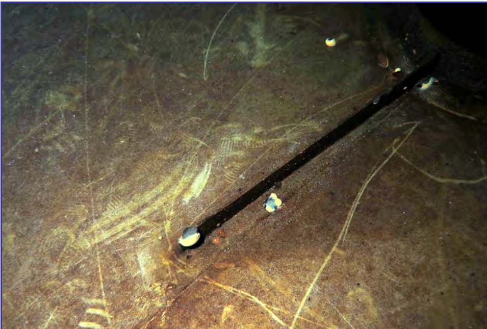
INTERIOR - Calaveras Public Utility District - Clear Well Tank - Maintenance Inspection -062
