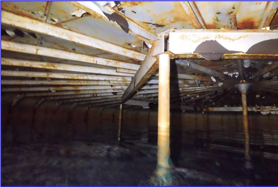
INTERIOR - CPUD - San Andaras Reservoir - Maintenance Inspection -008
