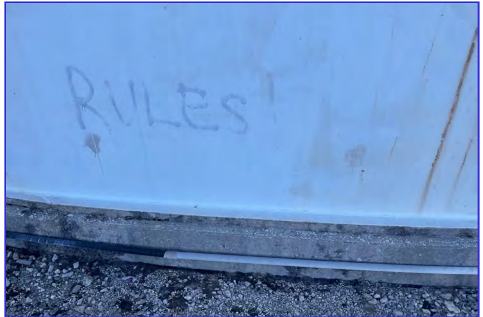
EXTERIOR - CPUD - San Andreas Reservoir - Maintenance Inspection -167
