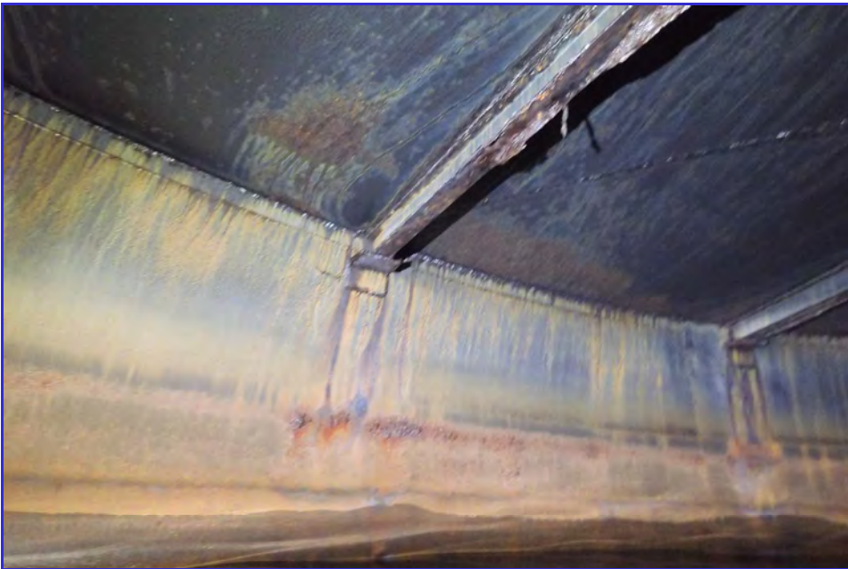
INTERIOR - CPUD - Paloma Reservoir - Maintenance Inspection -010
