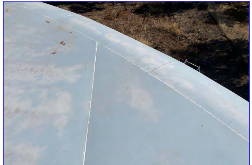
EXTERIOR - CPUD - Mokelumne Reservoir - Maintenance Inspection -051
