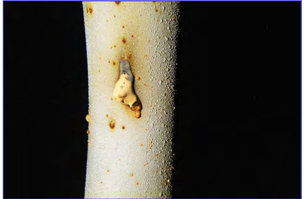
INTERIOR - CPUD - San Andaras Reservoir - Maintenance Inspection -157
