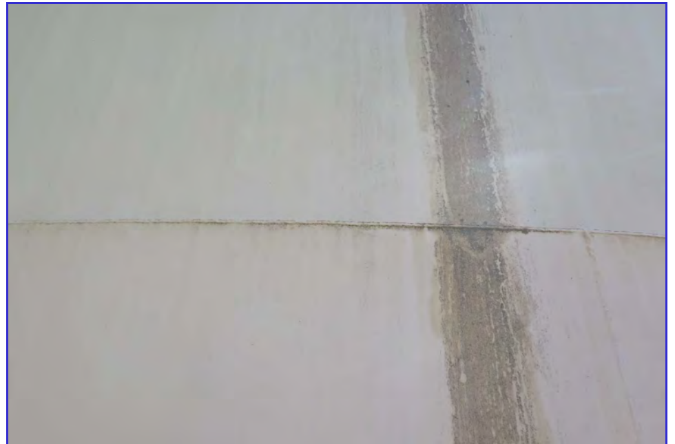
EXTERIOR - Calaveras Public Utility District - Clear Well Tank - Maintenance Inspection -087
