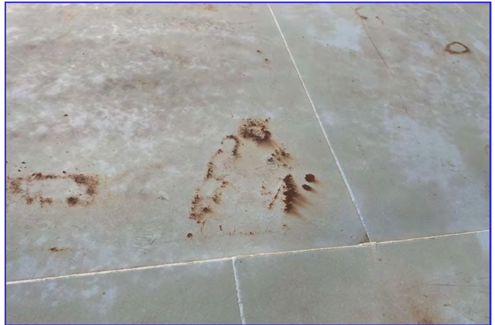
EXTERIOR - CPUD - San Andreas Reservoir - Maintenance Inspection -079
