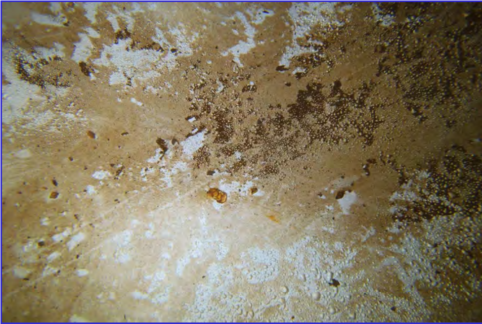
INTERIOR - CPUD - San Andaras Reservoir - Maintenance Inspection -188
