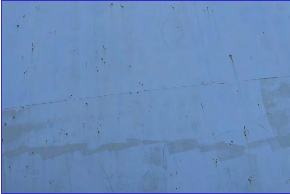
EXTERIOR - CPUD - San Andreas Reservoir - Maintenance Inspection -172
