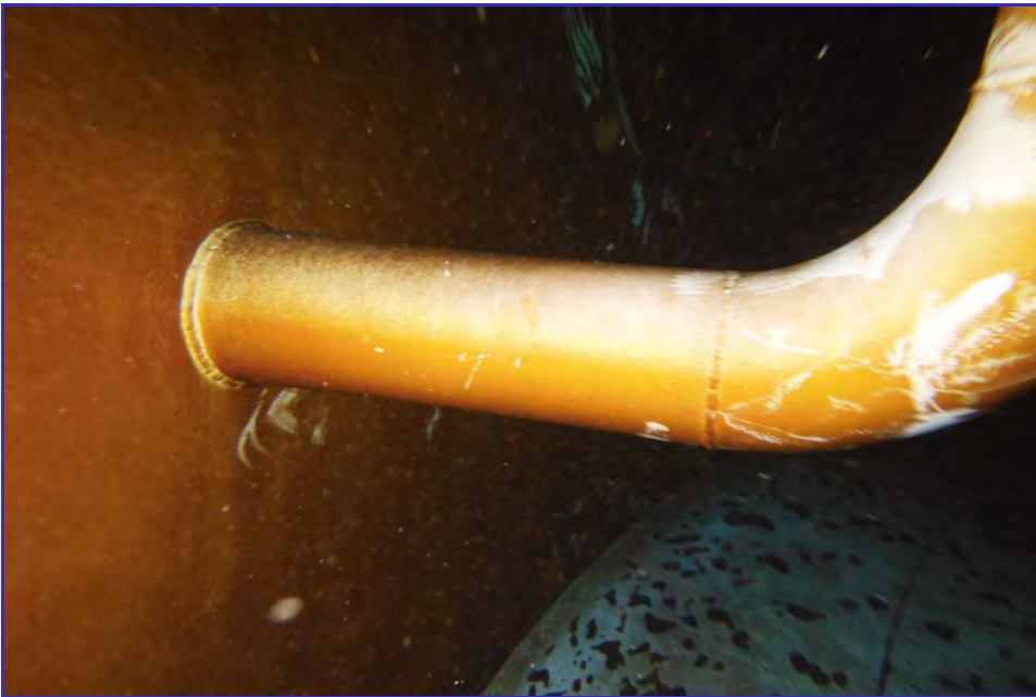
INTERIOR - CPUD - Railroad Flat Reservoir - Maintenance Inspection -166
