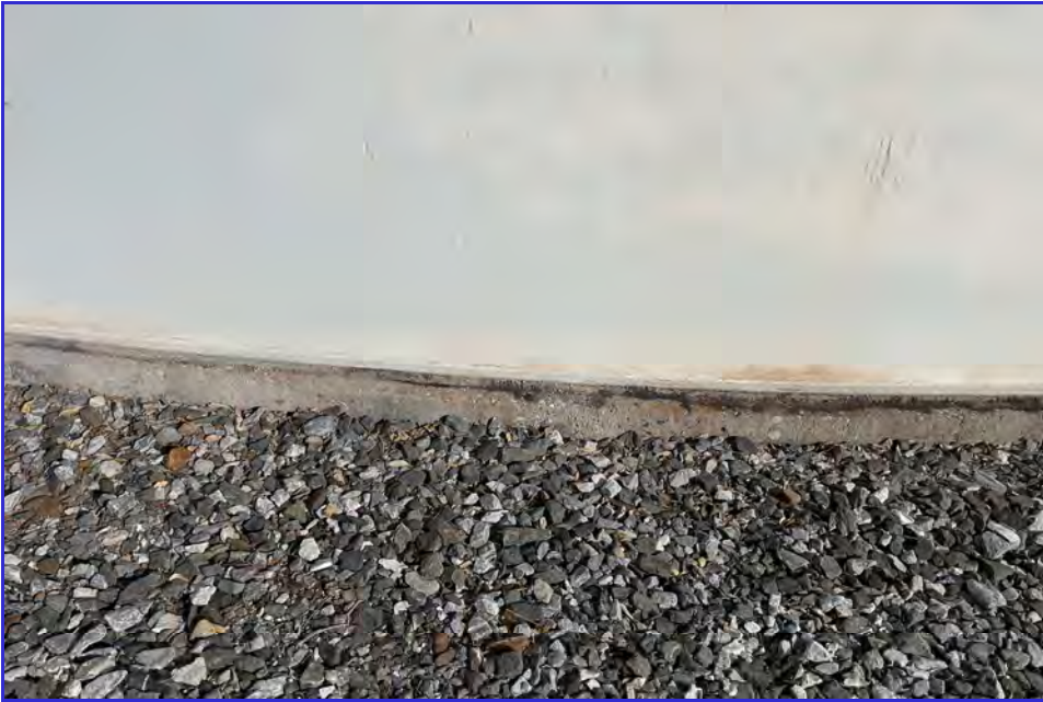
EXTERIOR - CPUD - Mokelumne Reservoir - Maintenance Inspection -160
