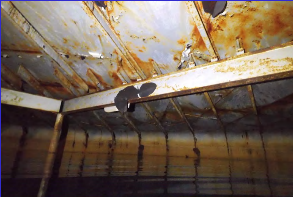
INTERIOR - CPUD - San Andaras Reservoir - Maintenance Inspection -080
