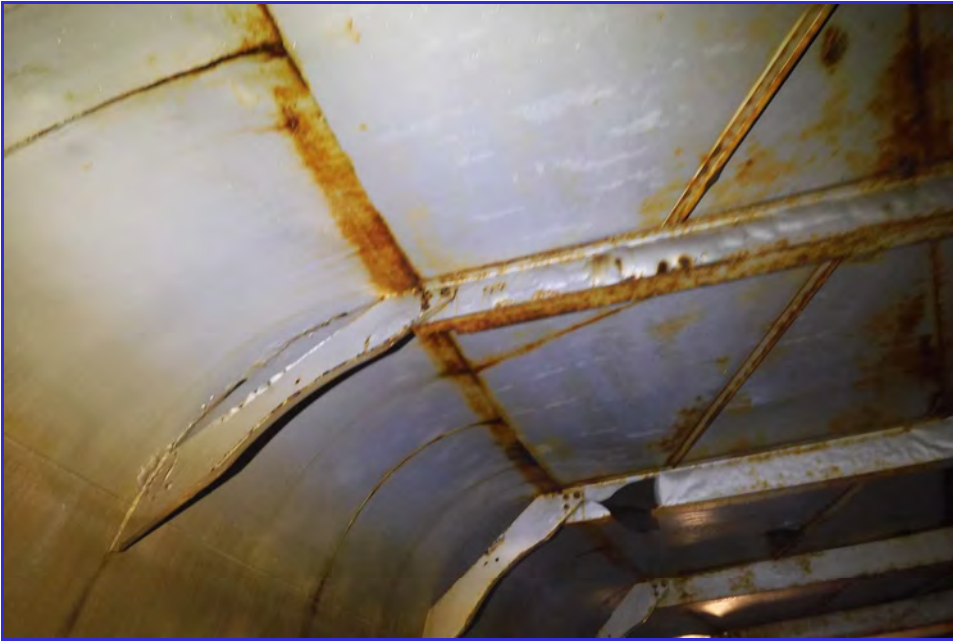
INTERIOR - CPUD - San Andaras Reservoir - Maintenance Inspection -020
