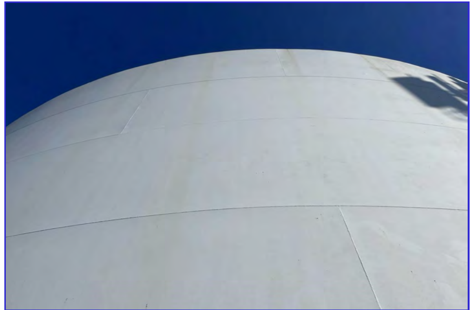
EXTERIOR - CPUD - San Andreas Reservoir - Maintenance Inspection -151
