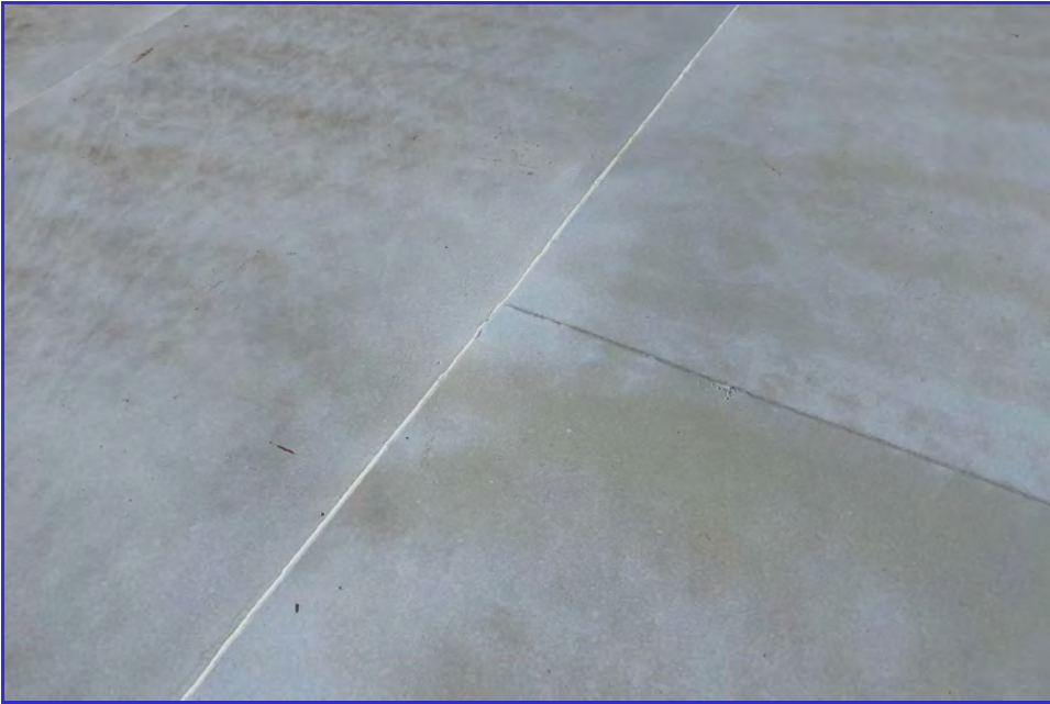
EXTERIOR - CPUD - San Andreas Reservoir - Maintenance Inspection -008
