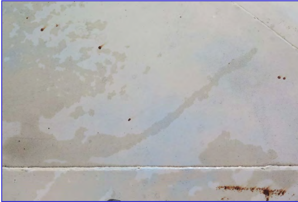
EXTERIOR - Calaveras Public Utility District - Clear Well Tank - Maintenance Inspection -036
