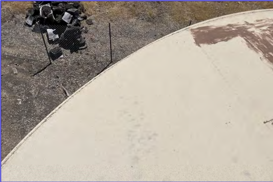
EXTERIOR - CPUD - Golden Hills - Maintenance Inspection -008
