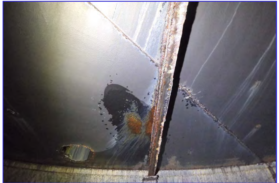
INTERIOR - CPUD - Paloma Reservoir - Maintenance Inspection -023
