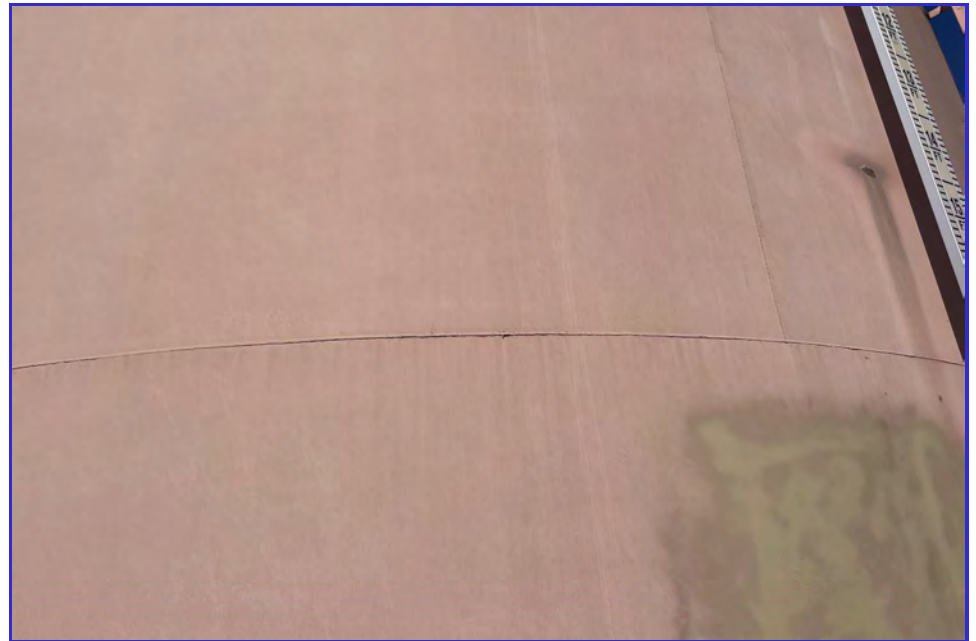
EXTERIOR - CPUD - Paloma Reservoir - Maintenance Inspection -071
