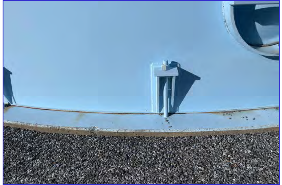
EXTERIOR - CPUD - Railroad Flat Reservoir - Maintenance Inspection -089
