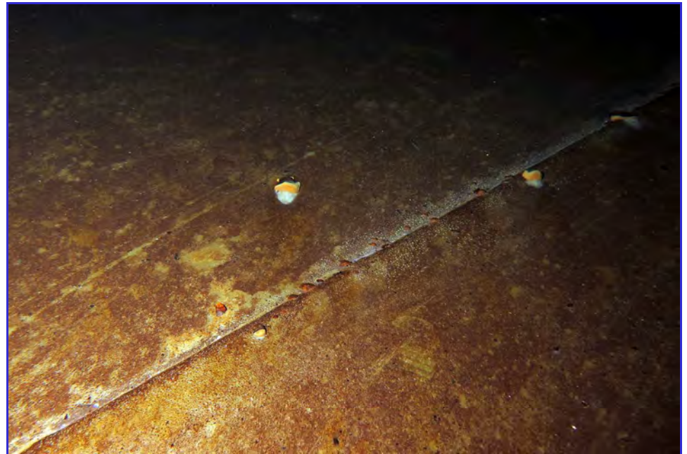
INTERIOR - Calaveras Public Utility District - Clear Well Tank - Maintenance Inspection -131
