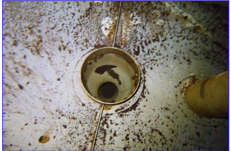
INTERIOR - CPUD - Mokelumne Hill Reservoir - Maintenance Inspection -109
