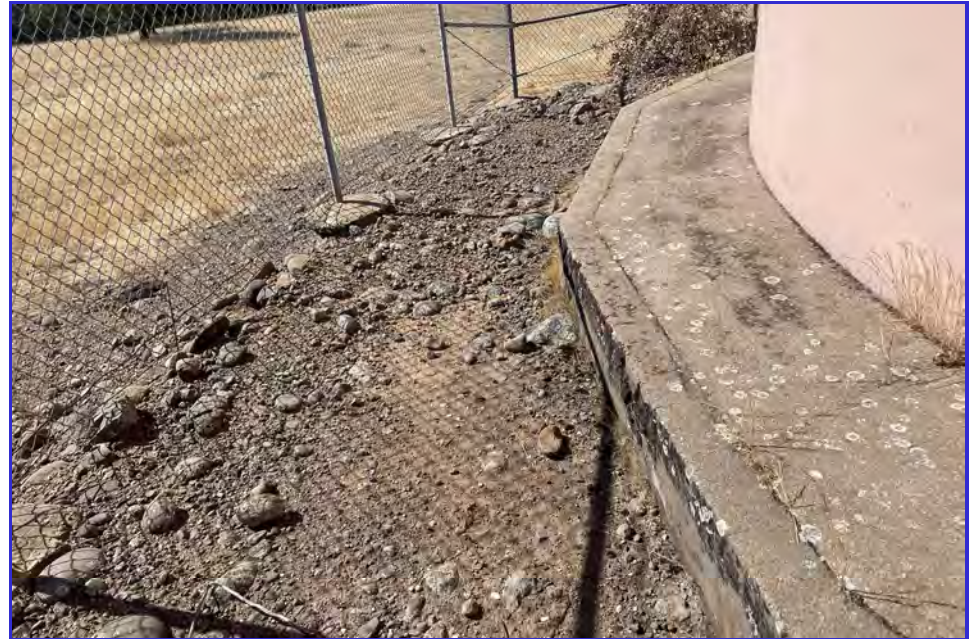
EXTERIOR - CPUD - Paloma Reservoir - Maintenance Inspection -053
