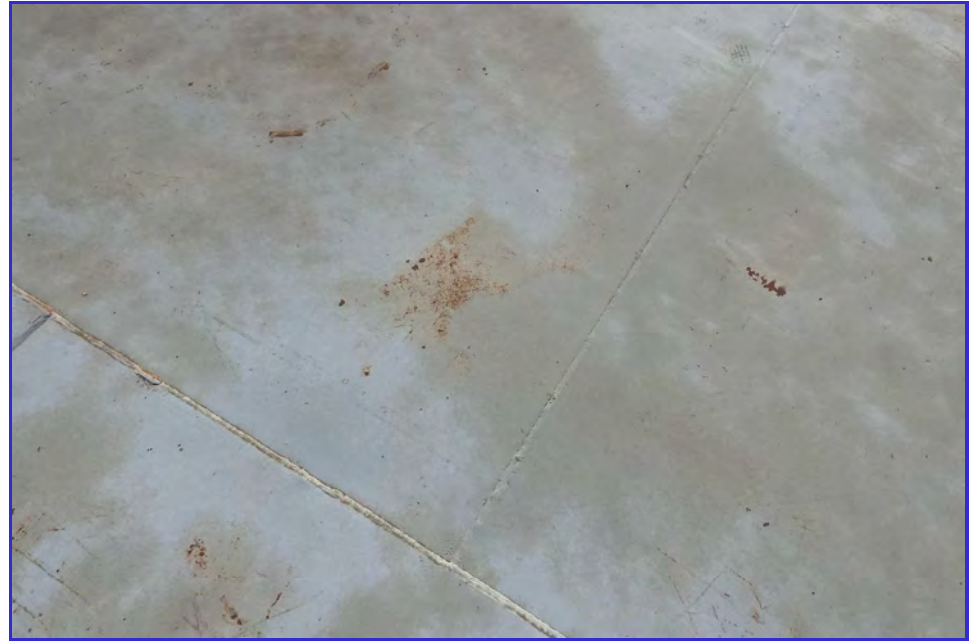
EXTERIOR - CPUD - San Andreas Reservoir - Maintenance Inspection -053
