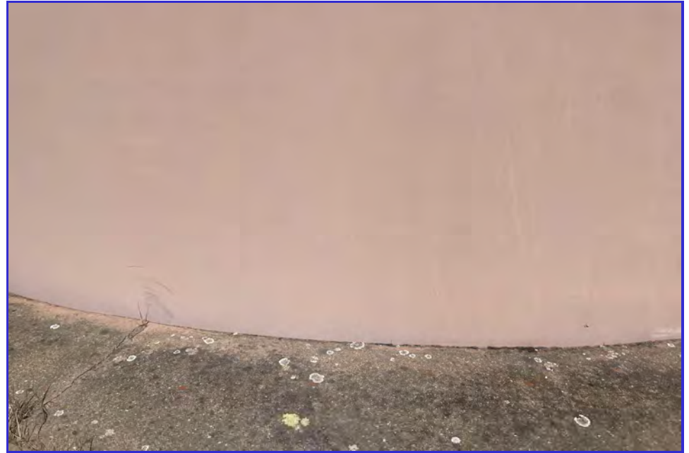
EXTERIOR - CPUD - Paloma Reservoir - Maintenance Inspection -073
