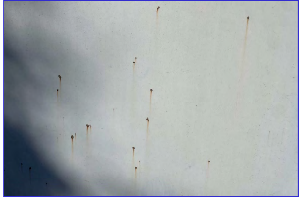
EXTERIOR - CPUD - Mokelumne Reservoir - Maintenance Inspection -089
