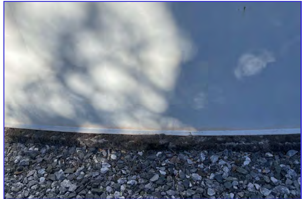
EXTERIOR - CPUD - Mokelumne Reservoir - Maintenance Inspection -167
