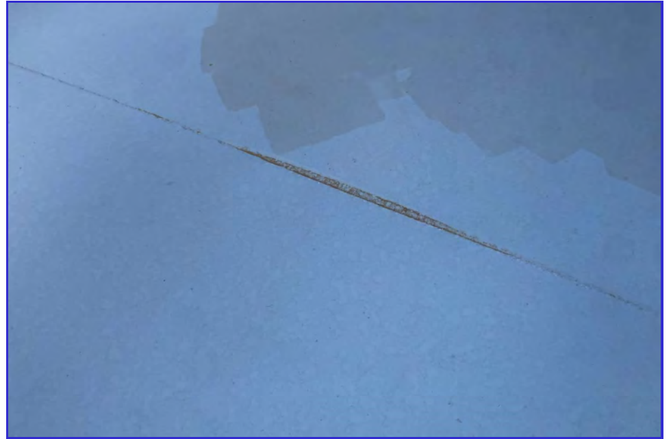
EXTERIOR - CPUD - Railroad Flat Reservoir - Maintenance Inspection -037
