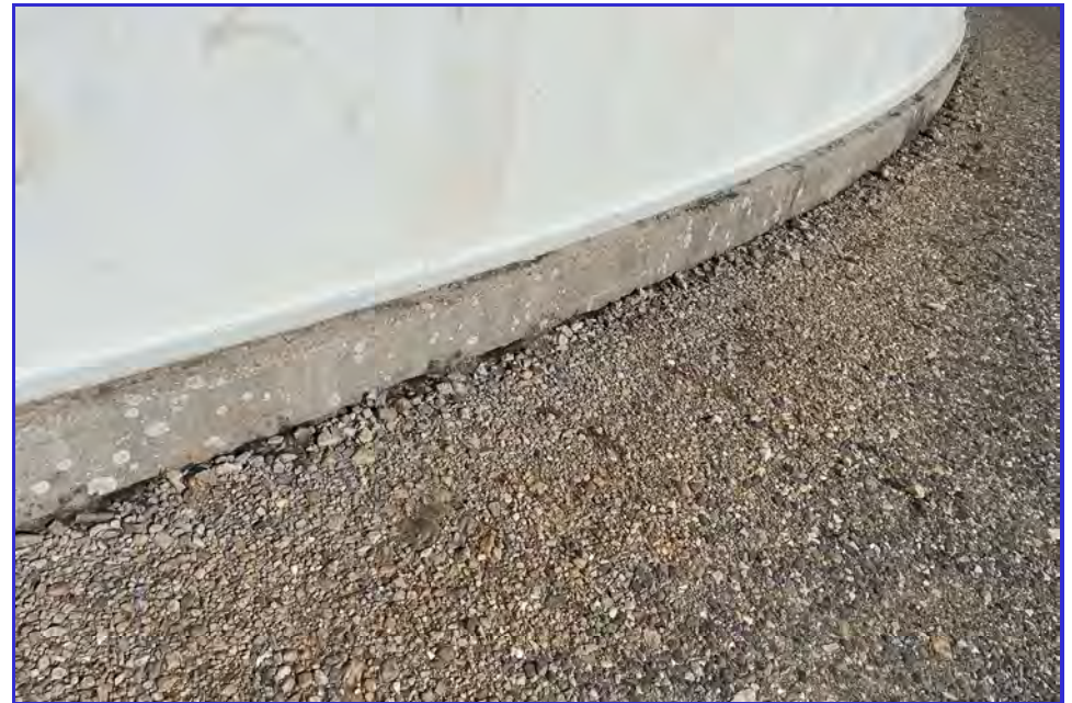
EXTERIOR - CPUD - San Andreas Reservoir - Maintenance Inspection -139
