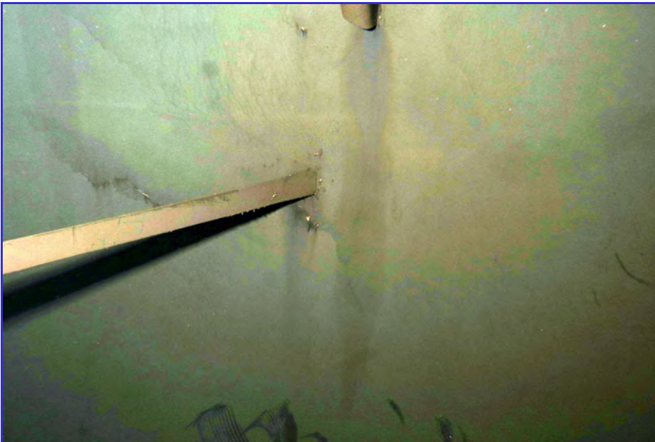
INTERIOR - Calaveras Public Utility District - Clear Well Tank - Maintenance Inspection -058
