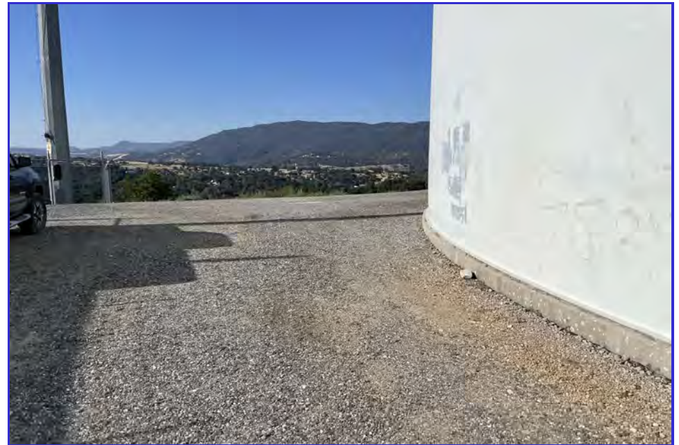
EXTERIOR - CPUD - San Andreas Reservoir - Maintenance Inspection -135
