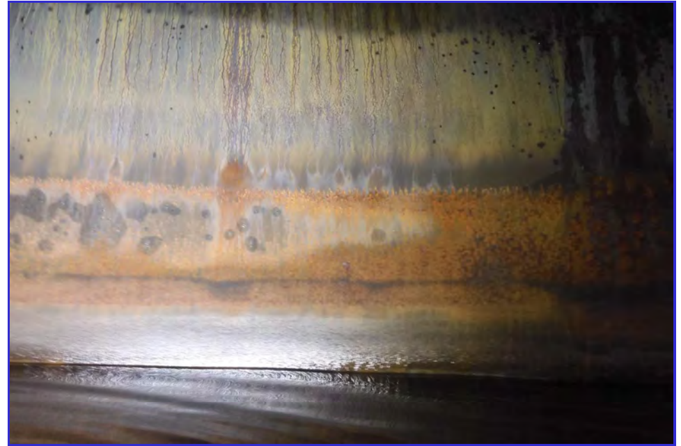
INTERIOR - CPUD - Paloma Reservoir - Maintenance Inspection -041
