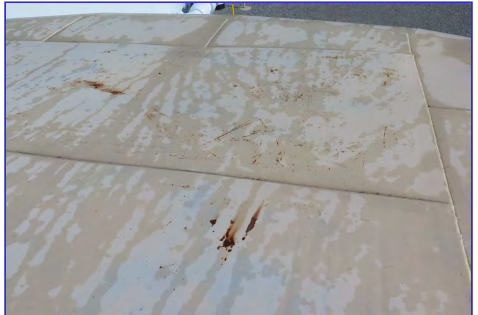
EXTERIOR - Calaveras Public Utility District - Clear Well Tank - Maintenance Inspection -007
