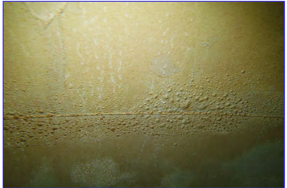
INTERIOR - CPUD - San Andaras Reservoir - Maintenance Inspection -123
