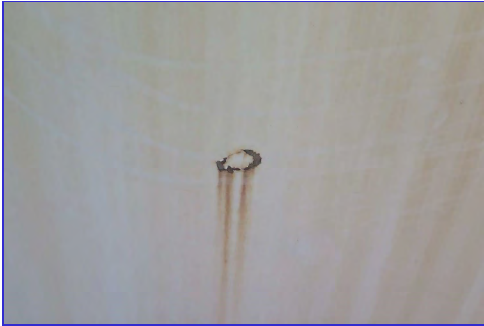
EXTERIOR - Calaveras Public Utility District - Clear Well Tank - Maintenance Inspection -100
