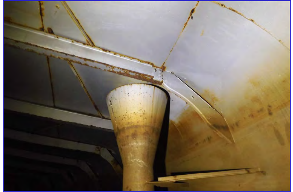
INTERIOR - CPUD - San Anderas Reservoir - Maintenance Inspection -041
