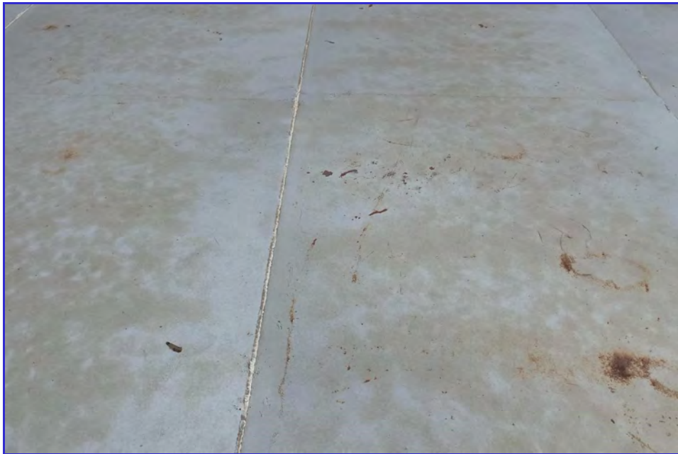
EXTERIOR - CPUD - San Andreas Reservoir - Maintenance Inspection -058
