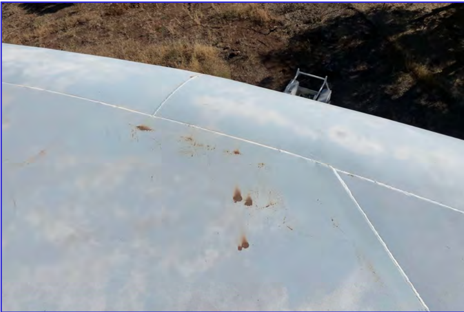
EXTERIOR - CPUD - Mokelumne Reservoir - Maintenance Inspection -050
