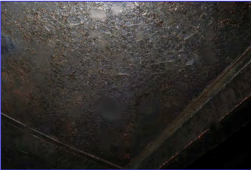
INTERIOR - Calaveras Public Utility District - Clear Well Tank - Maintenance Inspection -026
