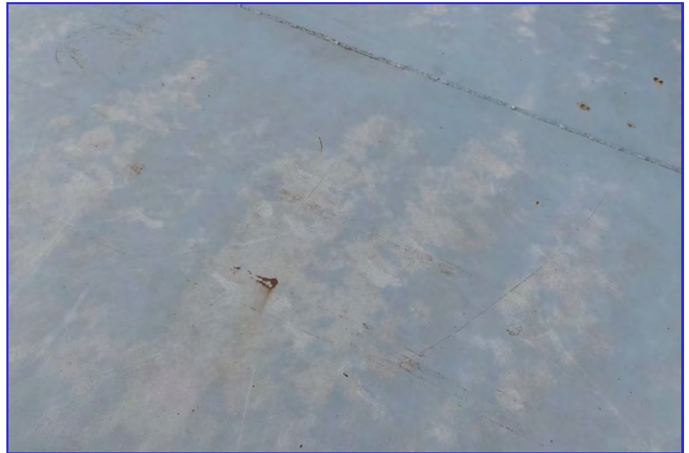
EXTERIOR - CPUD - Mokelumne Reservoir - Maintenance Inspection -007
