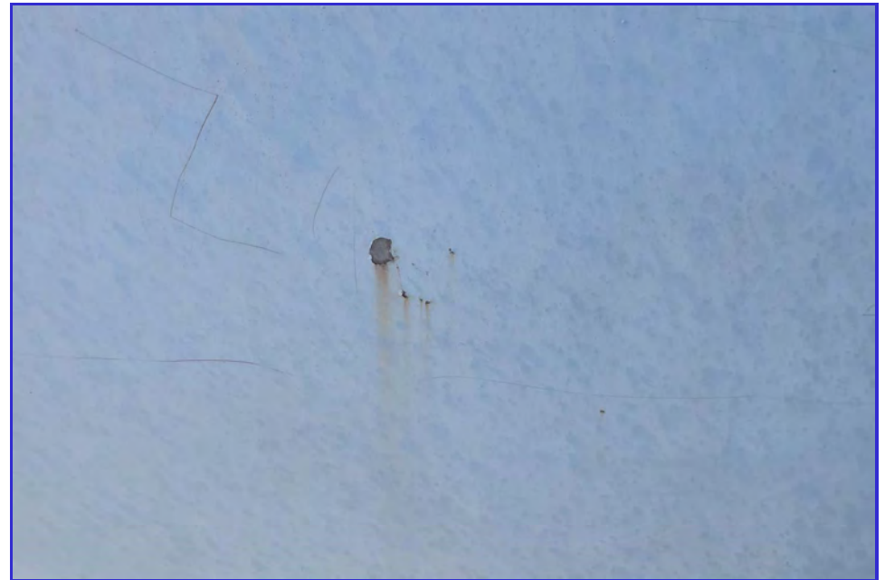
EXTERIOR - CPUD - San Andreas Reservoir - Maintenance Inspection -115
