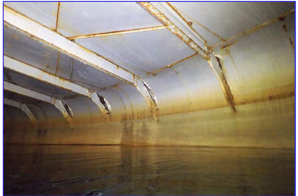
INTERIOR - CPUD - San Andreas Reservoir - Maintenance Inspection -047
