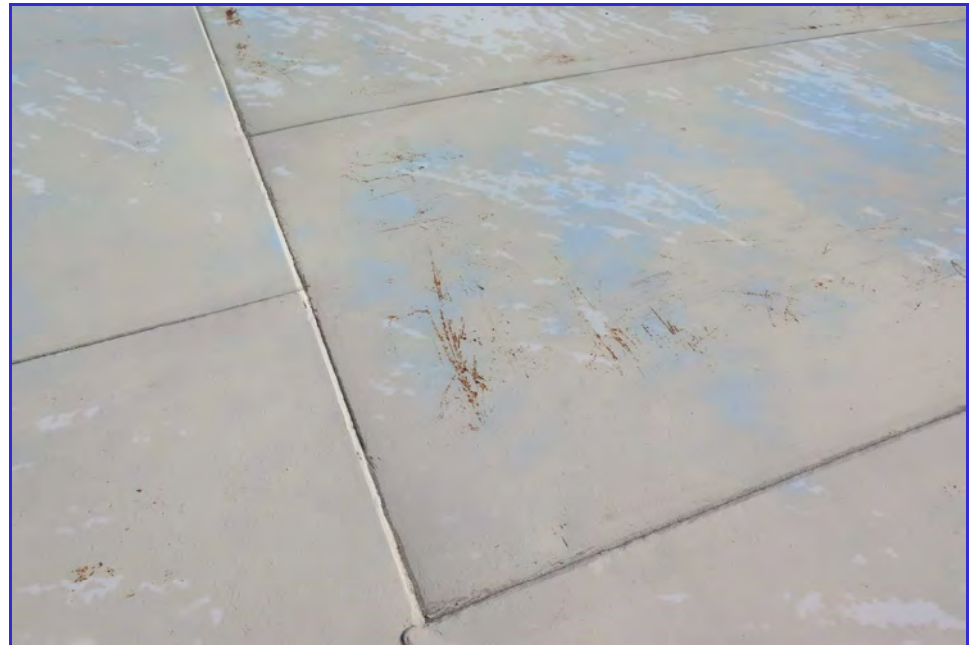
EXTERIOR - Calaveras Public Utility District - Clear Well Tank - Maintenance Inspection -047
