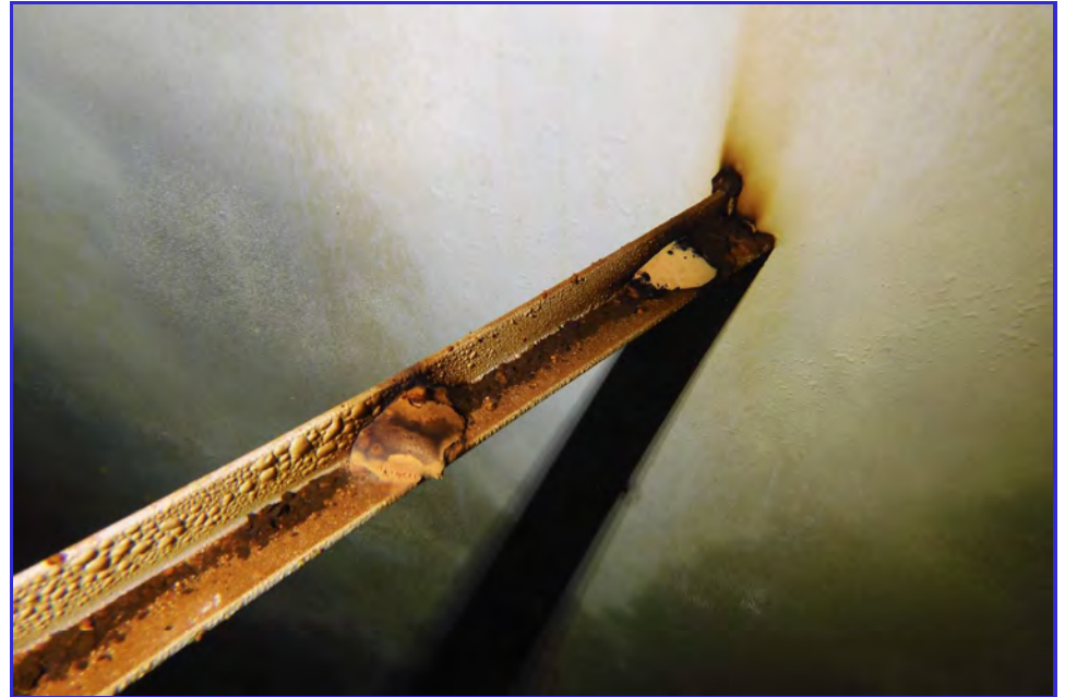
INTERIOR - CPUD - Mokelumne Hill Reservoir - Maintenance Inspection -117
