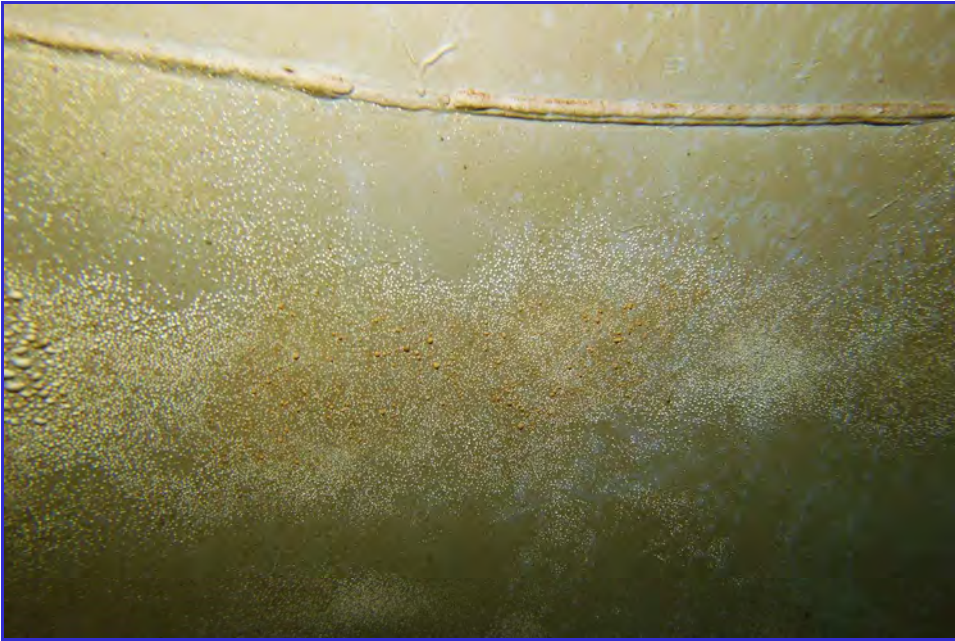
INTERIOR - CPUD - Mokelumne Hill Reservoir - Maintenance Inspection -088
