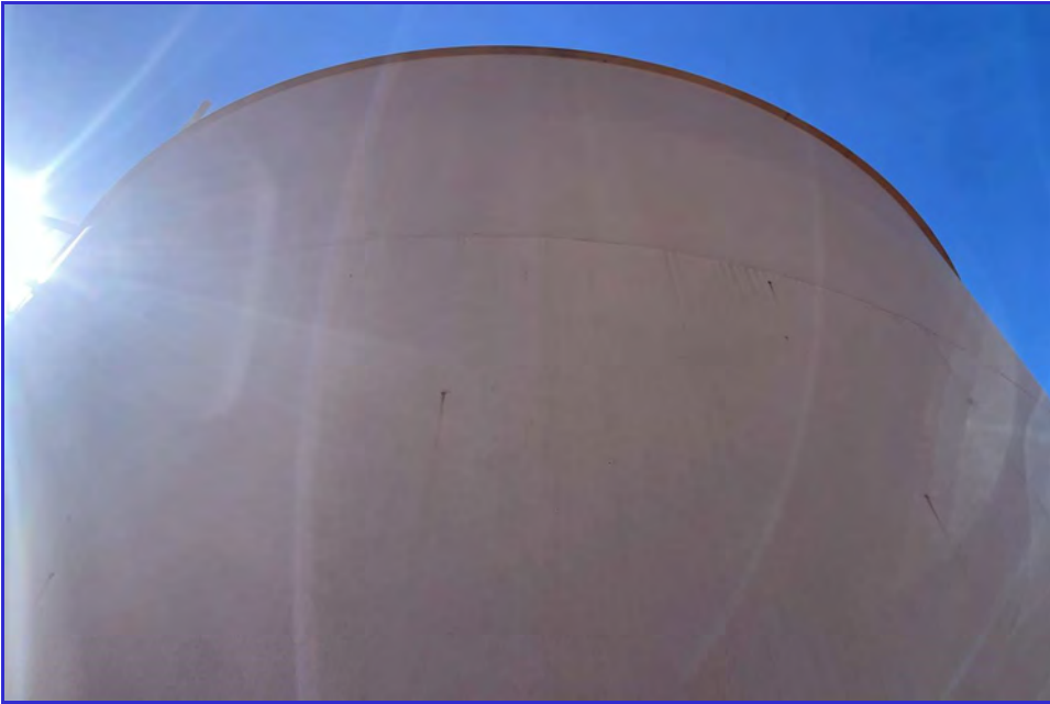
EXTERIOR - CPUD - Paloma Reservoir - Maintenance Inspection -068
