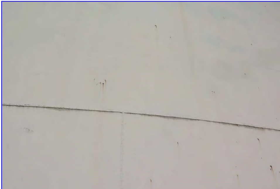
EXTERIOR - Calaveras Public Utility District - Clear Well Tank - Maintenance Inspection -062
