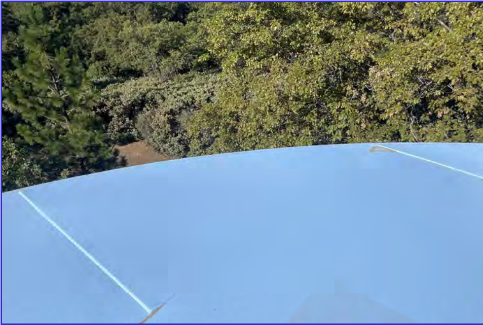
EXTERIOR - CPUD - Railroad Flat Reservoir - Maintenance Inspection -032
