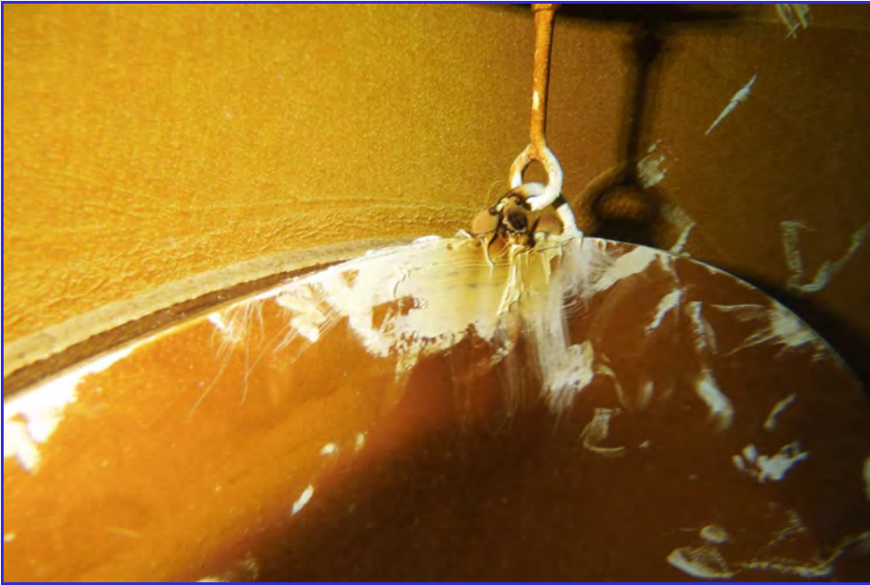
INTERIOR - CPUD - Railroad Flat Reservoir - Maintenance Inspection -088
