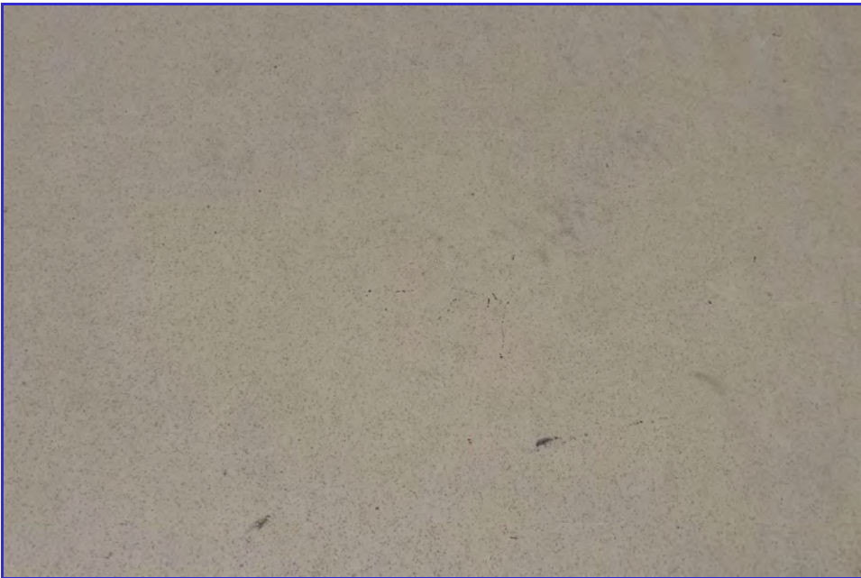
EXTERIOR - CPUD - Golden Hills - Maintenance Inspection -010
