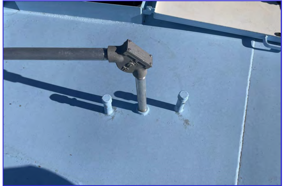
EXTERIOR - CPUD - Railroad Flat Reservoir - Maintenance Inspection -005
