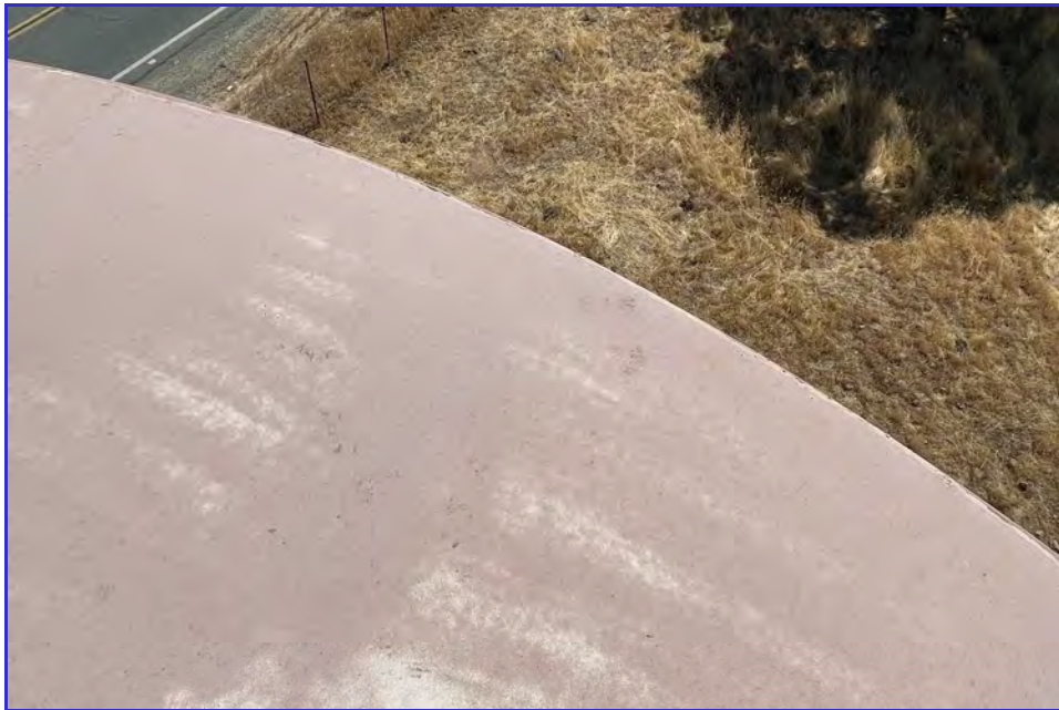
EXTERIOR - CPUD - Paloma Reservoir - Maintenance Inspection -022
