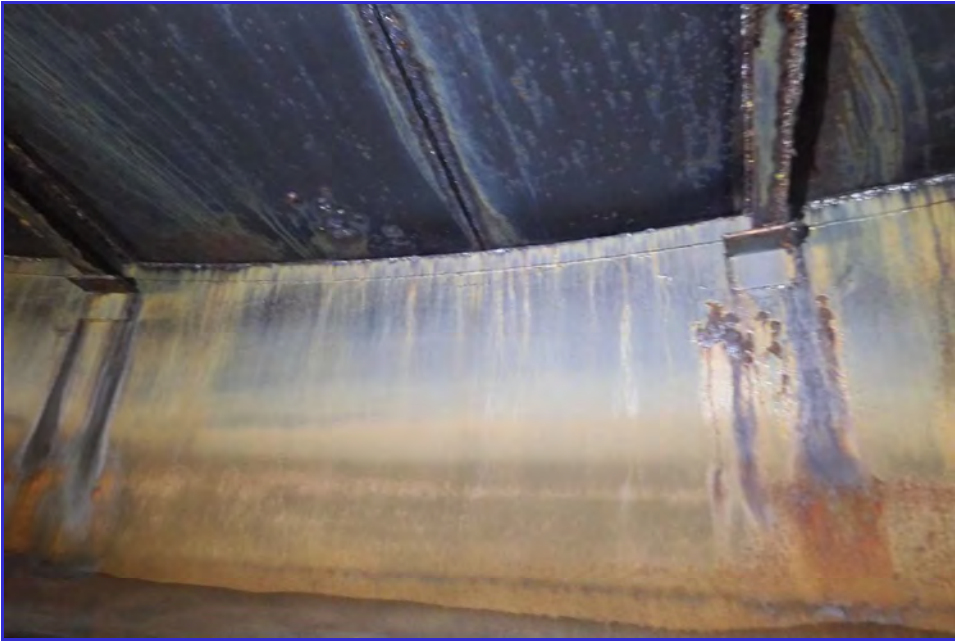
INTERIOR - CPUD - Paloma Reservoir - Maintenance Inspection -008
