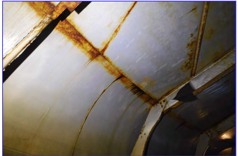
INTERIOR - CPUD - San Andaras Reservoir - Maintenance Inspection -019
