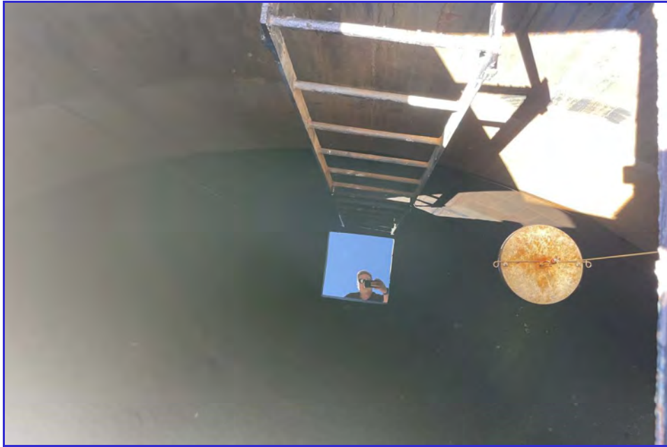
EXTERIOR - CPUD - Golden Hills - Maintenance Inspection -024
