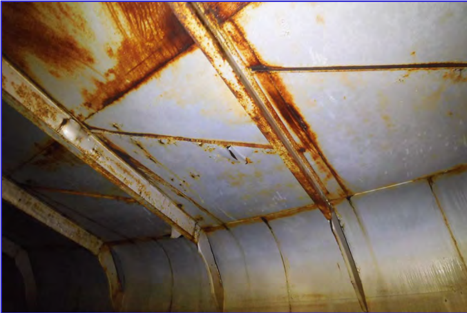
INTERIOR - CPUD - San Andreas Reservoir - Maintenance Inspection -012
