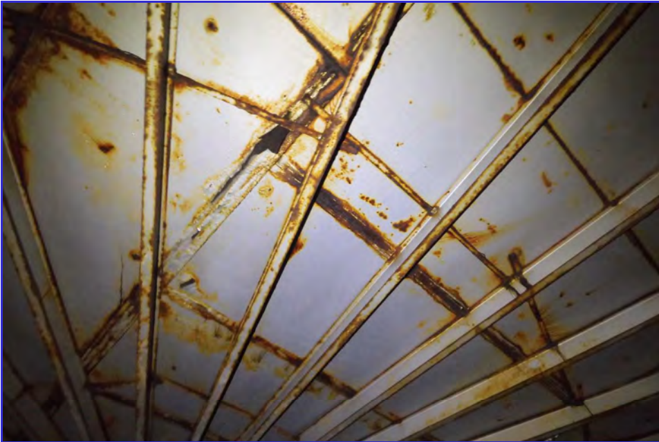
INTERIOR - CPUD - Mokelumne Hill Reservoir - Maintenance Inspection -056
