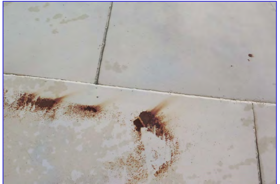
EXTERIOR - Calaveras Public Utility District - Clear Well Tank - Maintenance Inspection -031
