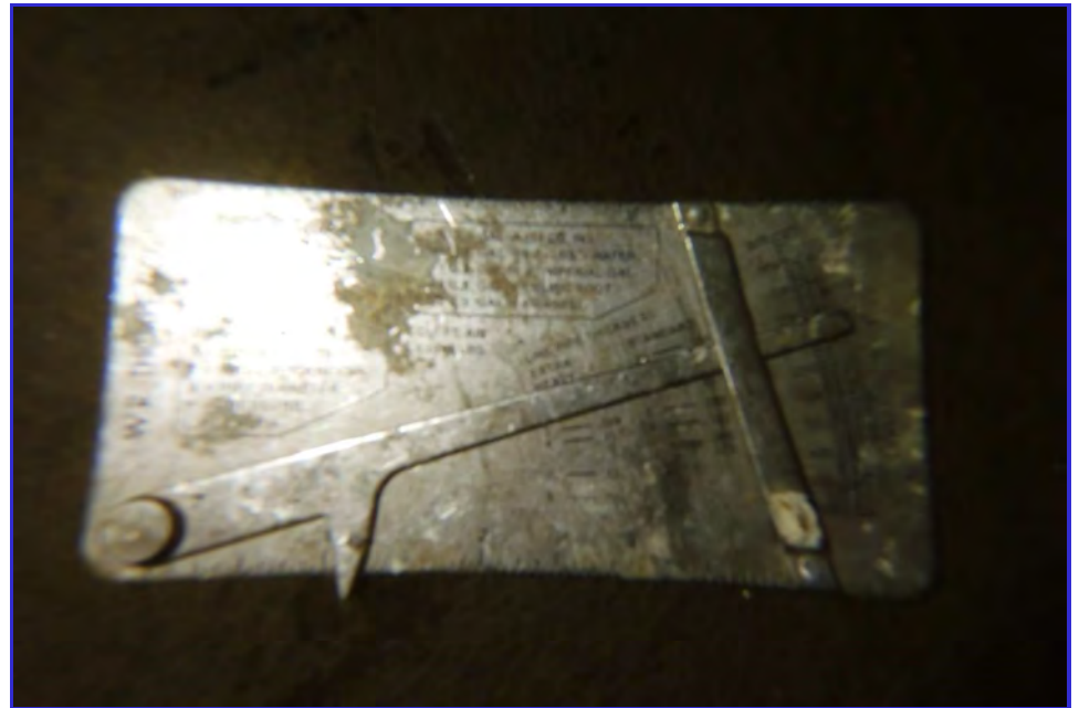
INTERIOR - CPUD - Golden Hills - Maintenance Inspection -115
