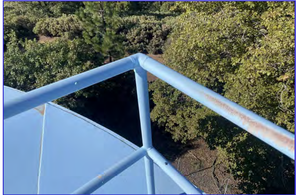
EXTERIOR - CPUD - Railroad Flat Reservoir - Maintenance Inspection -003
