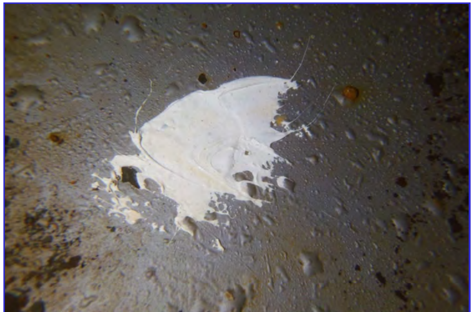
INTERIOR - CPUD - San Andaras Reservoir - Maintenance Inspection -247
