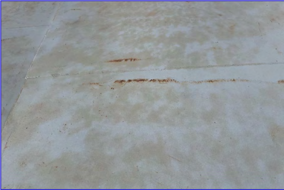
EXTERIOR - CPUD - San Andreas Reservoir - Maintenance Inspection -064
