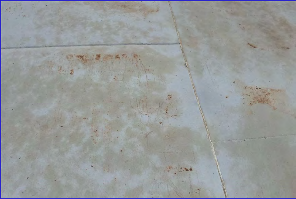
EXTERIOR - CPUD - San Andreas Reservoir - Maintenance Inspection -052
