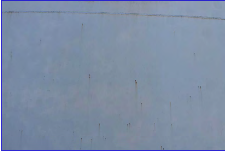
EXTERIOR - CPUD - Mokelumne Reservoir - Maintenance Inspection -112
