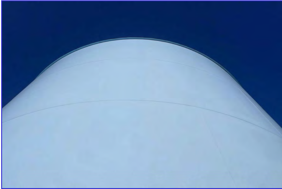
EXTERIOR - CPUD - Railroad Flat Reservoir - Maintenance Inspection -052
