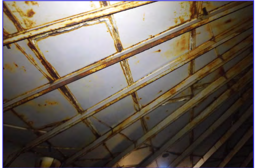
INTERIOR - CPUD - Mokelumne Hill Reservoir - Maintenance Inspection -017
