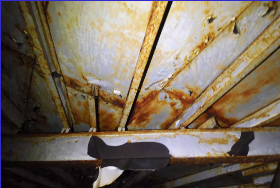
INTERIOR - CPUD - San Andaras Reservoir - Maintenance Inspection -092
