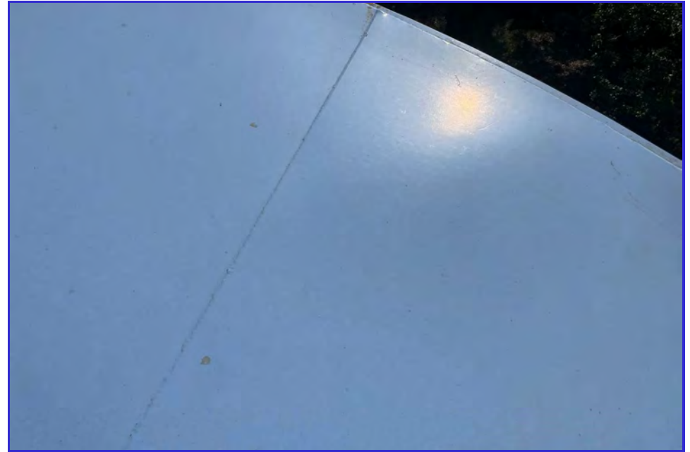
EXTERIOR - CPUD - Railroad Flat Reservoir - Maintenance Inspection -021
