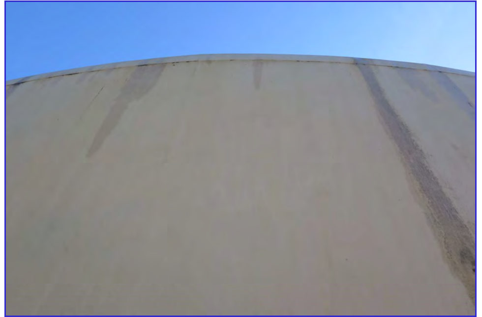
EXTERIOR - Calaveras Public Utility District - Clear Well Tank - Maintenance Inspection -093
