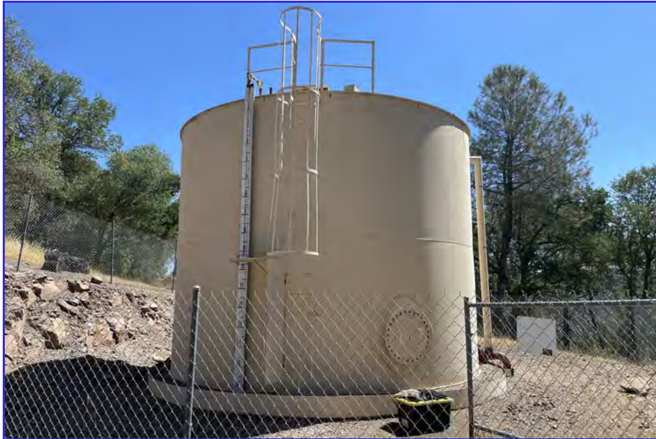
EXTERIOR - CPUD - Golden Hills - Maintenance Inspection
