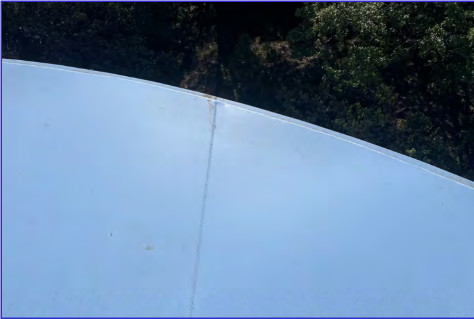
EXTERIOR - CPUD - Railroad Flat Reservoir - Maintenance Inspection -020
