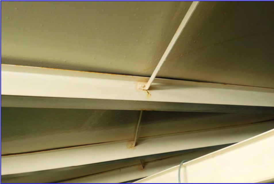
INTERIOR - CPUD - Railroad Flat Reservoir - Maintenance Inspection -016
