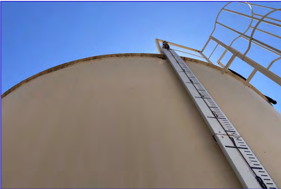
EXTERIOR - CPUD - Golden Hills - Maintenance Inspection -058
