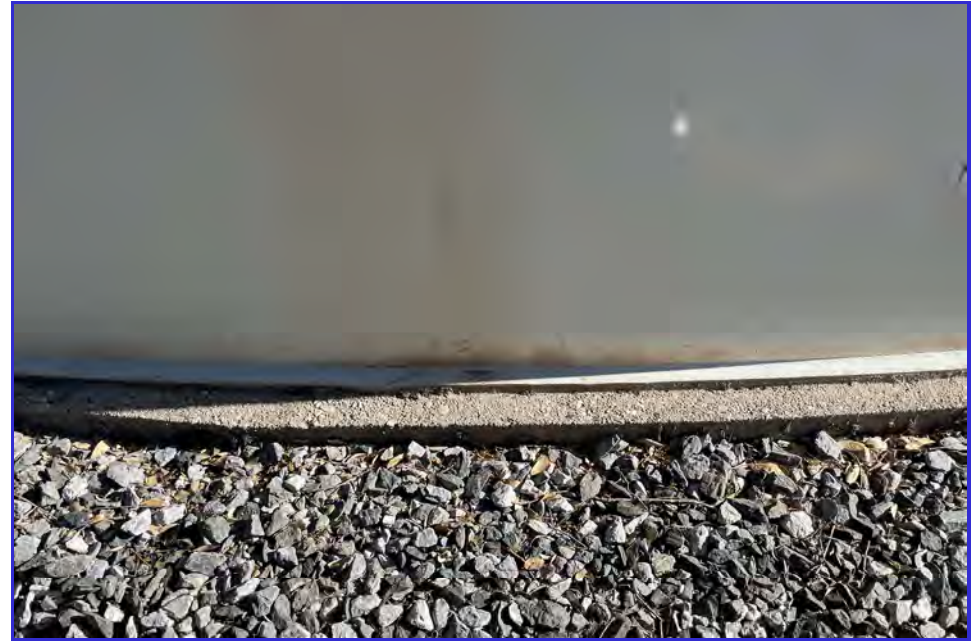
EXTERIOR - CPUD - Mokelumne Reservoir - Maintenance Inspection -157
