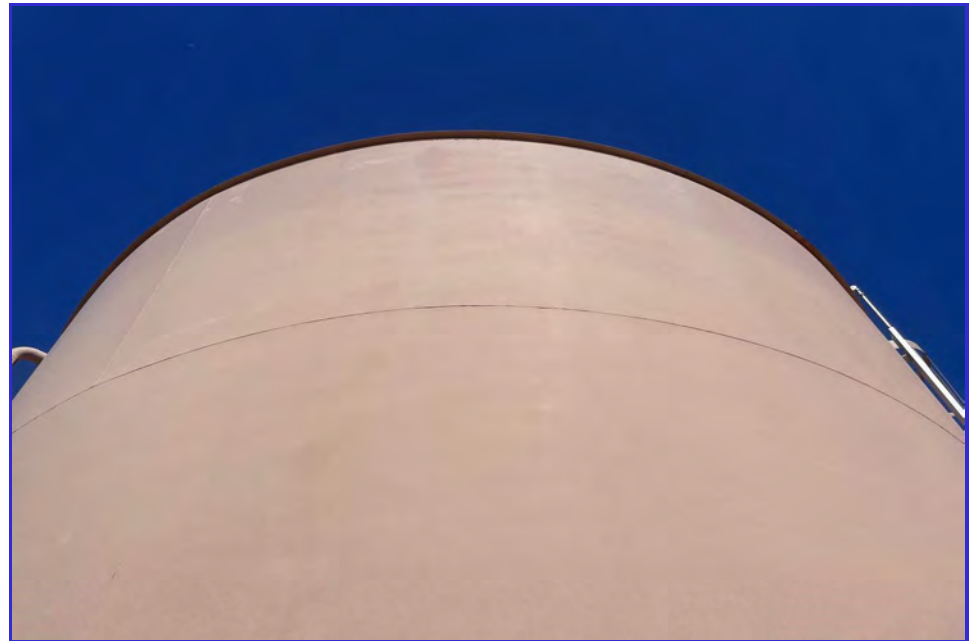
EXTERIOR - CPUD - Paloma Reservoir - Maintenance Inspection -075
