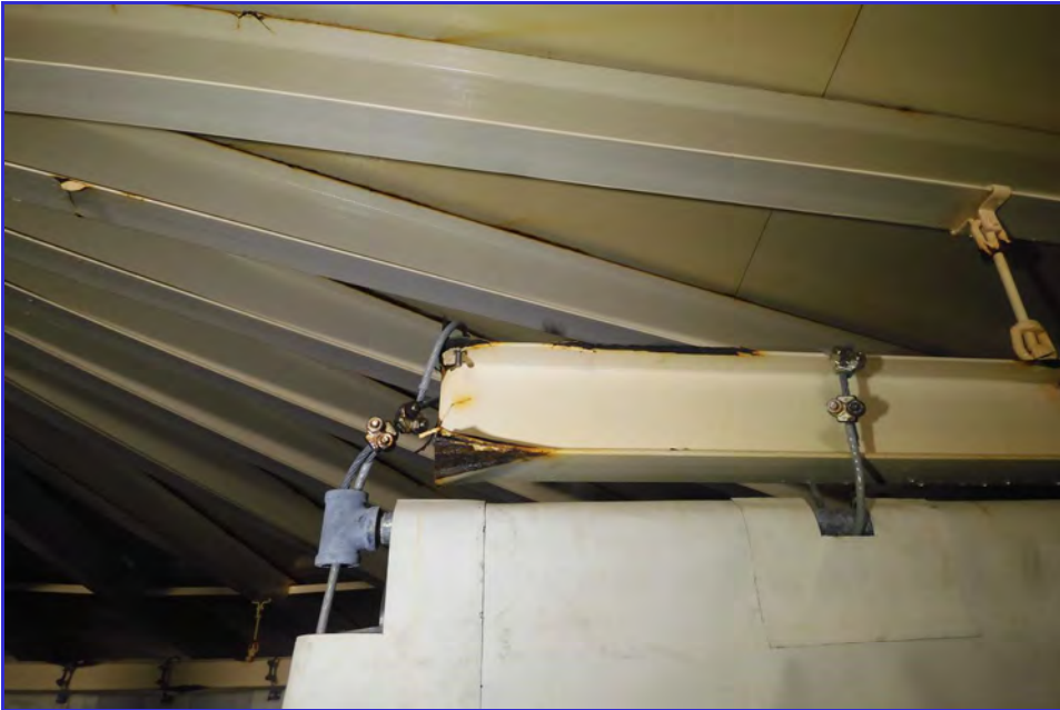
INTERIOR - CPUD - Railroad Flat Reservoir - Maintenance Inspection -032
