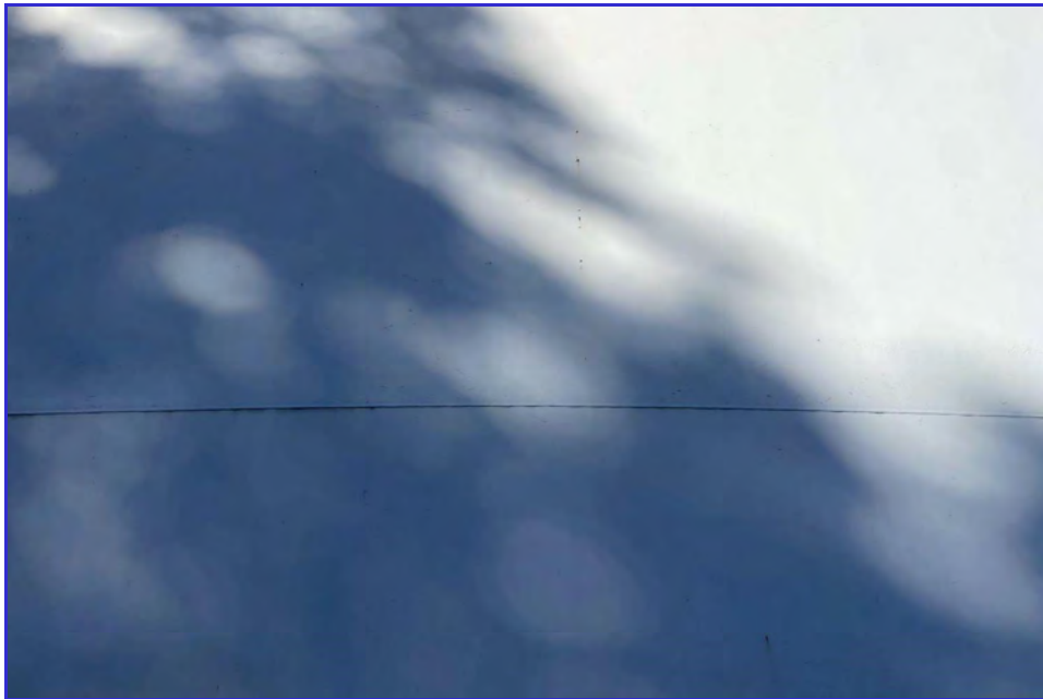
EXTERIOR - CPUD - Mokelumne Reservoir - Maintenance Inspection -090
