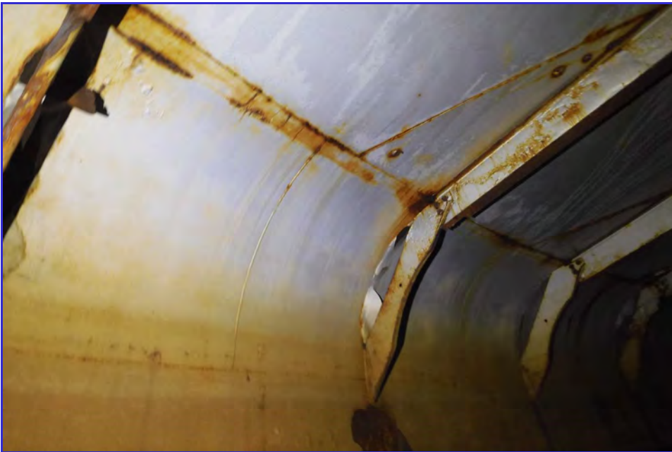
INTERIOR - CPUD - San Andaras Reservoir - Maintenance Inspection -098
