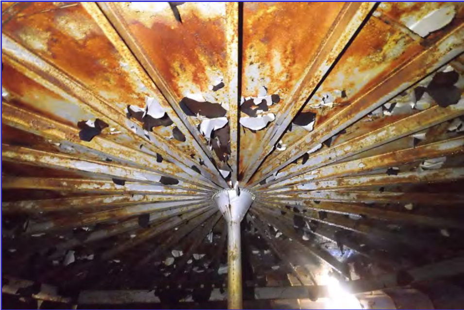
INTERIOR - CPUD - San Andaras Reservoir - Maintenance Inspection -076
