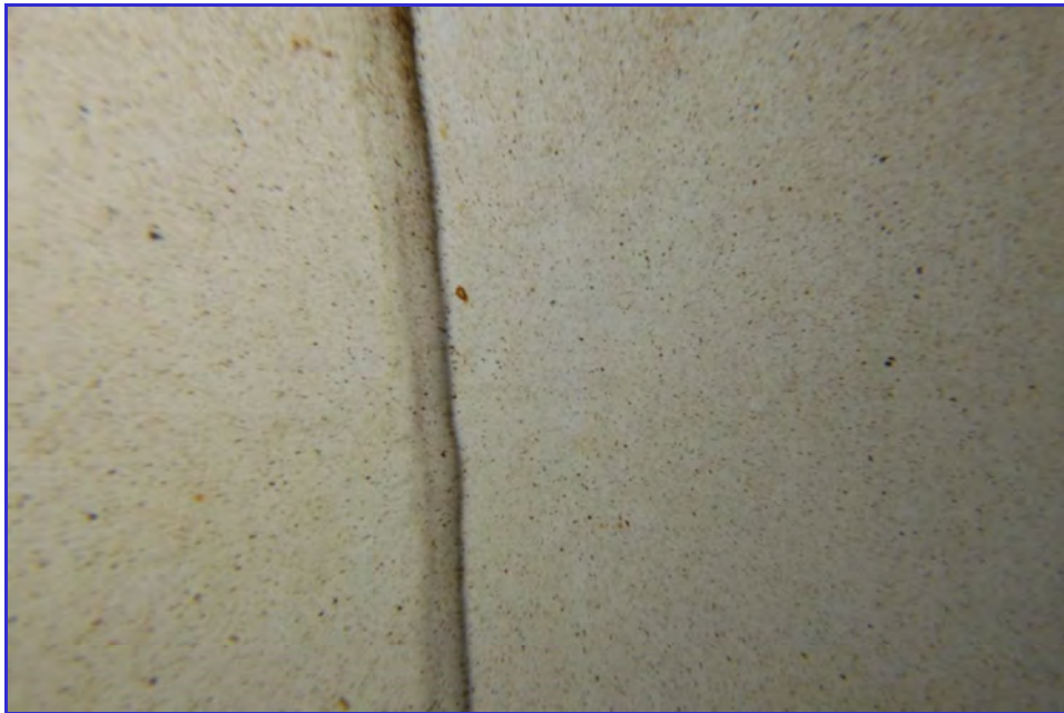
INTERIOR - CPUD - Railroad Flat Reservoir - Maintenance Inspection -154
