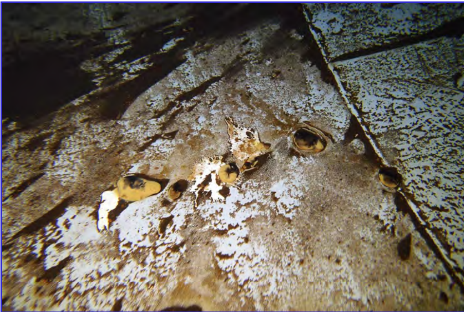
INTERIOR - CPUD - Mokelumne Hill Reservoir - Maintenance Inspection -130
