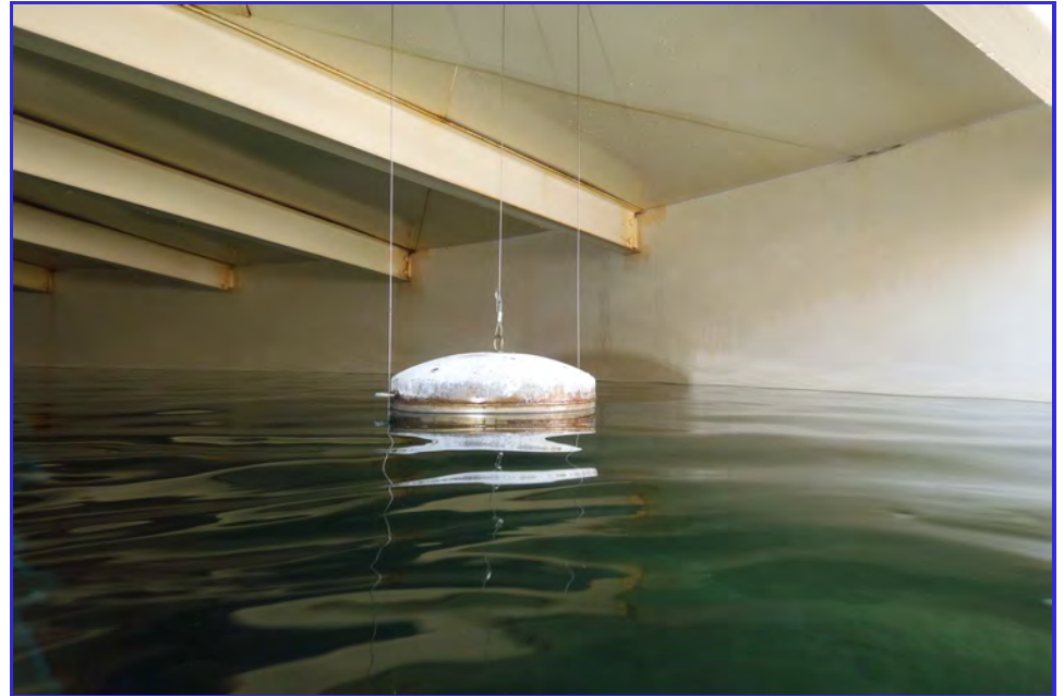
INTERIOR - CPUD - Railroad Flat Reservoir - Maintenance Inspection -005
