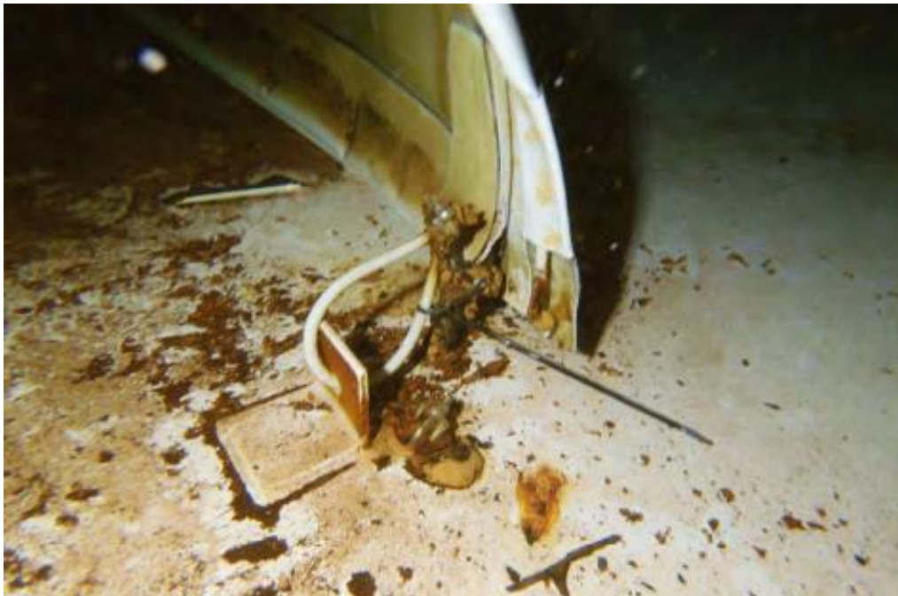
Figure 9-2. Rail Road Flat Tank Interior Floor Example
