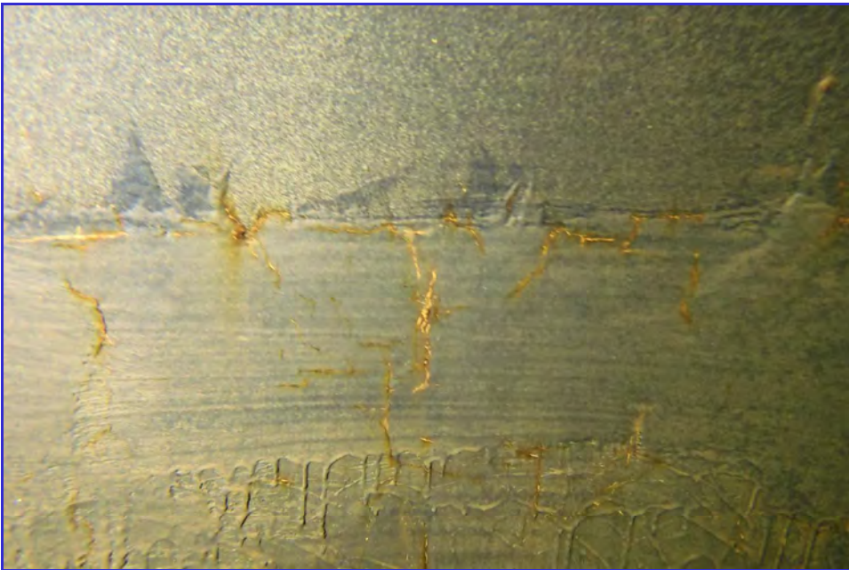
INTERIOR - CPUD - Paloma Reservoir - Maintenance Inspection -066
