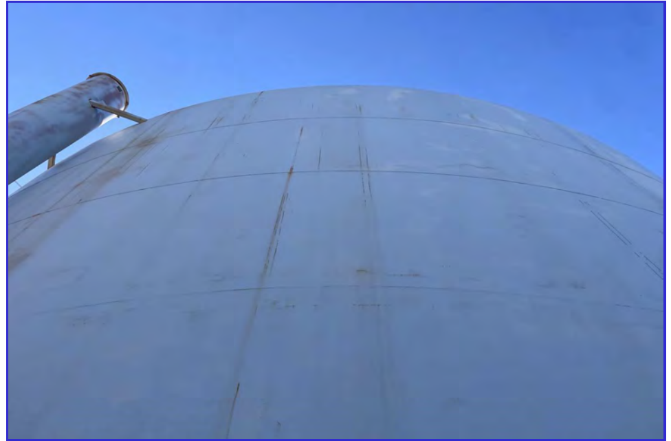
EXTERIOR - CPUD - Mokelumne Reservoir - Maintenance Inspection -125
