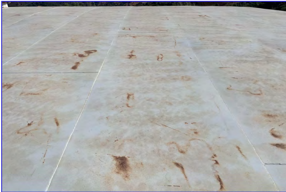
EXTERIOR - CPUD - San Andreas Reservoir - Maintenance Inspection -030
