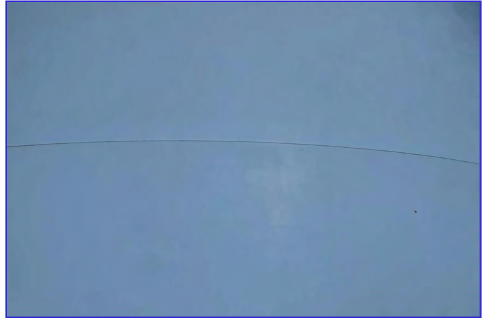
EXTERIOR - CPUD - Railroad Flat Reservoir - Maintenance Inspection -053
