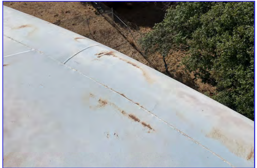
EXTERIOR - CPUD - Mokelumne Reservoir - Maintenance Inspection -063
