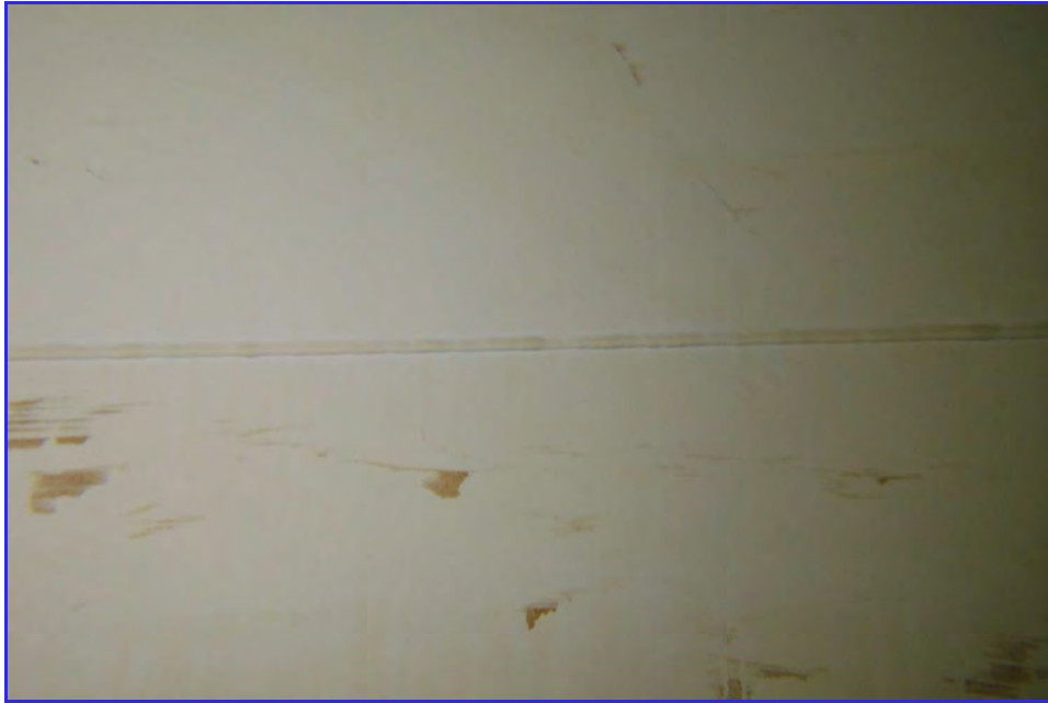
INTERIOR - CPUD - Railroad Flat Reservoir - Maintenance Inspection -072
