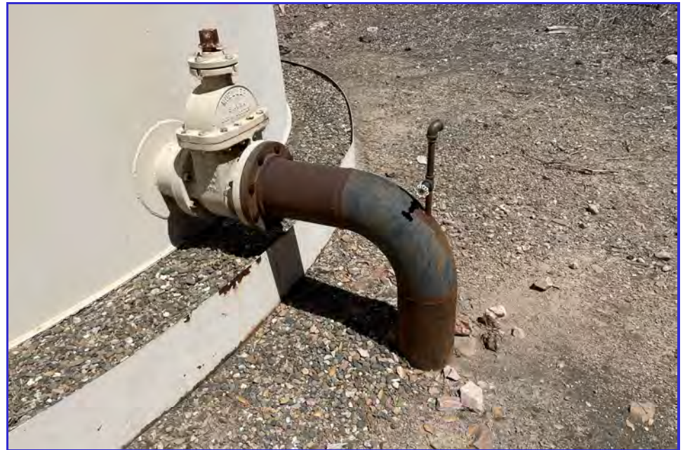
EXTERIOR - CPUD - Golden Hills - Maintenance Inspection -043
