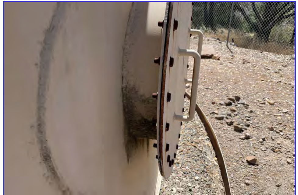
EXTERIOR - CPUD - Golden Hills - Maintenance Inspection -063
