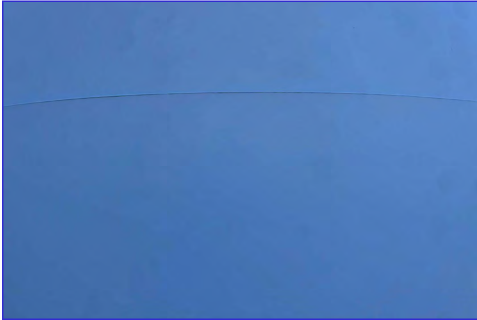
EXTERIOR - CPUD - Railroad Flat Reservoir - Maintenance Inspection -060
