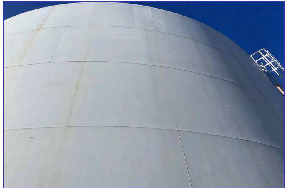
EXTERIOR - CPUD - Mokelumne Reservoir - Maintenance Inspection -175
