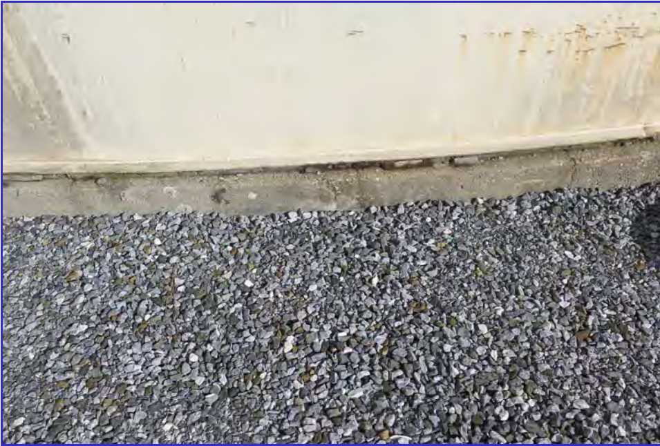
EXTERIOR - Calaveras Public Utility District - Clear Well Tank - Maintenance Inspection -072
