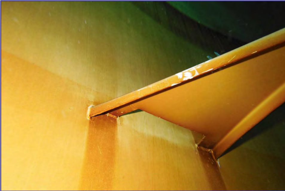
INTERIOR - CPUD - Railroad Flat Reservoir - Maintenance Inspection -172
