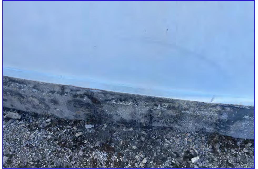
EXTERIOR - CPUD - San Andreas Reservoir - Maintenance Inspection -189
