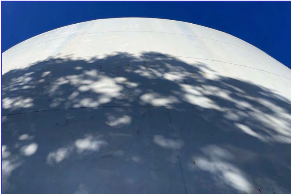
EXTERIOR - CPUD - Mokelumne Reservoir - Maintenance Inspection -168
