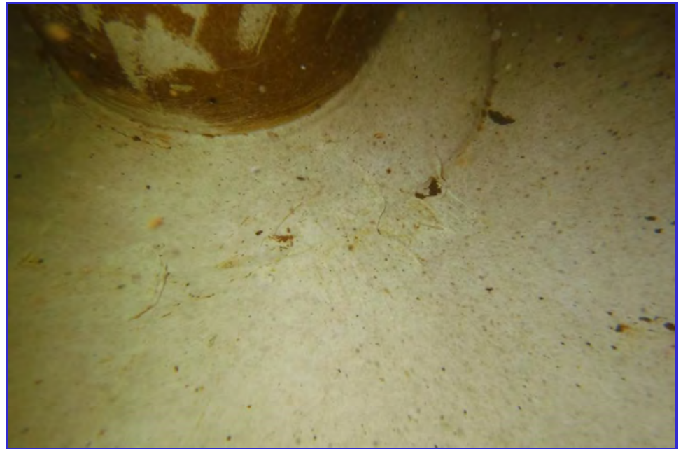
INTERIOR - CPUD - Railroad Flat Reservoir - Maintenance Inspection -163
