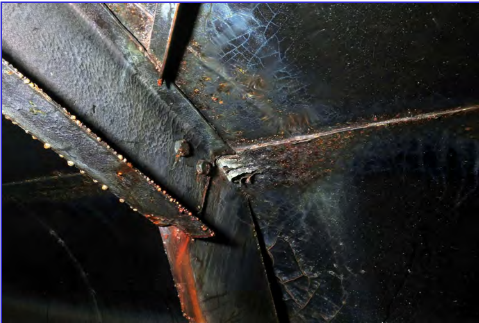
INTERIOR - Calaveras Public Utility District - Clear Well Tank - Maintenance Inspection -042
