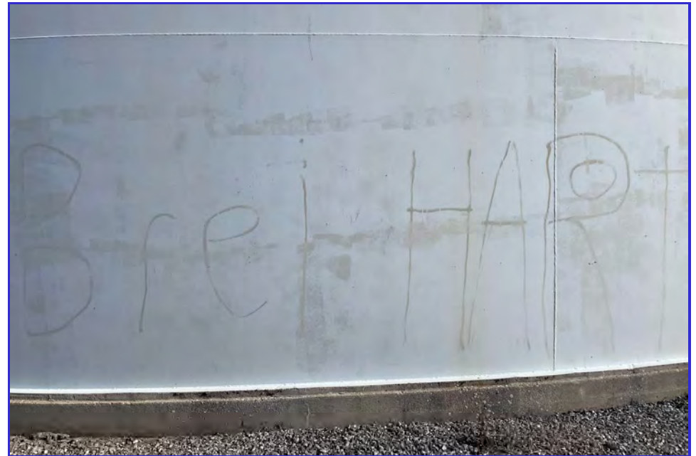
EXTERIOR - CPUD - San Andreas Reservoir - Maintenance Inspection -155
