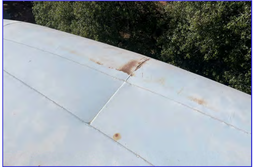
EXTERIOR - CPUD - Mokelumne Reservoir - Maintenance Inspection -065
