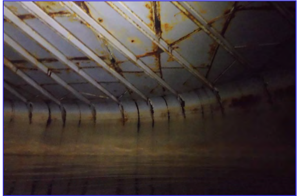
INTERIOR - CPUD - Mokelumne Hill Reservoir - Maintenance Inspection -021
