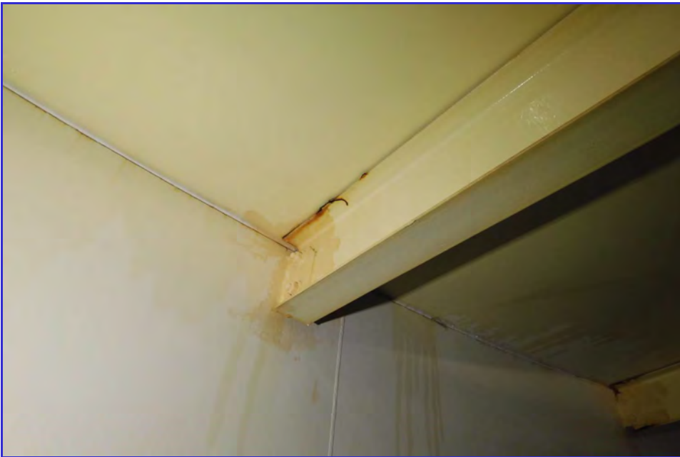
INTERIOR - CPUD - Railroad Flat Reservoir - Maintenance Inspection -054
