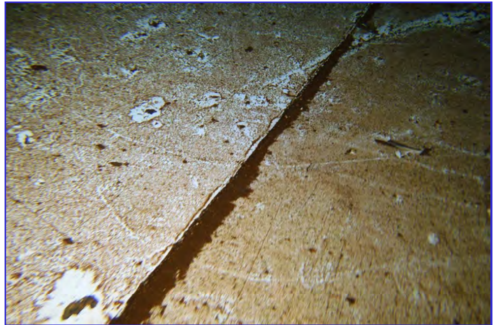
INTERIOR - CPUD - Mokelumne Hill Reservoir - Maintenance Inspection -135
