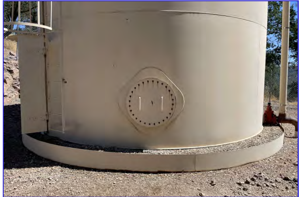
EXTERIOR - CPUD - Golden Hills - Maintenance Inspection -065
