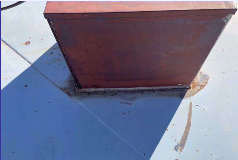
EXTERIOR - CPUD - Mokelumne Reservoir - Maintenance Inspection -074
