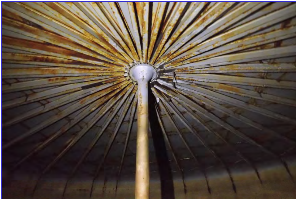
INTERIOR - CPUD - Mokelumne Hill Reservoir - Maintenance Inspection -054
