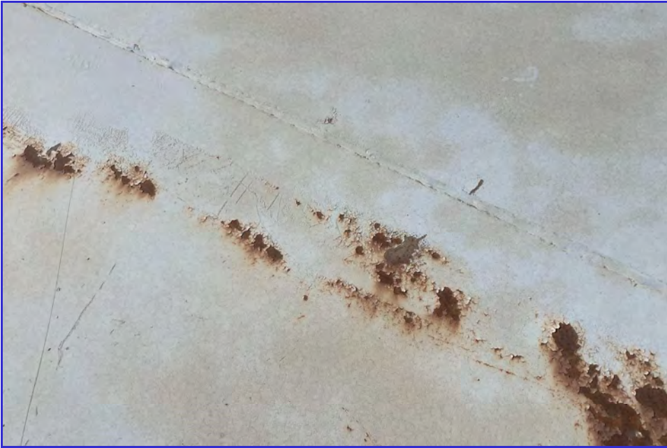
EXTERIOR - CPUD - San Andreas Reservoir - Maintenance Inspection -068
