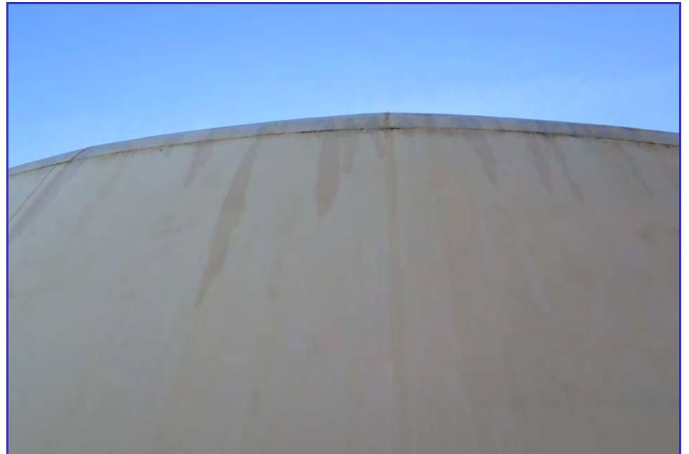
EXTERIOR - Calaveras Public Utility District - Clear Well Tank - Maintenance Inspection -103
