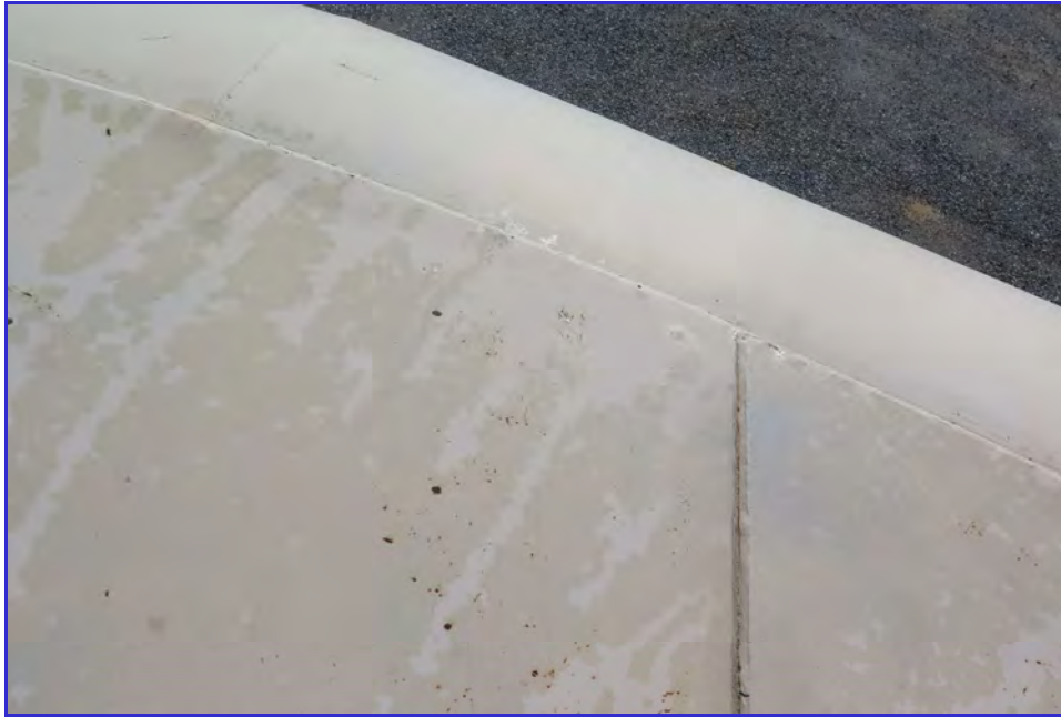
EXTERIOR - Calaveras Public Utility District - Clear Well Tank - Maintenance Inspection -040
