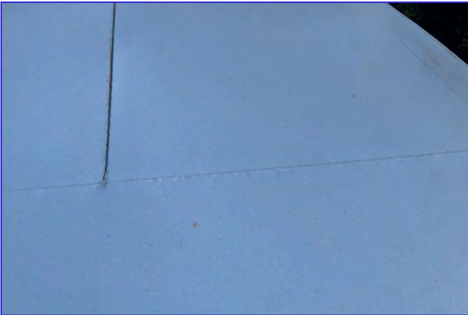
EXTERIOR - CPUD - Railroad Flat Reservoir - Maintenance Inspection -018
