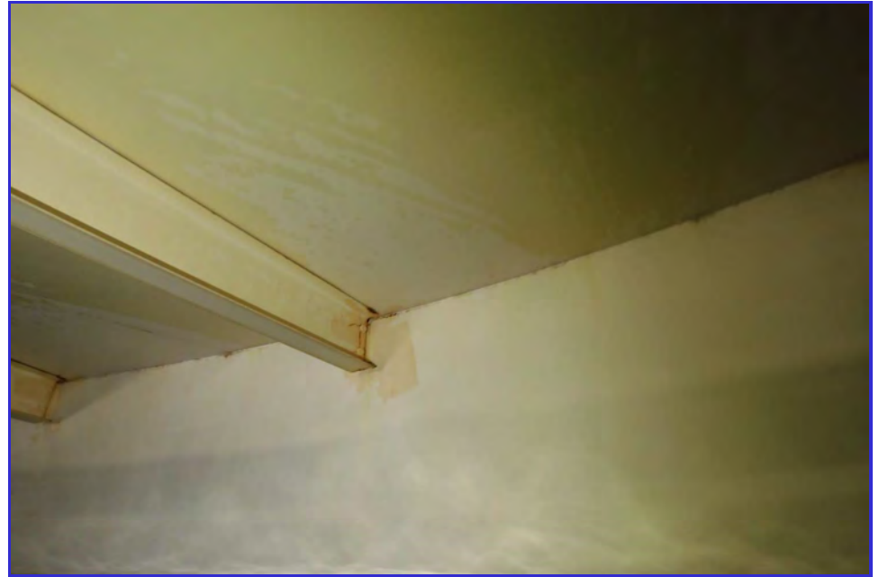
INTERIOR - CPUD - Railroad Flat Reservoir - Maintenance Inspection -061
