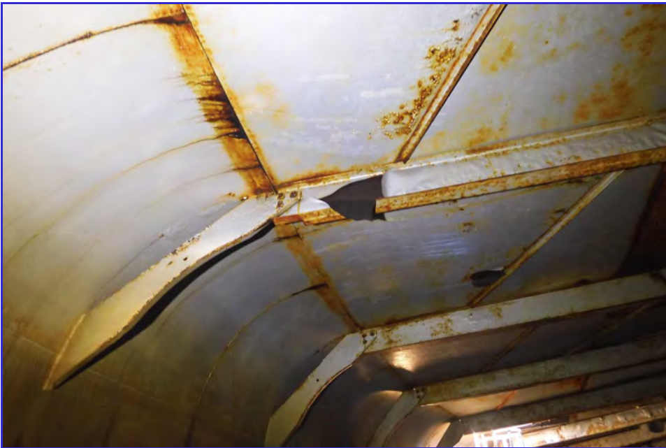
INTERIOR - CPUD - San Andaras Reservoir - Maintenance Inspection -018
