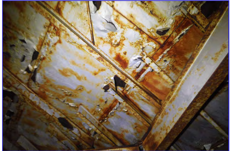
INTERIOR - CPUD - San Andaras Reservoir - Maintenance Inspection -073
