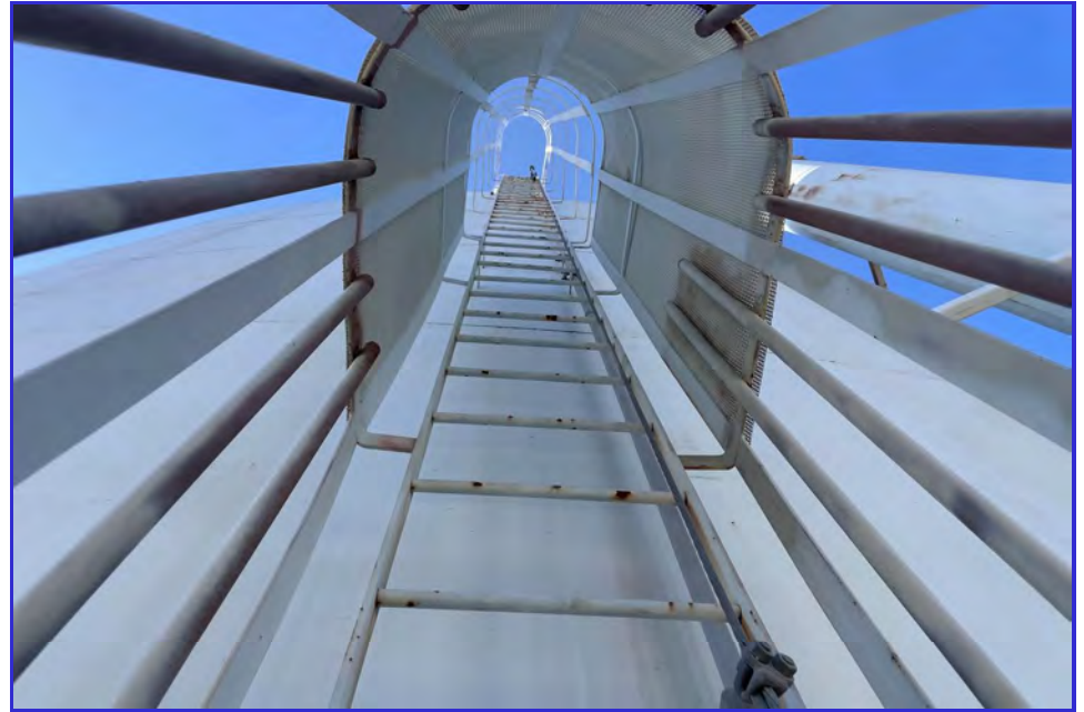
EXTERIOR - CPUD - Mokelumne Reservoir - Maintenance Inspection -137
