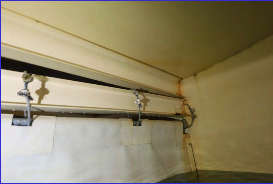
INTERIOR - CPUD - Railroad Flat Reservoir - Maintenance Inspection -028
