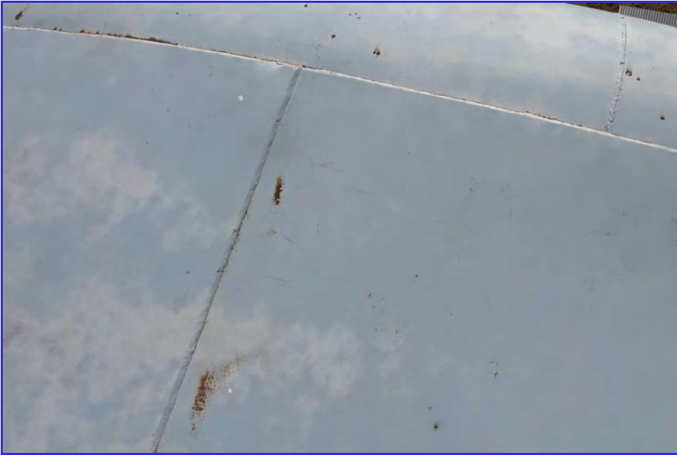
EXTERIOR - CPUD - Mokelumne Reservoir - Maintenance Inspection -056
