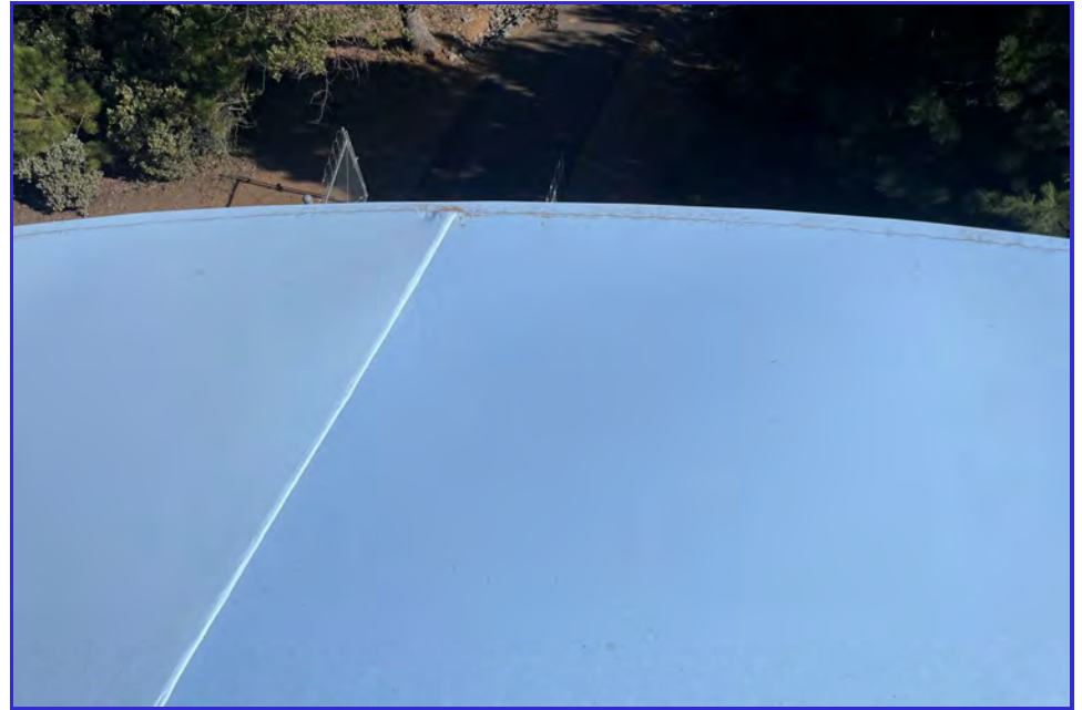
EXTERIOR - CPUD - Railroad Flat Reservoir - Maintenance Inspection -009
