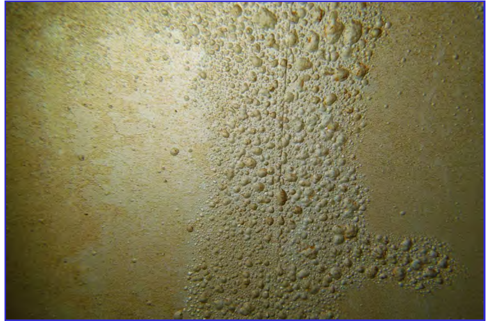
INTERIOR - CPUD - San Andaras Reservoir - Maintenance Inspection -121
