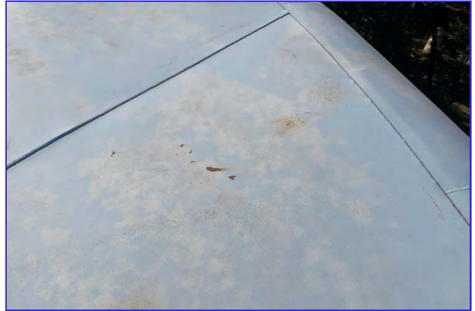
EXTERIOR - CPUD - Mokelumne Reservoir - Maintenance Inspection -069
