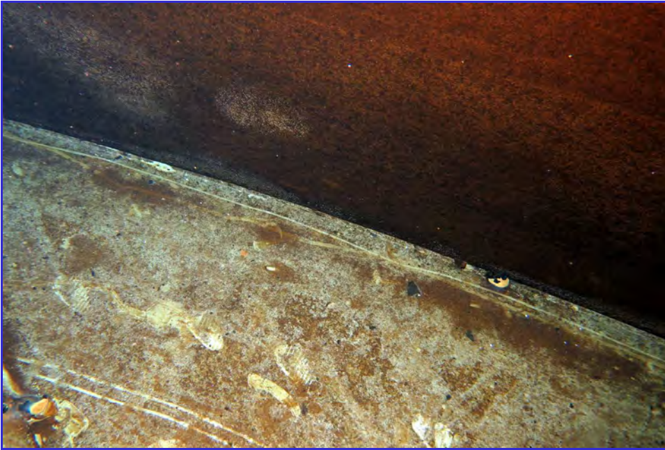
INTERIOR - Calaveras Public Utility District - Clear Well Tank - Maintenance Inspection -084
