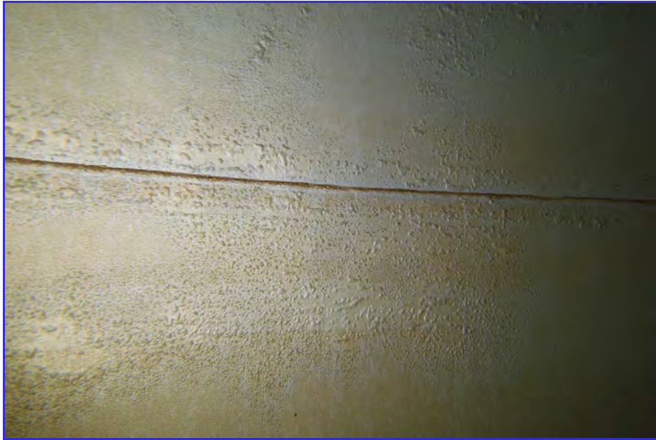
INTERIOR - CPUD - San Andaras Reservoir - Maintenance Inspection -116
