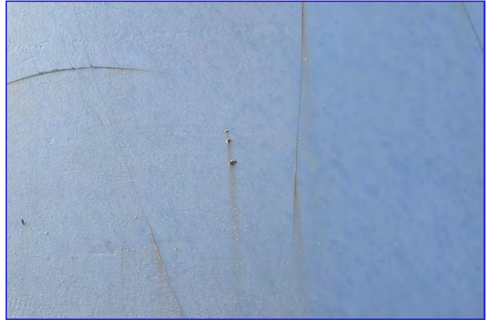
EXTERIOR - CPUD - San Andreas Reservoir - Maintenance Inspection -117
