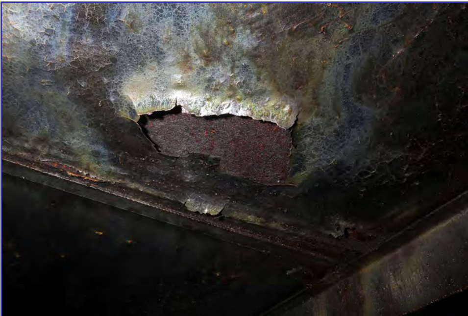
INTERIOR - Calaveras Public Utility District - Clear Well Tank - Maintenance Inspection -054
