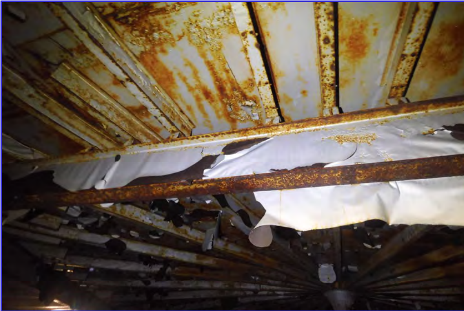
INTERIOR - CPUD - San Andaras Reservoir - Maintenance Inspection -052
