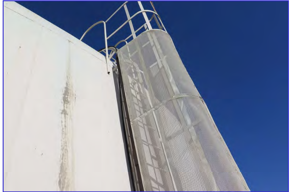
EXTERIOR - Calaveras Public Utility District - Clear Well Tank - Maintenance Inspection -055
