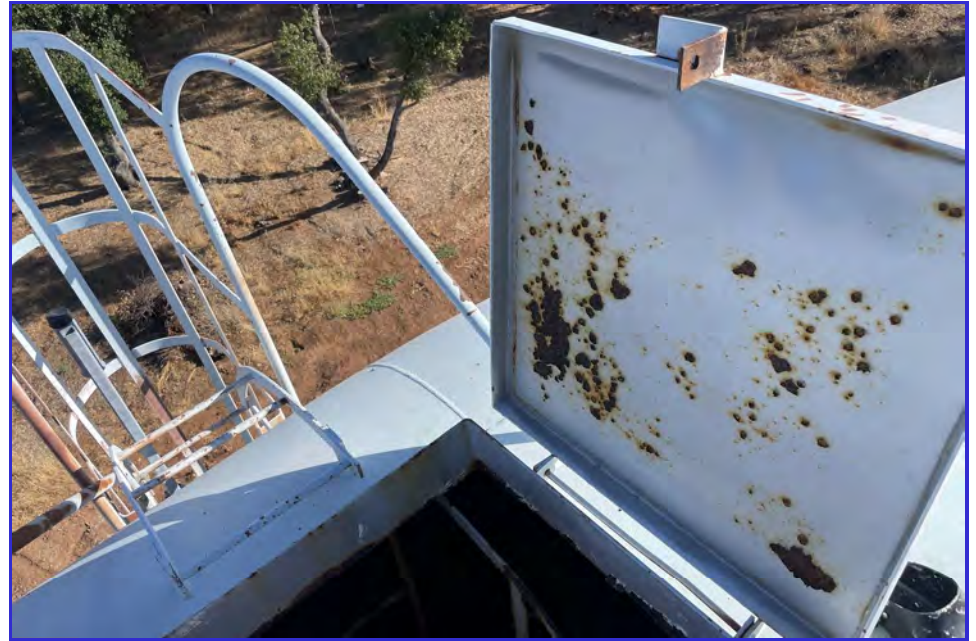
EXTERIOR - CPUD - Mokelumne Reservoir - Maintenance Inspection -001
