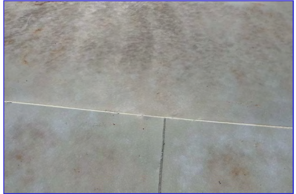
EXTERIOR - CPUD - San Andreas Reservoir - Maintenance Inspection -013
