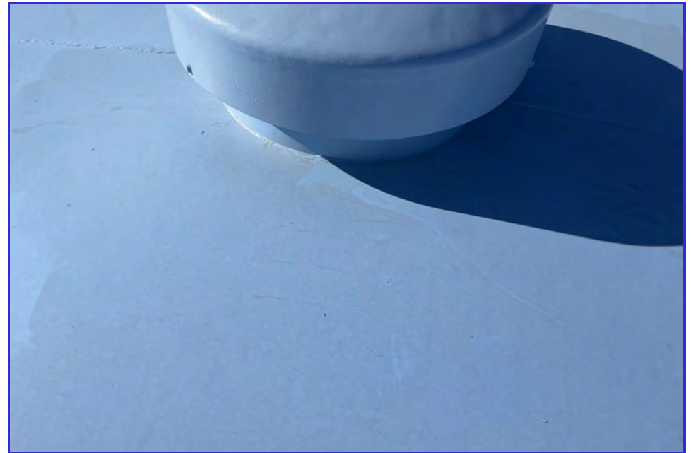
EXTERIOR - CPUD - Railroad Flat Reservoir - Maintenance Inspection -027
