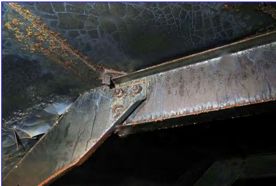
INTERIOR - Calaveras Public Utility District - Clear Well Tank - Maintenance Inspection -038
