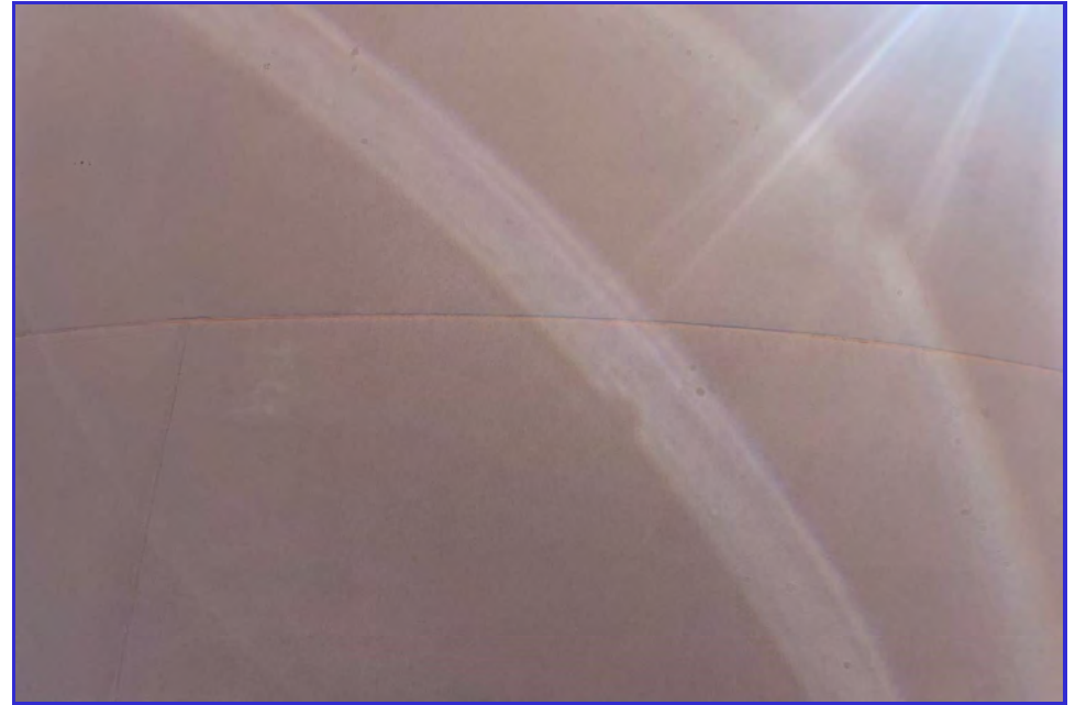
EXTERIOR - CPUD - Paloma Reservoir - Maintenance Inspection -041
