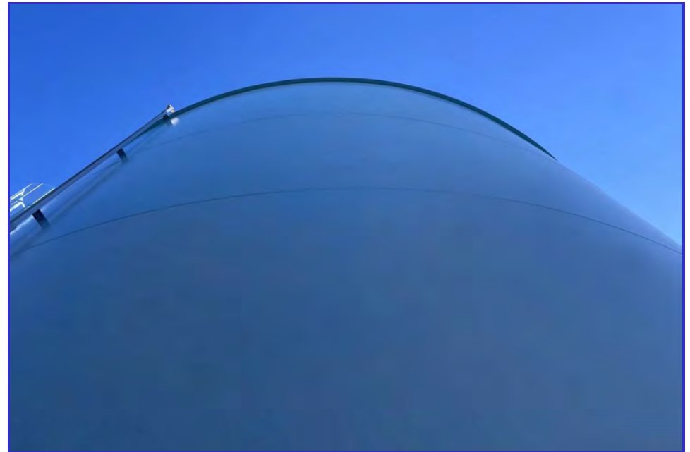
EXTERIOR - CPUD - Railroad Flat Reservoir - Maintenance Inspection -071
