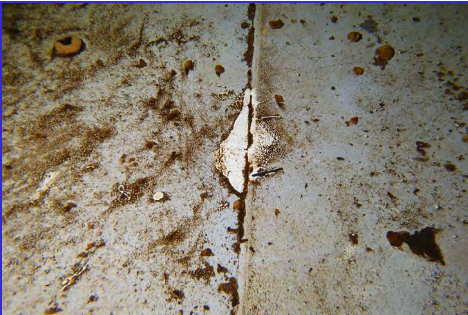
INTERIOR - CPUD - Mokelumne Hill Reservoir - Maintenance Inspection -162
