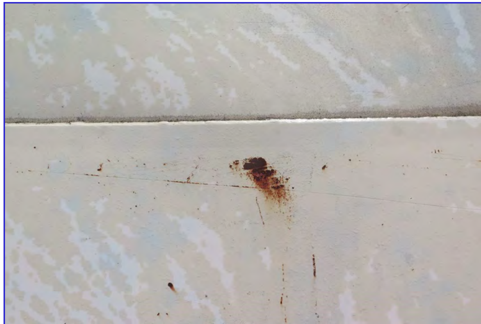
EXTERIOR - Calaveras Public Utility District - Clear Well Tank - Maintenance Inspection -021
