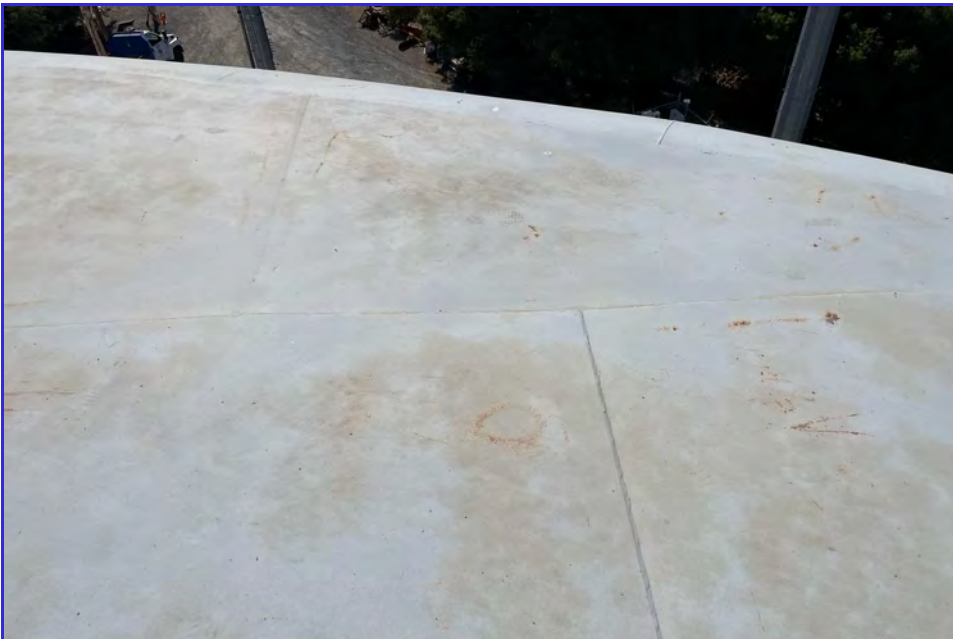
EXTERIOR - CPUD - San Andreas Reservoir - Maintenance Inspection -098
