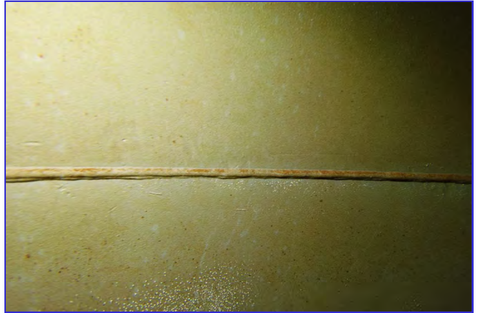
INTERIOR - CPUD - Mokelumne Hill Reservoir - Maintenance Inspection -097
