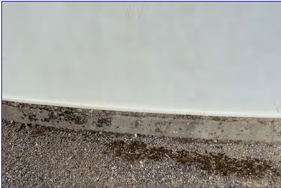
EXTERIOR - CPUD - San Andreas Reservoir - Maintenance Inspection -126
