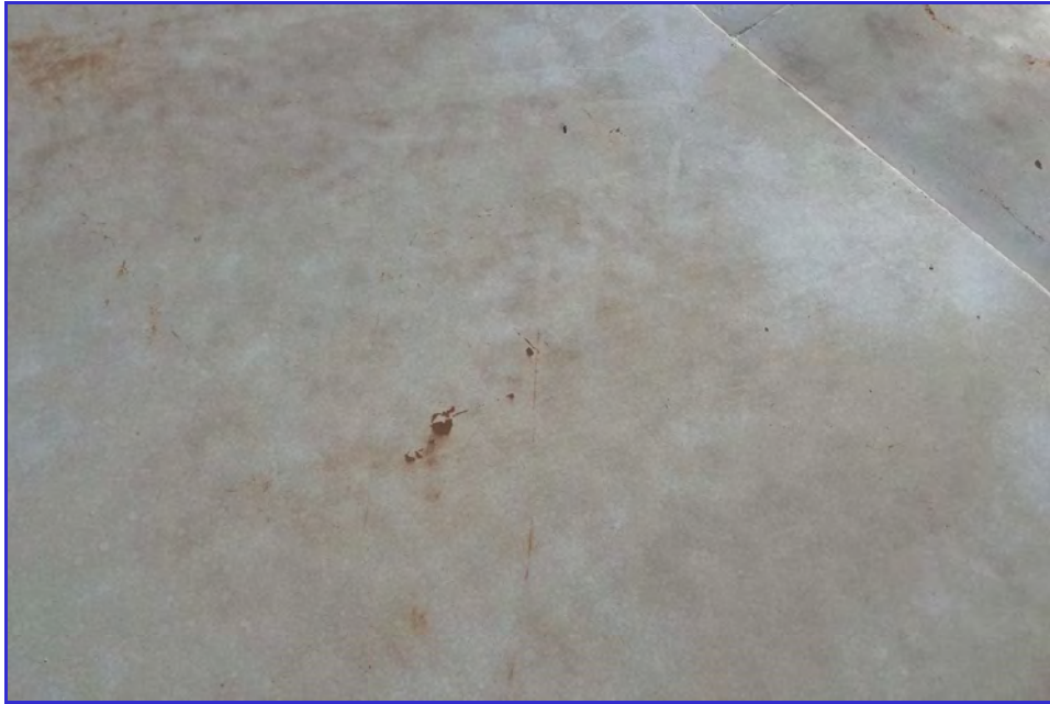
EXTERIOR - CPUD - San Andreas Reservoir - Maintenance Inspection -016
