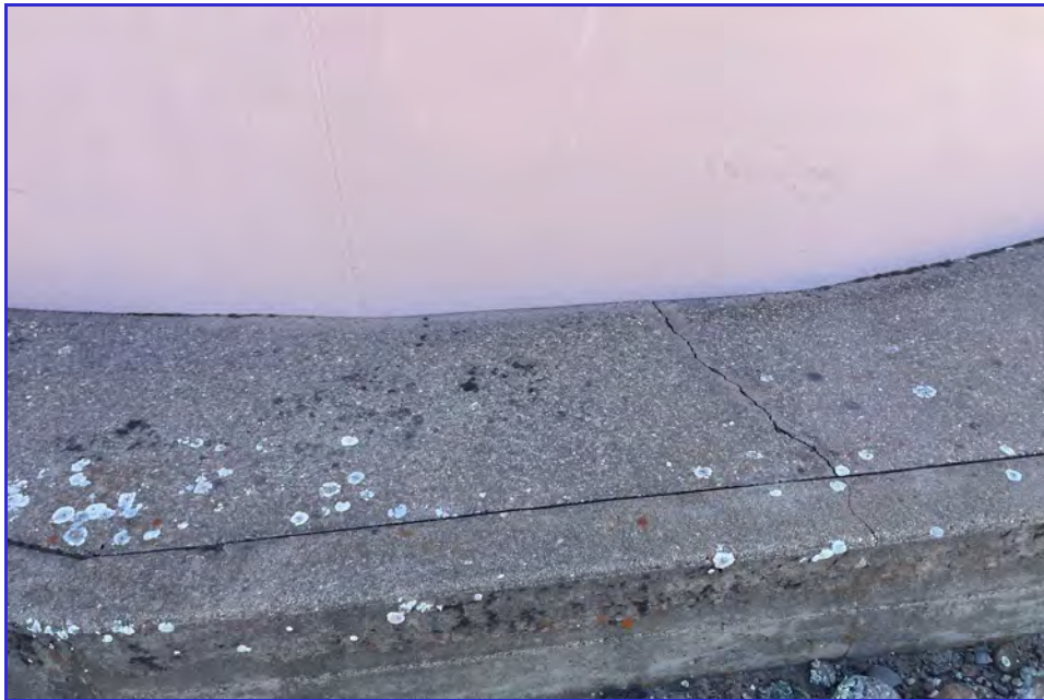
EXTERIOR - CPUD - Paloma Reservoir - Maintenance Inspection -078
