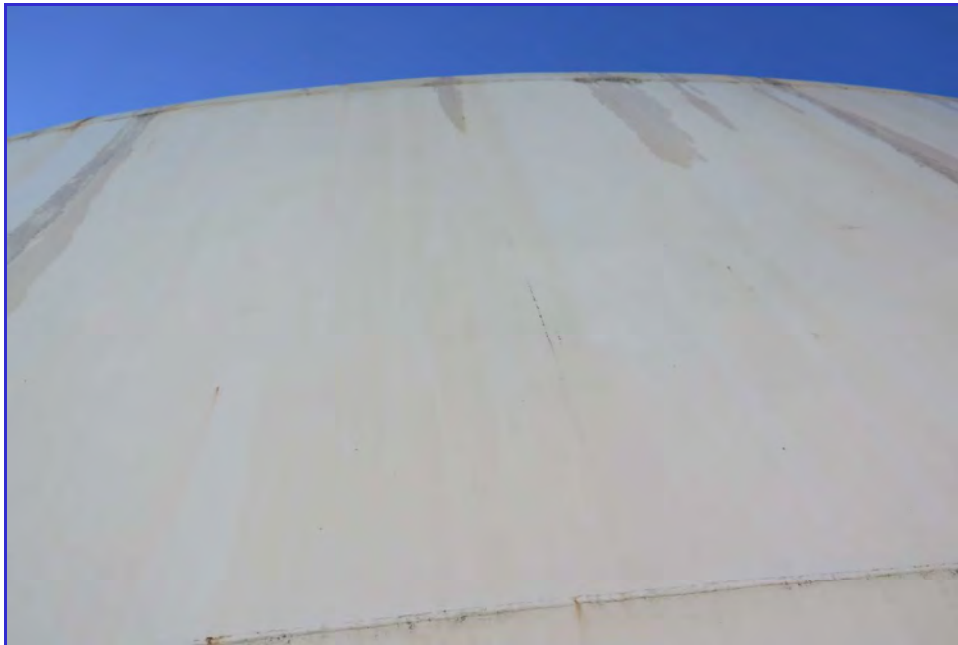
EXTERIOR - Calaveras Public Utility District - Clear Well Tank - Maintenance Inspection -110
