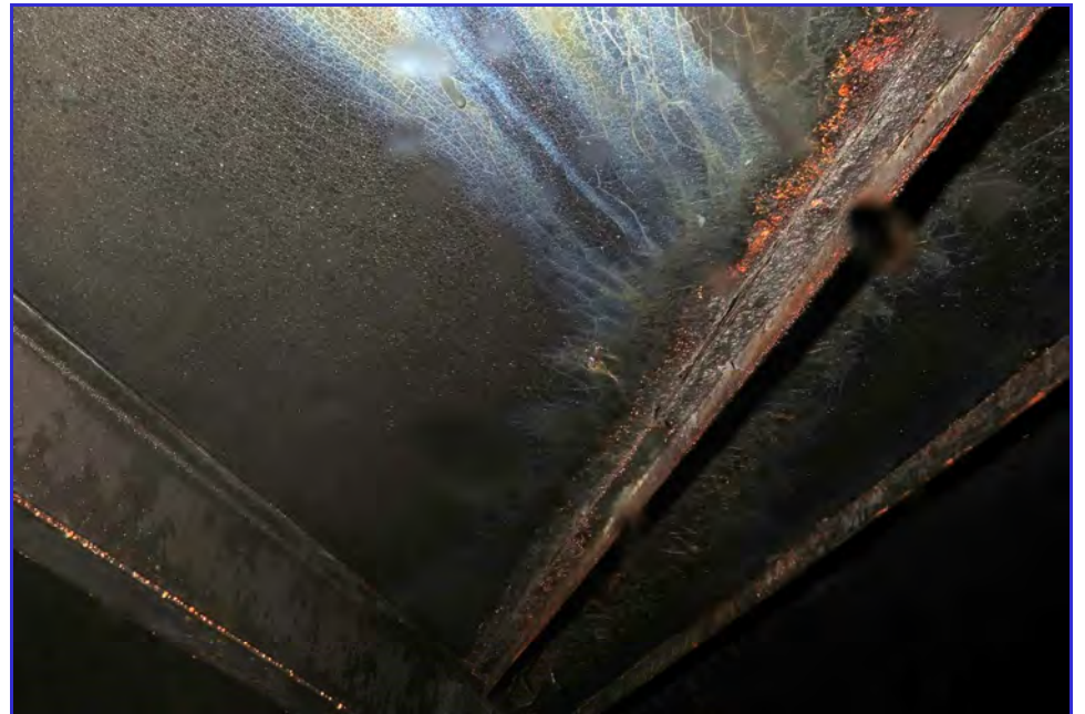
INTERIOR - Calaveras Public Utility District - Clear Well Tank - Maintenance Inspection -031
