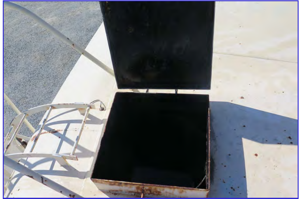
EXTERIOR - Calaveras Public Utility District - Clear Well Tank - Maintenance Inspection -001
