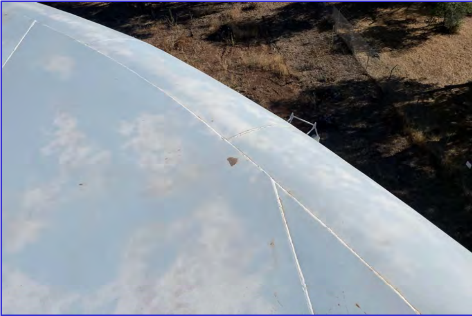
EXTERIOR - CPUD - Mokelumne Reservoir - Maintenance Inspection -052
