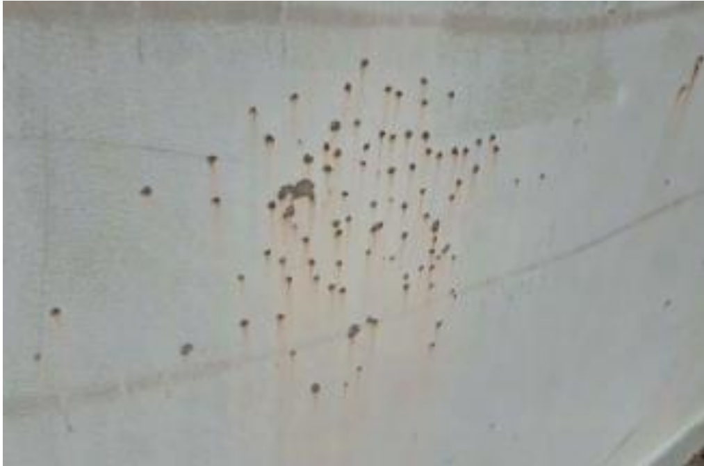
Figure 9-16. Example of San Andreas Tank Exterior Shell
