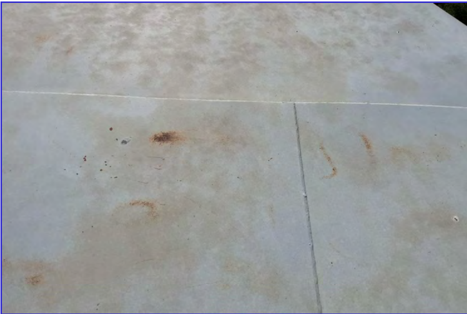
EXTERIOR - CPUD - San Andreas Reservoir - Maintenance Inspection -042
