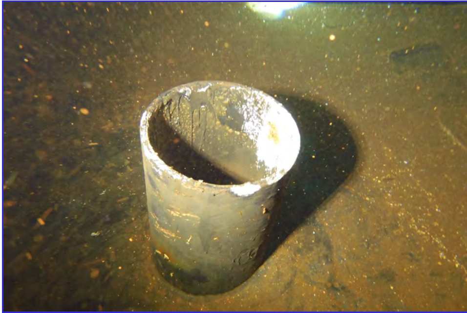
INTERIOR - CPUD - Paloma Reservoir - Maintenance Inspection -140
