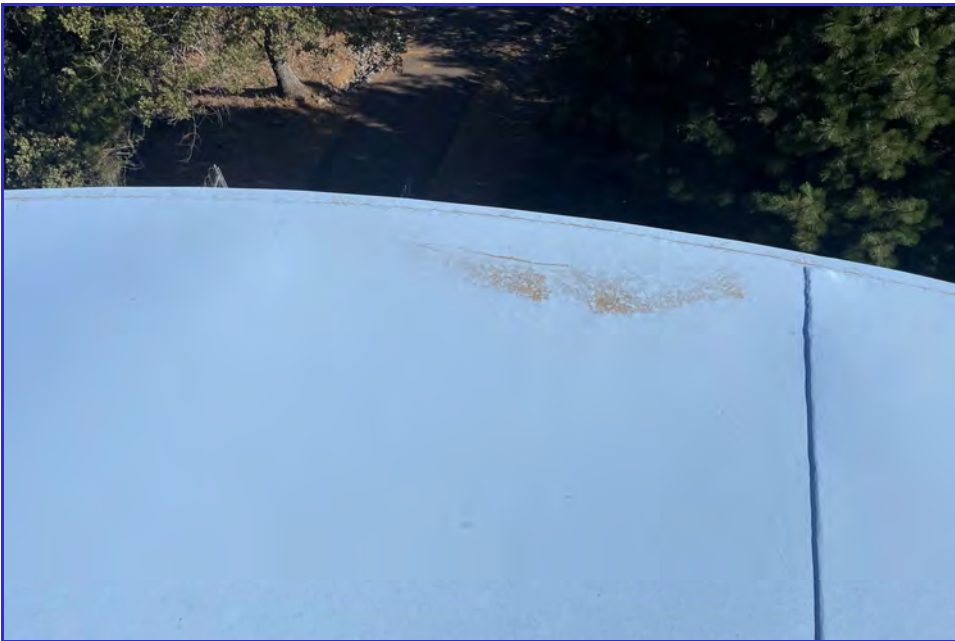
EXTERIOR - CPUD - Railroad Flat Reservoir - Maintenance Inspection -010
