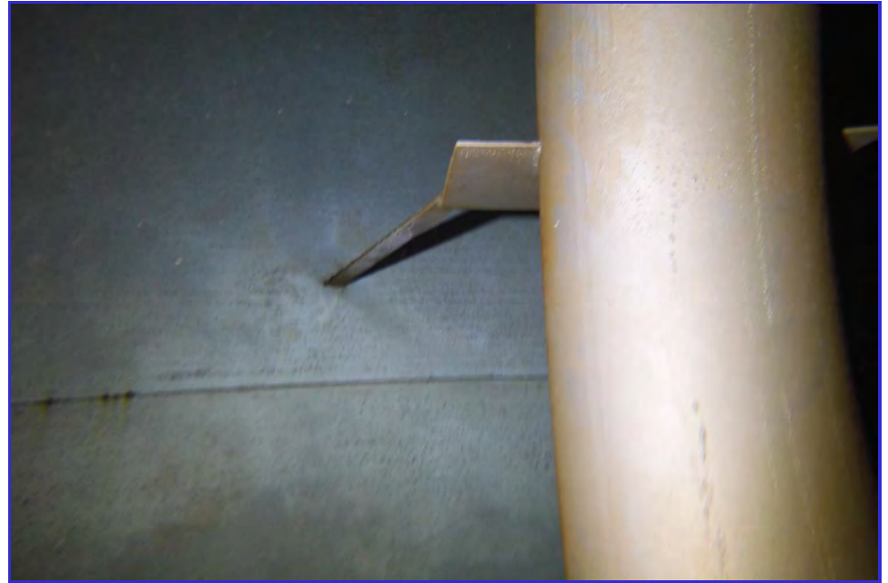
INTERIOR - CPUD - San Andaras Reservoir - Maintenance Inspection -145
