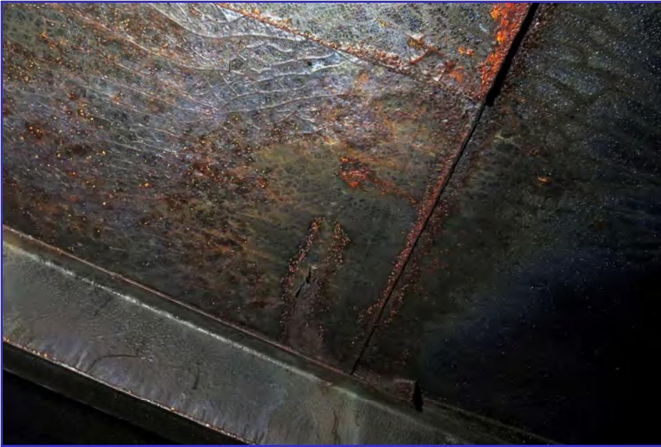
INTERIOR - Calaveras Public Utility District - Clear Well Tank - Maintenance Inspection -044
