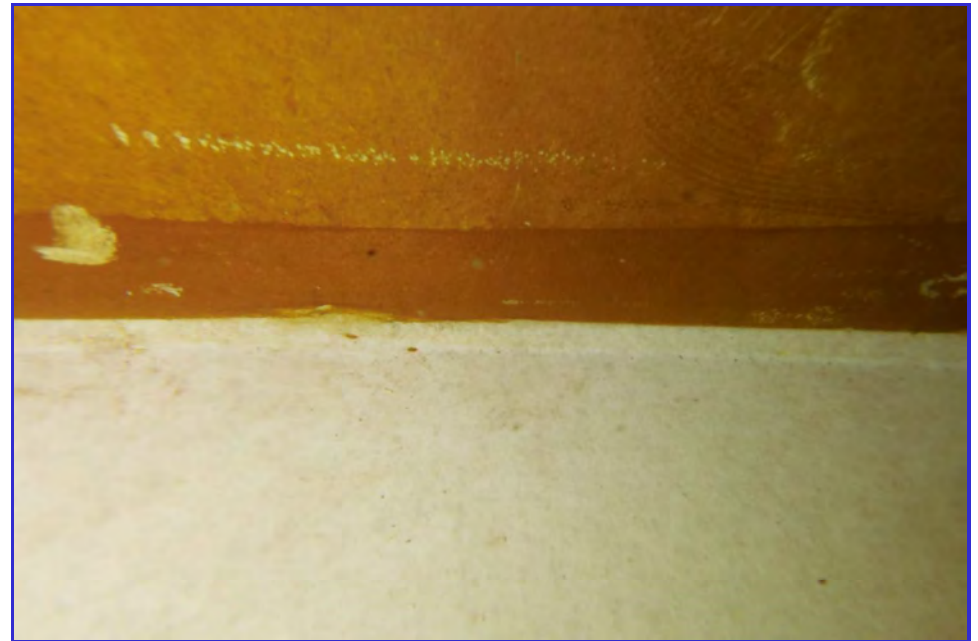
INTERIOR - CPUD - Railroad Flat Reservoir - Maintenance Inspection -115
