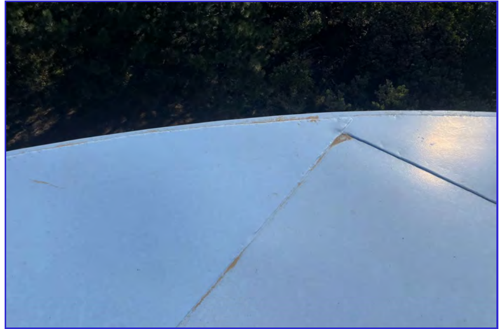
EXTERIOR - CPUD - Railroad Flat Reservoir - Maintenance Inspection -013
