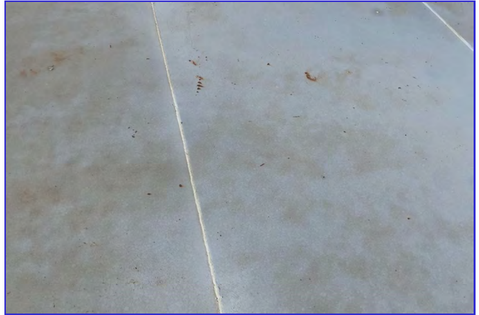
EXTERIOR - CPUD - San Andreas Reservoir - Maintenance Inspection -069
