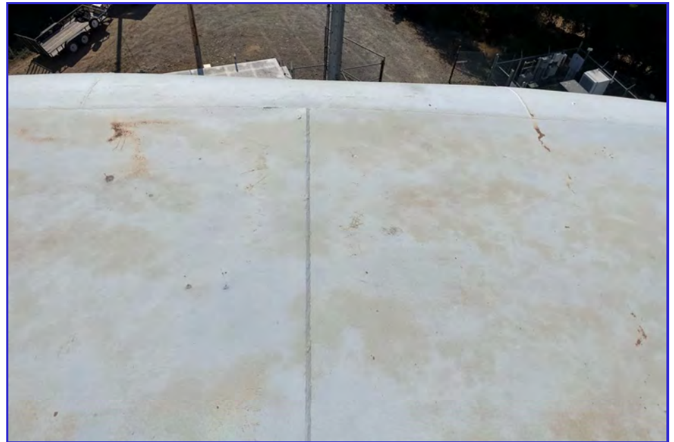
EXTERIOR - CPUD - San Andreas Reservoir - Maintenance Inspection -095
