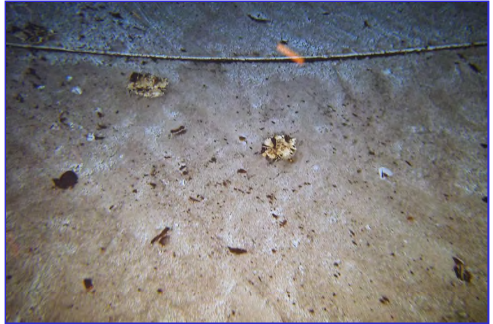
INTERIOR - CPUD - Mokelumne Hill Reservoir - Maintenance Inspection -129
