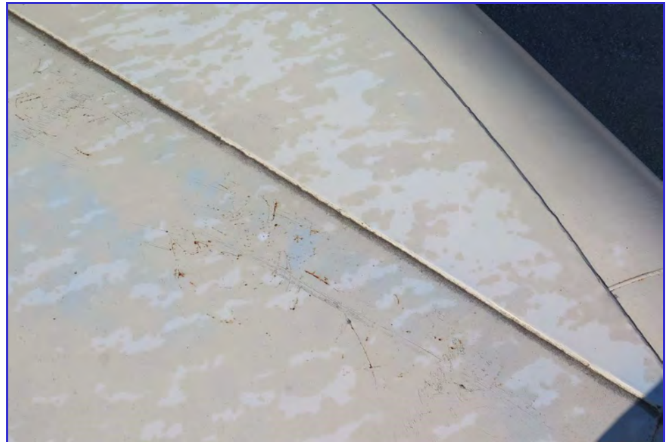
EXTERIOR - Calaveras Public Utility District - Clear Well Tank - Maintenance Inspection -015
