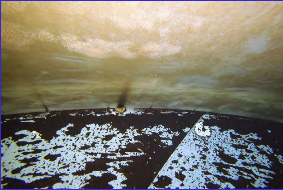
INTERIOR - CPUD - Mokelumne Hill Reservoir - Maintenance Inspection -076
