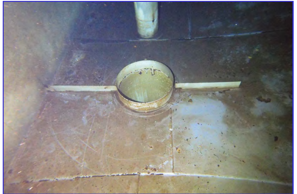
INTERIOR - CPUD - San Andaras Reservoir - Maintenance Inspection -183
