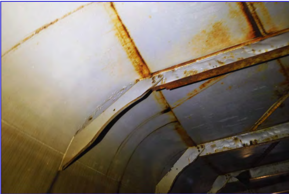
INTERIOR - CPUD - San Andaras Reservoir - Maintenance Inspection -022
