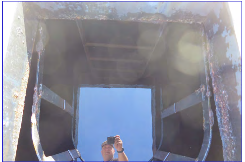
EXTERIOR - Calaveras Public Utility District - Clear Well Tank - Maintenance Inspection -003
