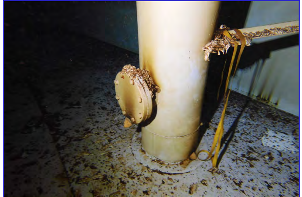
INTERIOR - CPUD - Mokelumne Hill Reservoir - Maintenance Inspection -065
