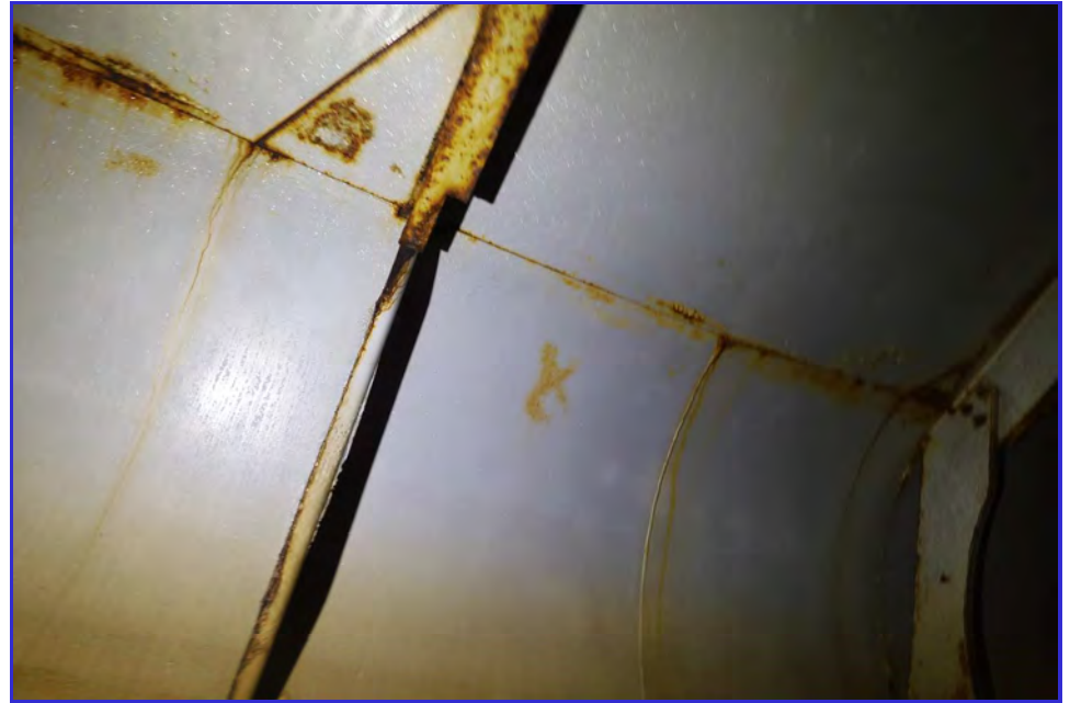
INTERIOR - CPUD - San Andaras Reservoir - Maintenance Inspection -033
