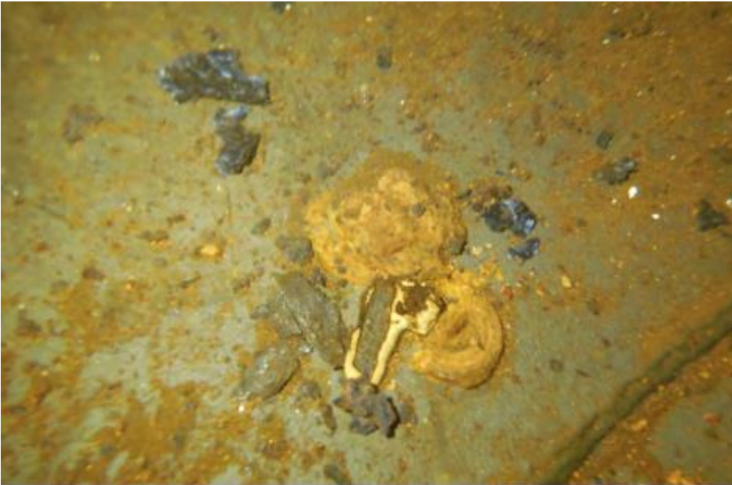
Figure 9-12. Example of Golden Hills Tank Interior Floor
