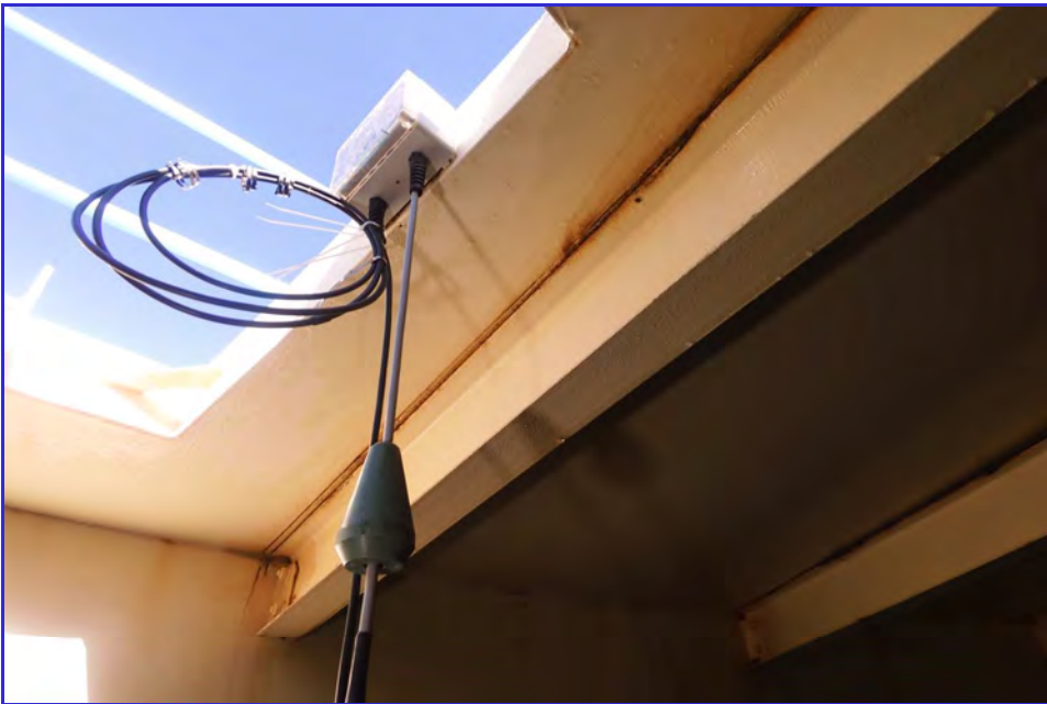
INTERIOR - CPUD - Railroad Flat Reservoir - Maintenance Inspection -002
