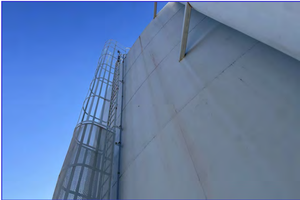
EXTERIOR - CPUD - Mokelumne Reservoir - Maintenance Inspection -138
