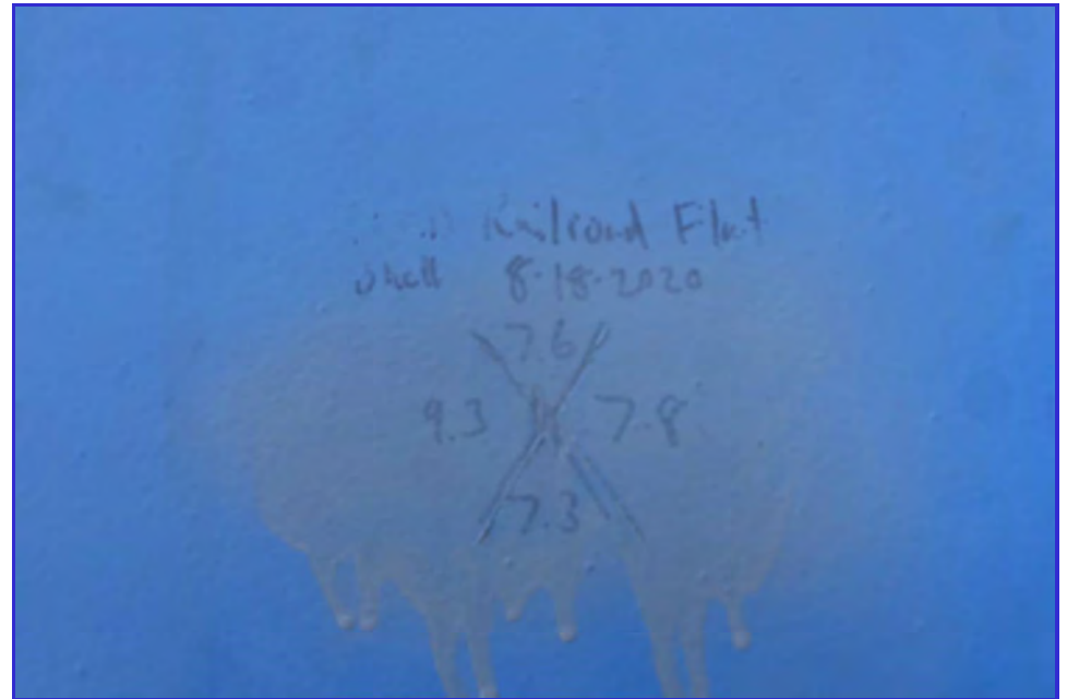
EXTERIOR - CPUD - Railroad Flat Reservoir - Maintenance Inspection -063
