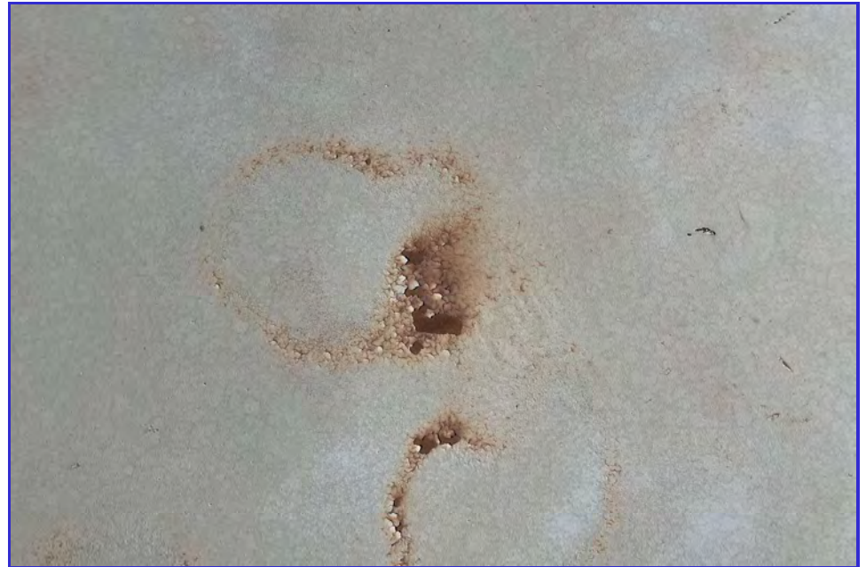
EXTERIOR - CPUD - San Andreas Reservoir - Maintenance Inspection -025
