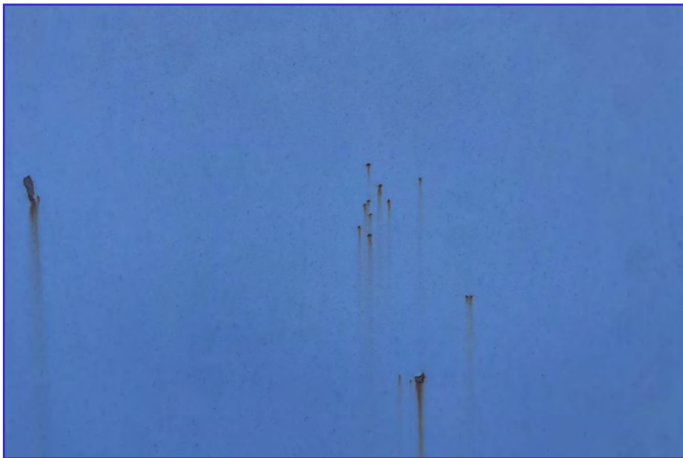
EXTERIOR - CPUD - Mokelumne Reservoir - Maintenance Inspection -122
