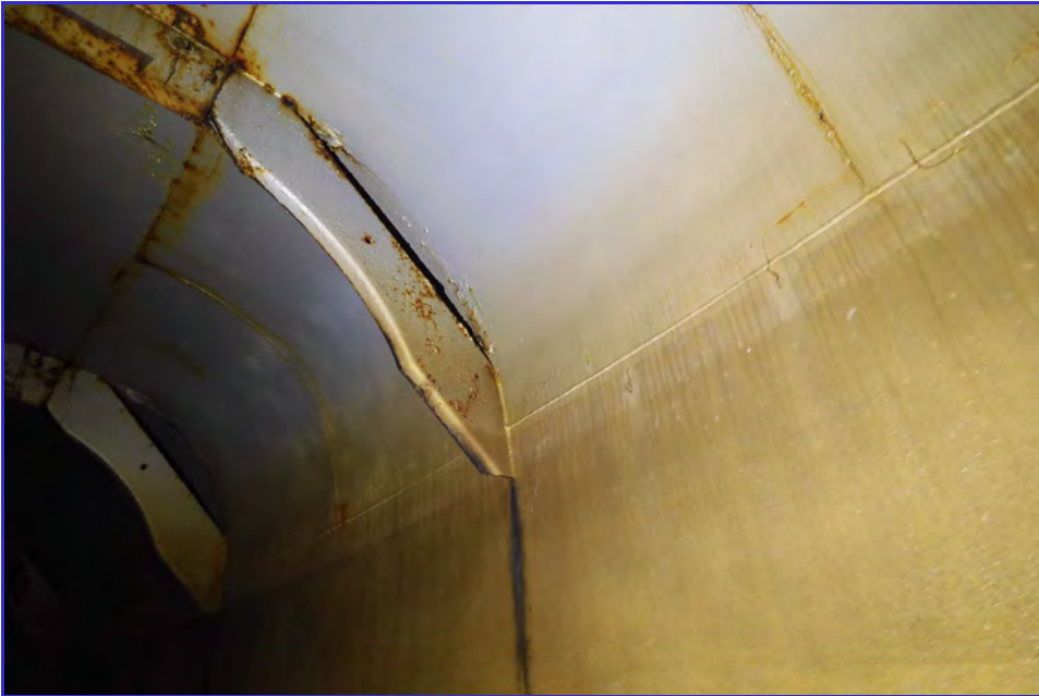
INTERIOR - CPUD - San Andaras Reservoir - Maintenance Inspection -028
