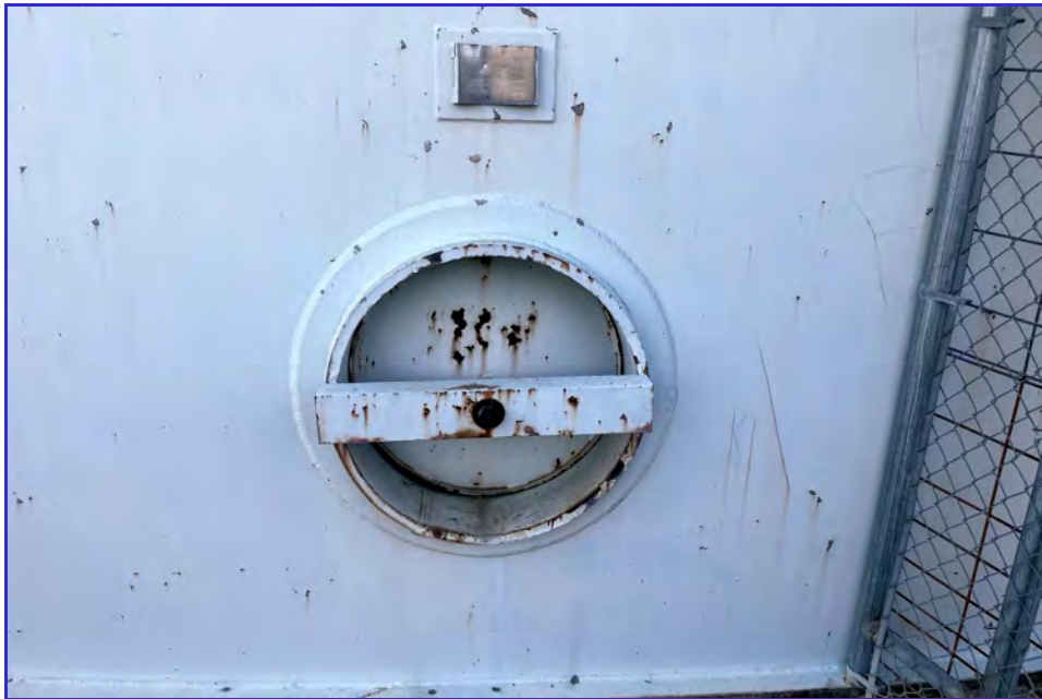
EXTERIOR - CPUD - San Andreas Reservoir - Maintenance Inspection -102
