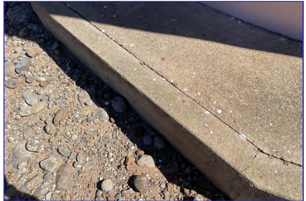
EXTERIOR - CPUD - Paloma Reservoir - Maintenance Inspection -043
