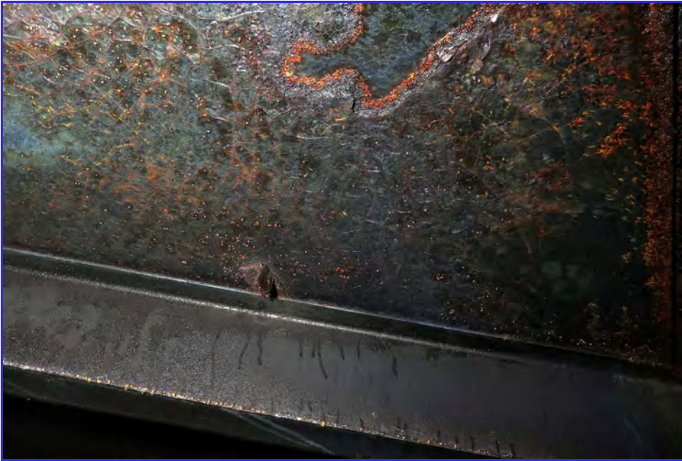
INTERIOR - Calaveras Public Utility District - Clear Well Tank - Maintenance Inspection -040
