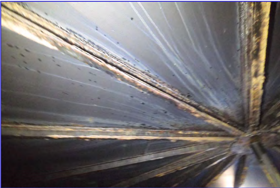
INTERIOR - CPUD - Paloma Reservoir - Maintenance Inspection -026
