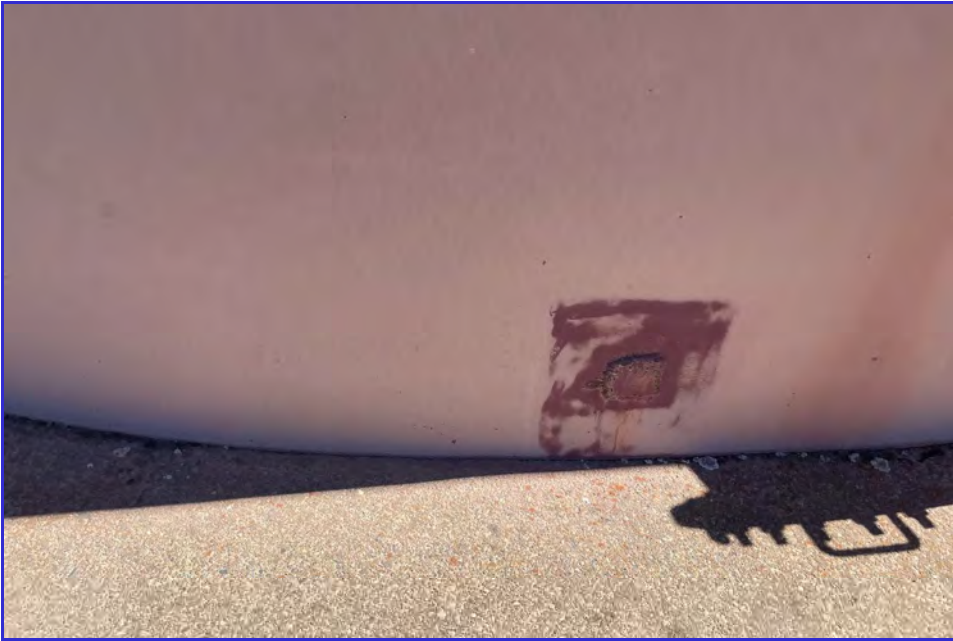
EXTERIOR - CPUD - Paloma Reservoir - Maintenance Inspection -044
