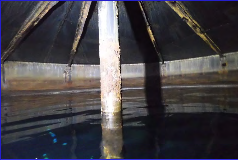
INTERIOR - CPUD - Paloma Reservoir - Maintenance Inspection -032
