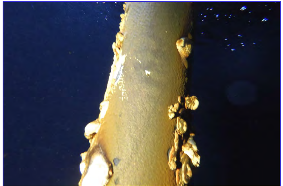
INTERIOR - CPUD - Paloma Reservoir - Maintenance Inspection -115
