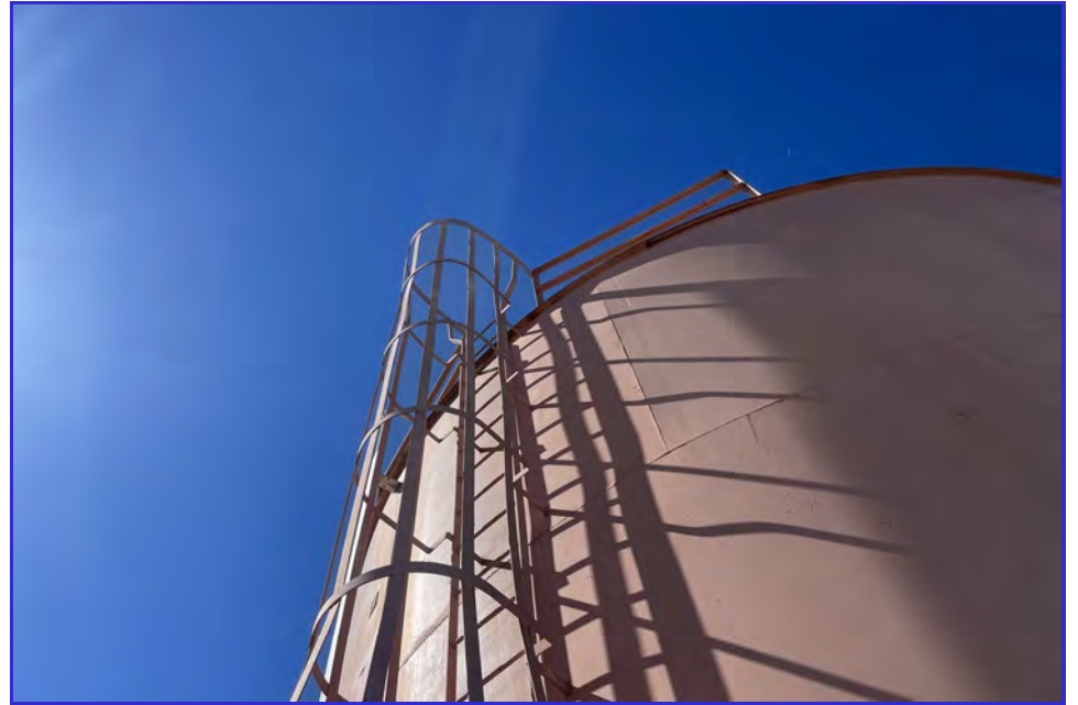
EXTERIOR - CPUD - Paloma Reservoir - Maintenance Inspection -061
