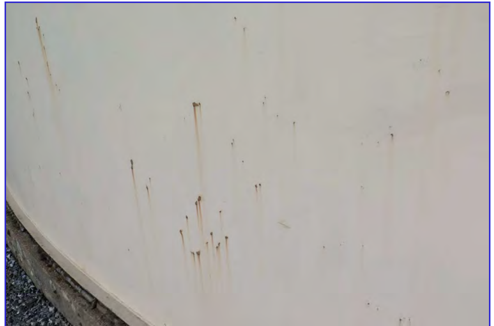
EXTERIOR - Calaveras Public Utility District - Clear Well Tank - Maintenance Inspection -059
