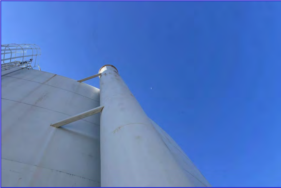
EXTERIOR - CPUD - Mokelumne Reservoir - Maintenance Inspection -140
