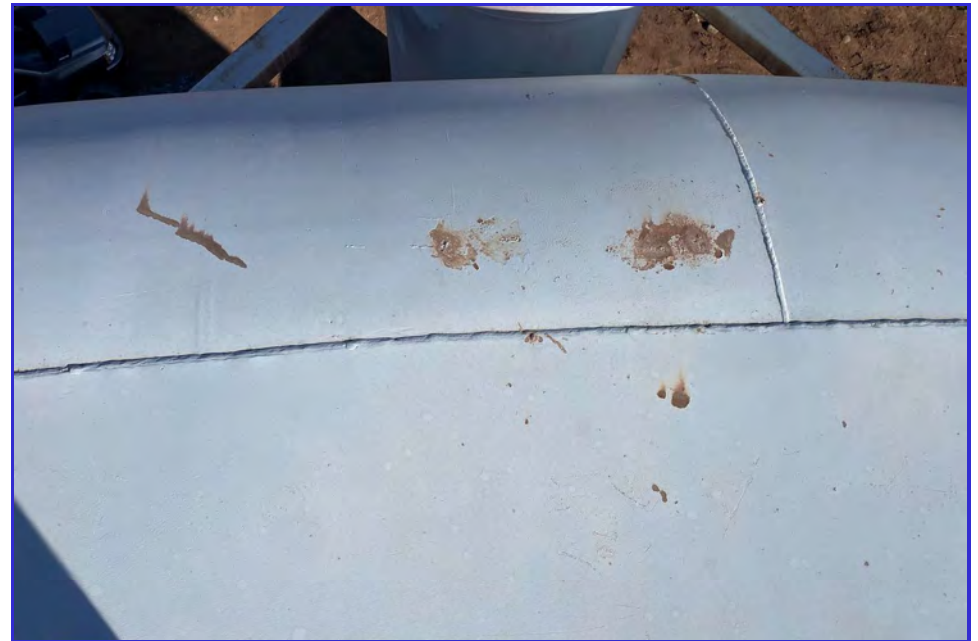
EXTERIOR - CPUD - Mokelumne Reservoir - Maintenance Inspection -075
