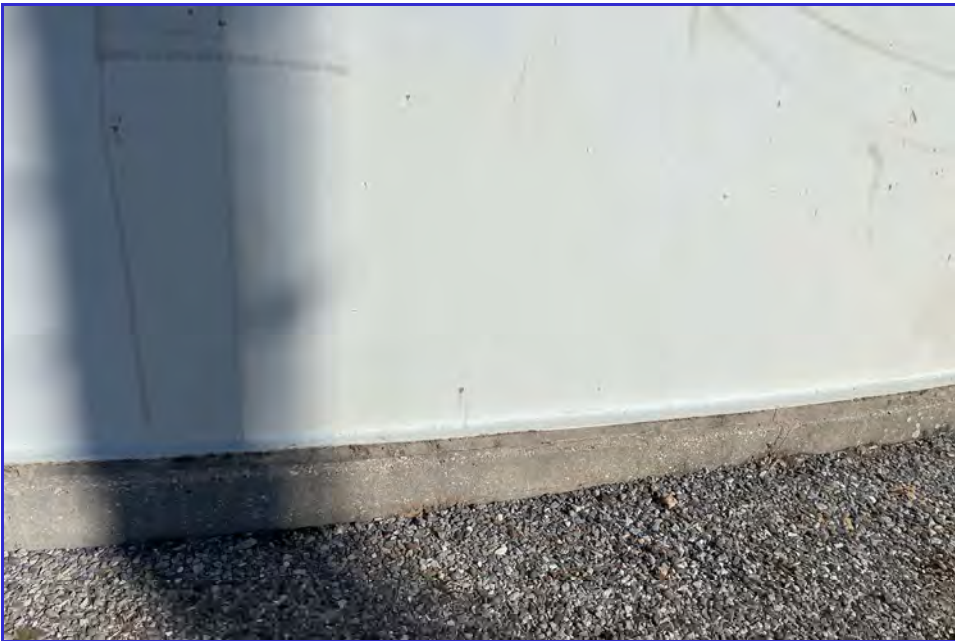
EXTERIOR - CPUD - San Andreas Reservoir - Maintenance Inspection -146
