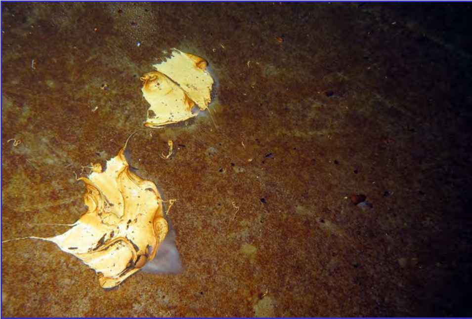
INTERIOR - Calaveras Public Utility District - Clear Well Tank - Maintenance Inspection -128
