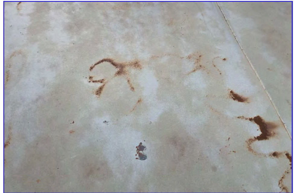
EXTERIOR - CPUD - San Andreas Reservoir - Maintenance Inspection -023
