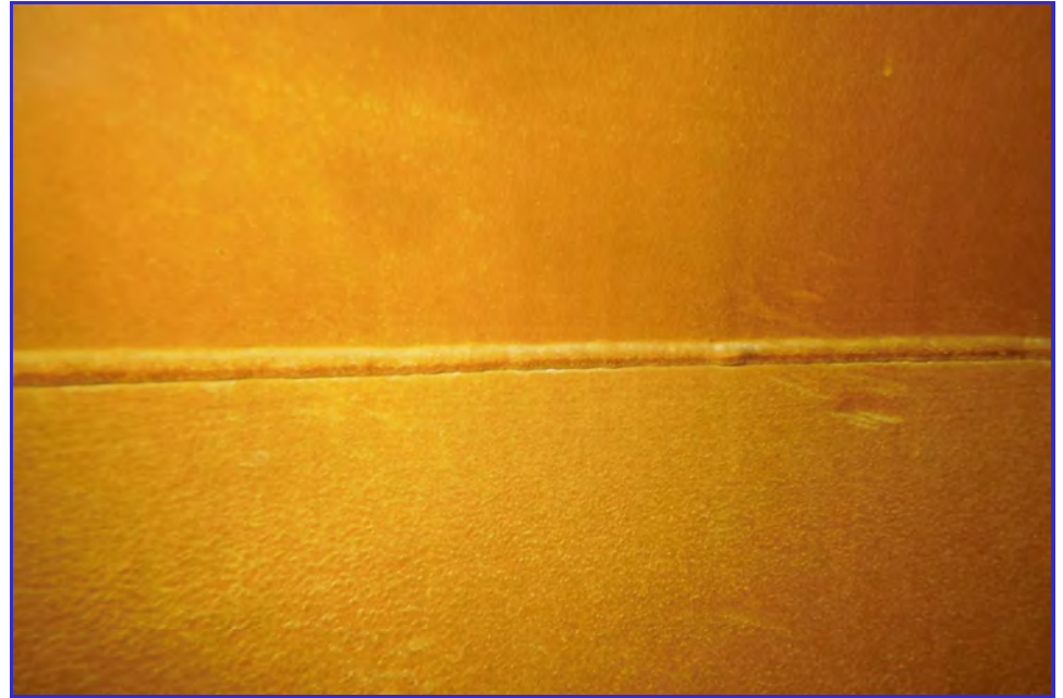
INTERIOR - CPUD - Railroad Flat Reservoir - Maintenance Inspection -101
