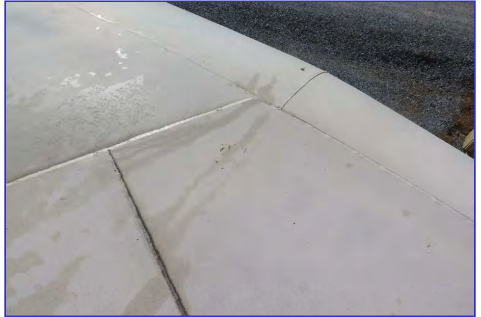
EXTERIOR - Calaveras Public Utility District - Clear Well Tank - Maintenance Inspection -033
