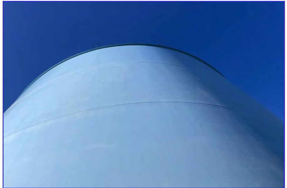
EXTERIOR - CPUD - Railroad Flat Reservoir - Maintenance Inspection -091
