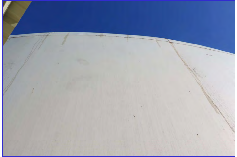
EXTERIOR - Calaveras Public Utility District - Clear Well Tank - Maintenance Inspection -077
