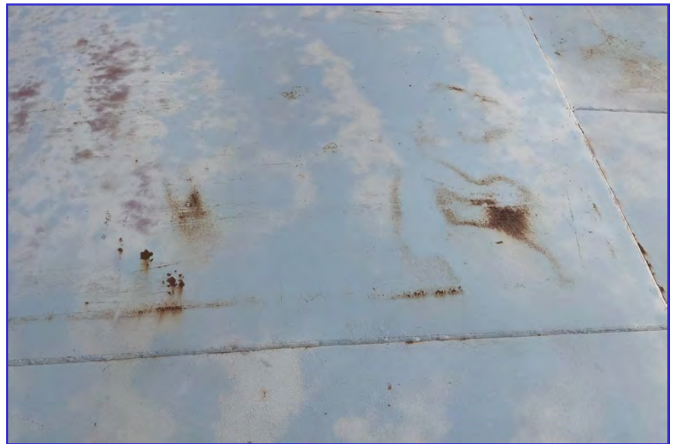
EXTERIOR - CPUD - Mokelumne Reservoir - Maintenance Inspection -043
