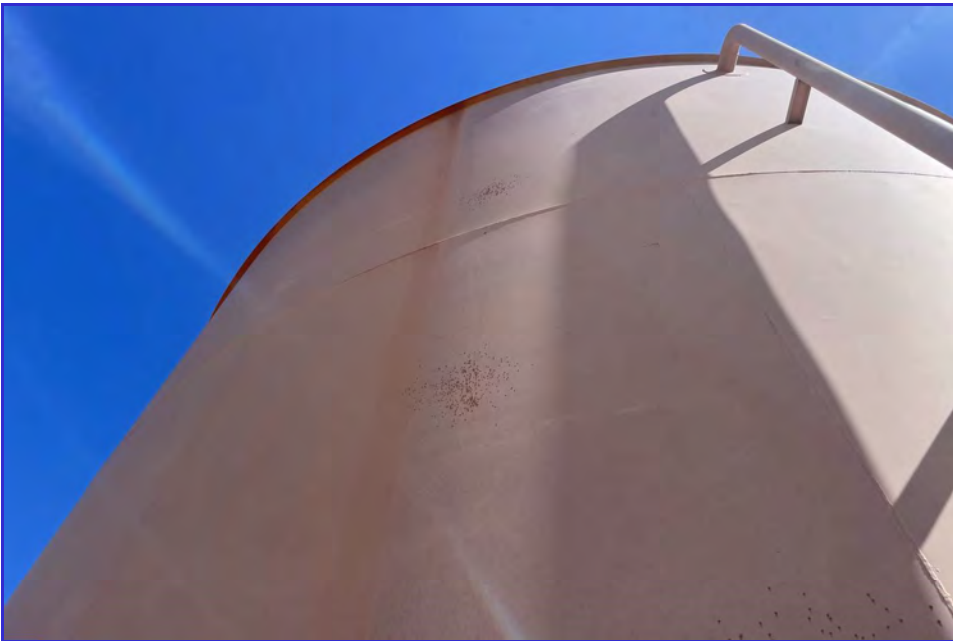
EXTERIOR - CPUD - Paloma Reservoir - Maintenance Inspection -046
