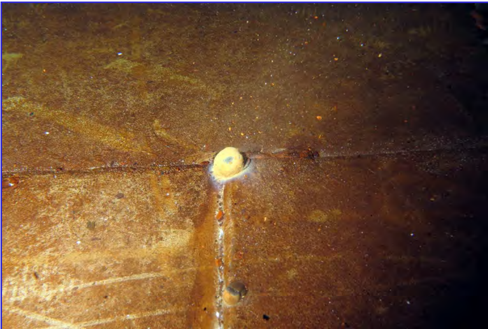
INTERIOR - Calaveras Public Utility District - Clear Well Tank - Maintenance Inspection -138
