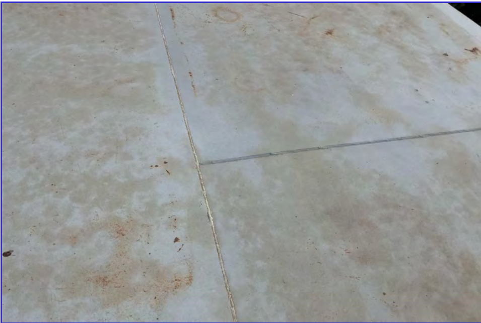
EXTERIOR - CPUD - San Andreas Reservoir - Maintenance Inspection -054
