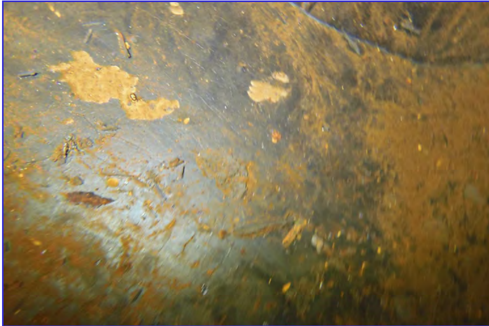
INTERIOR - CPUD - Paloma Reservoir - Maintenance Inspection -120
