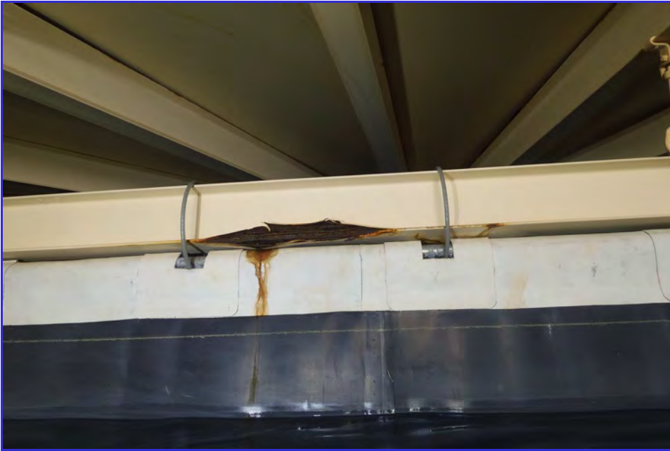
INTERIOR - CPUD - Railroad Flat Reservoir - Maintenance Inspection -008
