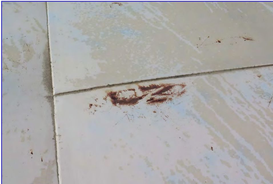
EXTERIOR - Calaveras Public Utility District - Clear Well Tank - Maintenance Inspection -042
