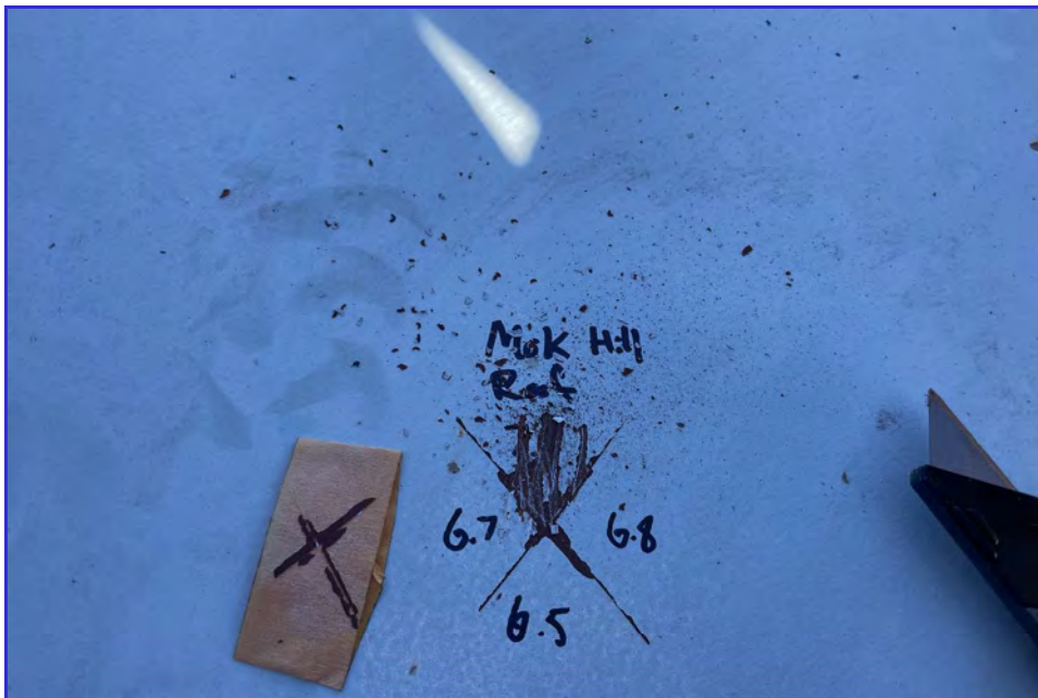
EXTERIOR - CPUD - Mokelumne Reservoir - Maintenance Inspection -078
