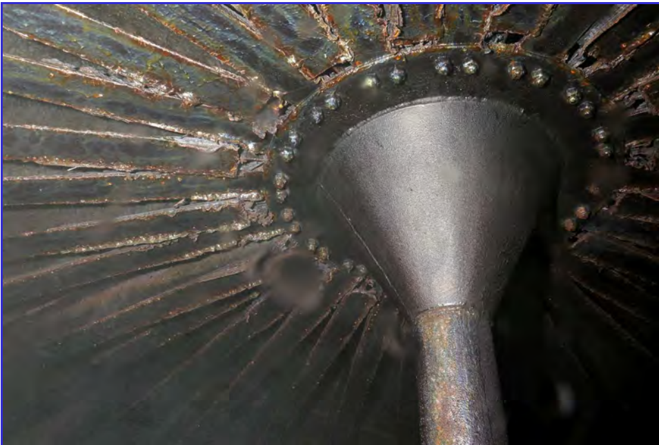
INTERIOR - Calaveras Public Utility District - Clear Well Tank - Maintenance Inspection -018
