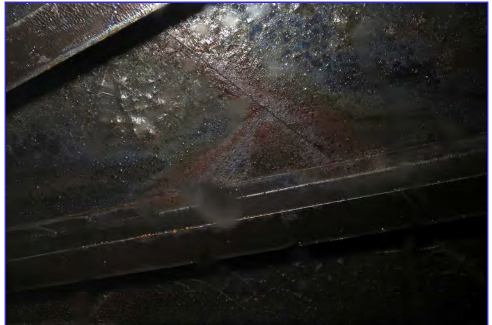
INTERIOR - Calaveras Public Utility District - Clear Well Tank - Maintenance Inspection -011
