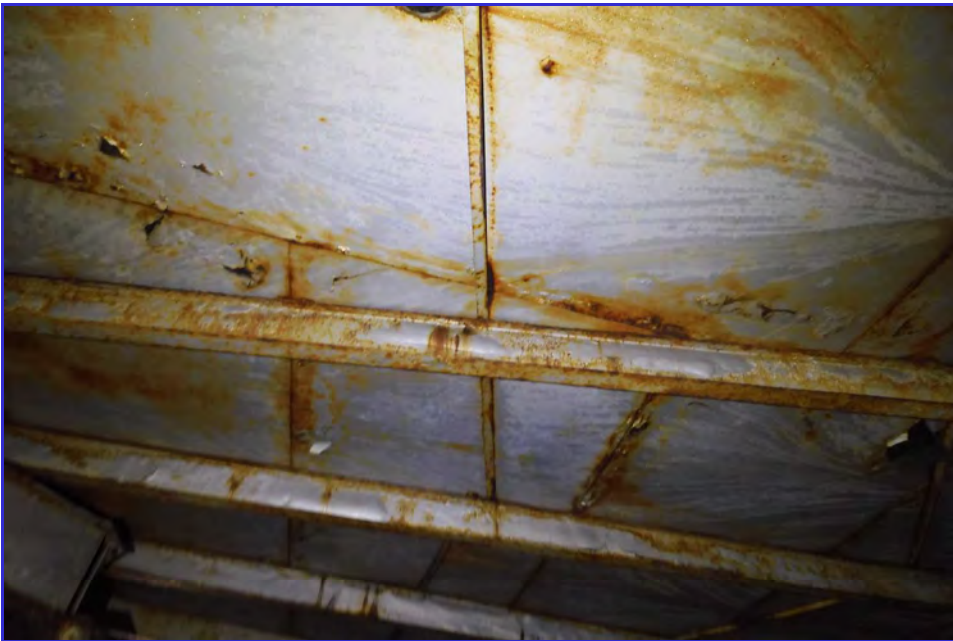
INTERIOR - CPUD - San Andaras Reservoir - Maintenance Inspection -094
