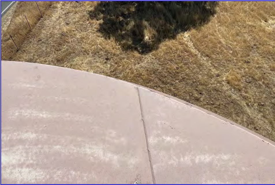
EXTERIOR - CPUD - Paloma Reservoir - Maintenance Inspection -024
