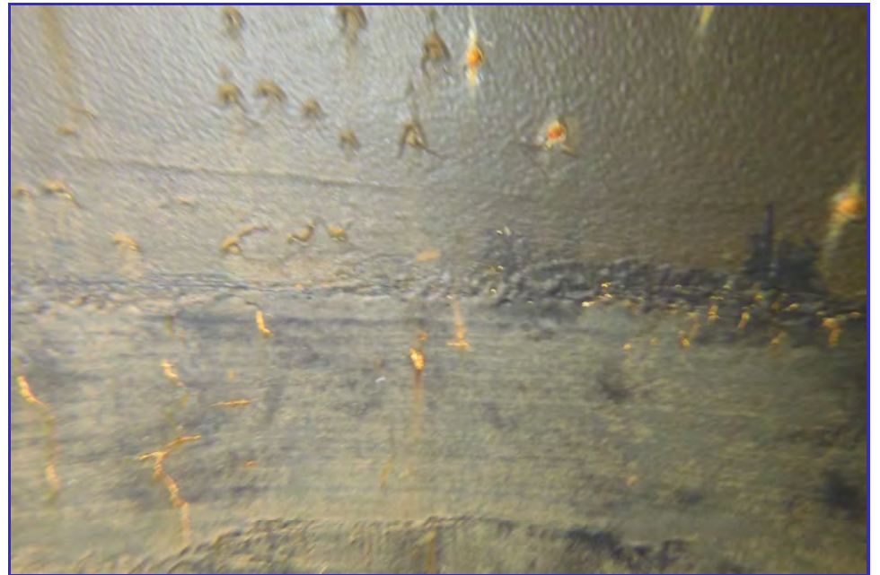
INTERIOR - CPUD - Paloma Reservoir - Maintenance Inspection -059
