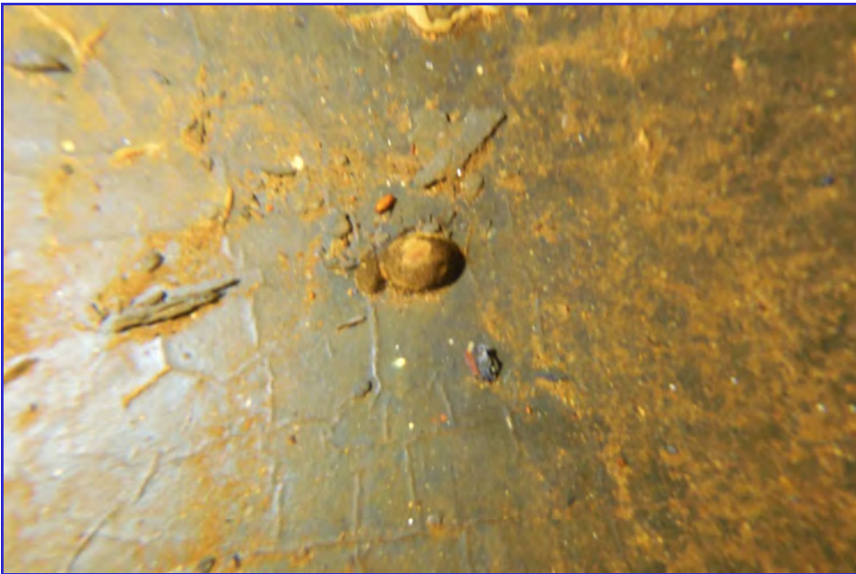
INTERIOR - CPUD - Paloma Reservoir - Maintenance Inspection -146
