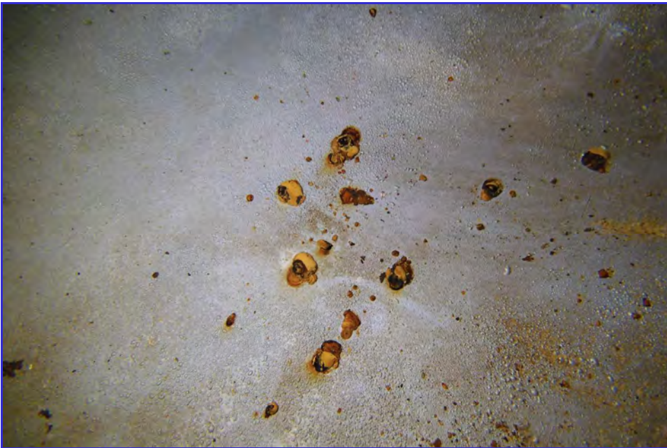
INTERIOR - CPUD - San Andaras Reservoir - Maintenance Inspection -162
