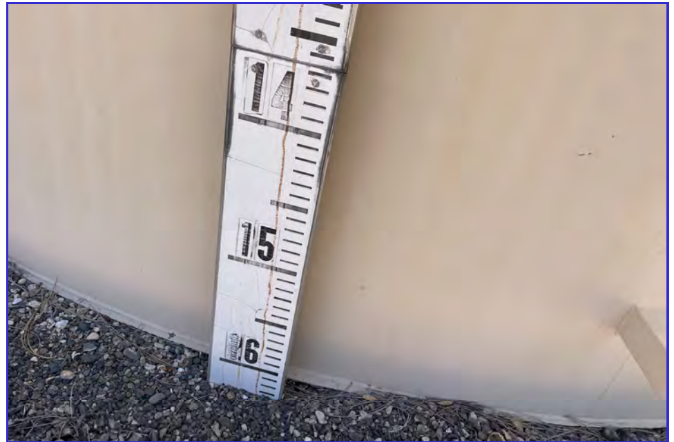
EXTERIOR - CPUD - Golden Hills - Maintenance Inspection -039
