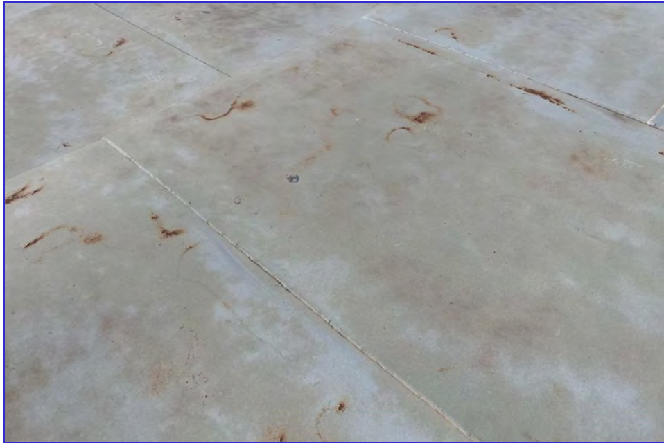
EXTERIOR - CPUD - San Andreas Reservoir - Maintenance Inspection -024
