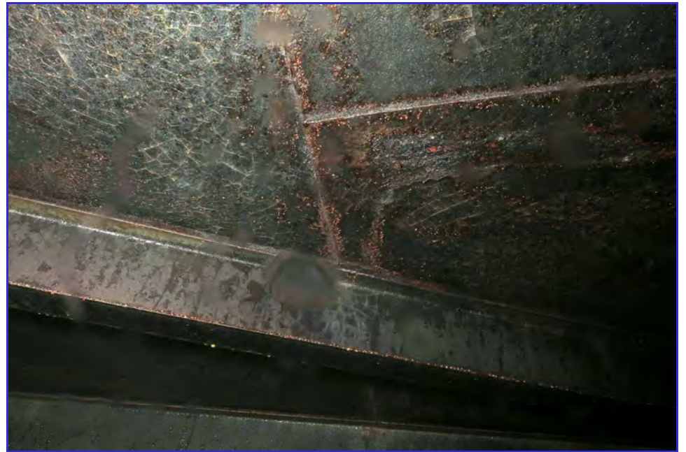
INTERIOR - Calaveras Public Utility District - Clear Well Tank - Maintenance Inspection -027
