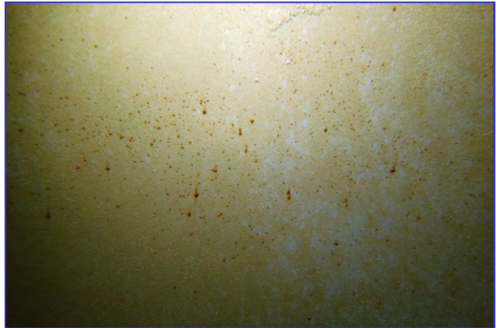
INTERIOR - CPUD - Mokelumne Hill Reservoir - Maintenance Inspection -079
