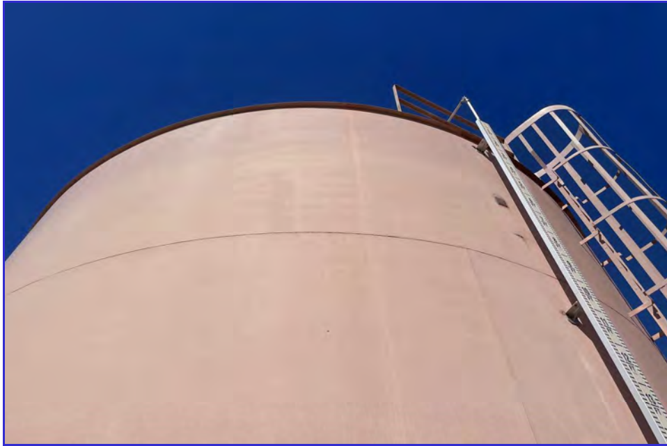
EXTERIOR - CPUD - Paloma Reservoir - Maintenance Inspection -072
