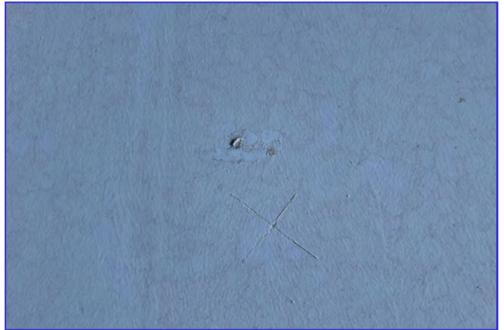
EXTERIOR - CPUD - Railroad Flat Reservoir - Maintenance Inspection -043
