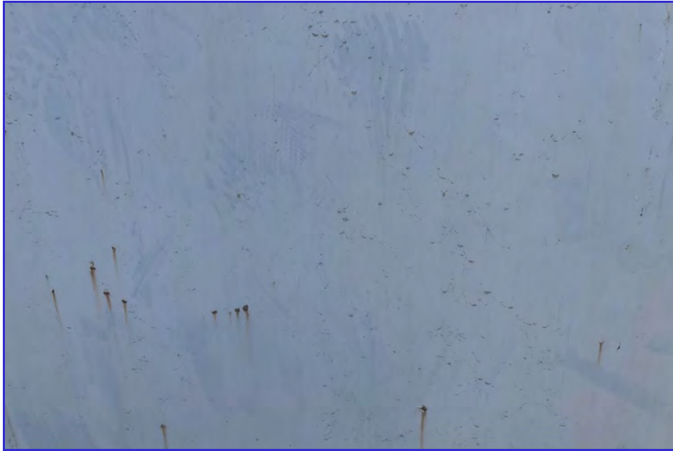
EXTERIOR - CPUD - Mokelumne Reservoir - Maintenance Inspection -132
