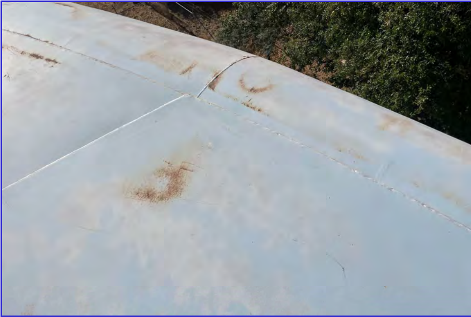
EXTERIOR - CPUD - Mokelumne Reservoir - Maintenance Inspection -064
