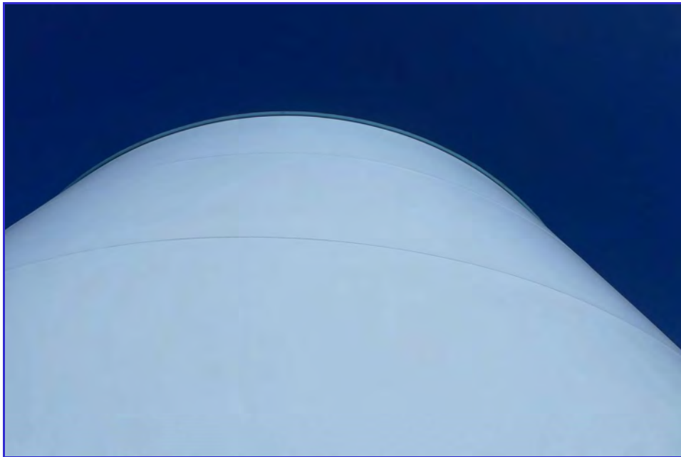
EXTERIOR - CPUD - Railroad Flat Reservoir - Maintenance Inspection -054
