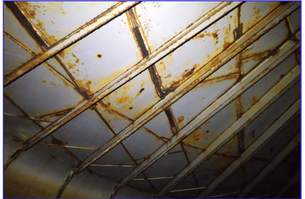
INTERIOR - CPUD - Mokelumne Hill Reservoir - Maintenance Inspection -045
