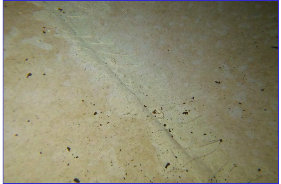
INTERIOR - CPUD - Railroad Flat Reservoir - Maintenance Inspection -149
