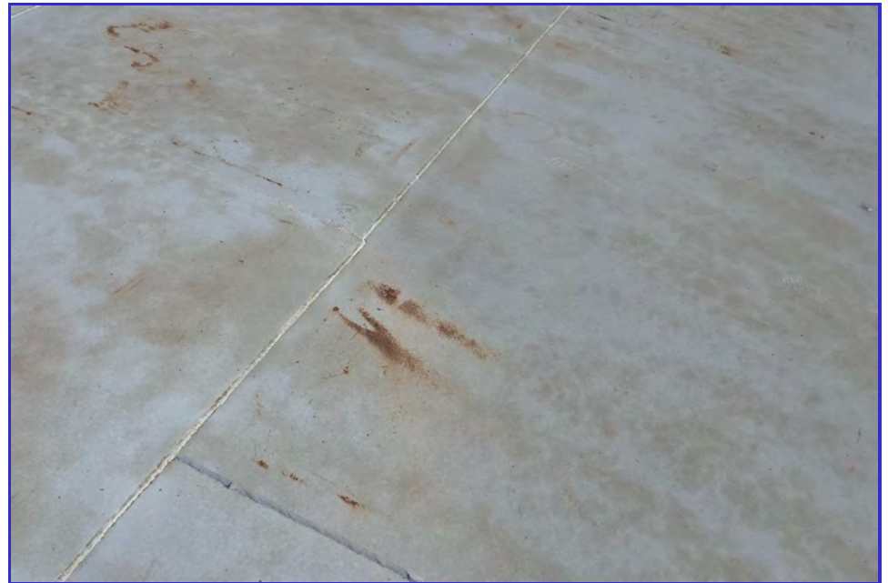
EXTERIOR - CPUD - San Andreas Reservoir - Maintenance Inspection -047
