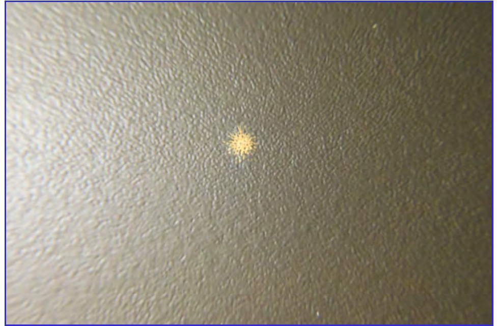
INTERIOR - CPUD - Paloma Reservoir - Maintenance Inspection -061
