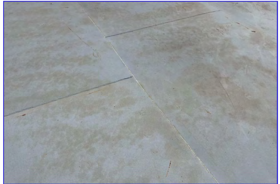
EXTERIOR - CPUD - San Andreas Reservoir - Maintenance Inspection -035
