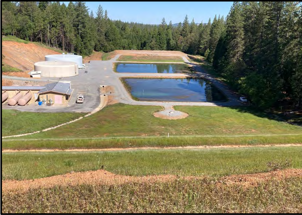
CPUD Water Treatment Plant, looking northwest from the Jeff Davis Reservoir Dam; 05/15/24.
