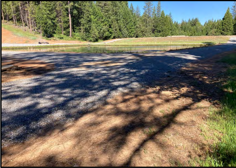
Gravel roads along the edge of the backwash ponds where the backwash recycle pump station will be constructed, looking west; 05/15/24.
