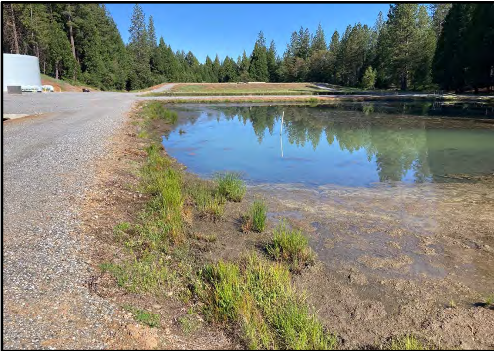
East backwash pond, looking northwest; 05/15/24.
