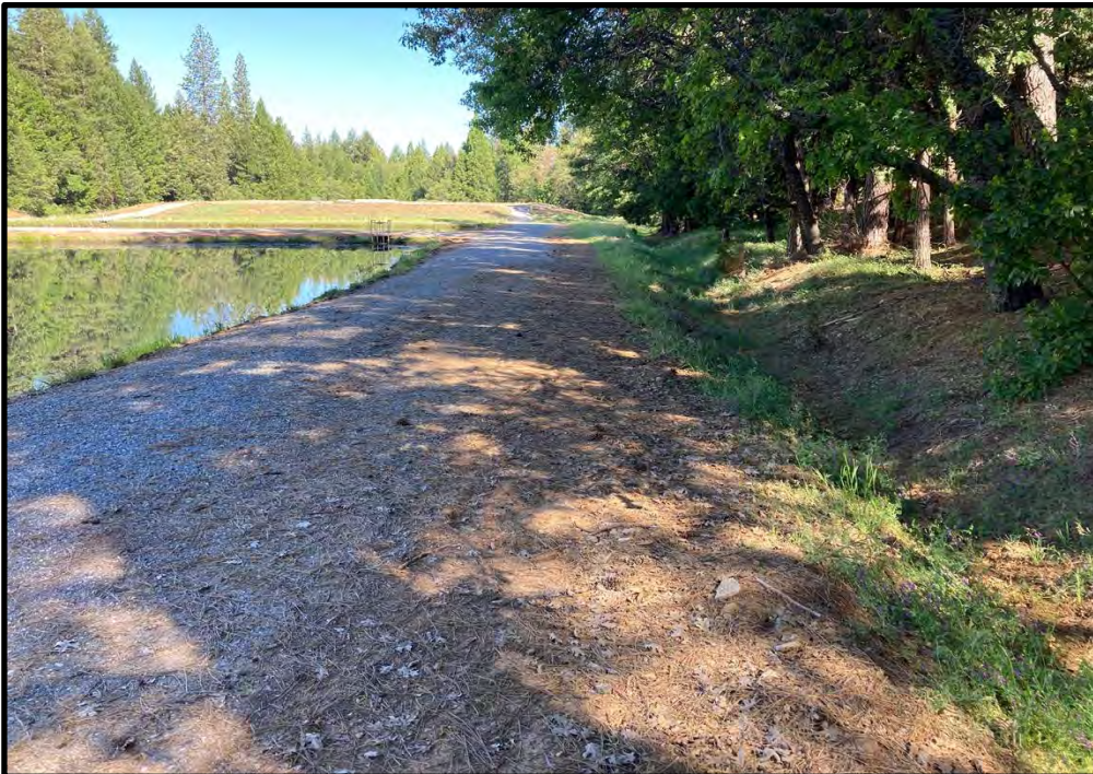
Gravel road along the edge of the east backwash pond, looking northwest; 05/15/24. The first part of the pipeline from the backwash recycle pump station to the reservoir will be trenched in this road.
