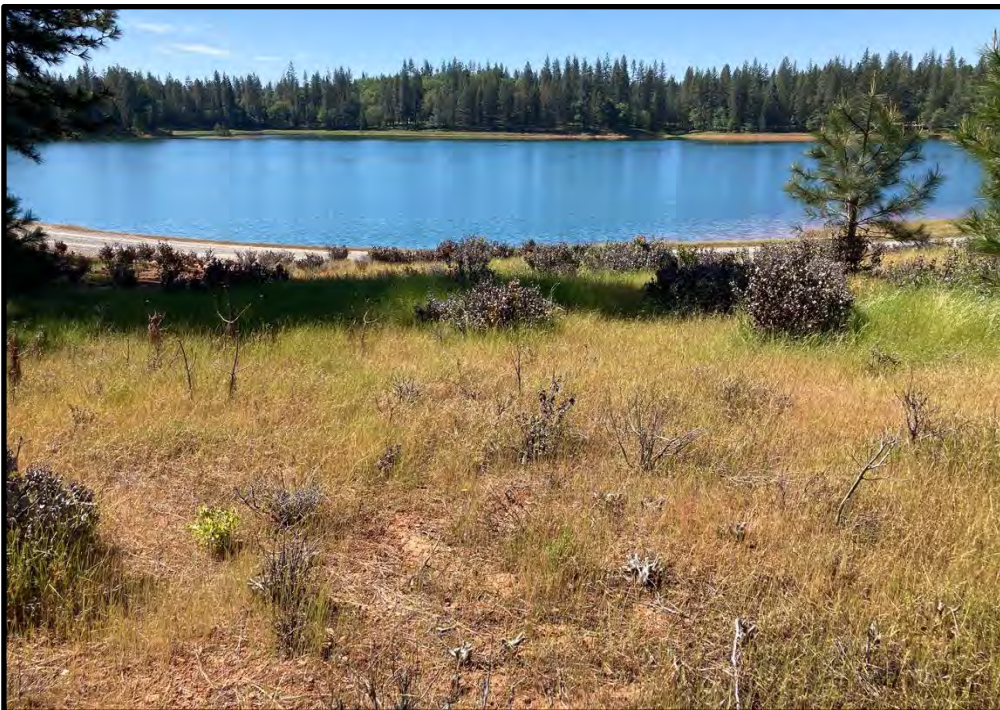
Pipeline alignment transitioning down to the reservoir, looking south from the sharp turn in the pipeline; 05/15/24.
