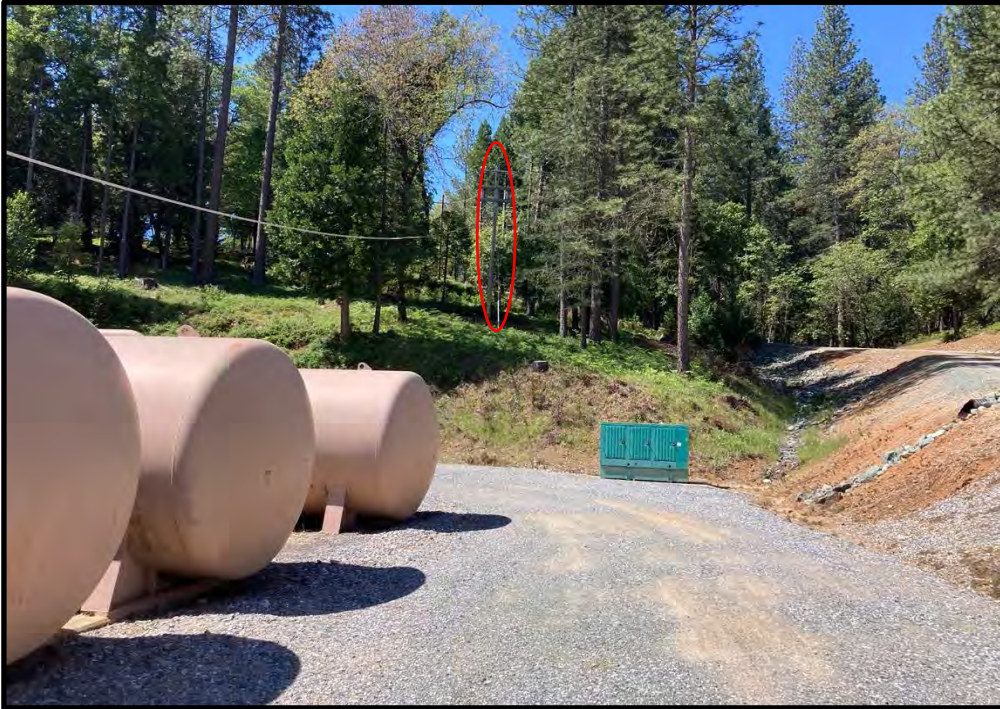
Gravel road and hillside adjacent to the water treatment plant, looking southwest; 05/15/24. New electrical conduit will be trenched between the PG&E service pole (noted) to the water treatment plant.
